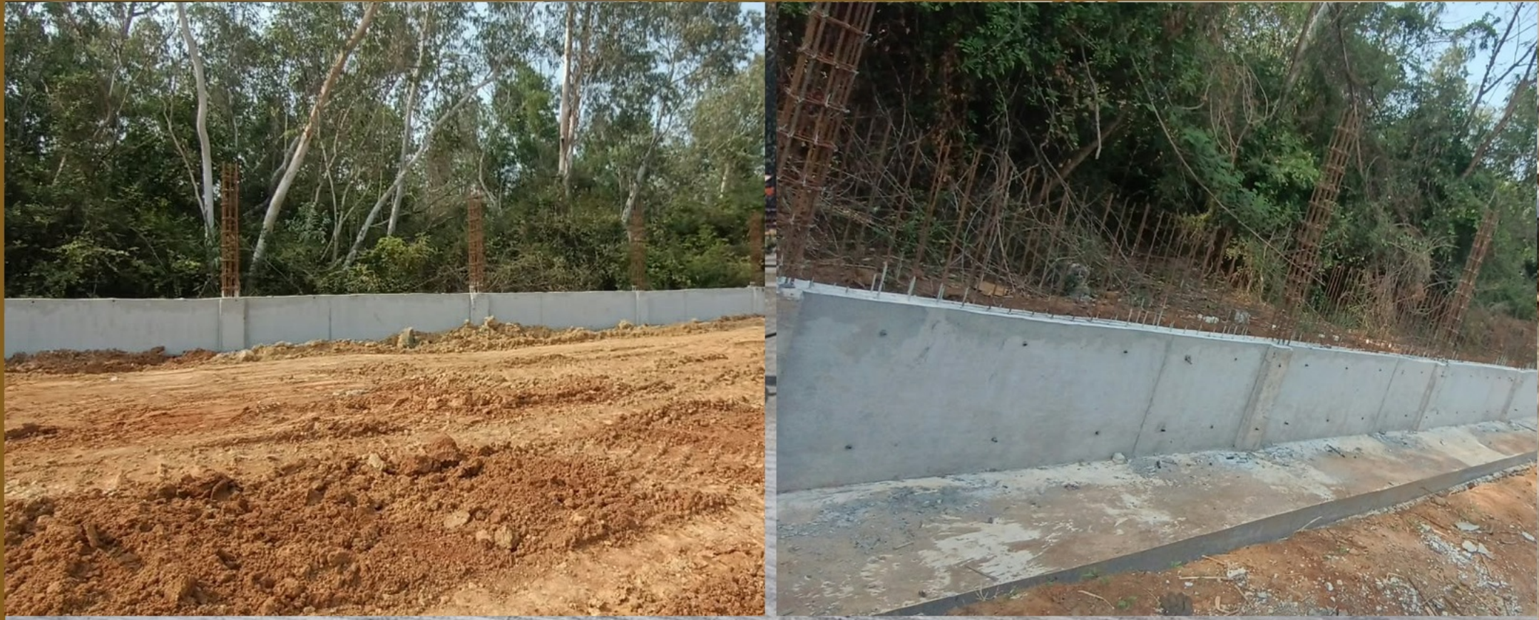
Compound Wall Work - Forest Side
