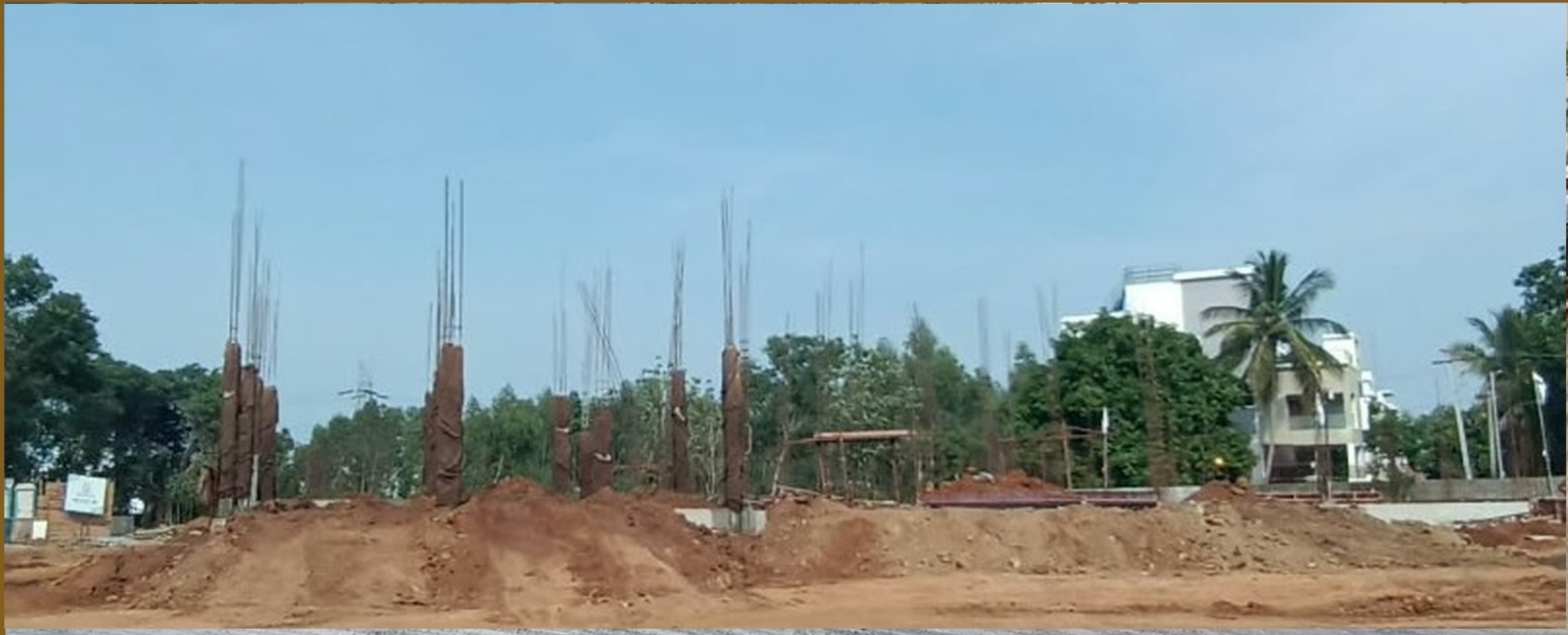
G.F Column & Plinth Beam Work
