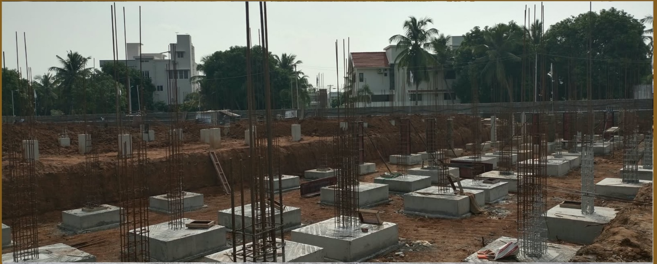
Footing & Column Work
