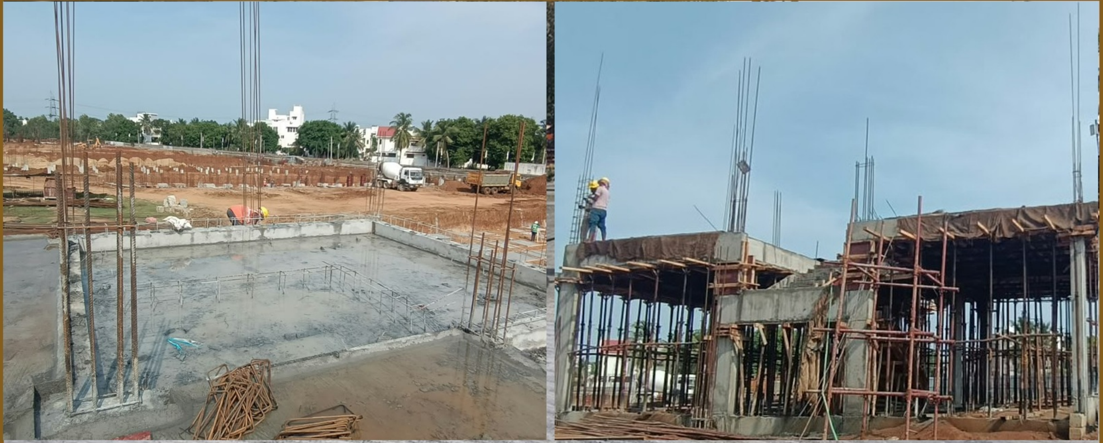
Ground Floor Roof Slab Work
