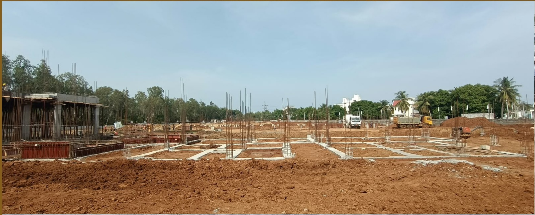
Plinth Beam Work
