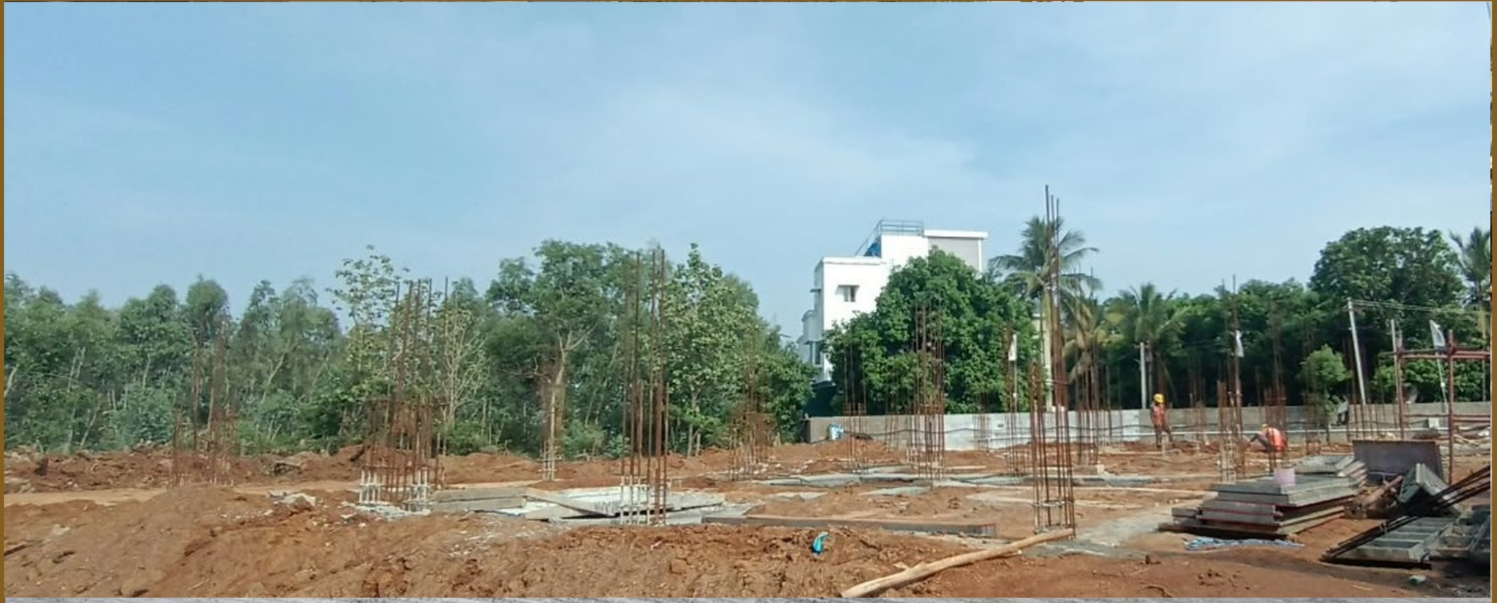
Plinth Beam Work
