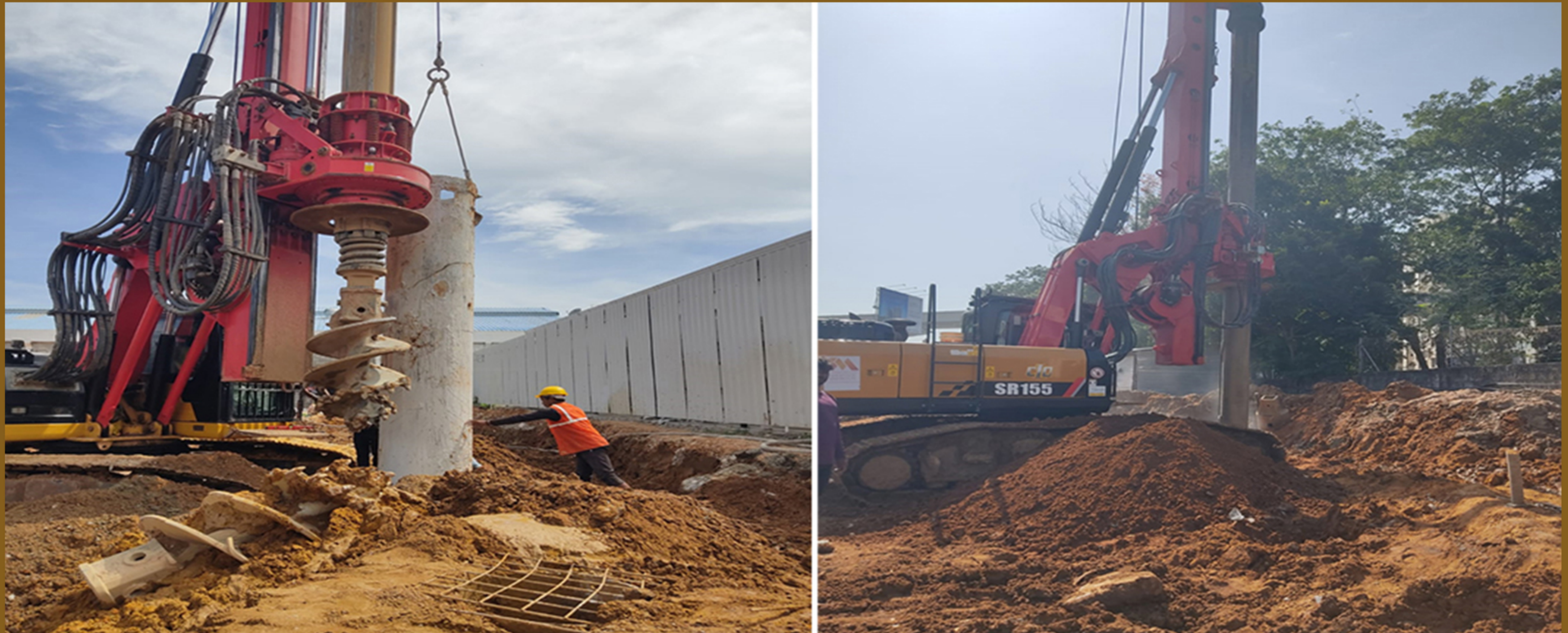
BLOCK B PILE BORING WORKS
