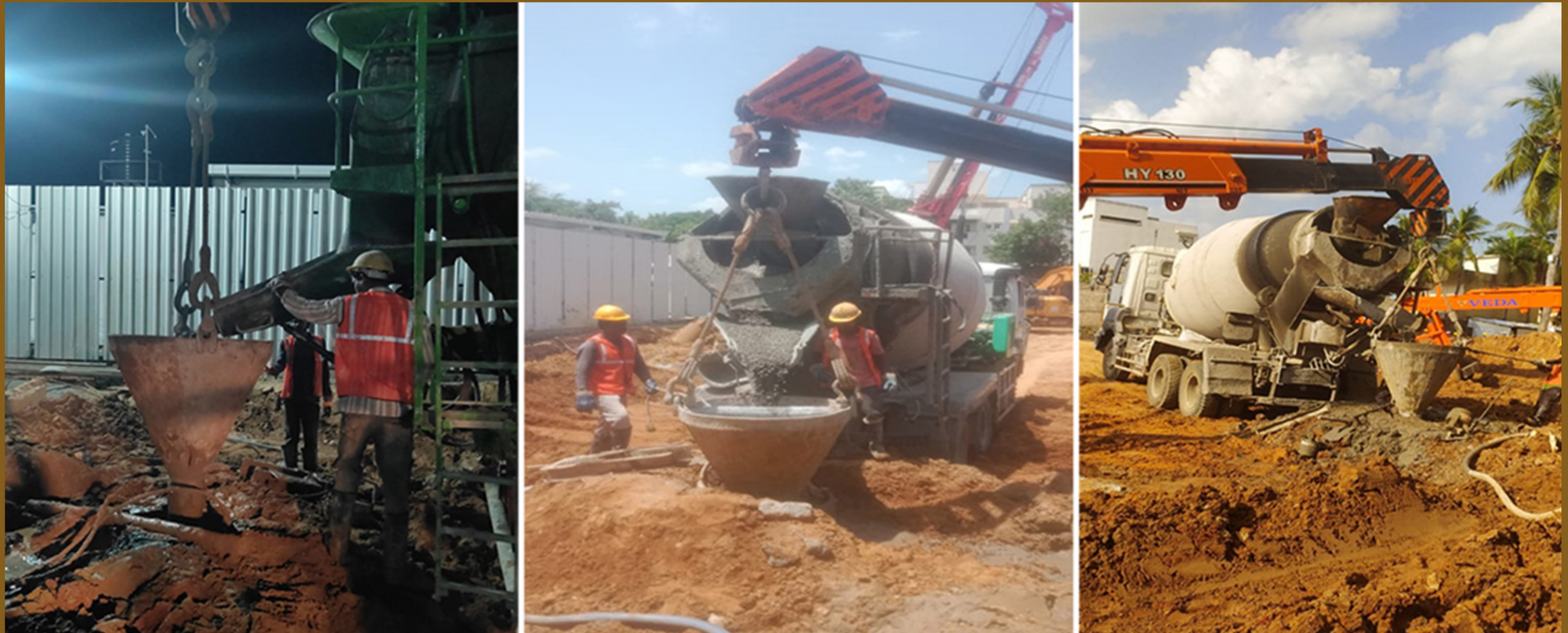
BLOCK B PILE CONCRETE WORKS
