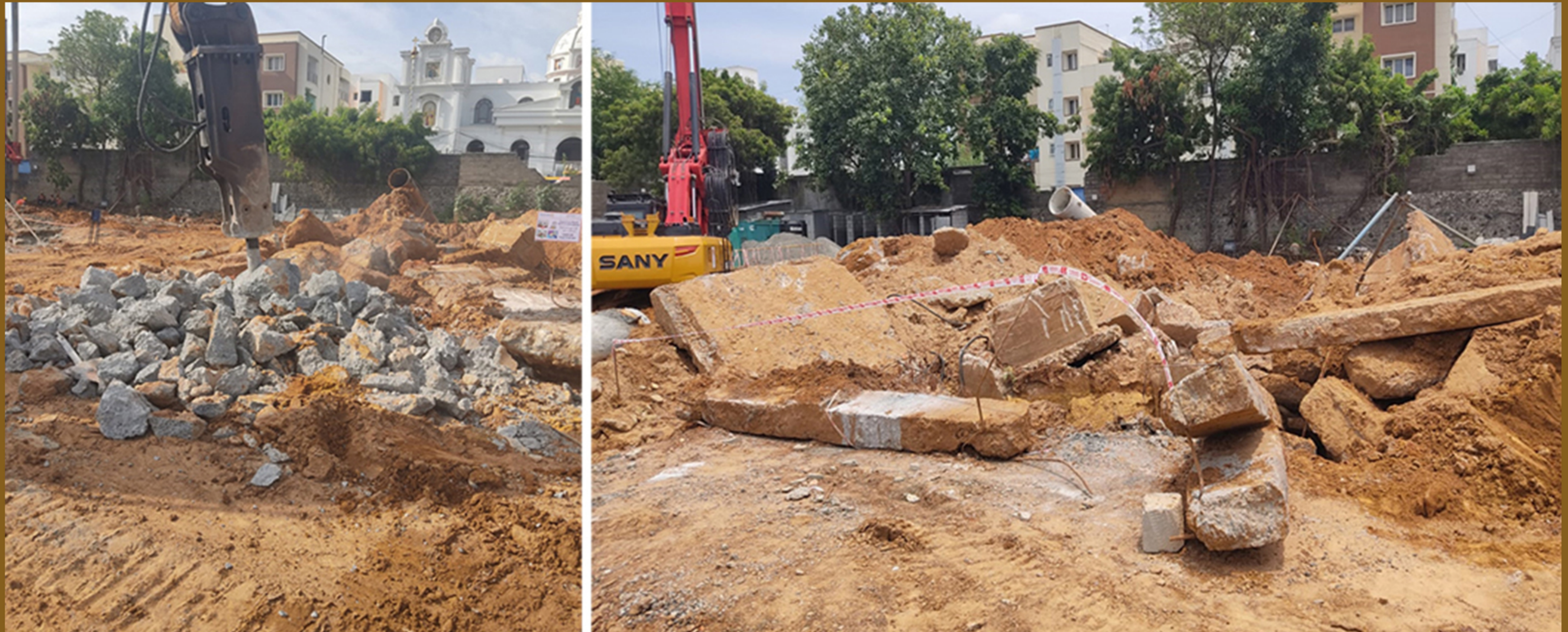
BLOCK B EXISTING BUILDING CONCRETE DISMANTLE
