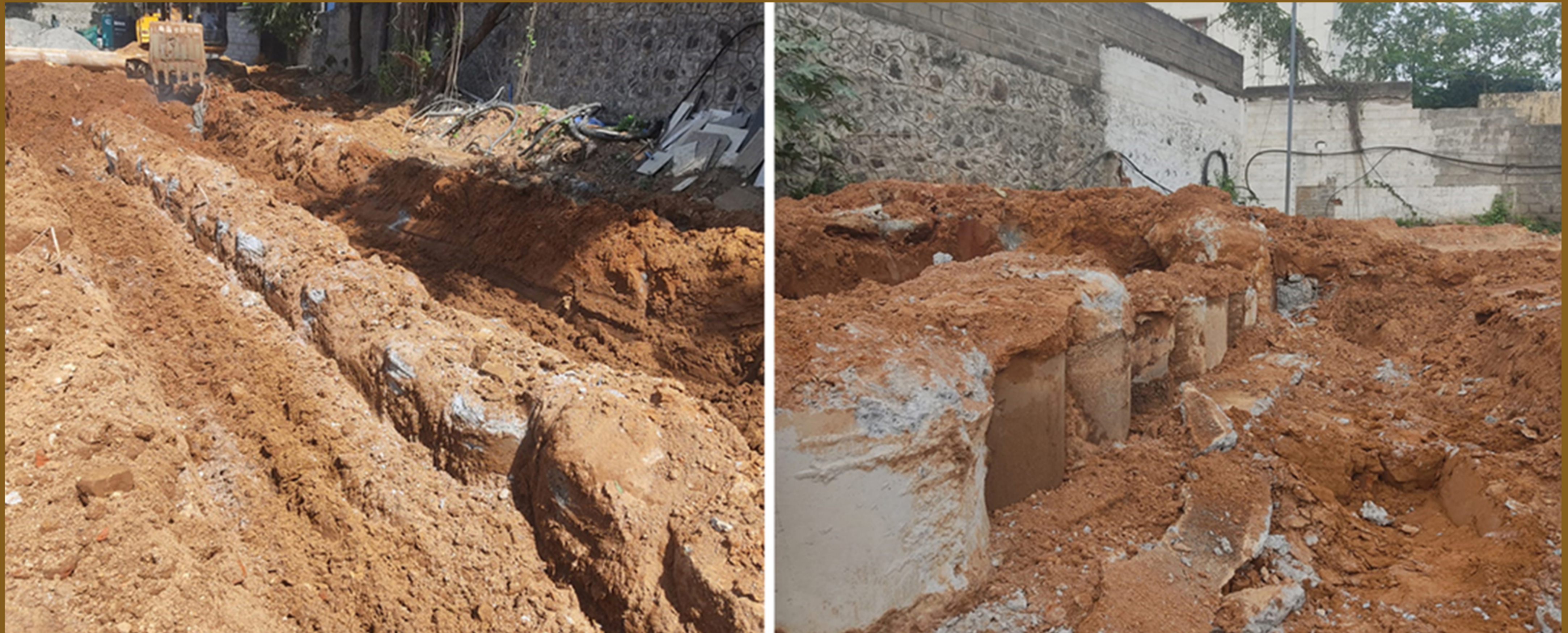
BLOCK B GUIDE BEAM REMOVAL
