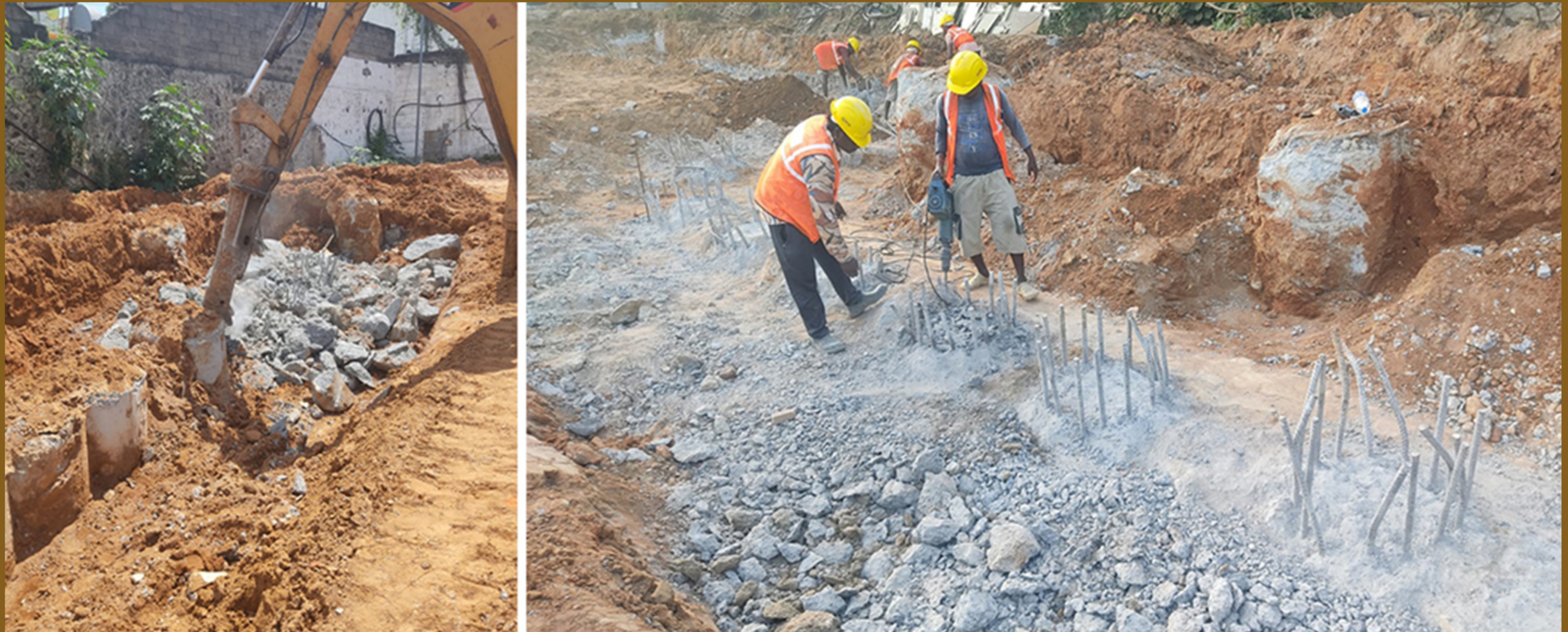
BLOCK B PILE CONCRETE DISMANTLING
