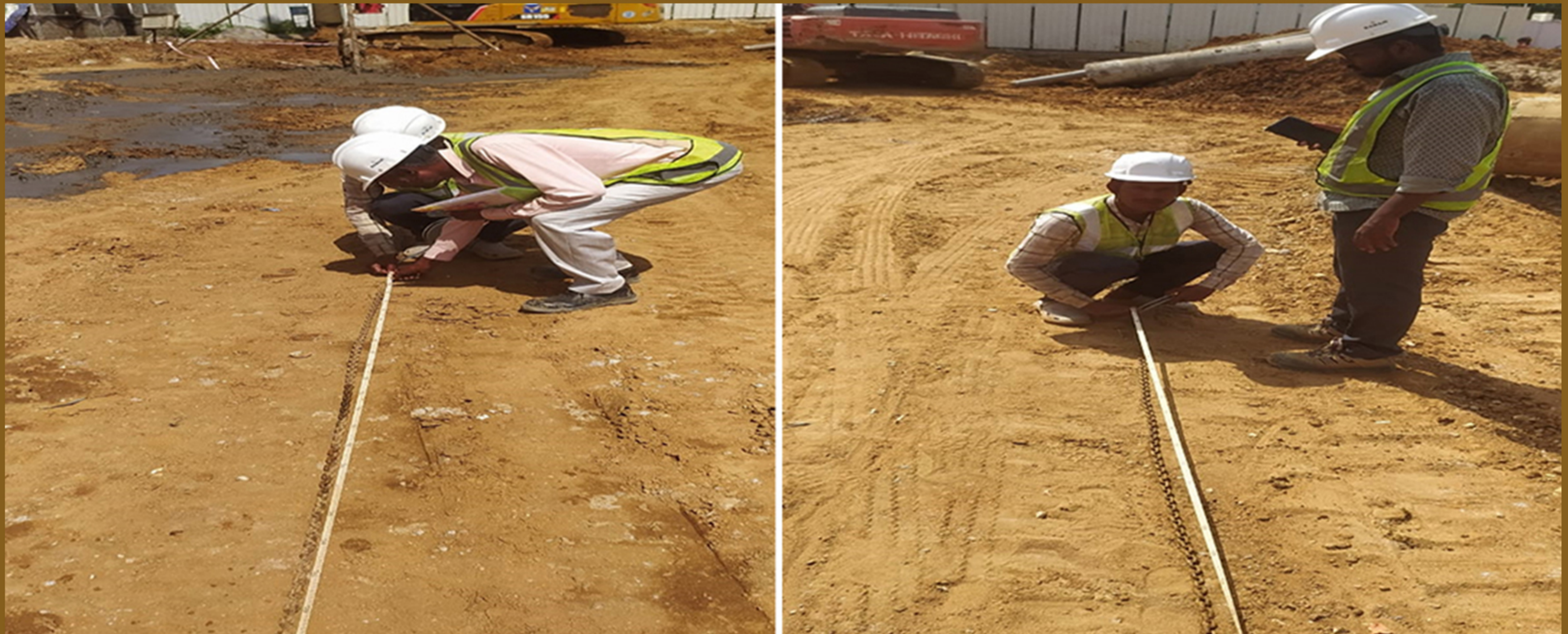
BLOCK B PILE DEPTH CHECKING WORKS
