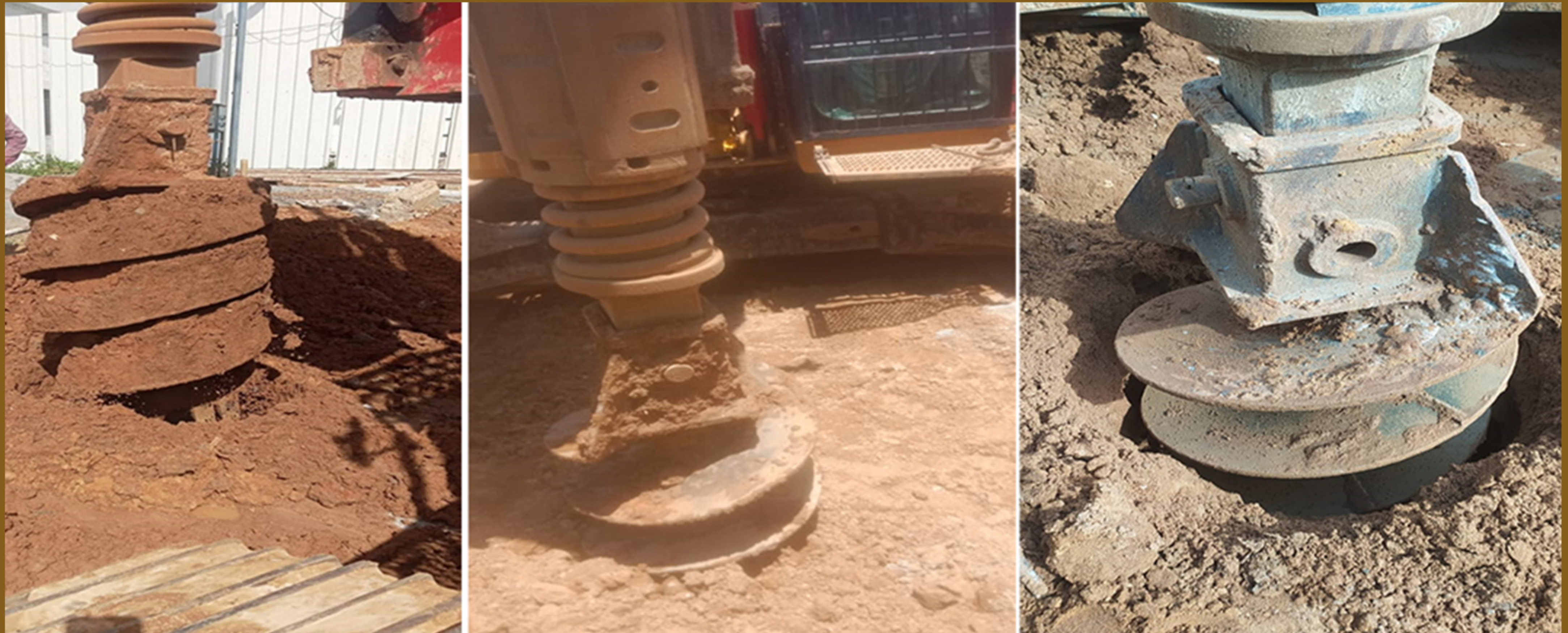
BLOCK B PILE BORING WORKS
