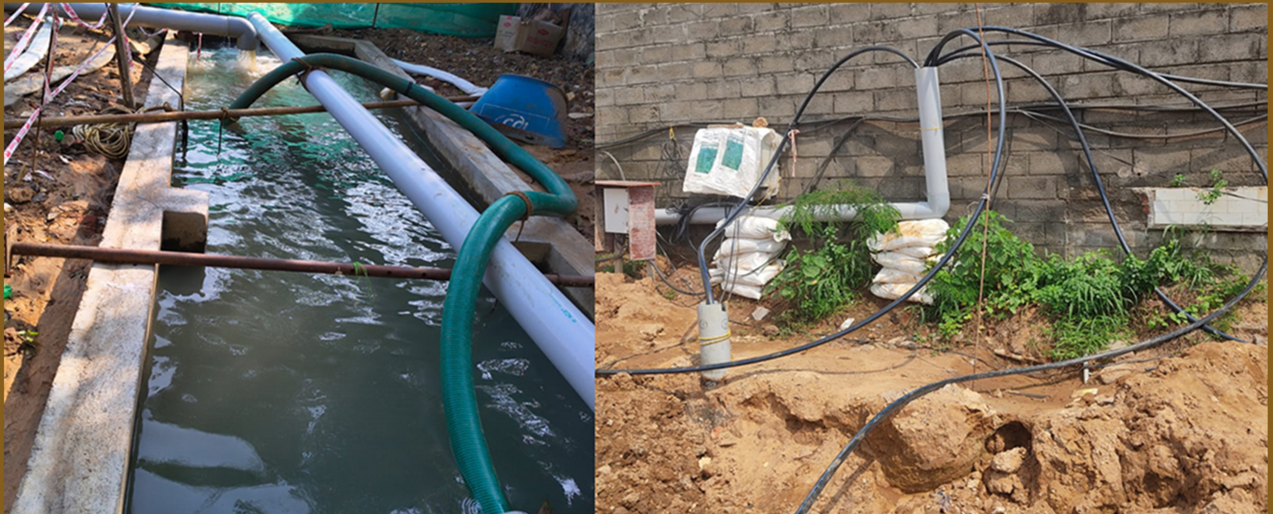
BLOCK B DEWATERING WORK
