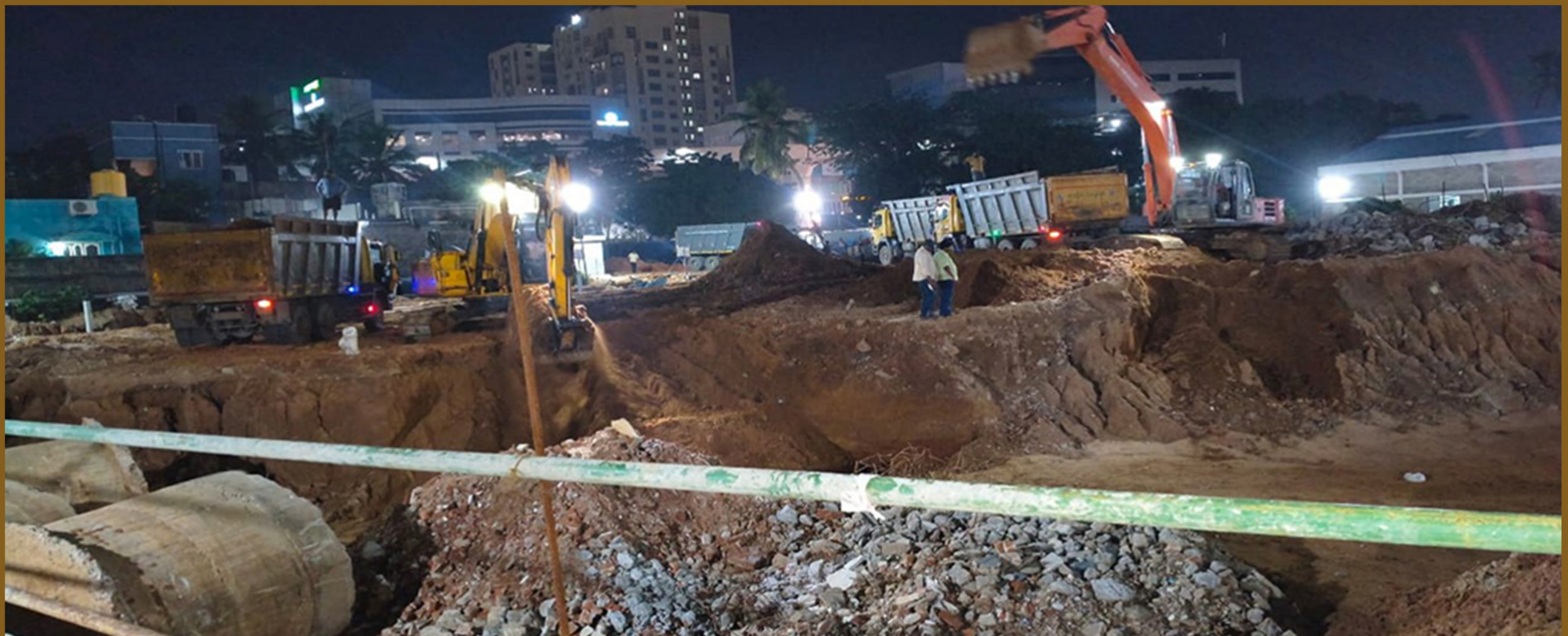
BLOCK B EARTH EXCAVATION WORKS
