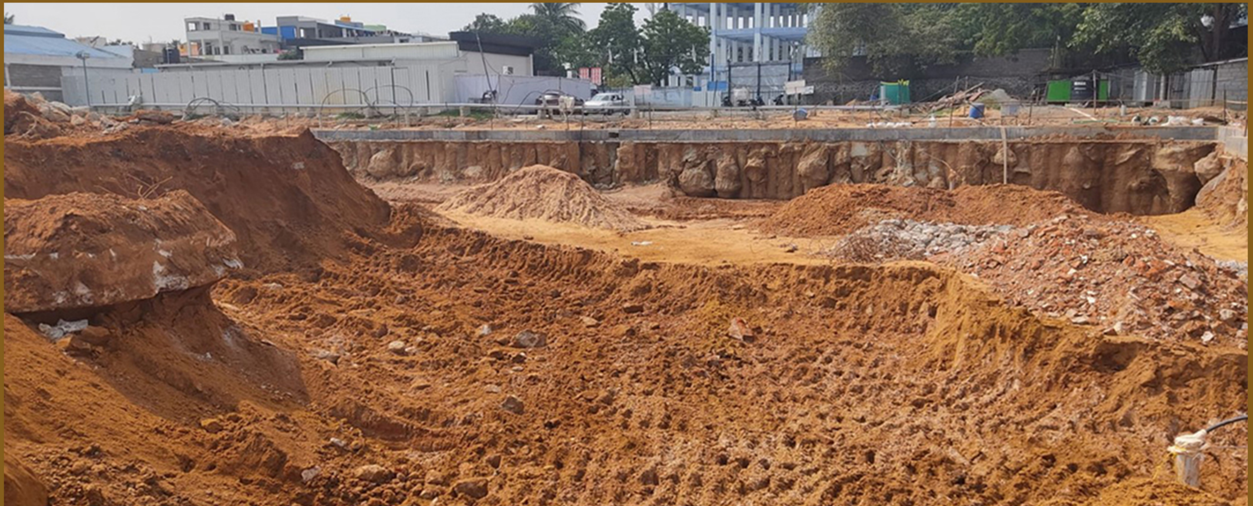
BLOCK B EARTH EXCAVATION WORKS
