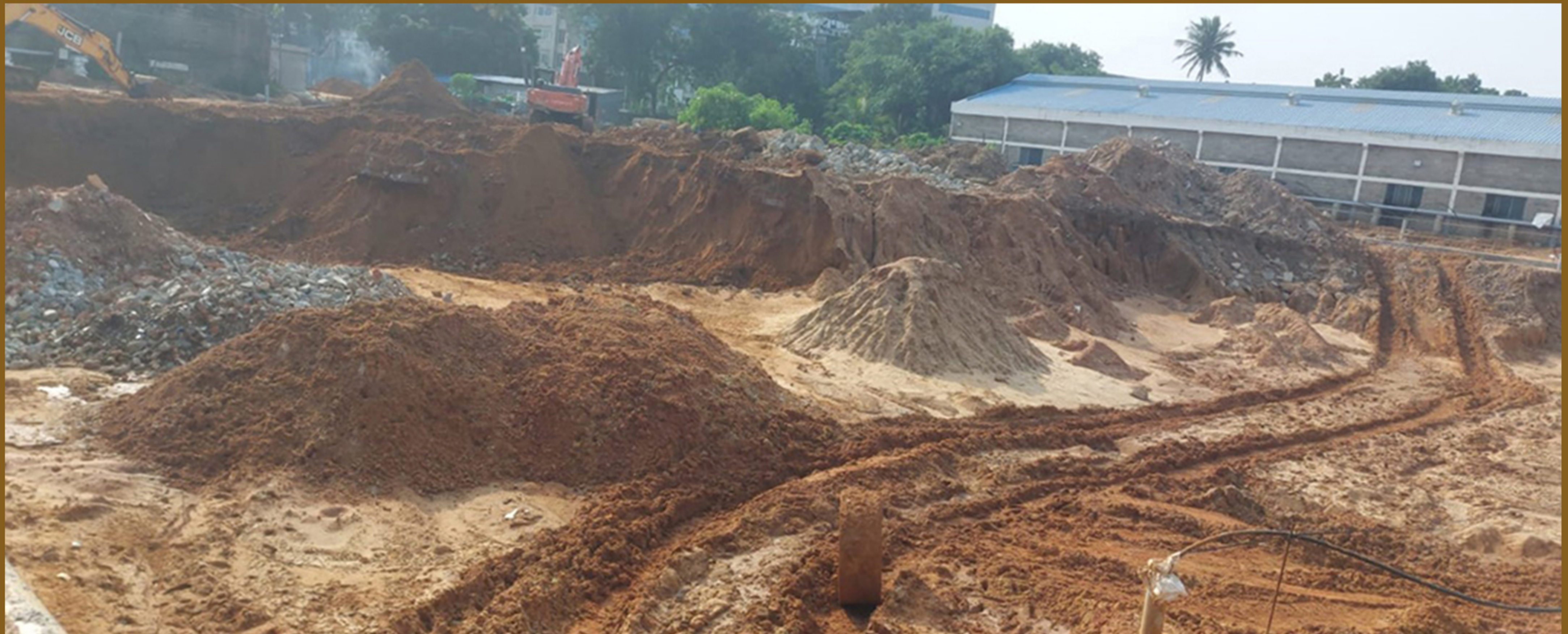
BLOCK B EARTH EXCAVATION WORKS
