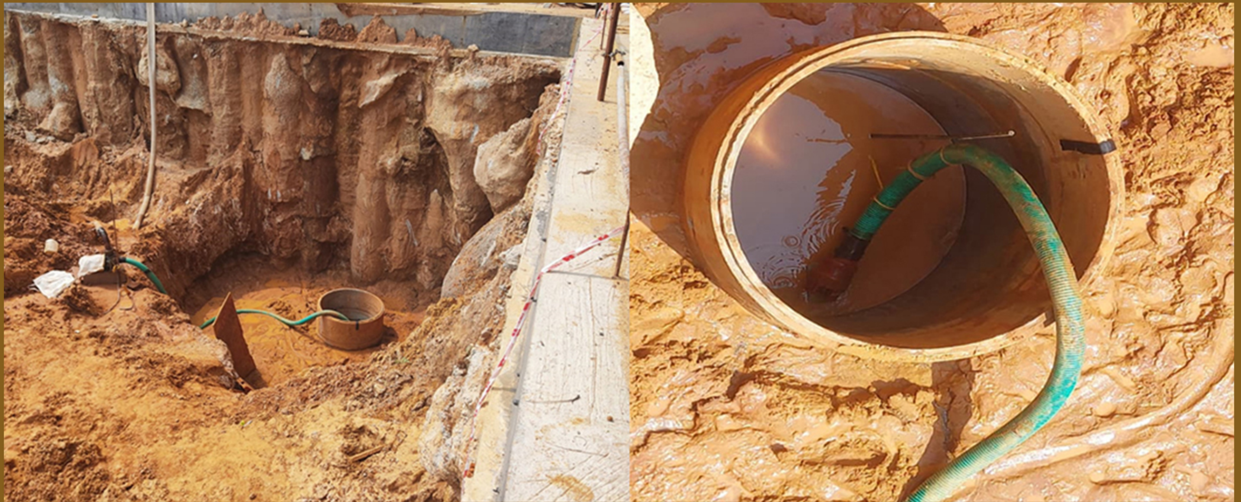
BLOCK B DEWATERING SYSTEM WORK
