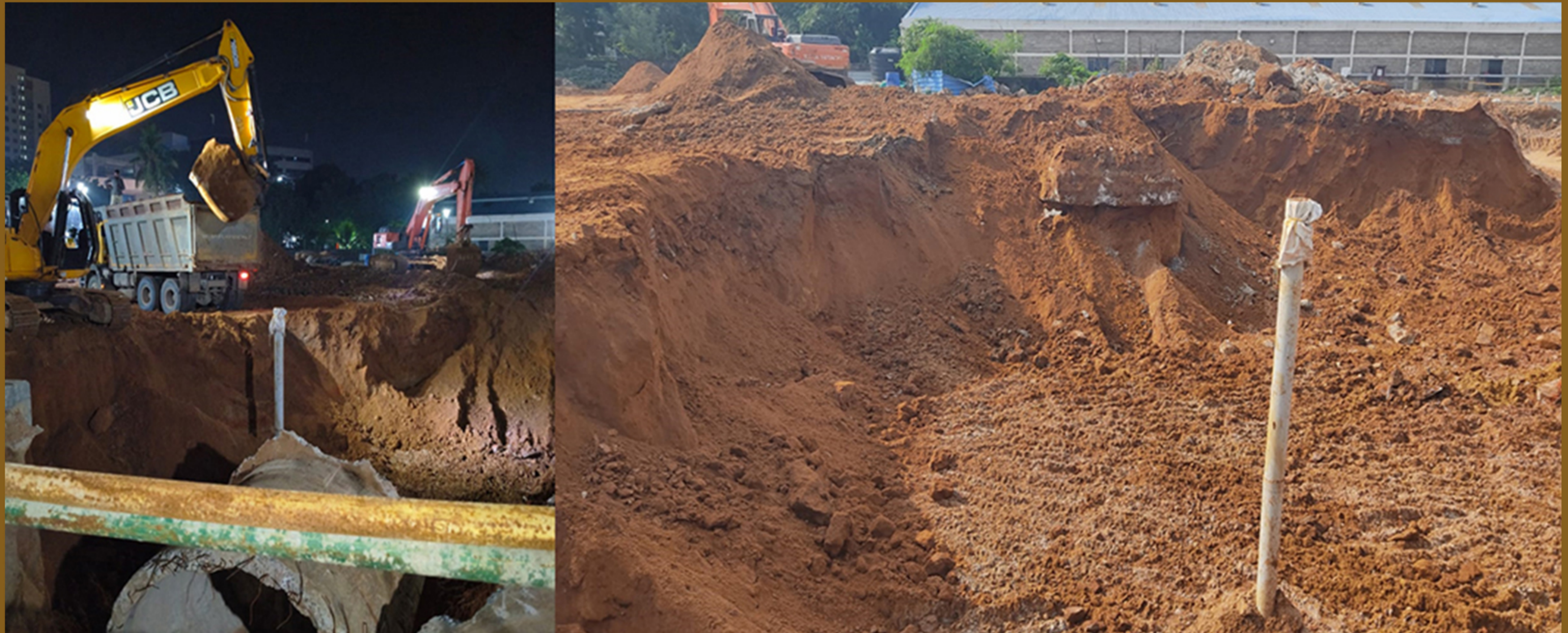
BLOCK B EARTH EXCAVATION WORKS
