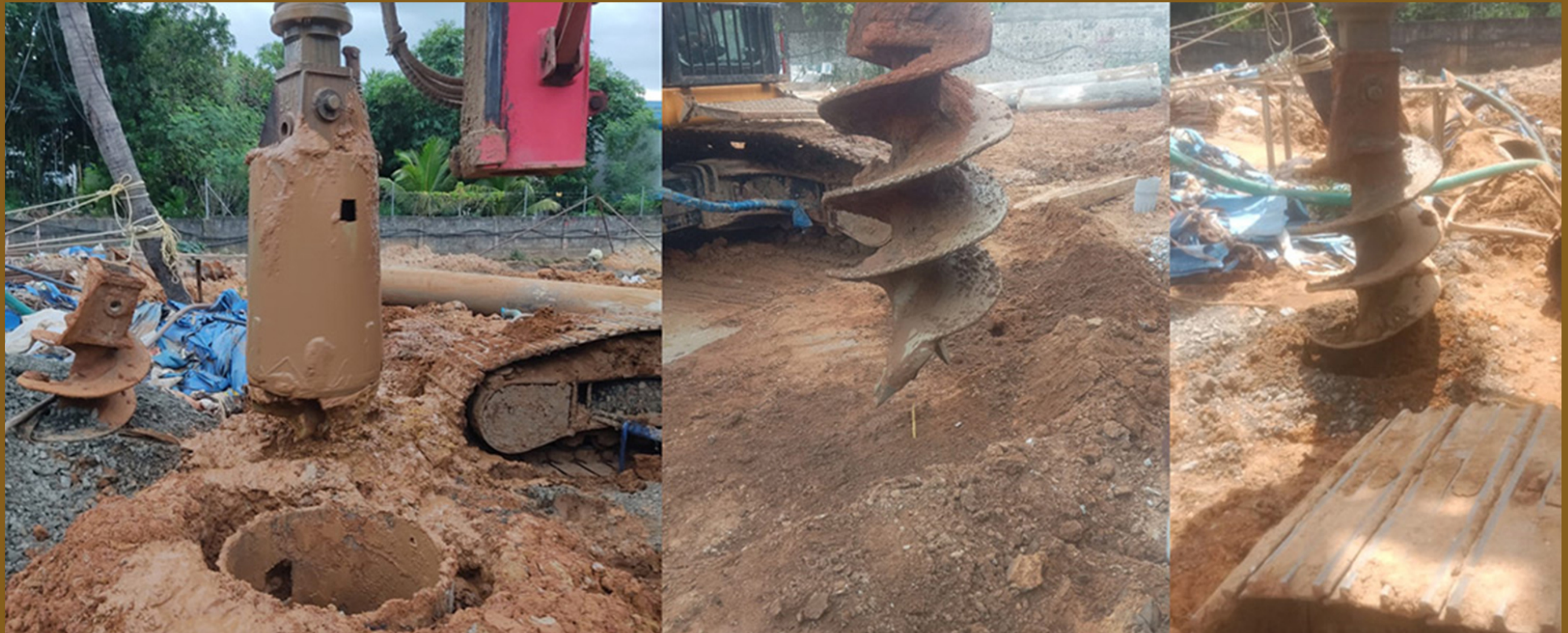
BLOCK B PILE BORING WORKS
