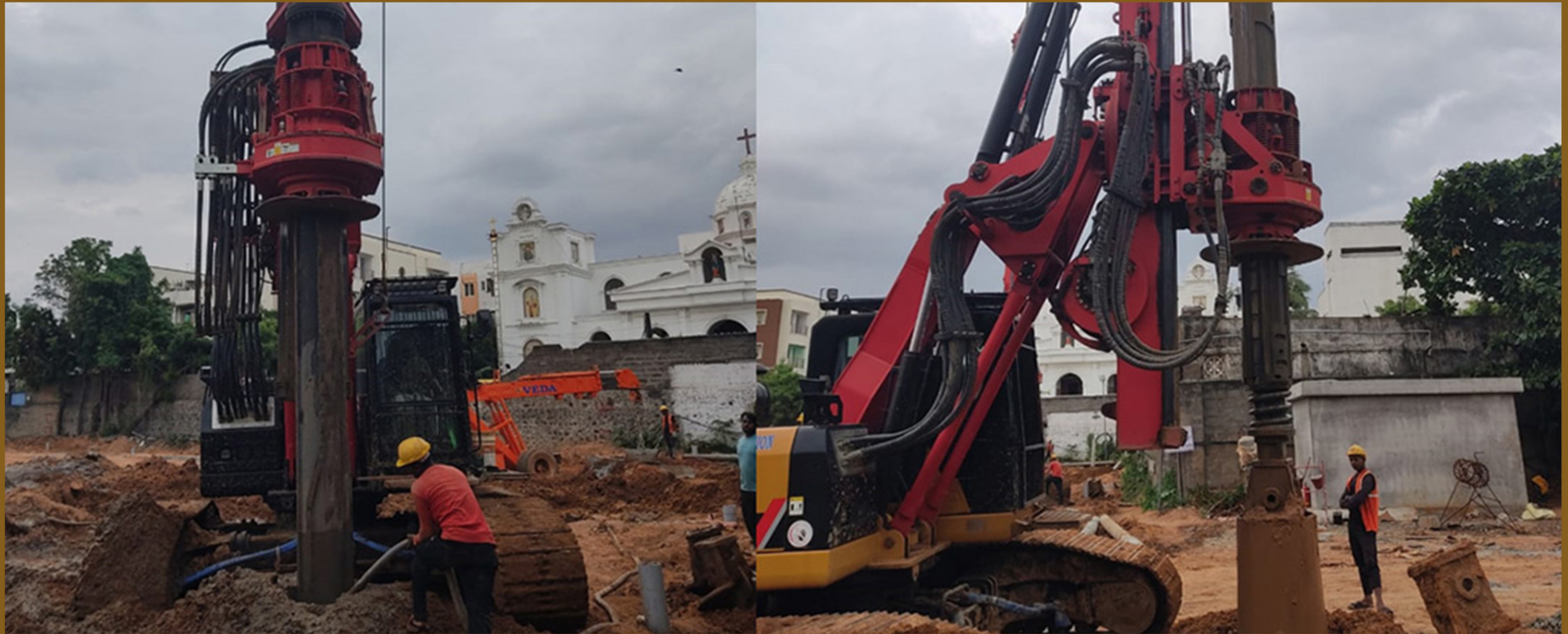
BLOCK B PILE BORING WORKS
