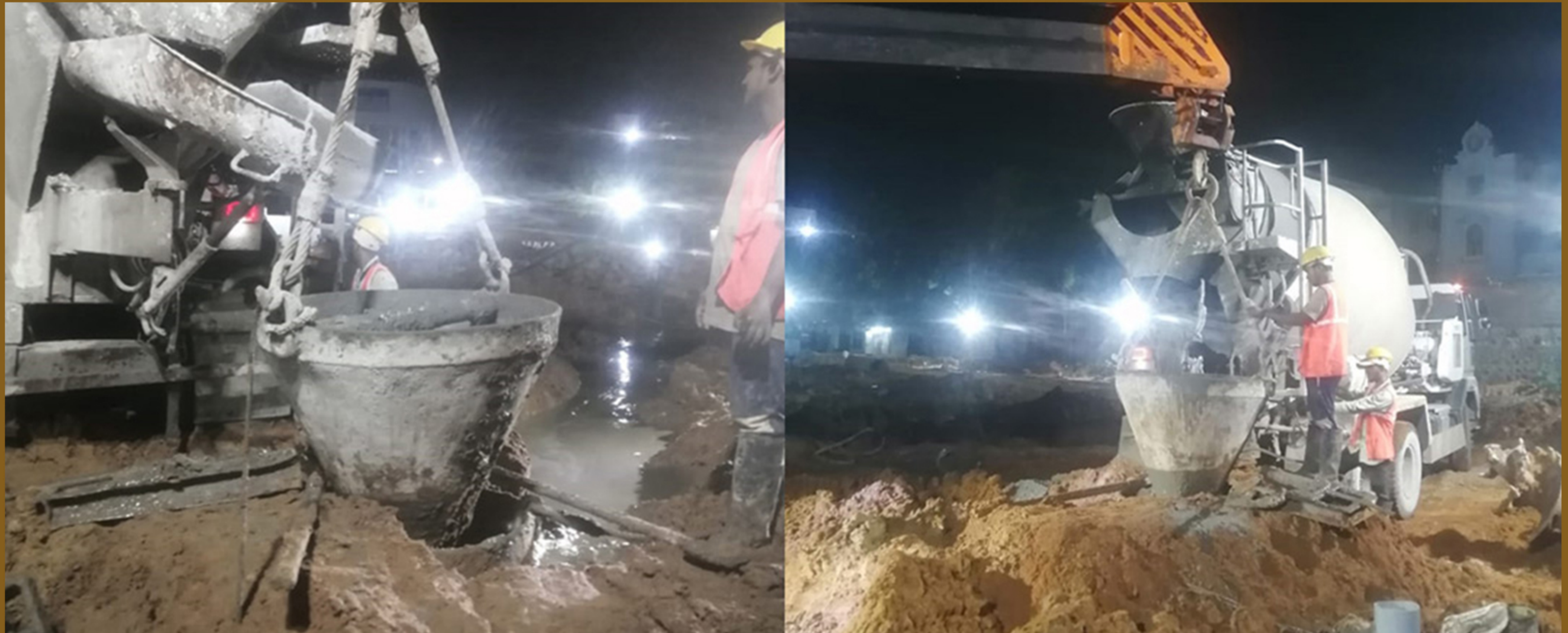
BLOCK B PILE CONCRETE WORKS
