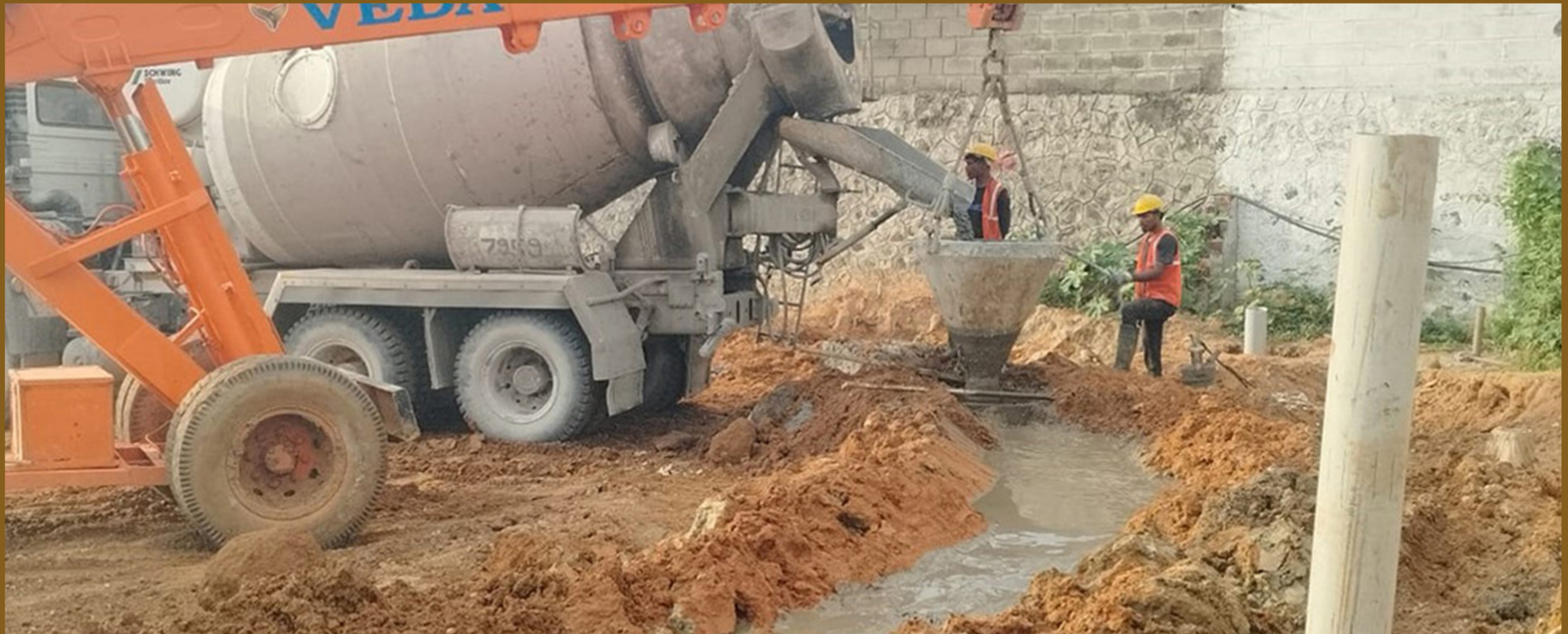
BLOCK B PILE CONCRETE WORKS
