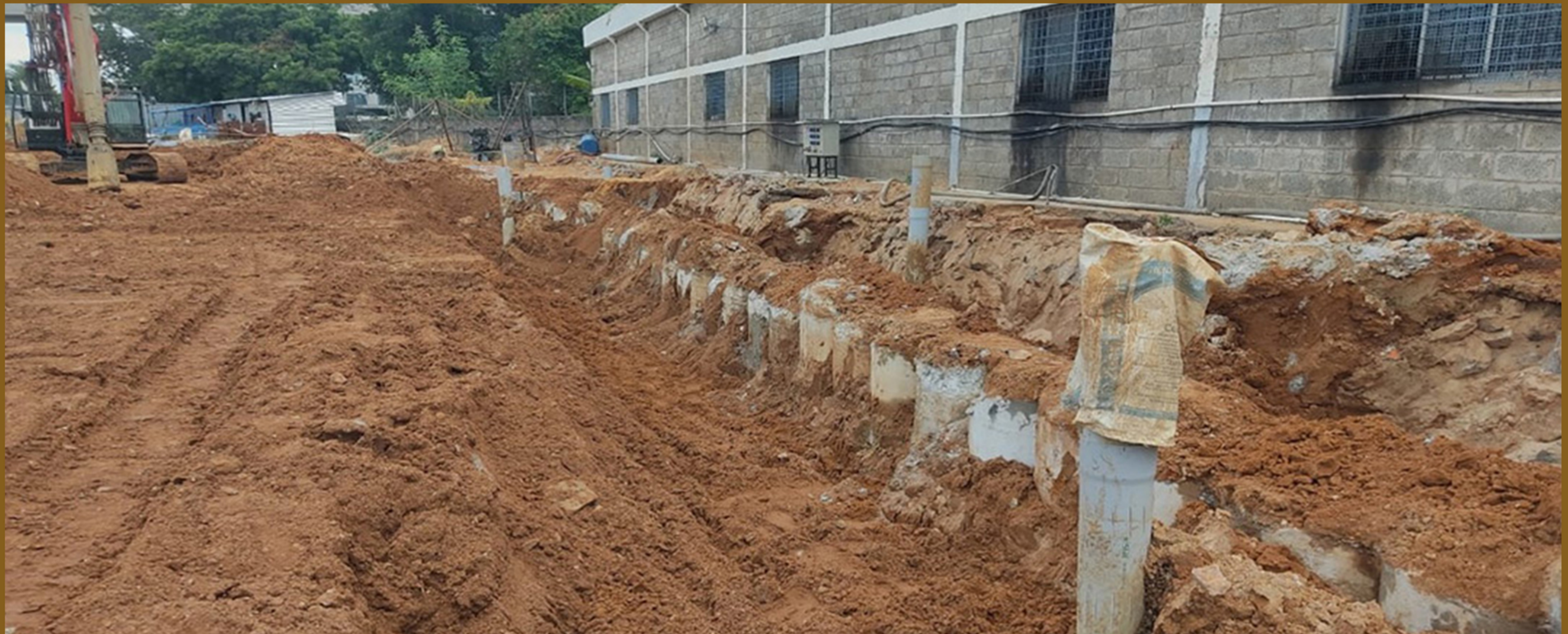
BLOCK B TIE BEAM EXCAVATION WORK
