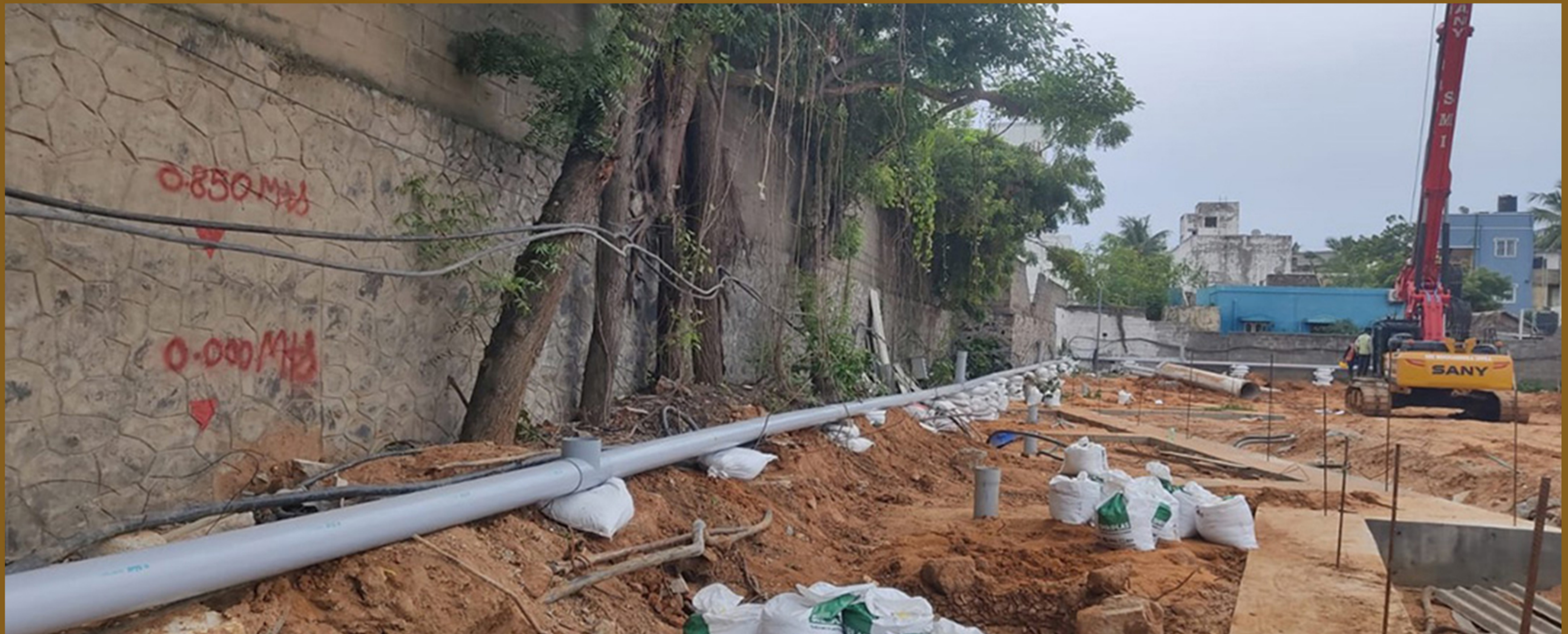
BLOCK B DEWATERING PIPE RING MAIN WORK
