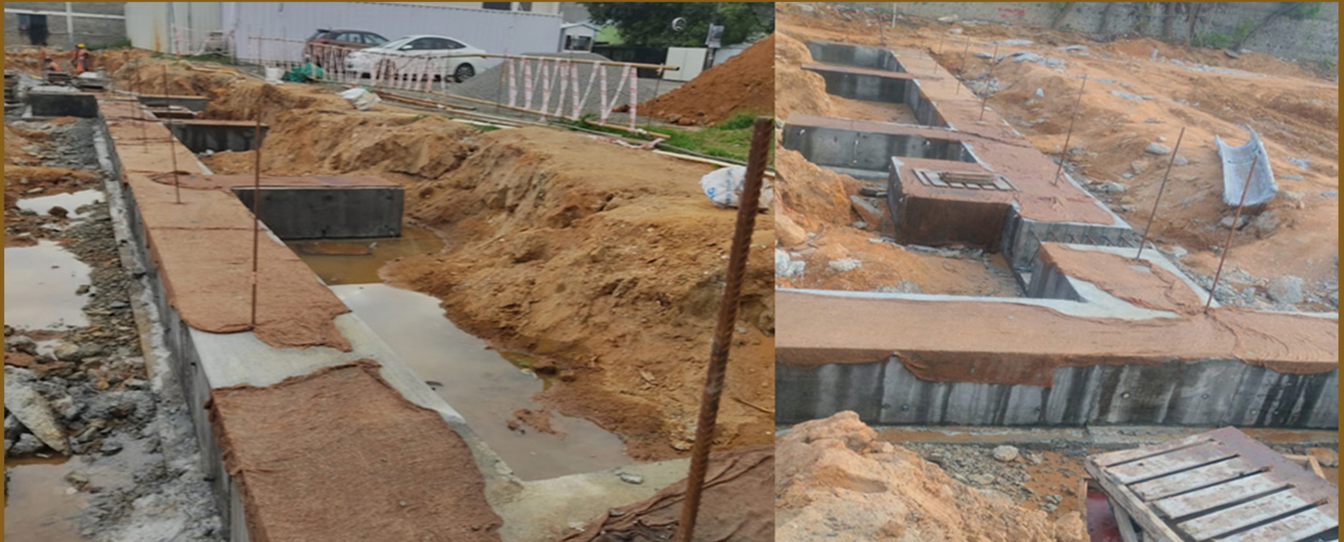
BLOCK B TIE BEAM CURING WORK
