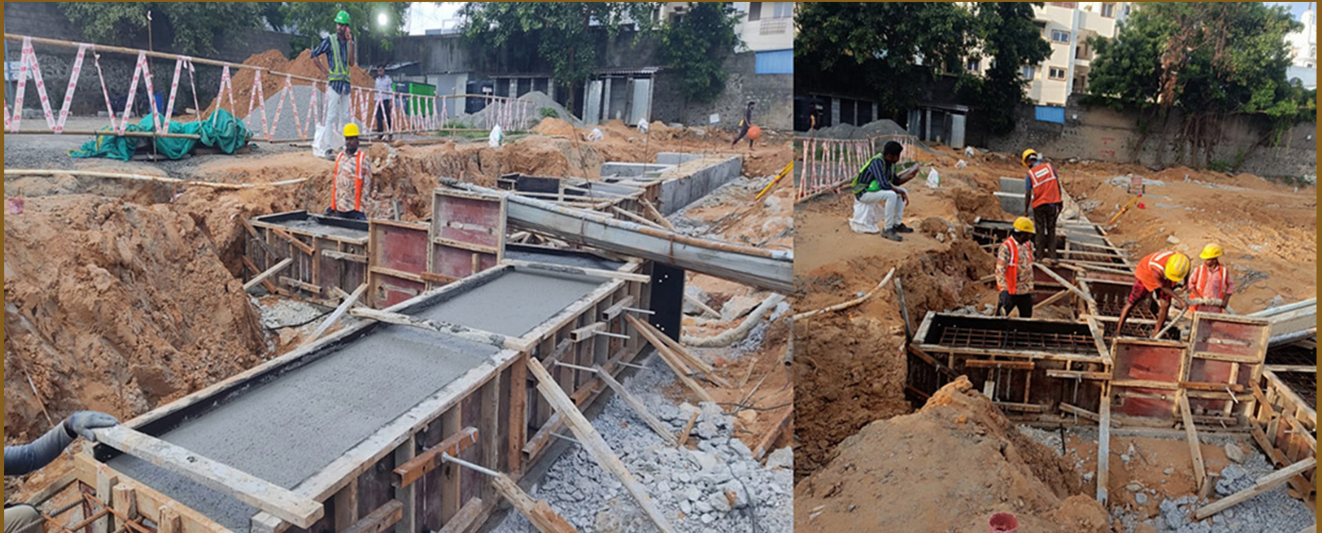
BLOCK B TIE BEAM RCC CONCRETE LAYING
