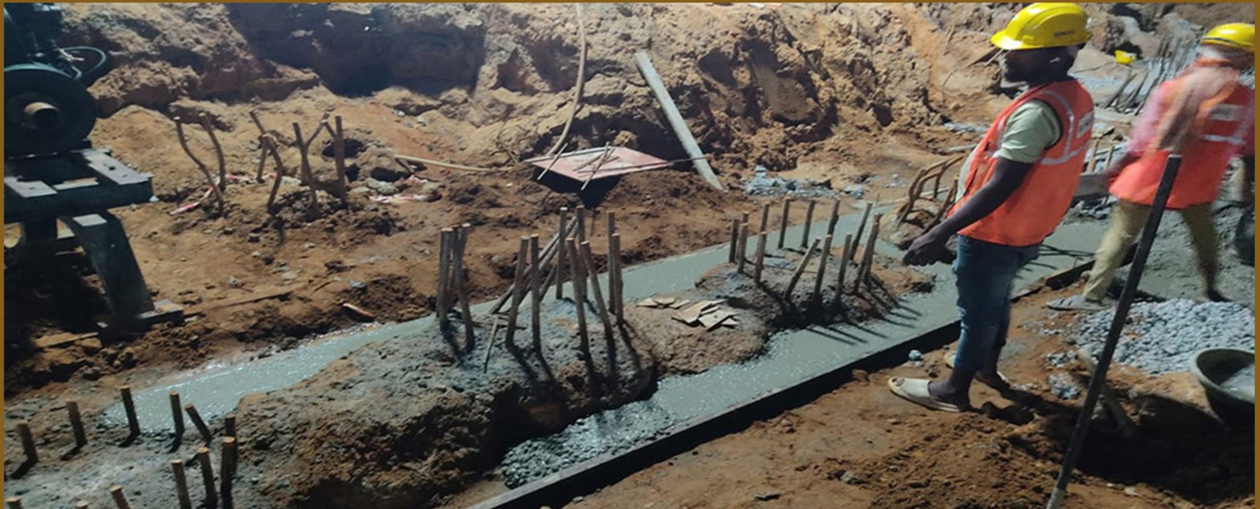
BLOCK B TIE BEAM PCC CONCRETE WORK
