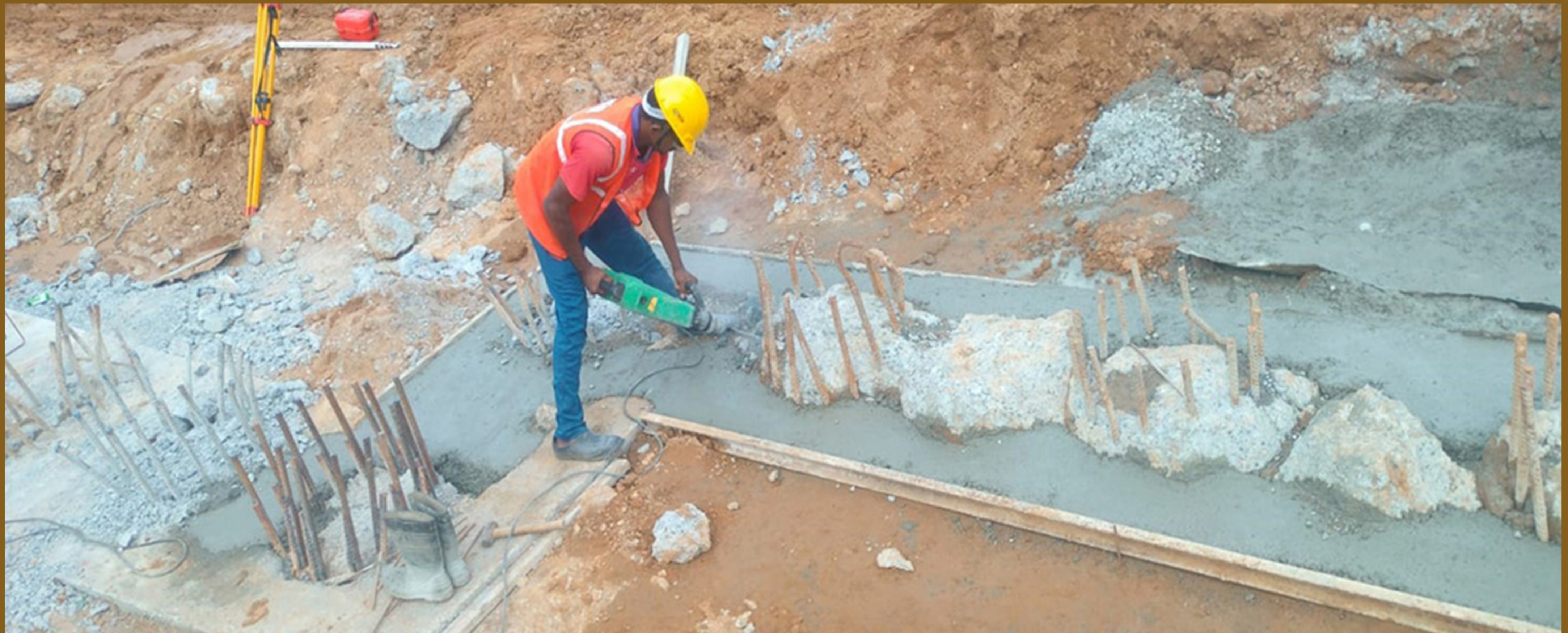
BLOCK B PILE CONCRETE CHIPPING WORK
