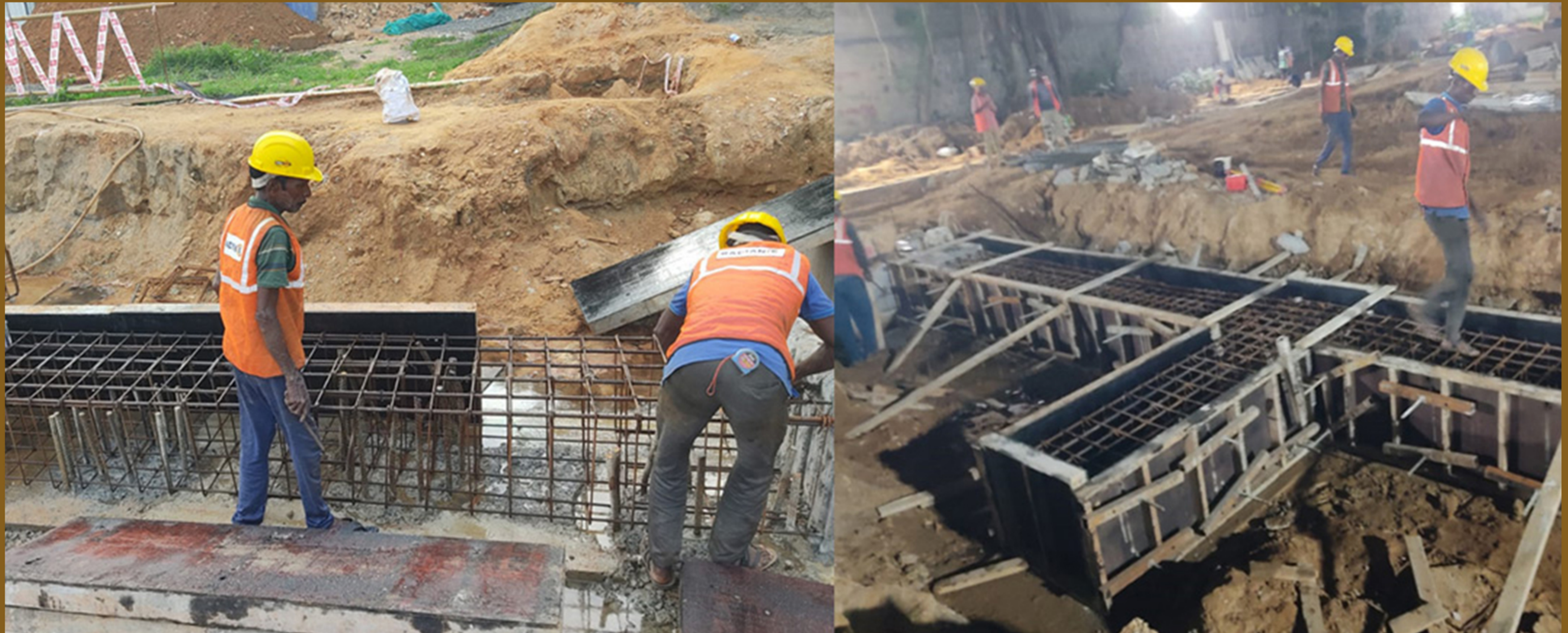
BLOCK B TIE BEAM SHUTTERING WORK
