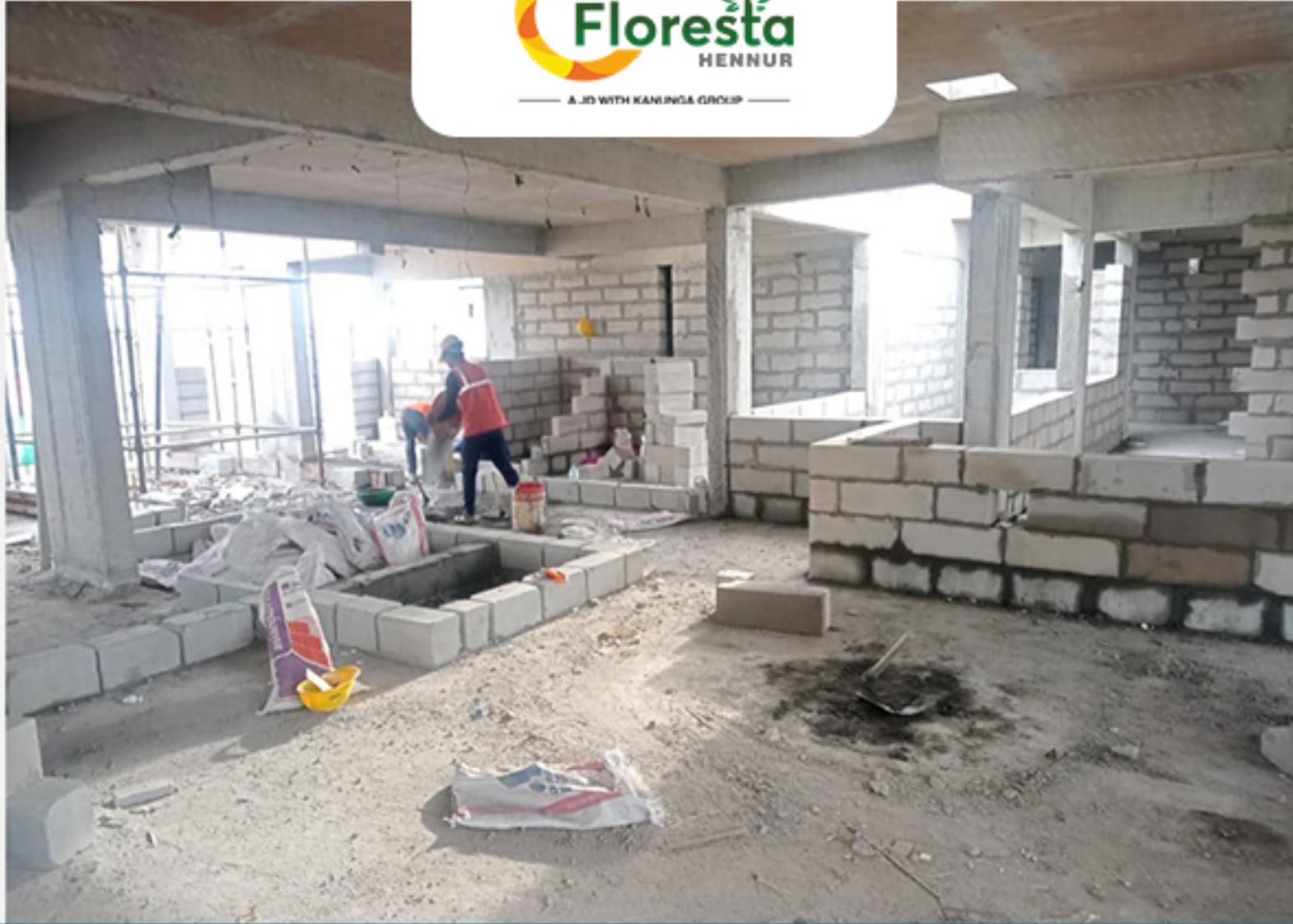
B-BLOCK CLUSTER-02 4TH FLOOR BLOCK WORK IN PROGRESS
