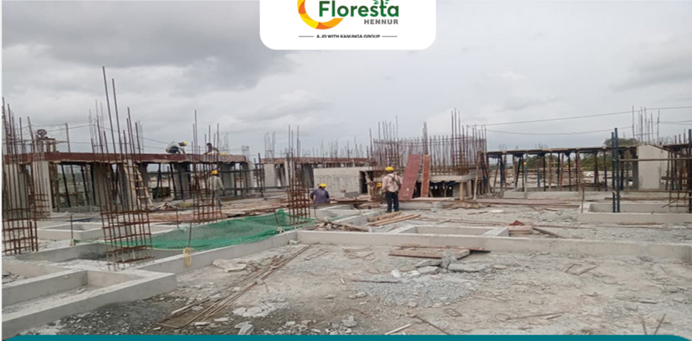
B-BLOCK CLUSTER-02 ELEVATION SLAB AND OHT SLAB SHUTTERING WORK IN PROGRESS
