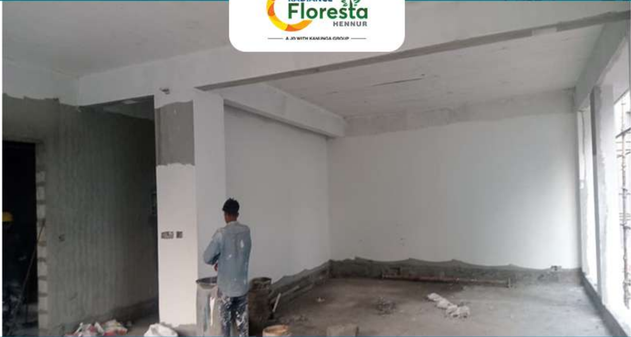
Club House Internal Putty Work in Progress
