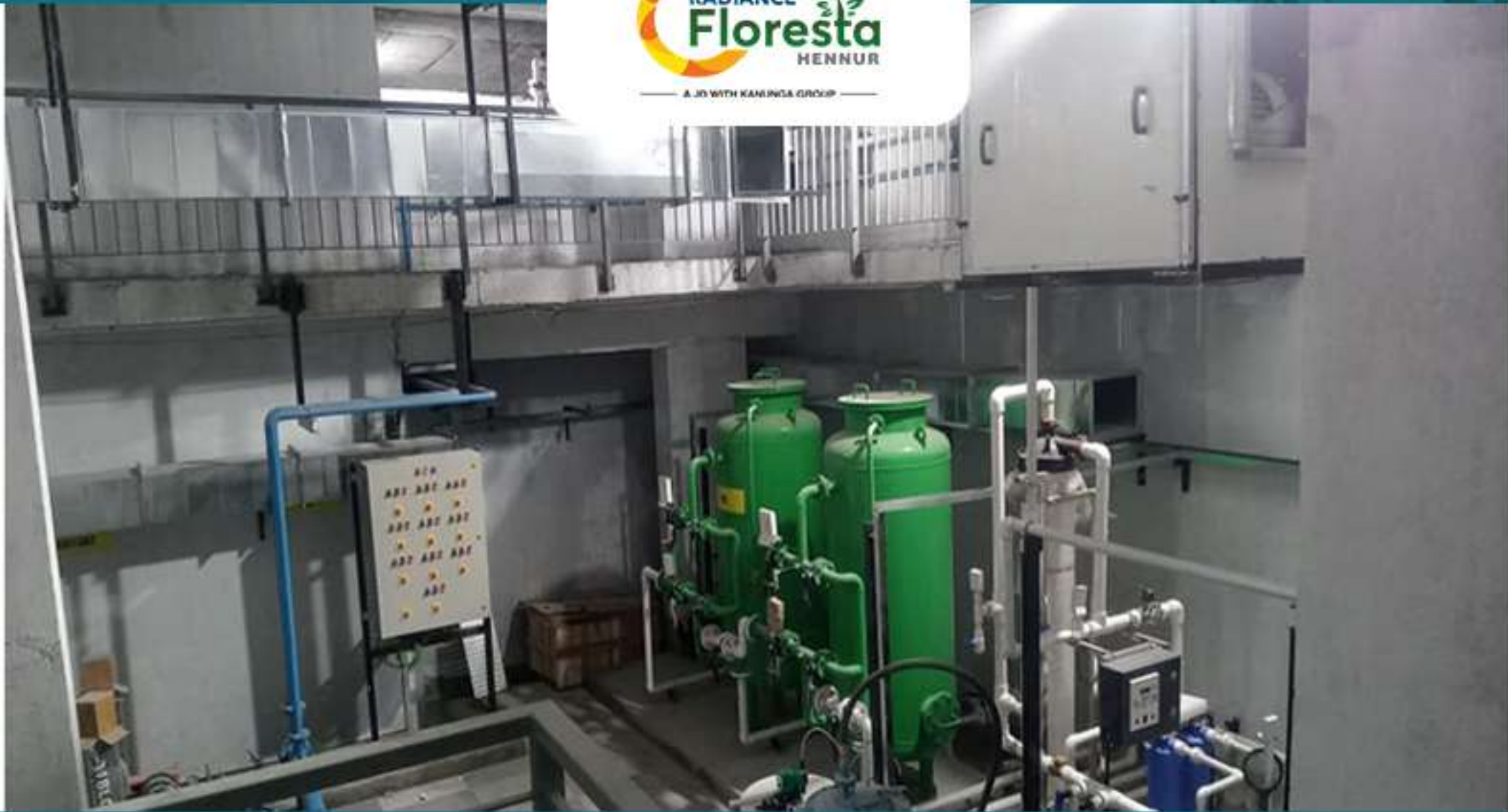
STP and WTP Machinery Work
