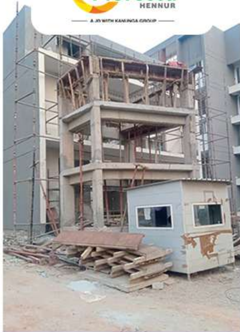
Entry Portal Structural Work in Progress
