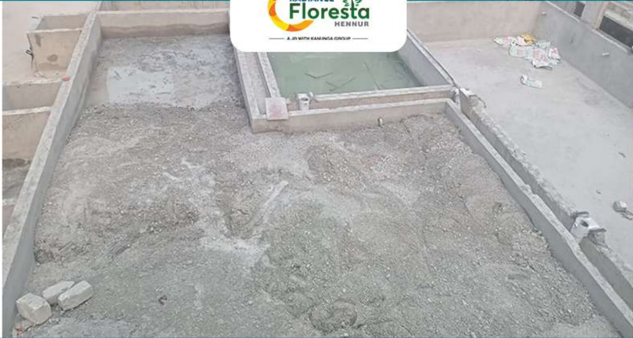
Pool Deck Area Cinder Filling Work in Progress
