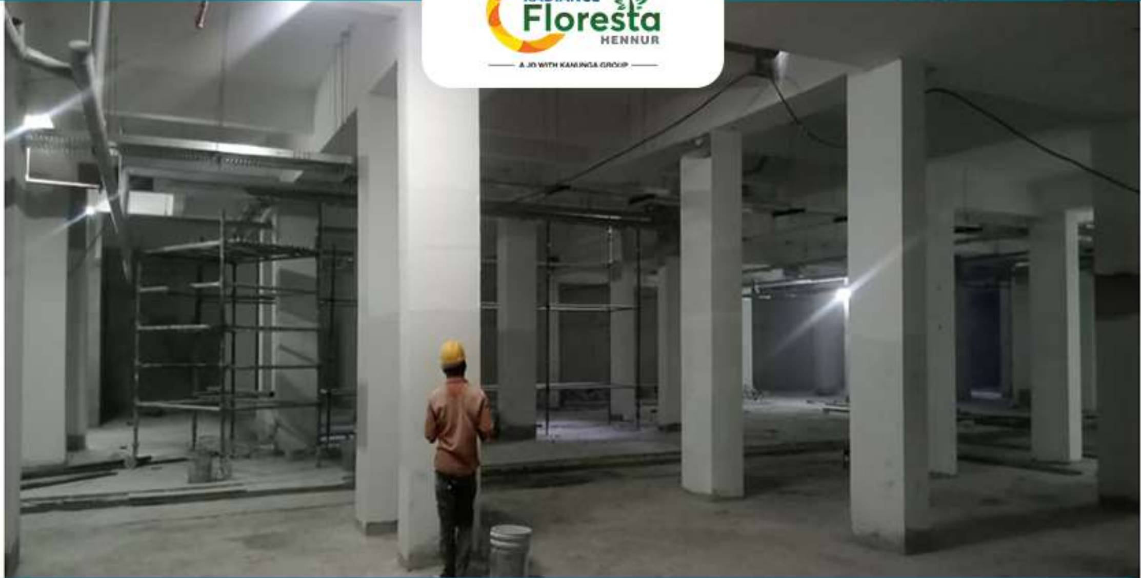
Basement Painting Work in Progress
