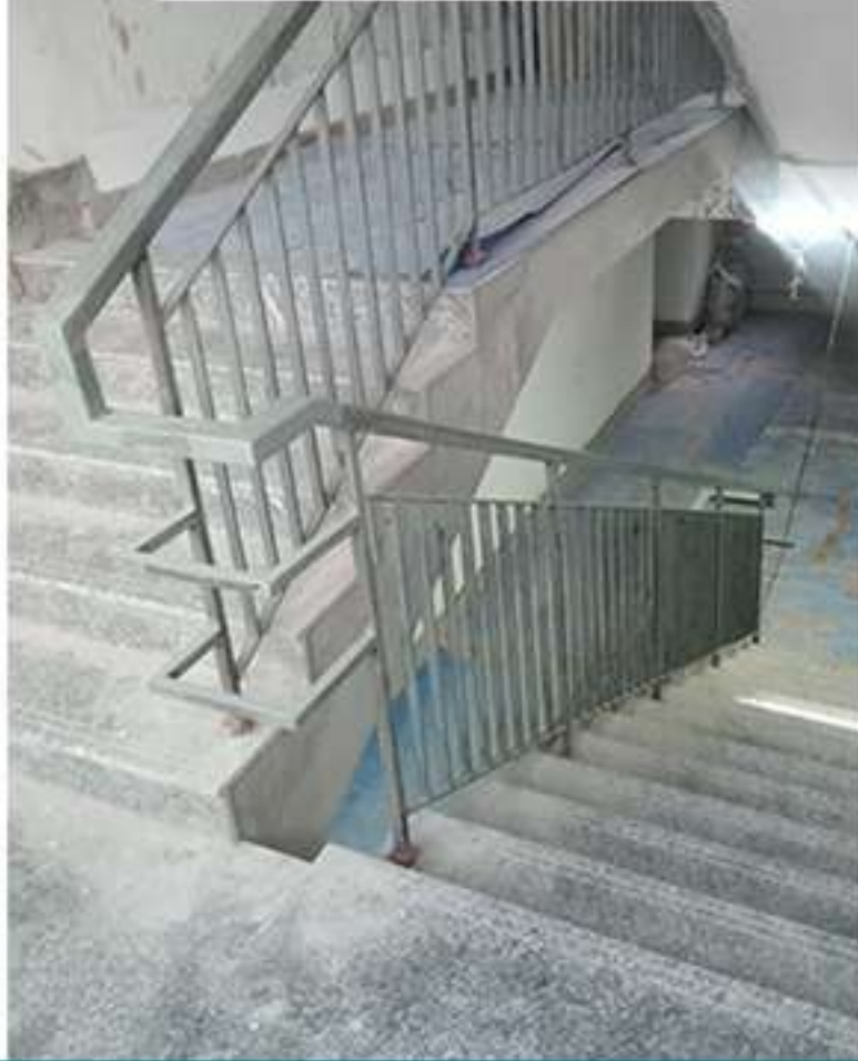
A-Block Common Staircase Handrail Work In Progress
