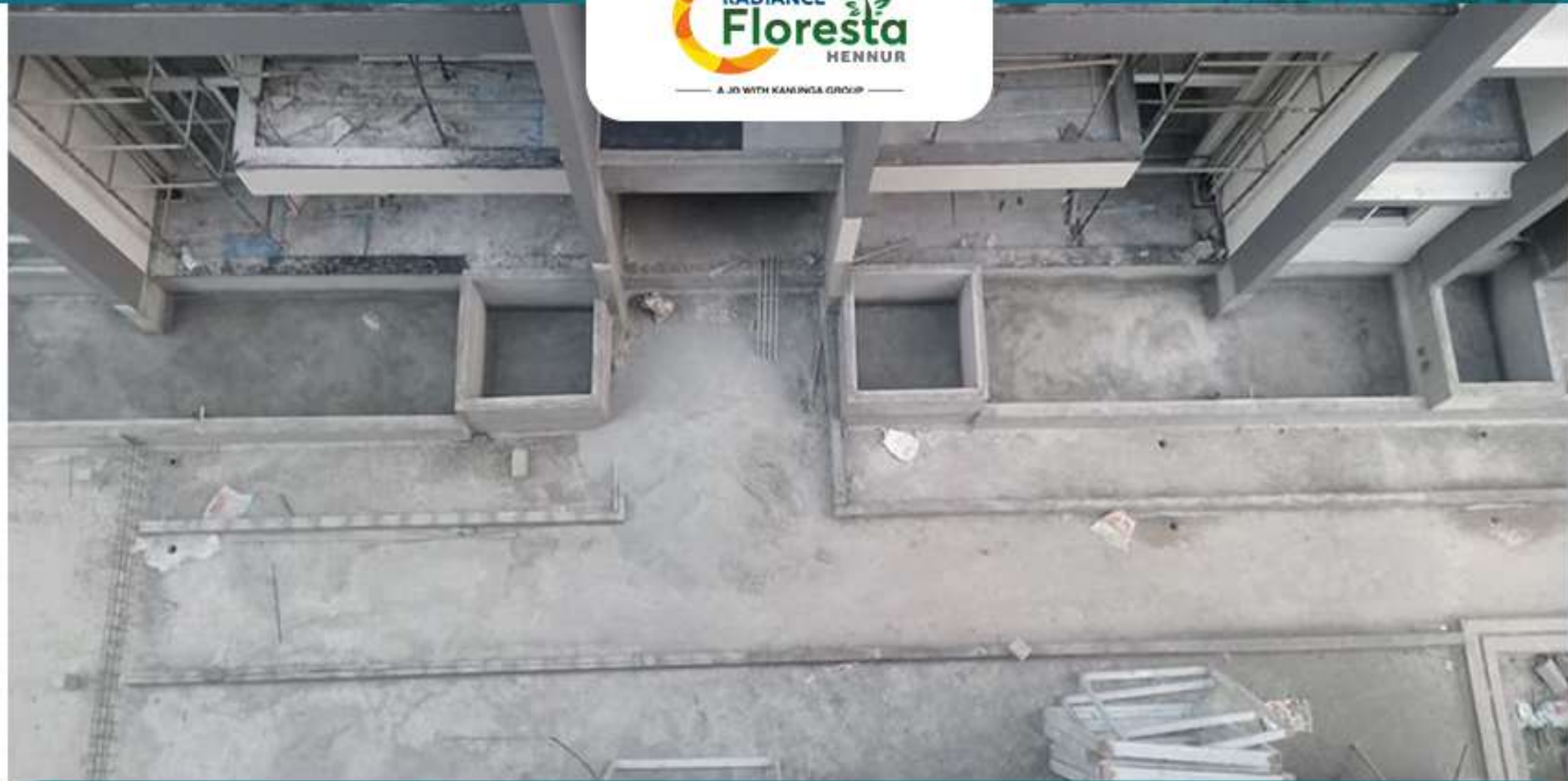
Planter Box Water Proofing Work in Progress
