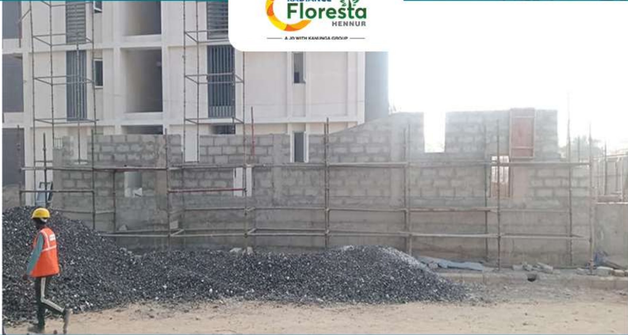
West Side Compound Wall Block Work in Progress
