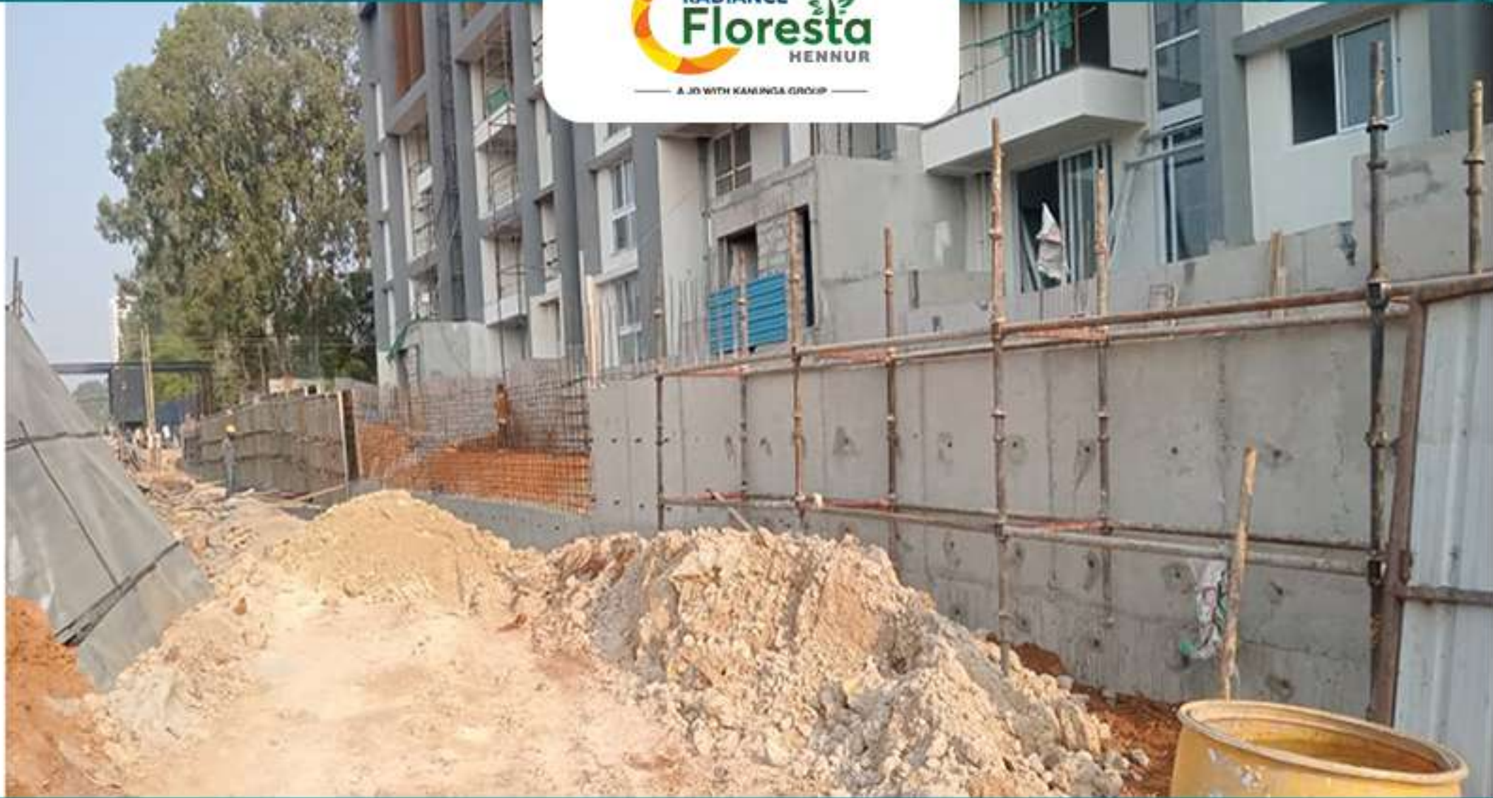
South Side Compound Wall RCC Work in Progress
