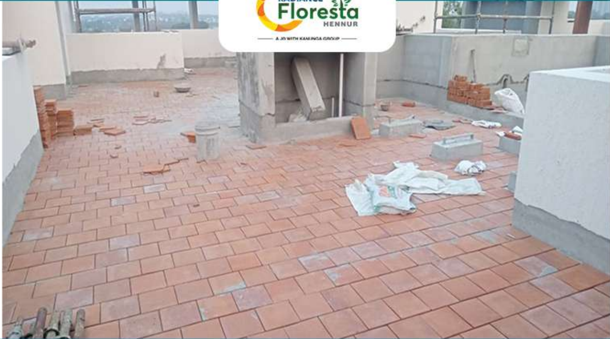
A-Block Cluster-01 Terrace Clay Tile Work In Progress
