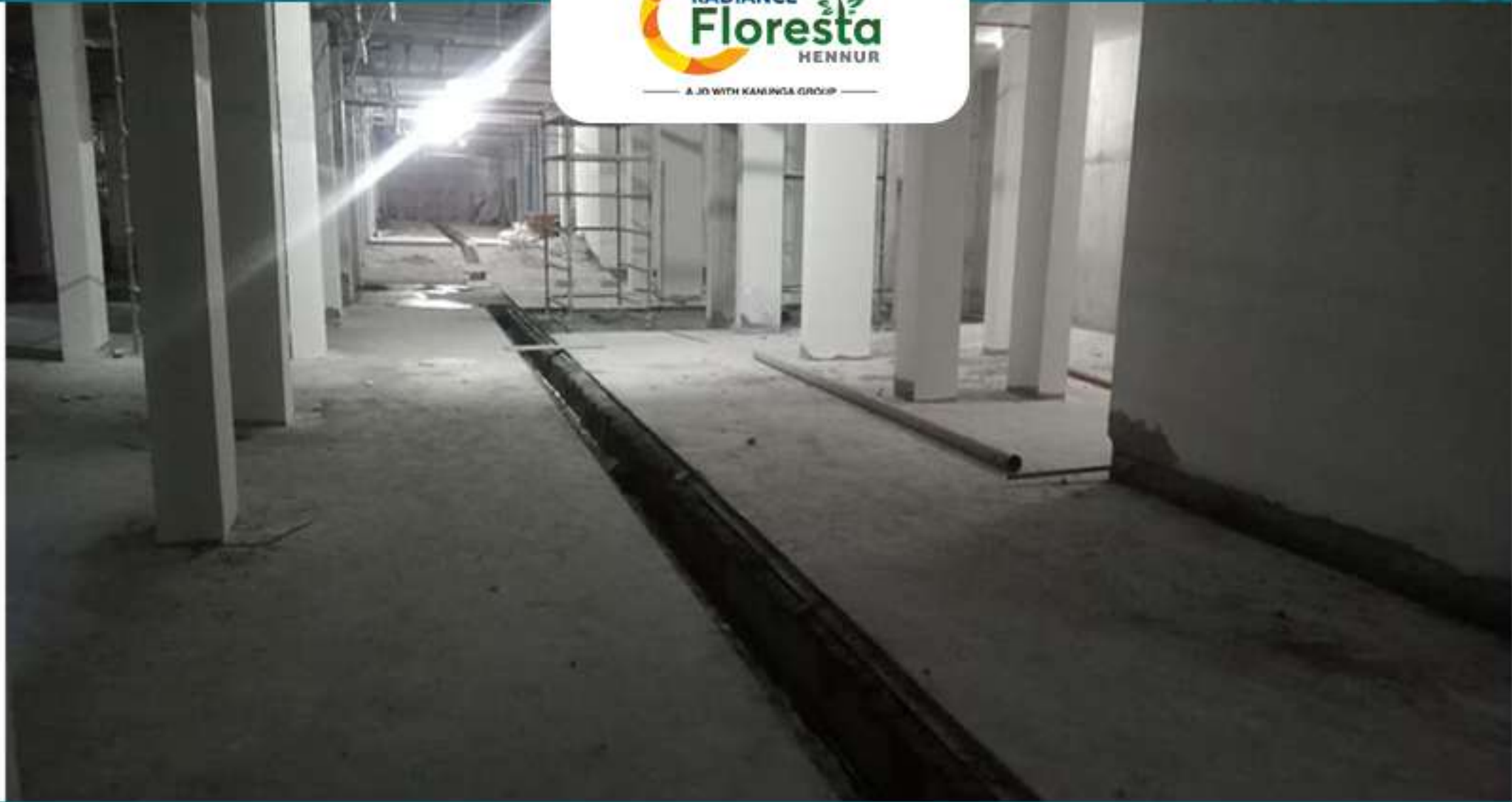
A-Block Basement Screed Concrete Work Completed
