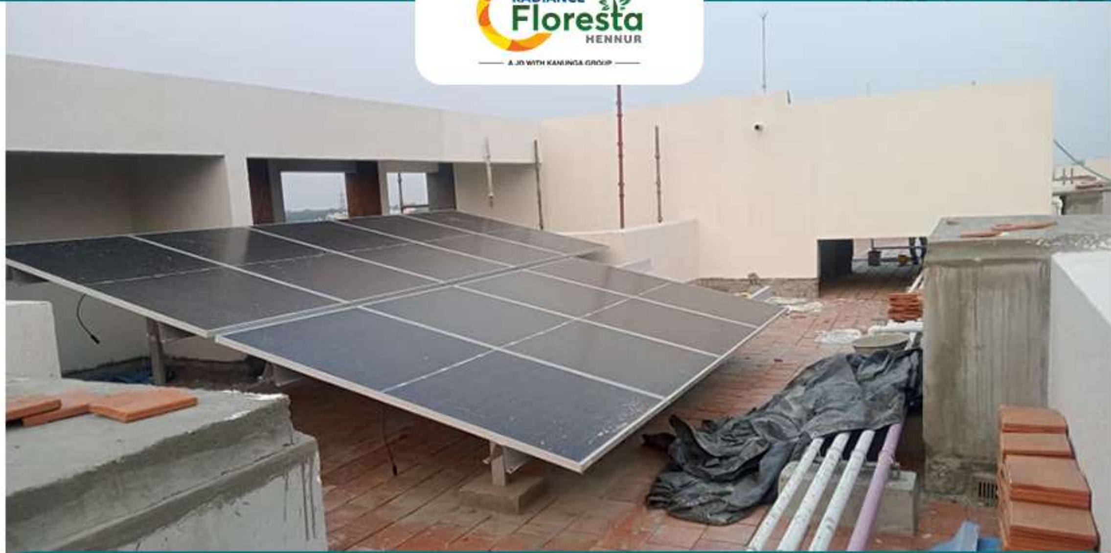
Solar Provision Work in Progress
