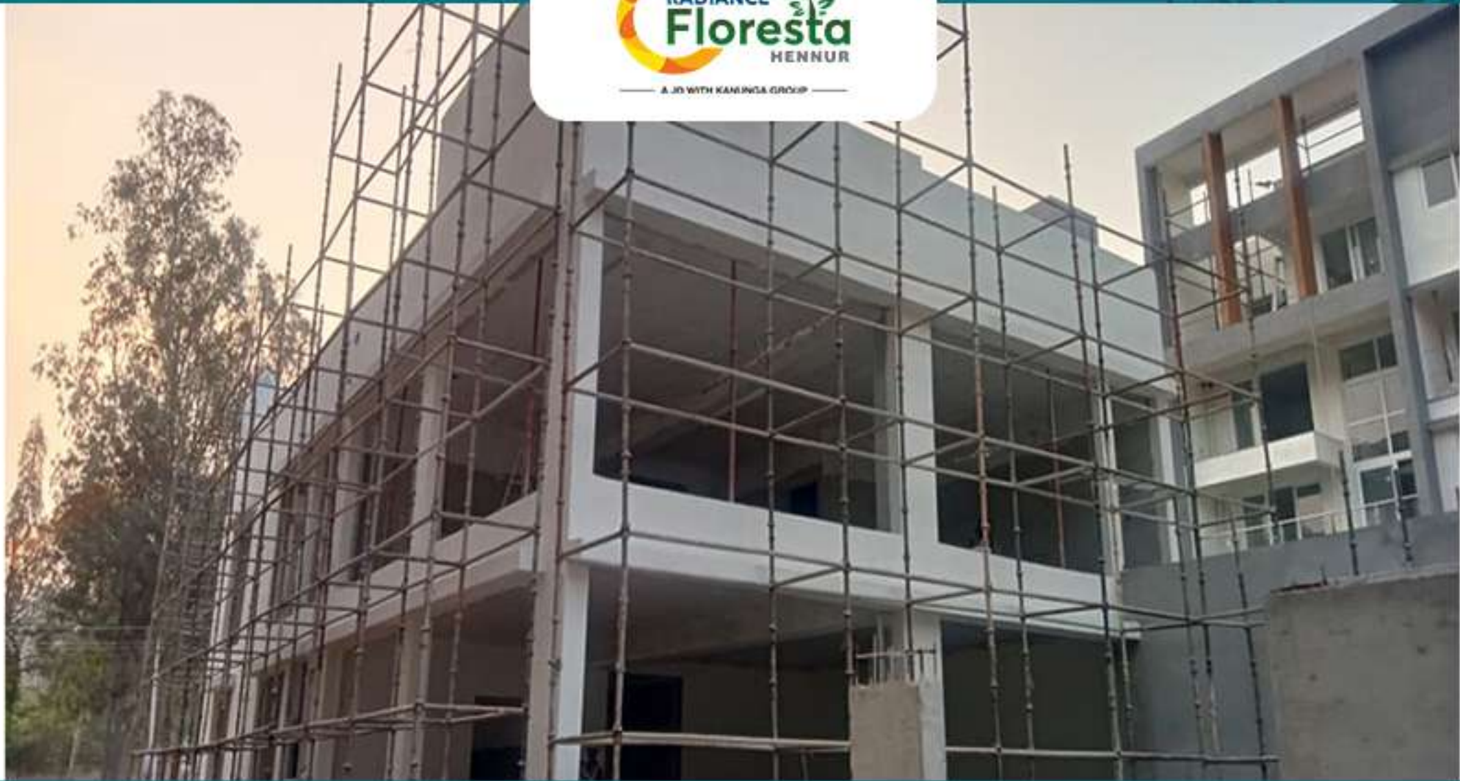
Club House External Painting Work in Progress
