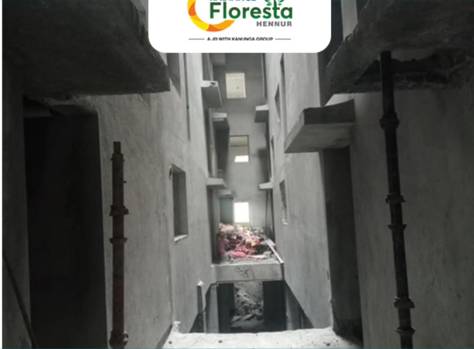
B-Block cluster-01, 02 OTS External plastering completed
