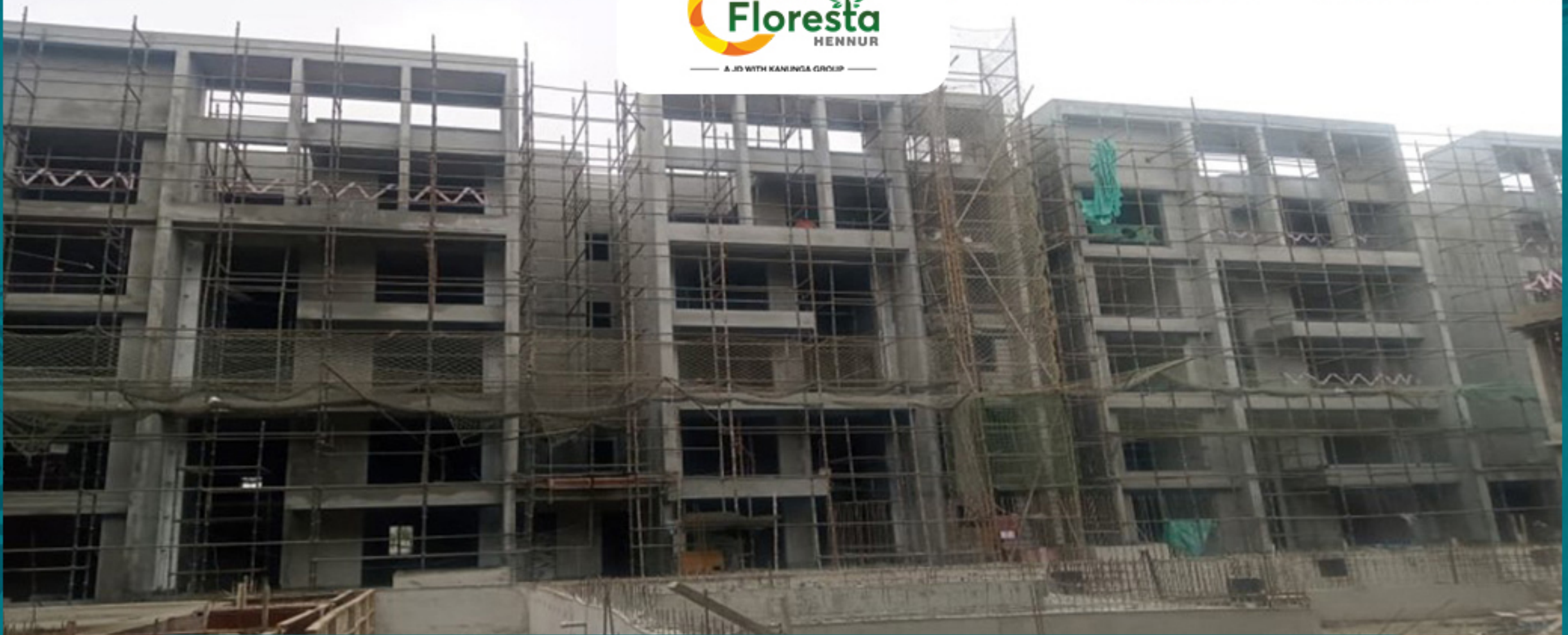
B-Block cluster-01, 02 external plastering completed
