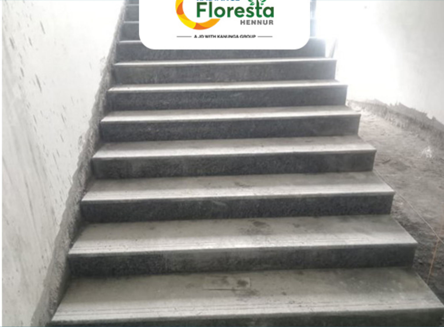
B-Block cluster-01 common staircase granite work in progress
