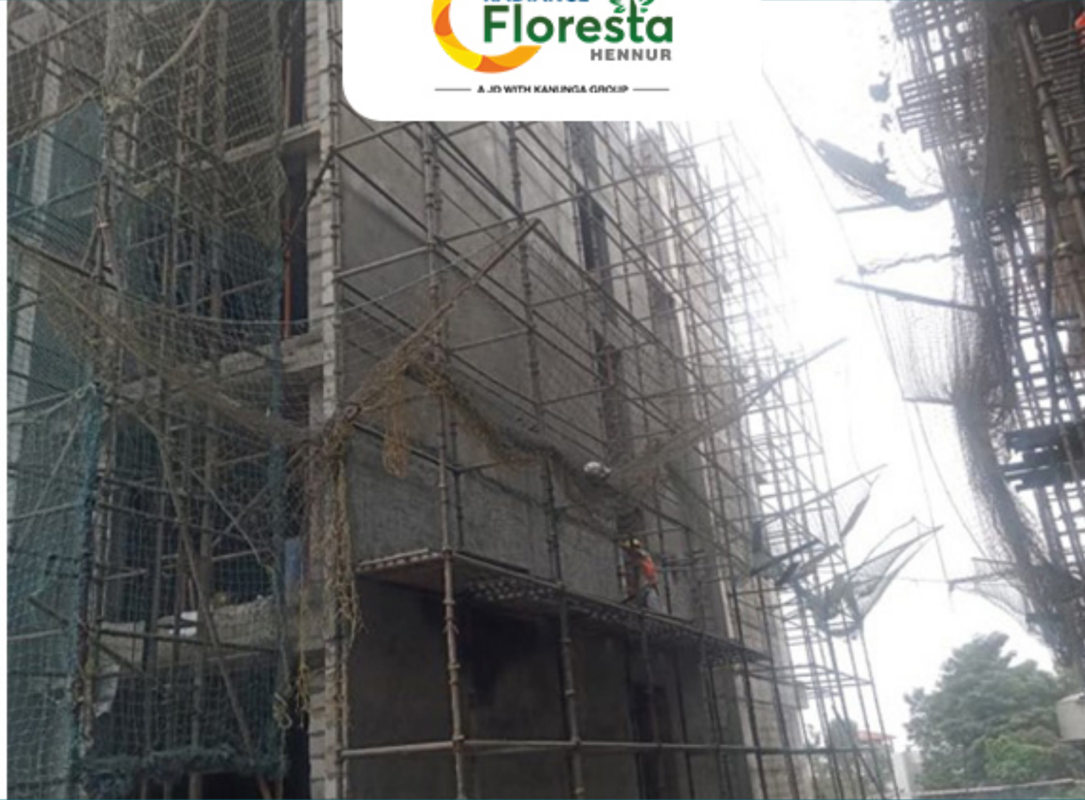
C-Block south side External plastering
