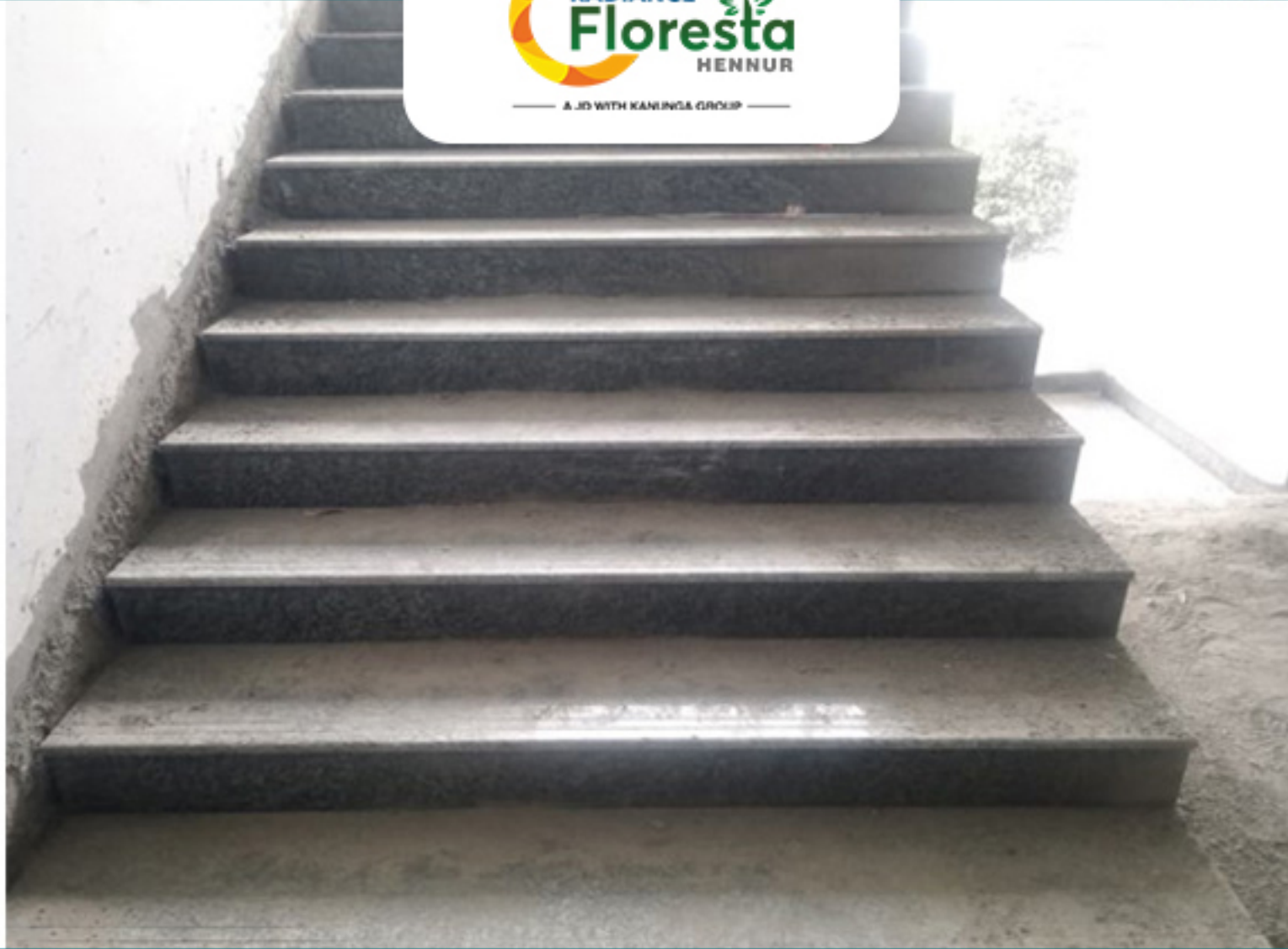
A-Block cluster-01 common staircase granite work in progress
