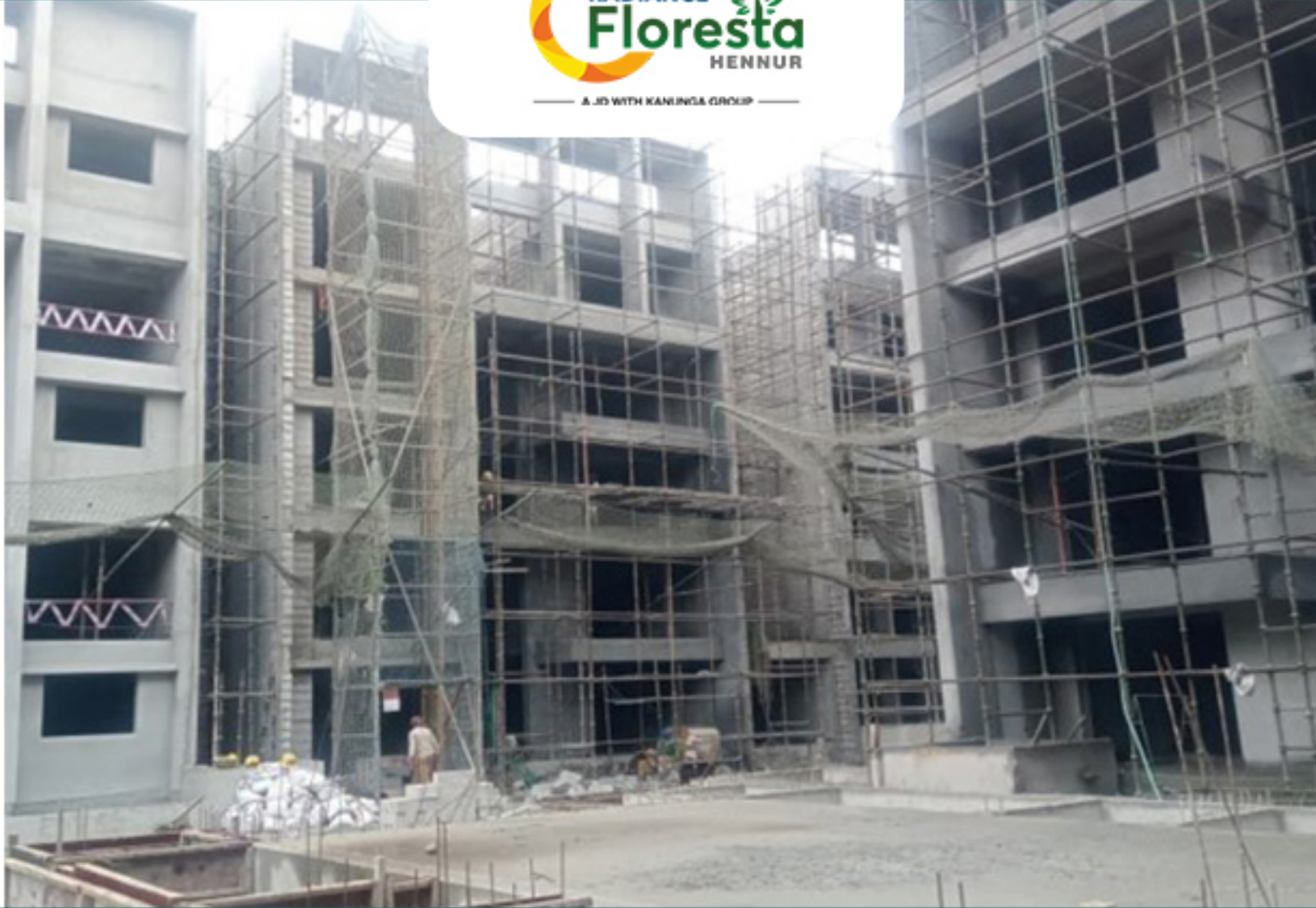
A-Block cluster-03 south side external plastering work in progress
