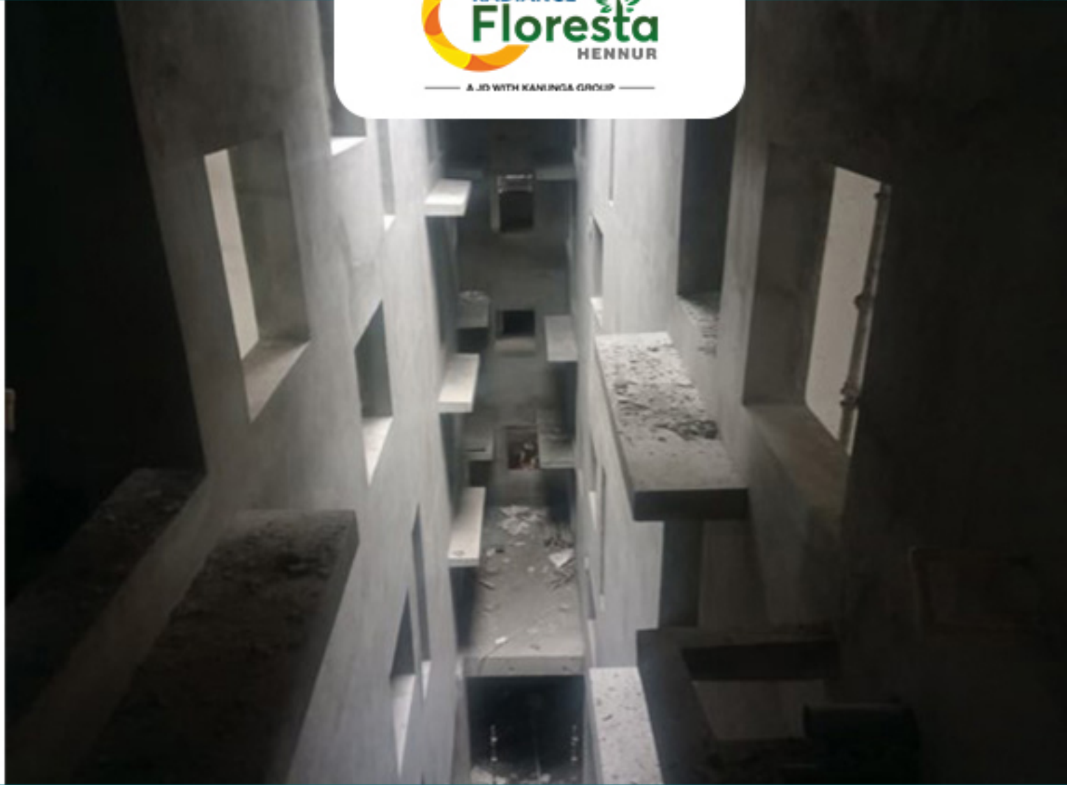
A-Block cluster-01, 02 ots external plastering completed
