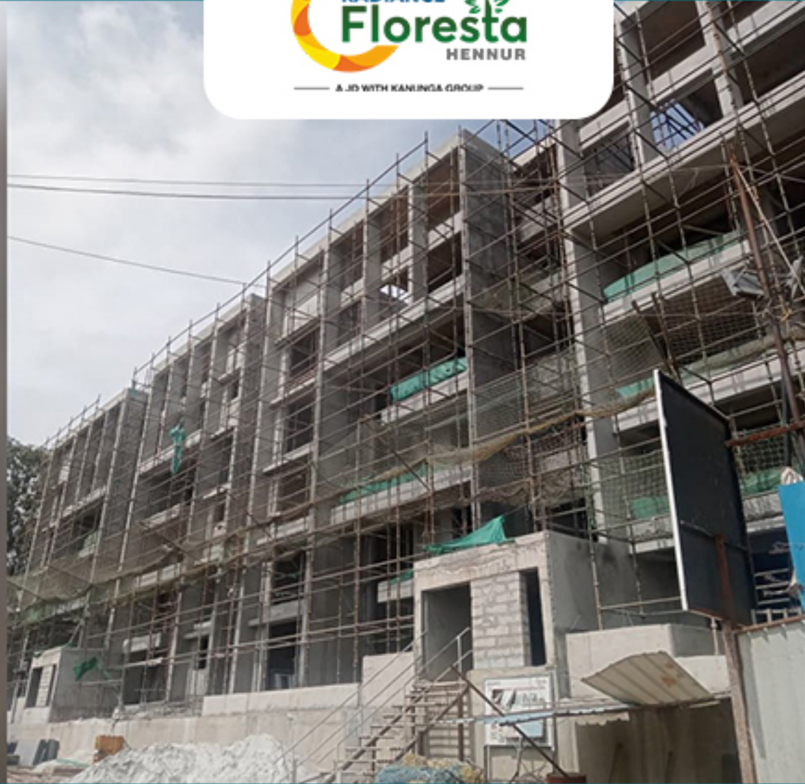
B-BLOCK SOUTH SIDE EXTERNAL PLASTERING
