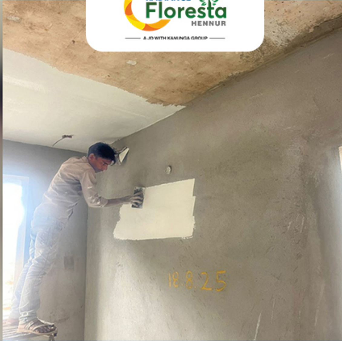
A-BLOCK CLUSTER-01 GF CEILING AND WALL PUTTY WORK IN PROGRESS
