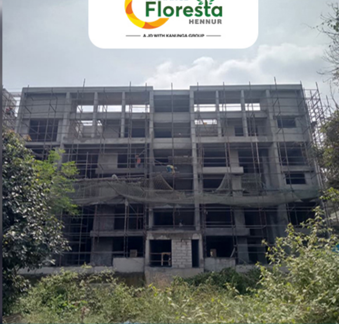
A-BLOCK NORTH SIDE EXTERNAL PLASTERING
