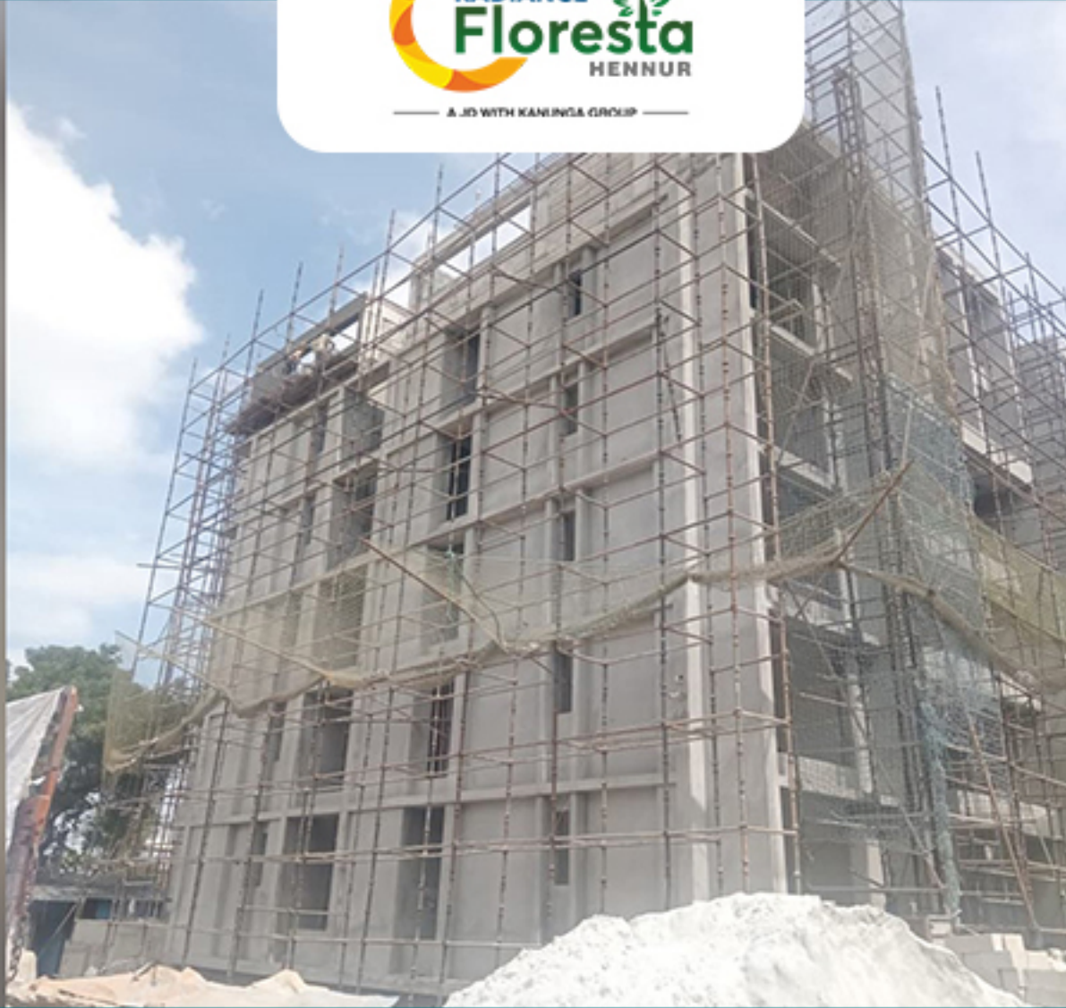
A-BLOCK WEST SIDE EXTERNAL PLASTERING
