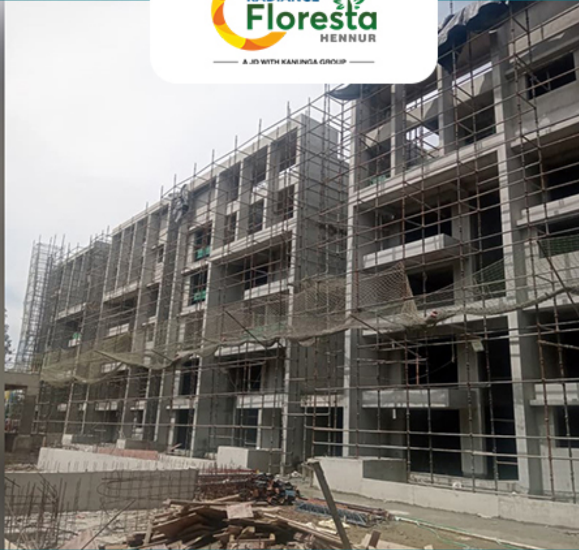
A-BLOCK CLUSTER-01, 02 SOUTH SIDE EXTERNAL PLASTERING
