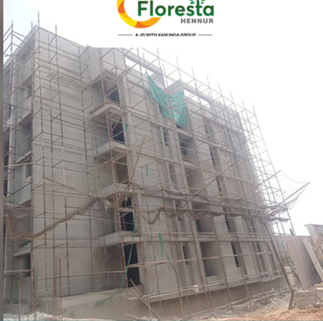
B-BLOCK WEST SIDE EXTERNAL PLASTERING
