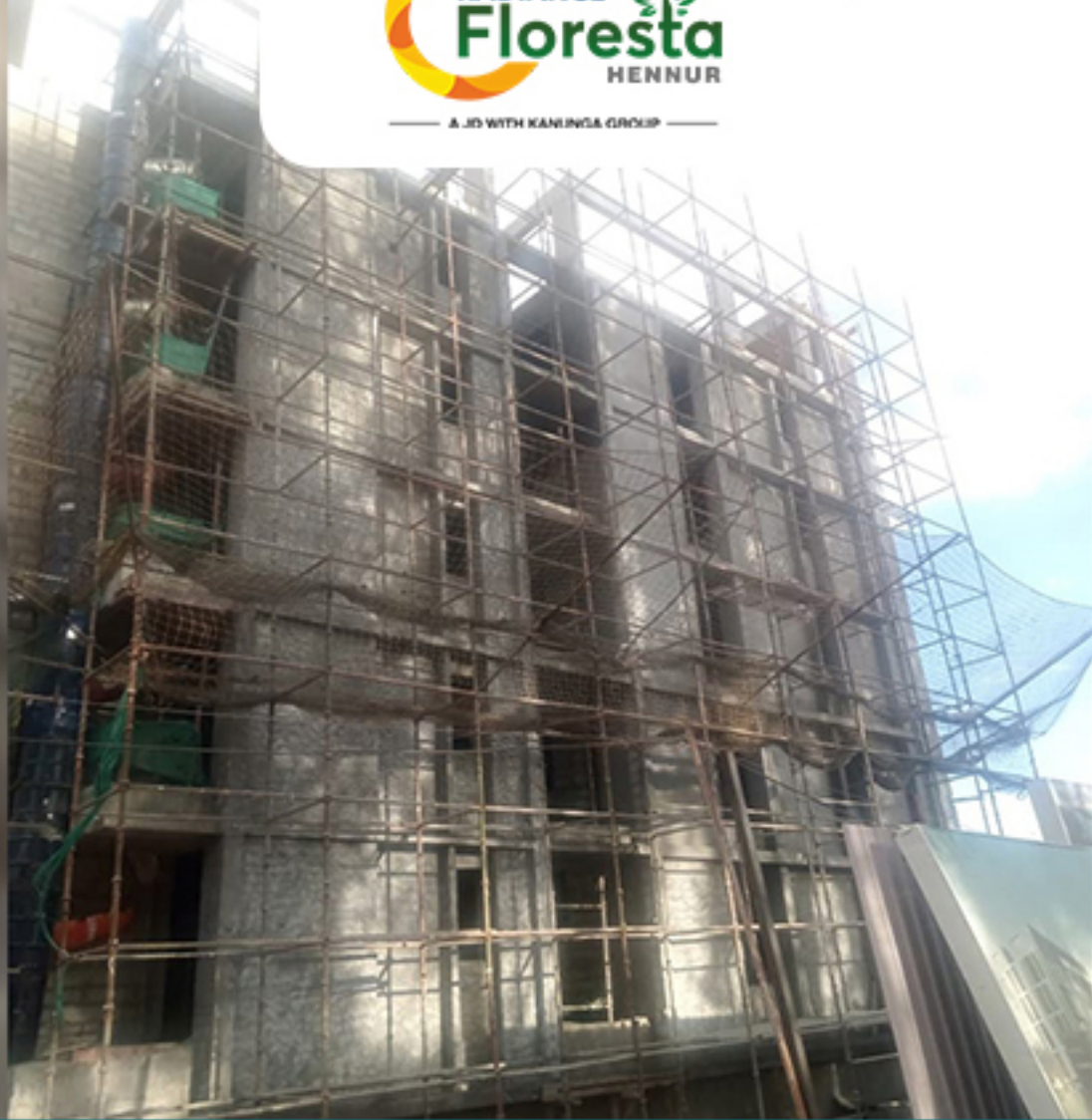
B-BLOCK WEST SIDE EXTERNAL PLASTERING IN PROGRESS
