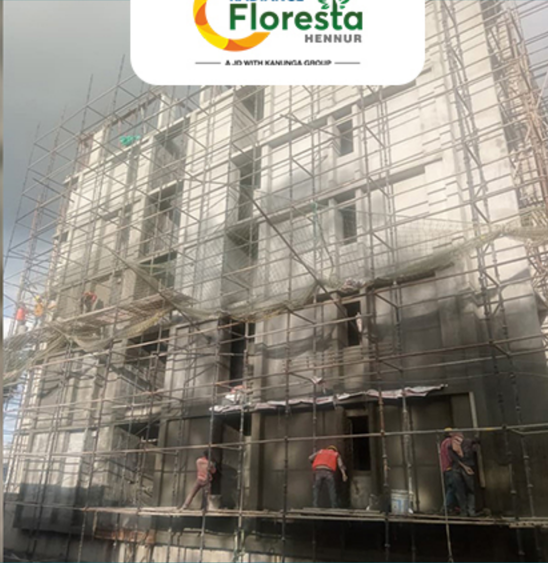
A-BLOCK WEST SIDE EXTERNAL PLASTERING WORK IN PROGRESS
