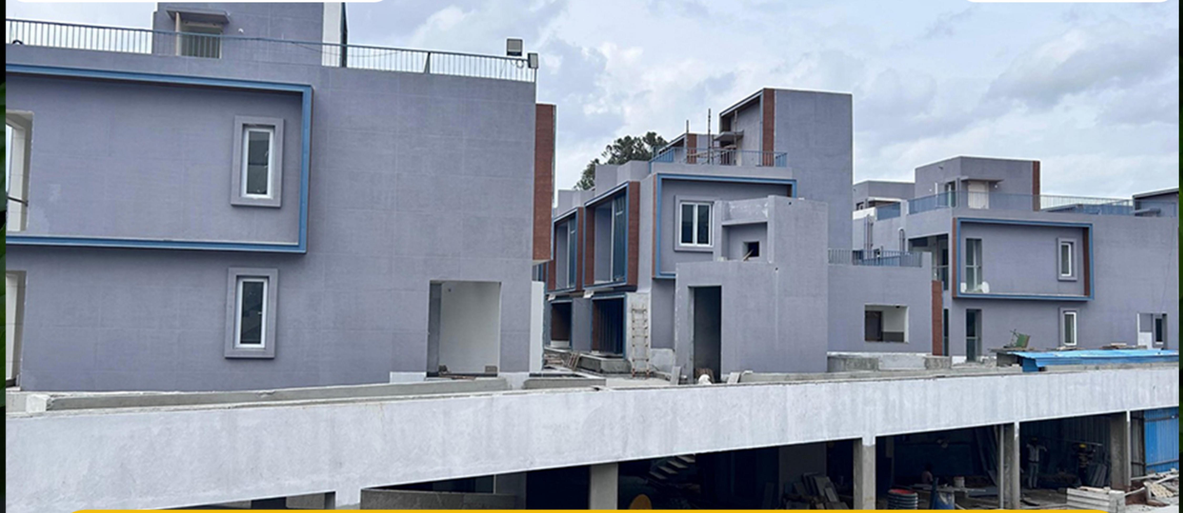
ROW HOUSE - BLOCK B - 1st COAT PAINT UNDER PROGRESS
