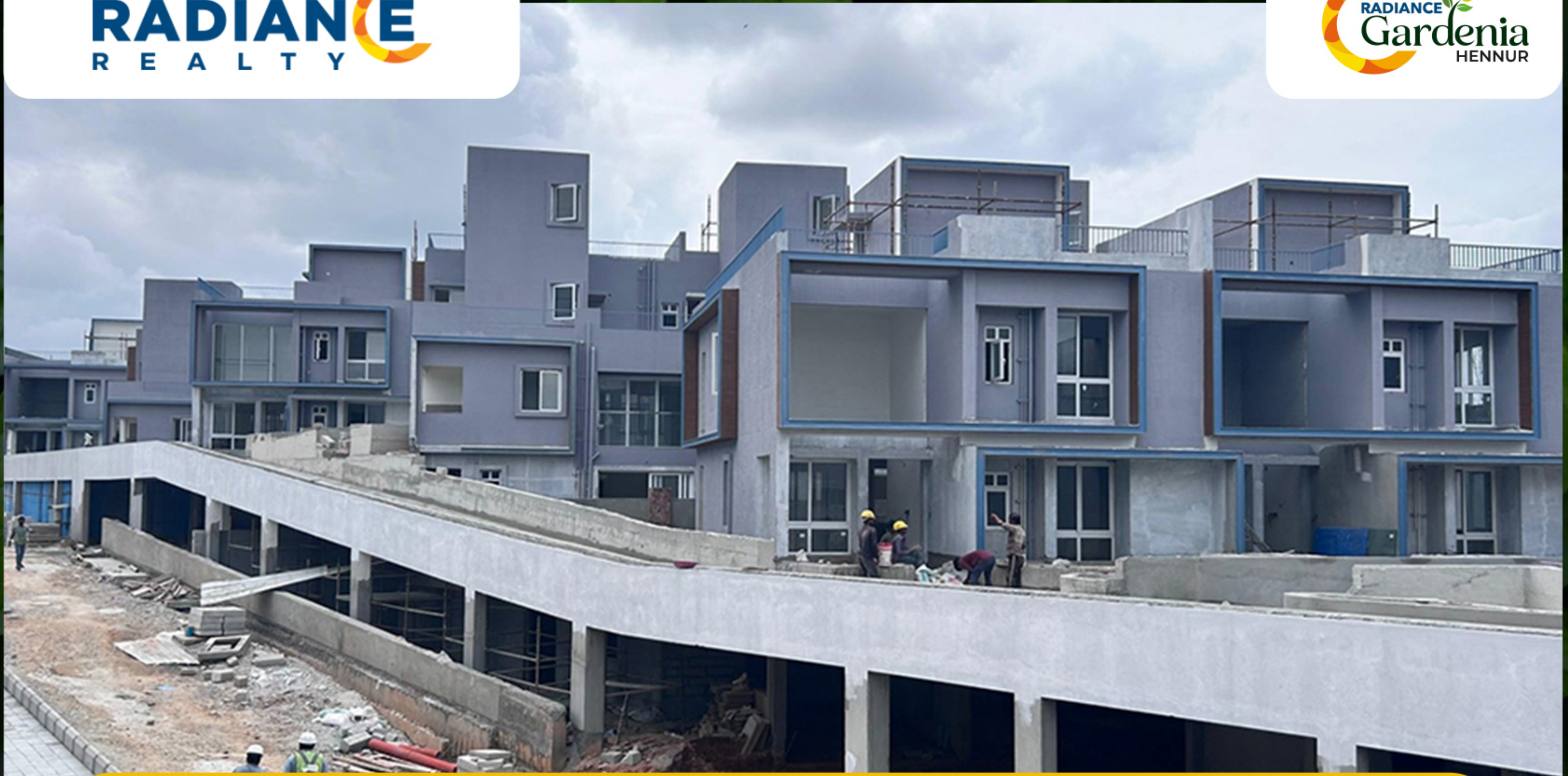
ROW HOUSE - BLOCK C - 1st COAT PAINT UNDER PROGRESS
