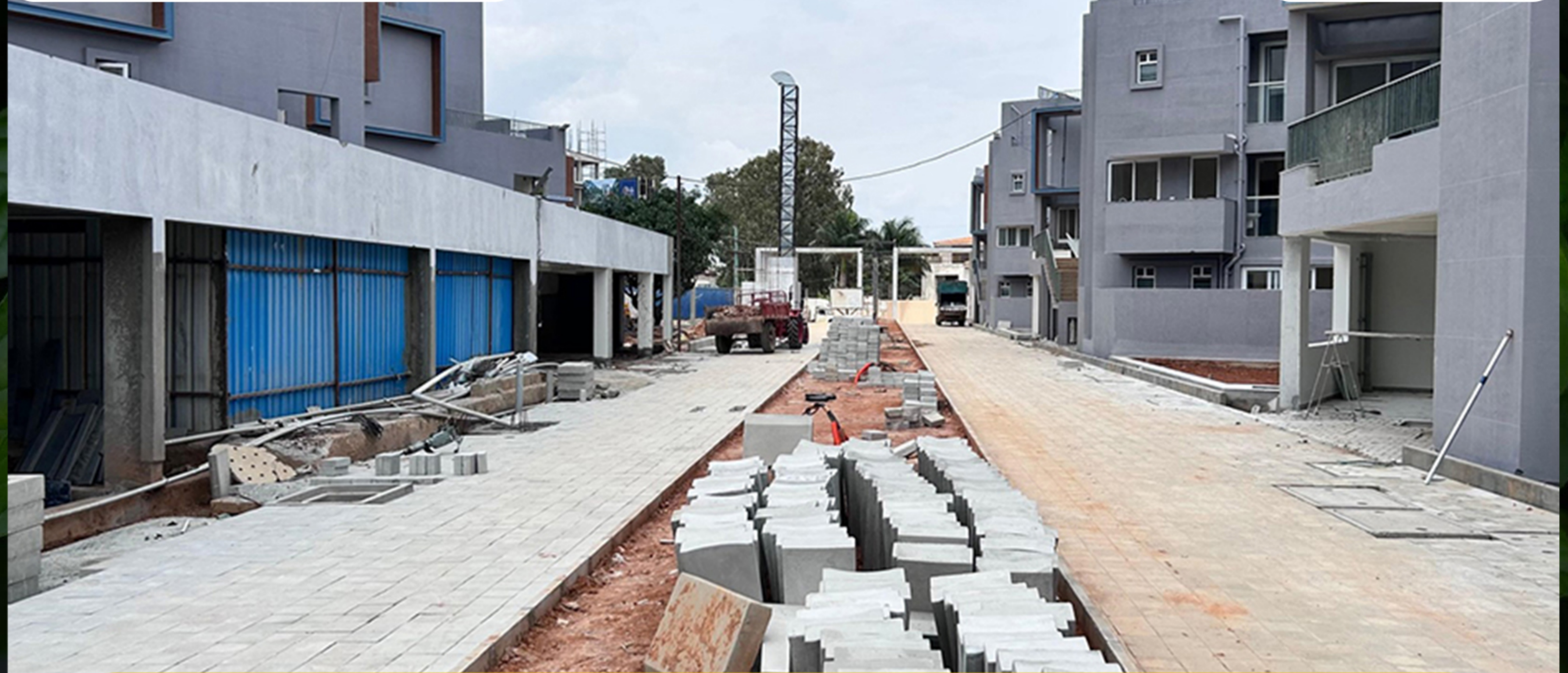
ROW HOUSE - PAVER LAYING WORK UNDER PROGRESS
