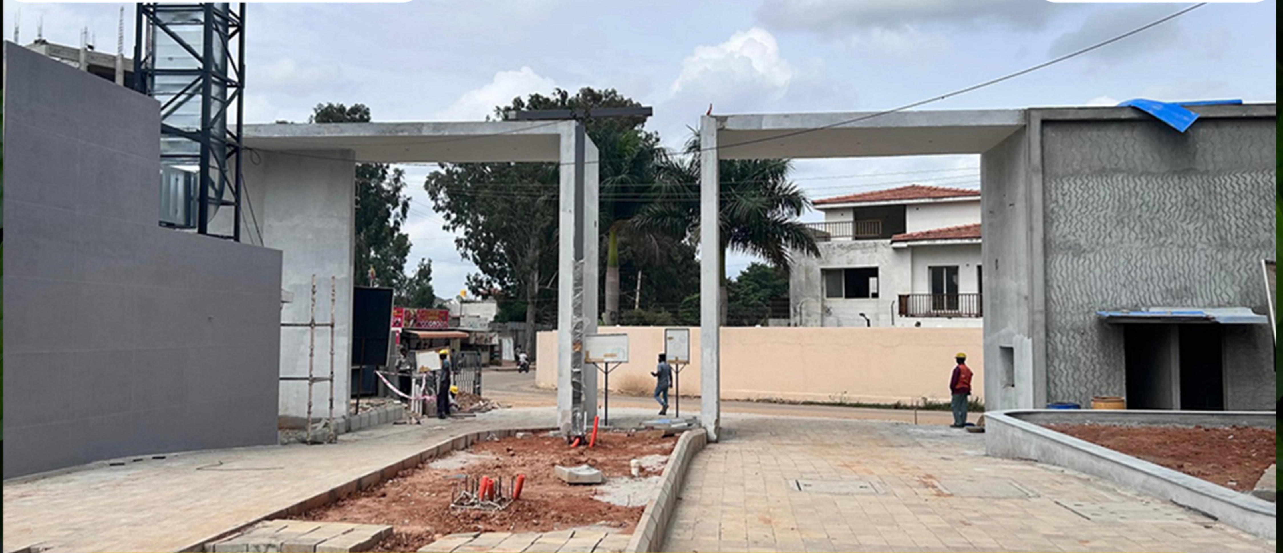
ENTRY PORTAL - FINISHING WORK UNDER PROGRESS
