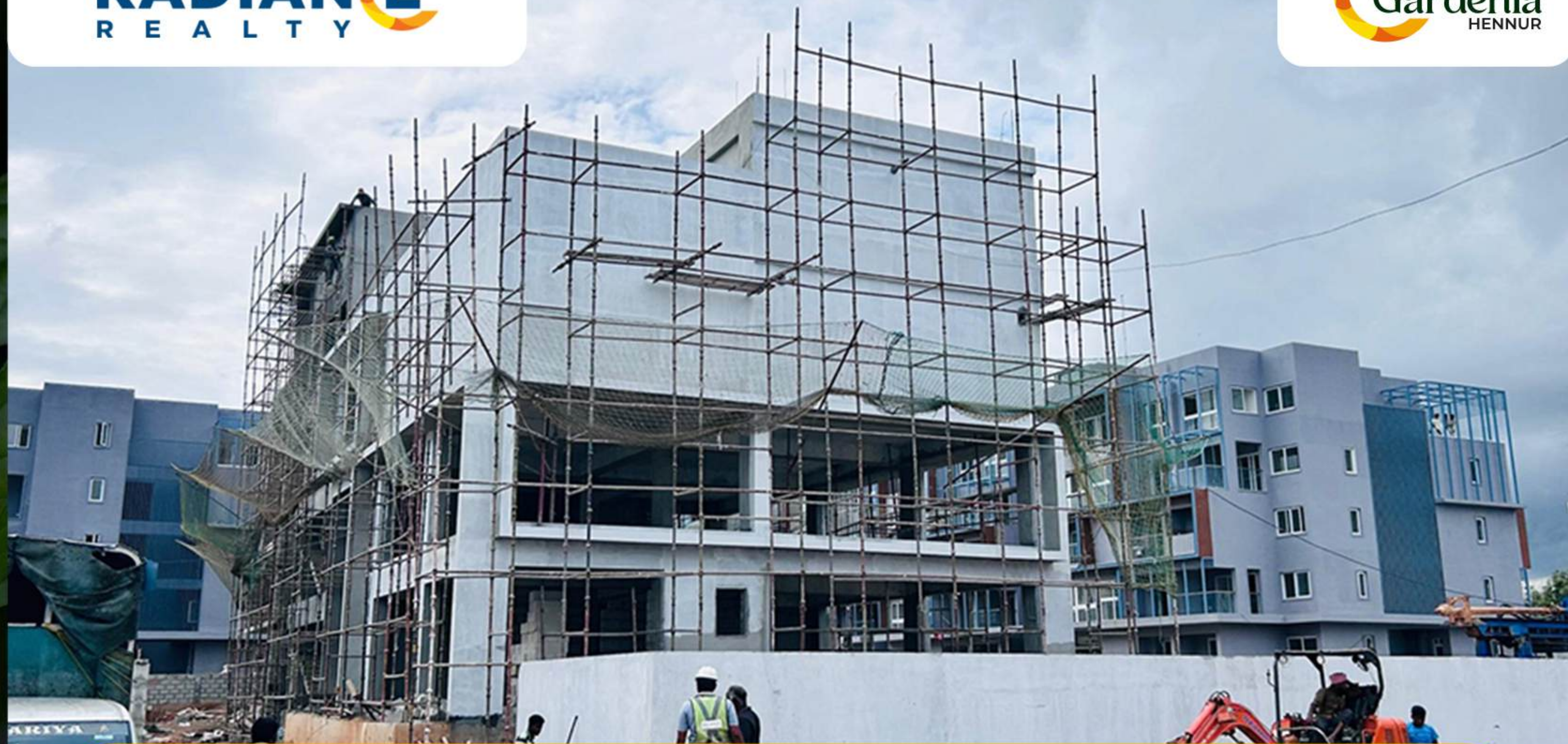
CLUB HOUSE - EAST SIDE
