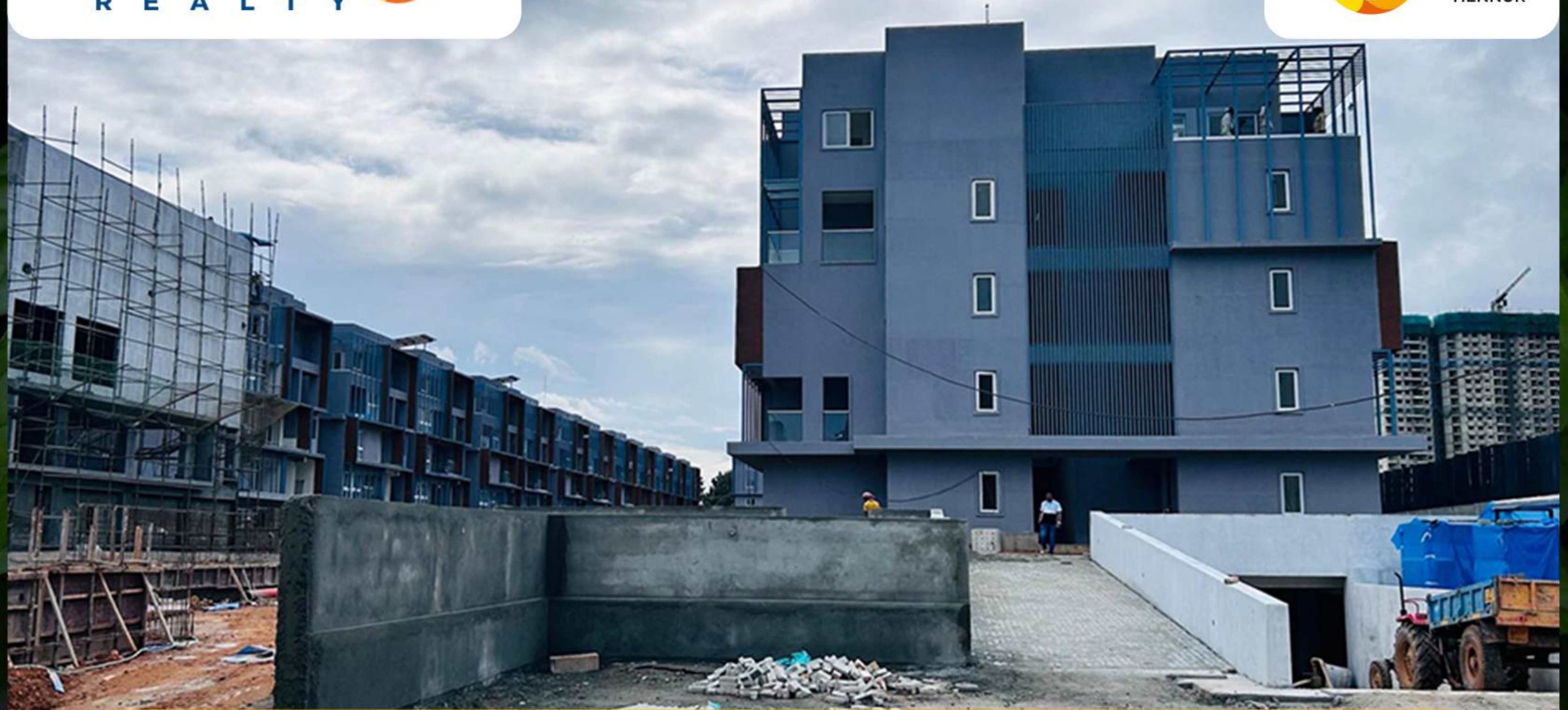
VILLAMENT- BLOCK F ENTRY RAMP
