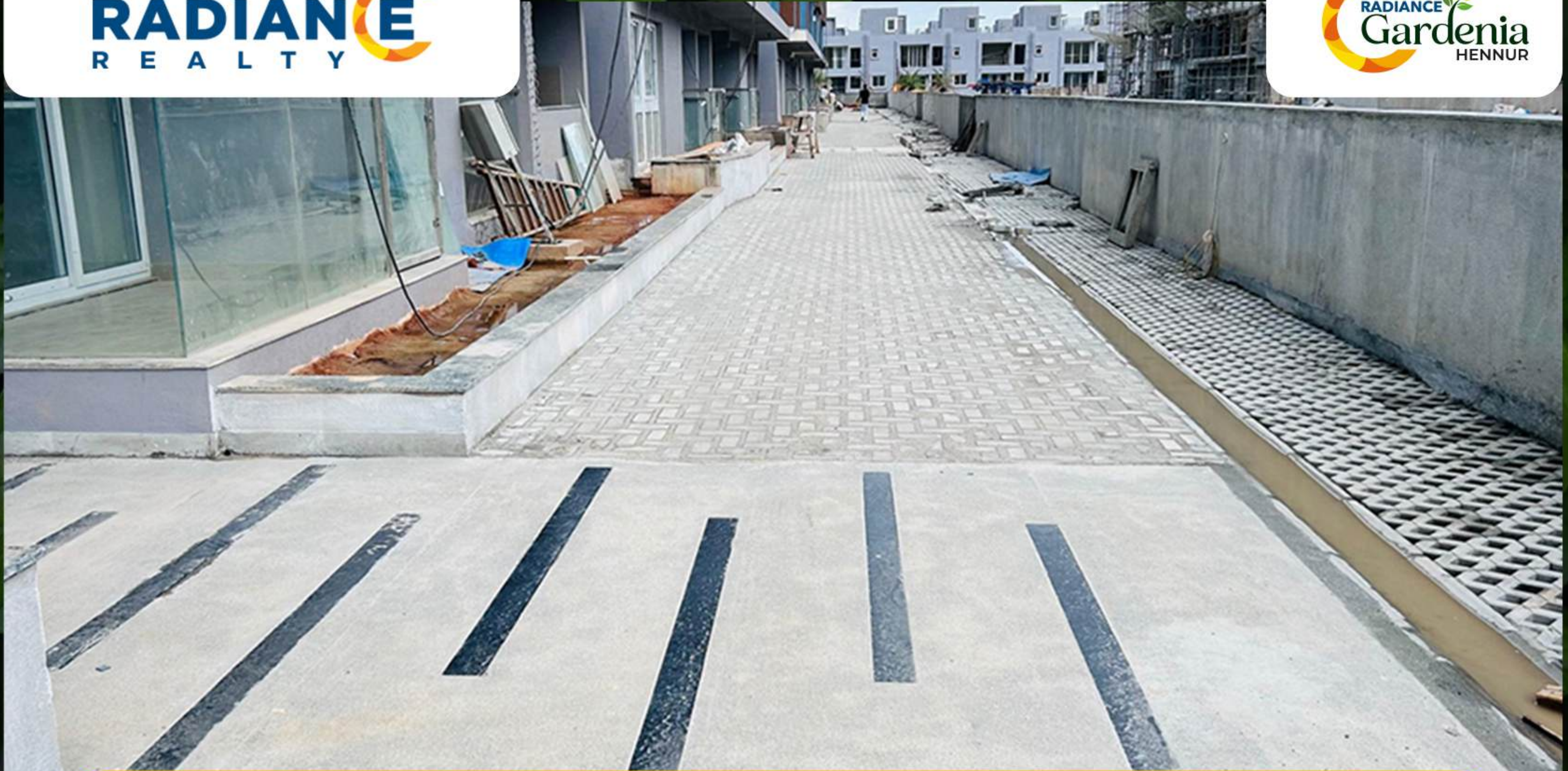
VILLAMENT- BLOCK F – SOUTH SIDE PODIUM
