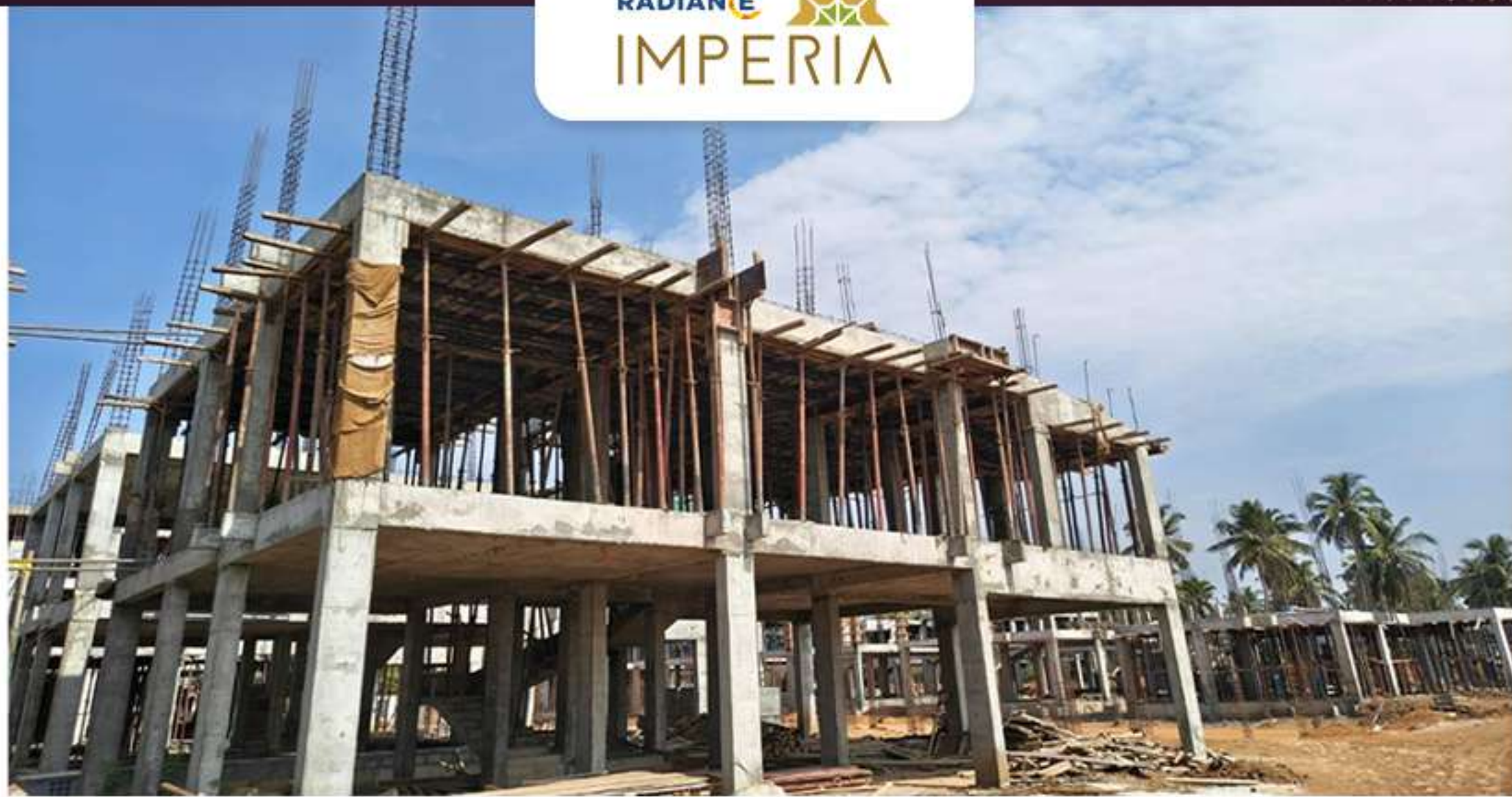
Villa- 65 2nd Floor Column Work in Progress
