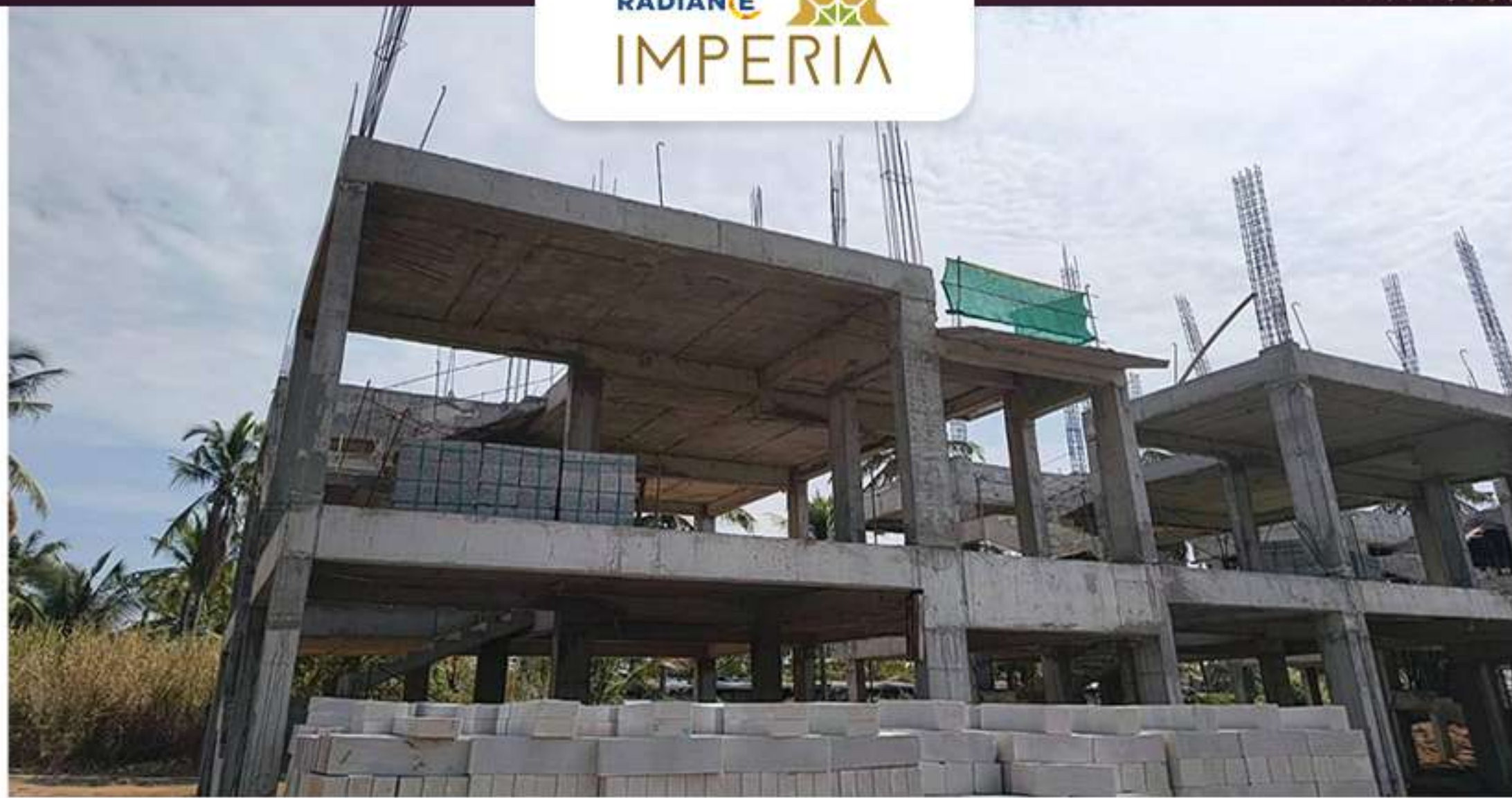
Villas-88 2nd Floor Column Work in Progress
