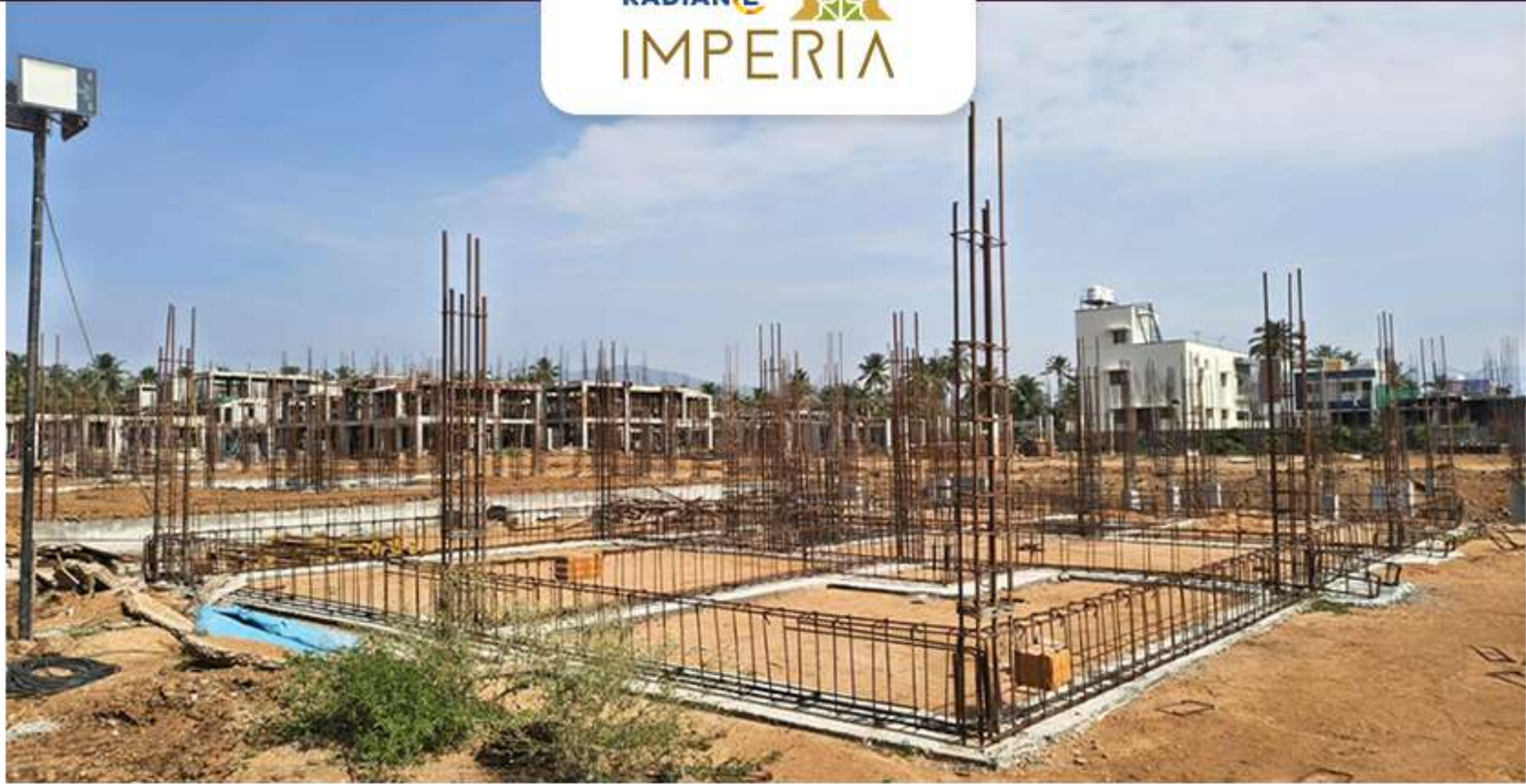
Villa 28 Plinth Beam Reinforcement Work in Progress
