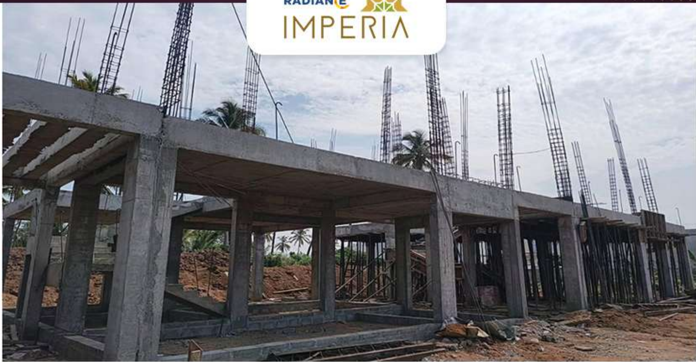
Villas- 96 1st Floor Column Work in Progress
