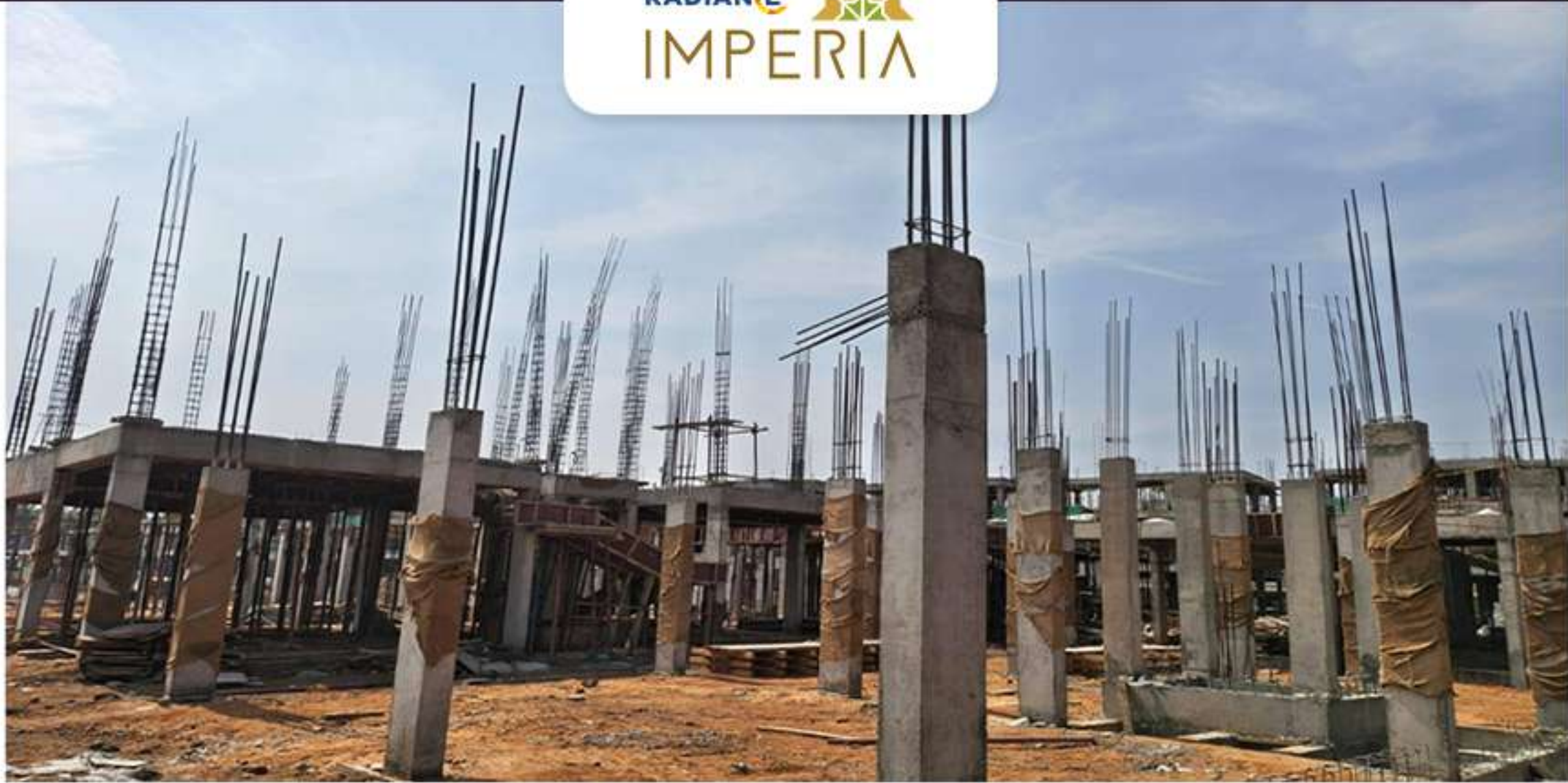
Villa-41 Ground Floor Roof Shuttering Work in Progress
