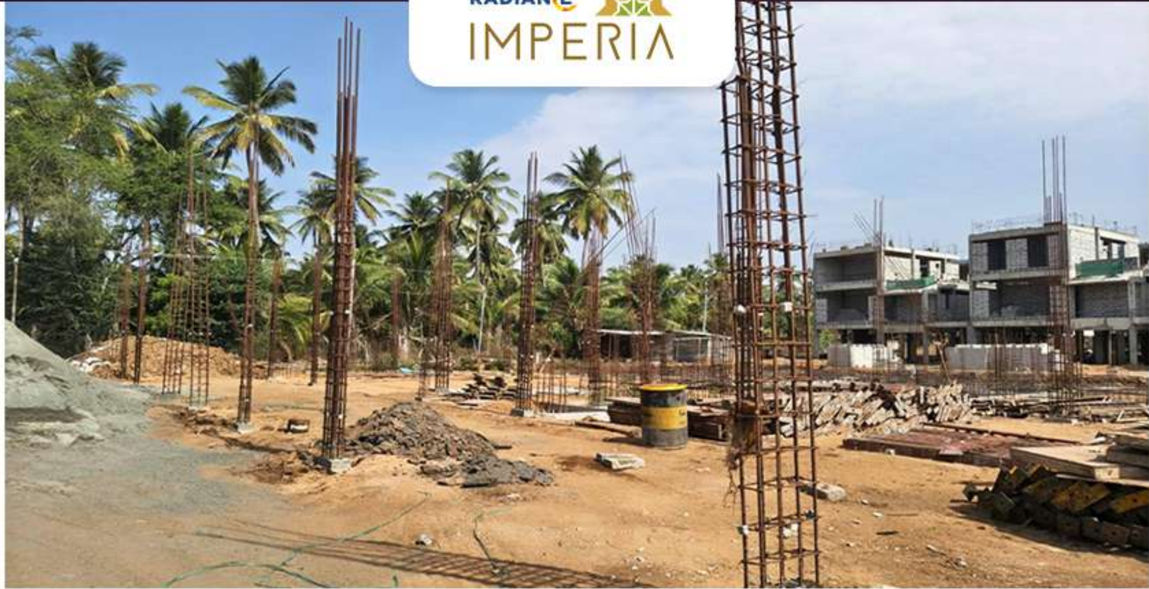
Villa 19 & 20 Ground Floor Column Work in Progress
