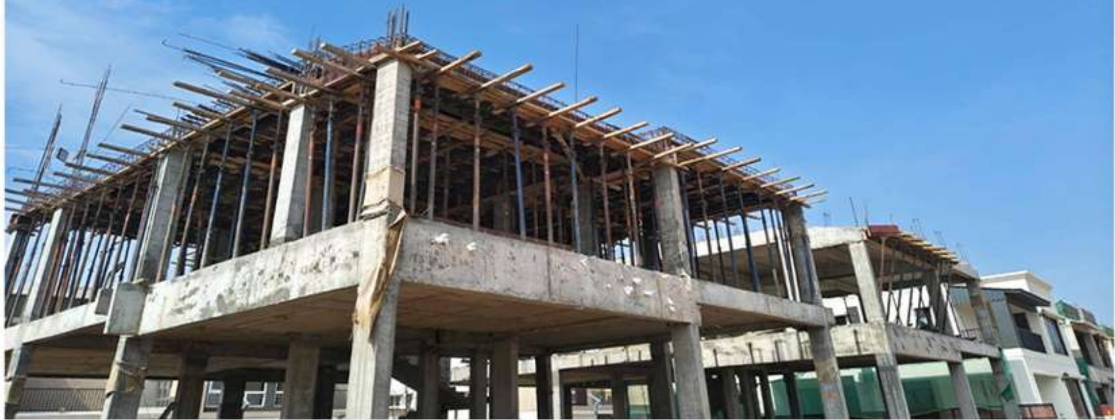
Villa no. 3 first floor Slab Shuttering Work in Progress
