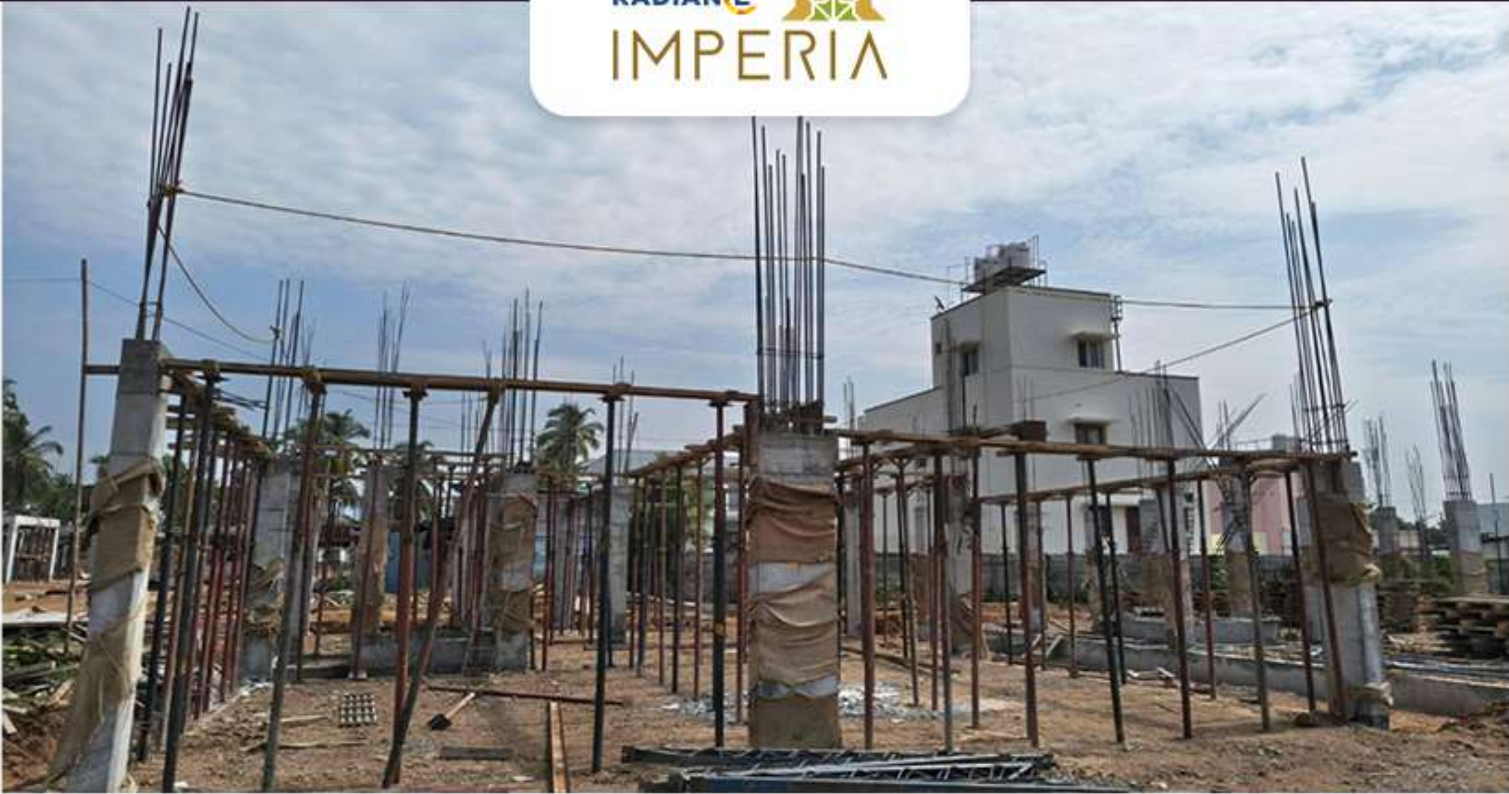
Villas- 52 Ground Floor Roof Slab Shuttering work in progress
