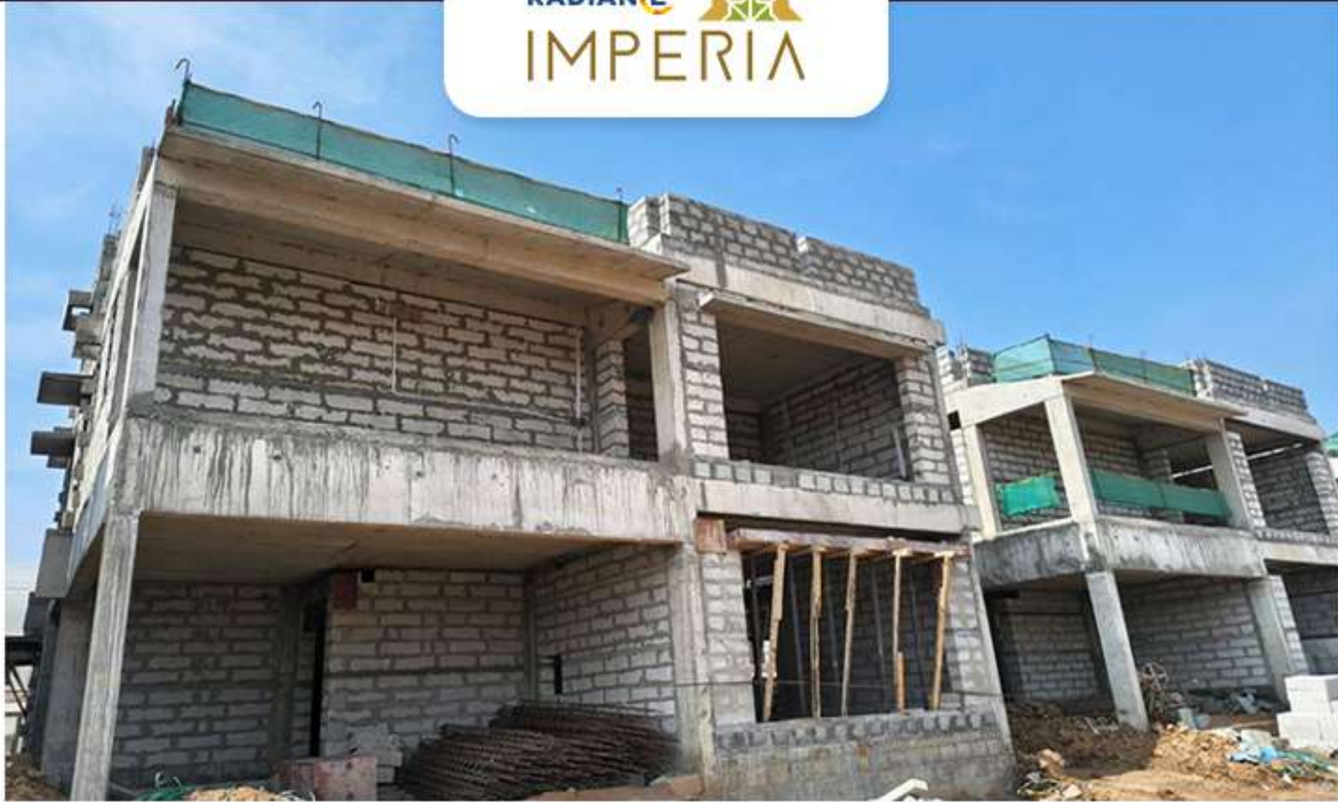
Villa 7 Block Work in Progress
