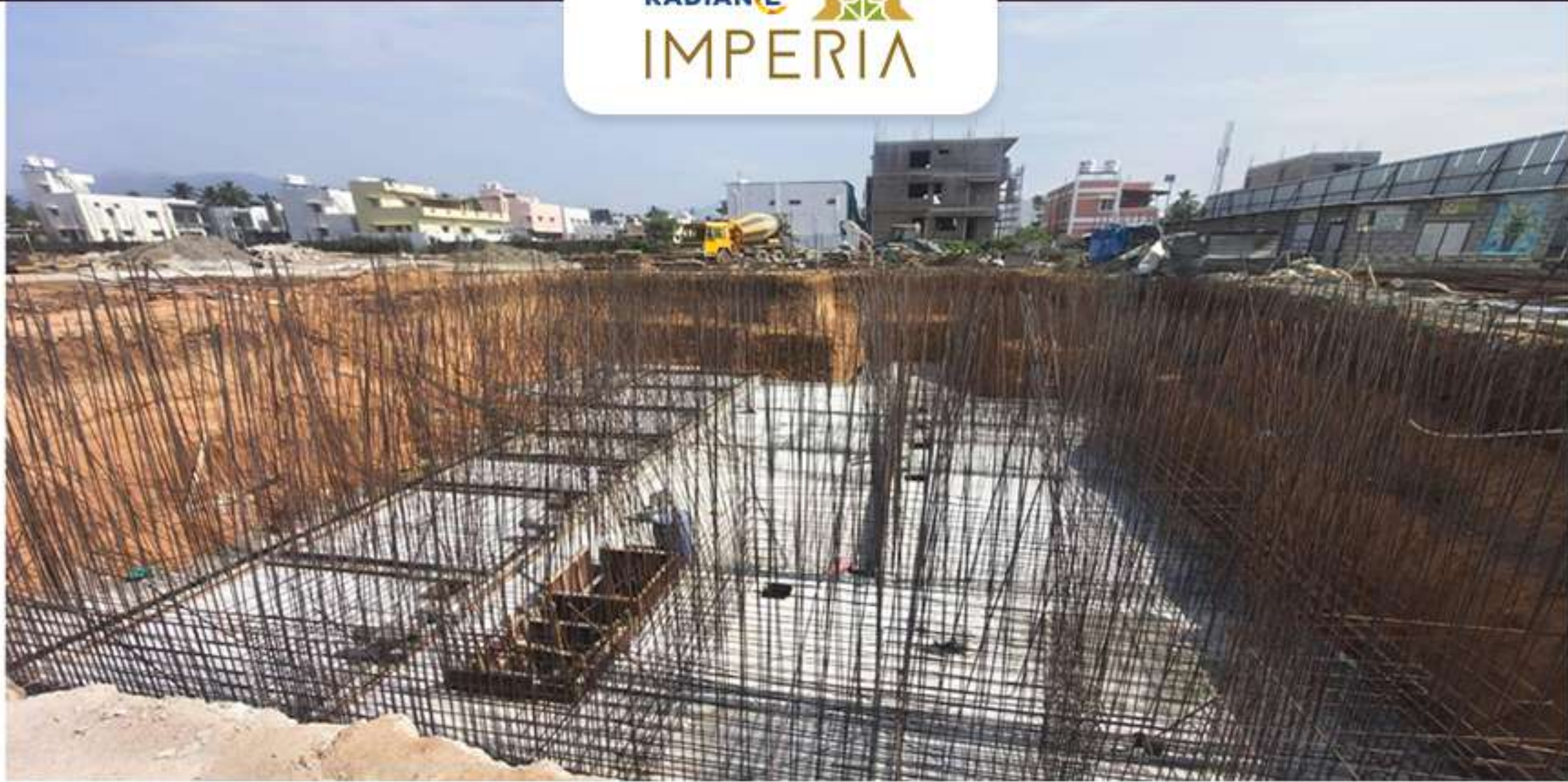
STP & WTP Wall Reinforcement Work in Progress
