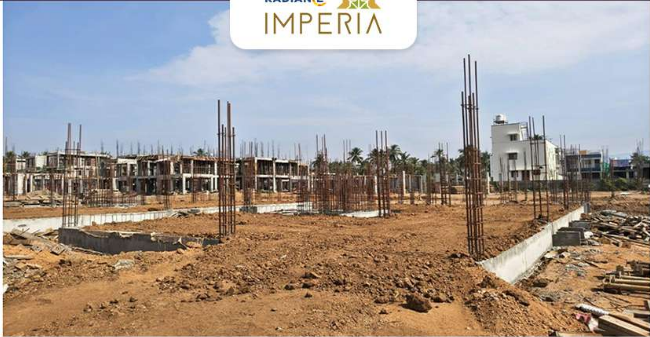
Villa 27 Plinth Beam Level Soil Filling Work in Progress
