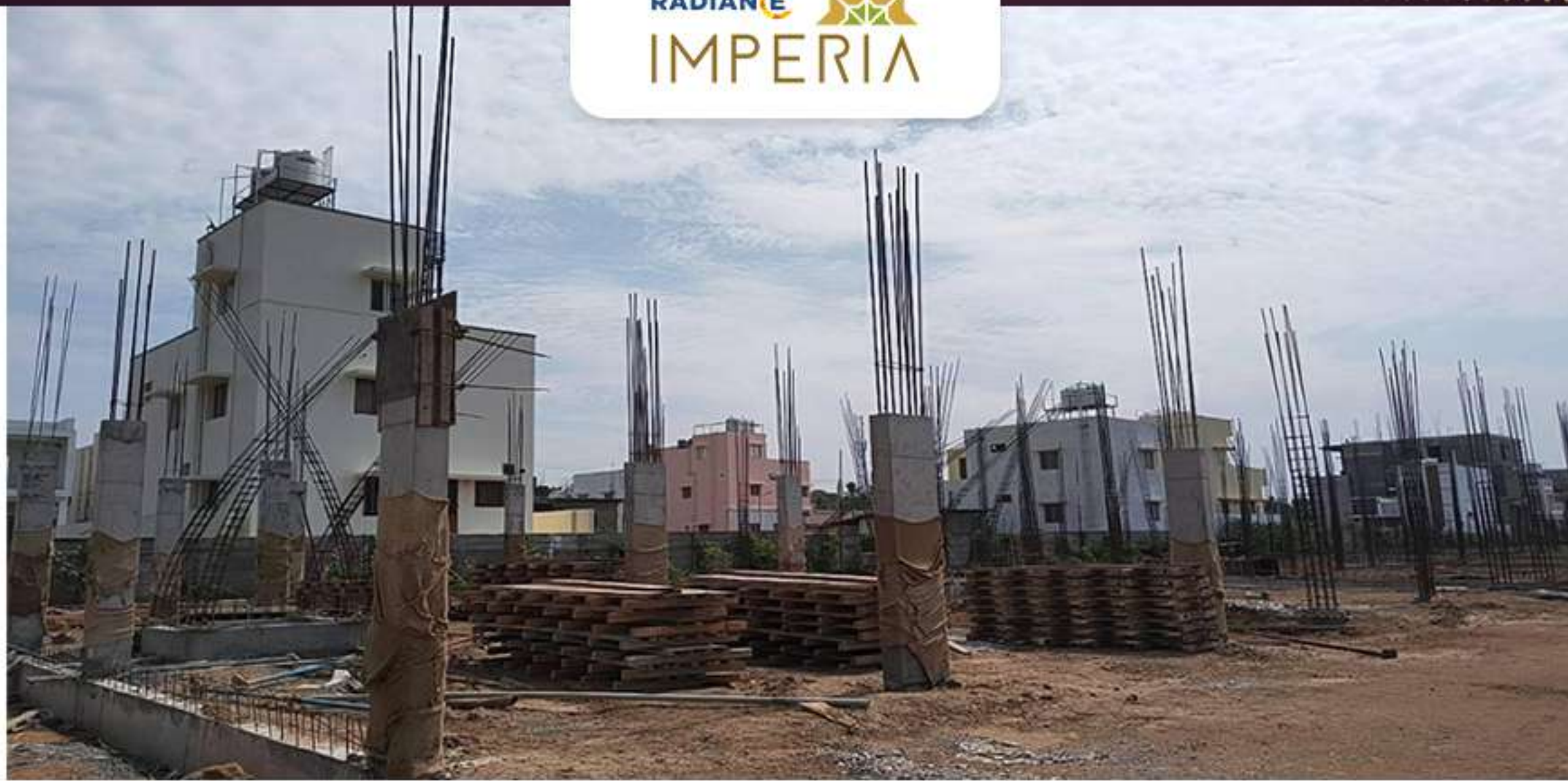
Villas- 54 Ground Floor Column Completed
