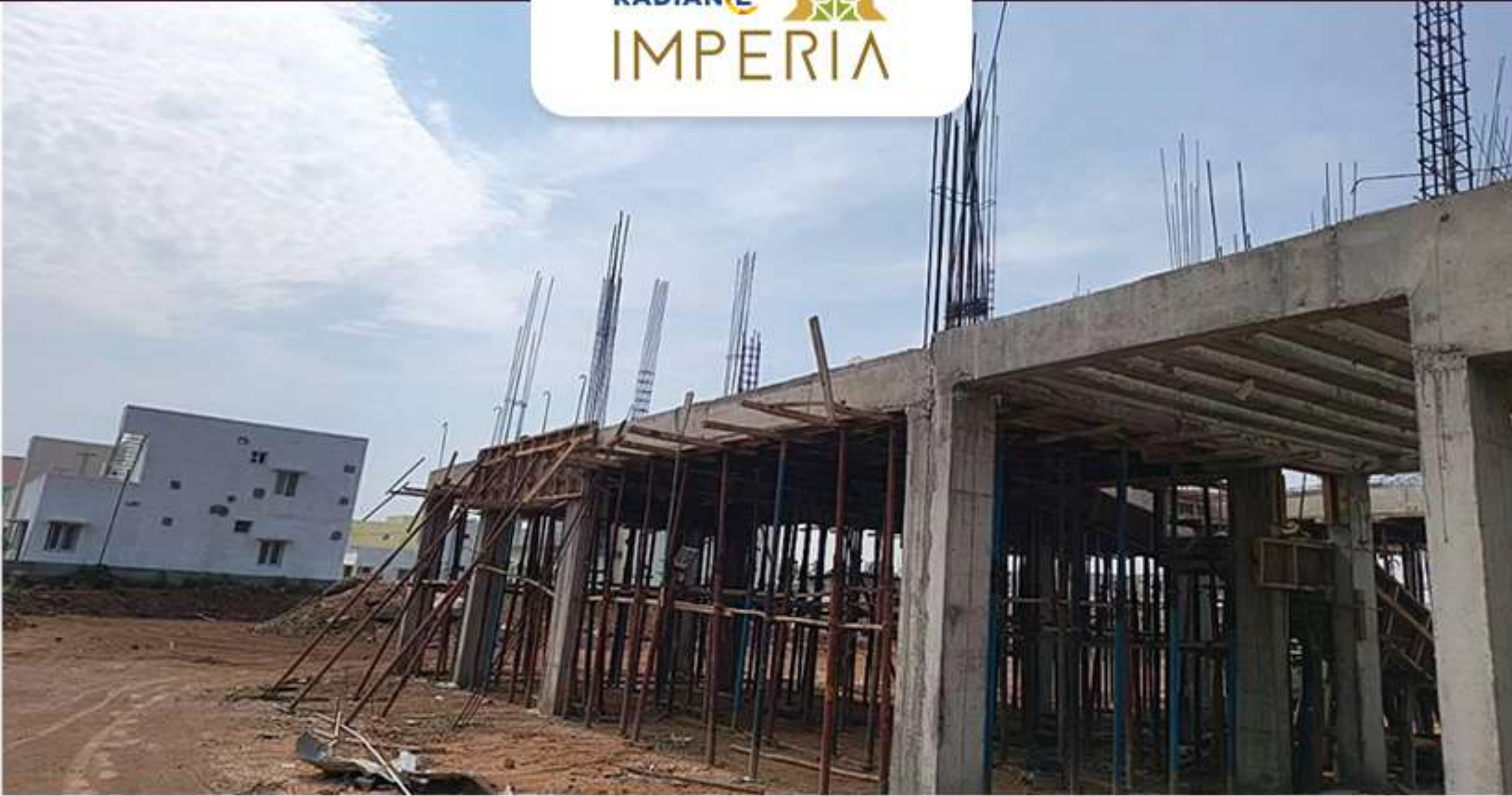
Villas- 81 1st Floor Column Work in Progress
