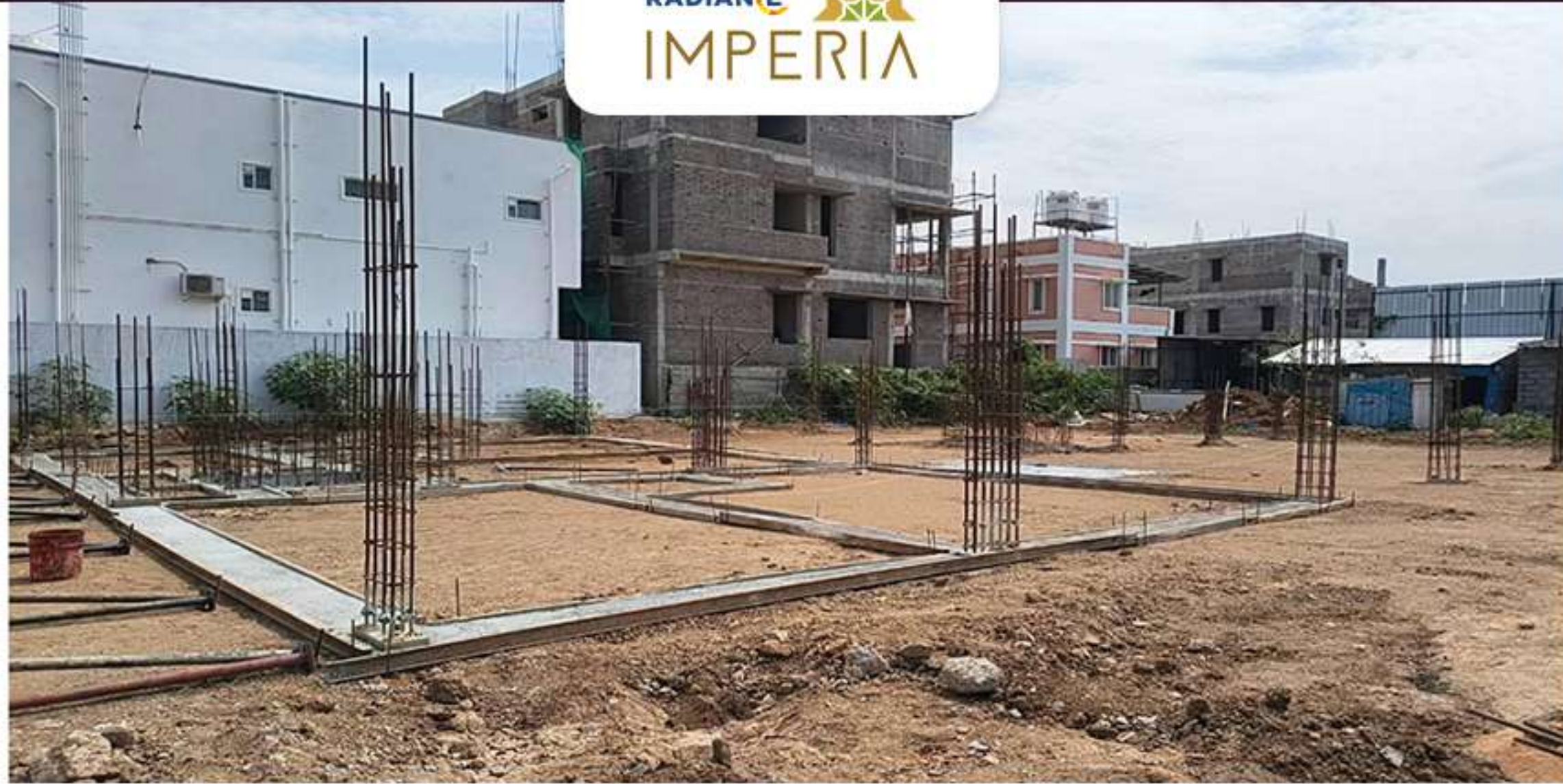
Villas- 63 Plinth Beam Shuttering Work in Progress
