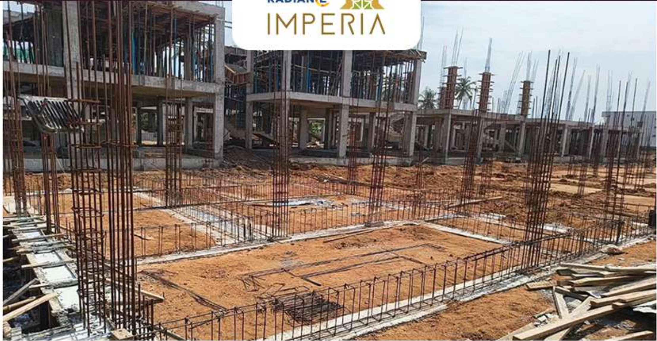
Villas-74 Plinth Beam Reinforcement Work in Progress
