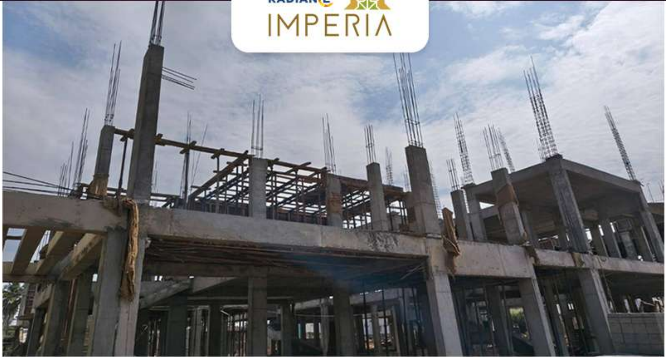
Villa-48 First Floor Roof Shuttering Work in Progress
