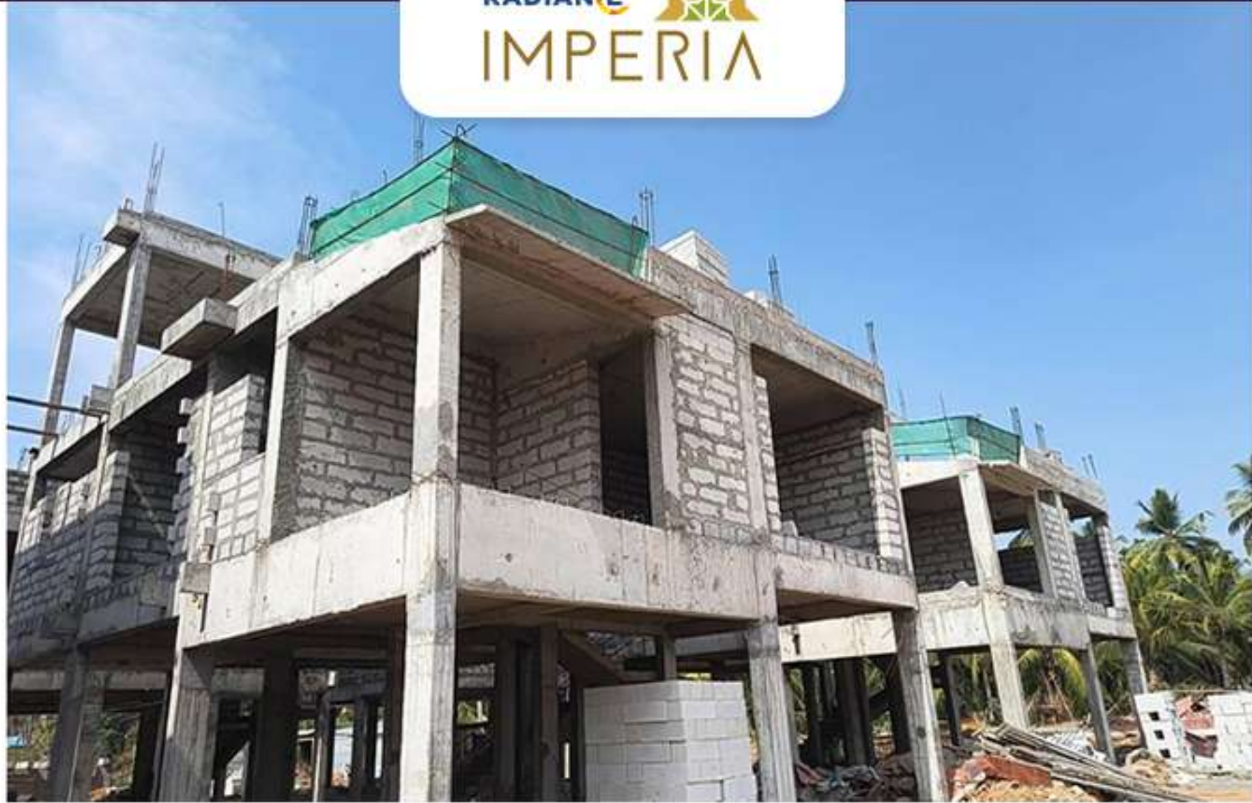
Villas-72 Block Work in Progress
