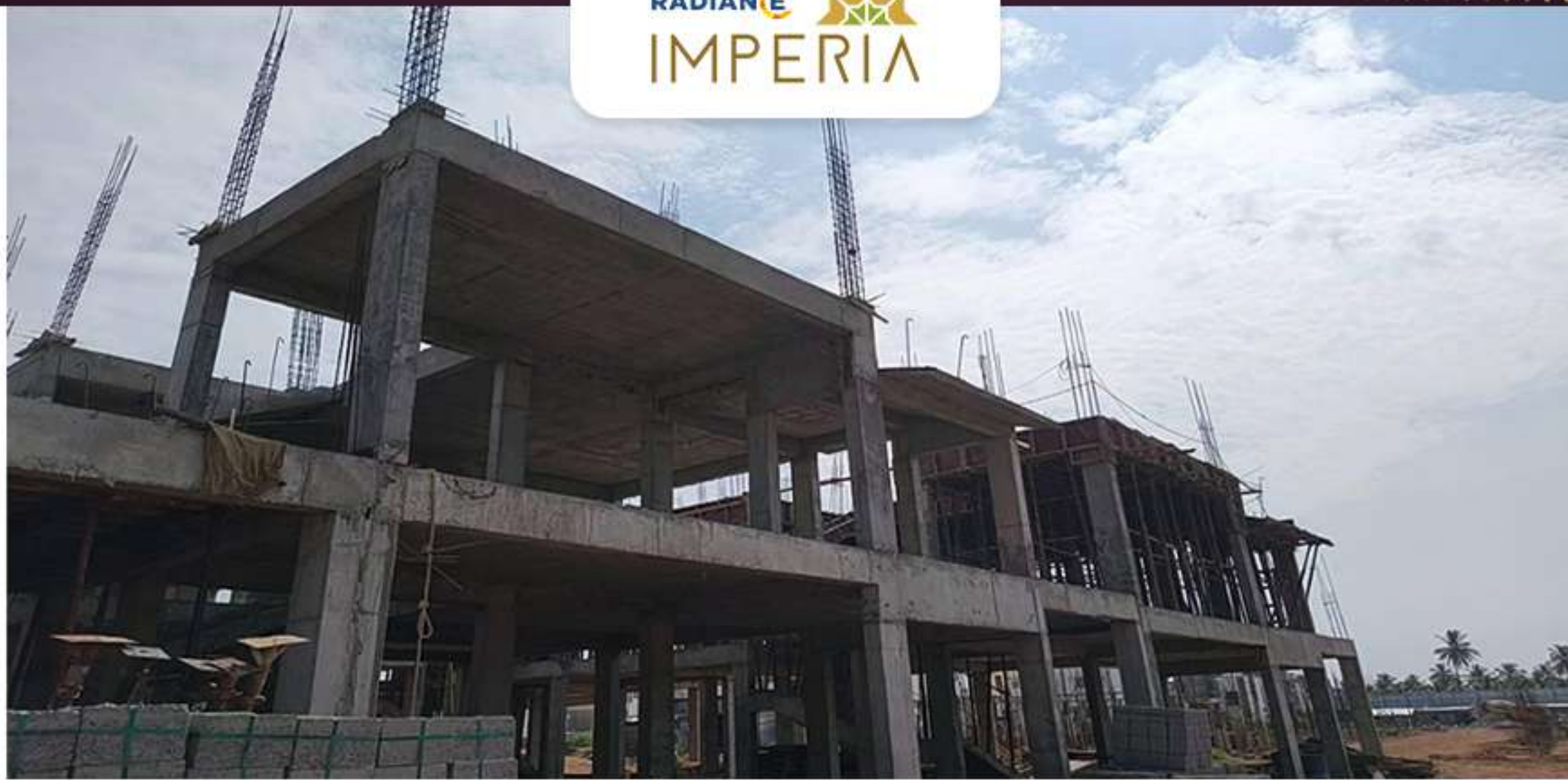
Villa-50 2nd Floor Column Work in Progress
