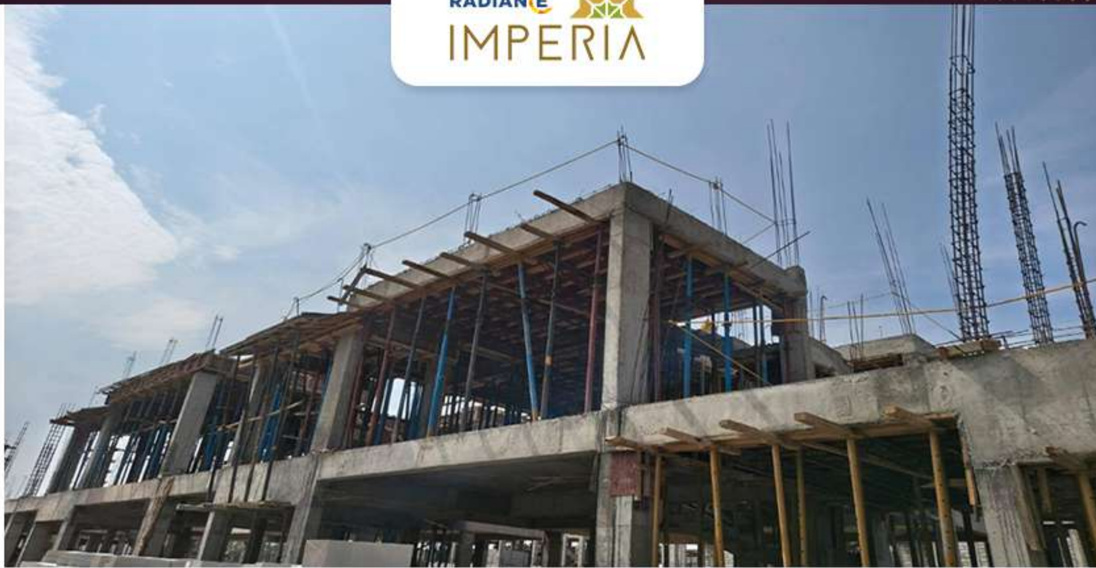
Villas- 86 First Floor Roof Slab Completed
