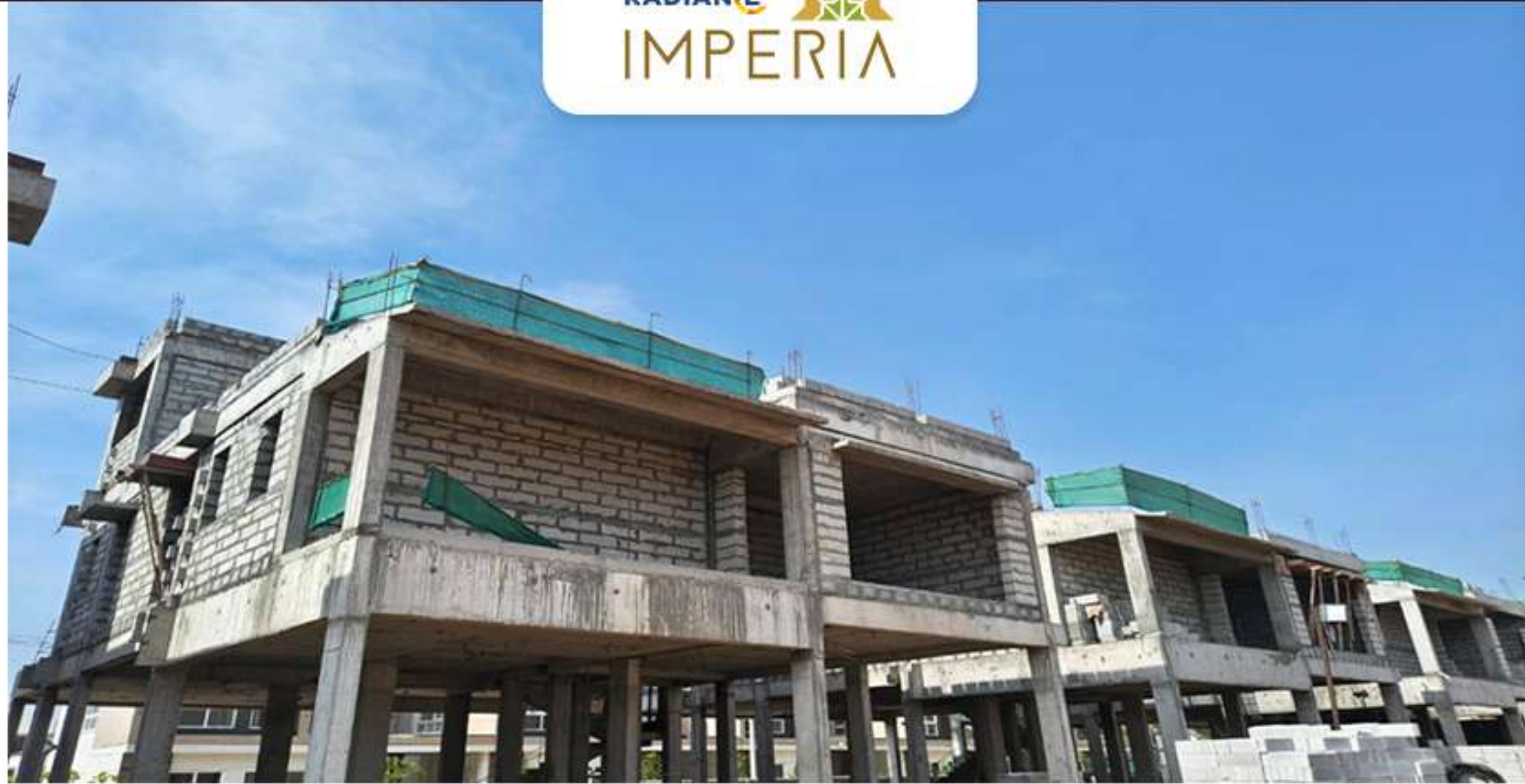
Villa 12 Block Work in Progress
