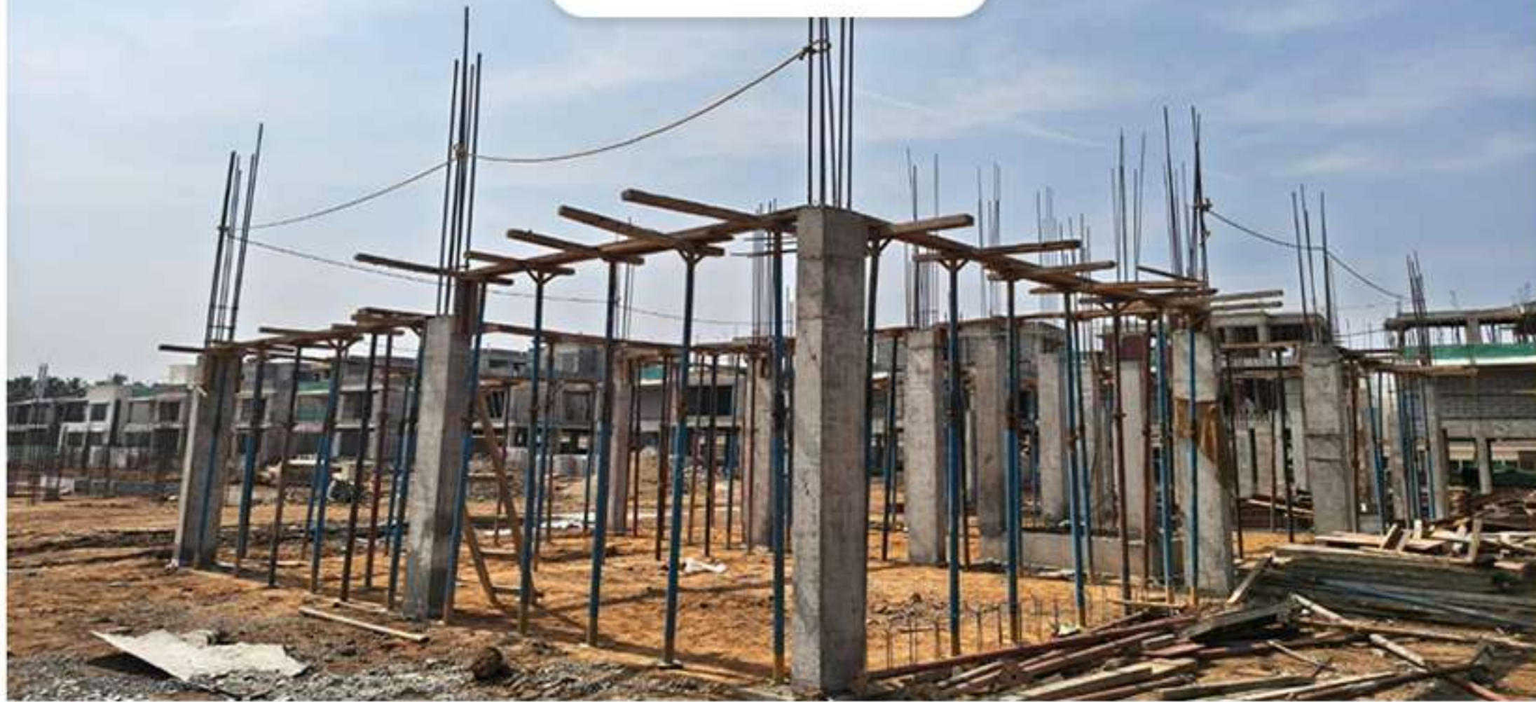
Villa-39 Ground Floor Roof Slab Shuttering Work in Progress
