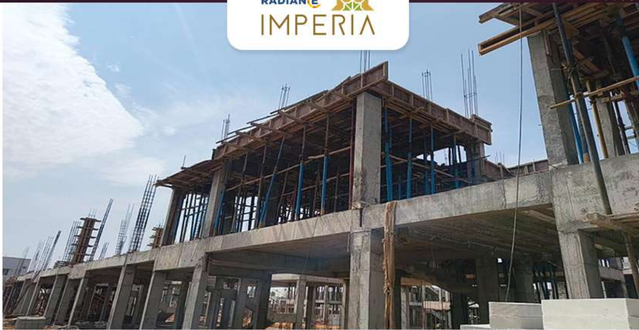
Villas- 84 First Floor Roof Slab Shuttering Work in progress
