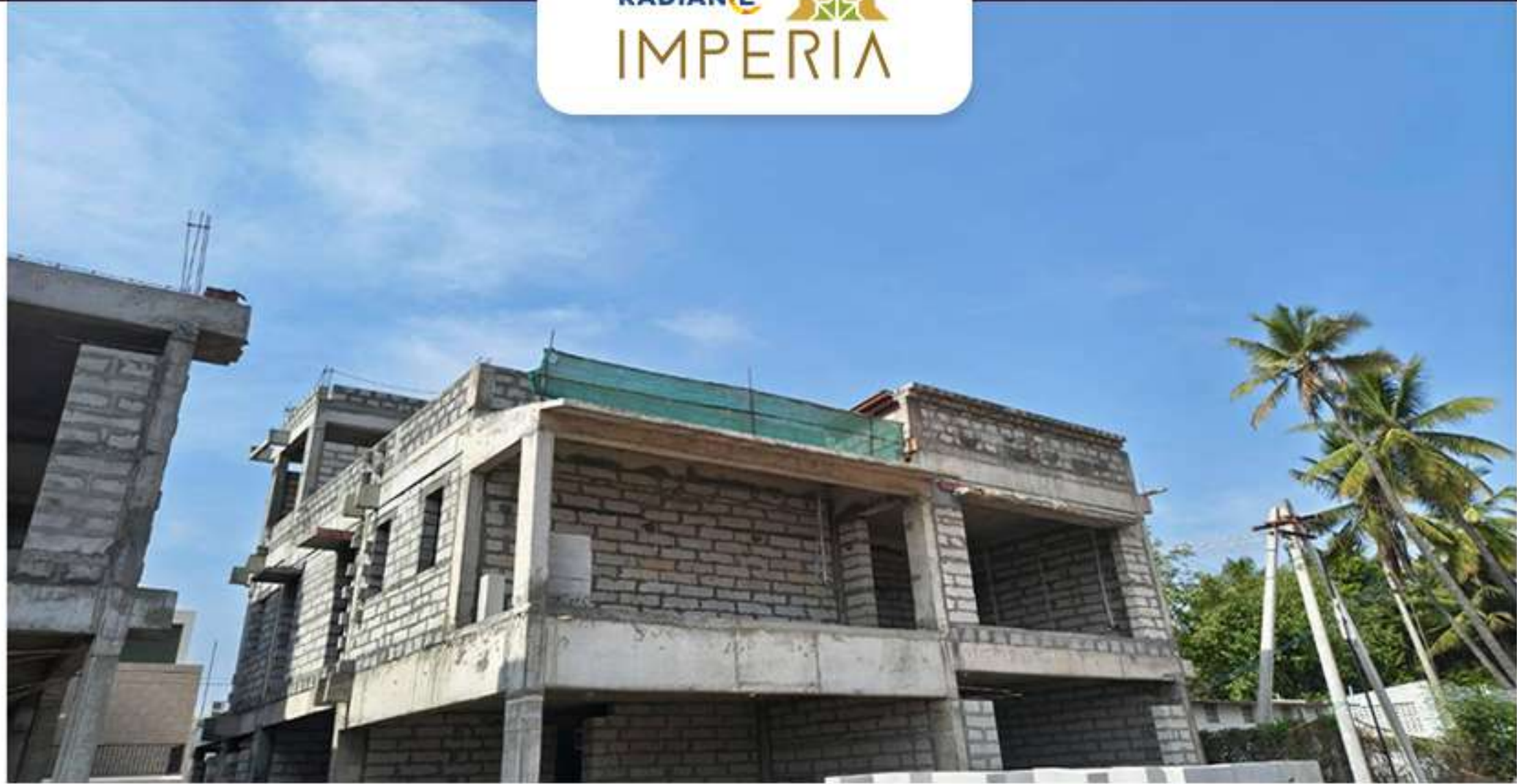
Villa 18 Block Work in Progress
