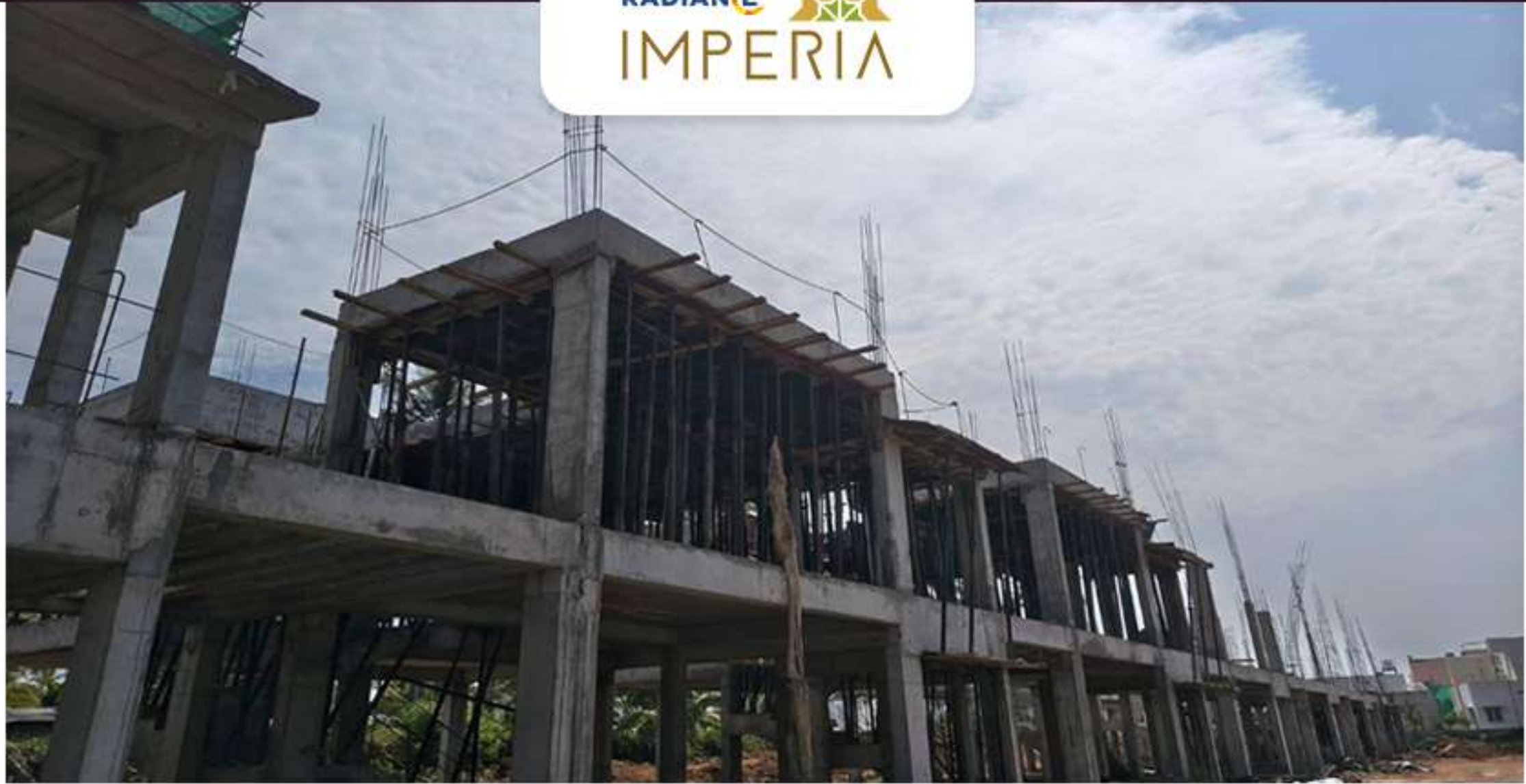
Villas- 91 First Floor Roof Slab Completed
