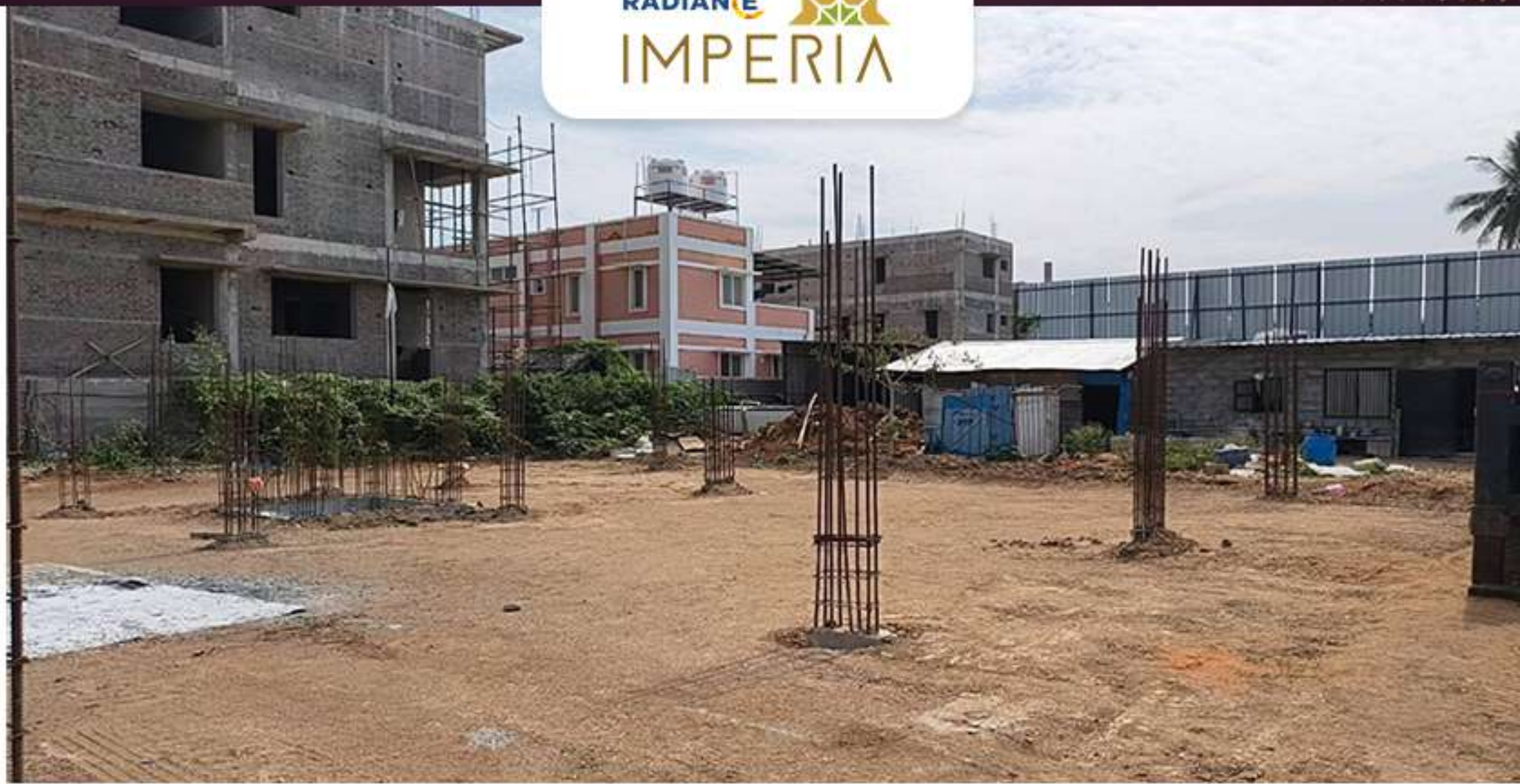
Villa 64: Plinth beam soil sectioning work in progress
