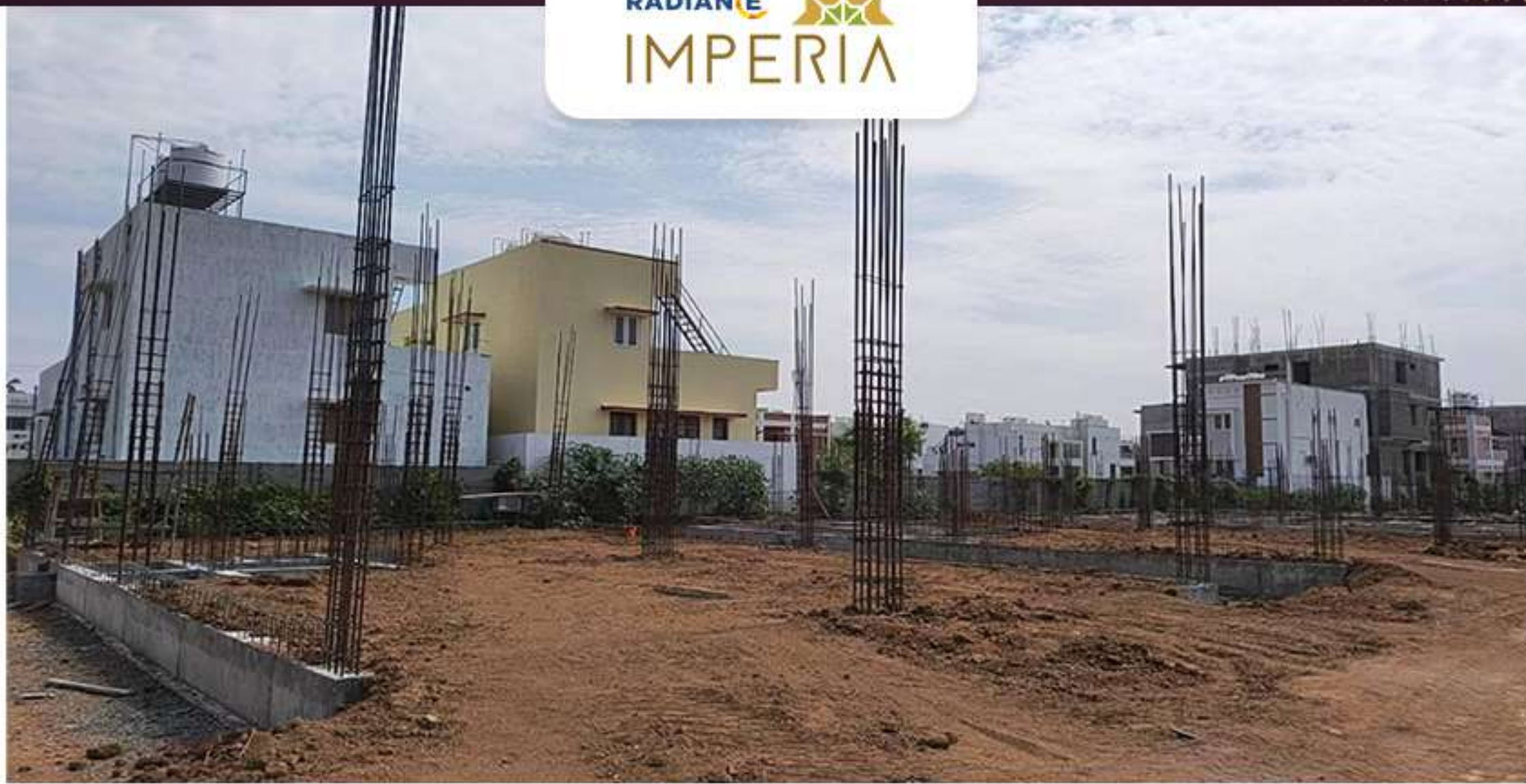
Villas- 59 Ground Floor Column Work in Progress
