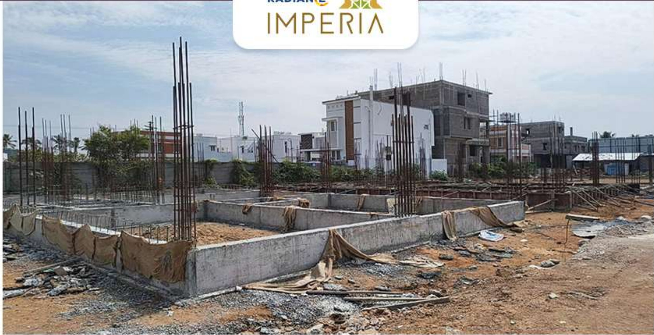
Villas- 61 Plinth Beam Completed
