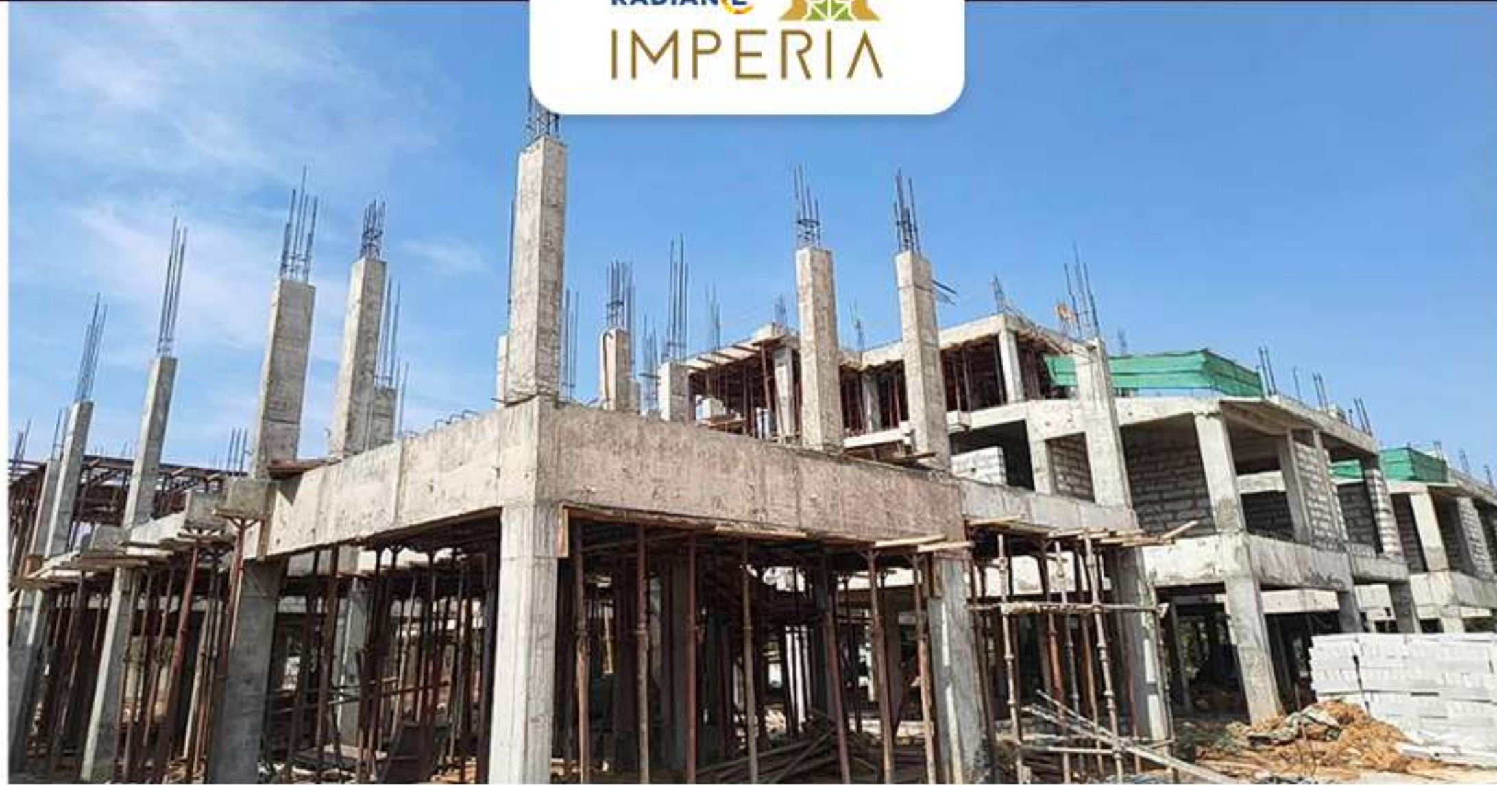
Villas-68 1st Floor Column Completed
