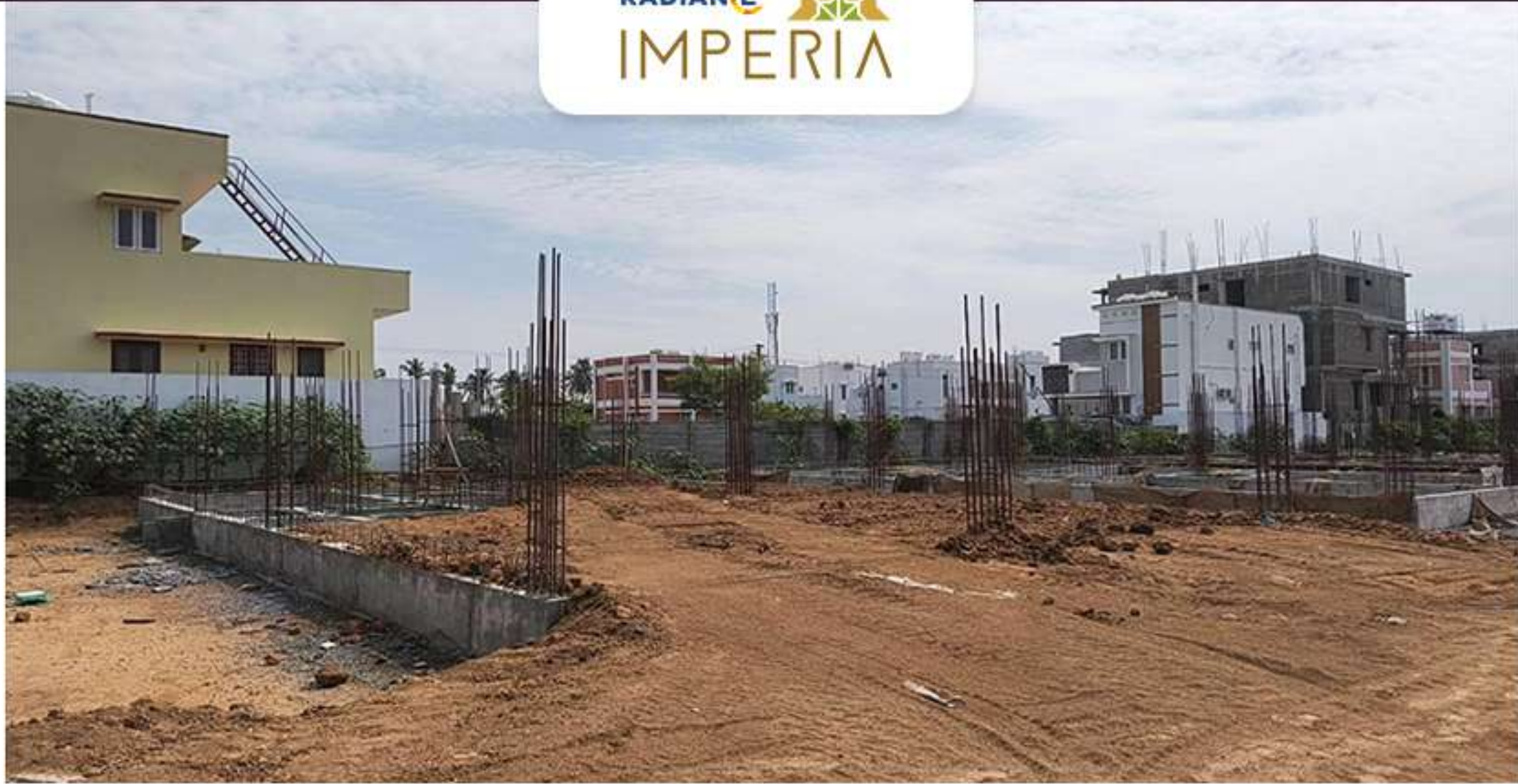
Villas- 60 Ground Floor Column Work in Progress
