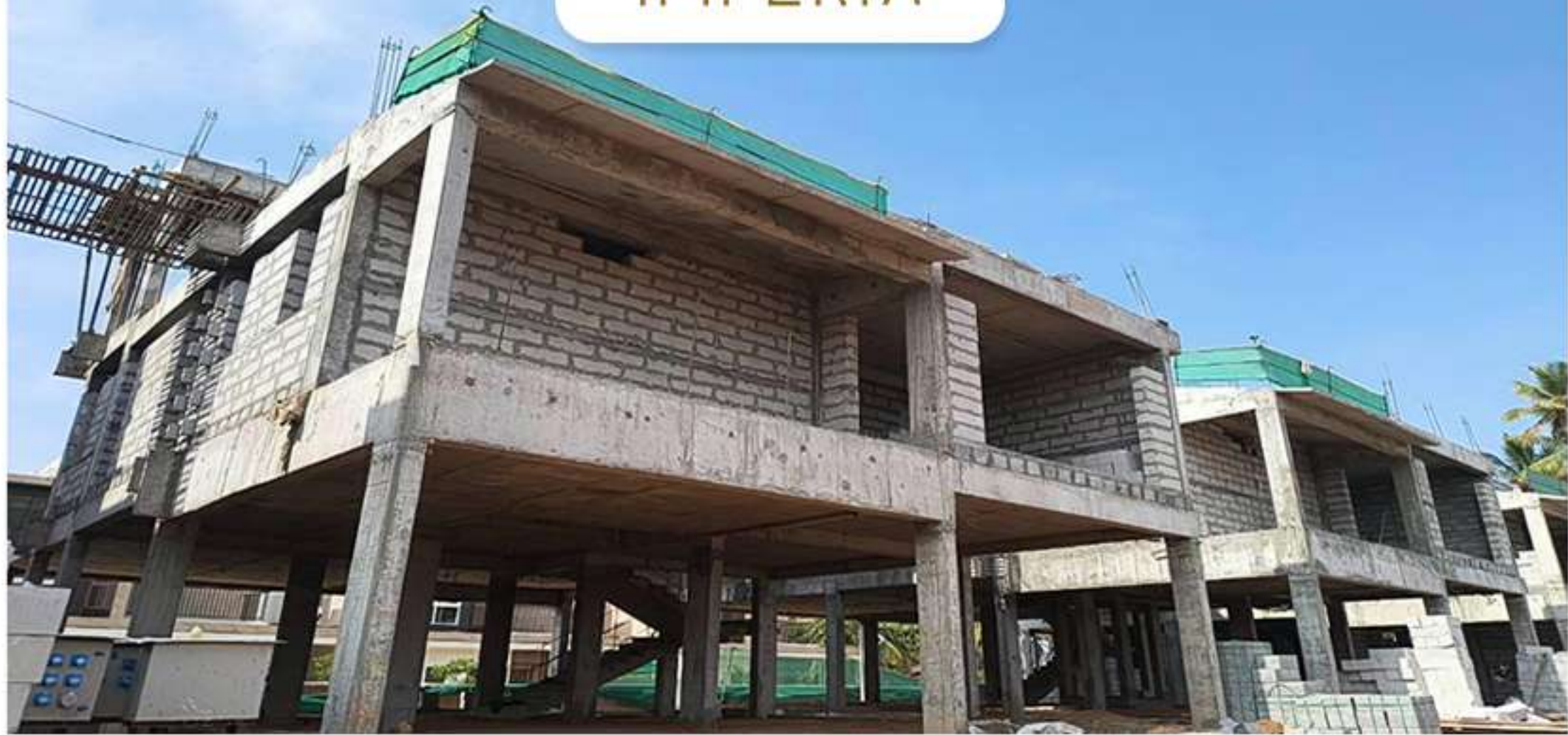
Villa 15 Block Work in Progress
