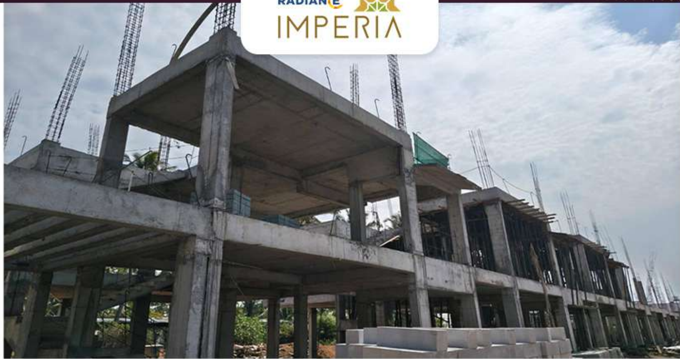
Villas-90 2nd Floor Column Work in Progress
