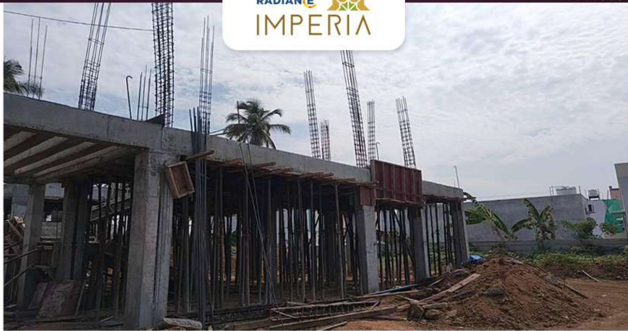
Villas- 97 1st Floor Column Work in Progress
