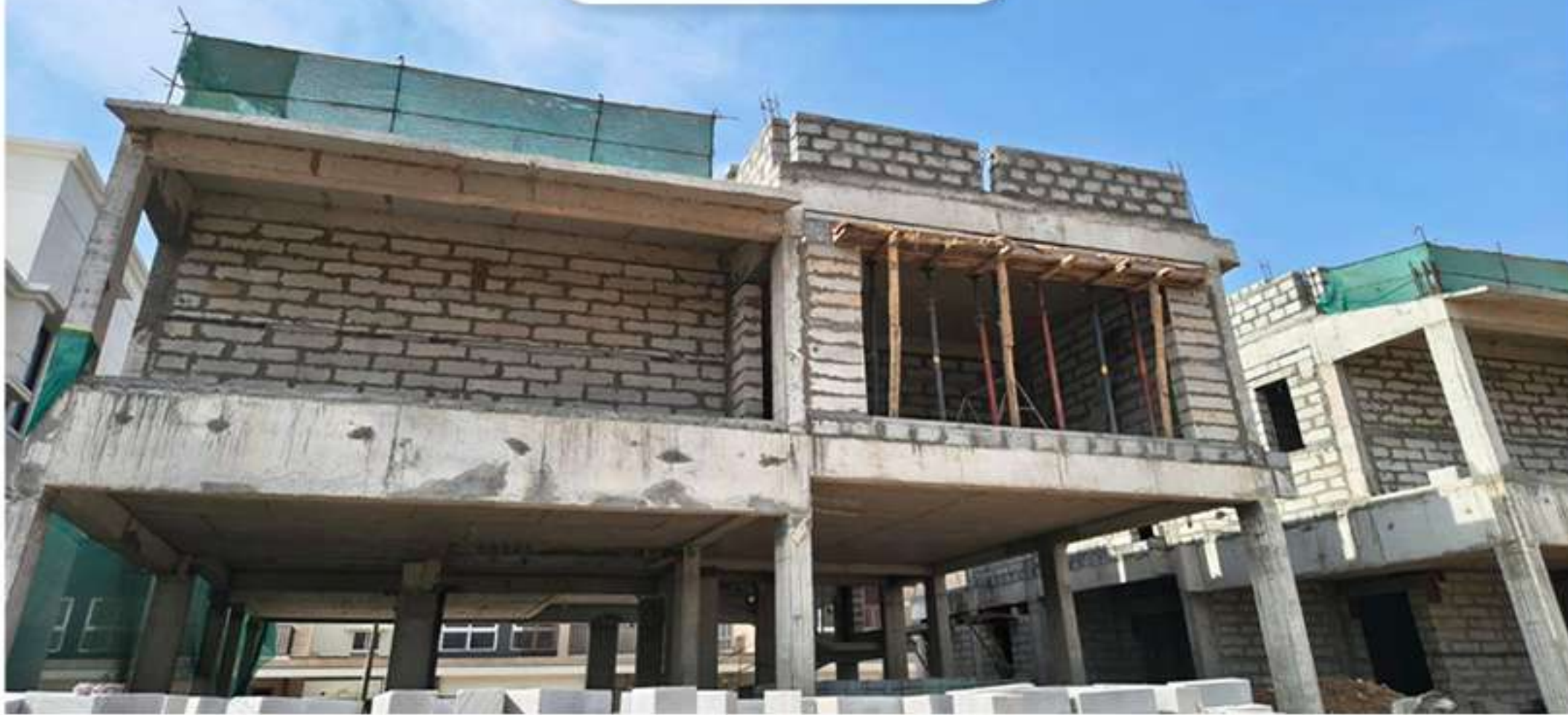
Villa 6 Block Work in Progress
