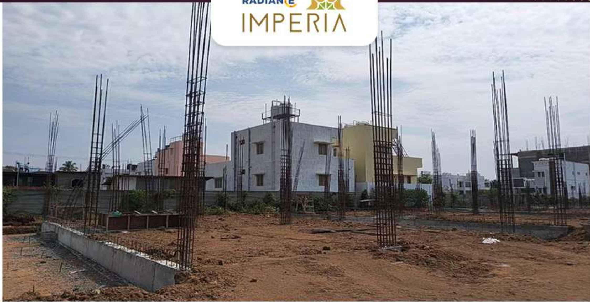
Villas- 57 Ground Floor Column Work in Progress
