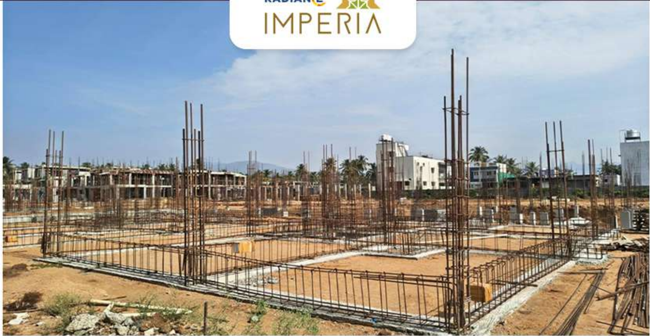
Villa 29 Plinth Beam Reinforcement Work in Progress
