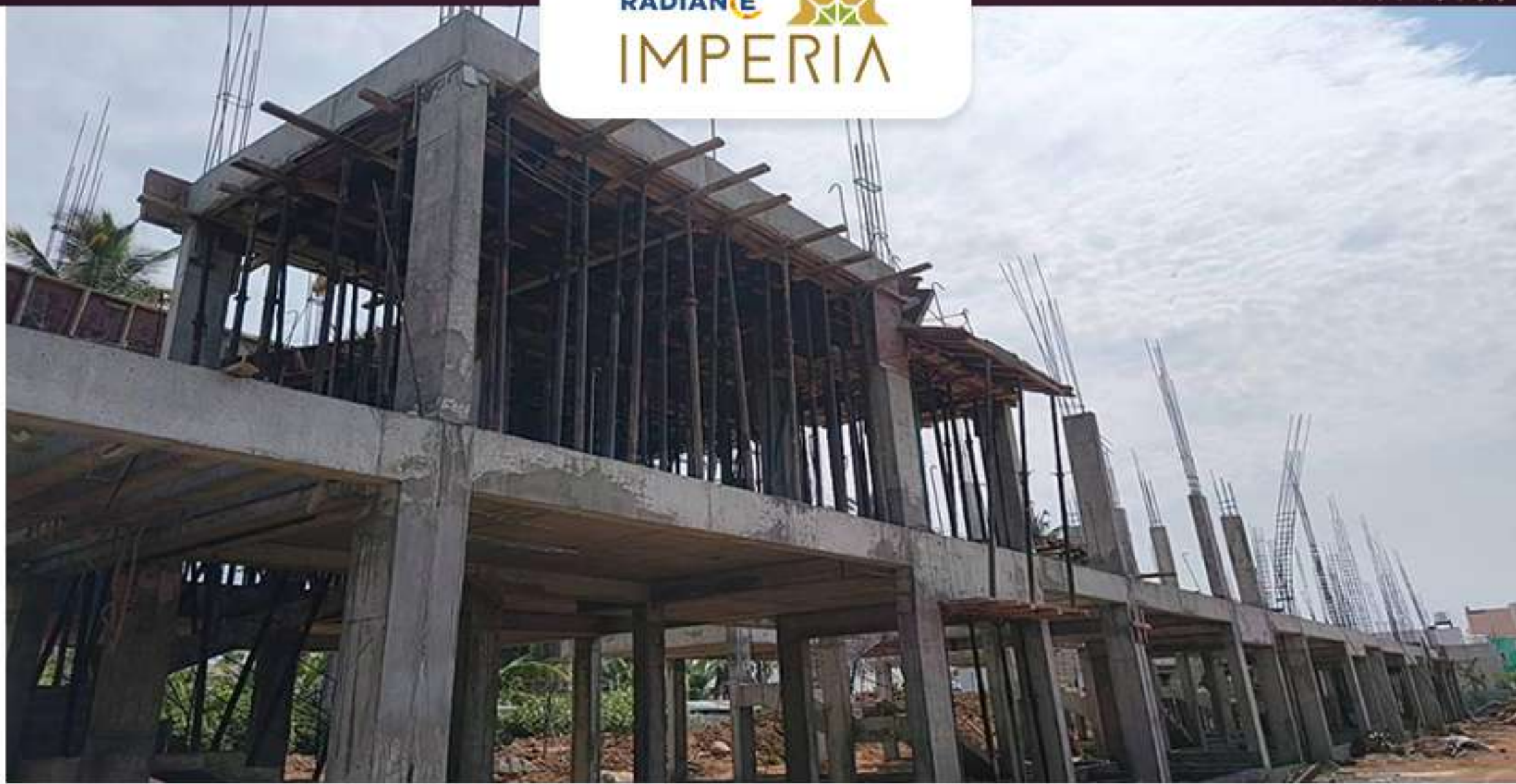
Villas- 92 1st Floor Roof Completed
