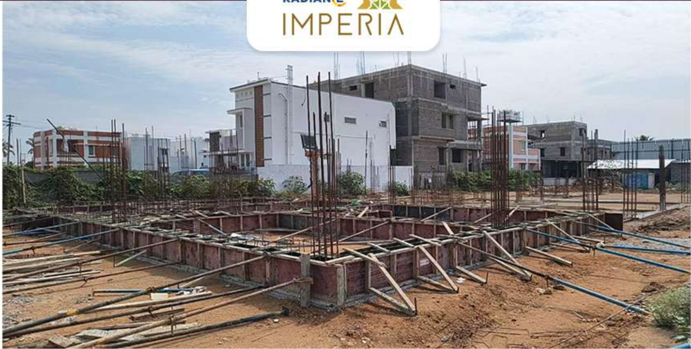
Villas- 62 Plinth Beam Shuttering Work in Progress
