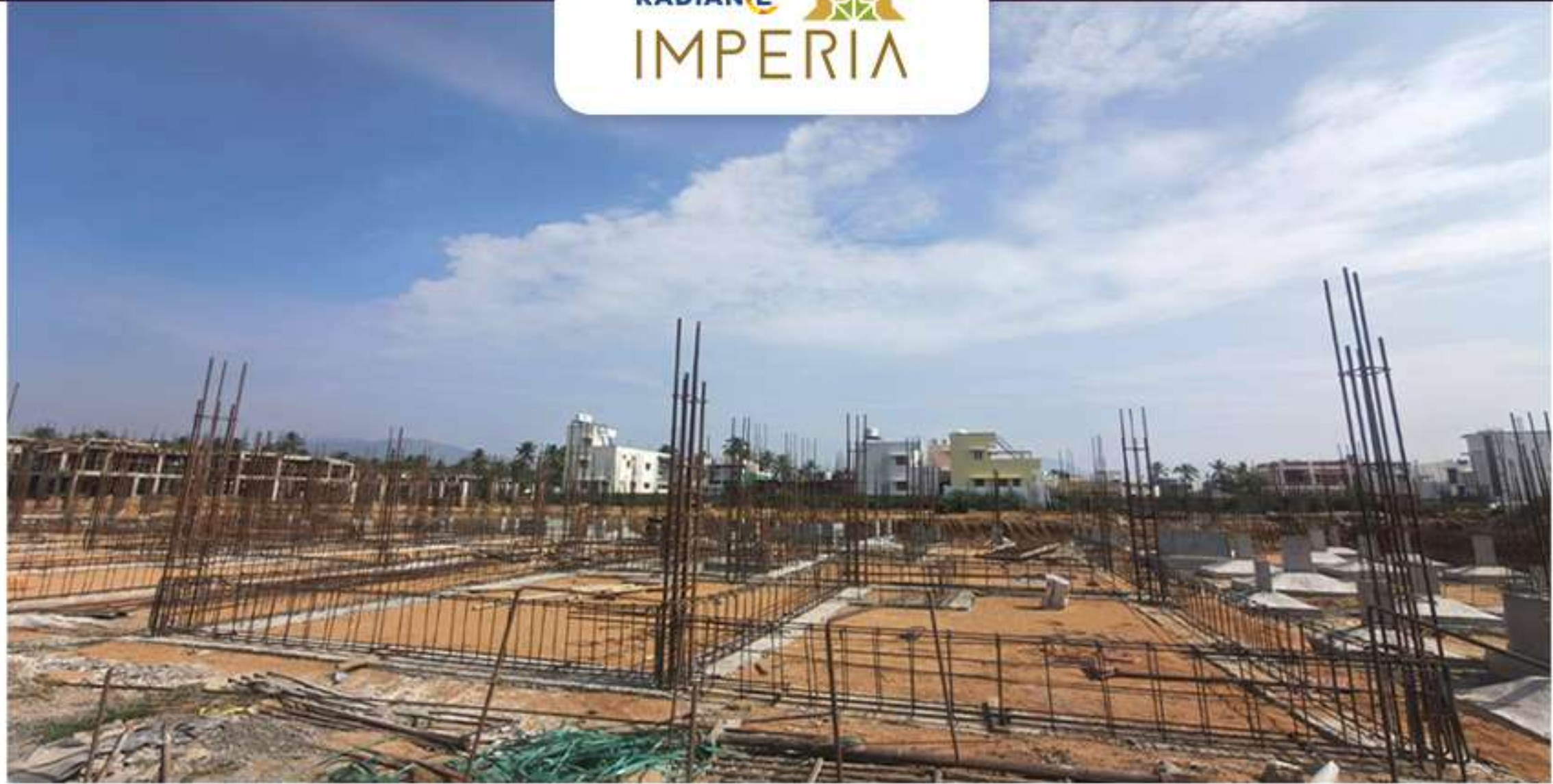
Villa 30 Plinth Beam Reinforcement Work in progress
