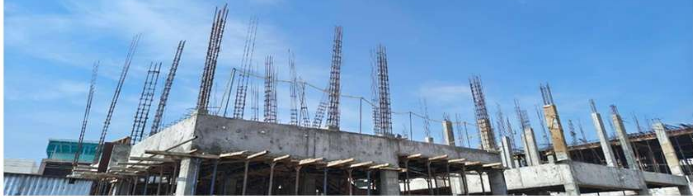
Villa no. 1 First Floor Column Work in Progress
