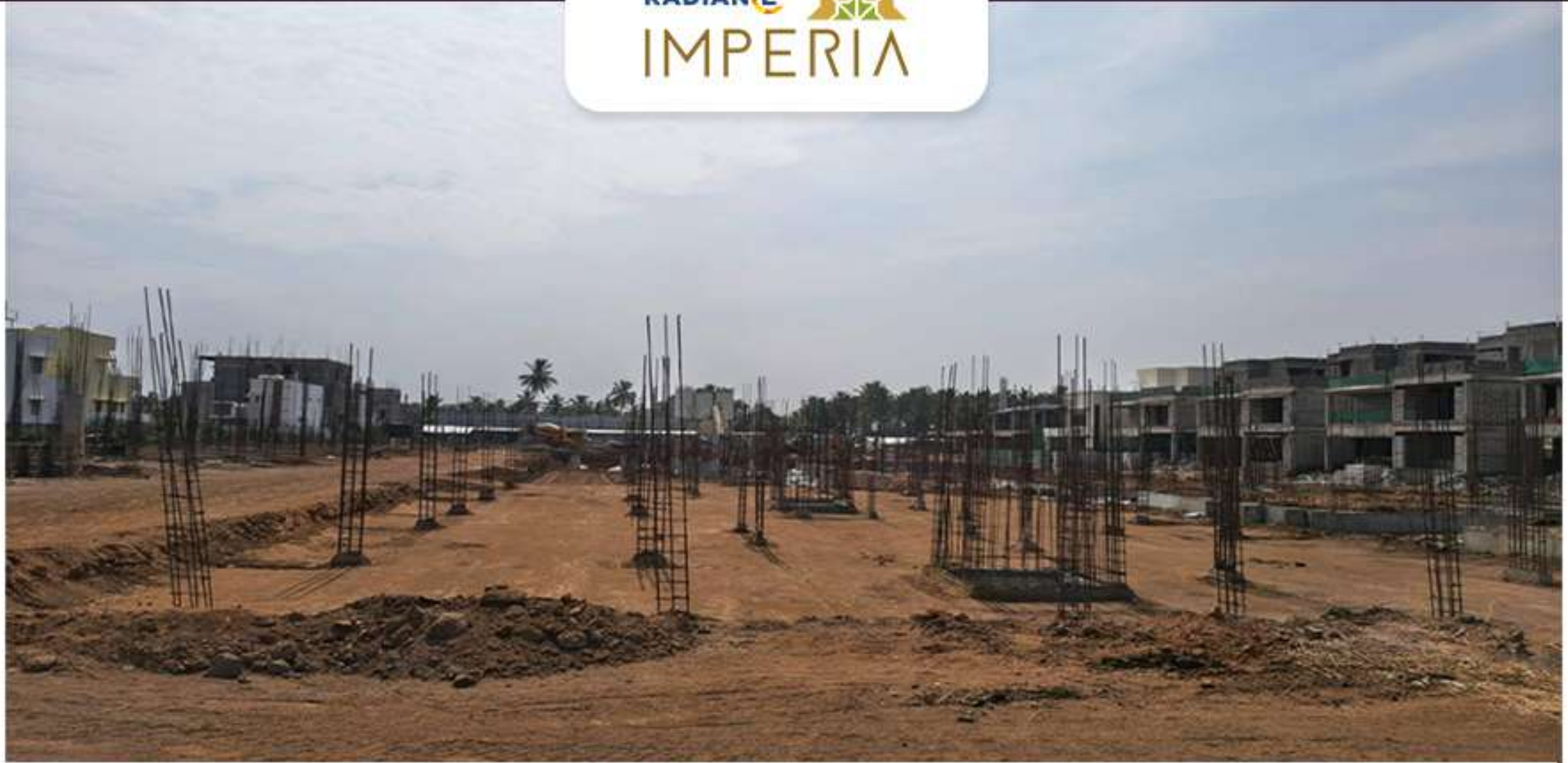
Villa- 38 to 32 Backfilling Work in Progress
