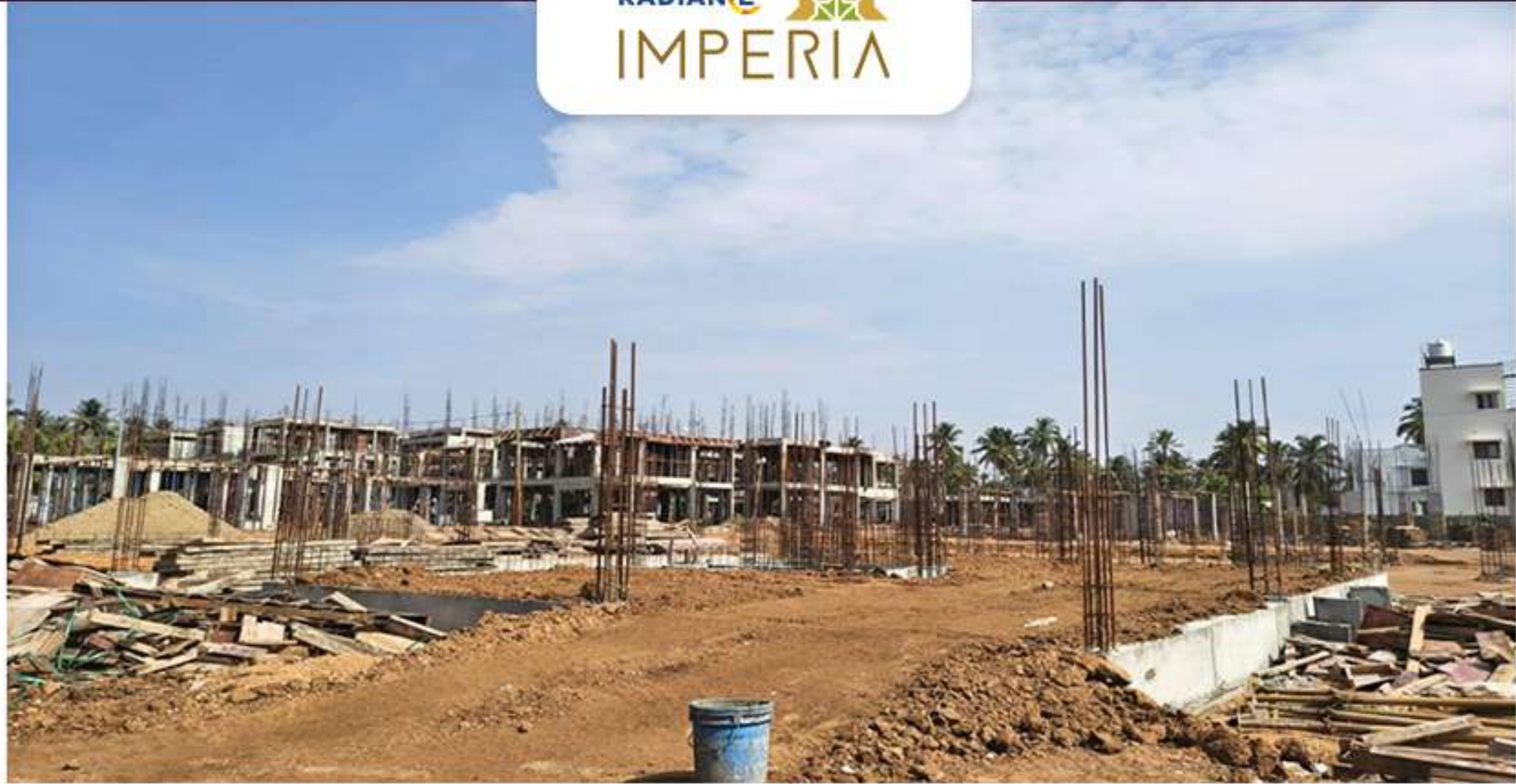
Villa 25 Plinth Beam Level Soil Filling Work in Progress
