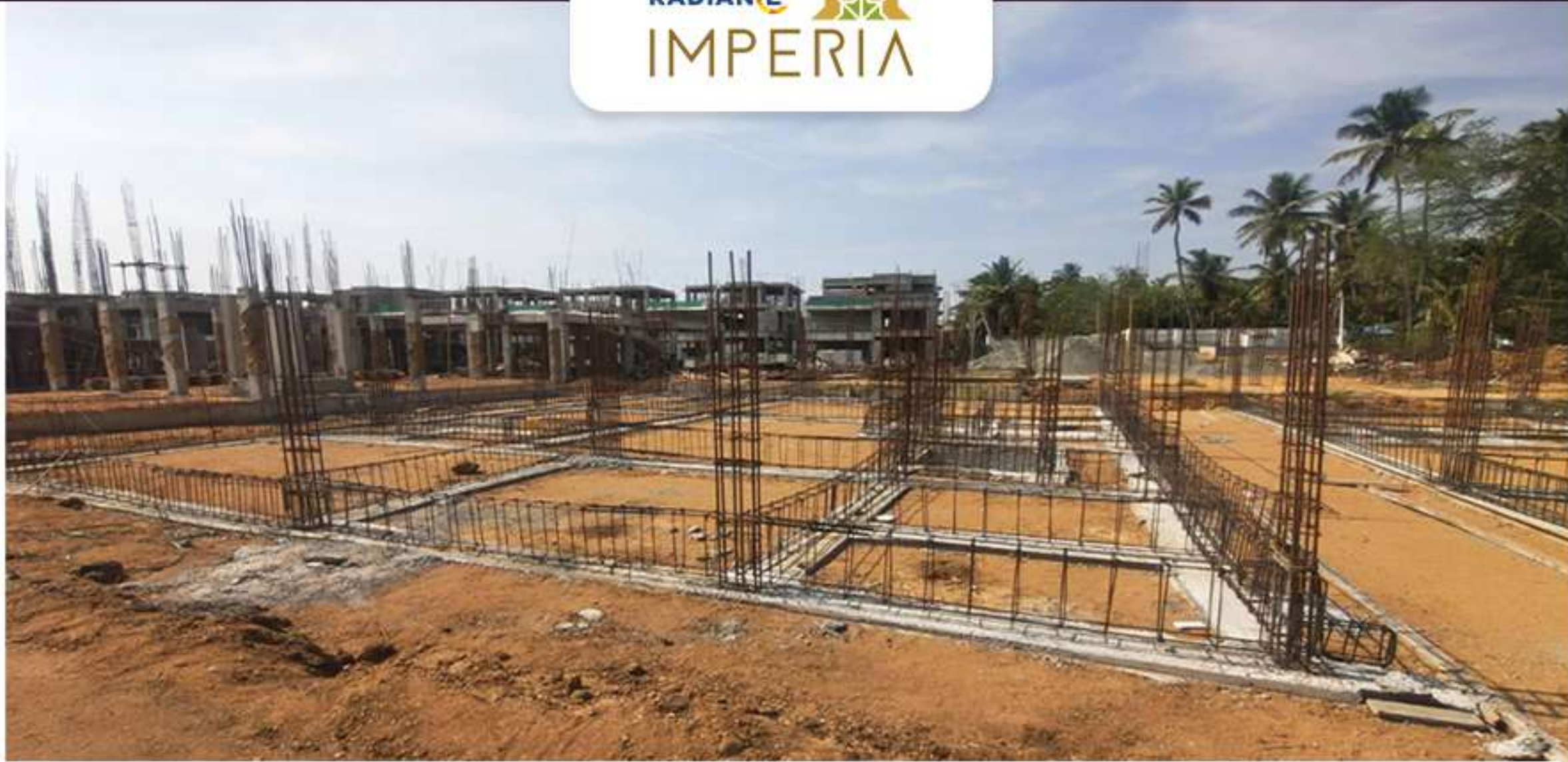
Villa 42 Plinth Beam Work in Progress
