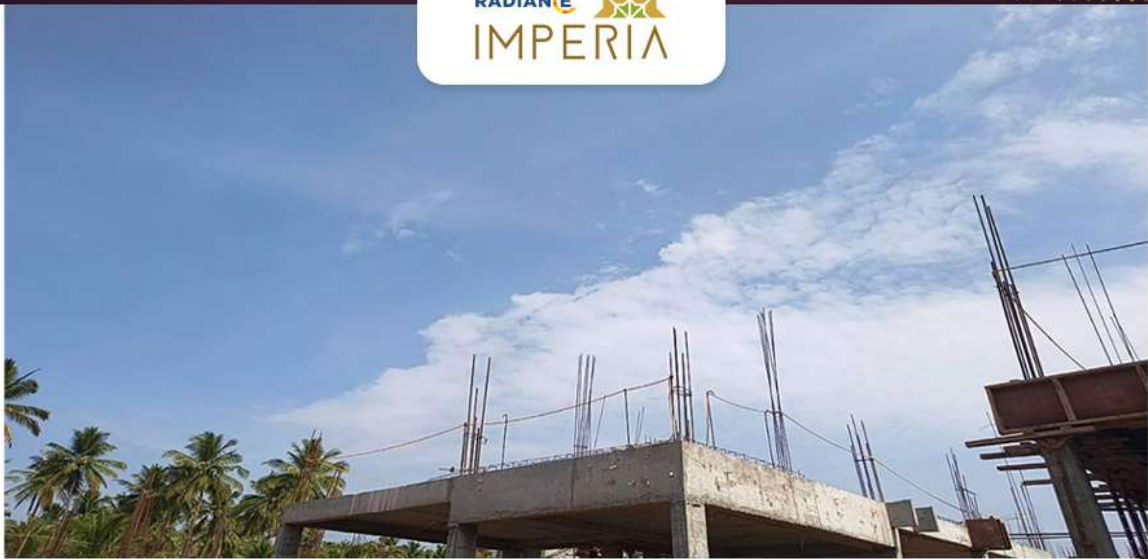
Villa 21 First Floor Column Work in progress
