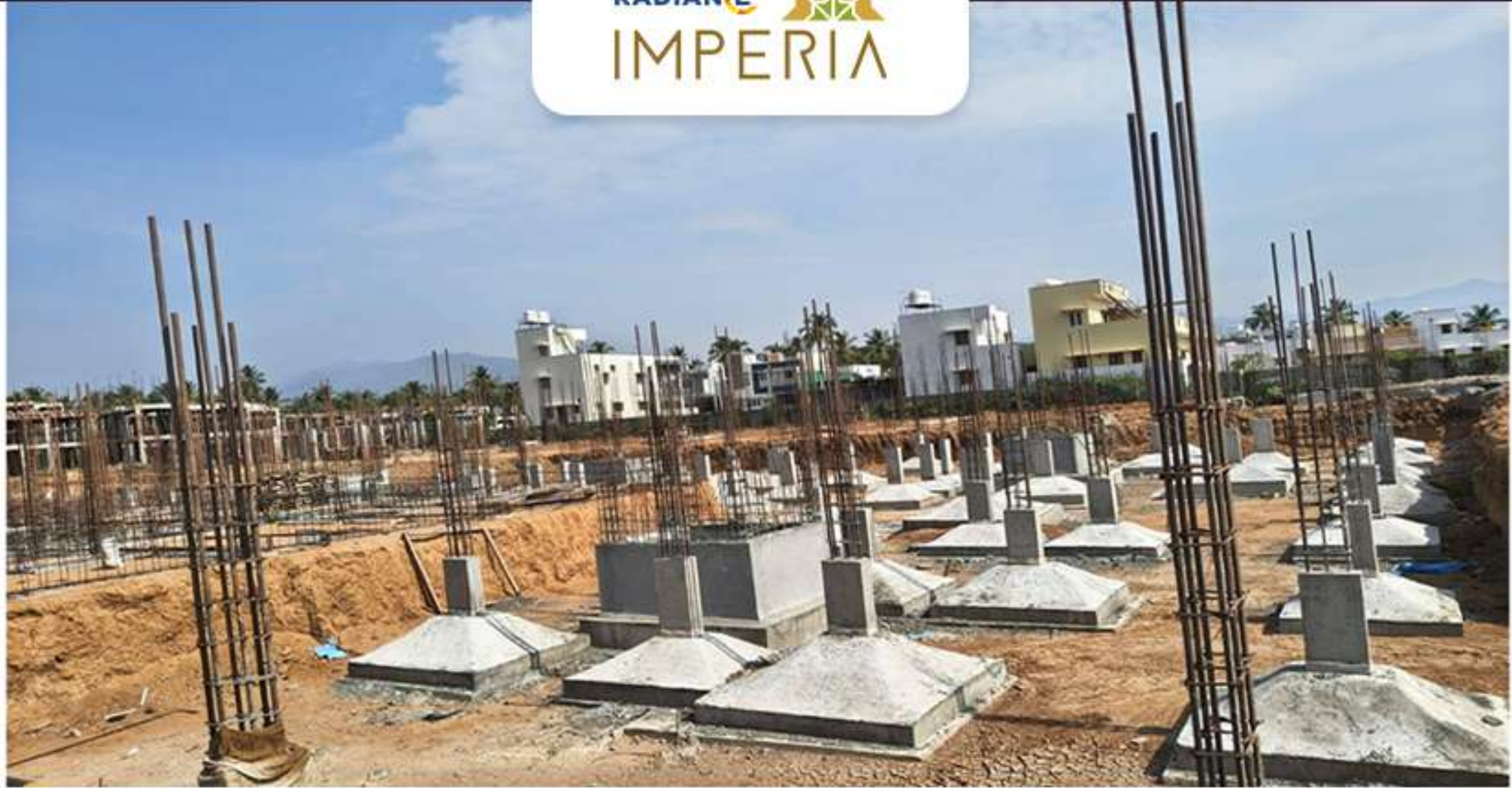
Villa 31 Back Filling Work in Progress
