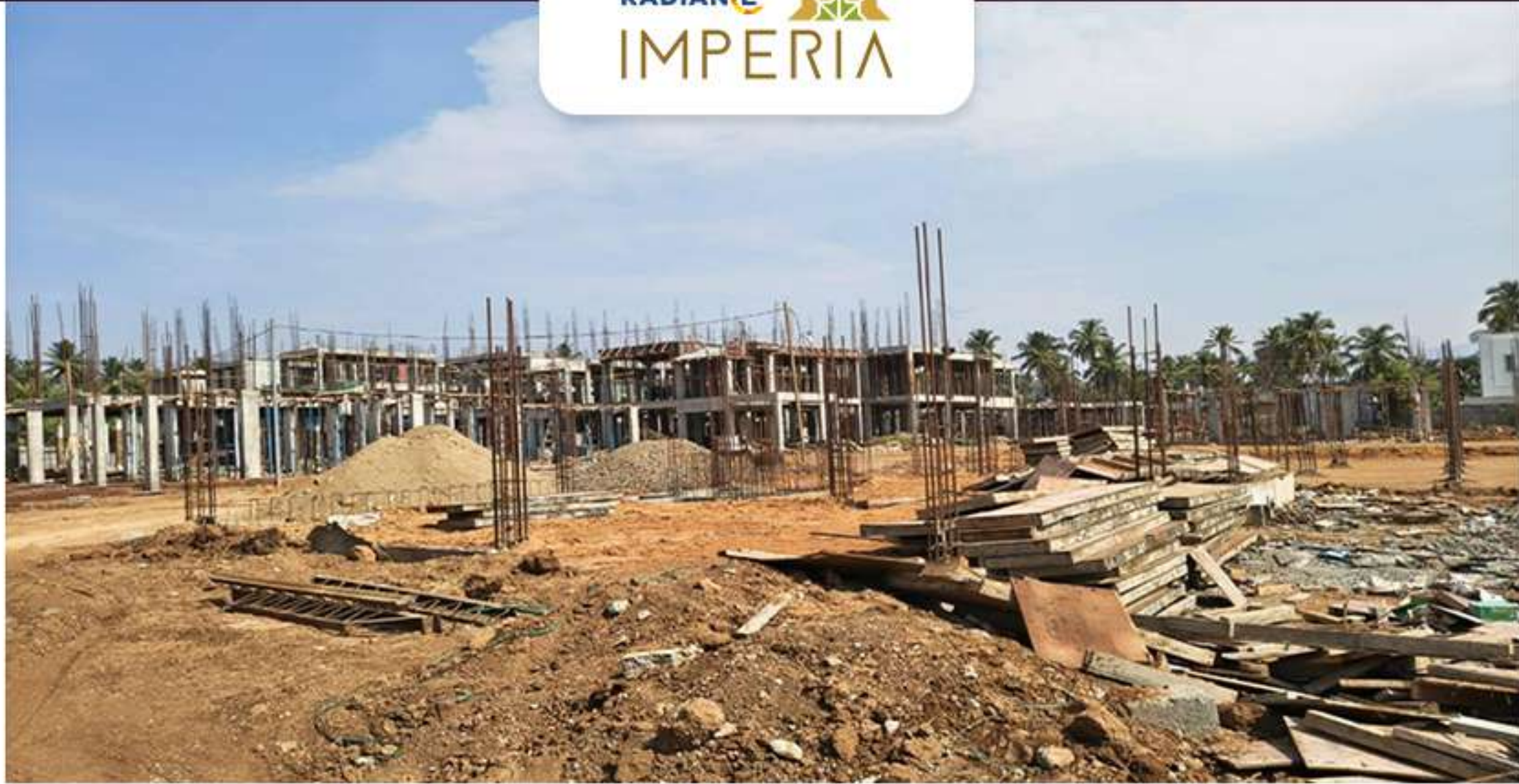
Villa 24 Plinth Beam Level Soil Filling Work in Progress
