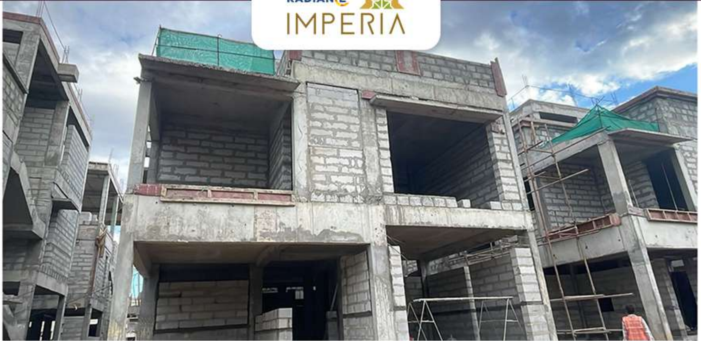
Villa no -69 – Block Work in progress.
