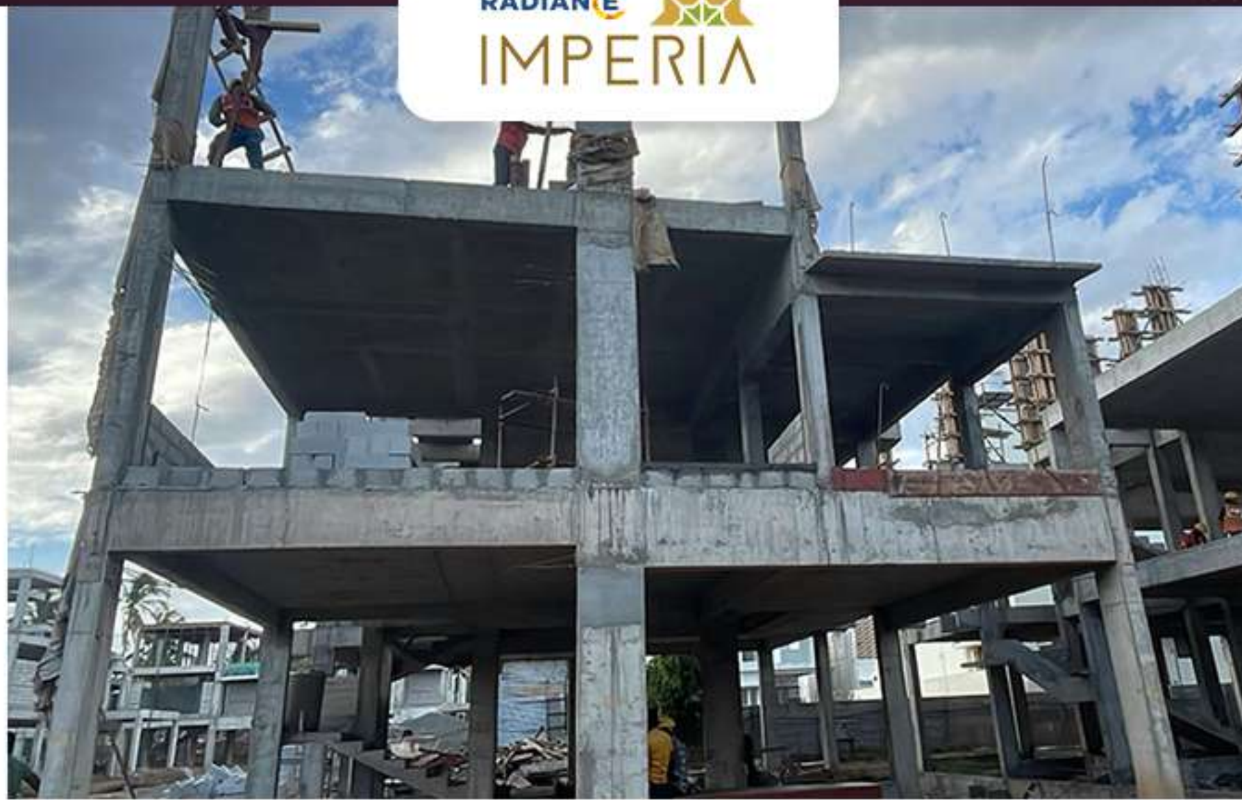
Villa no – 52 SF Roof slab shuttering work in progress
