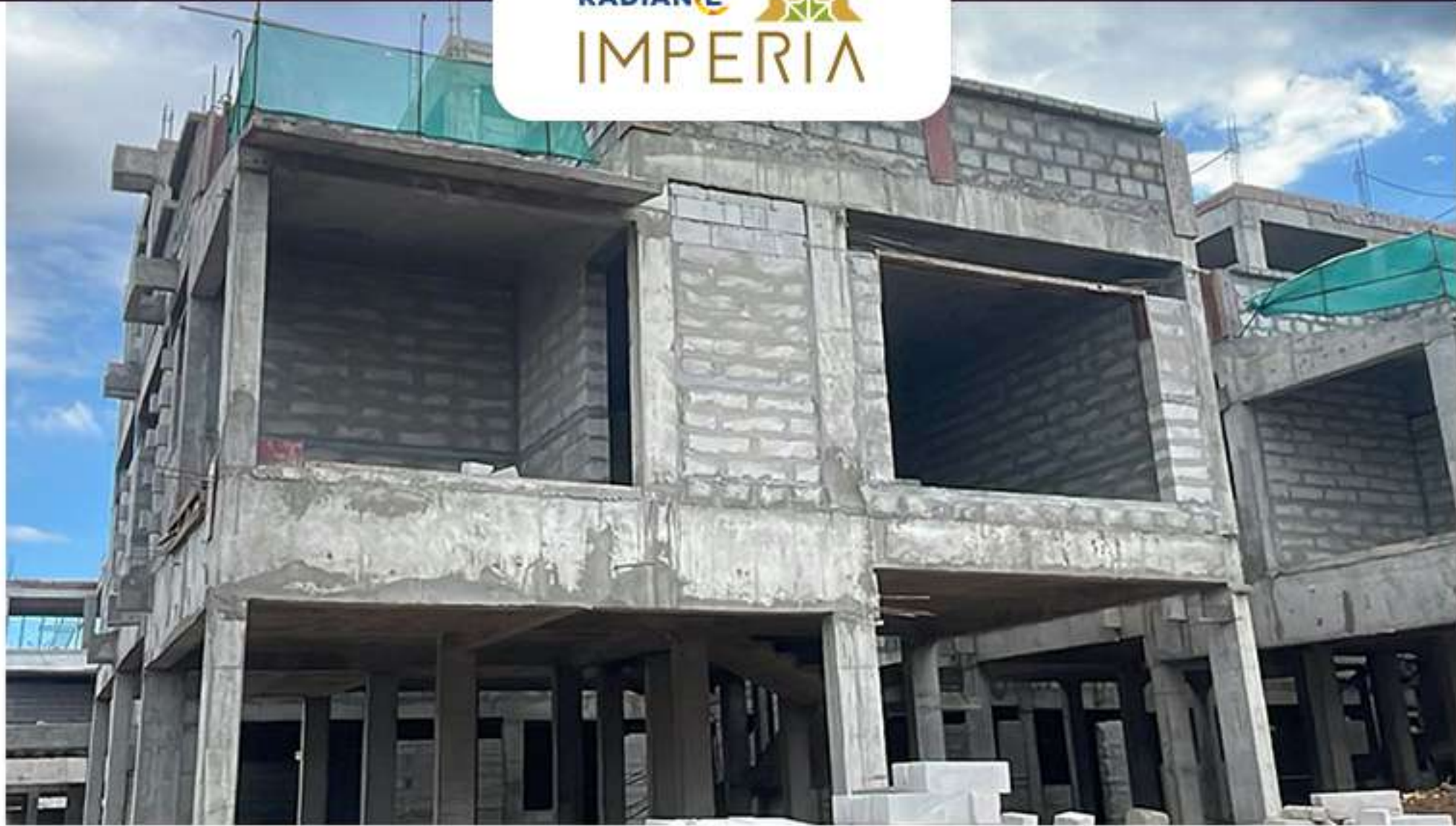
Villa no -65 – Block work in progress
