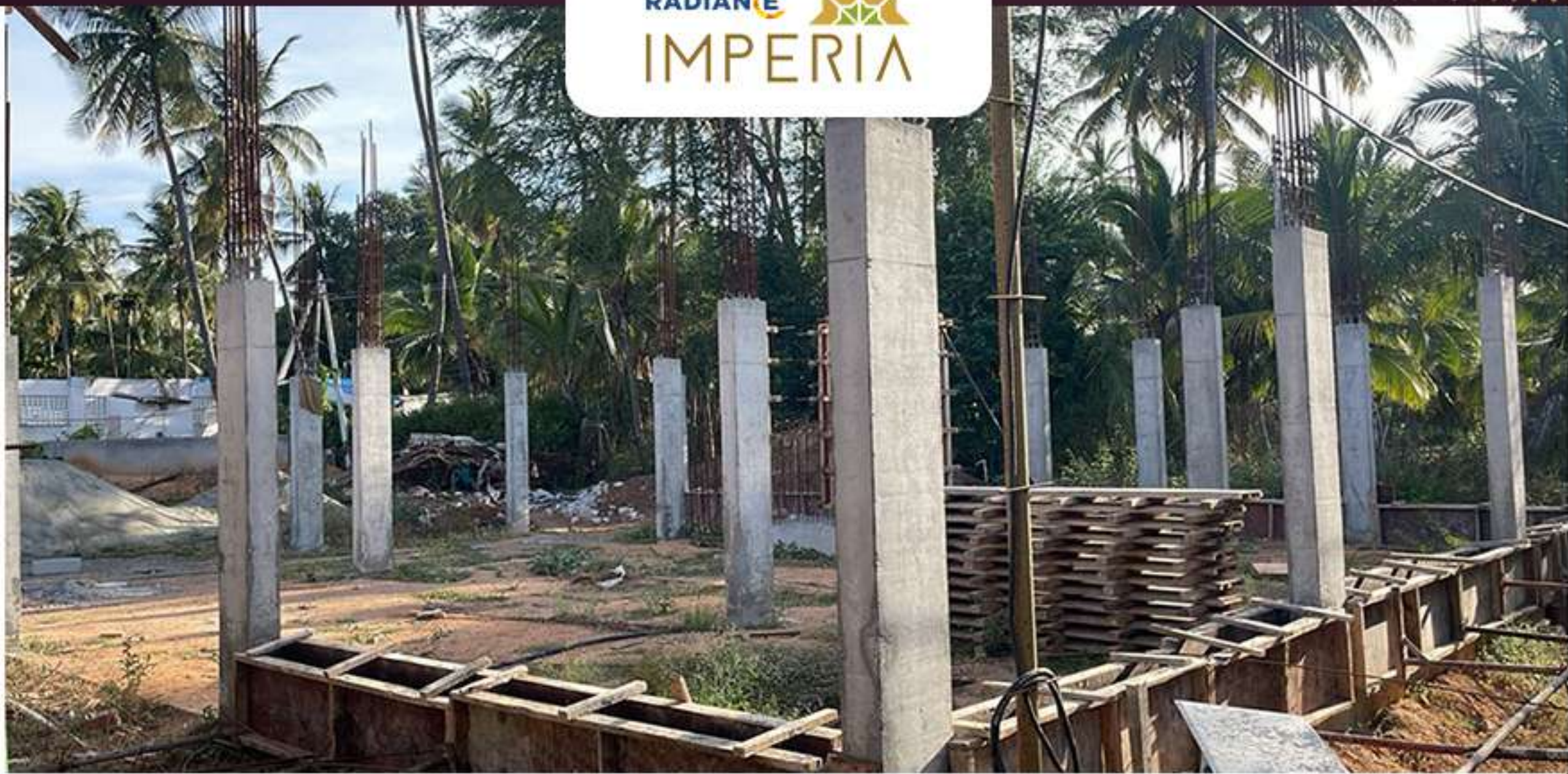
Villa no -19 Ground Floor Column completed
