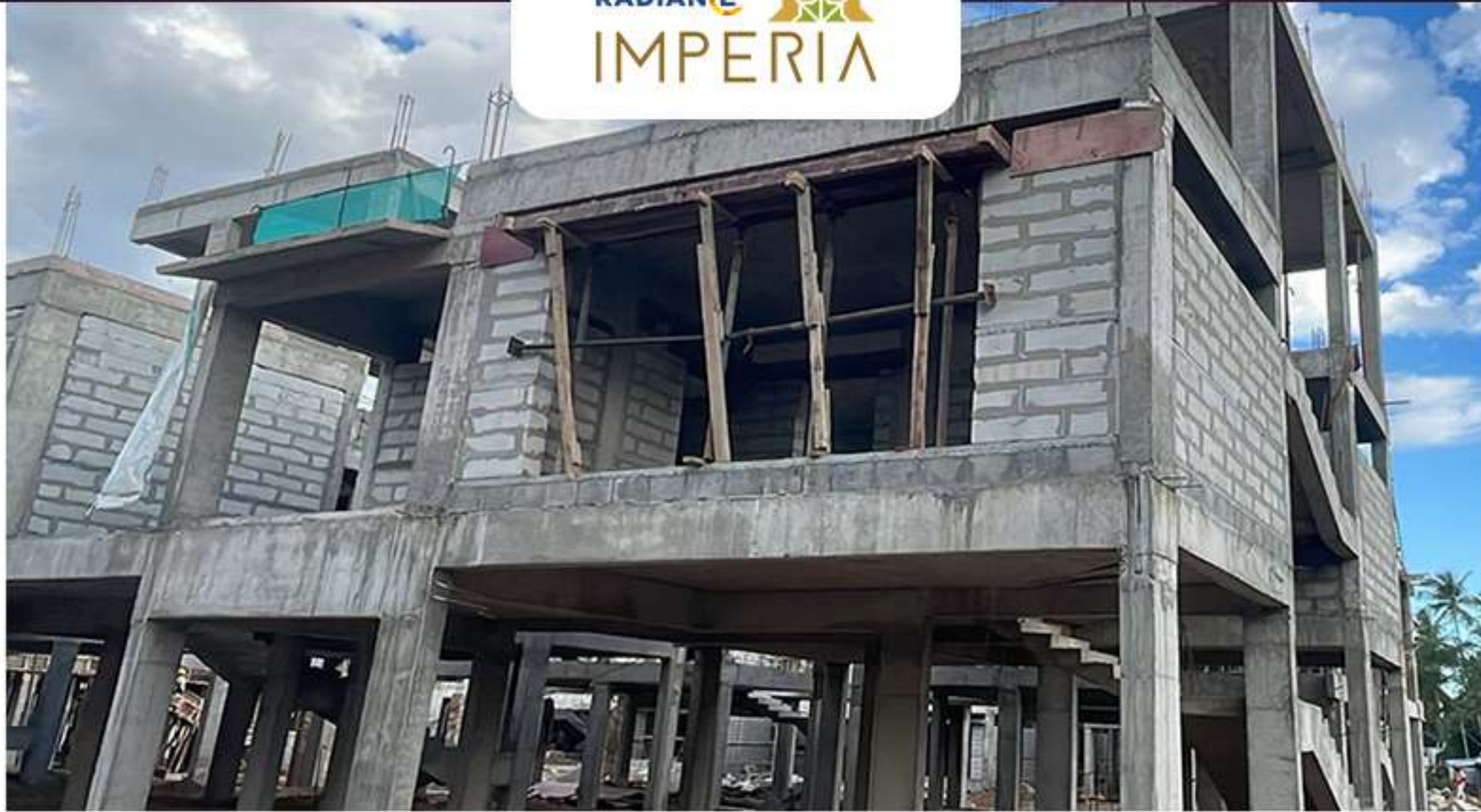
Villa no – 87 – Block work in progress.
