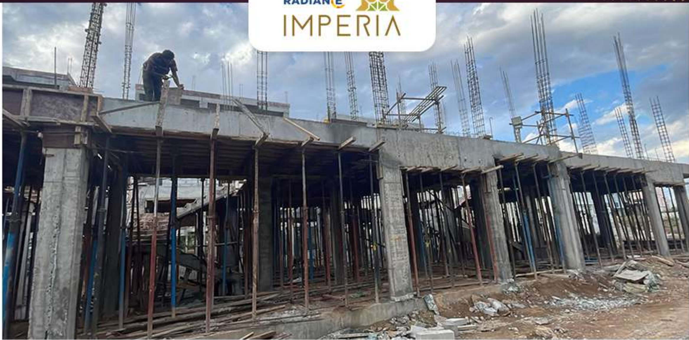
Villa no -78 – GF Slab concrete completed
