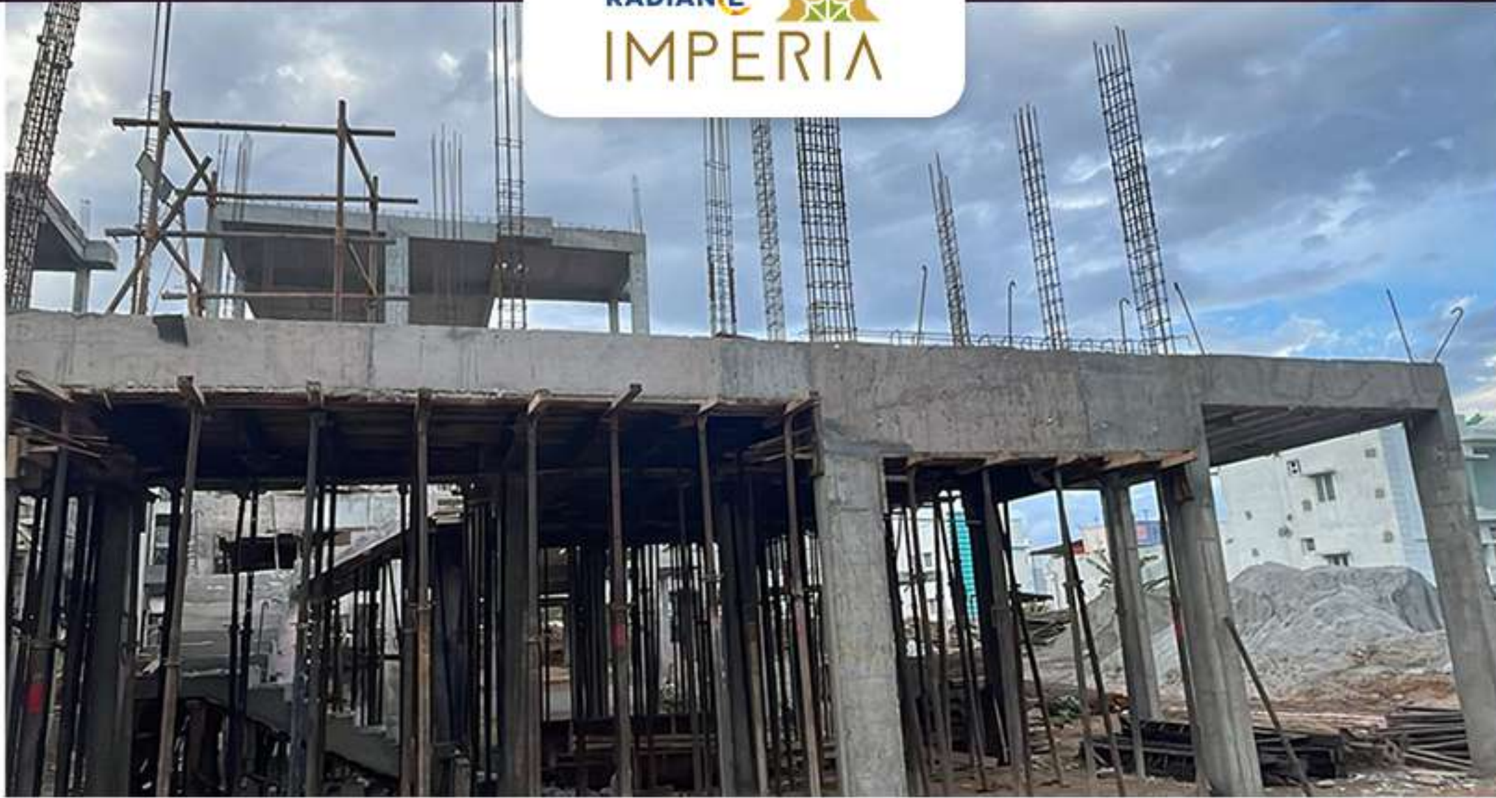
Villa no -79 – GF roof slab completed.
