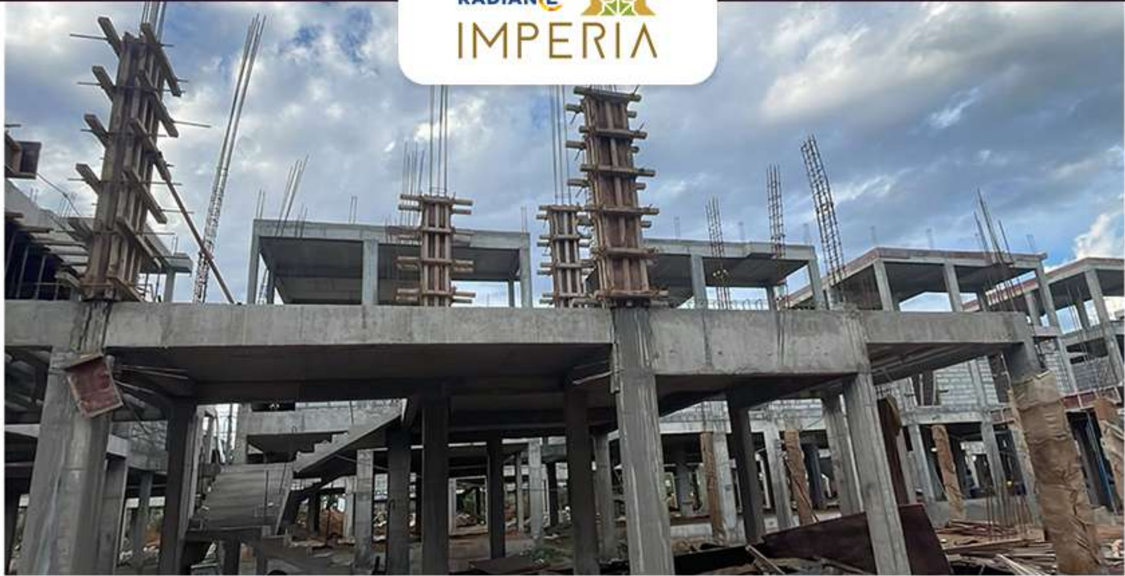
Villa no -74 FF Column work in progress
