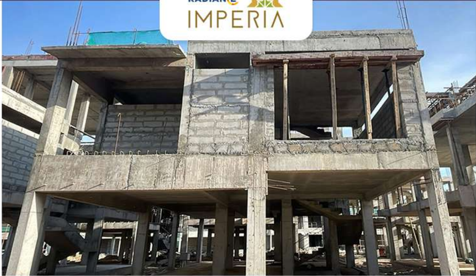
Villa no -40 Block work in process.
