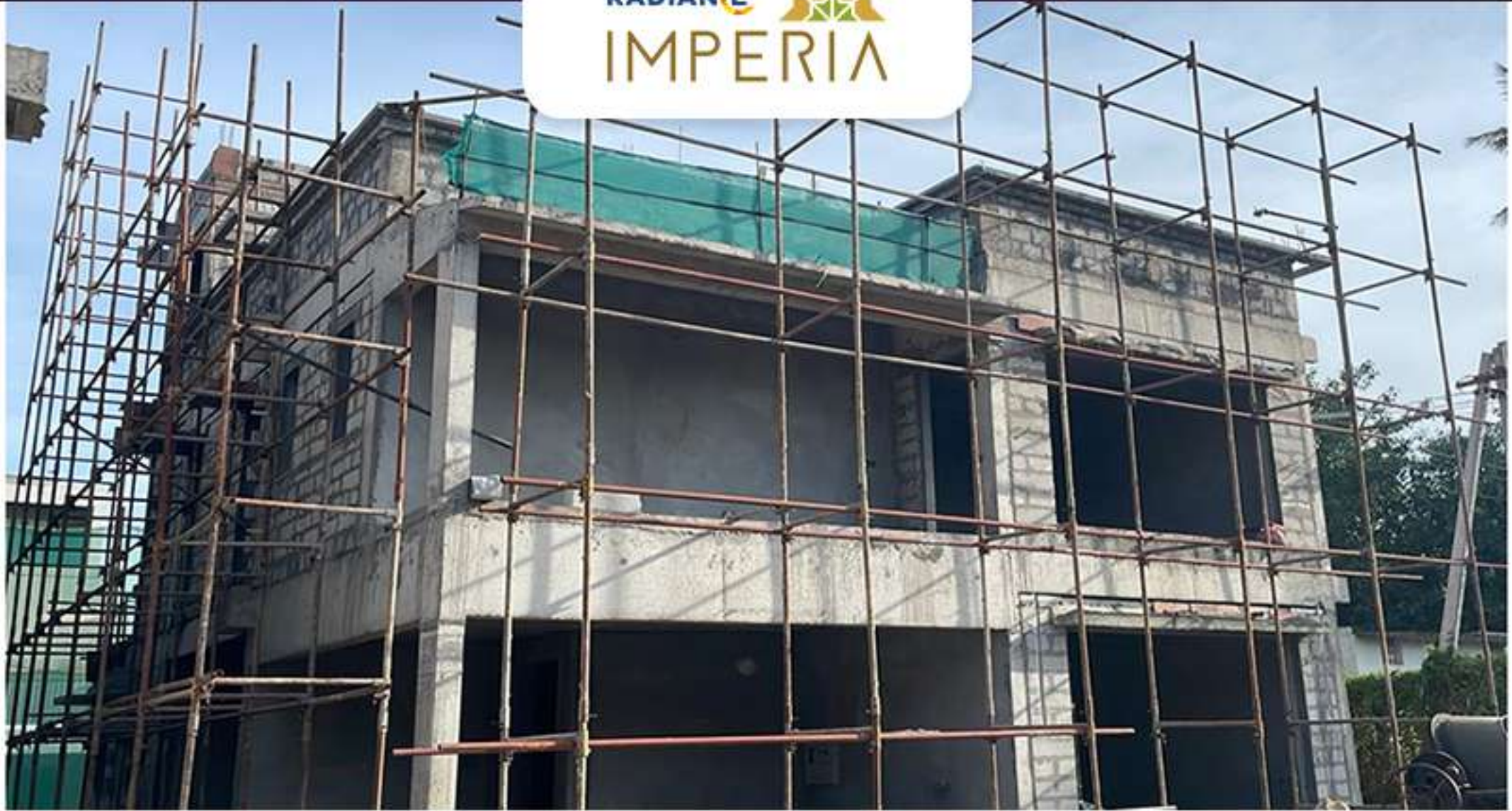
Villa no -18 – Plastering work in progress
