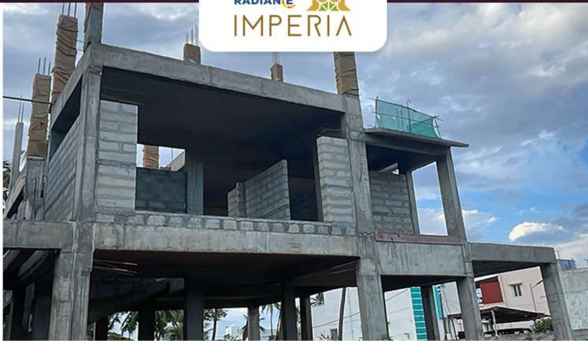
Villa no – 97 – SF Column completed & Block work in progress
