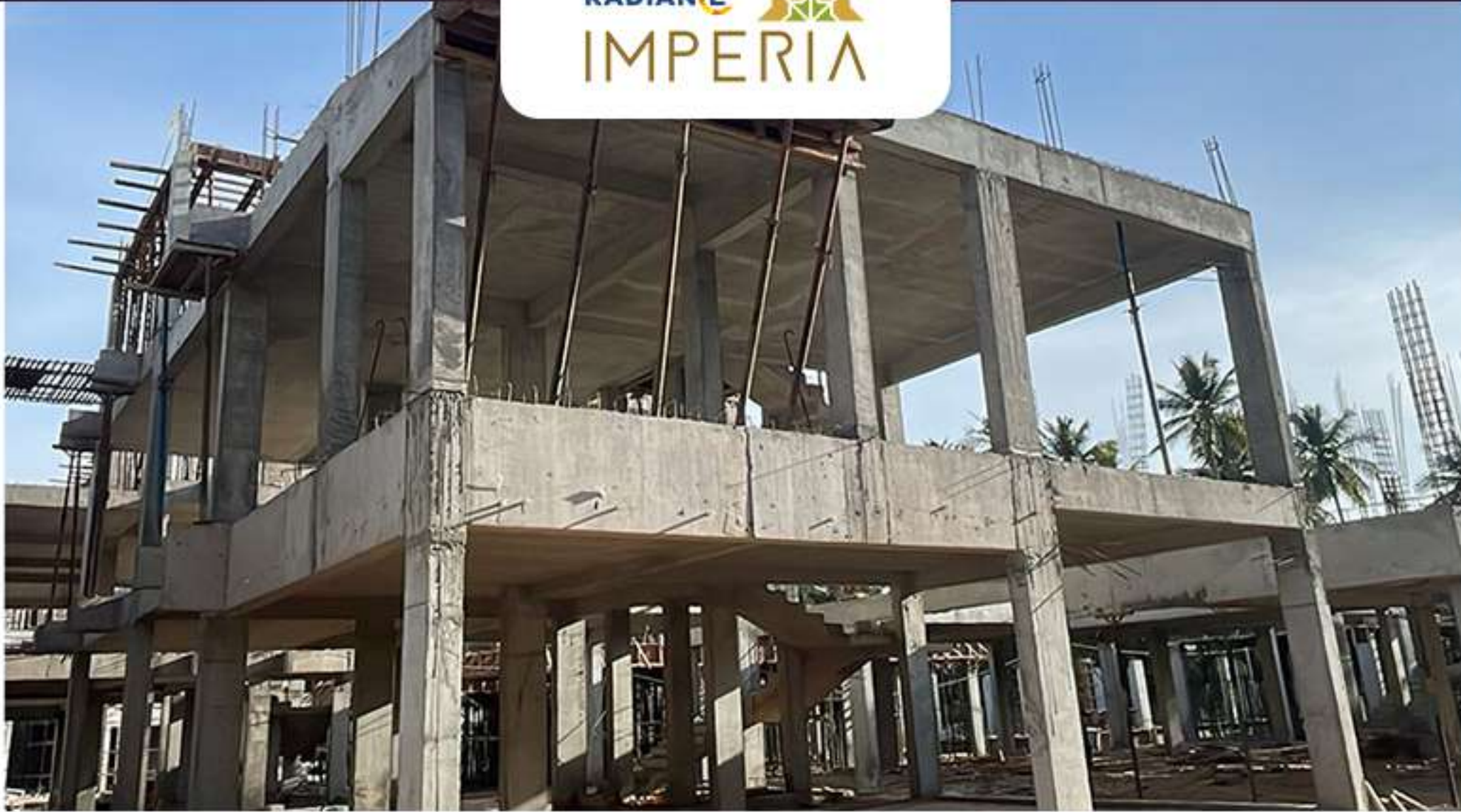
Villa no -41 – 2nd Floor roof Slab Work in progress.
