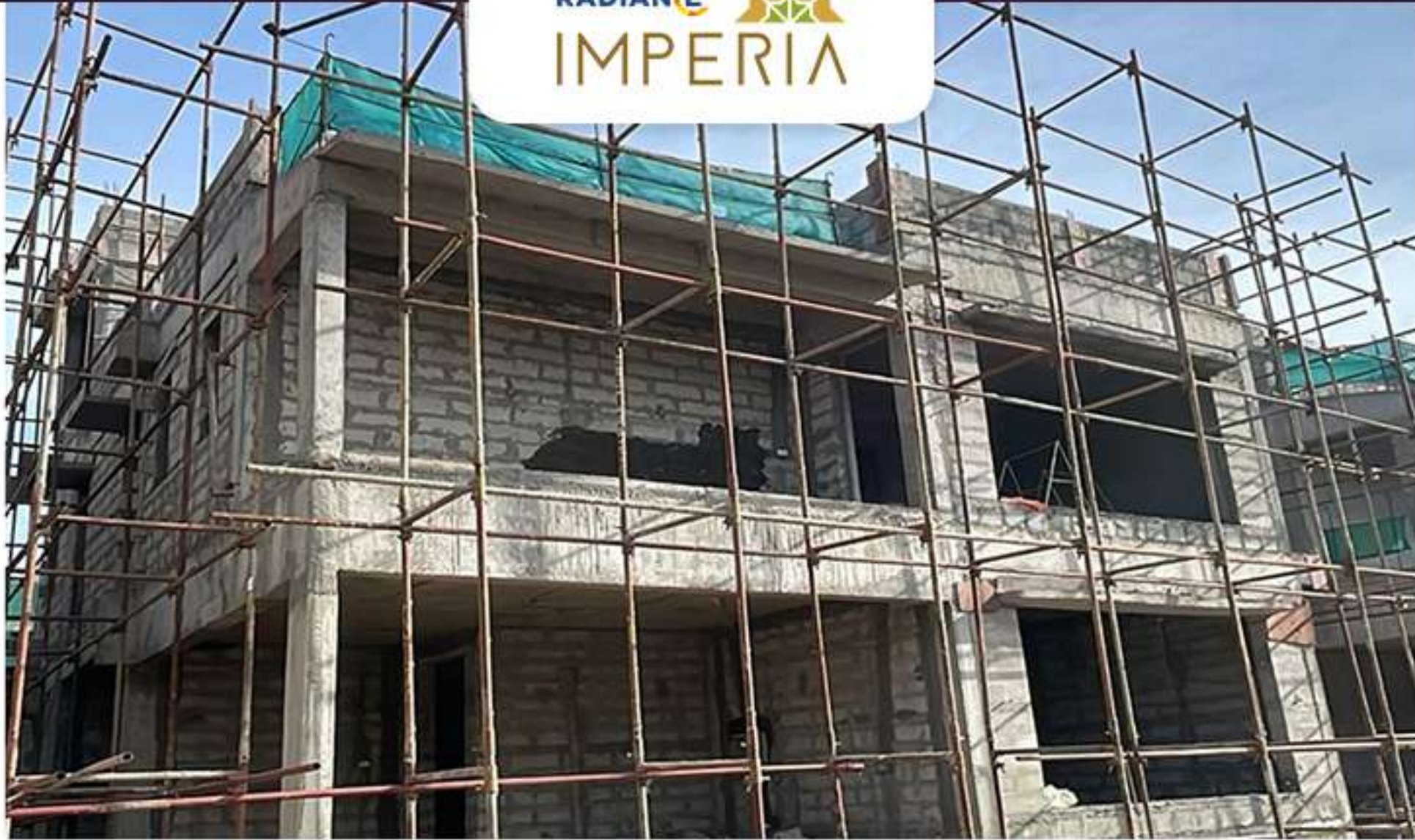
Villa no -11 Block Work completed.
