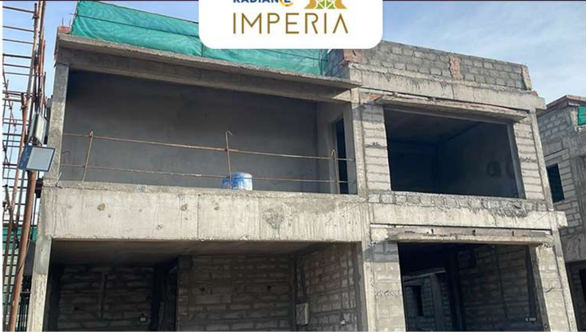
Villa no -14 – Plastering work in progress
