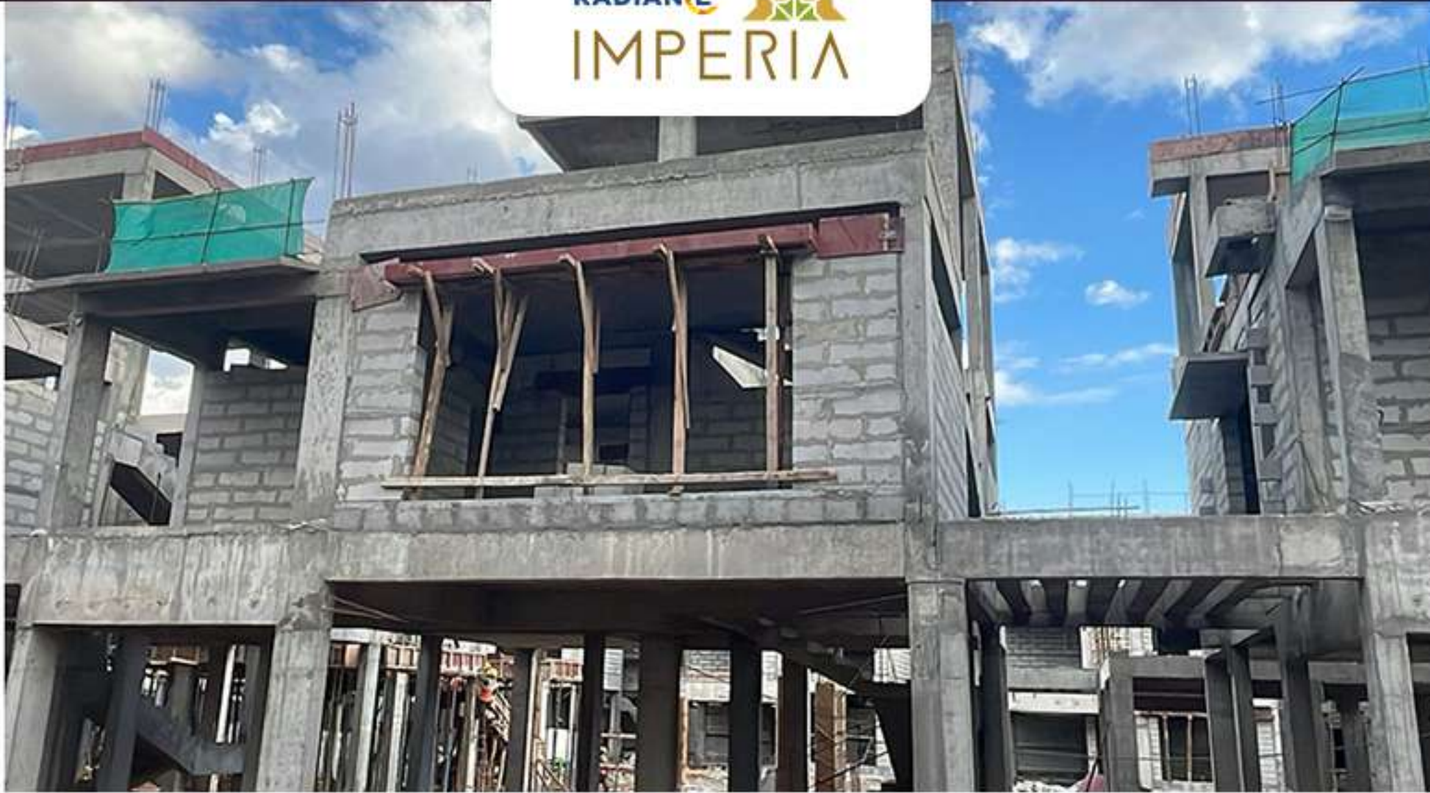
Villa no - 84 - Lintel work in progress
