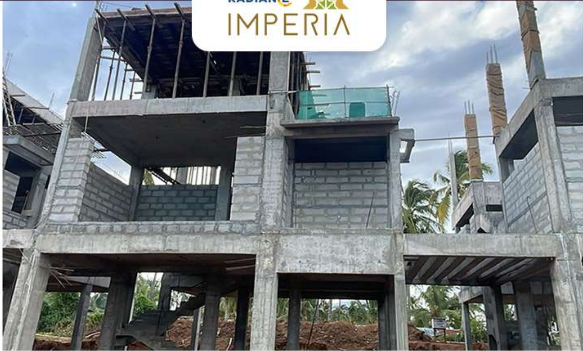
Villa no – 96 – SF roof shuttering Work in progress.
