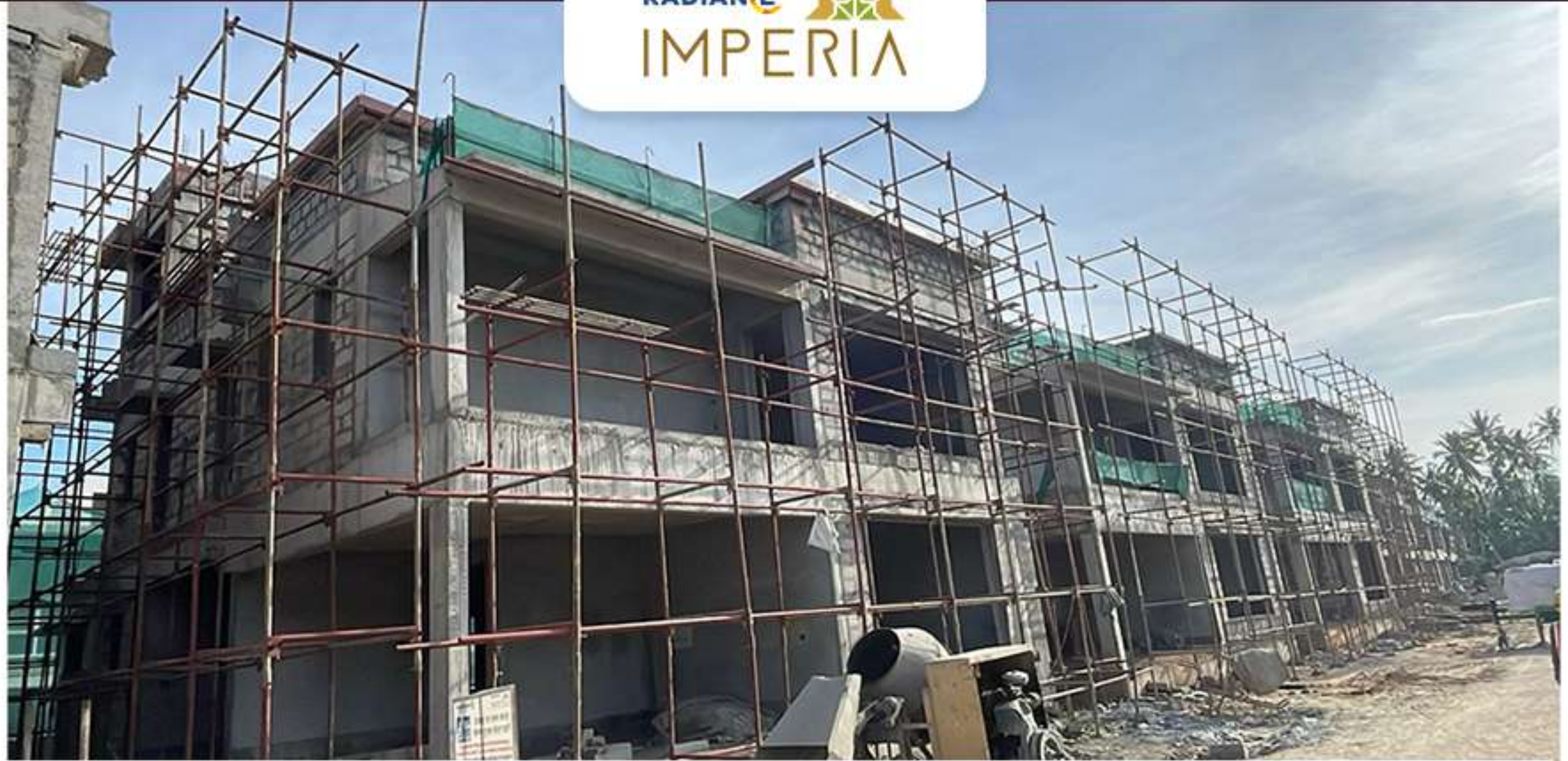
Villa no 7 Plastering Work in Progress.
