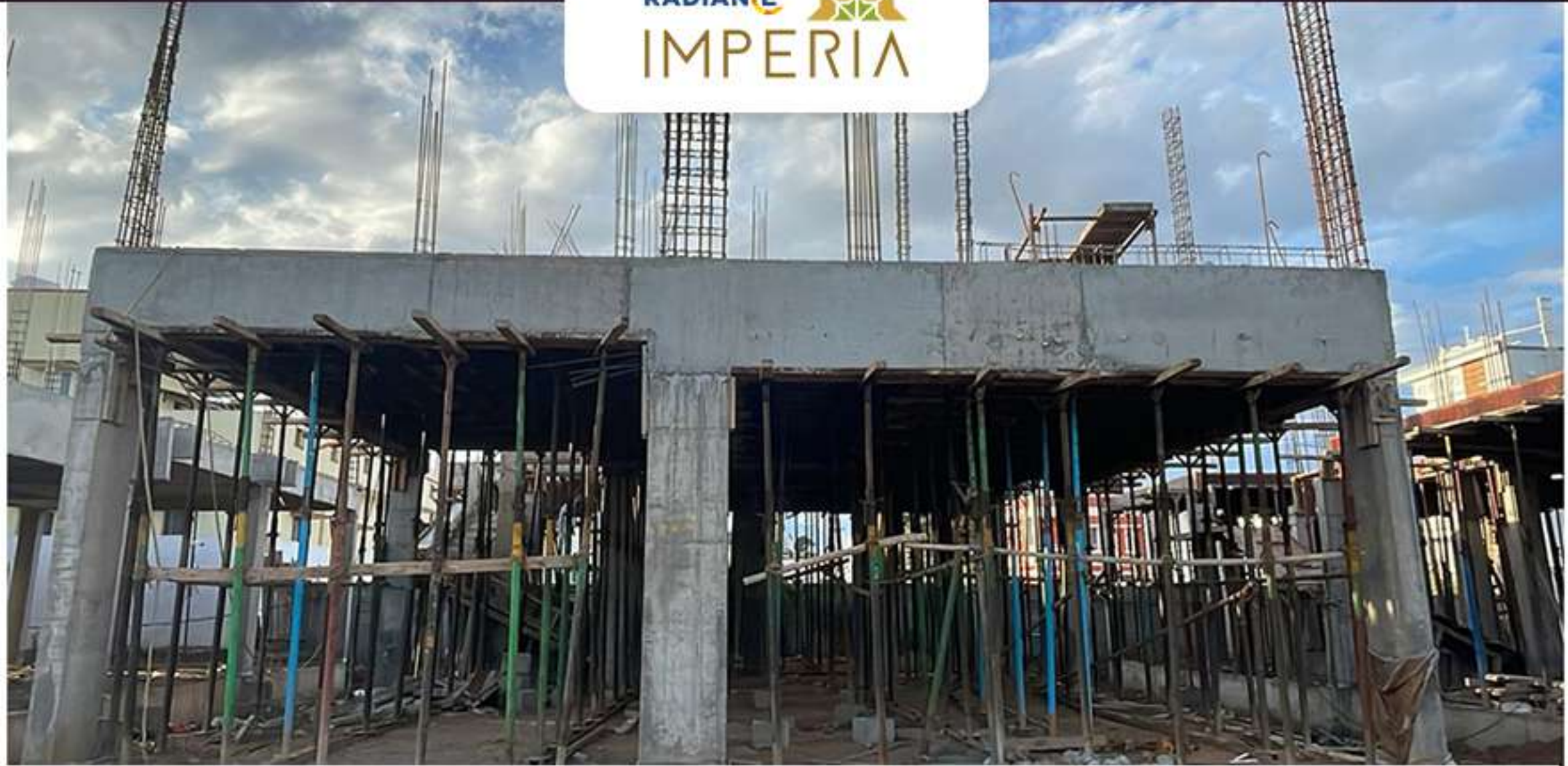
Villa no 60 – FF Column Work in Progres
