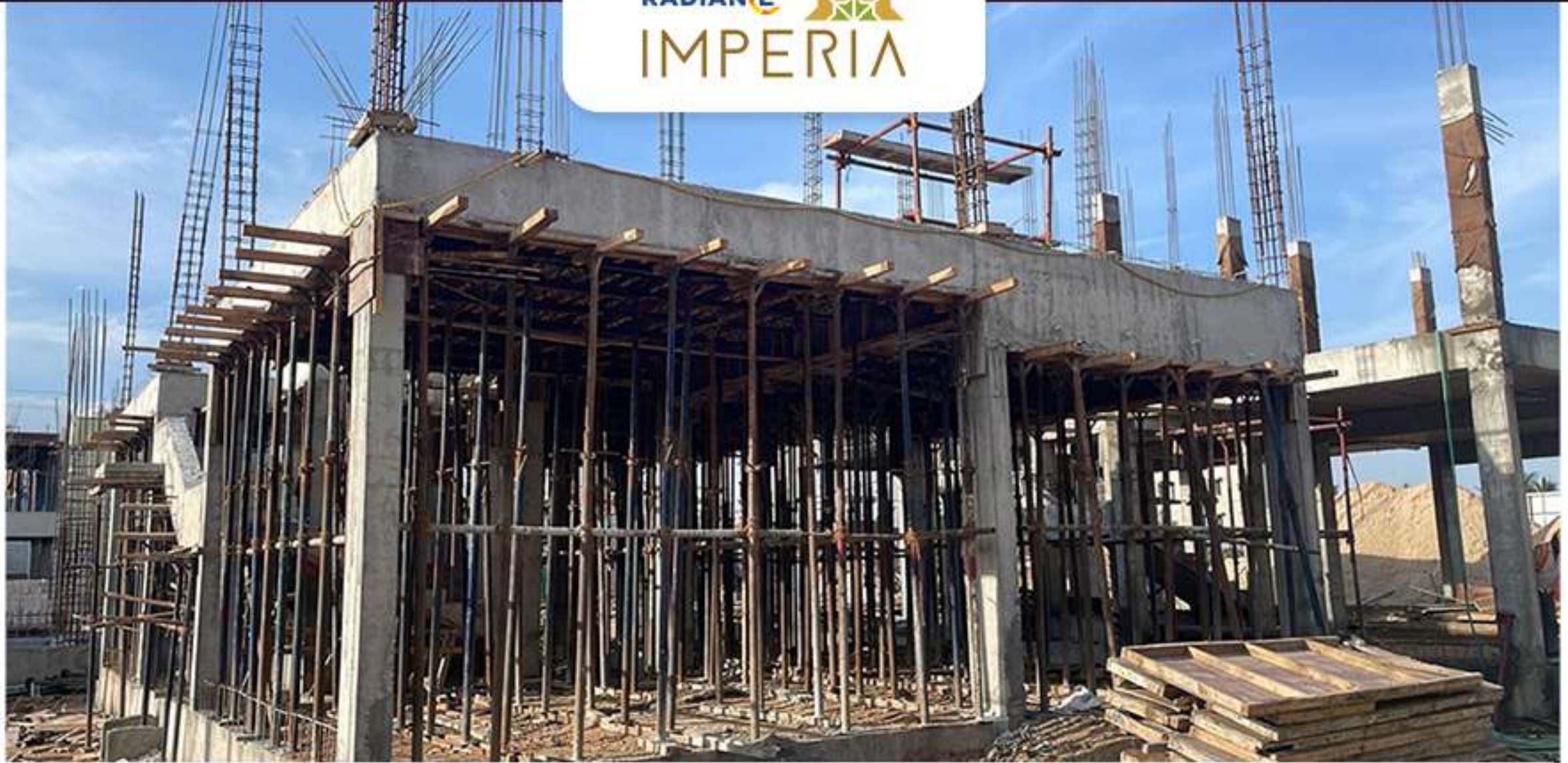
Villa no-30 – FF column shuttering Work in Progress
