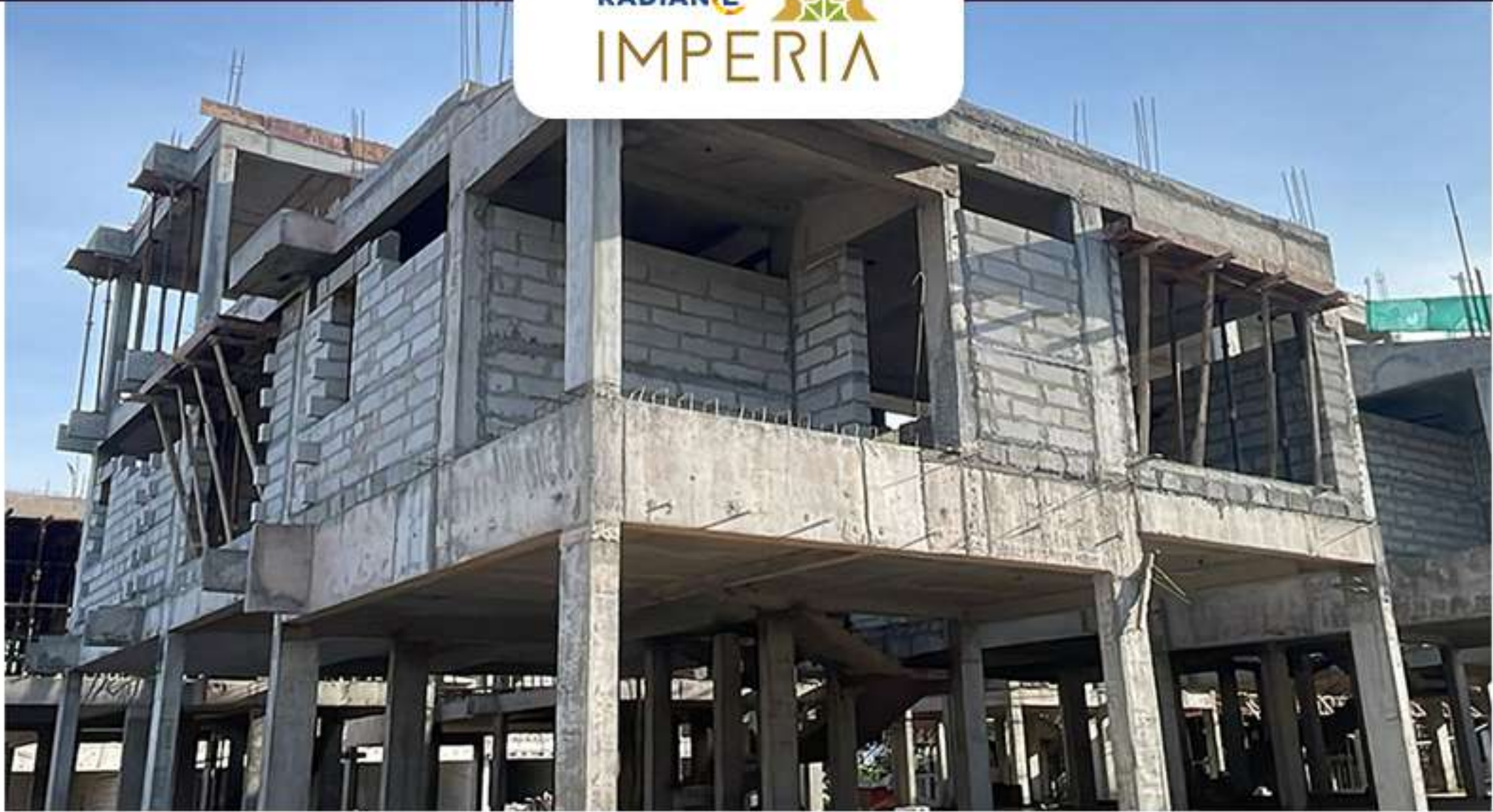
Villa no -39 First floor Block work in progress.
