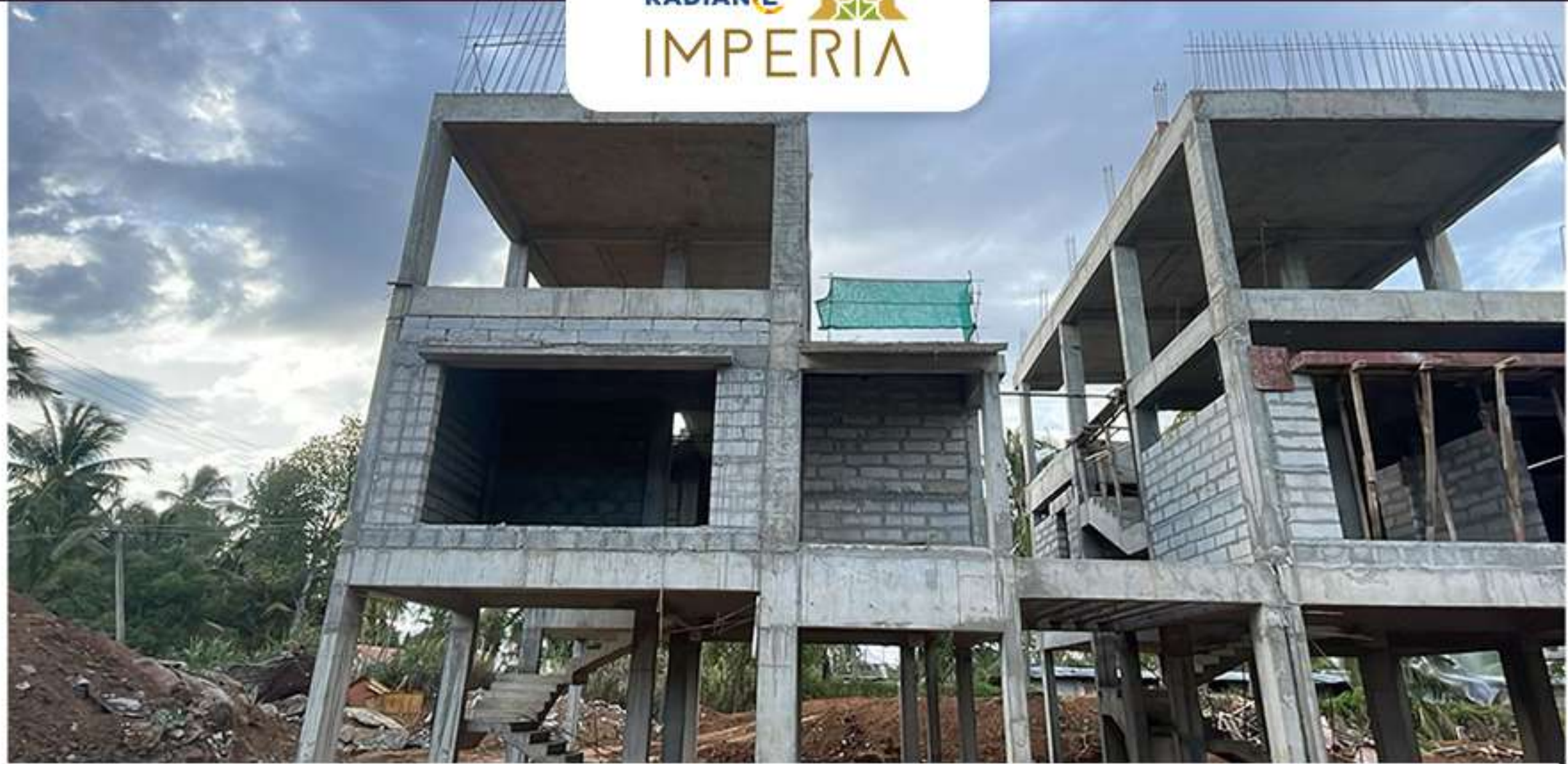
Villa no – 88 – Block work in progress.
