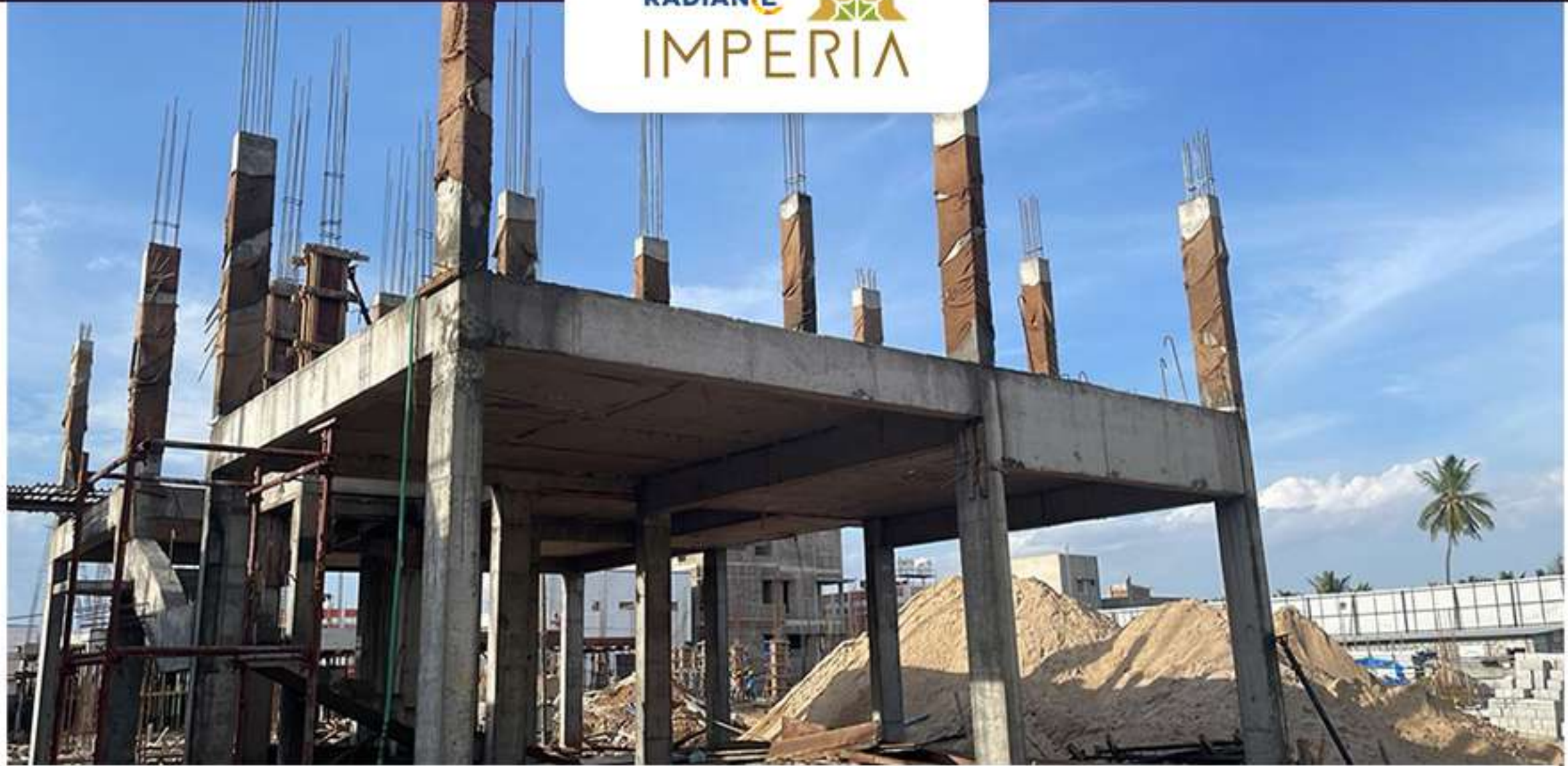
Villa no-31 – FF column completed.
