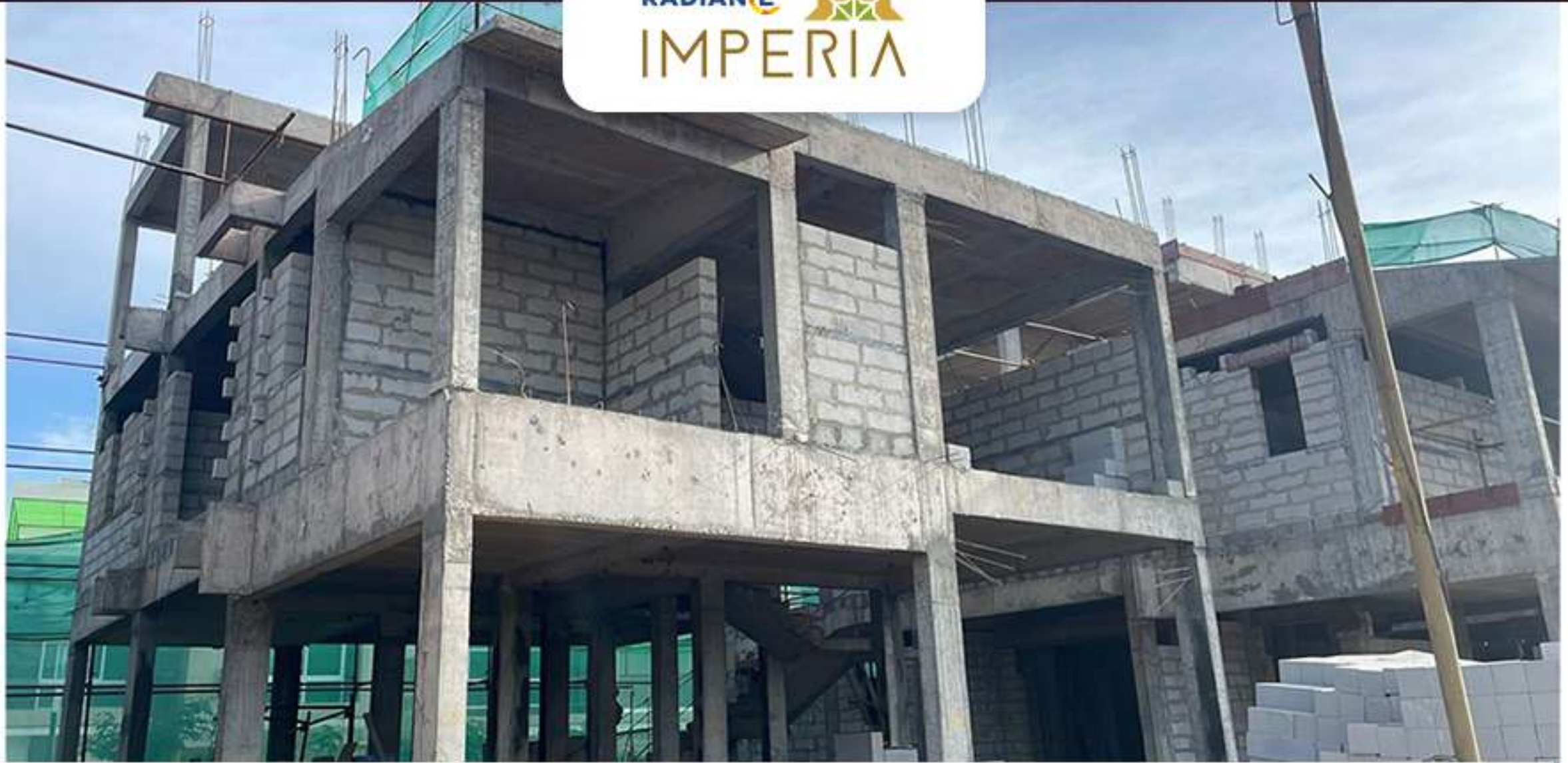
Villa no. 2 – First floor Block Work in Progress
