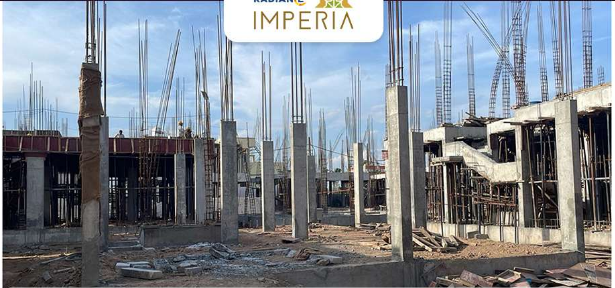
Villa no -29 GF Column completed
