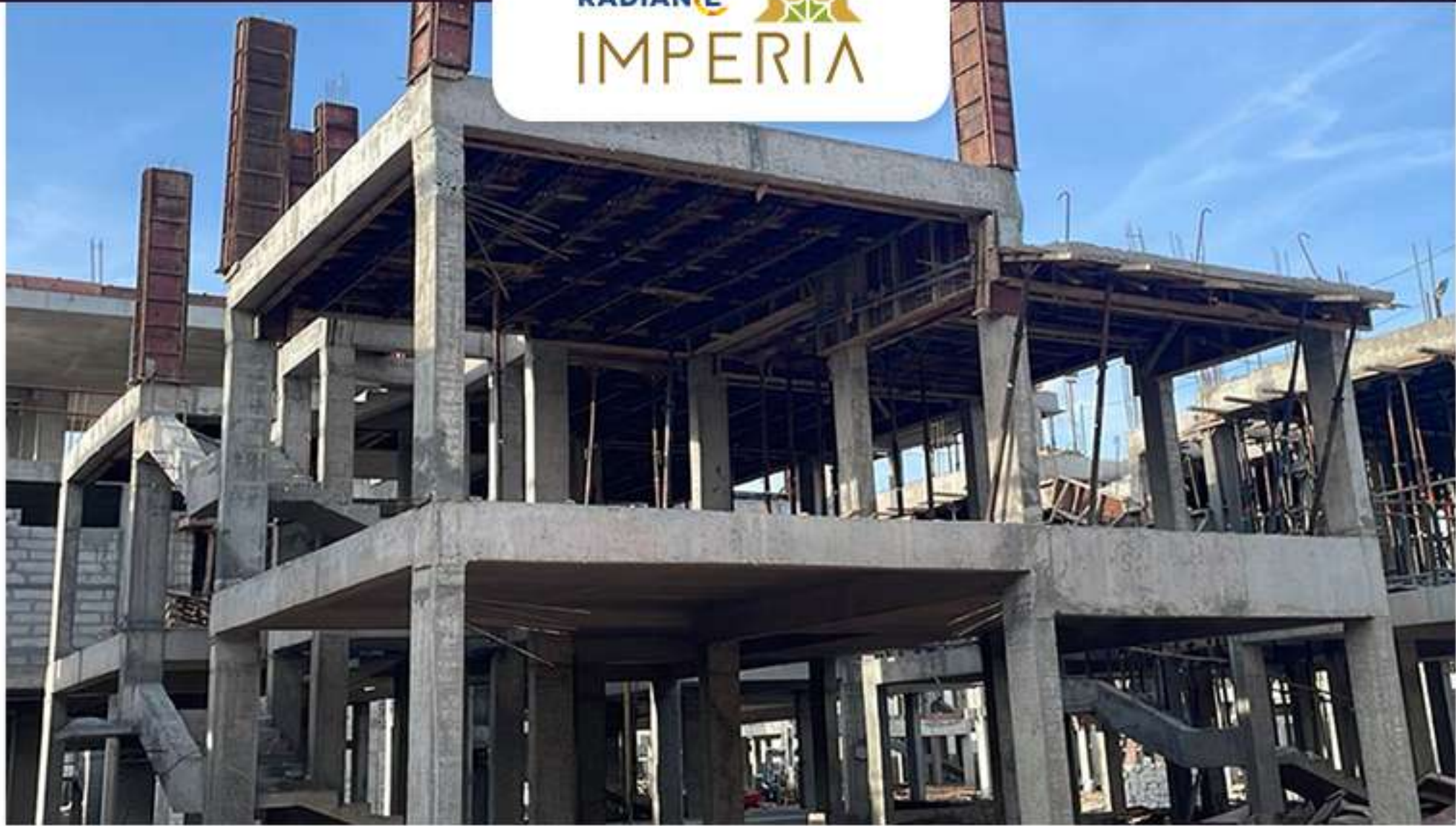
Villa no -22 – 2nd Floor column box fixing work
