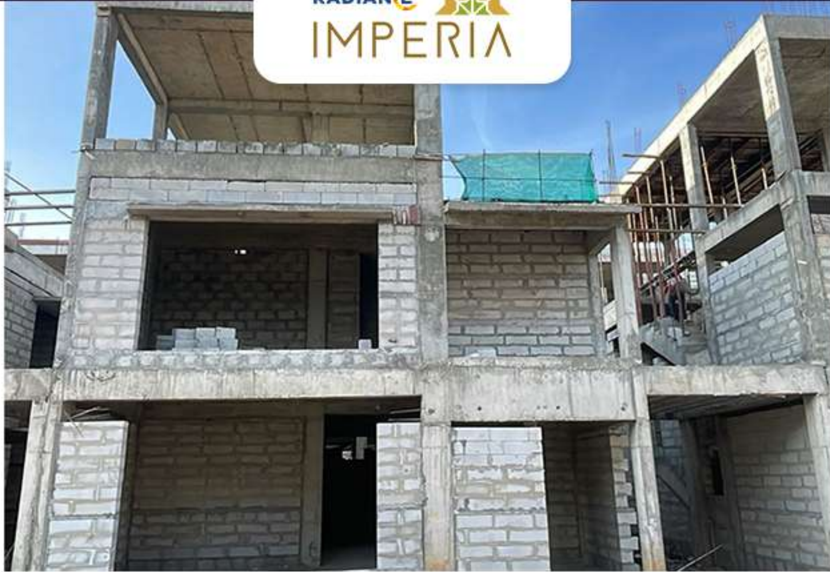
Villa no -50 – Block work in progres
