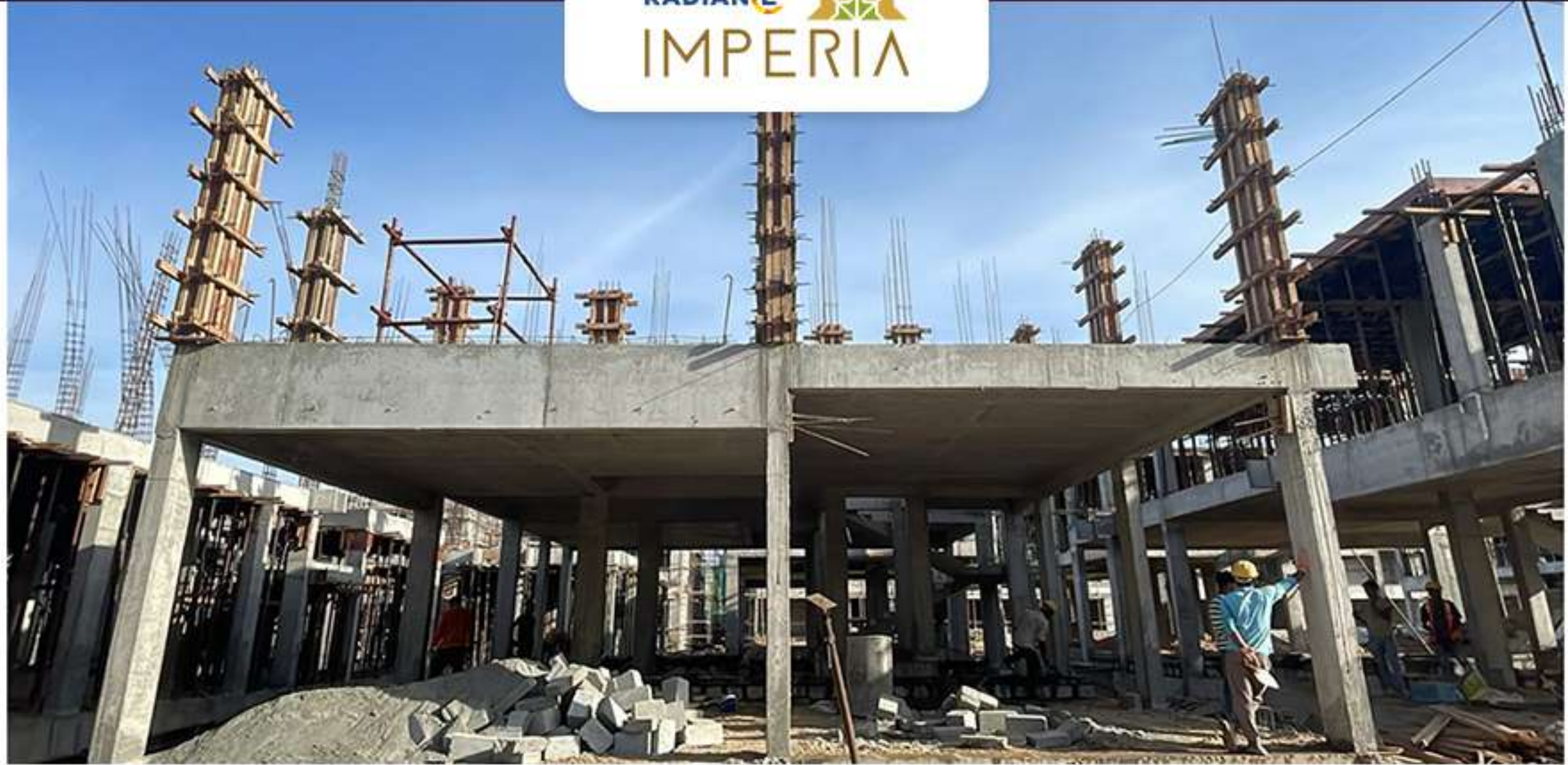
Villa no -37 – 1st Floor column Work in Progress.
