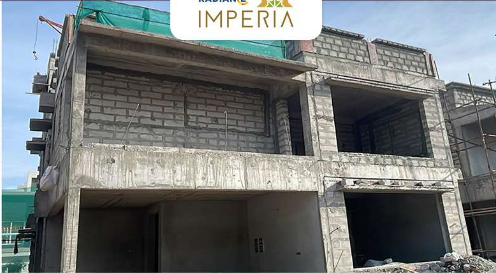
Villa no -16 Plastering Work in progress.
