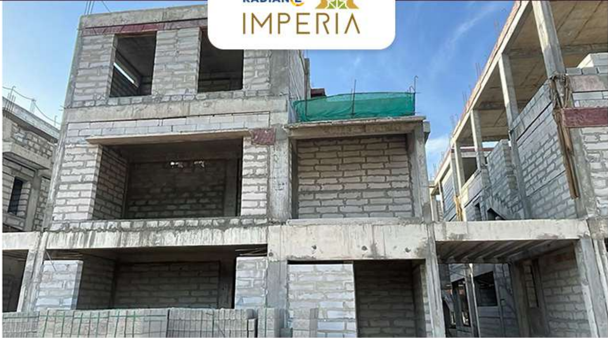
Villa no – 47 - Block Work in progress.
