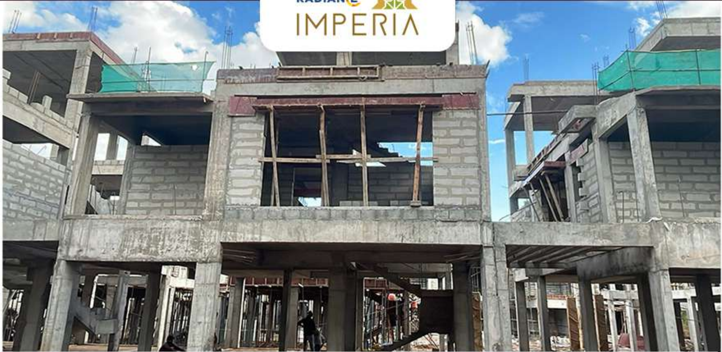
Villa no – 83 – Block work in progress
