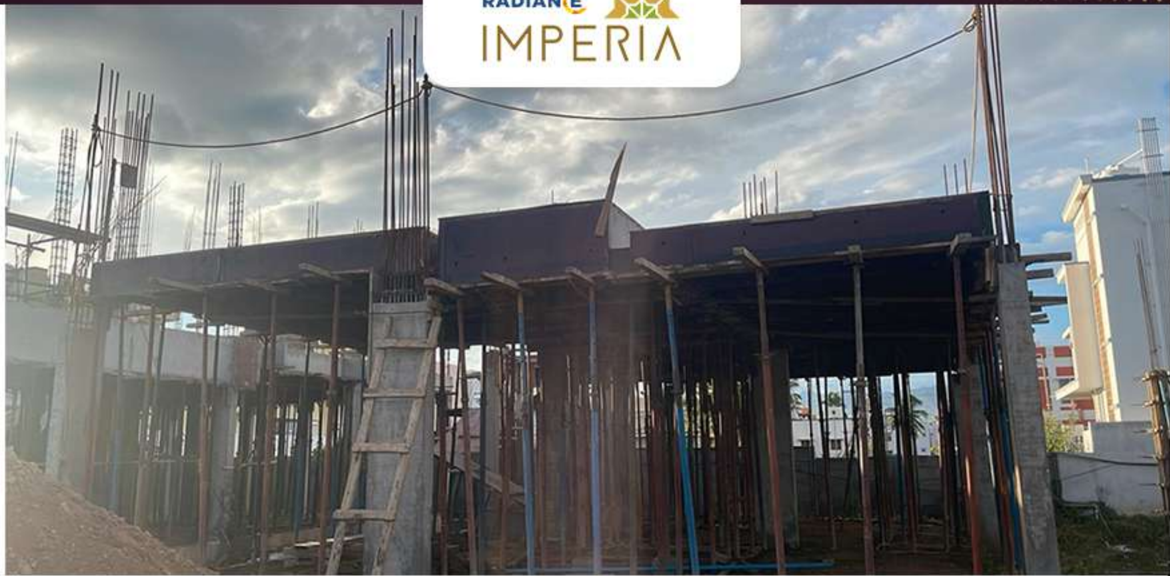
Villa no 61 Ground Floor slab shuttering Work in Progress.☑
