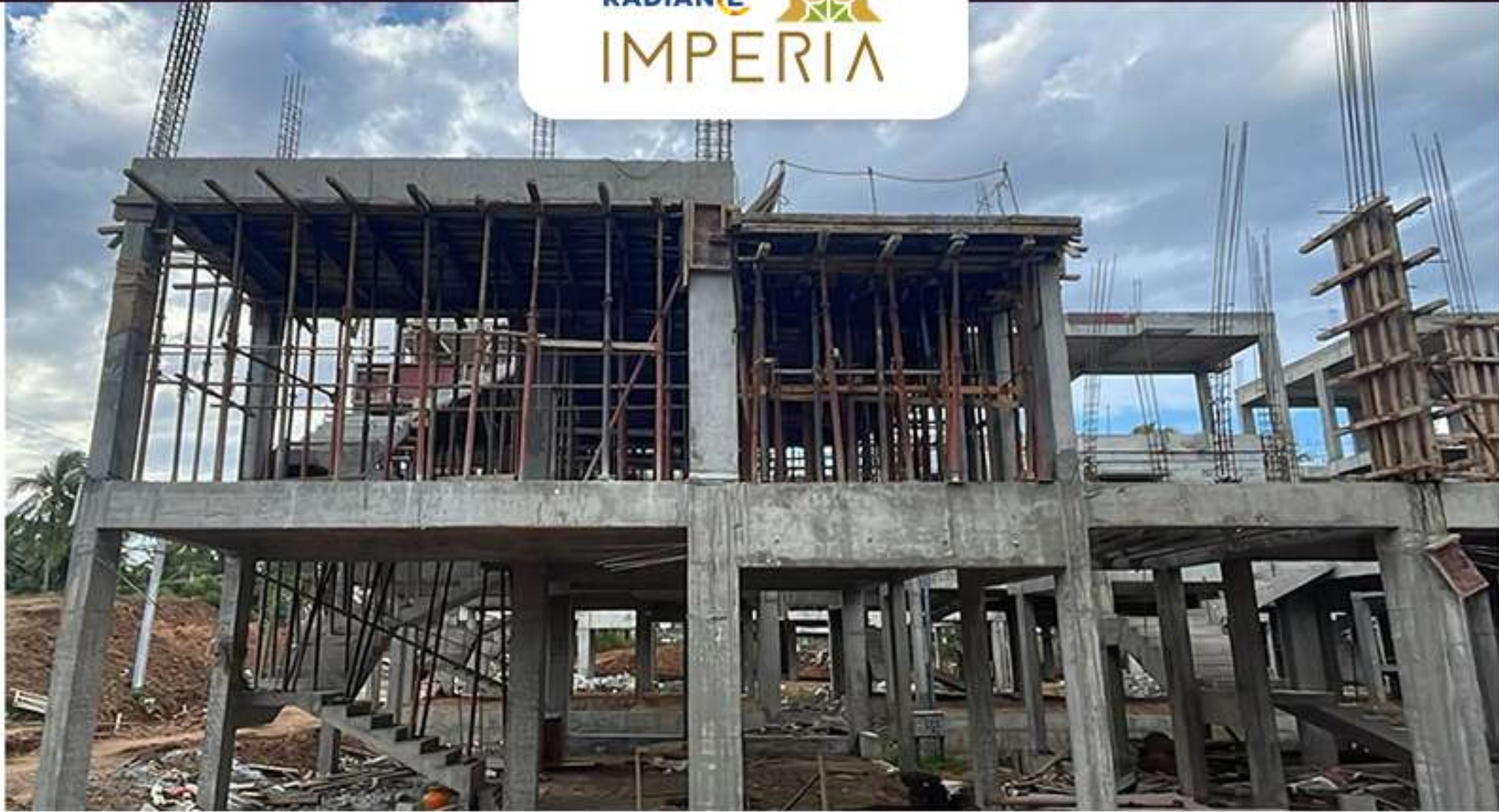
Villa no -73 SF Column reinforcement Work in Progress.
