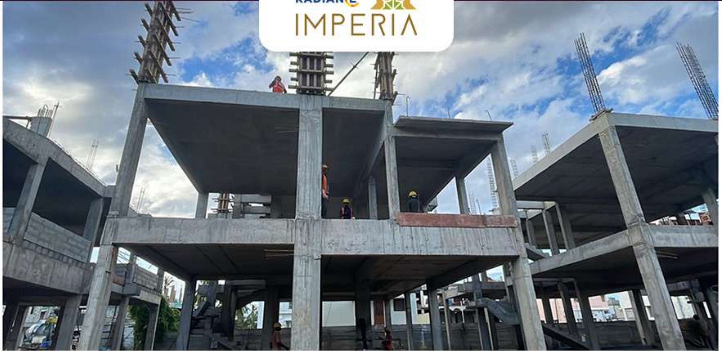
Villa no -54 – 2nd Floor column Work in Progress.
