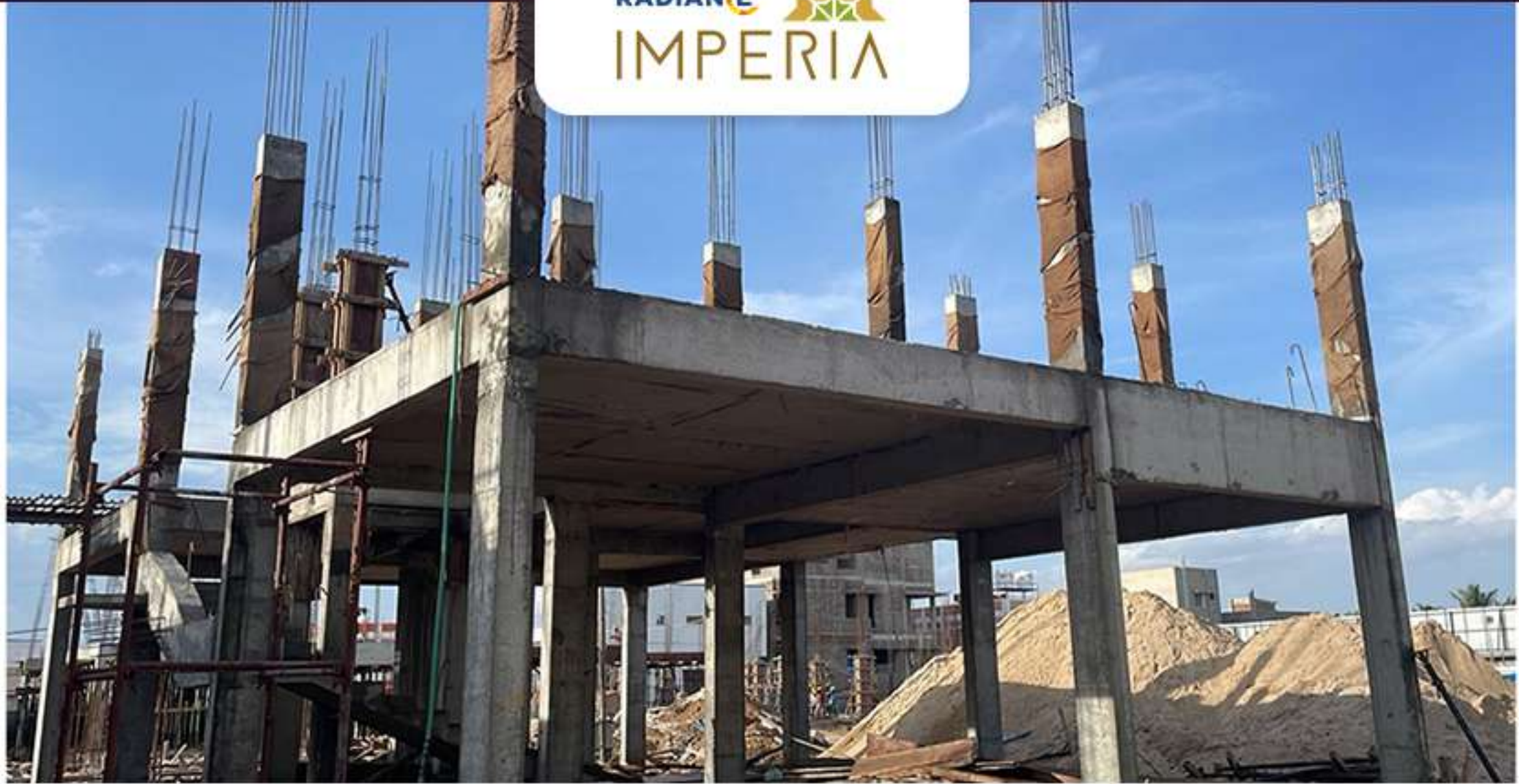
Villa no. 31 – 1st floor Column completed
