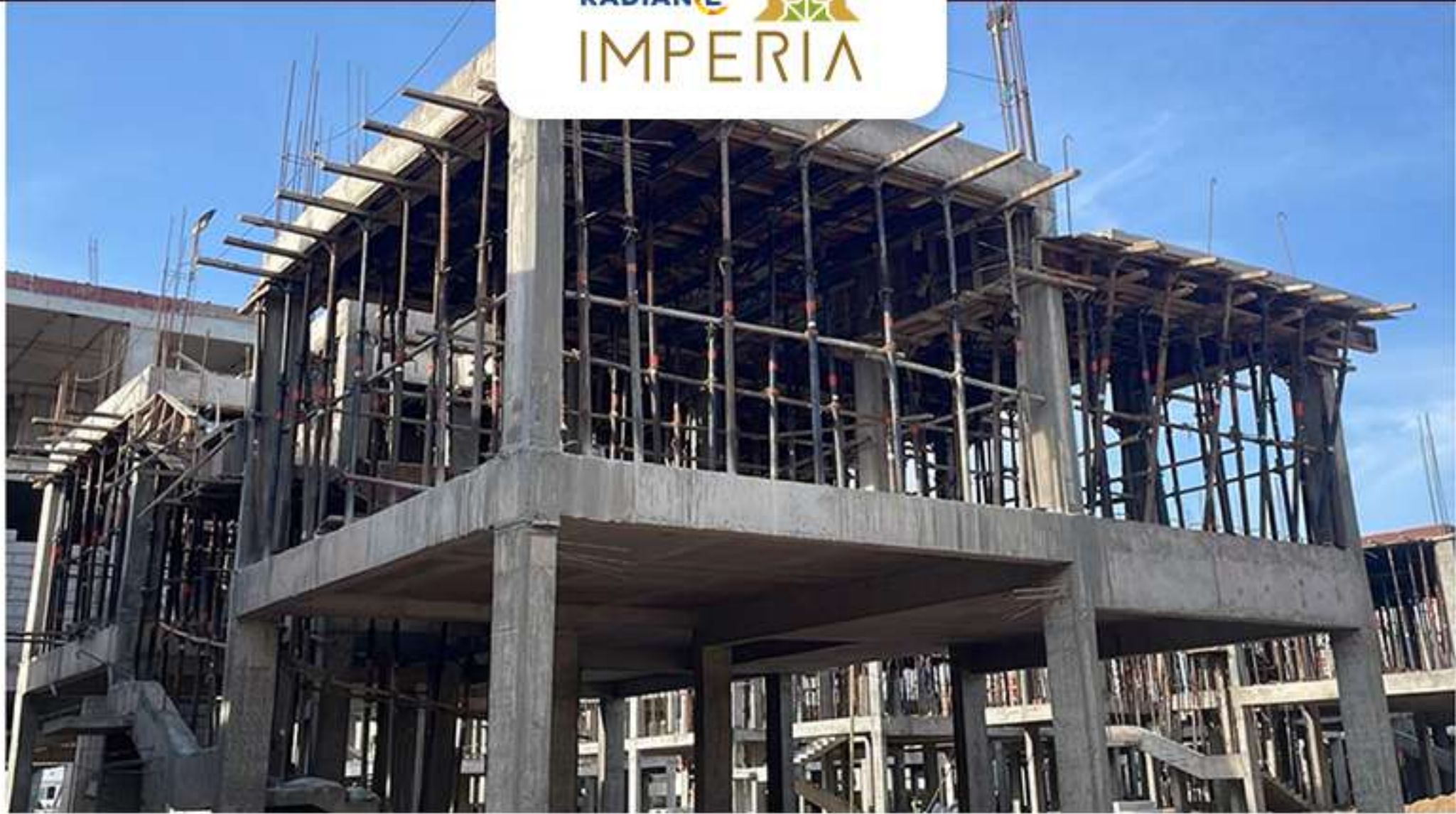
Villa no -23 – 1st Floor roof slab completed.
