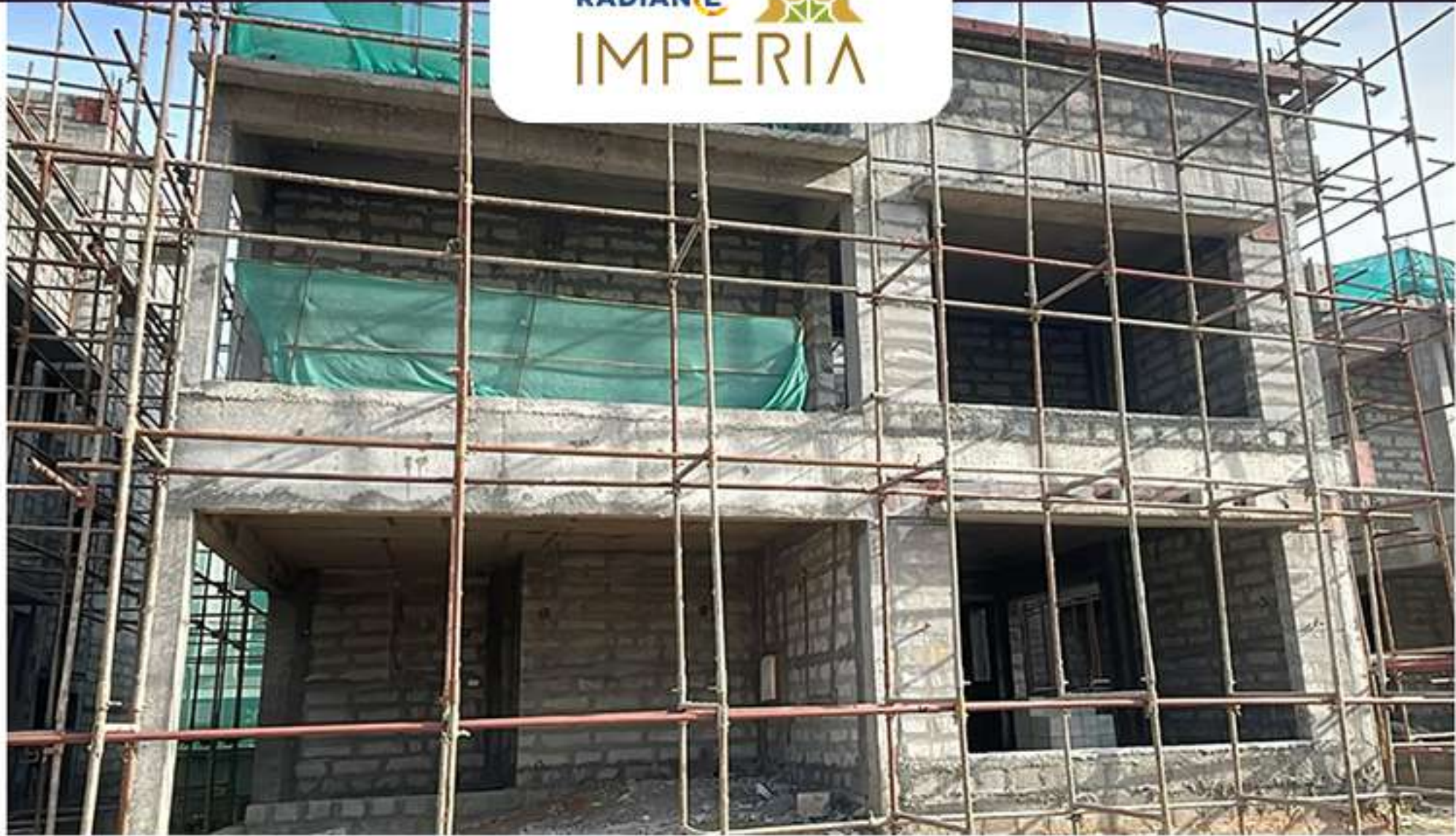
Villa no -10 Block Work Completed.
