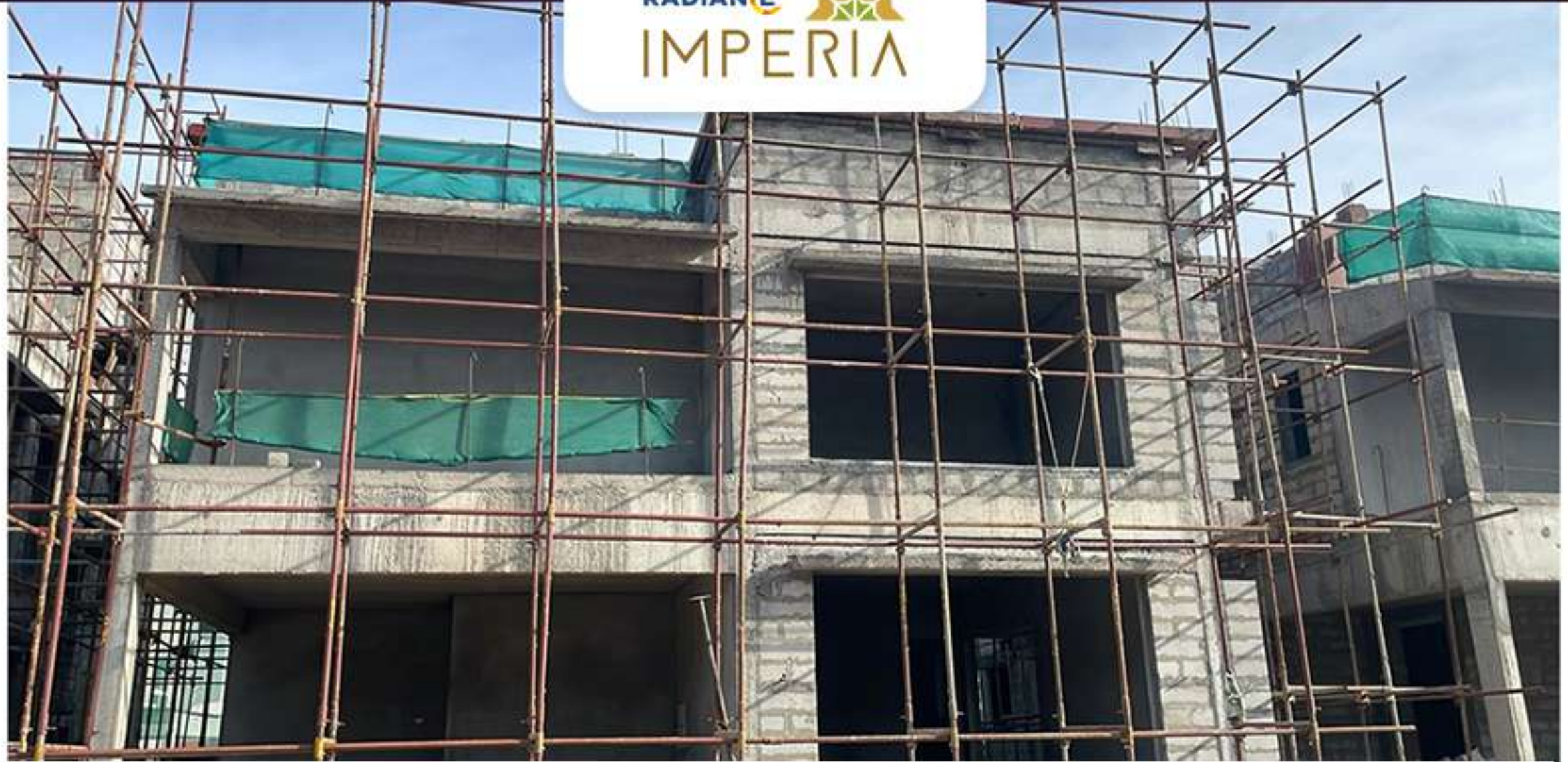
Villa no -12 Plastering work in progress
