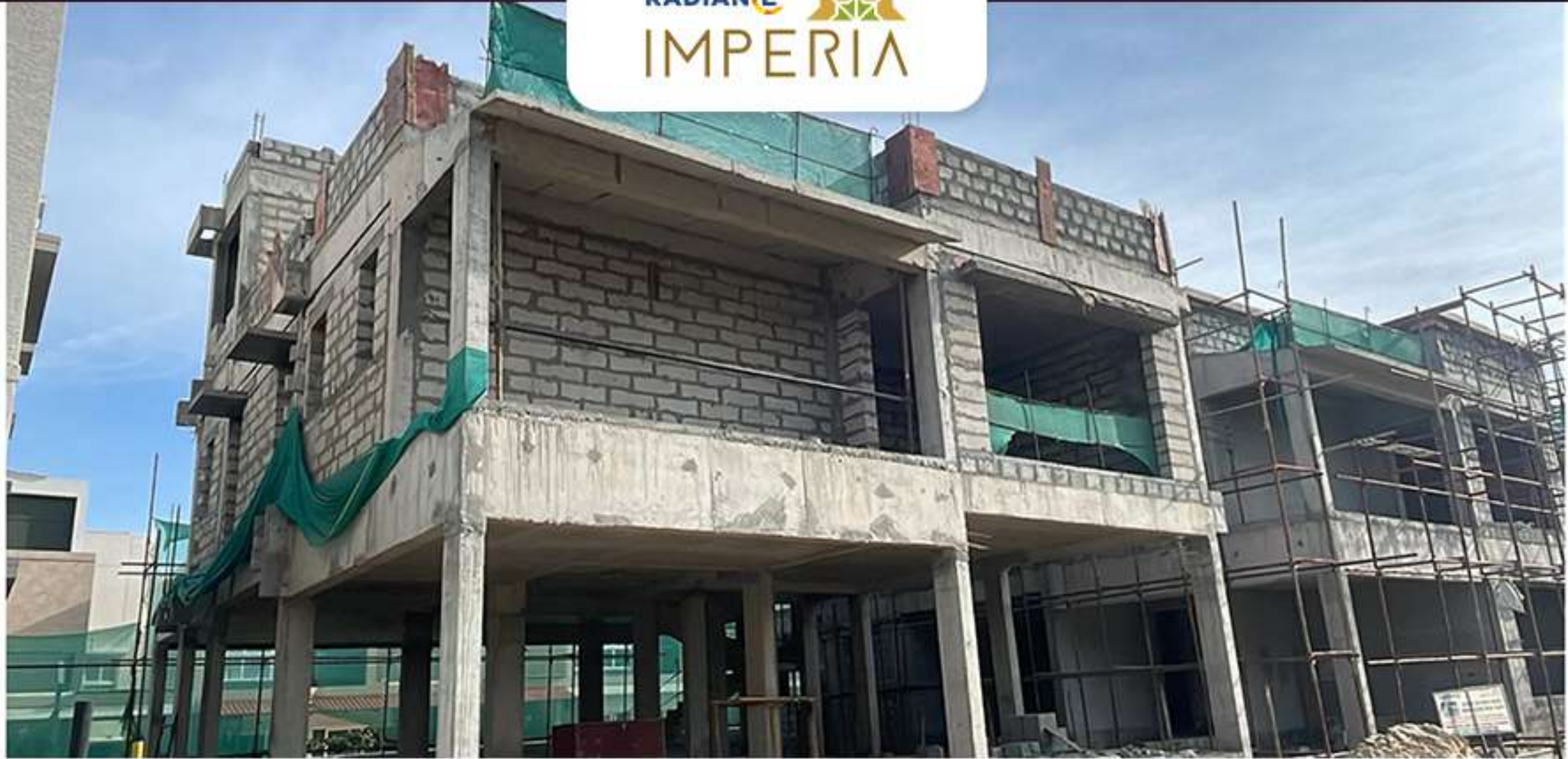
Villa no. 6 Block Work in progress.
