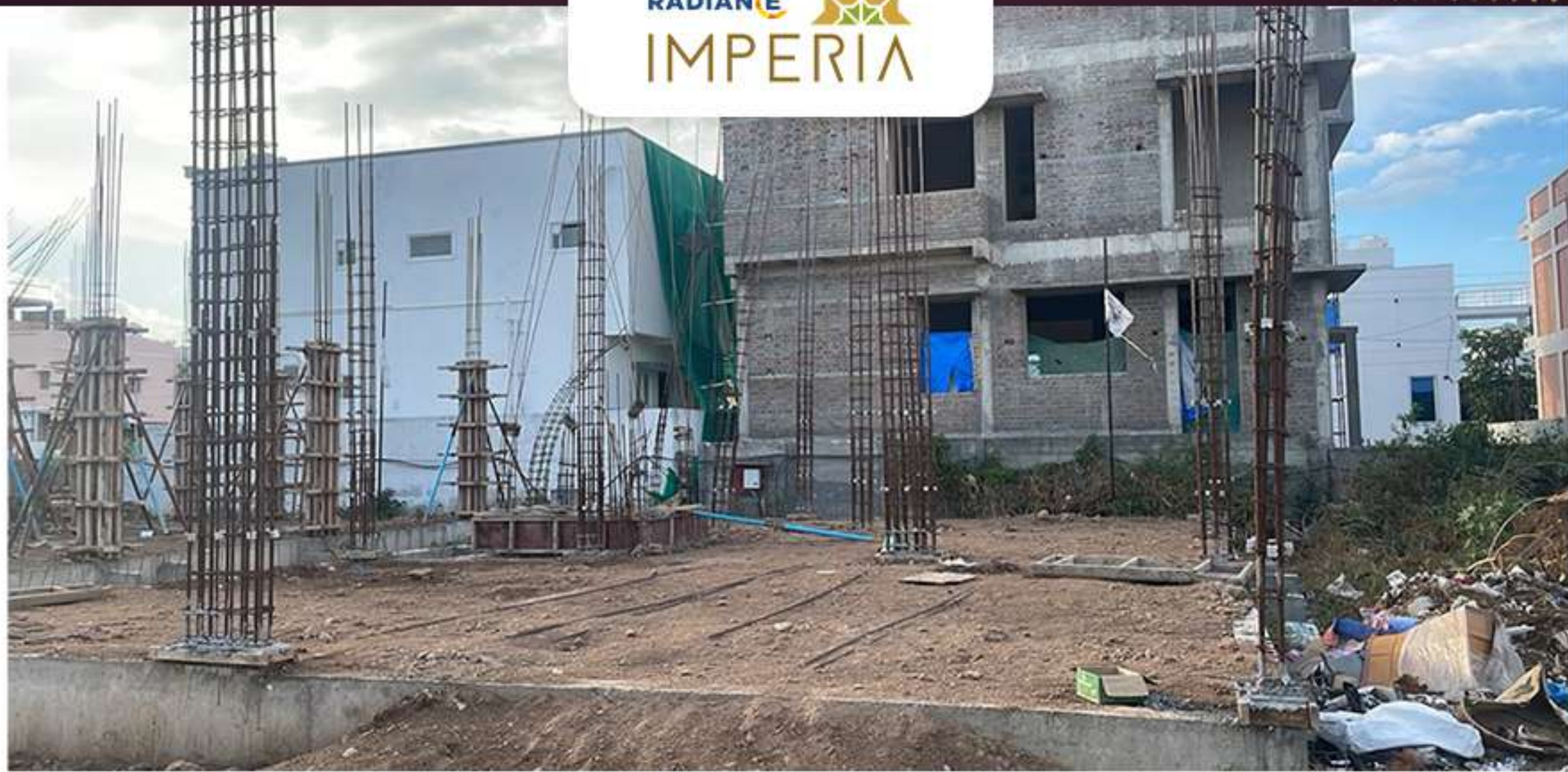
Villa no 64 – GF Column work in progress
