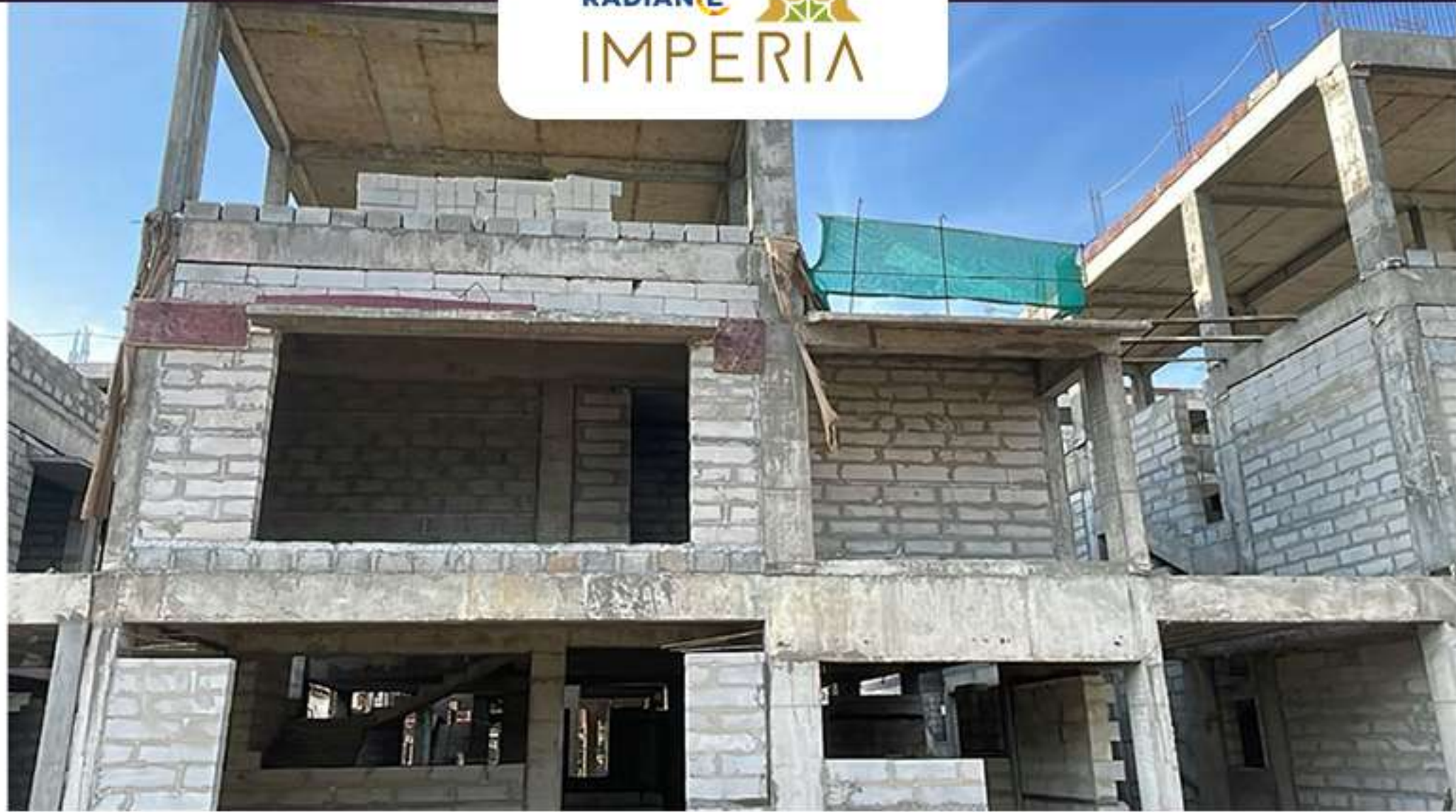
Villa no -48 Block Work in progress.
