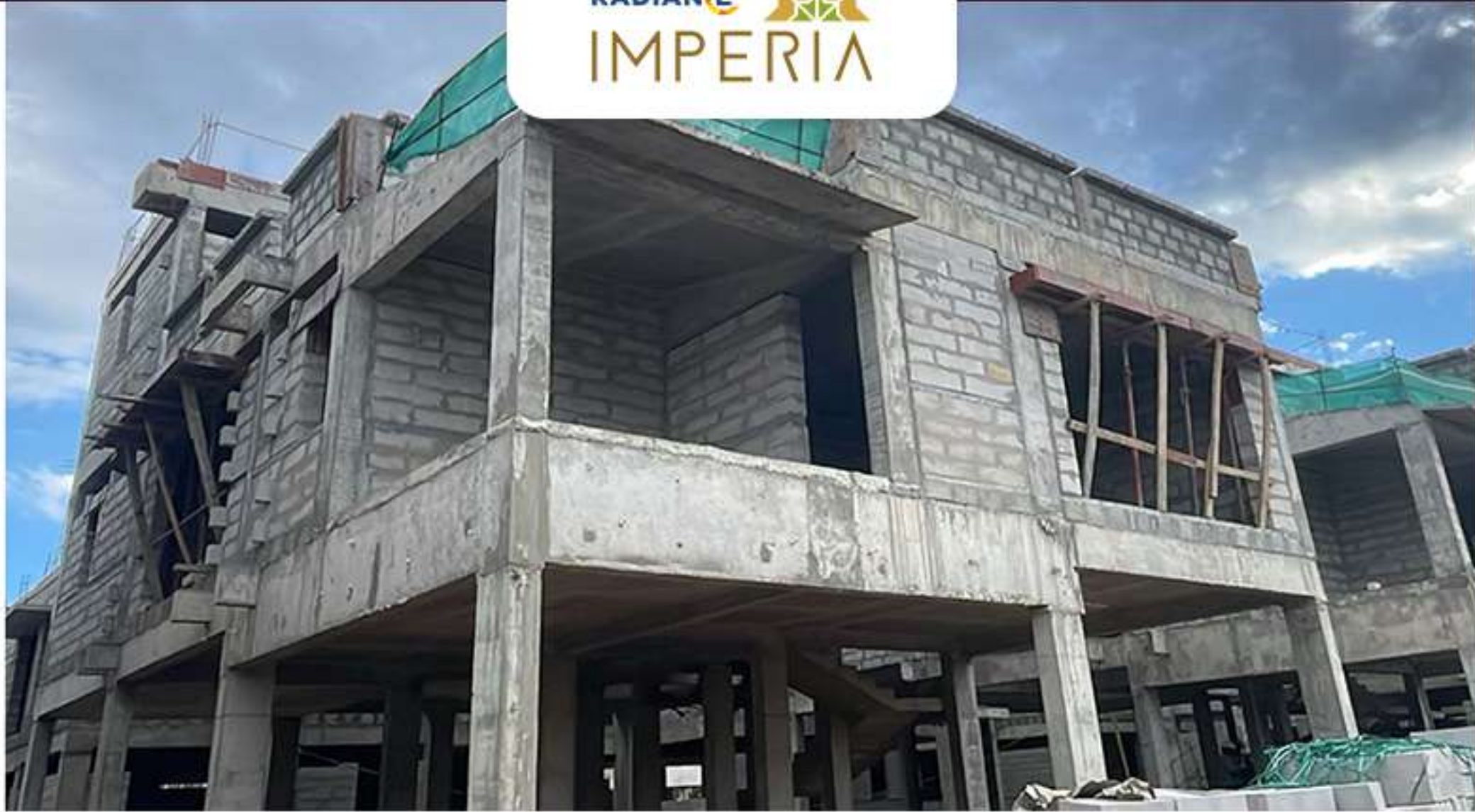
Villa no -66 – Block Work in progress.
