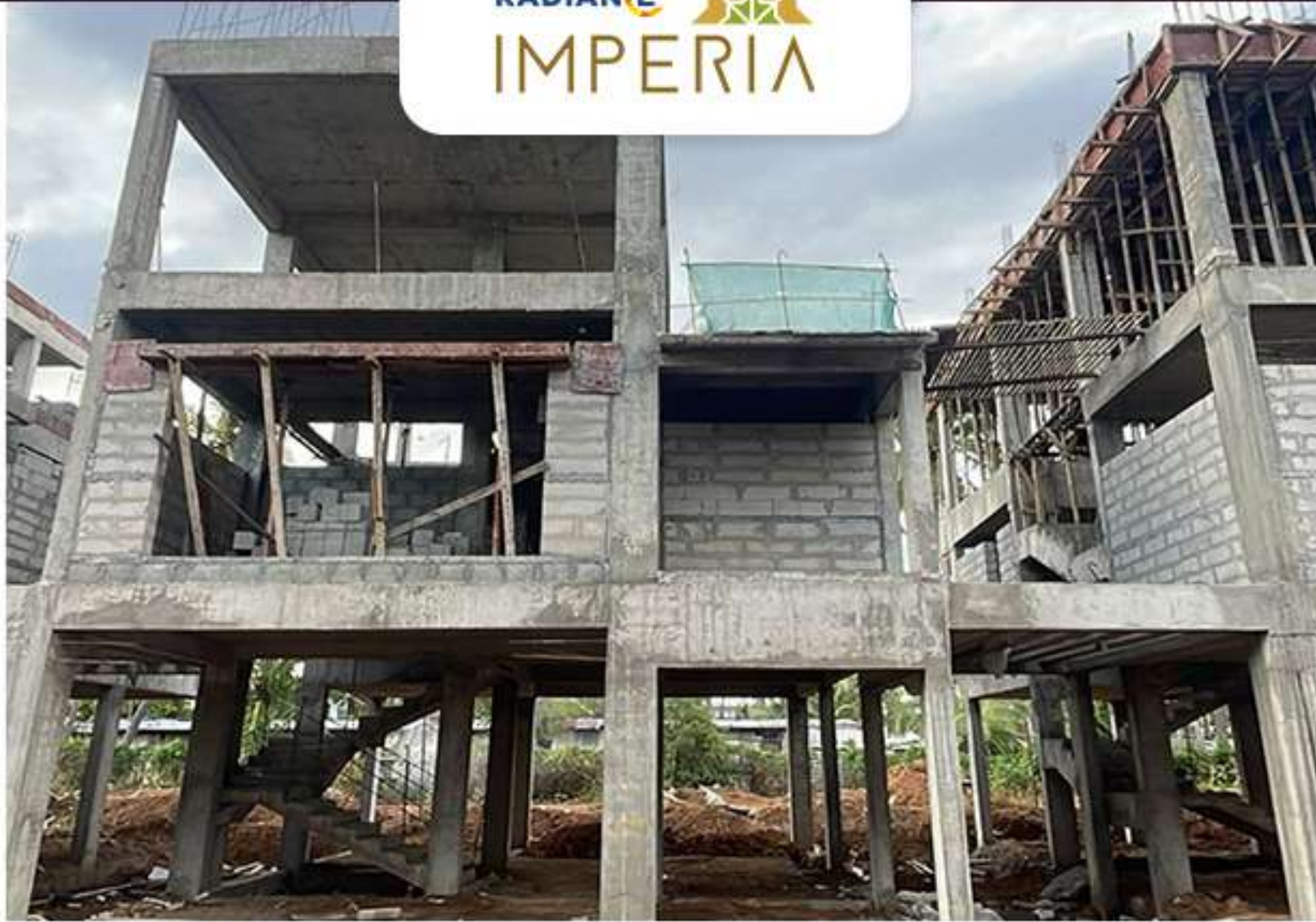
Villa no – 92 – Block Work in Progress
