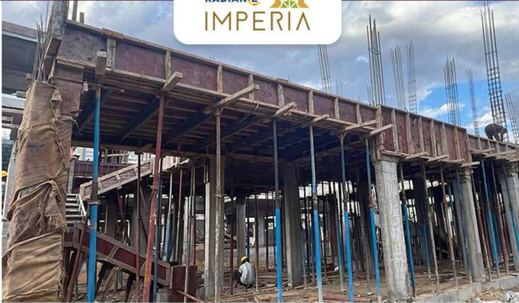
Villa no -77 – GF roof slab work in progress
