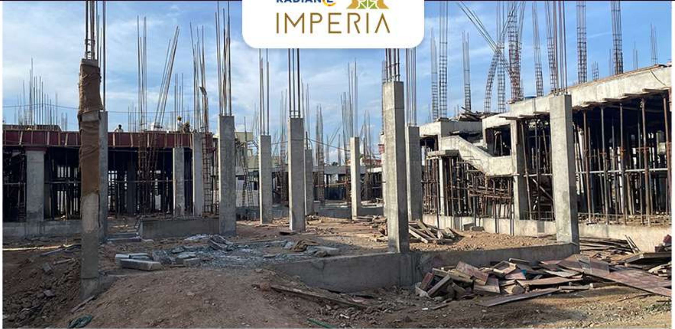
Villa no-29 – GF Column completed.
