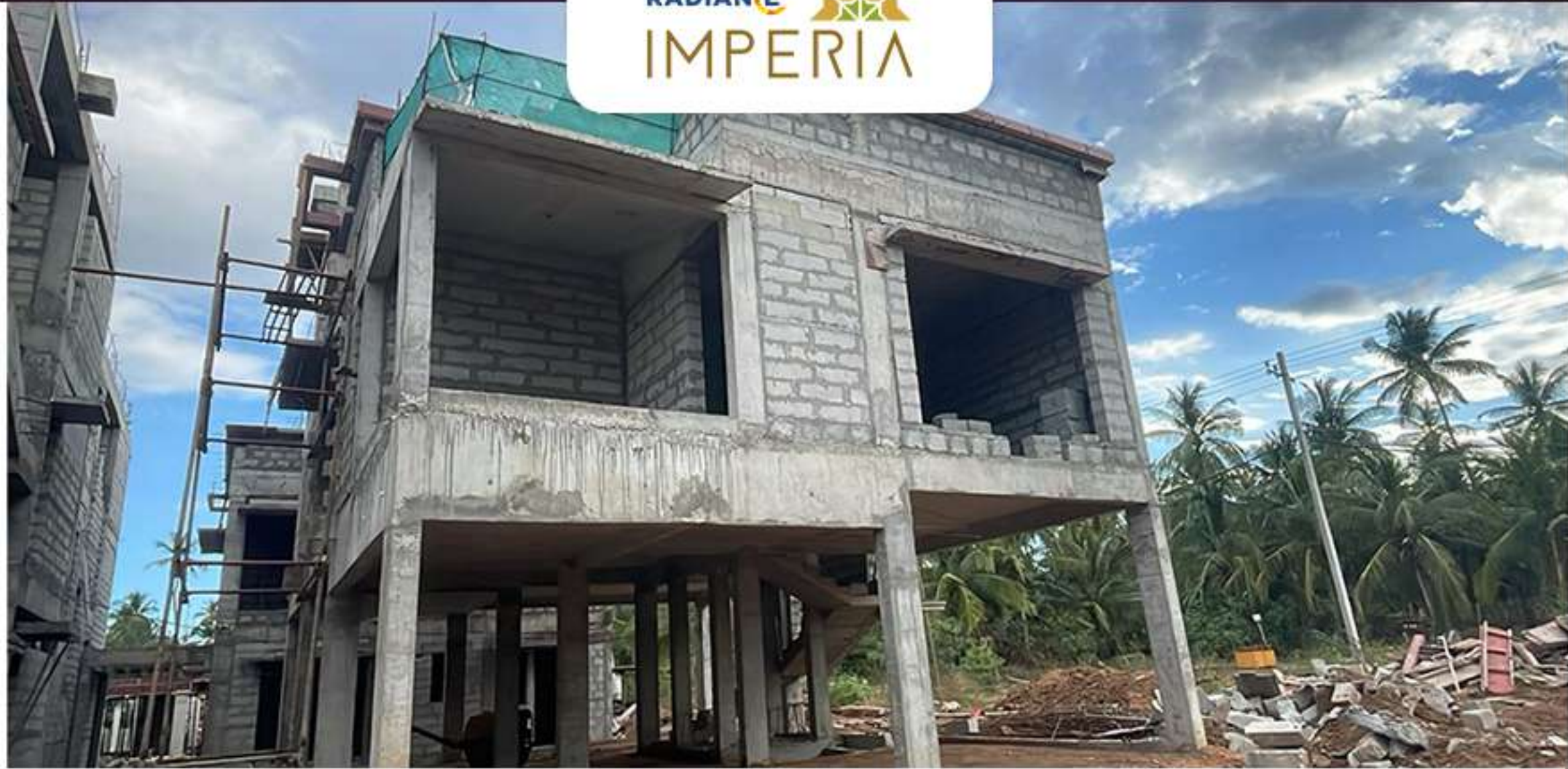
Villa no -72 block Work in progress.
