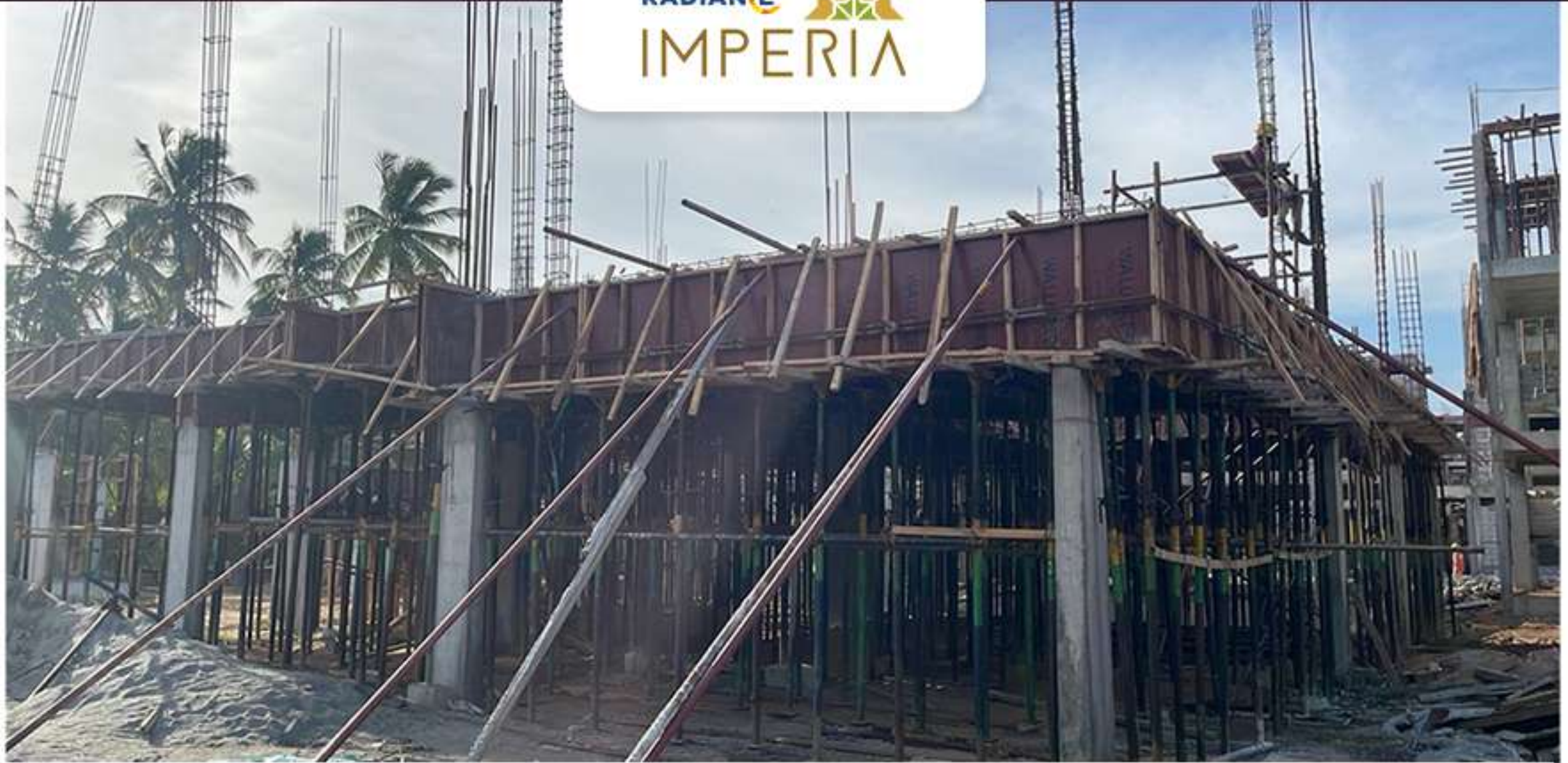
Villa no -20 1st Floor Column reinforcement work in progress.
