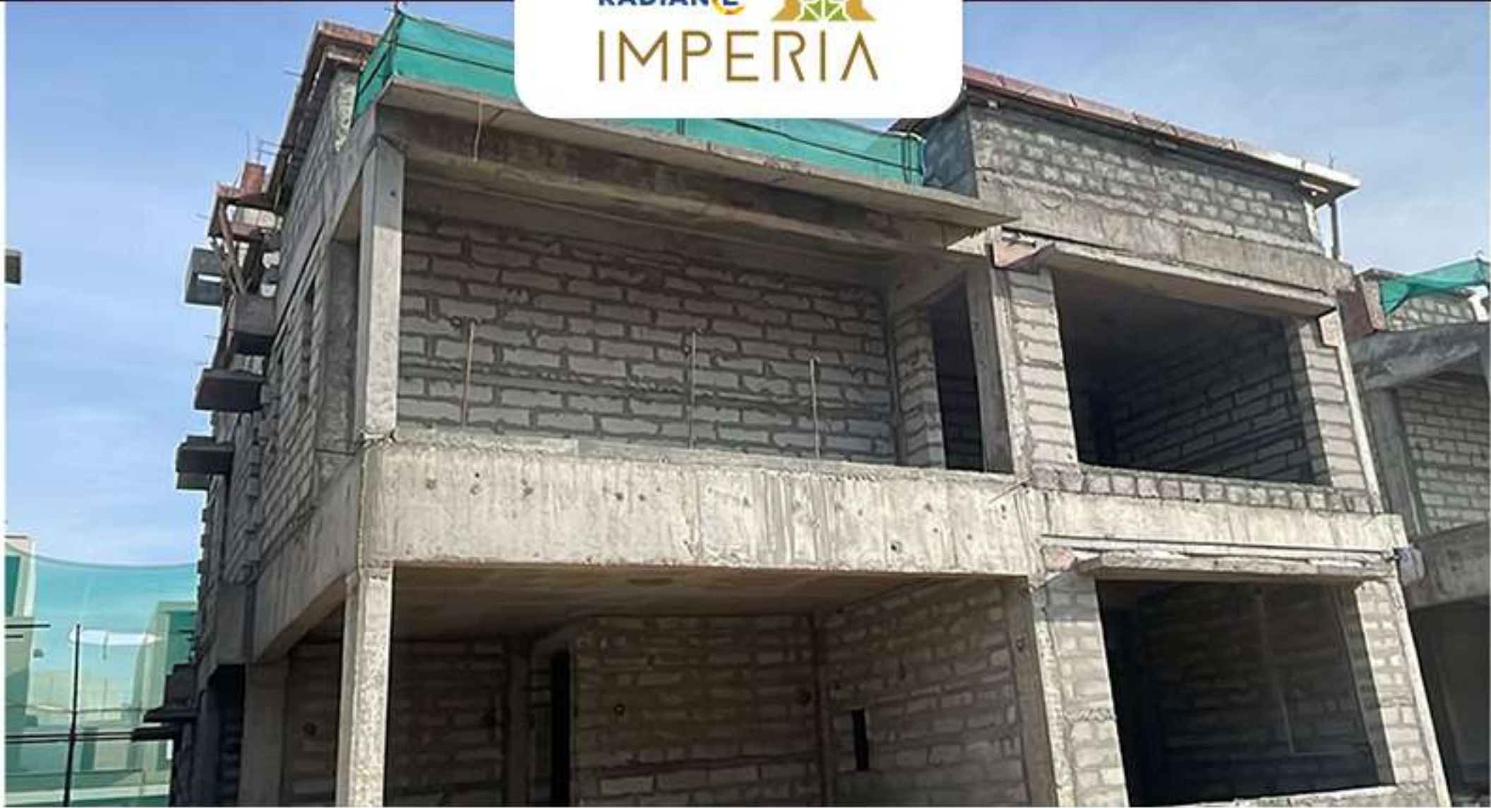
Villa no -15 Block Work completed
