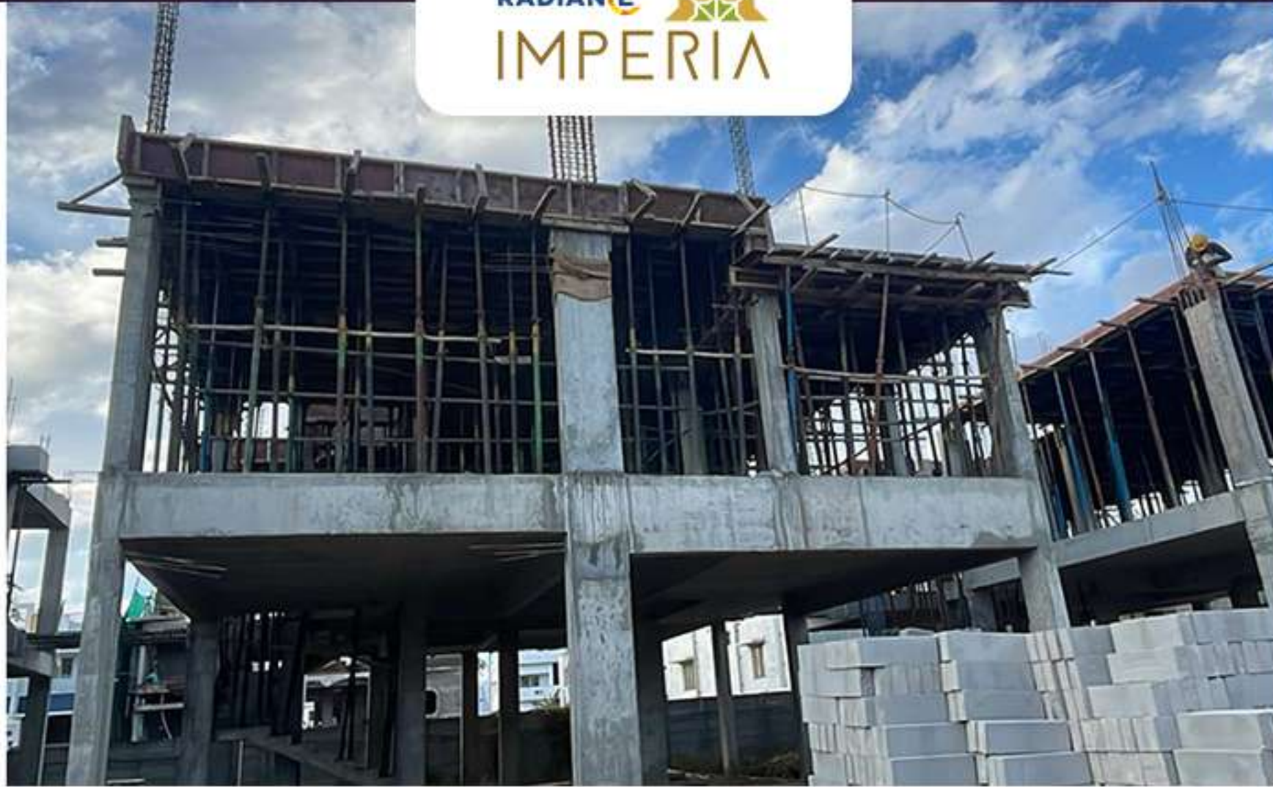
Villa no -56 – FF Roof slab work in progress
