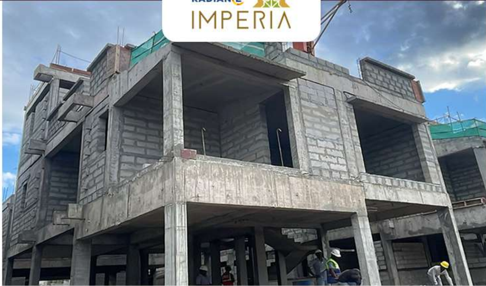
Villa no -68 – Block work in progress.
