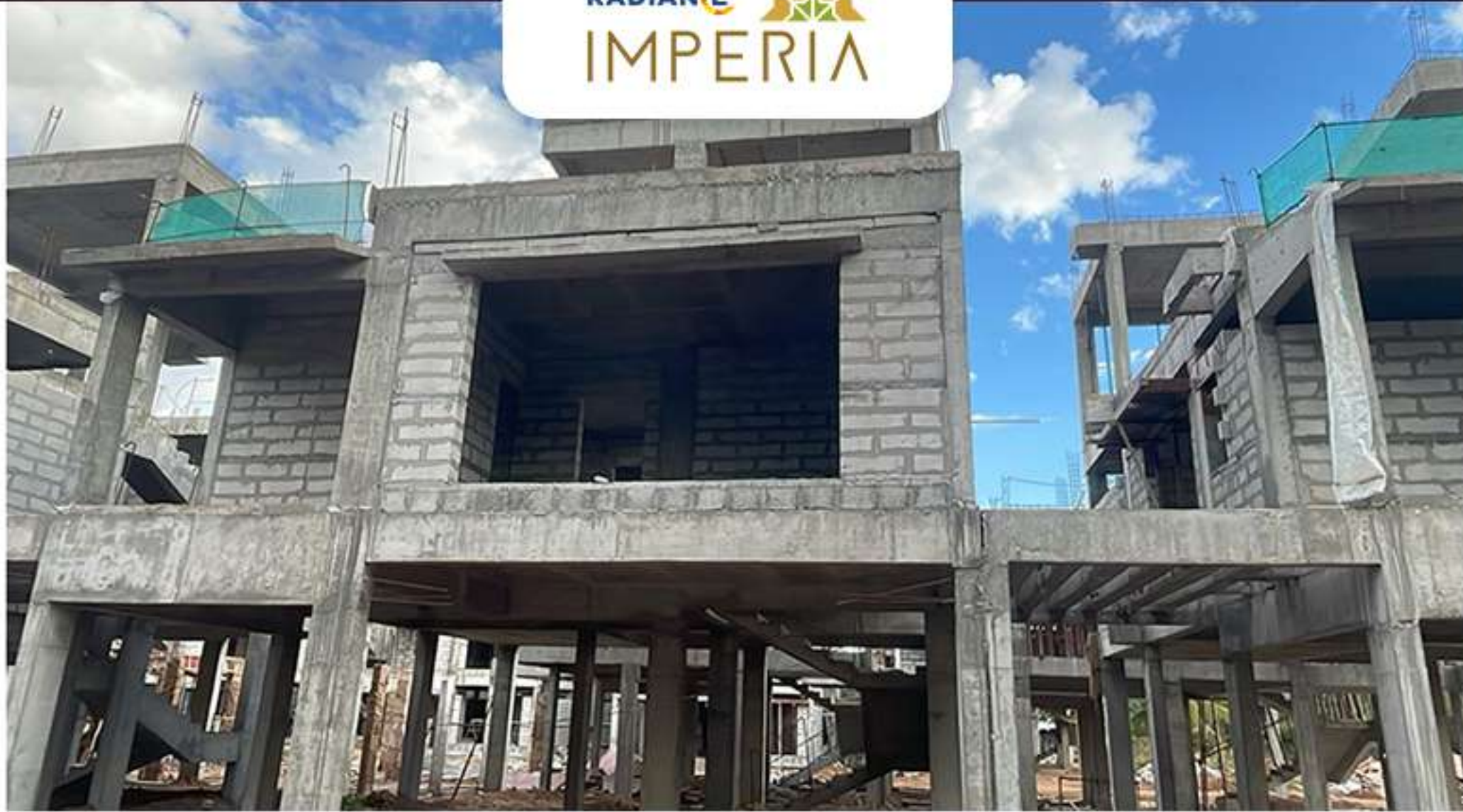
Villa no – 86 – Block work in progress
