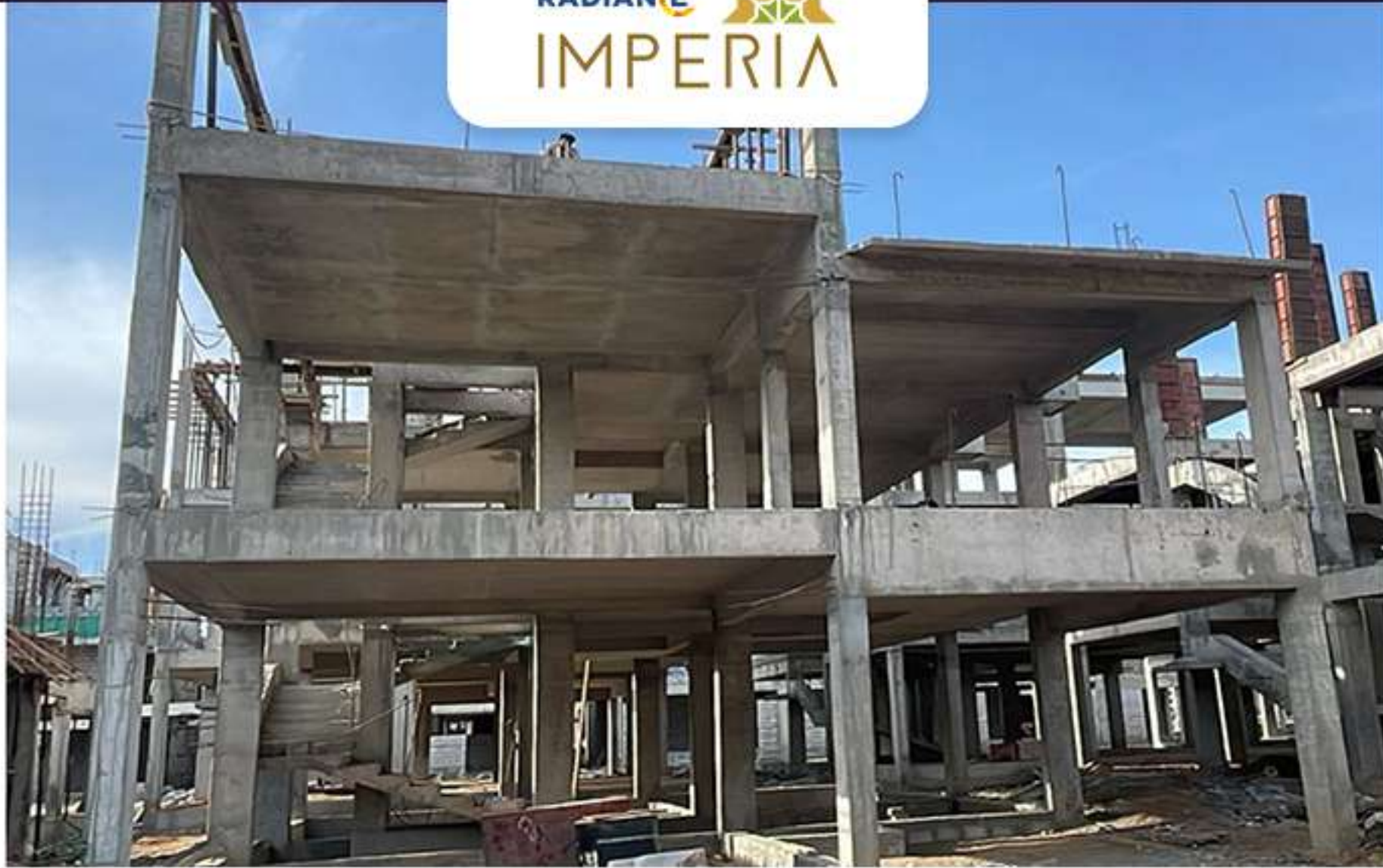
Villa no -21 – 2nd Floor roof shuttering Work in Progress.
