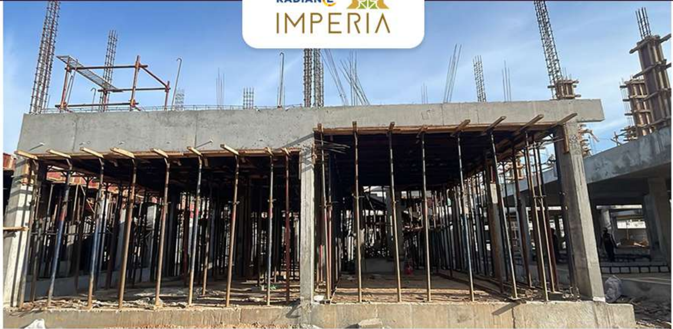
Villa no -36 – FF Column reinforcement Work in Progress.
