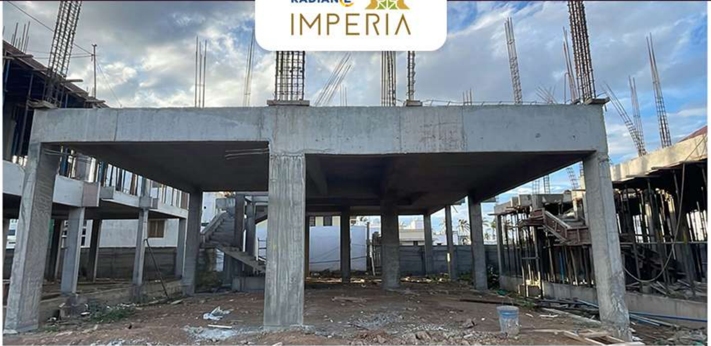
Villa no -59 FF Column Completed.
