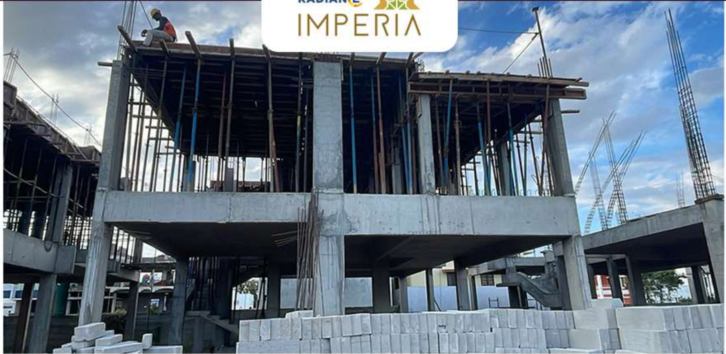
Villa no -57 1st Floor Slab Work in Progress.
