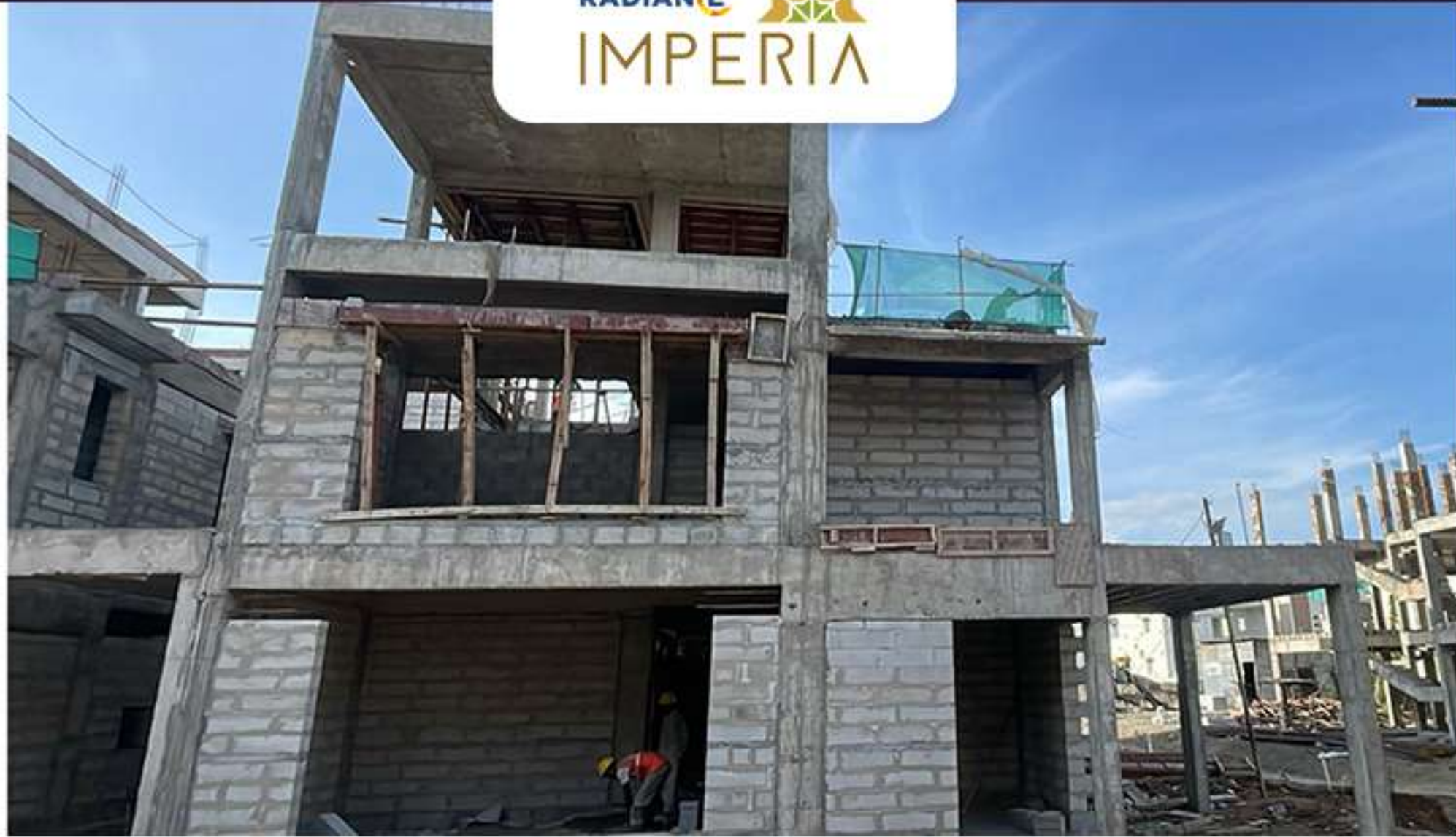
Villa no -51 – Block work in progress.
