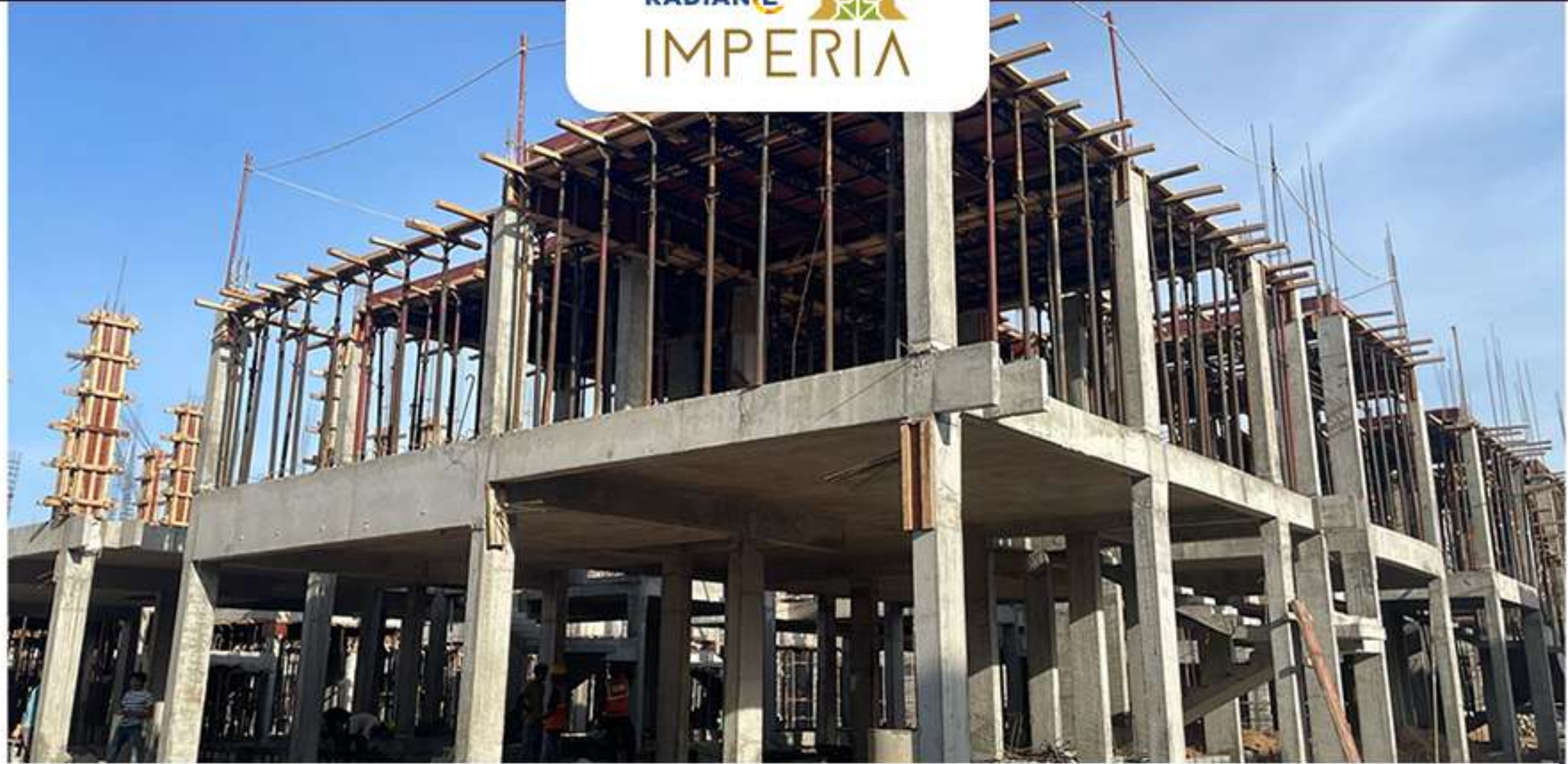
Villa no – 38 – FF roof slab shuttering Work in Progress.
