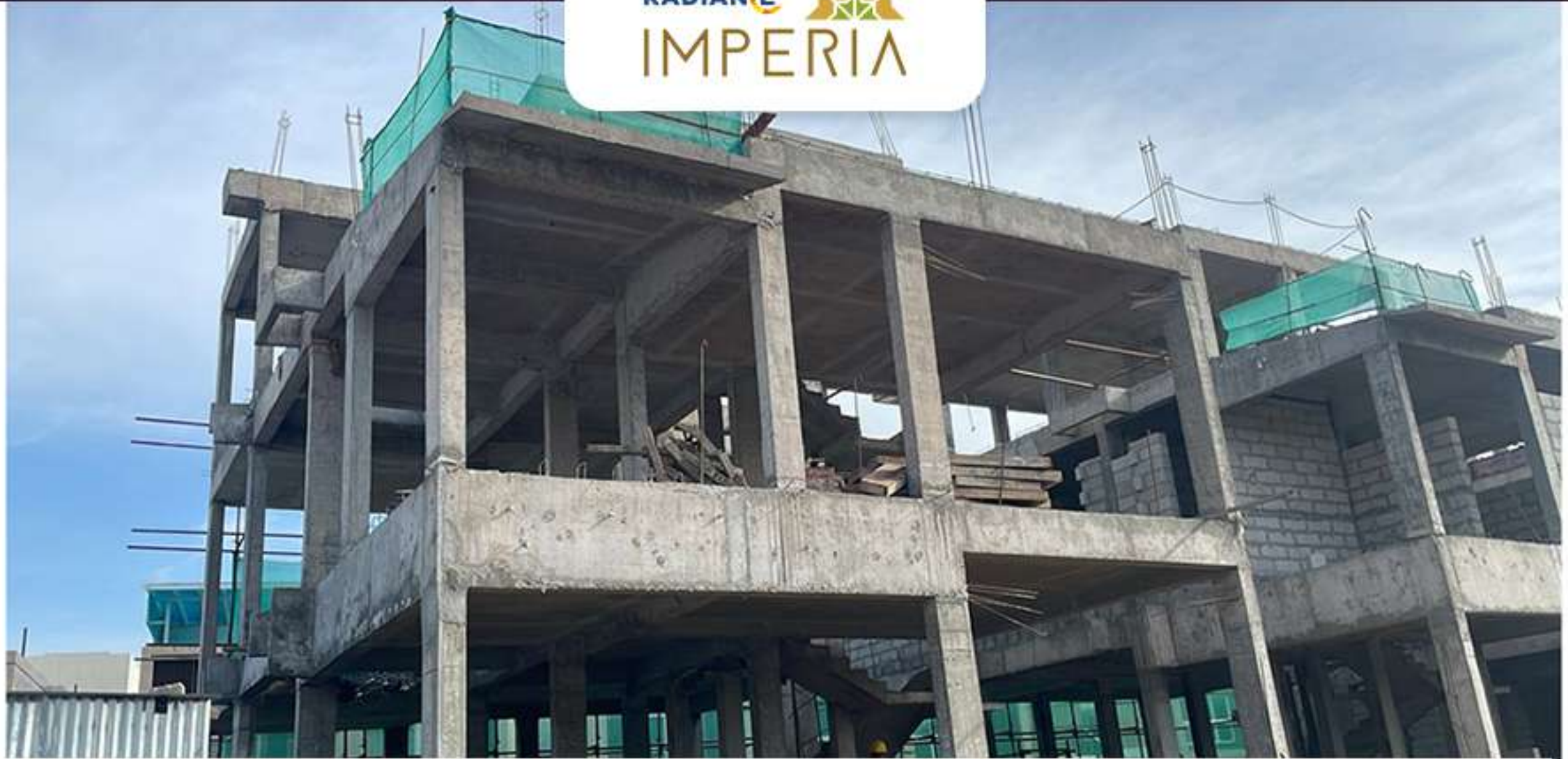
Villa no. 1 – Grade slab preparation Work in Progress
