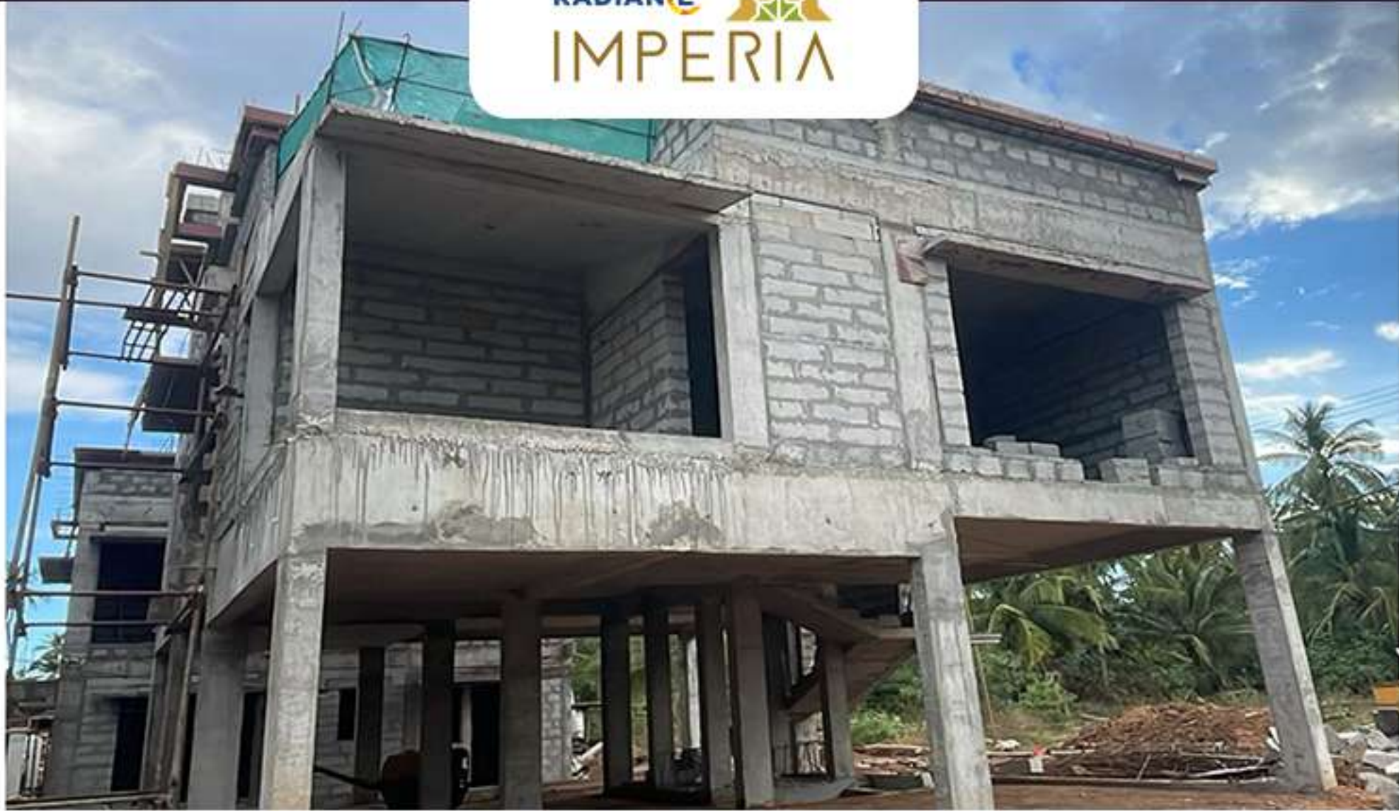
Villa no -70 - Block Work in progress.
