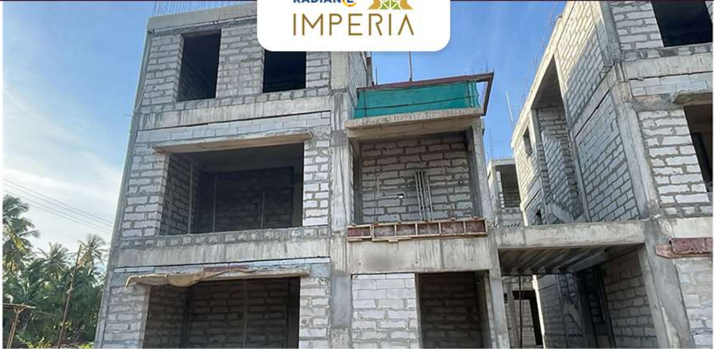
Villa no -45 block Work completed.
