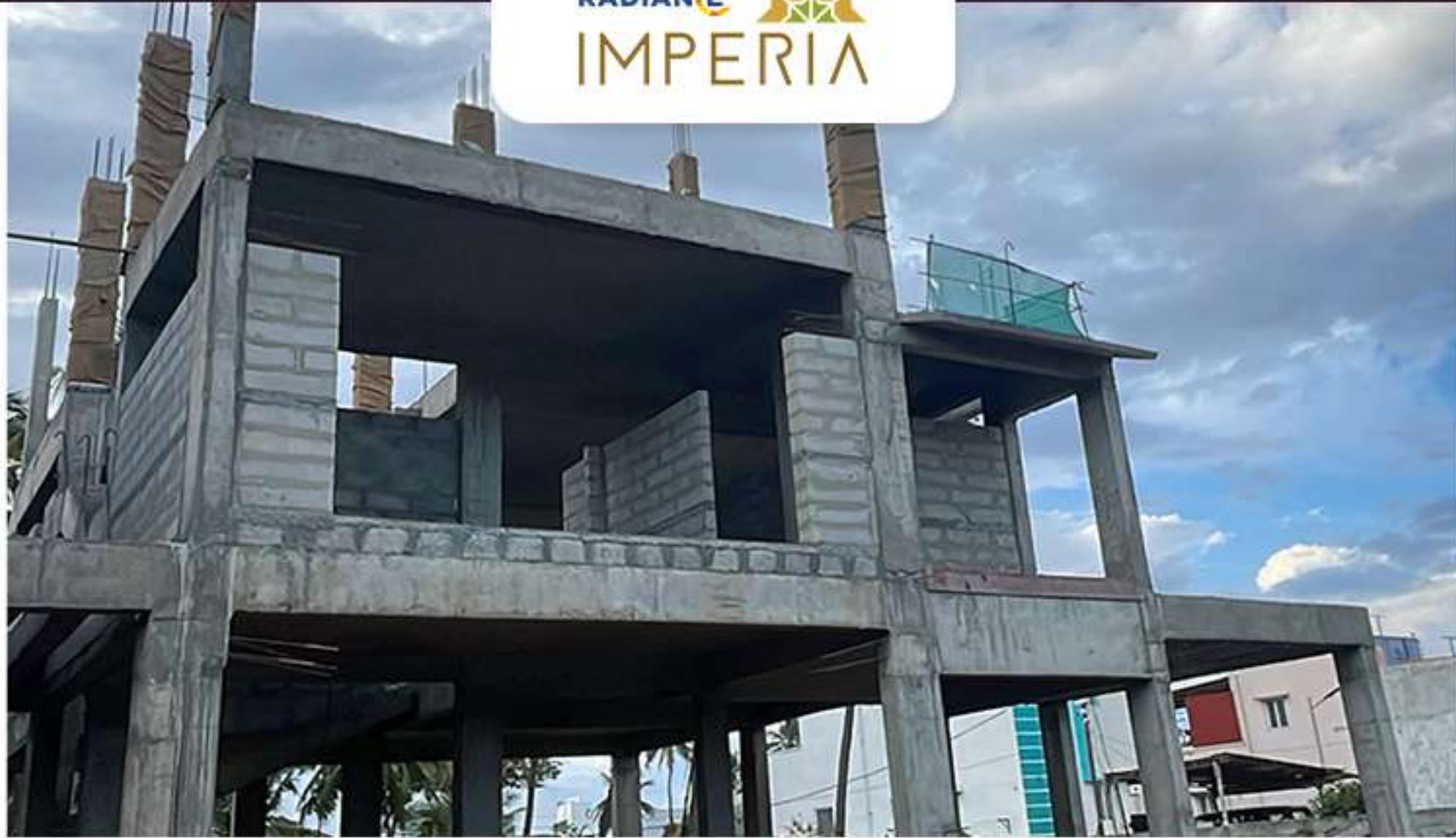
Villa no – 81 Block work in progress
