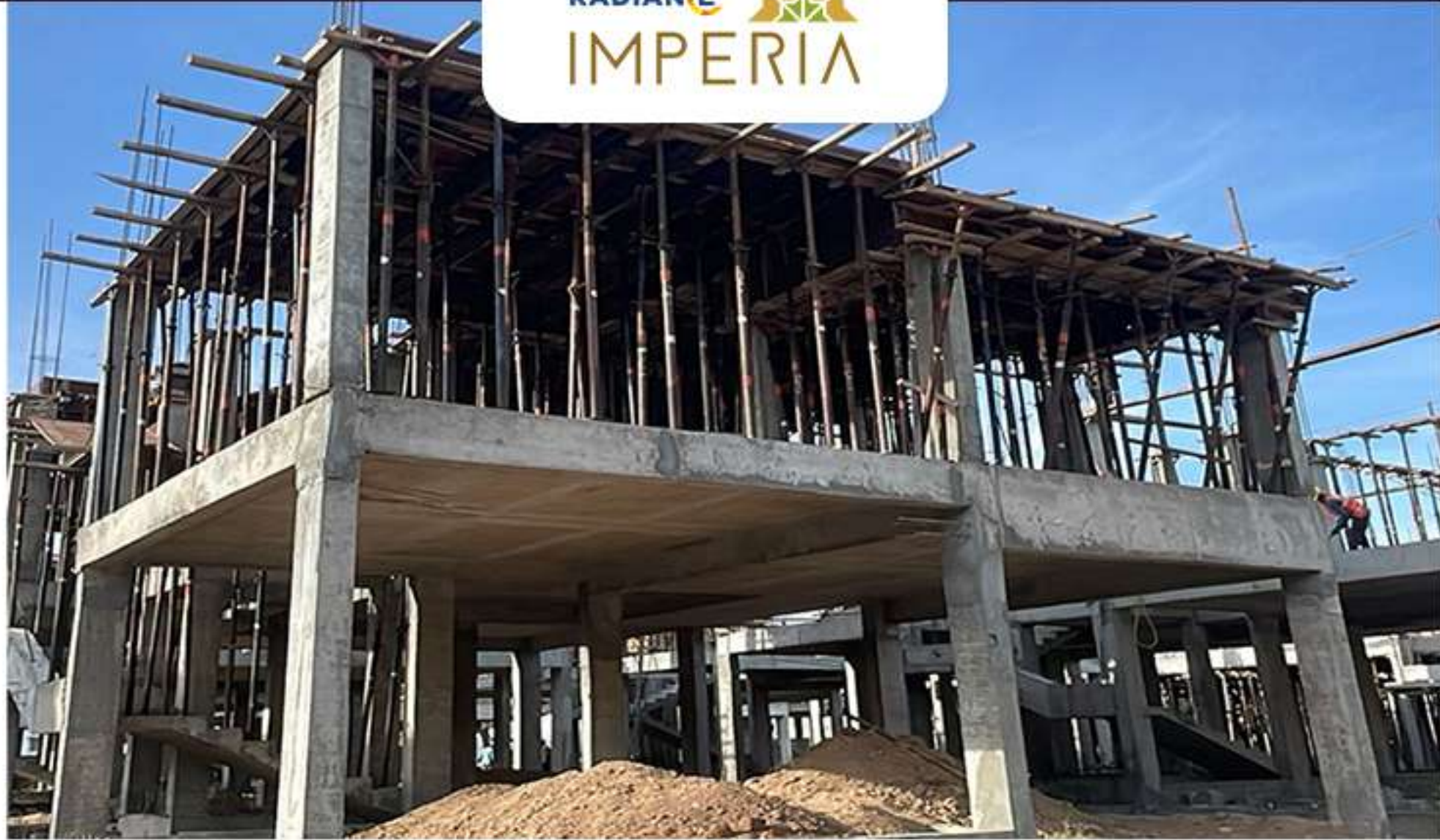
Villa no -24 1st Floor slab shuttering work in progress
