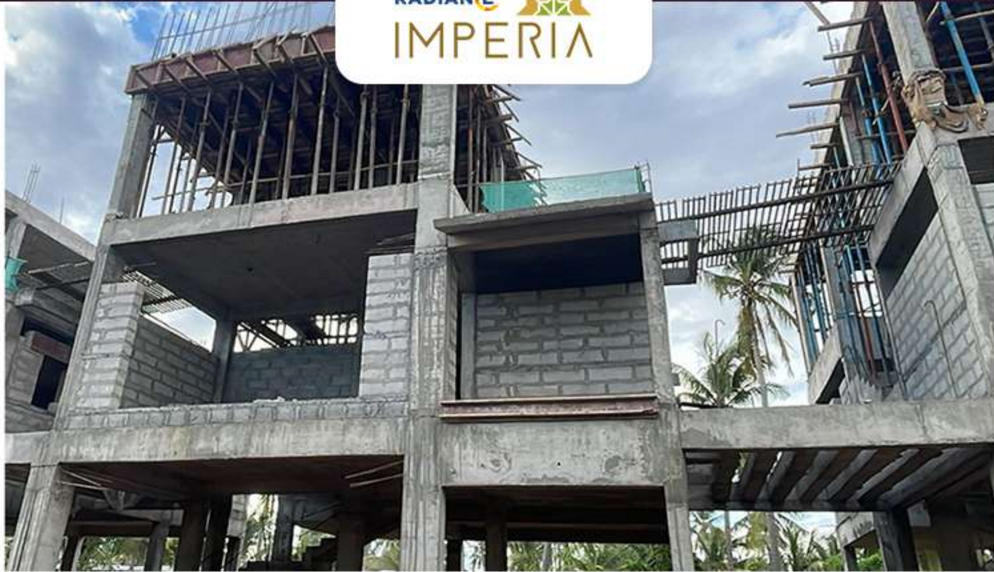
Villa no – 93 – Block work in progress
