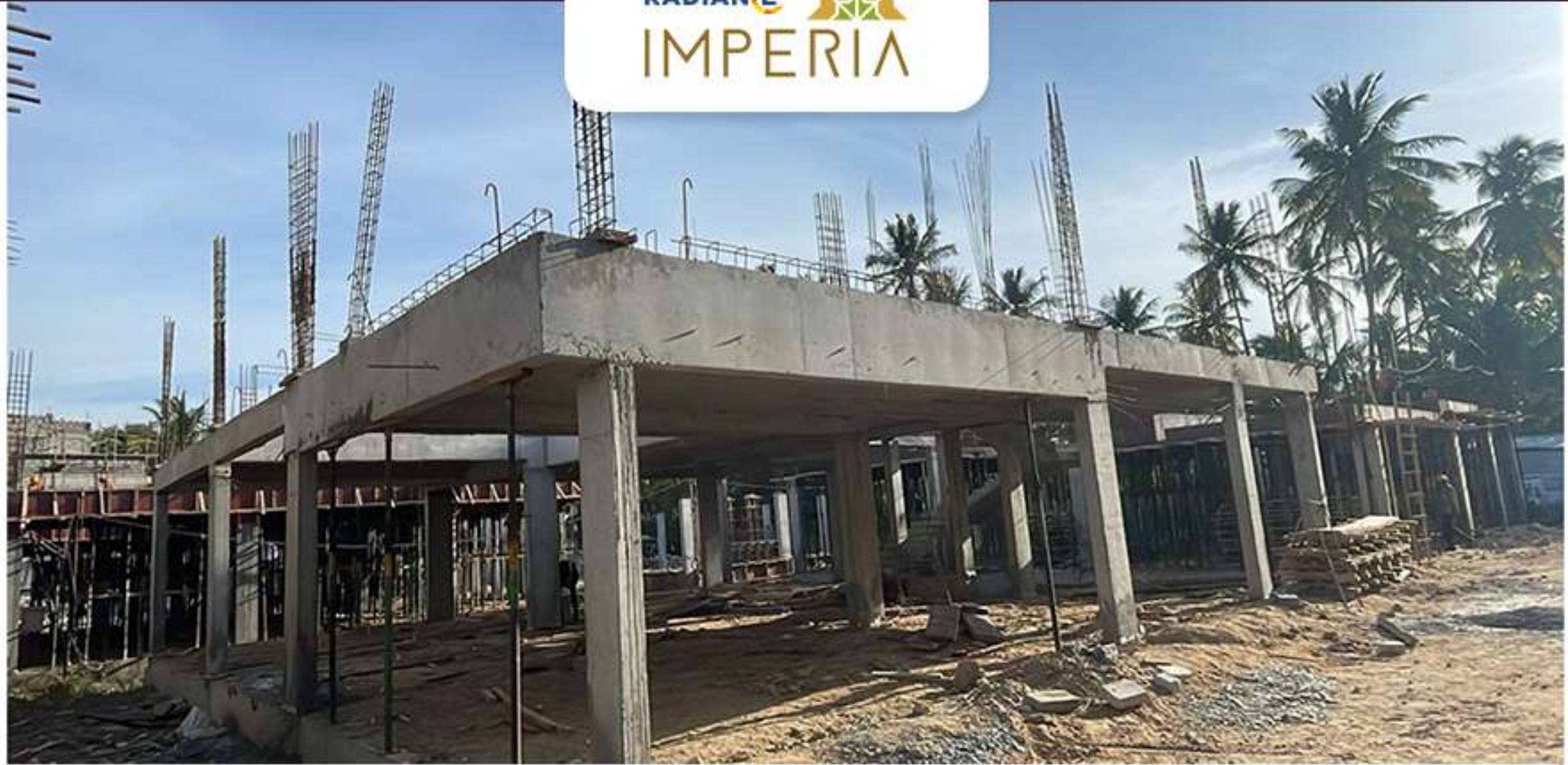
Villa no -42 1st Floor column reinforcement Work in progress.
