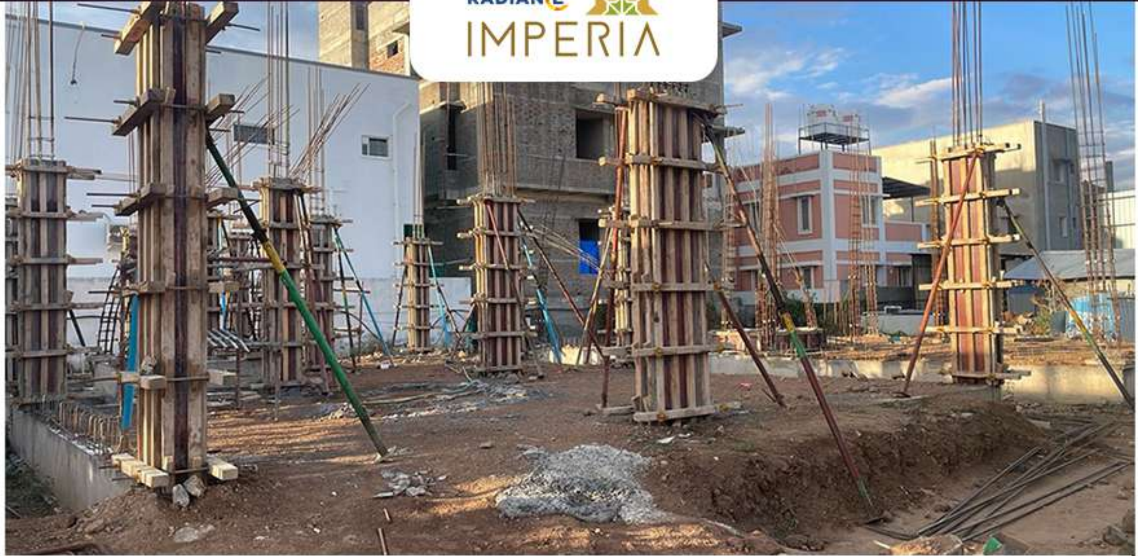
Villa no 63 – GF Column work in progress
