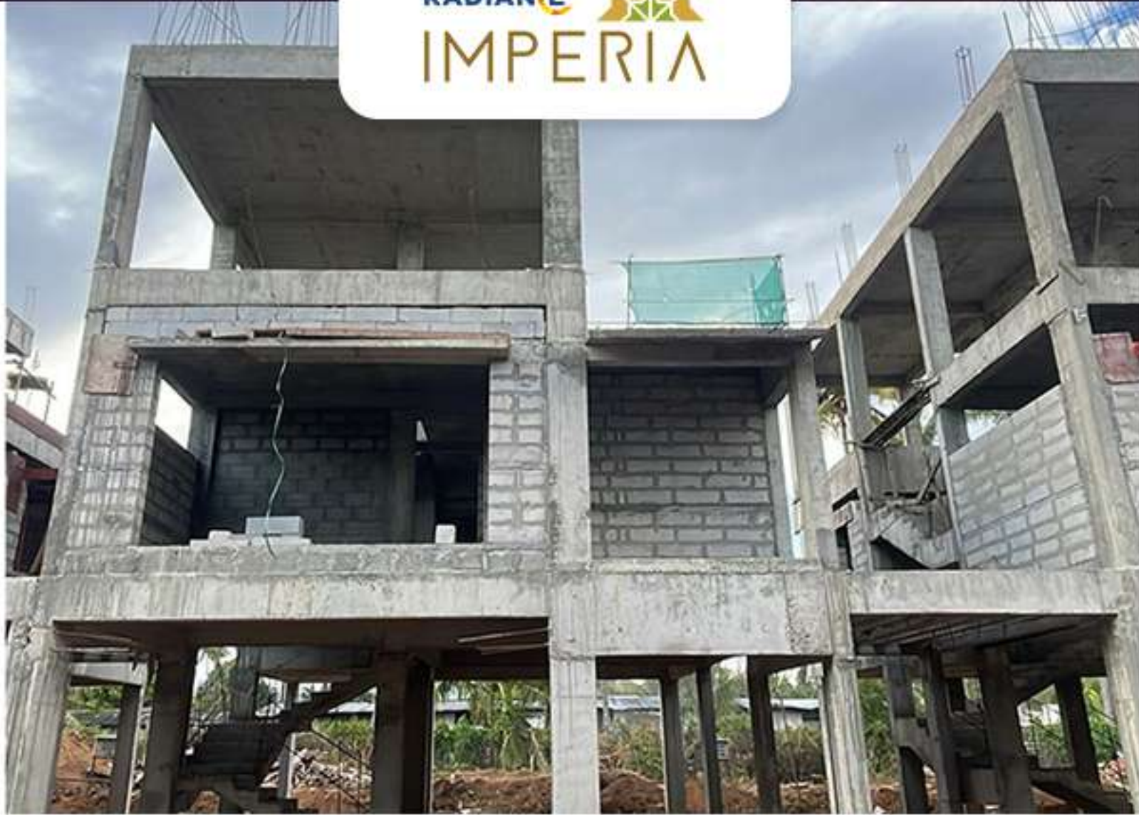
Villa no – 91 – Block work in progress.
