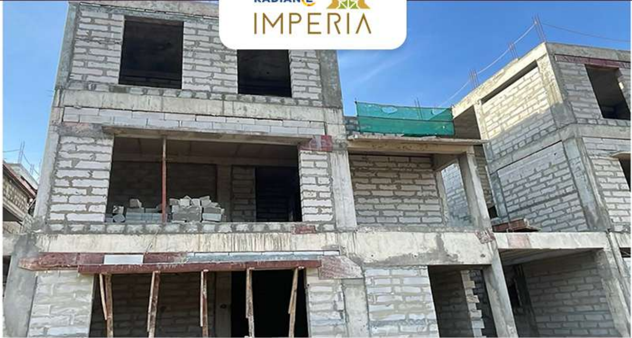
Villa no -46 - Block Work completed
