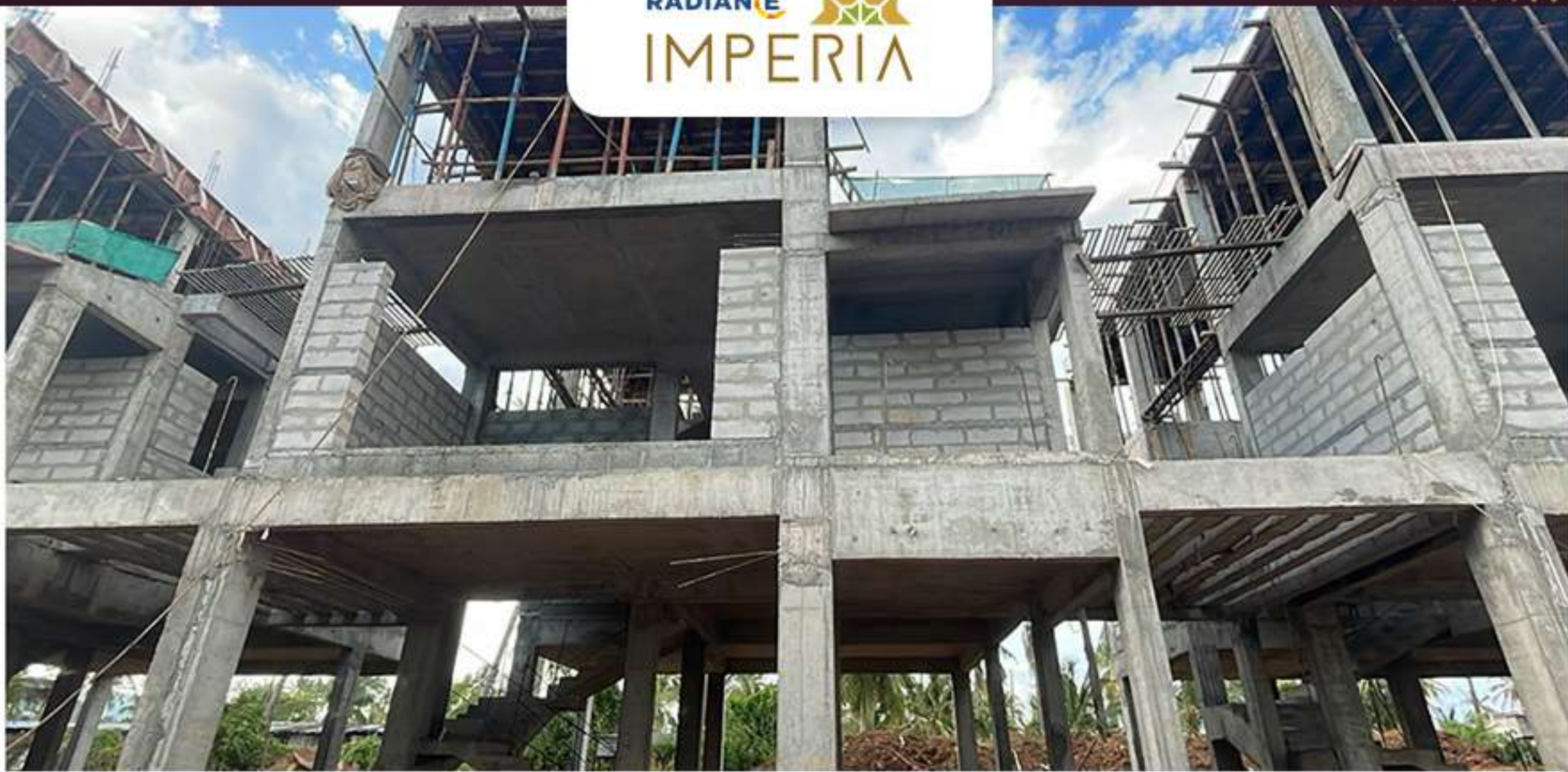
Villa no – 95 Block work in progress
