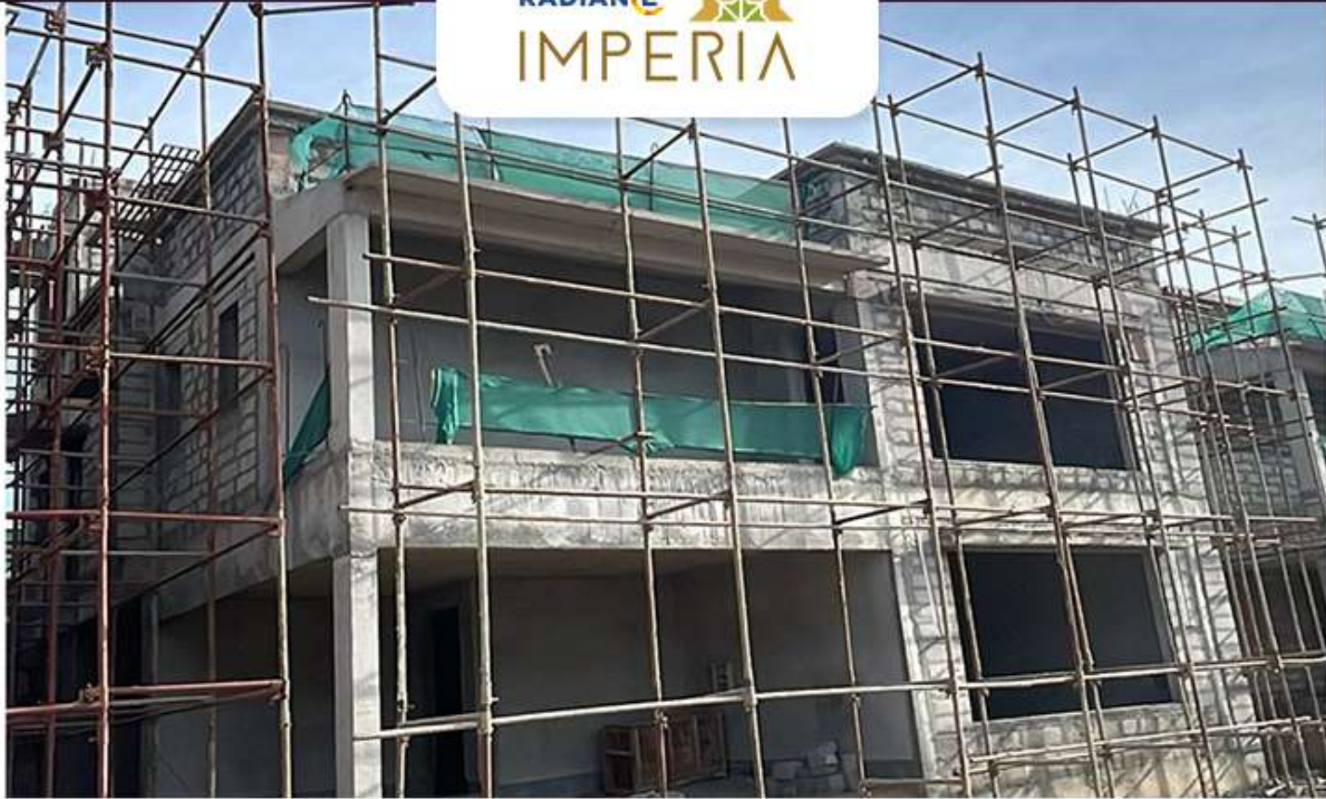
Villa no 9 Plastering Work in progress.
