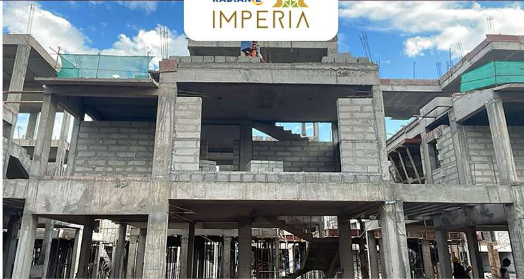
Villa no – 82 – Block Work in Progress.
