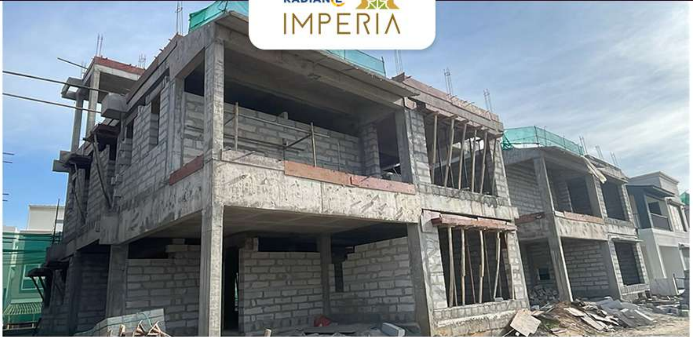
Villa no. 3 - Ground floor Lintel work in progress
