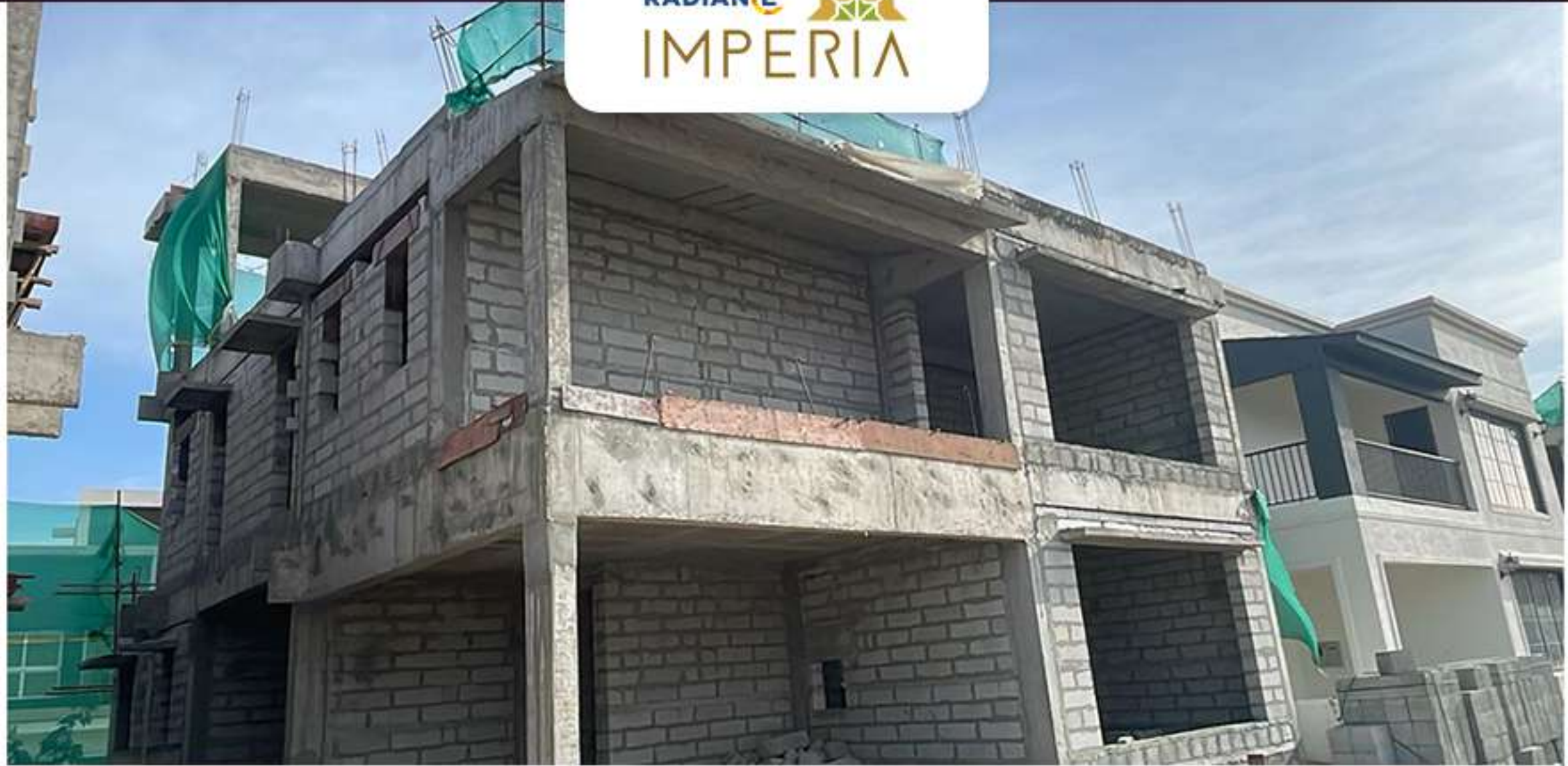
Villa no. 4 – 2nd Floor Block work in progress
