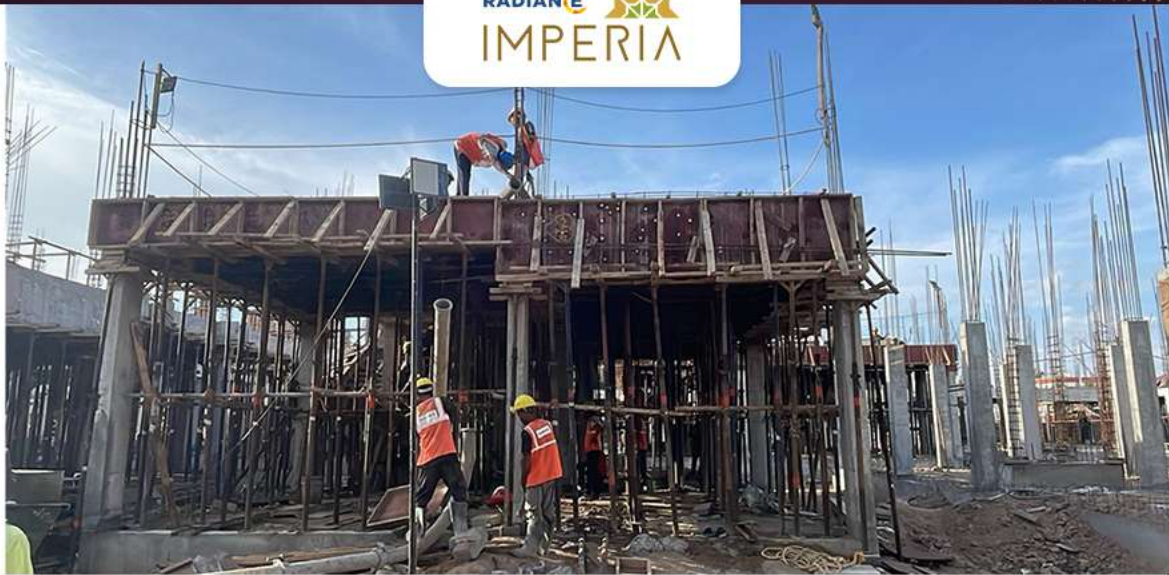
Villa no 28 – GF Roof slab concrete Pouring today
