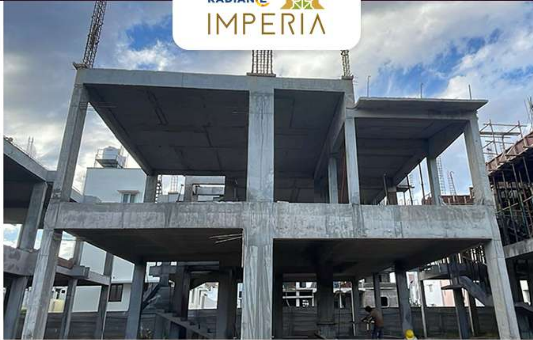
Villa no -55 SF column work in progress.
