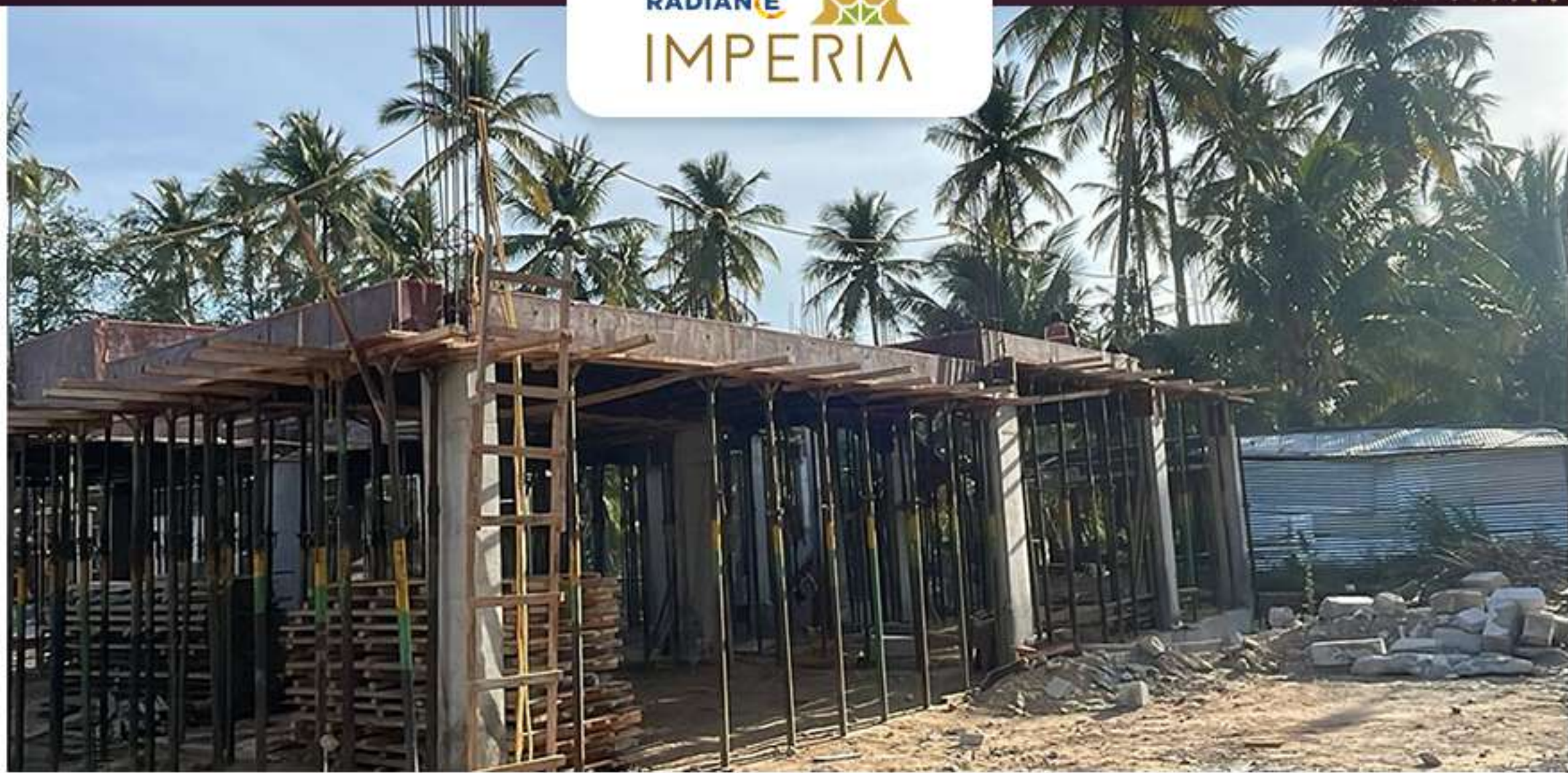
Villa no -43 – GF roof shuttering work in progress.
