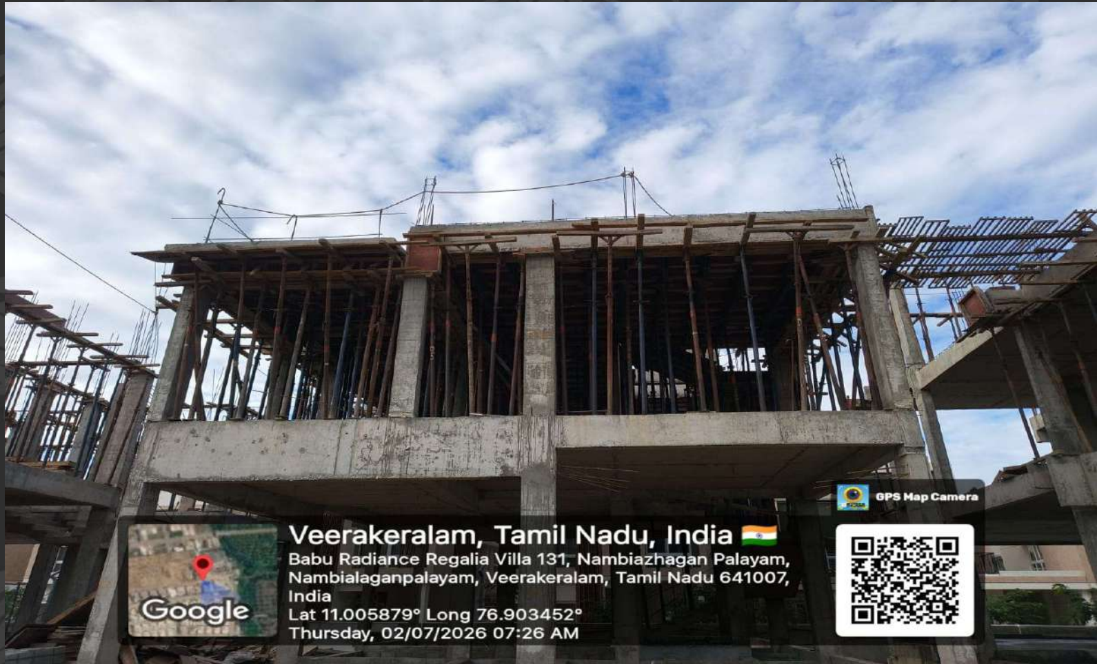
Villa no. 2 First Floor Roof Slab Completed
