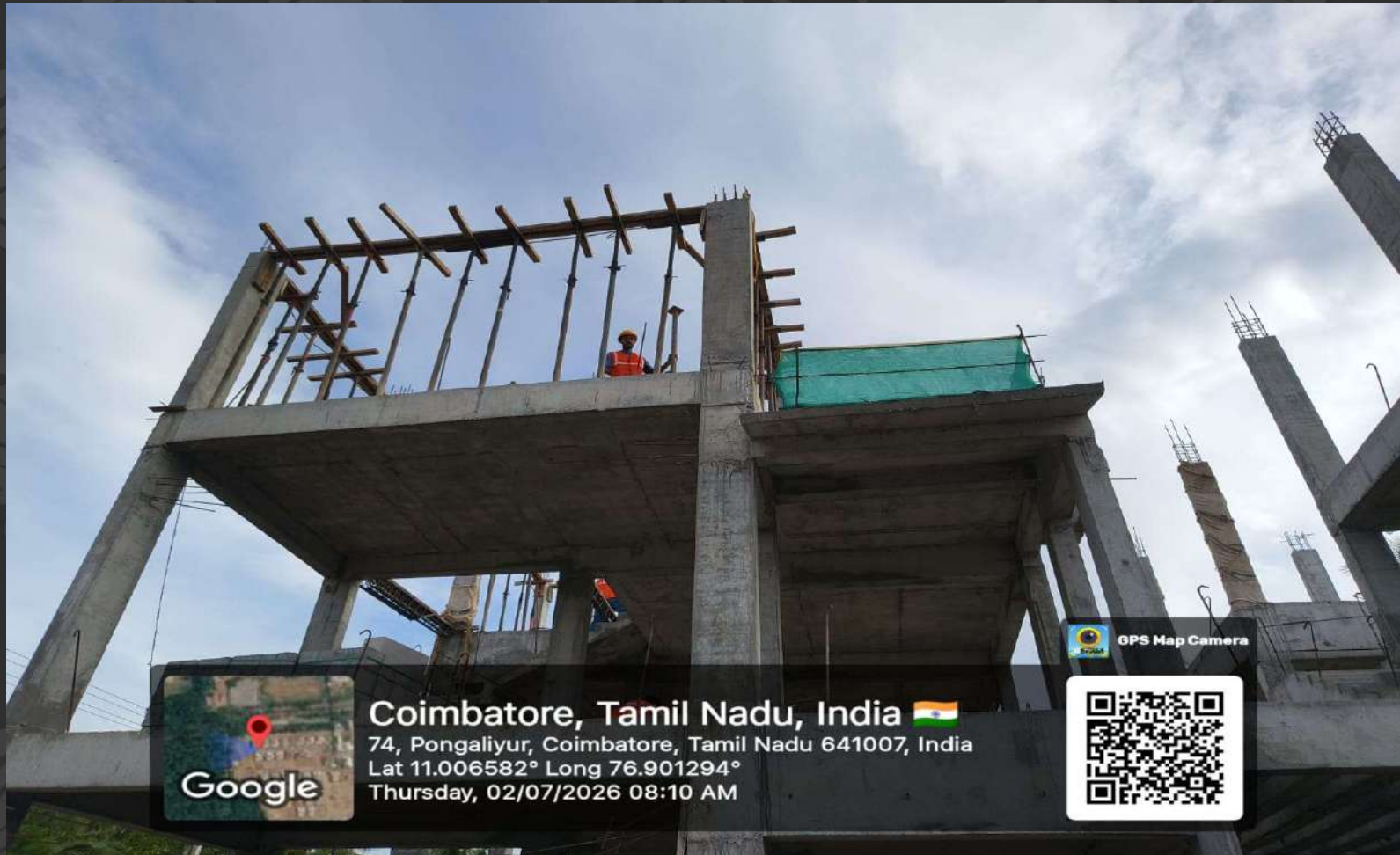
Villas- 88 2 nd Floor Roof Slab Shuttering Work in Progress
