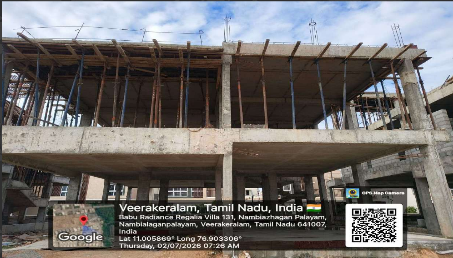
Villa no-3 First Floor Roof Slab Completed
