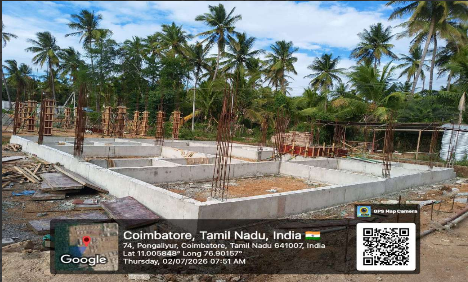
Villa-43 Plinth Beam Concrete Work Completed .
