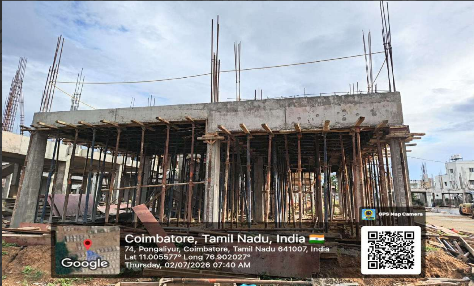
Villa 23 Ground Floor Roof Slab Completed.
