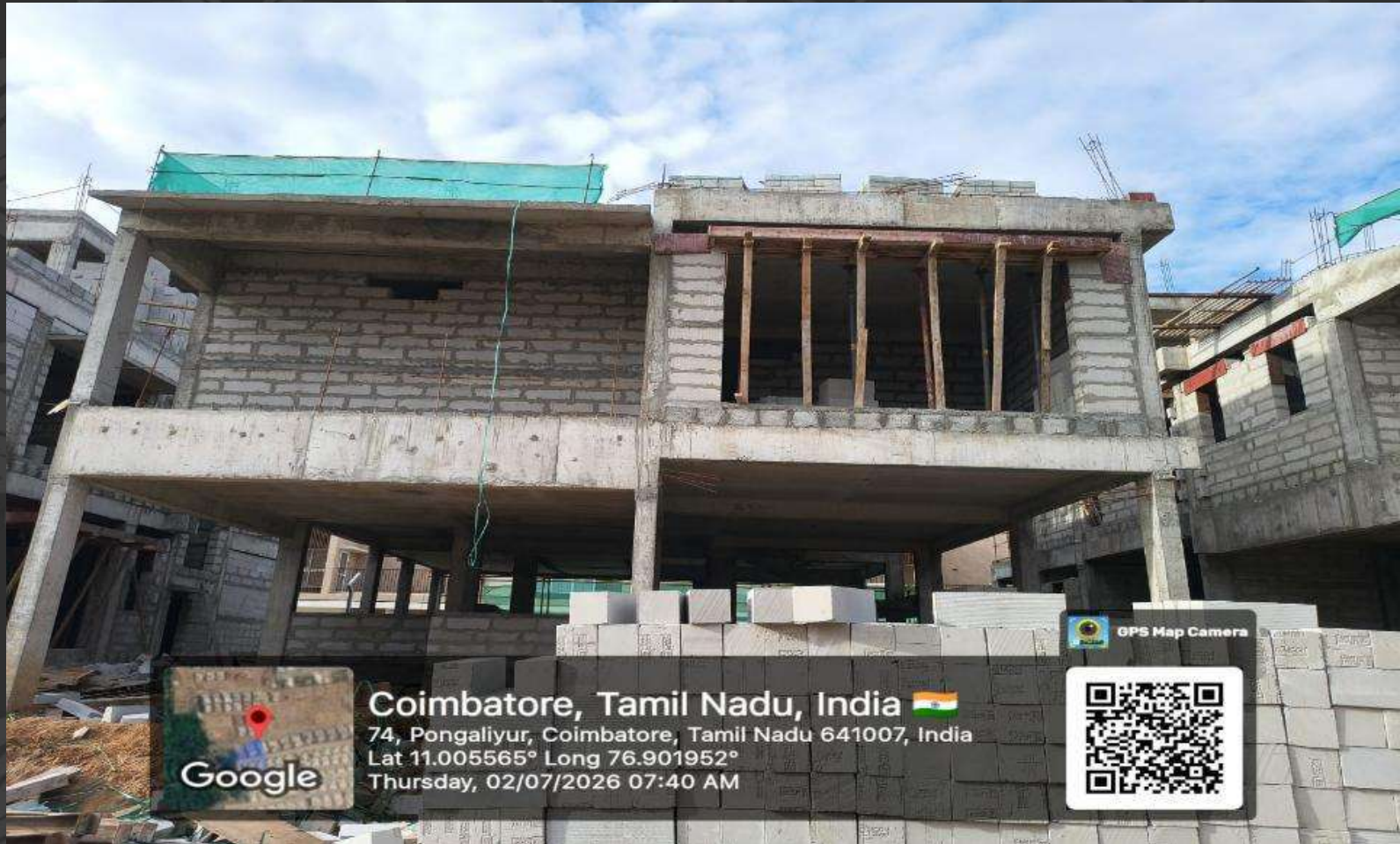
Villa 15 Block Work in Progress.
