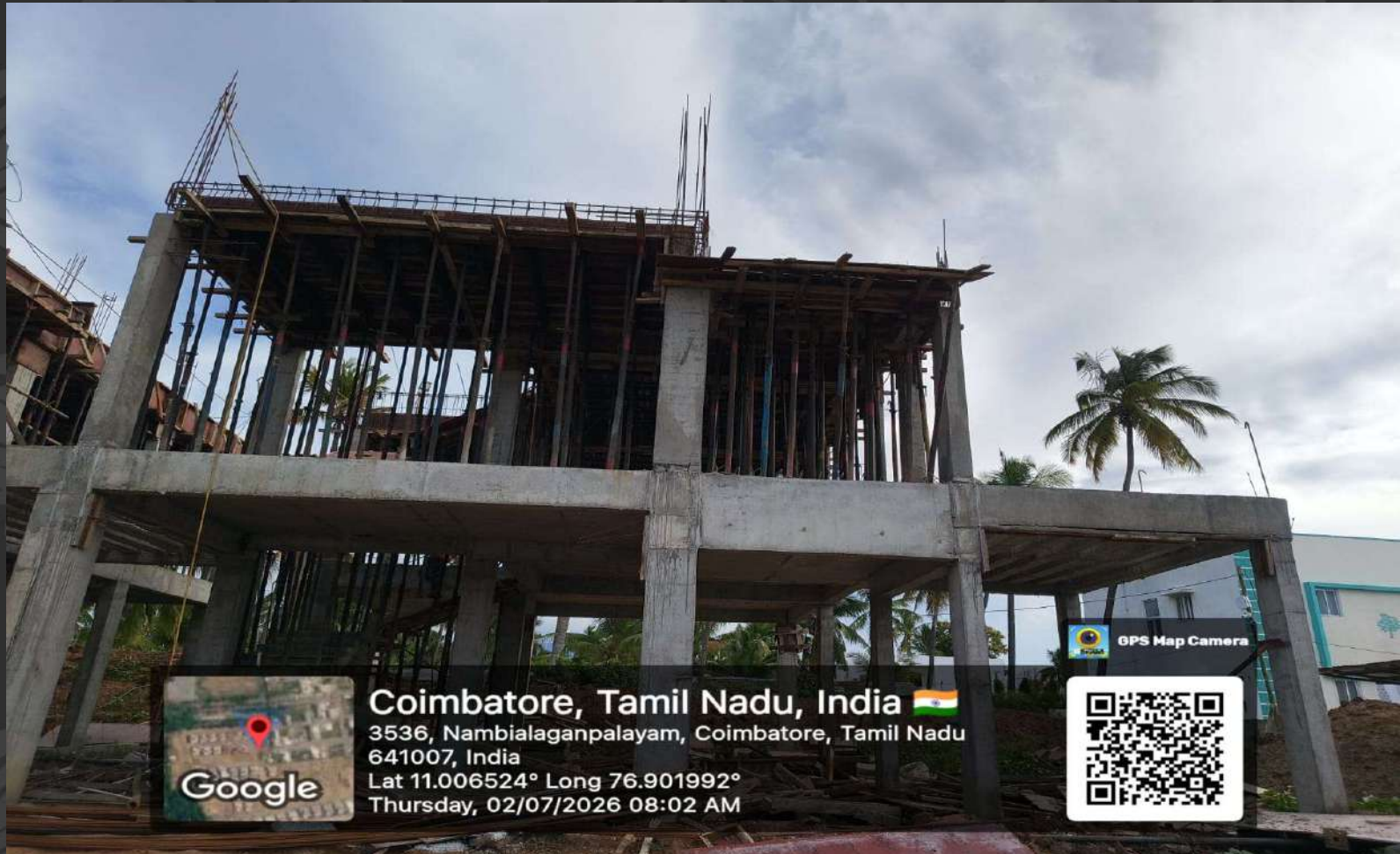
Villas-97 First Floor Roof Slab Shuttering Work in Progress..
