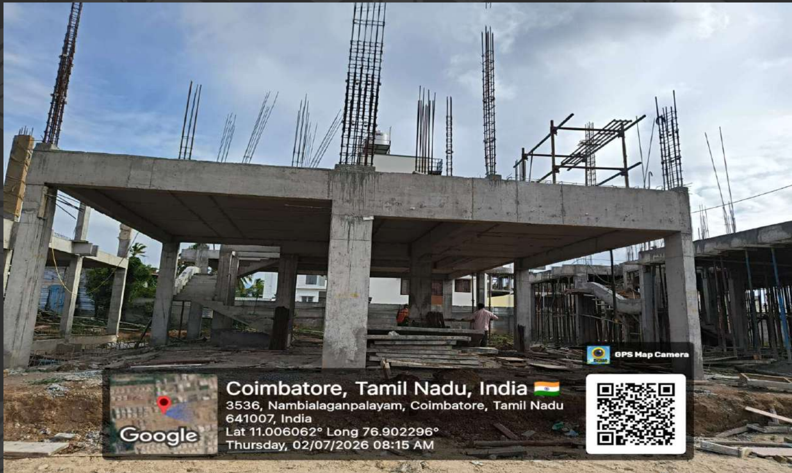
Villas- 54 First Floor Column Work in Progress
