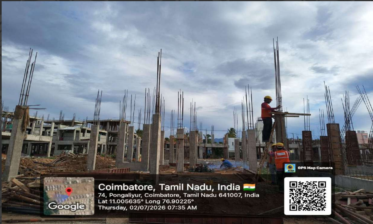
Villa 24 Ground Floor Roof Slab Work in Progress.
