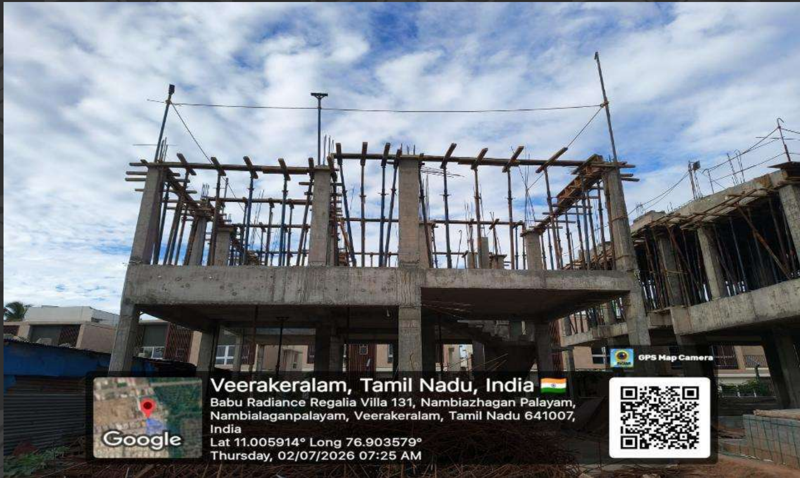
Villa no. 1 Floor roof Slab Shuttering Work in Progress
