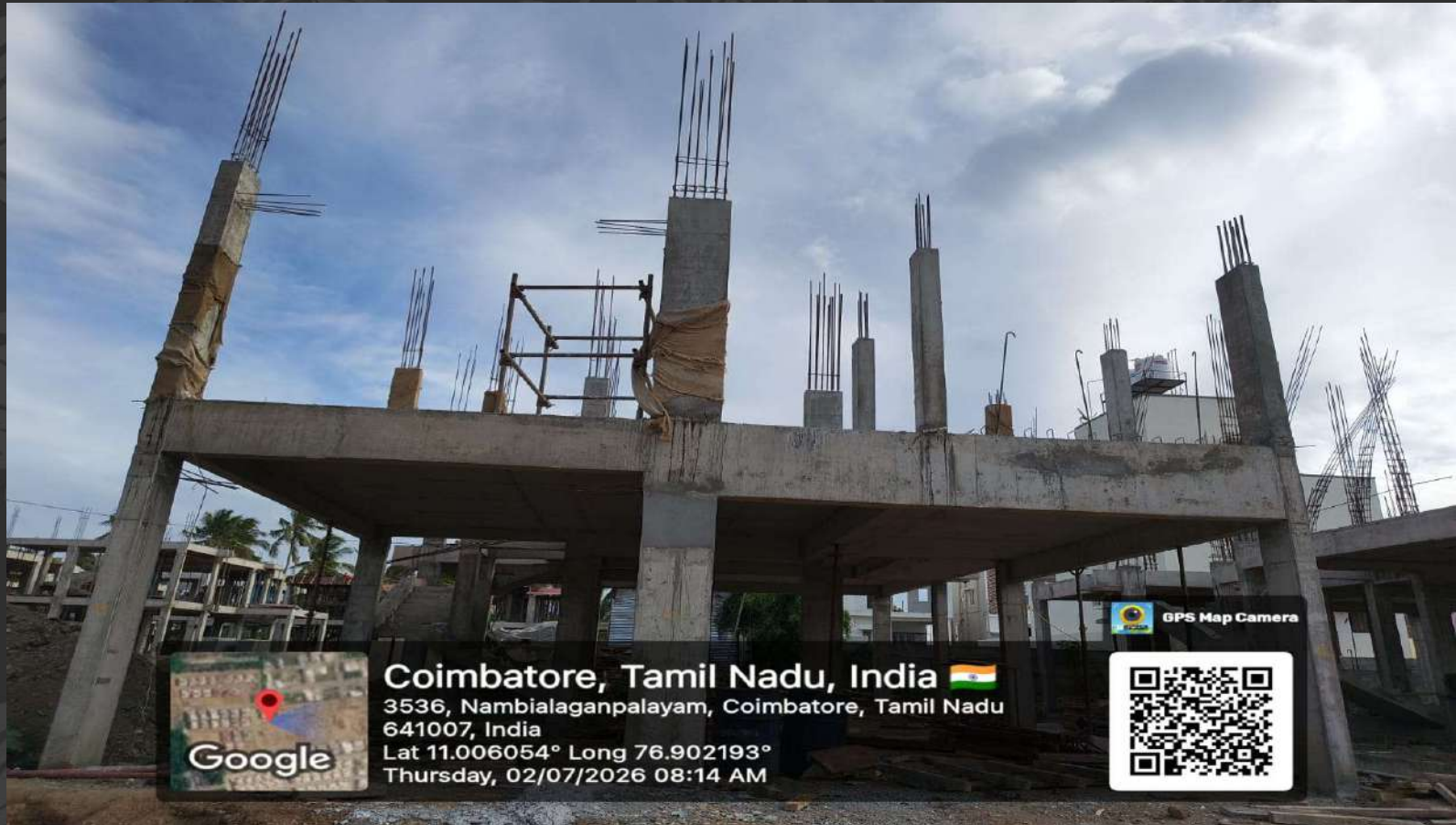
Villas- 52 First Floor Column Completed
