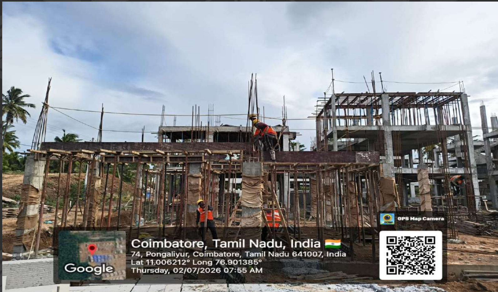
Villa- 73 Ground Floor Roof Slab Shuttering in Progress.
