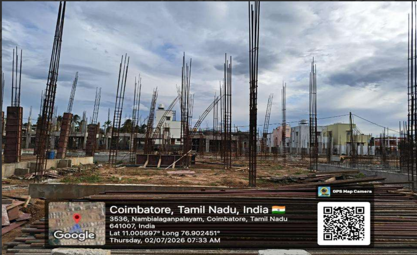
Villa 27 Plinth Beam Completed.
