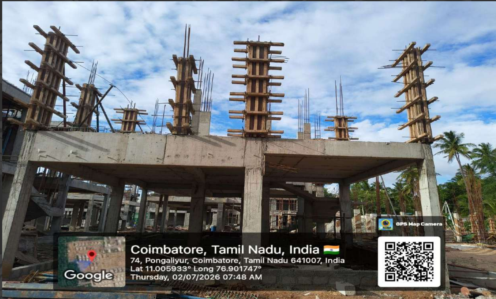
Villa-41 First Floor Column Work in Progress .
