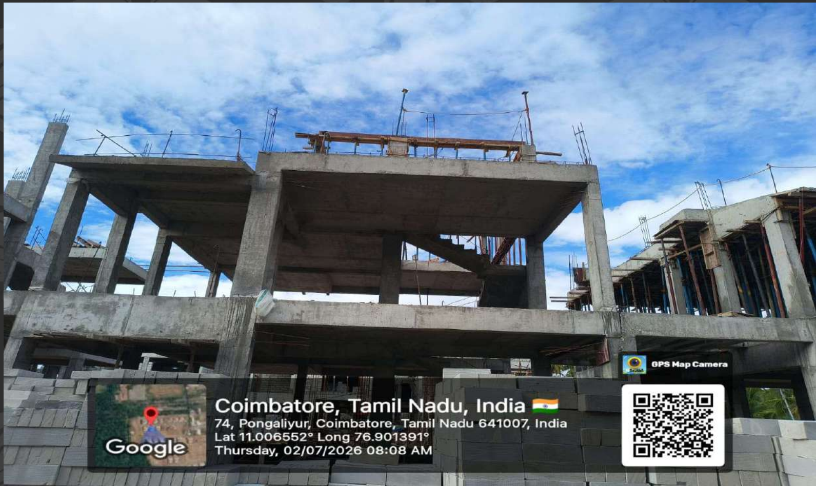
Villas- 86 2 nd Floor roof Slab Work in Progress
