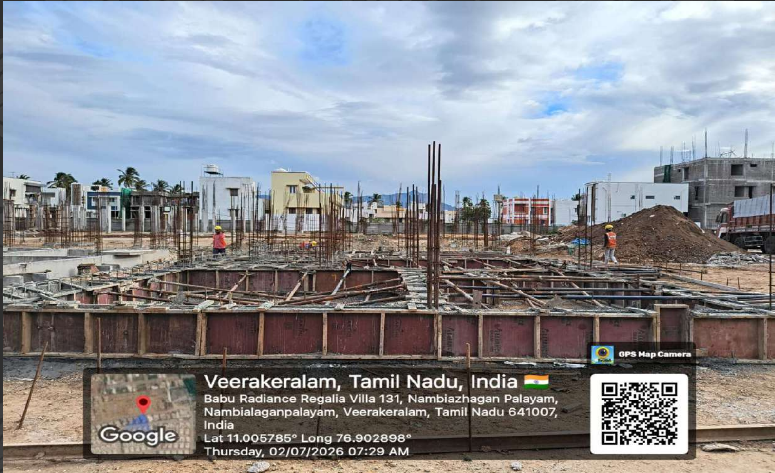
Villa 31 Plinth Beam Concrete Work Completed .
