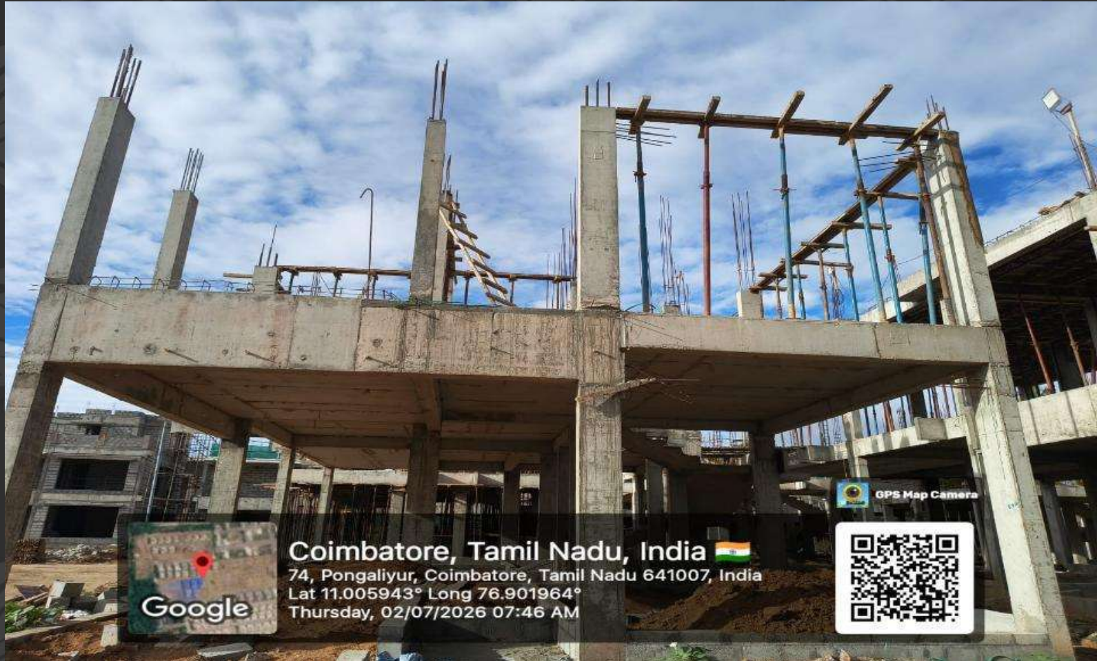
Villa 39 First Floor Roof Slab Work in Progress.
