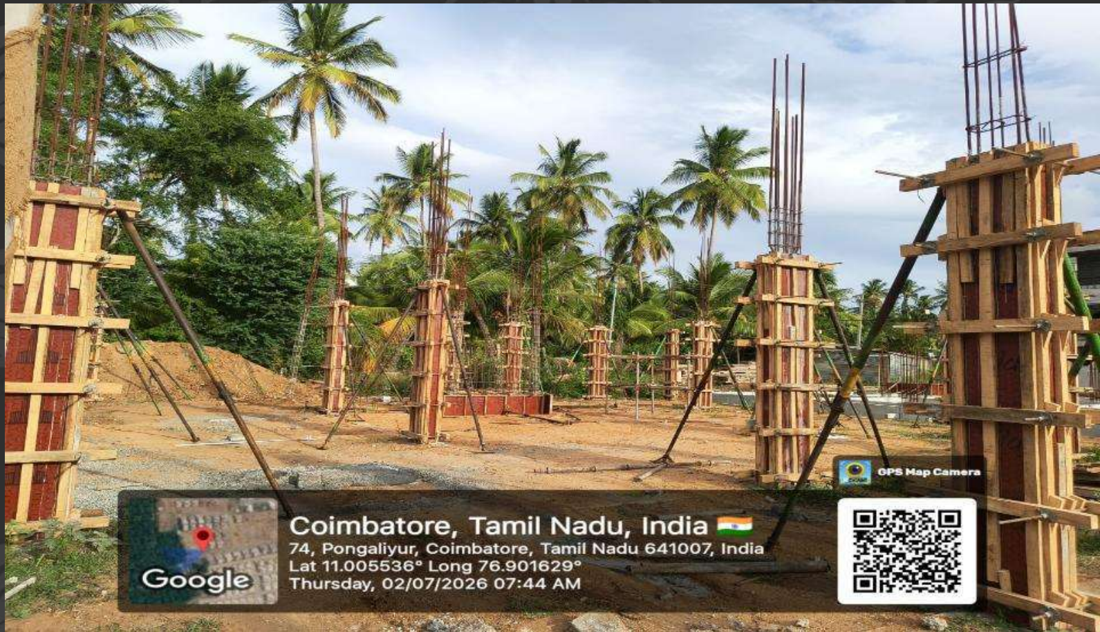
Villa 19 Ground Floor Column Completed.
