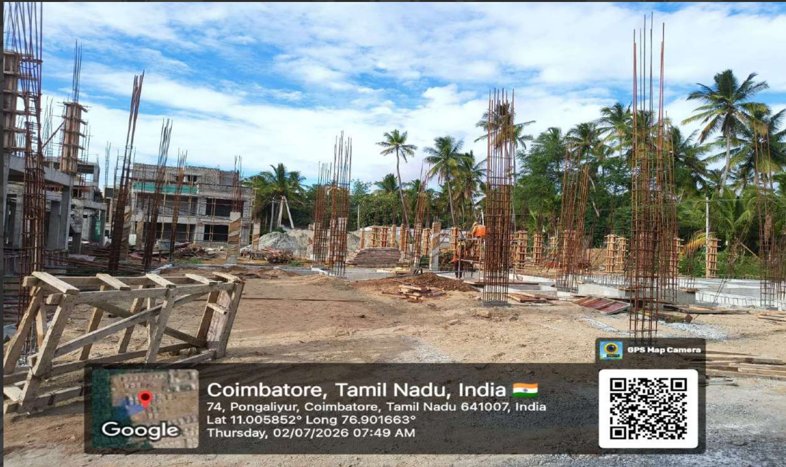
Villa-42 Ground Floor Column Reinforcement Work in Progress .
