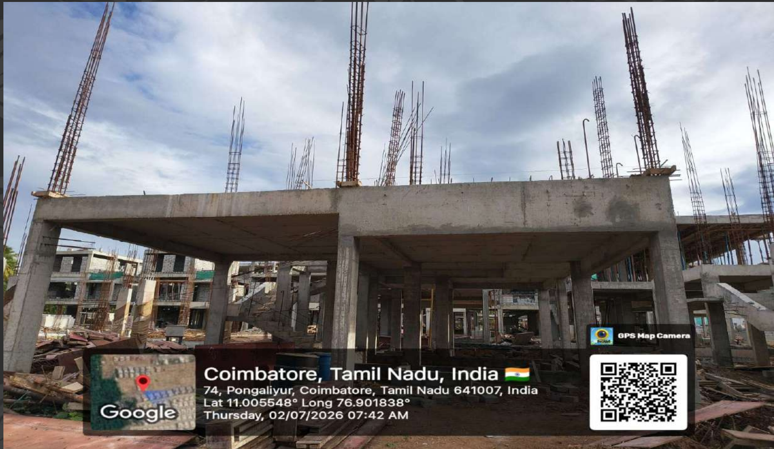
Villa 21 First Floor Column Work in progress.
