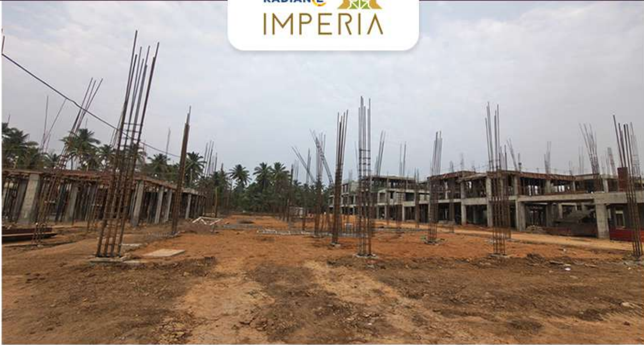
Villa no. 39 Ground Floor Column Progress
