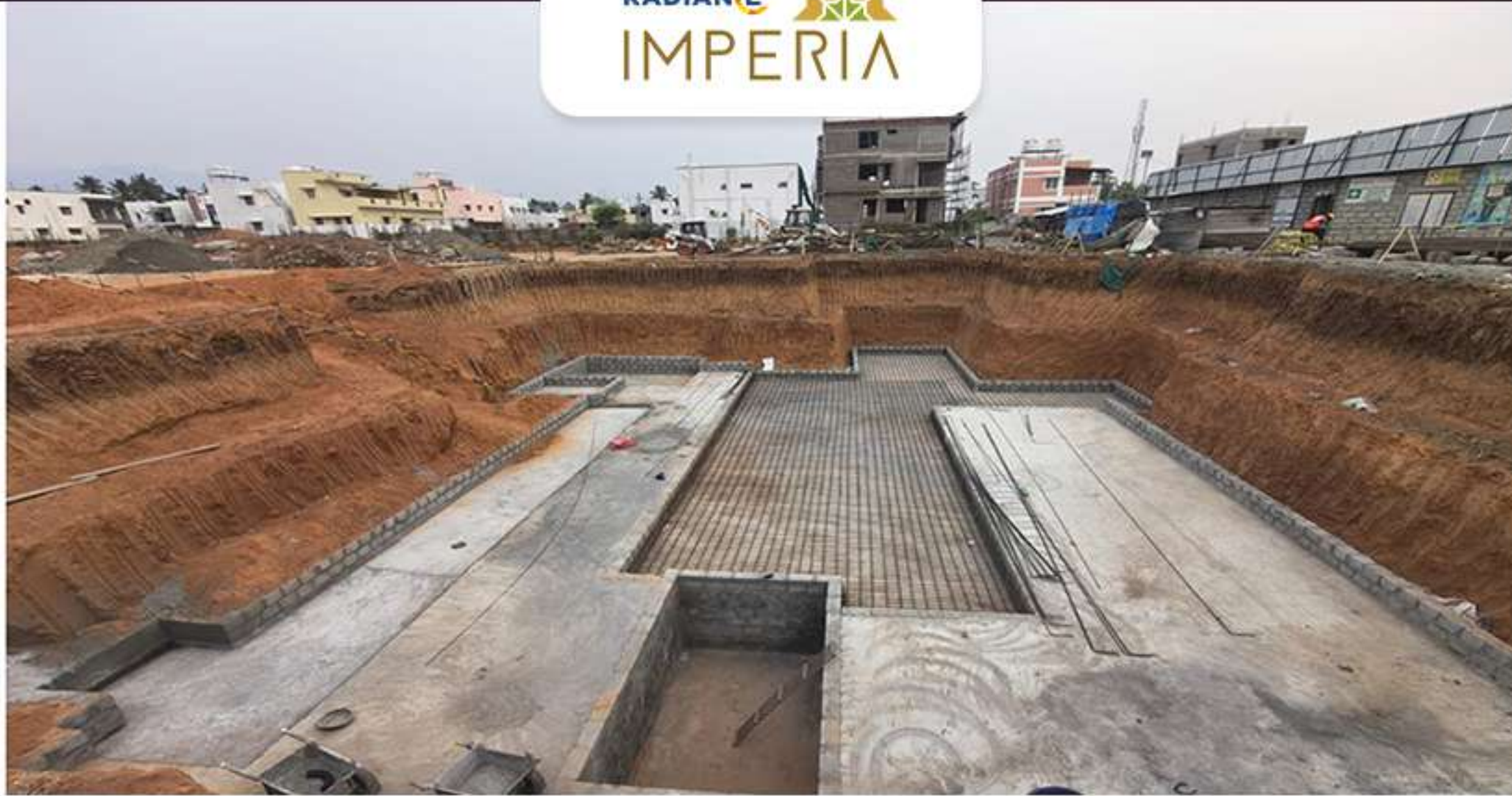
STP & WTP Reinforcement Work in Progress
