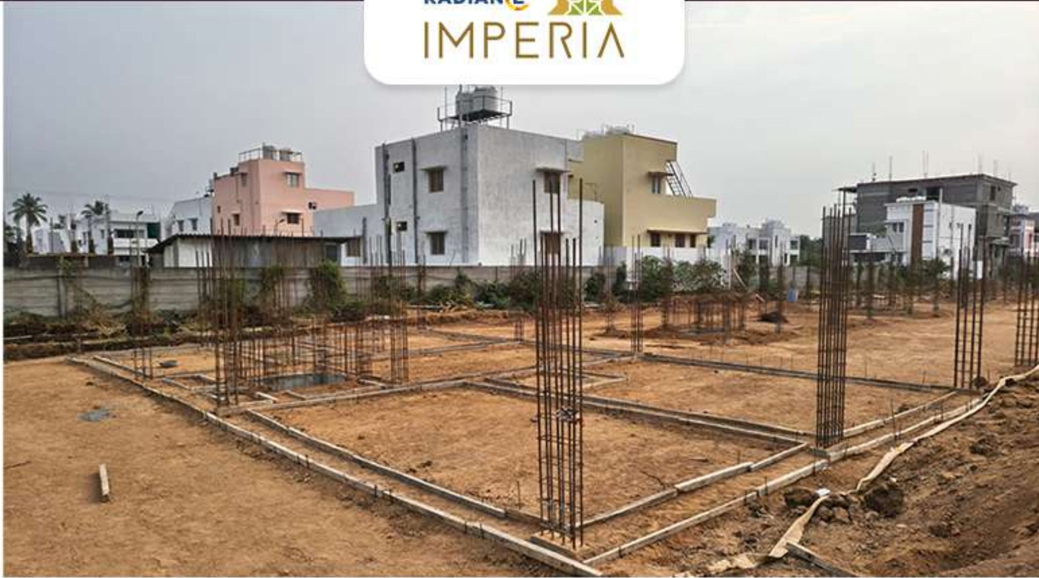
Villa 56 plinth Beam Shuttering Work in Progress
