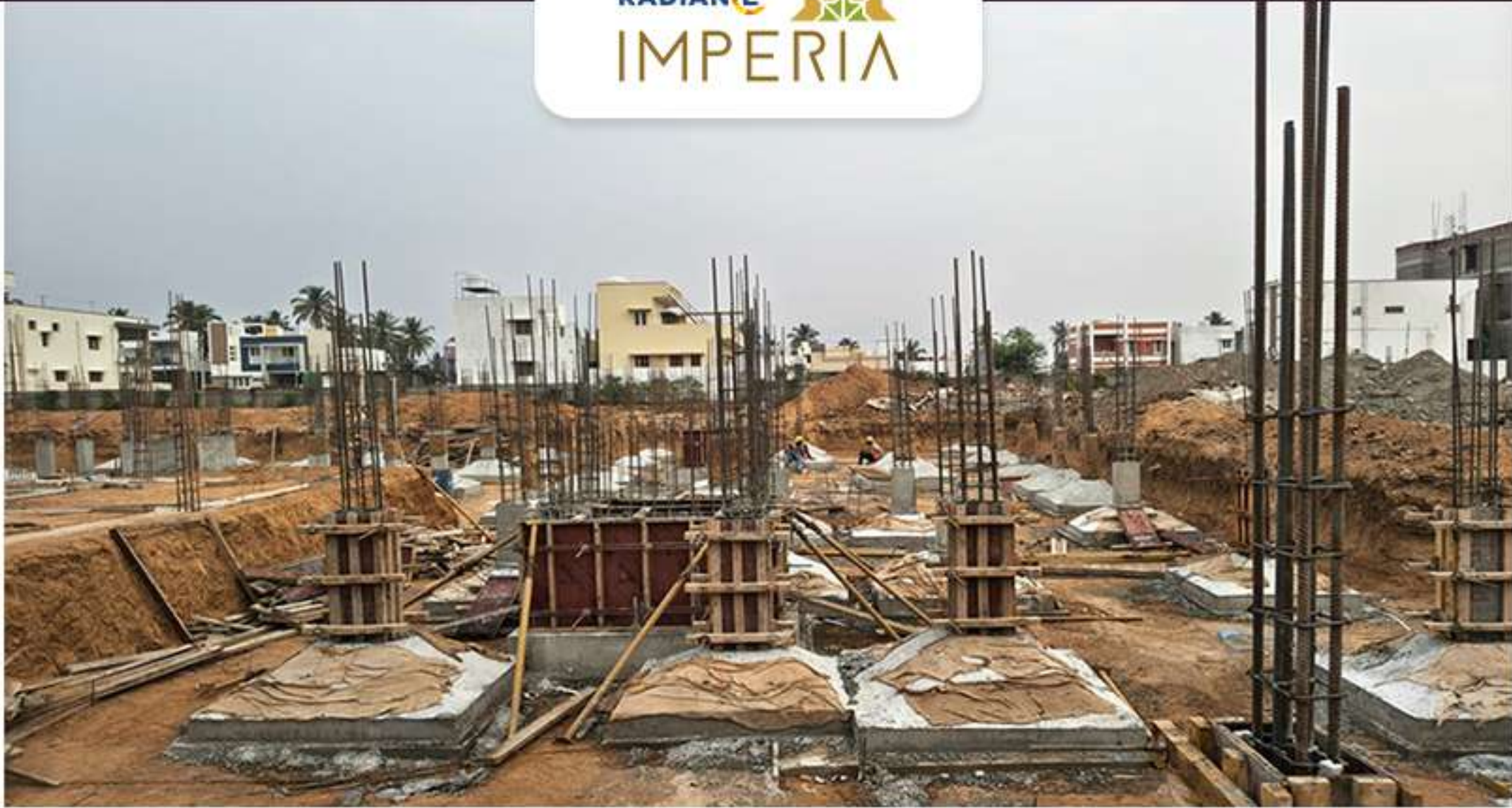
Villa no 31 pedestal column De-shuttering Work In progress
