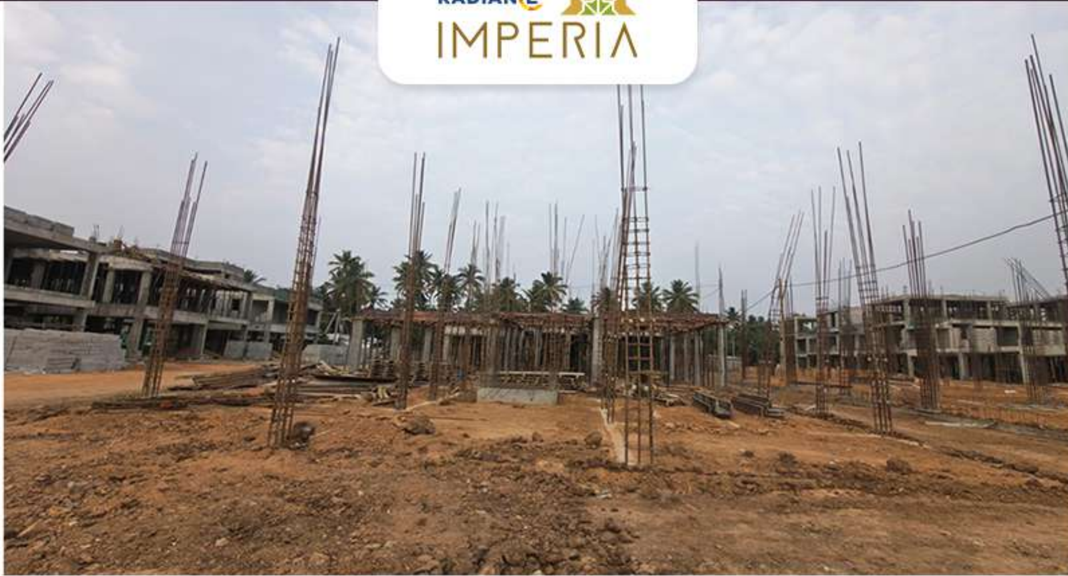
Villa no. 23 Plinth Beam level Soil Filling Work in Progress
