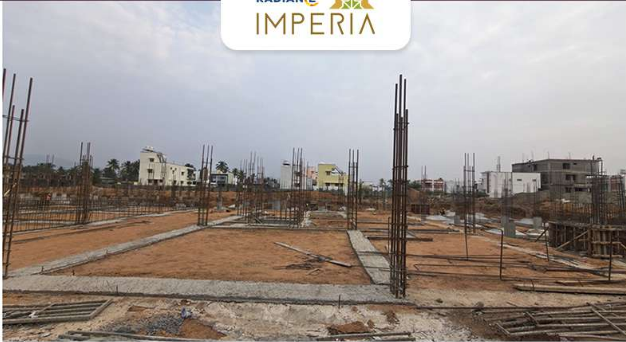
Villa no 30-Plinth Beam Work in Progress
