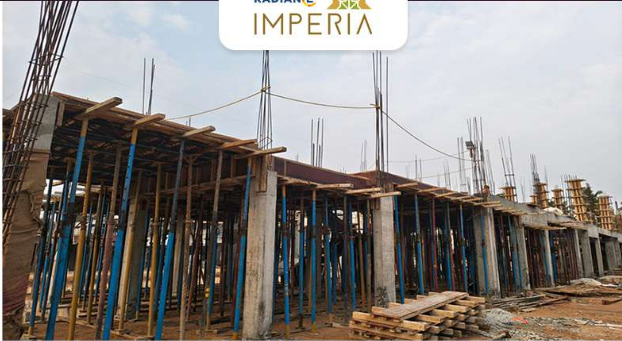
Villa 82 Ground Floor Roof Slab Shuttering Work in Progress
