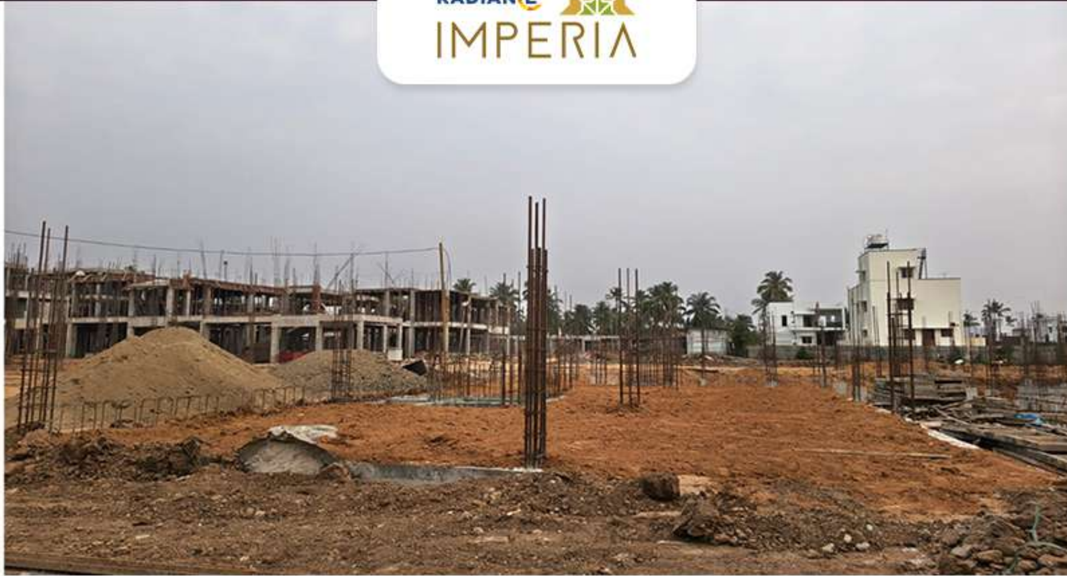
Villa no. 25 Plinth Beam Level Soil Filling Work in Progress
