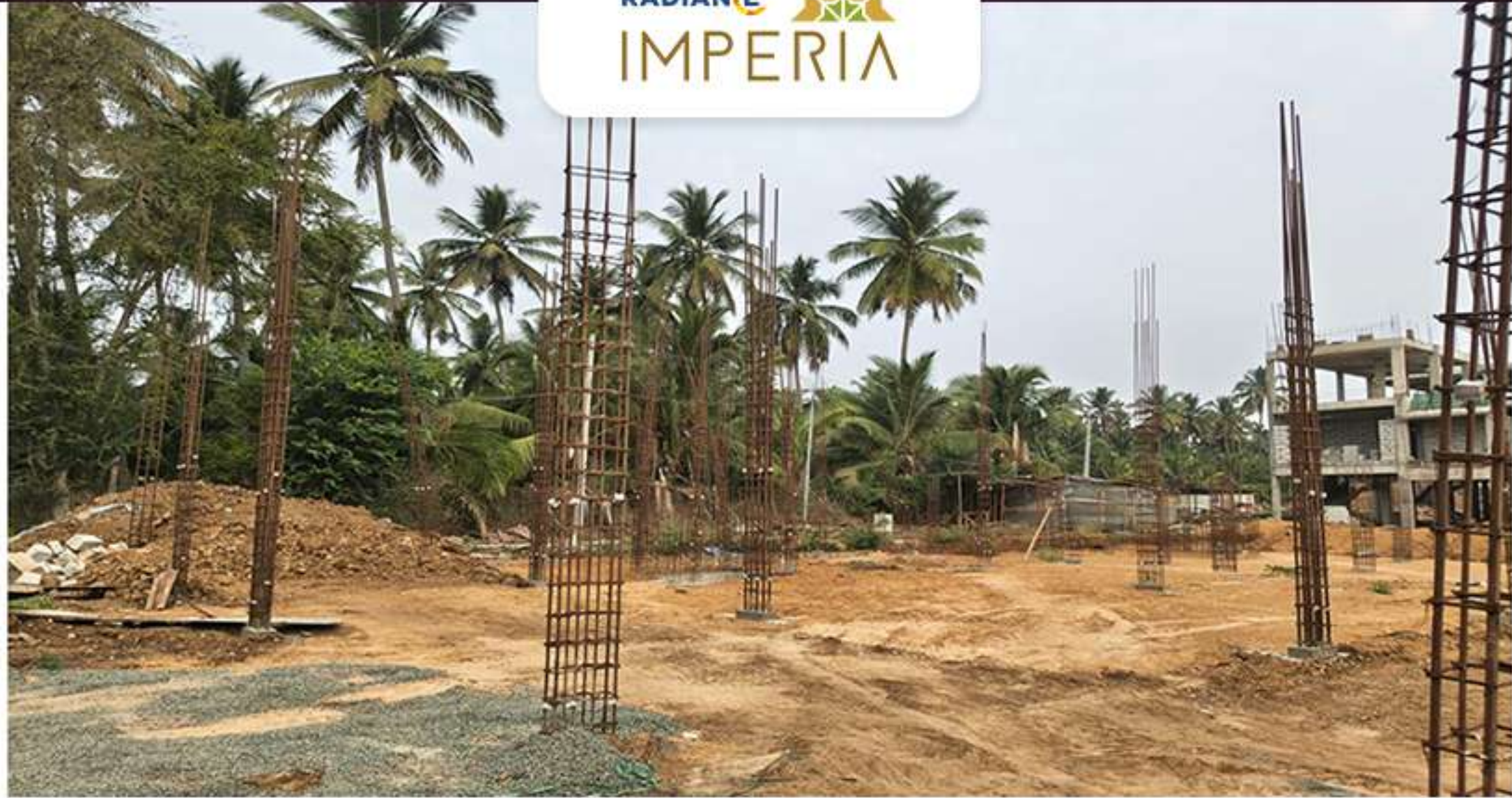
Villa no. 19 Ground Floor Column Work in Progress
