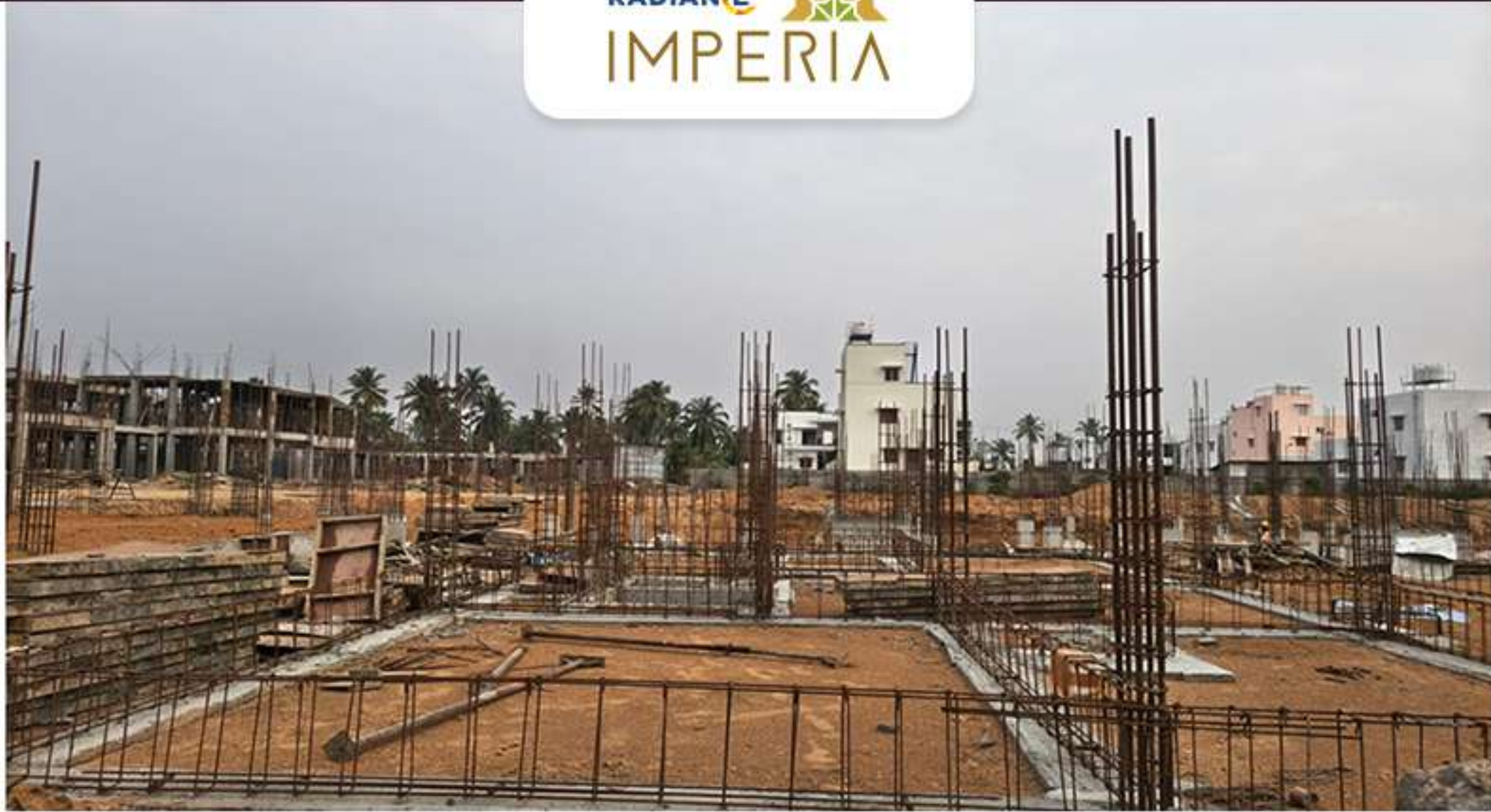
Villa no. 25 Plinth Beam Work in Progress
