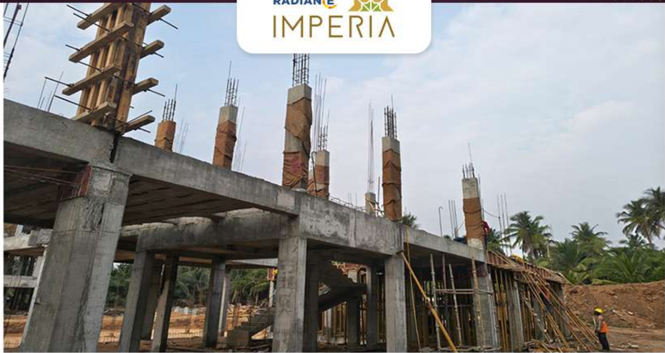
Villa 86 First Floor Column completed
