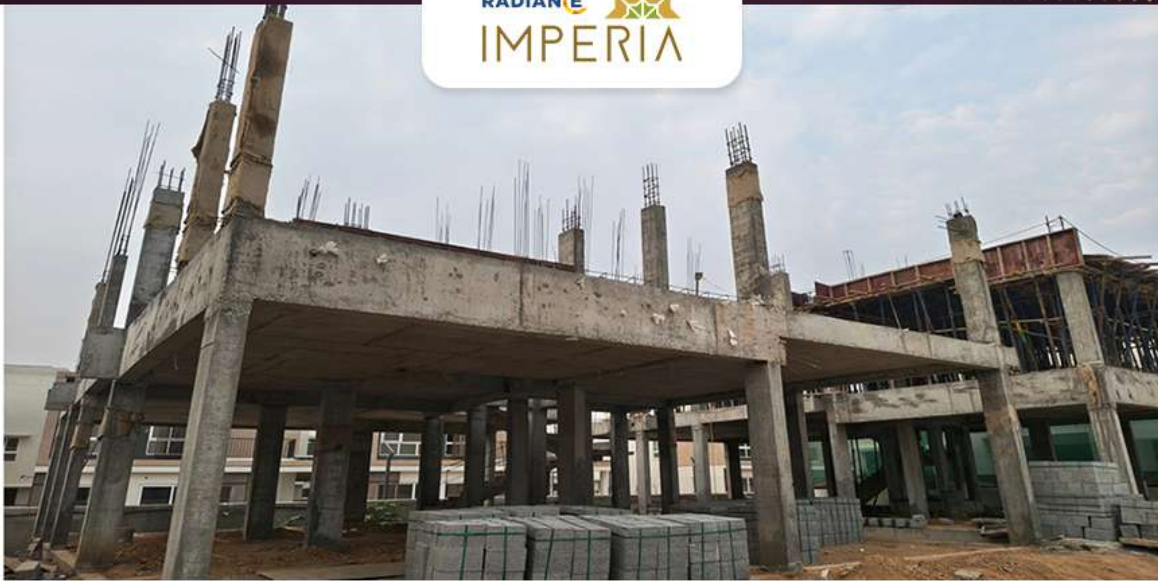
Villa no. 3 1st Floor Roof Slab Shuttering Work in Progress
