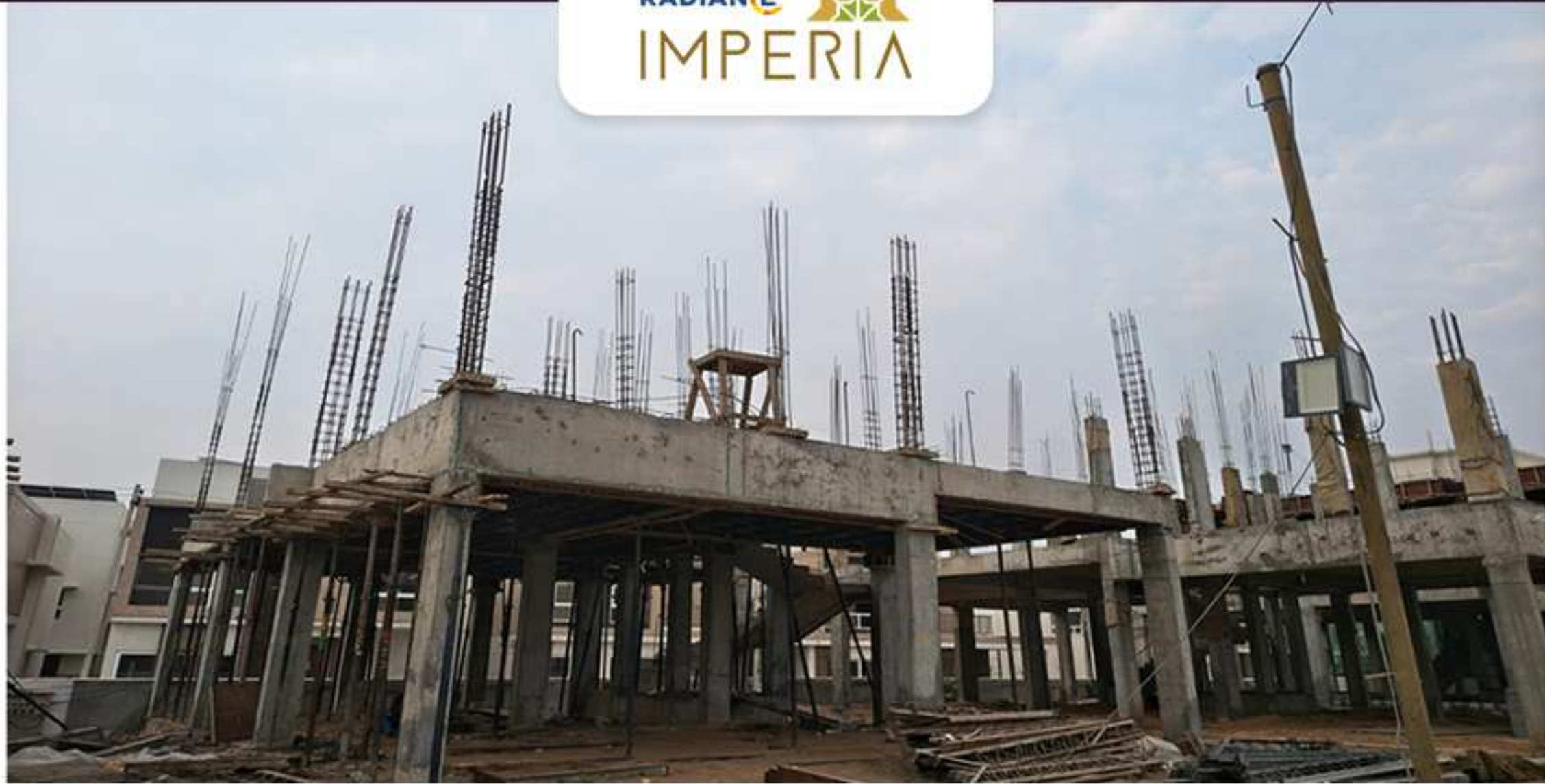
Villa no. 2 1st Floor Column Marking Work in Progress
