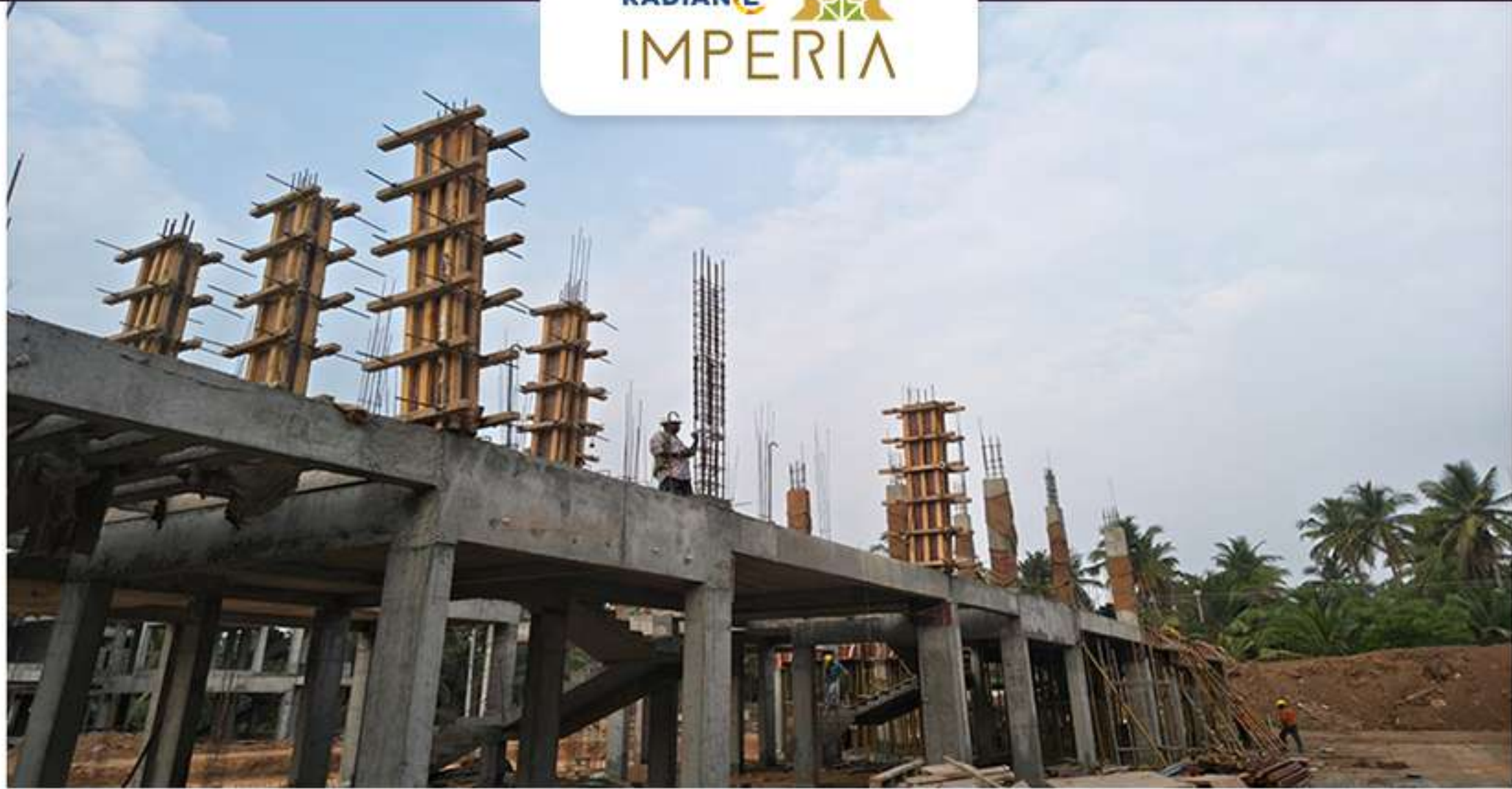
Villa 84 First Floor Column Work in Progress
