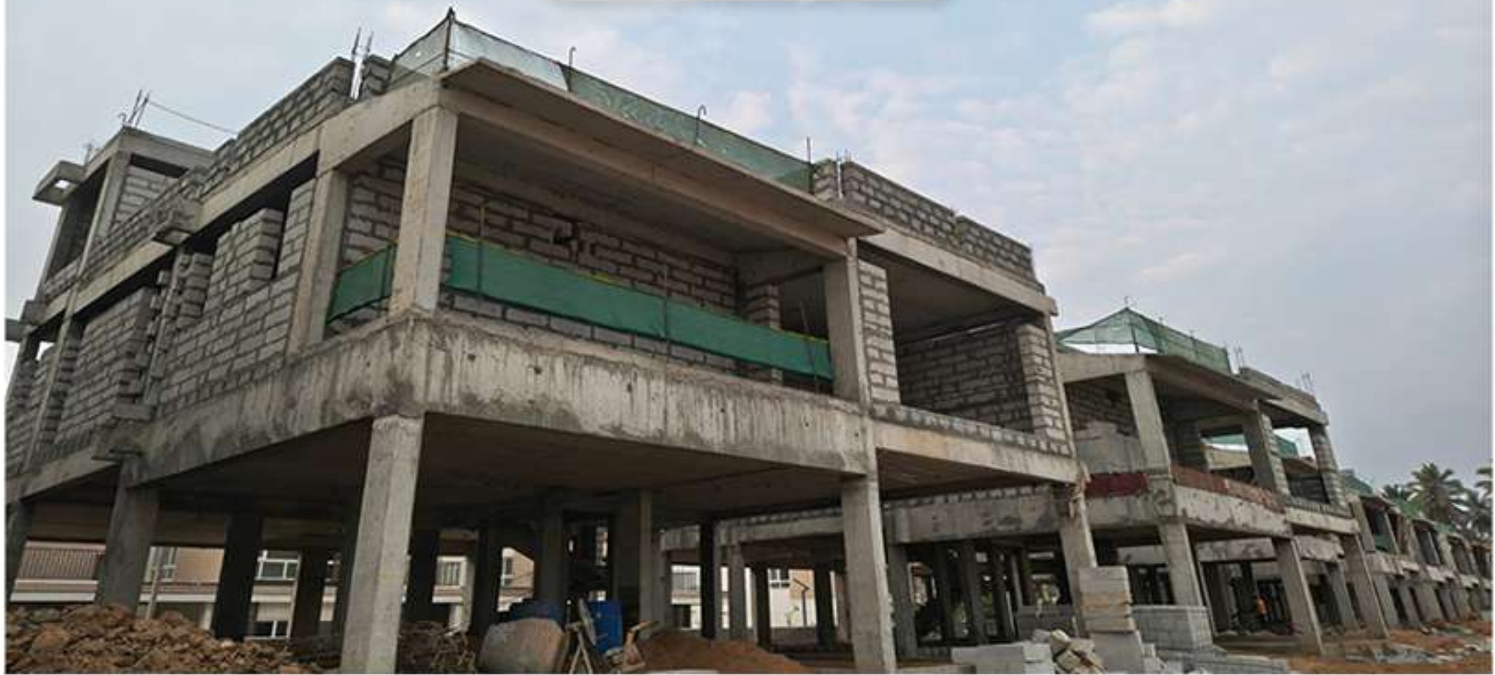
Villa no 9 Block Work is Work in Progress
