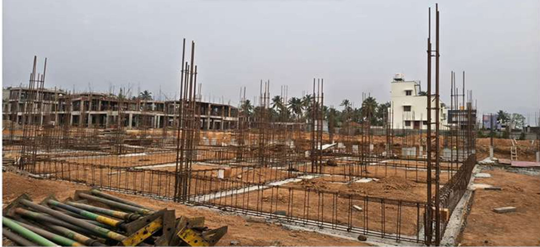
Villa no. 27 Plinth Beam Work in Progress
