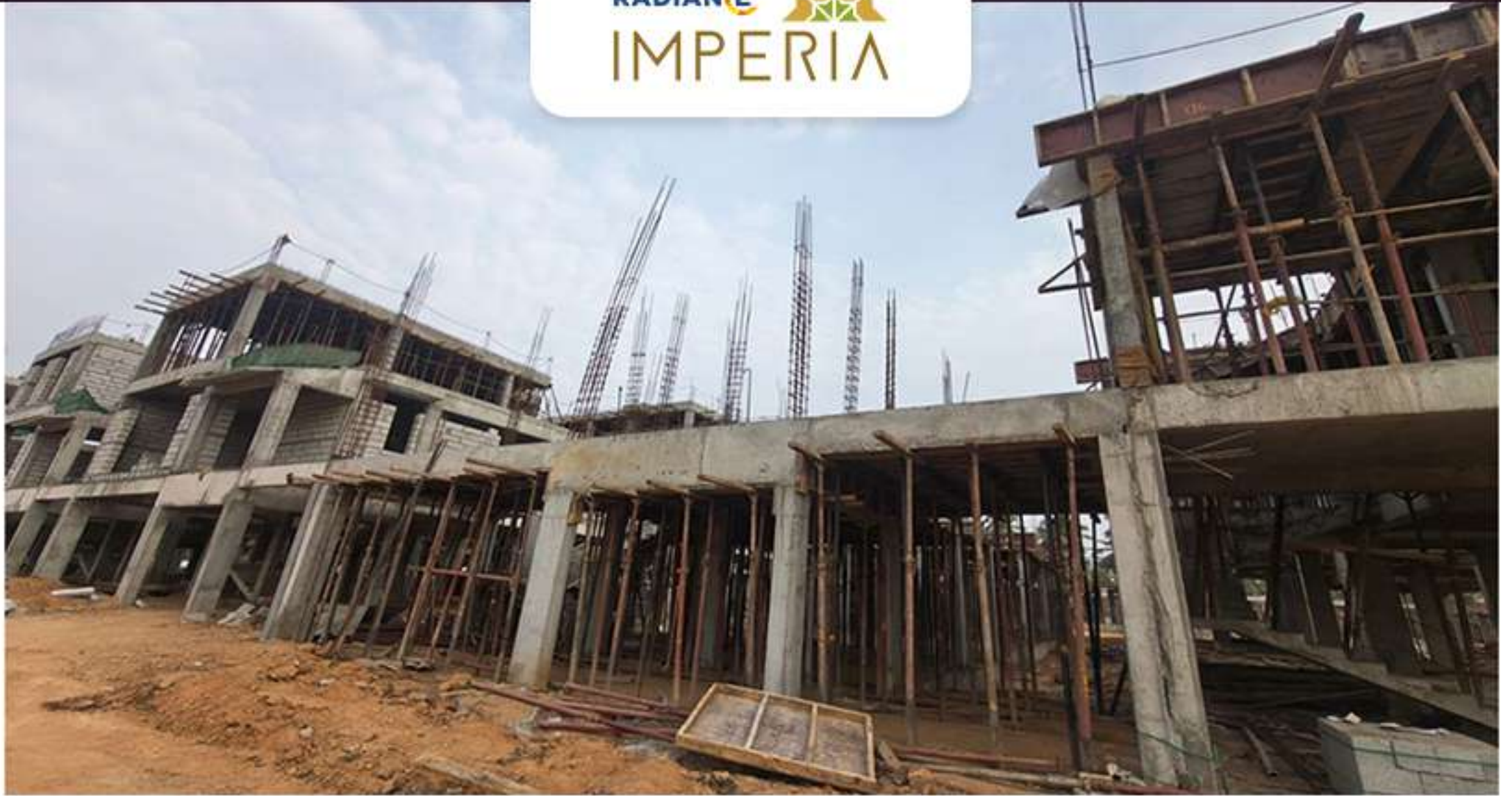
Villa 48 First Floor Column Work in Progress
