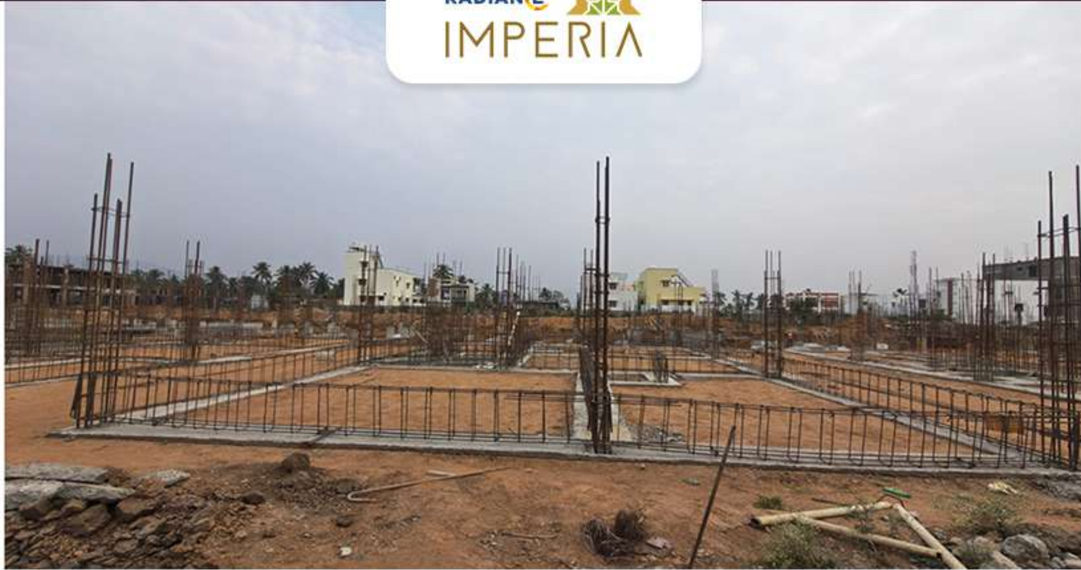
Villa no. 29 Plinth Beam Work in Progress
