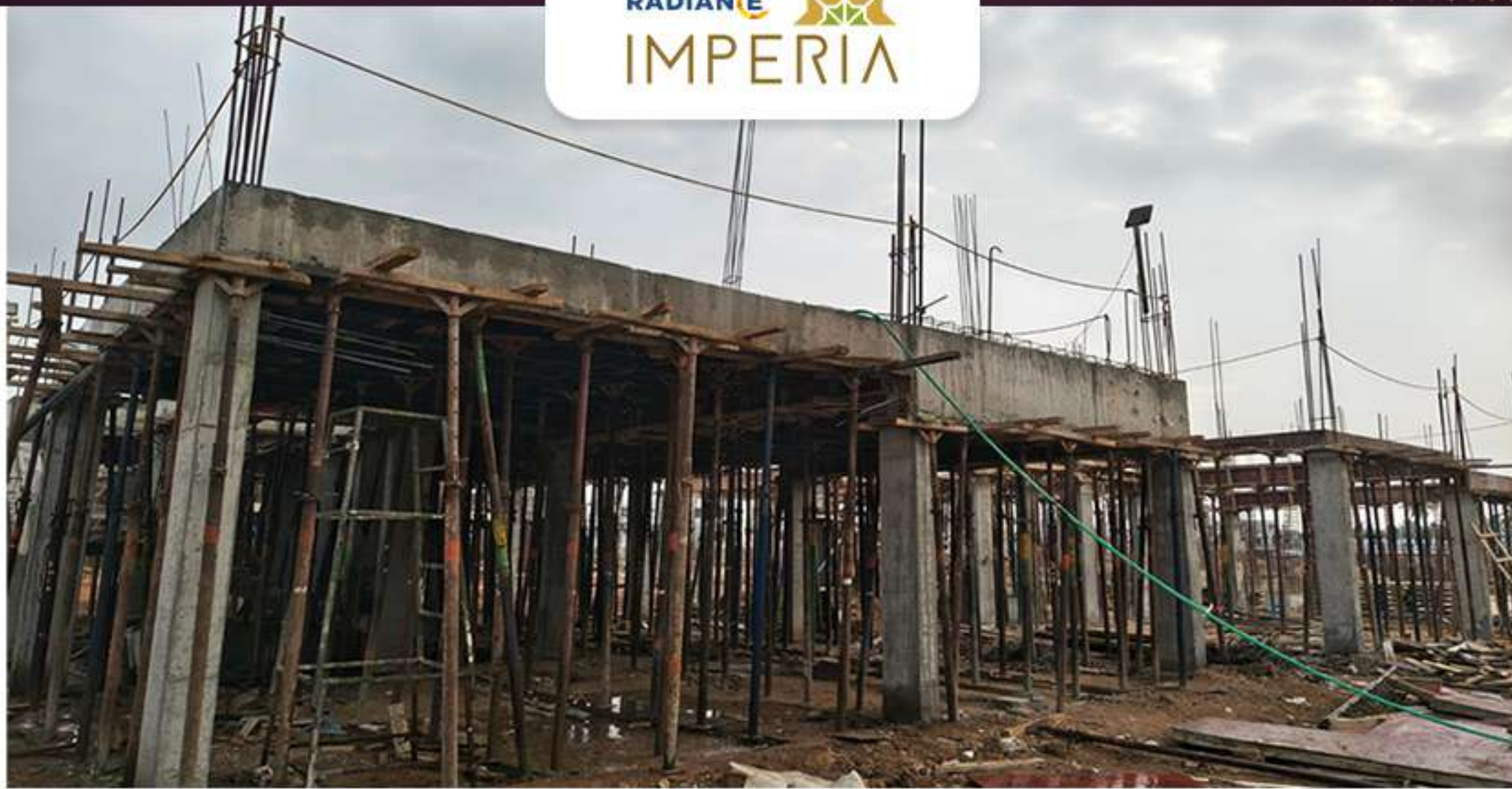
Villa no. 21 1st Floor Column Work in Progress
