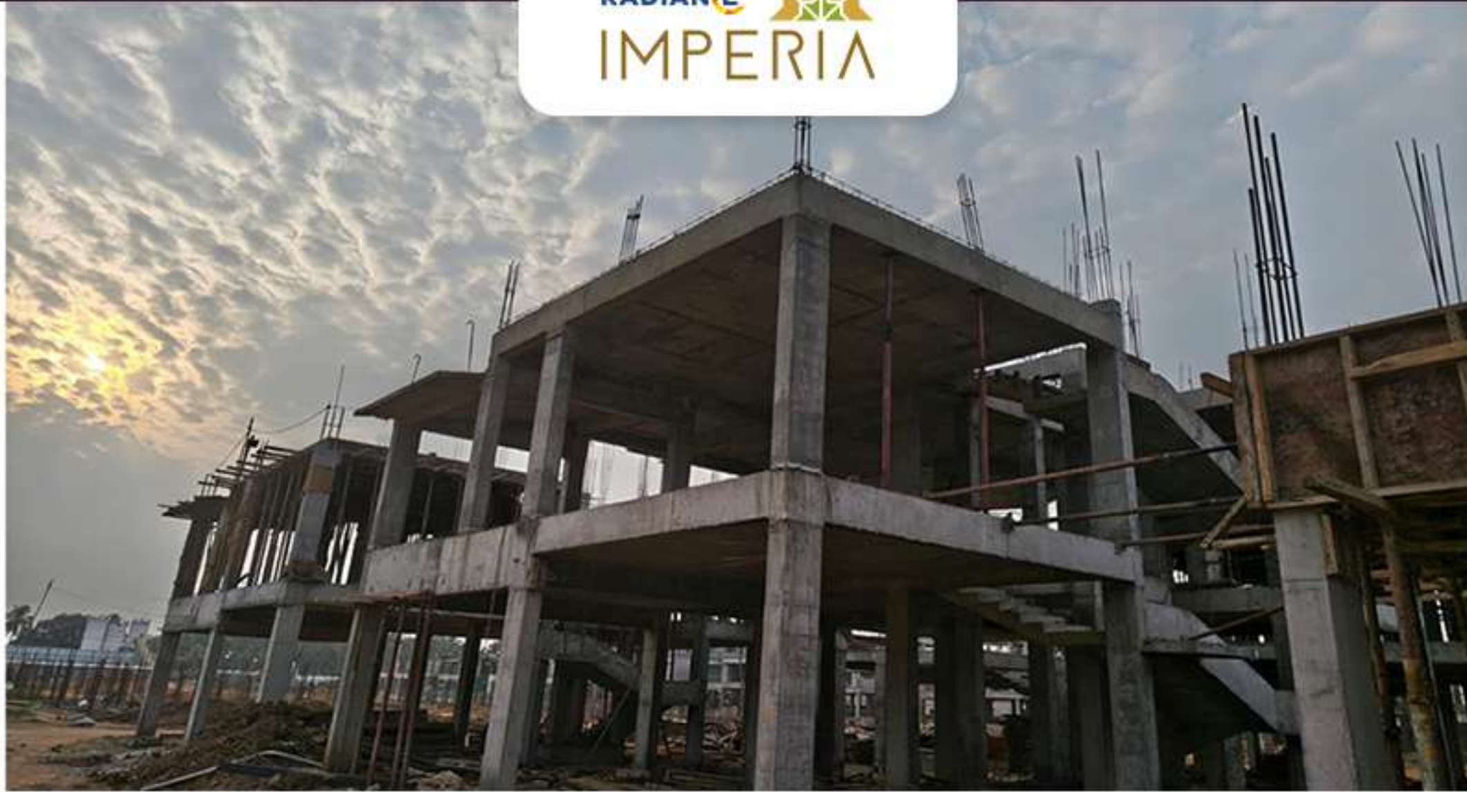
Villa 66 2nd Floor Column Work in Progress
