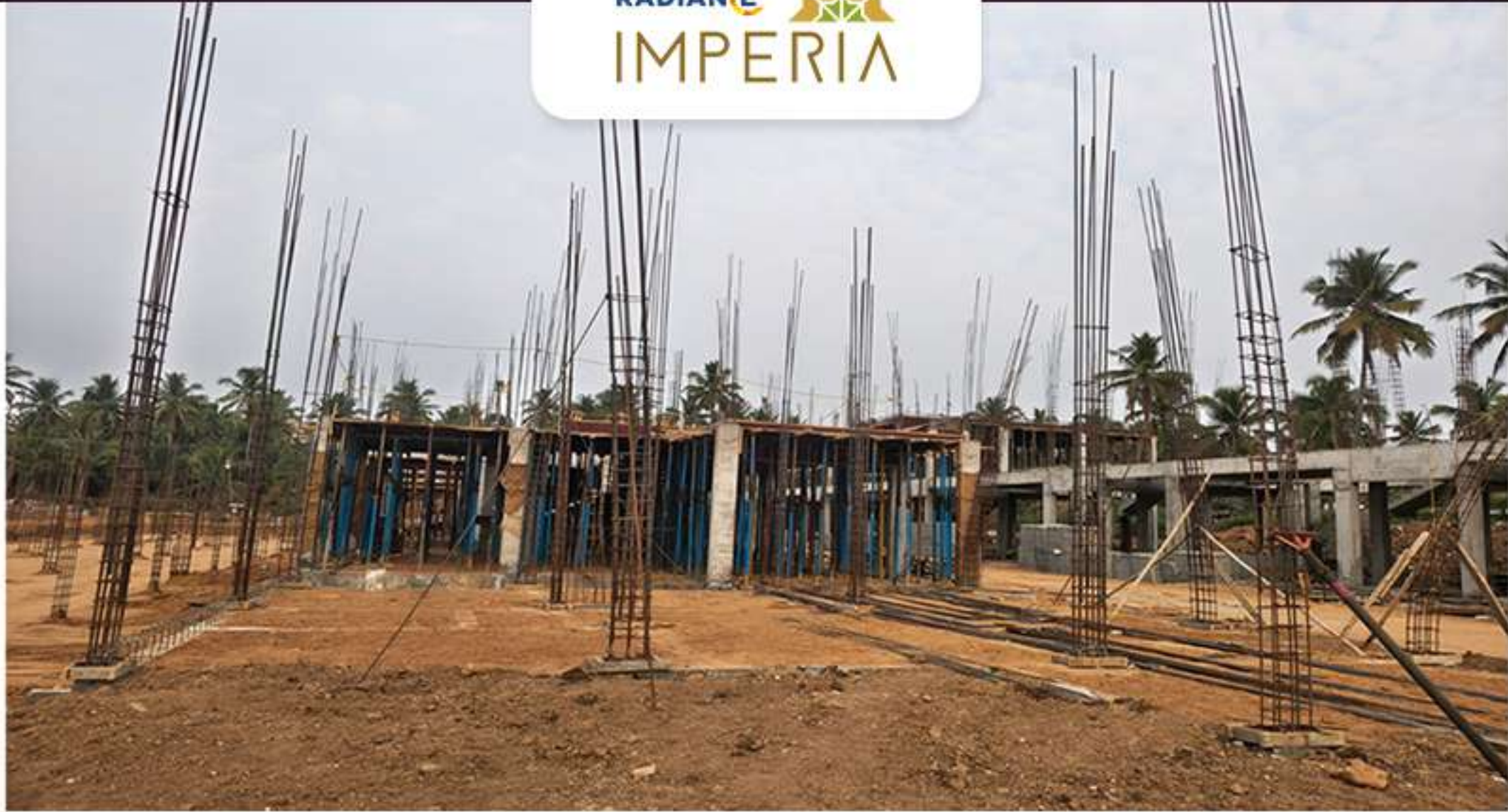
Villa 81 Ground Floor Column Work in Progress
