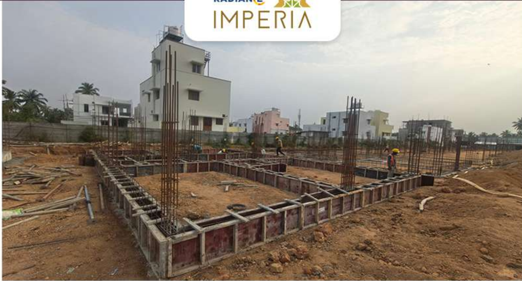
Villa 54 Plinth Beam Shuttering Work in Progress
