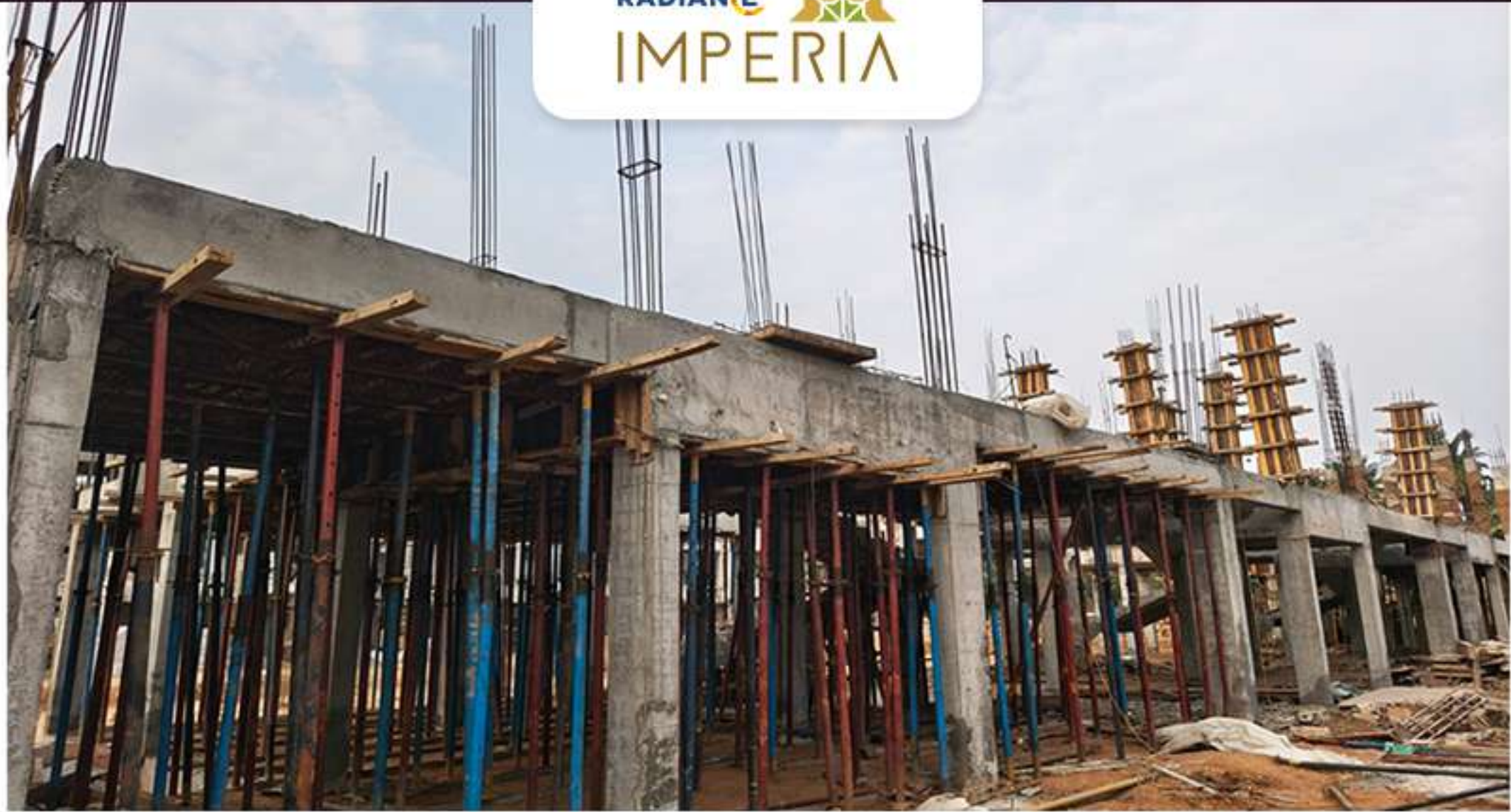
Villa 83 Ground Floor Roof Slab Completed
