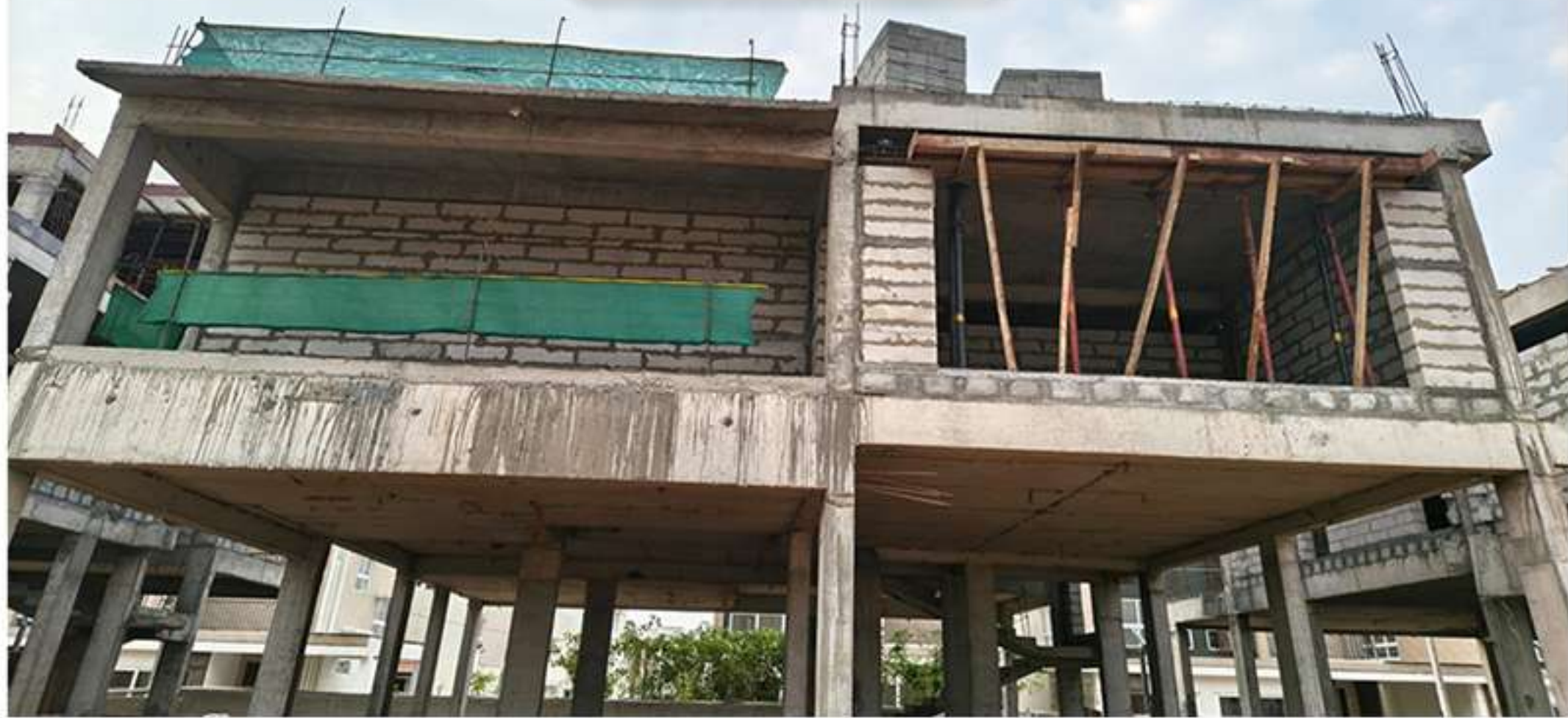
Villa no 12 Block Work is Work in Progress
