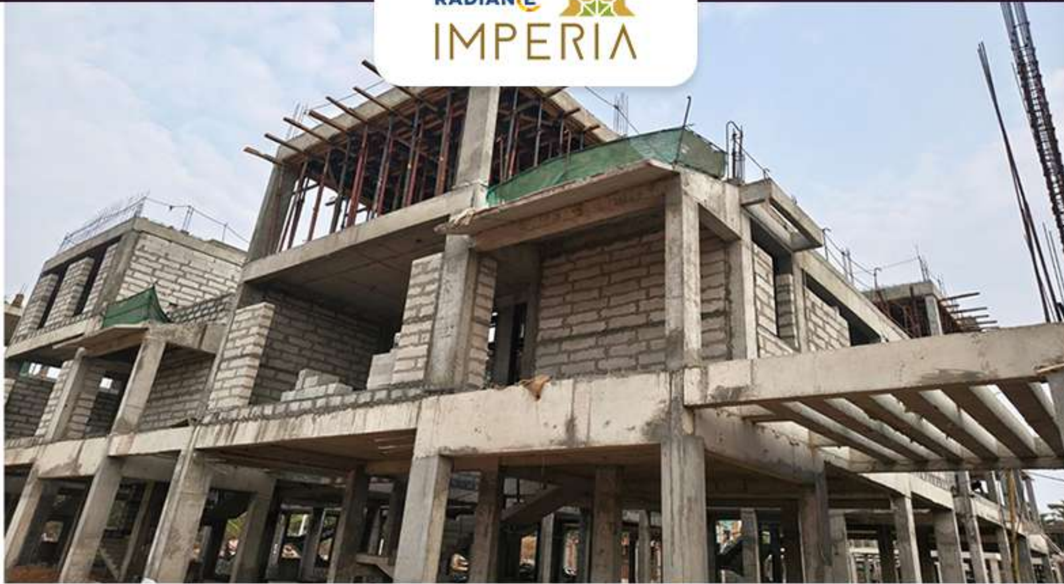
Villa 47 Block Work in Progress
