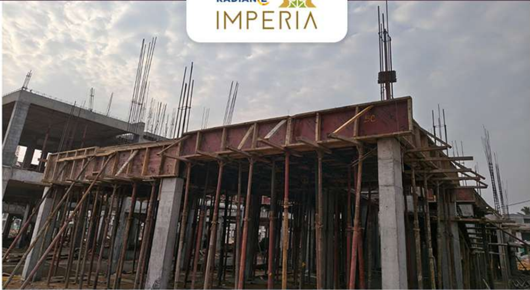
Villa 68 Ground Floor Slab Shuttering Work in Progress
