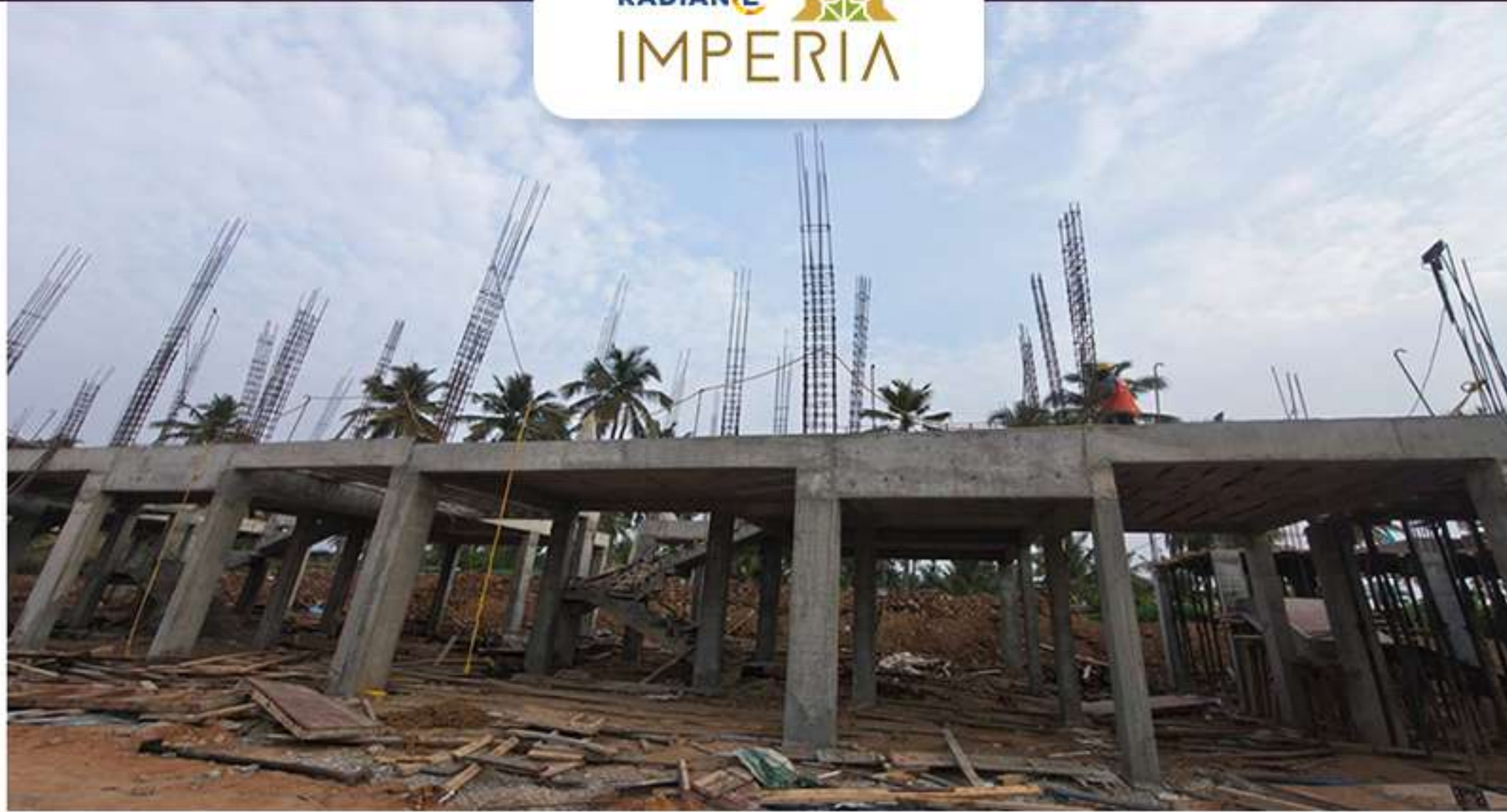
Villa 96 Ground Floor Roof Slab Completed
