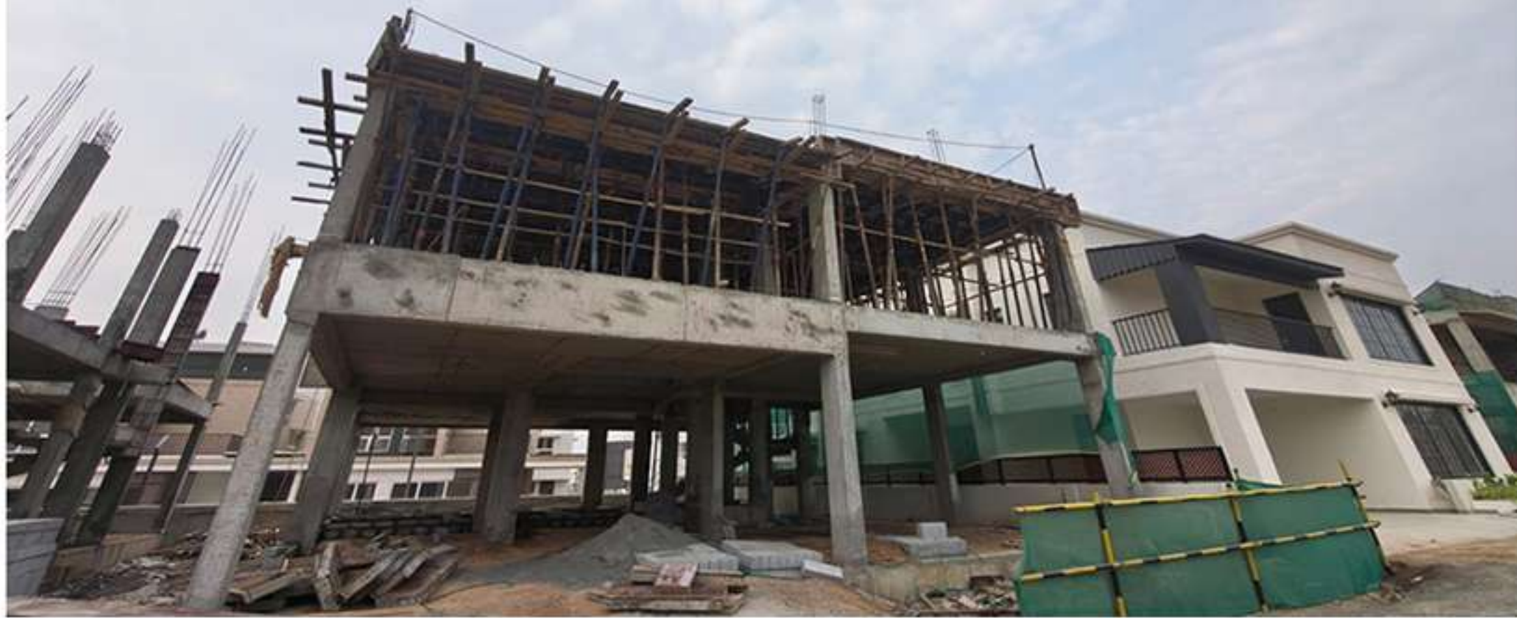
Villa no.4 1st Floor Roof Slab Work in Progress.
