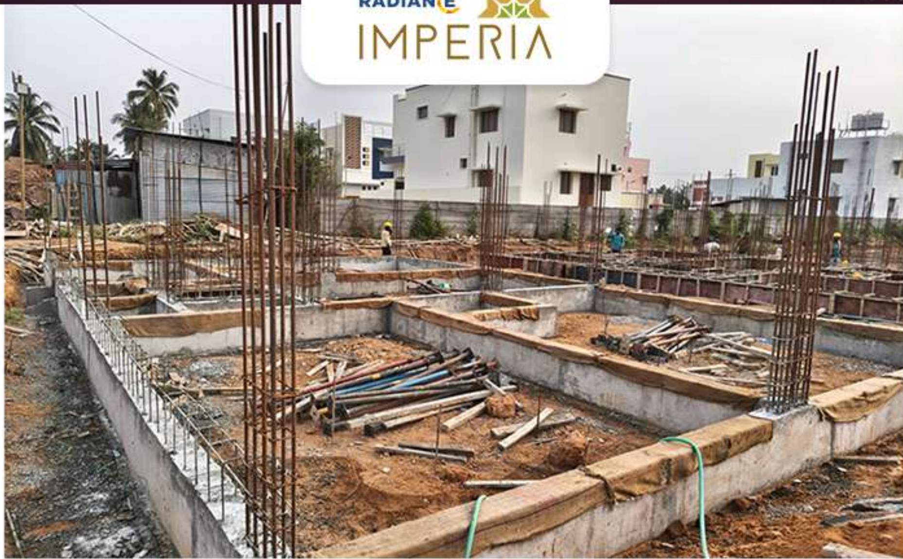
Villa 52 Plinth Beam Completed
