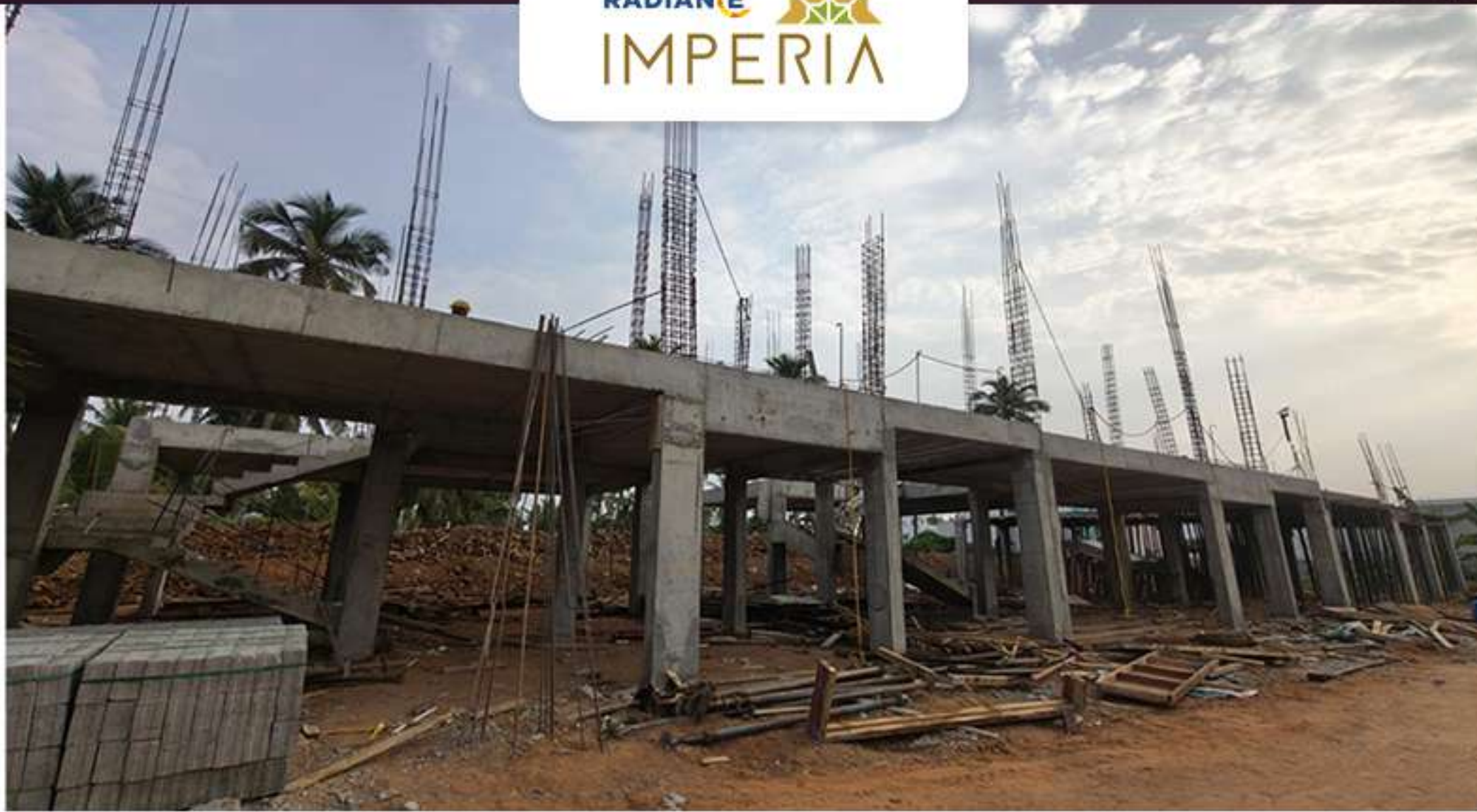
Villa 95 Ground Floor Roof Slab completed
