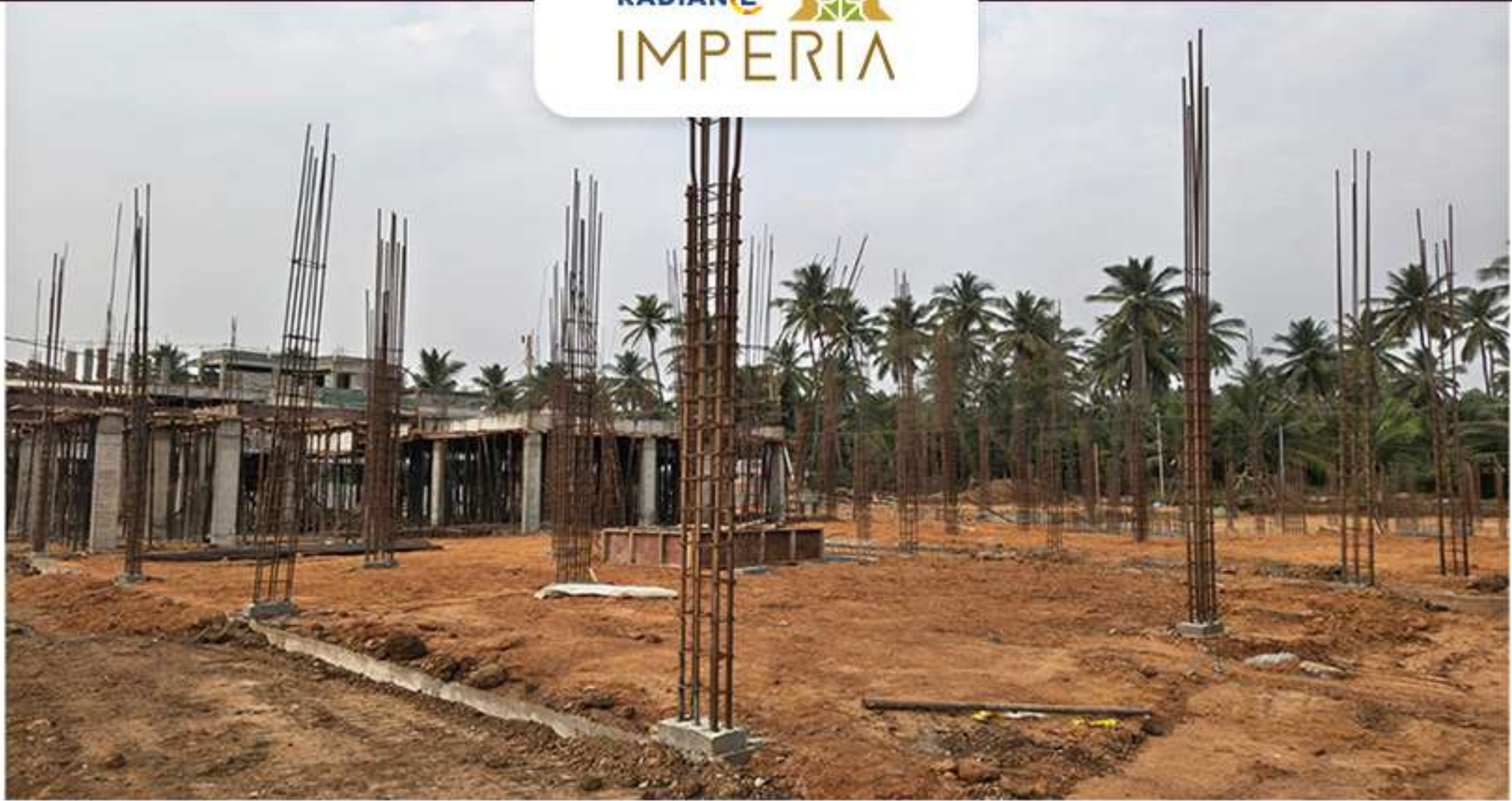
Villa 40 Ground Floor Column Work in Progress
