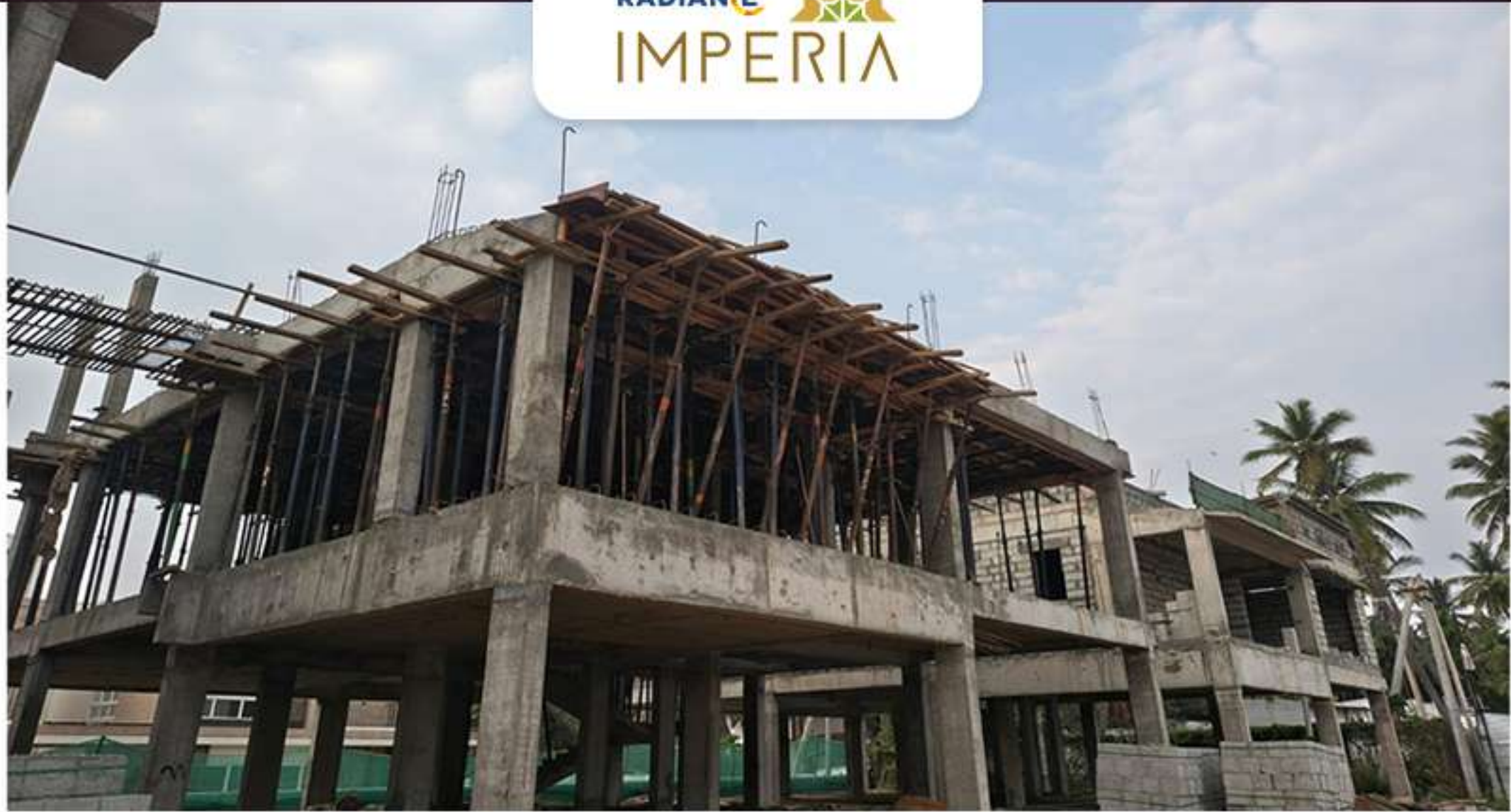
Villa no. 16 2nd Floor Roof Slab Work in Progress
