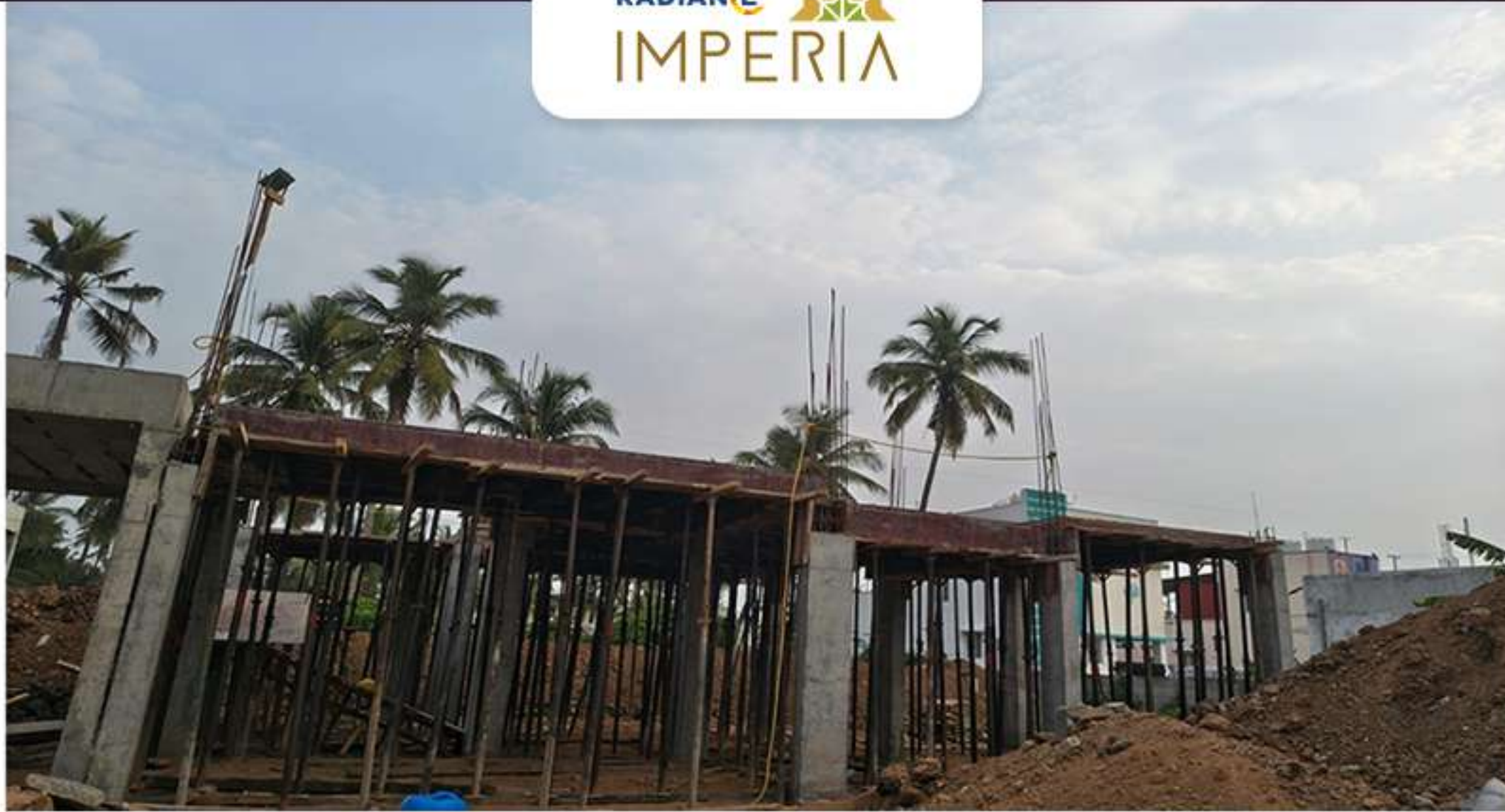
Villa 97 Ground Floor Roof Slab Shuttering Work in Progress
