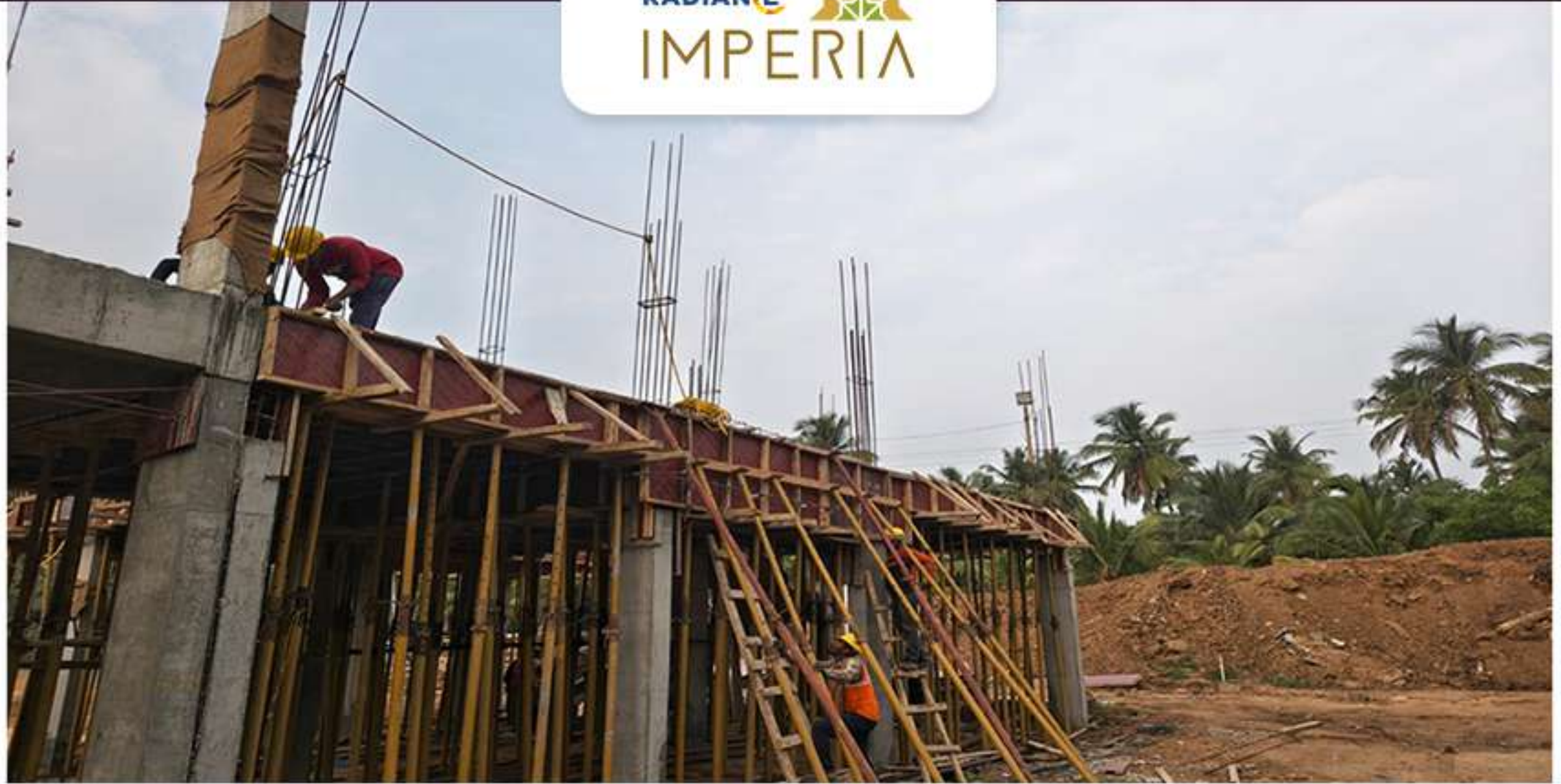
Villa 87 Ground Floor Slab Shuttering Work in Progress
