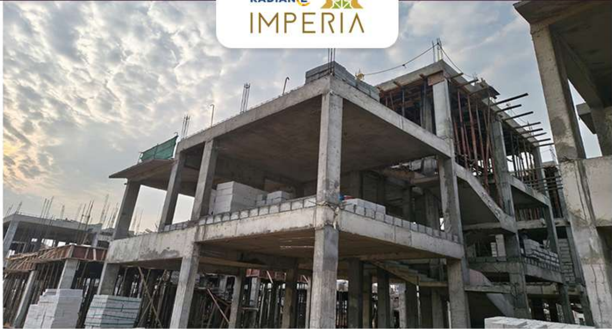
Villa 69 Block Work in Progress
