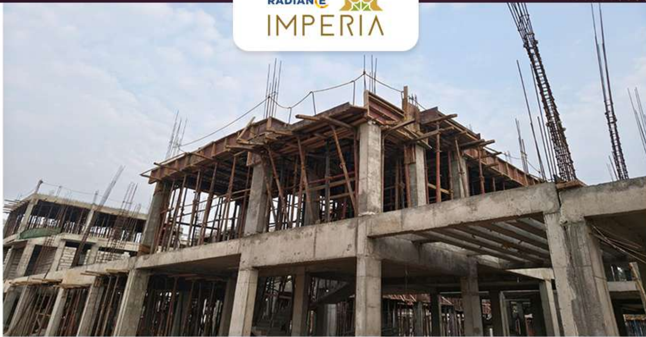
Villa 50 First Floor Slab Concrete Completed
