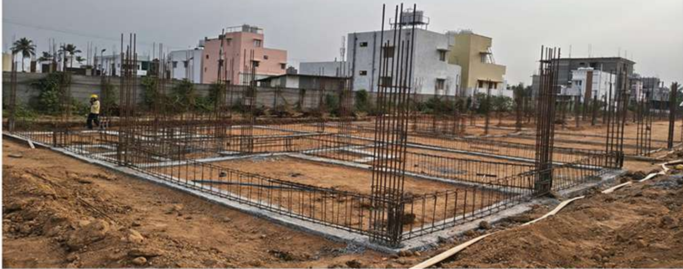
Villa 55 Plinth Beam Shuttering Work in Progress
