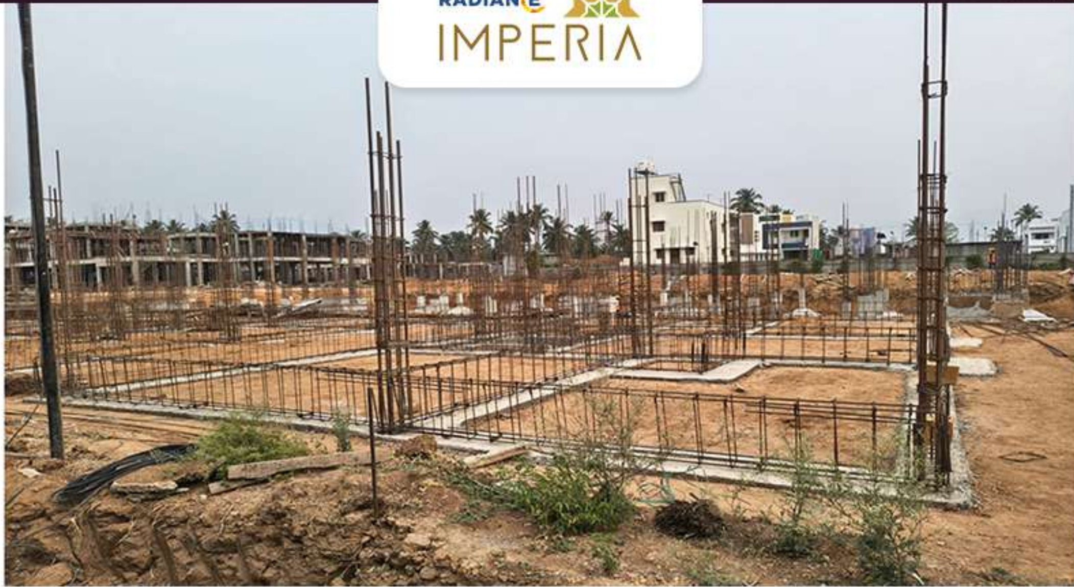
Villa no. 28 Plinth Beam Work in Progress
