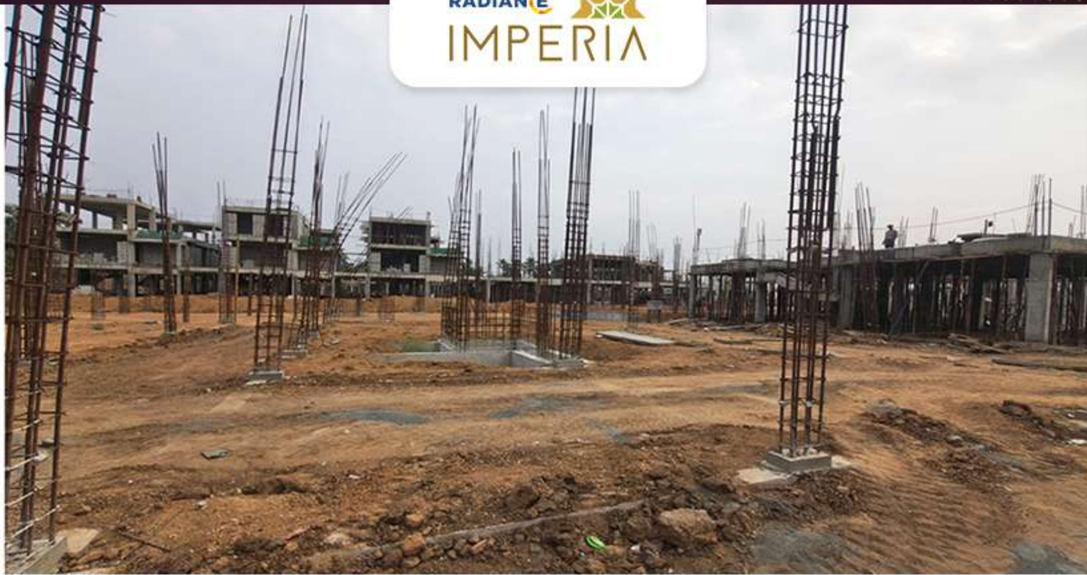
Villa no. 20 Ground Floor Column Work in Progress
