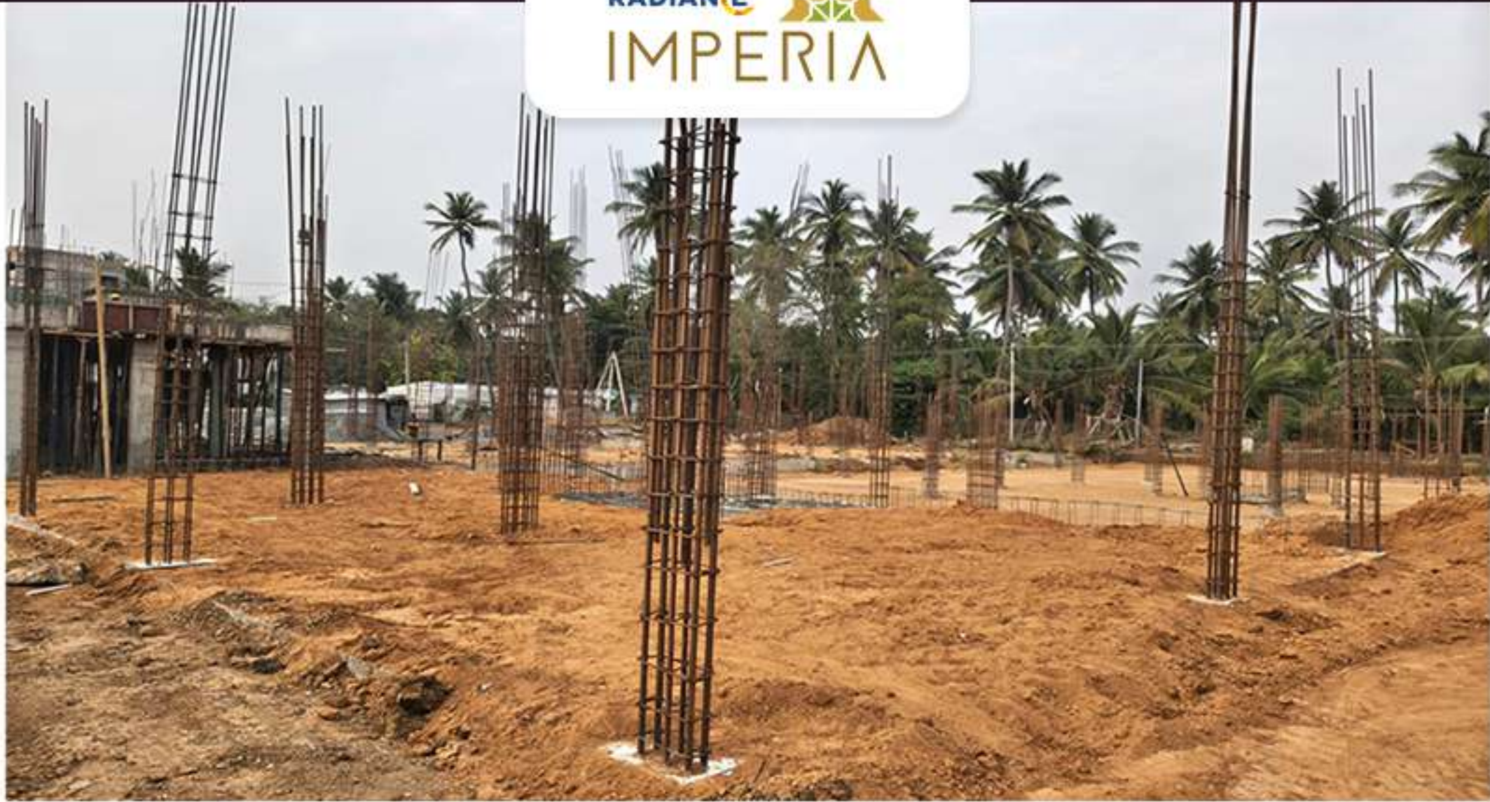
Villa 41 ground Floor Column Work in Progress
