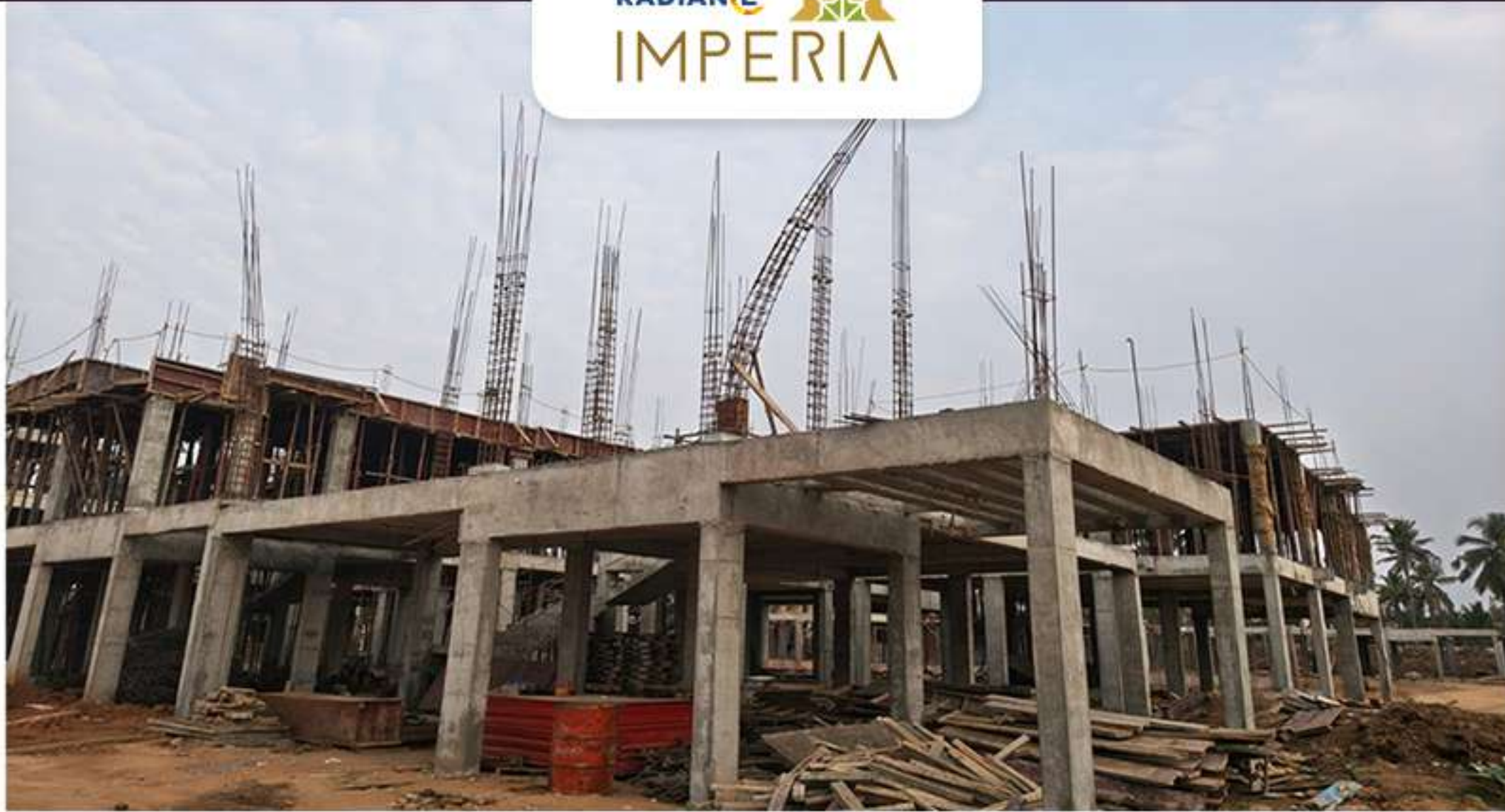
Villa 51 First Floor Column Work in Progress
