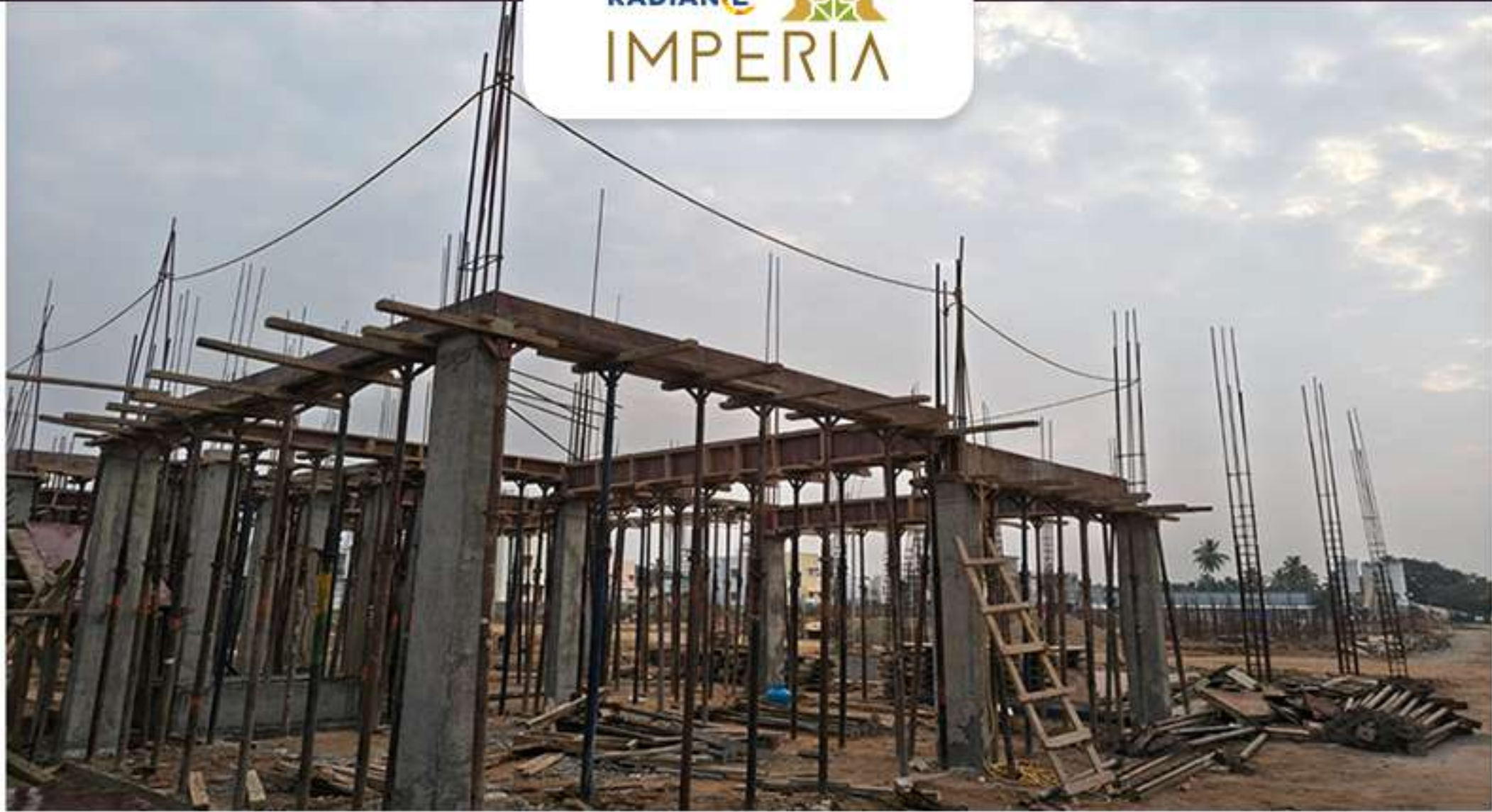
Villa no. 22 Ground Floor Roof Slab Work in Progress
