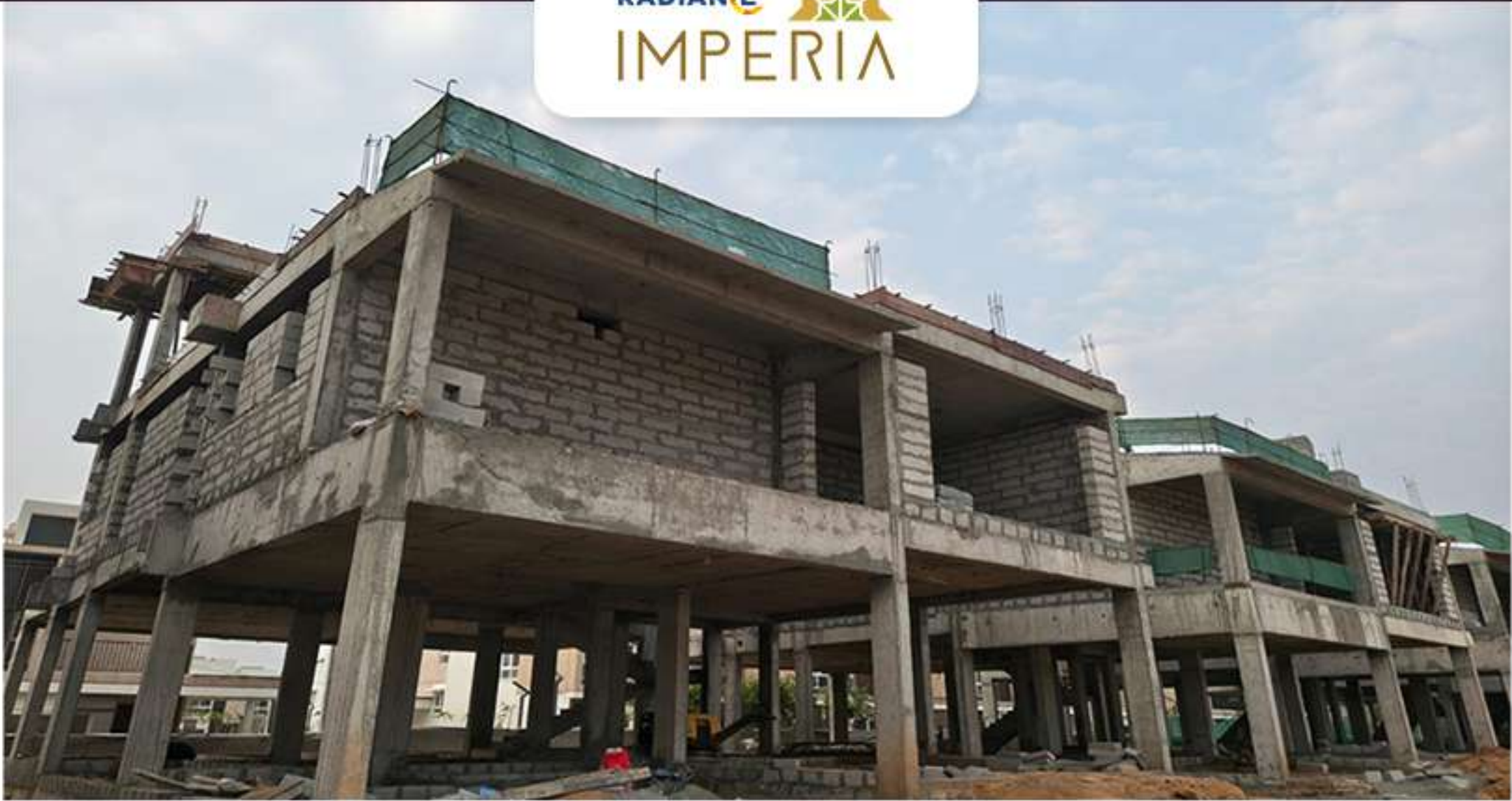
Villa no. 11 Block Work is Work in Progress
