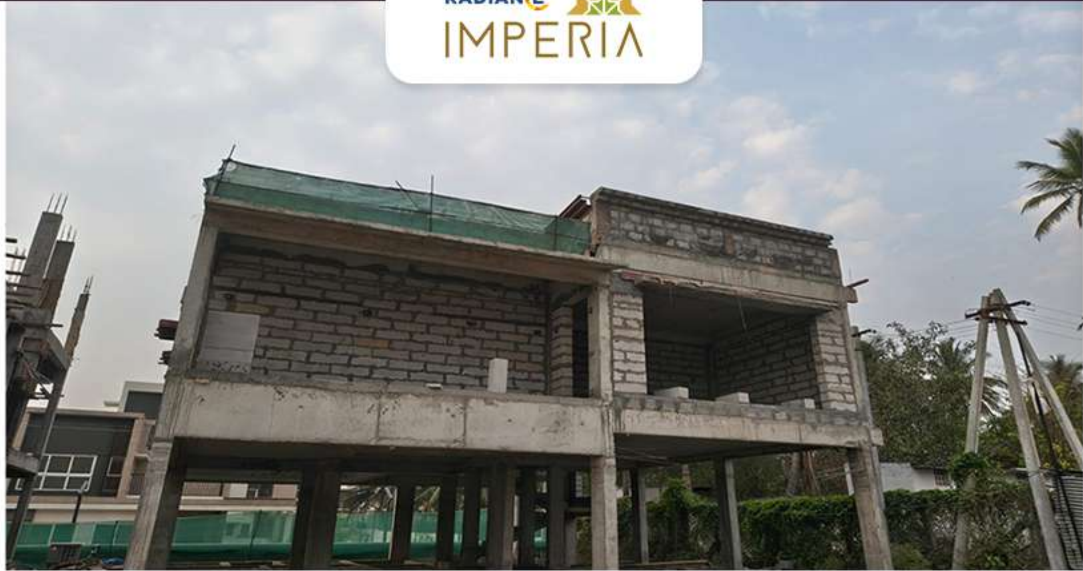
Villa no. 18 Block Work in Progress
