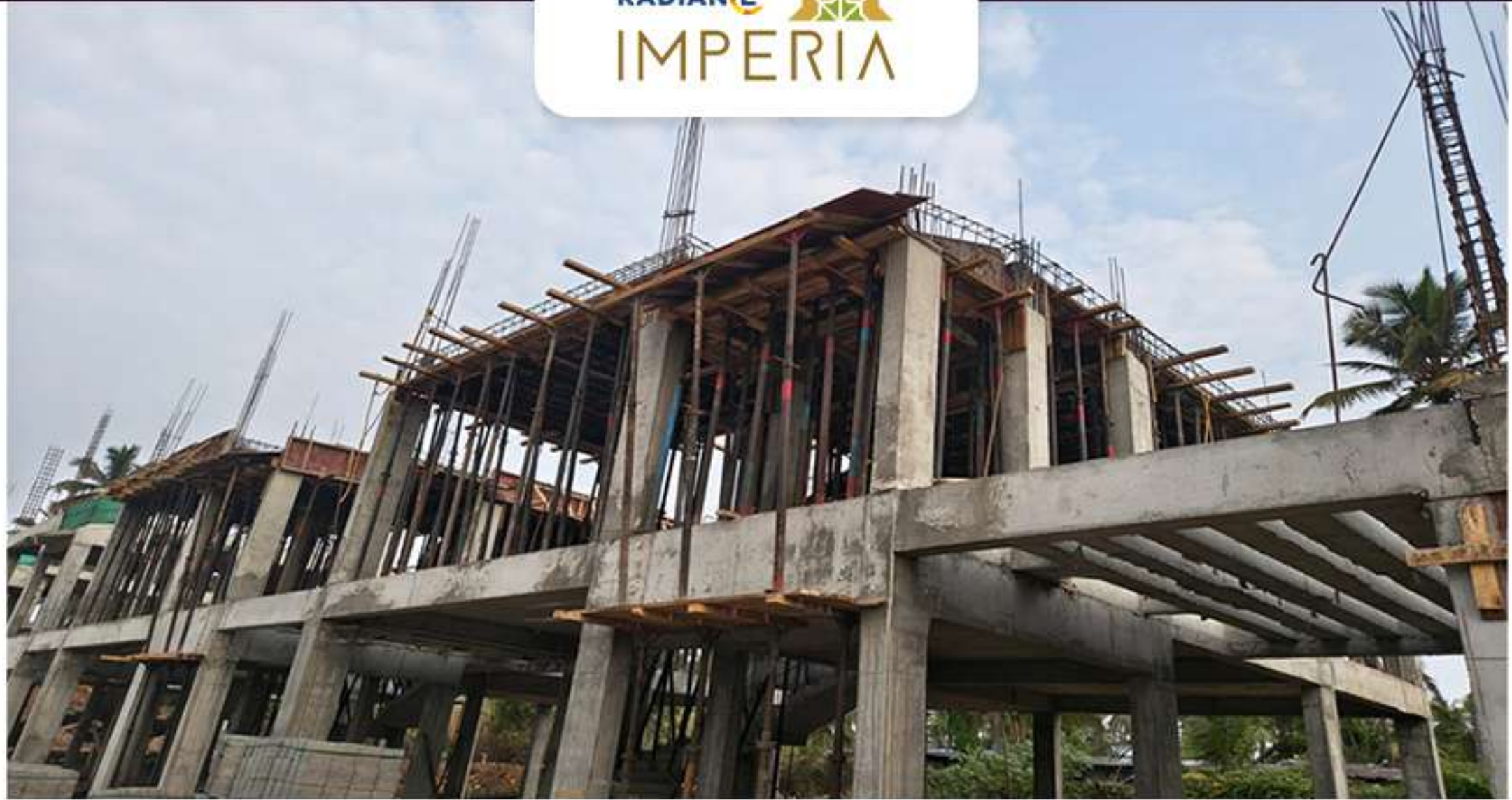
Villa 92 1st Floor Roof Slab Shuttering Work in Progress
