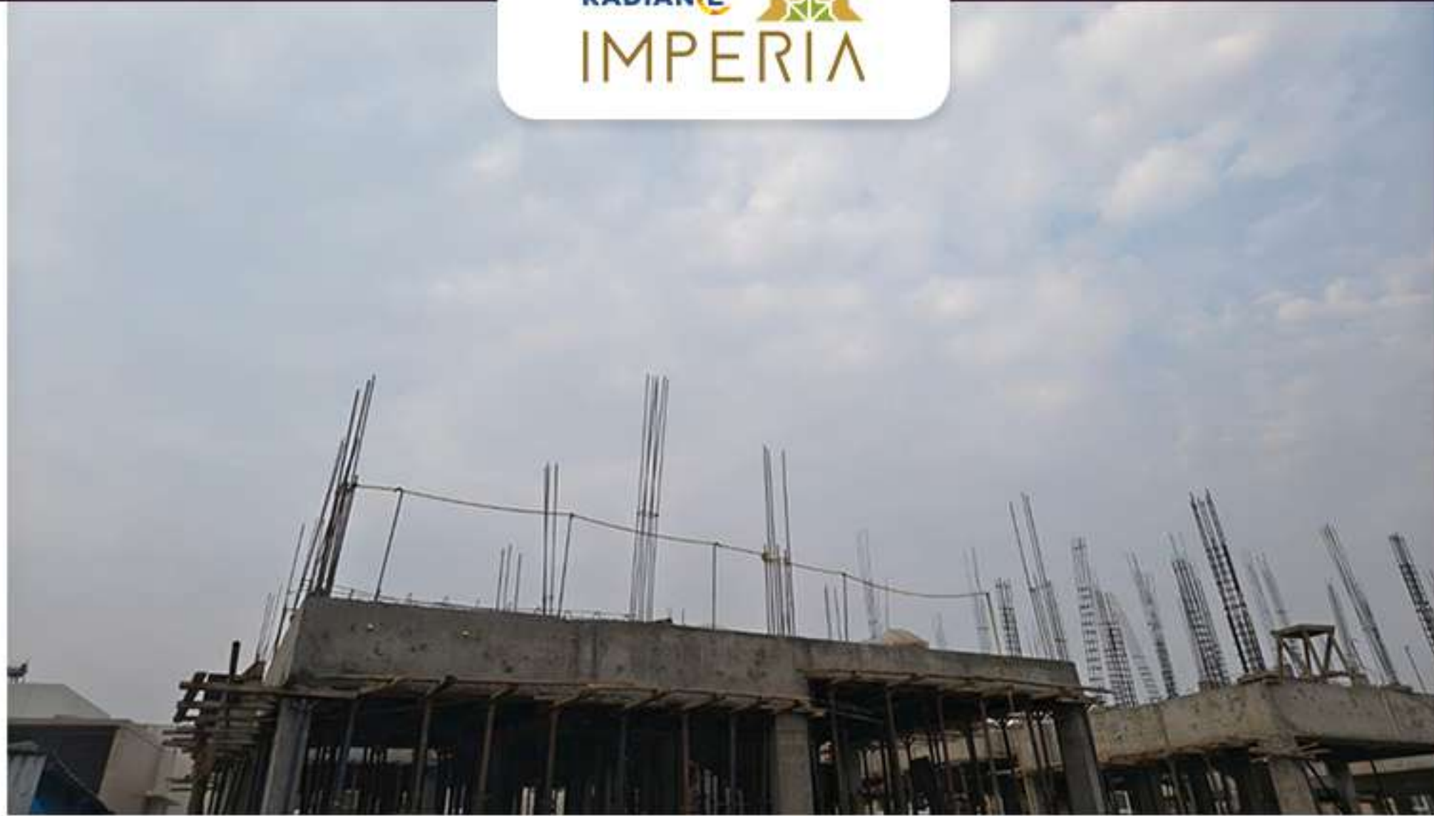
Villa No. 1 -1st Floor Column Marking Work In Progress
