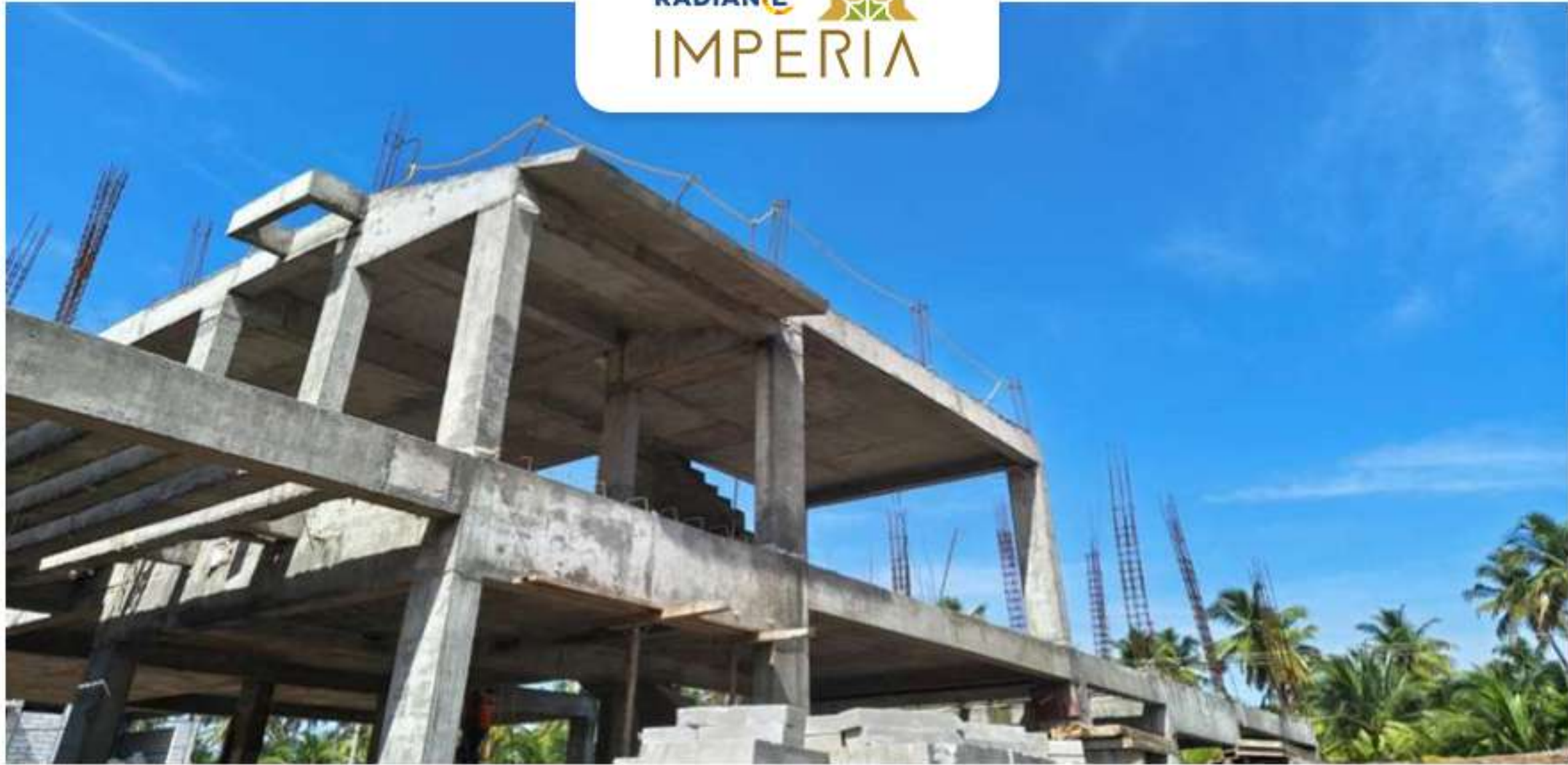
Villa no – 86 First Floor Roof Slab Completed
