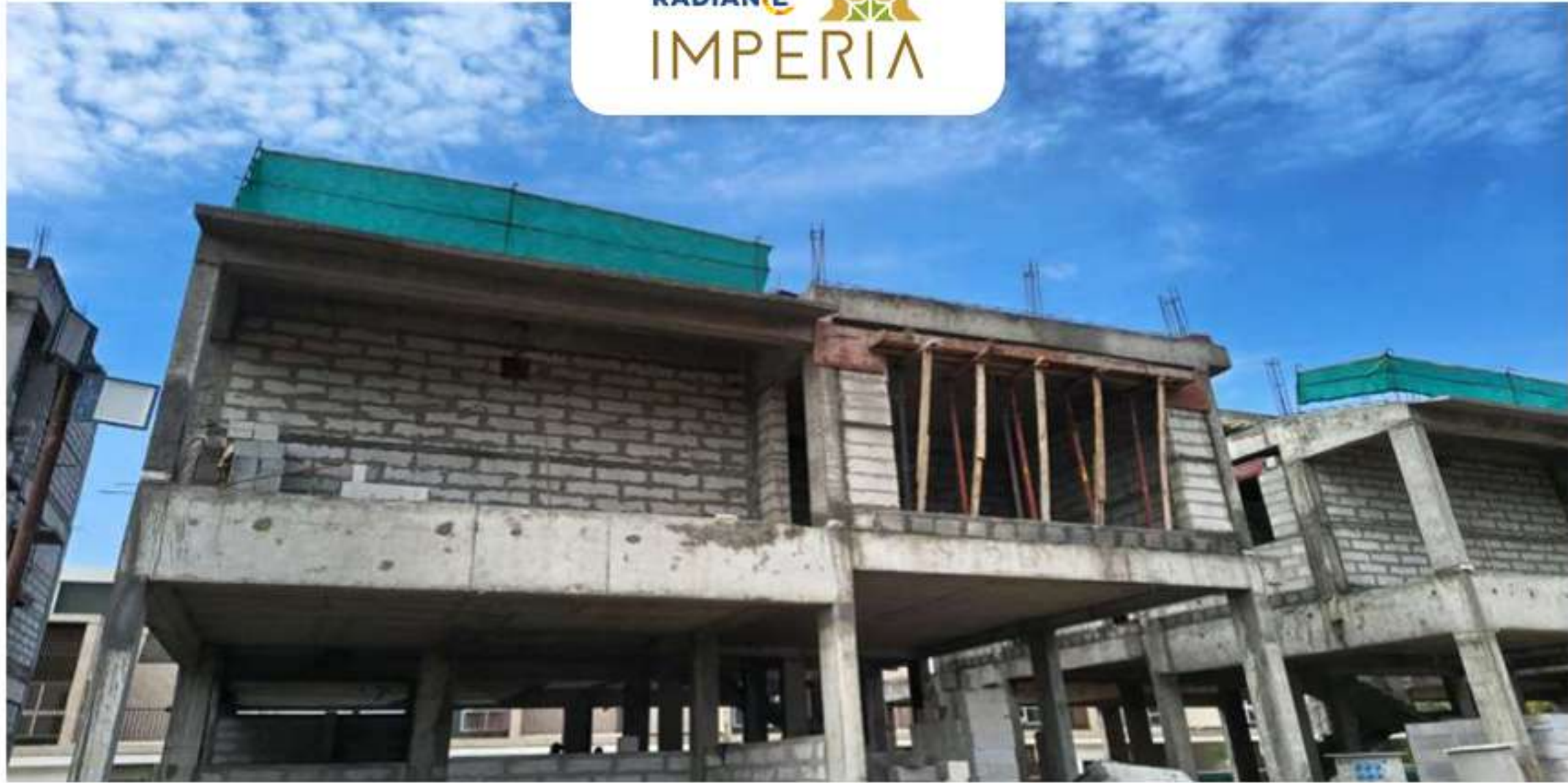
Villa no -14 Block Work in progress
