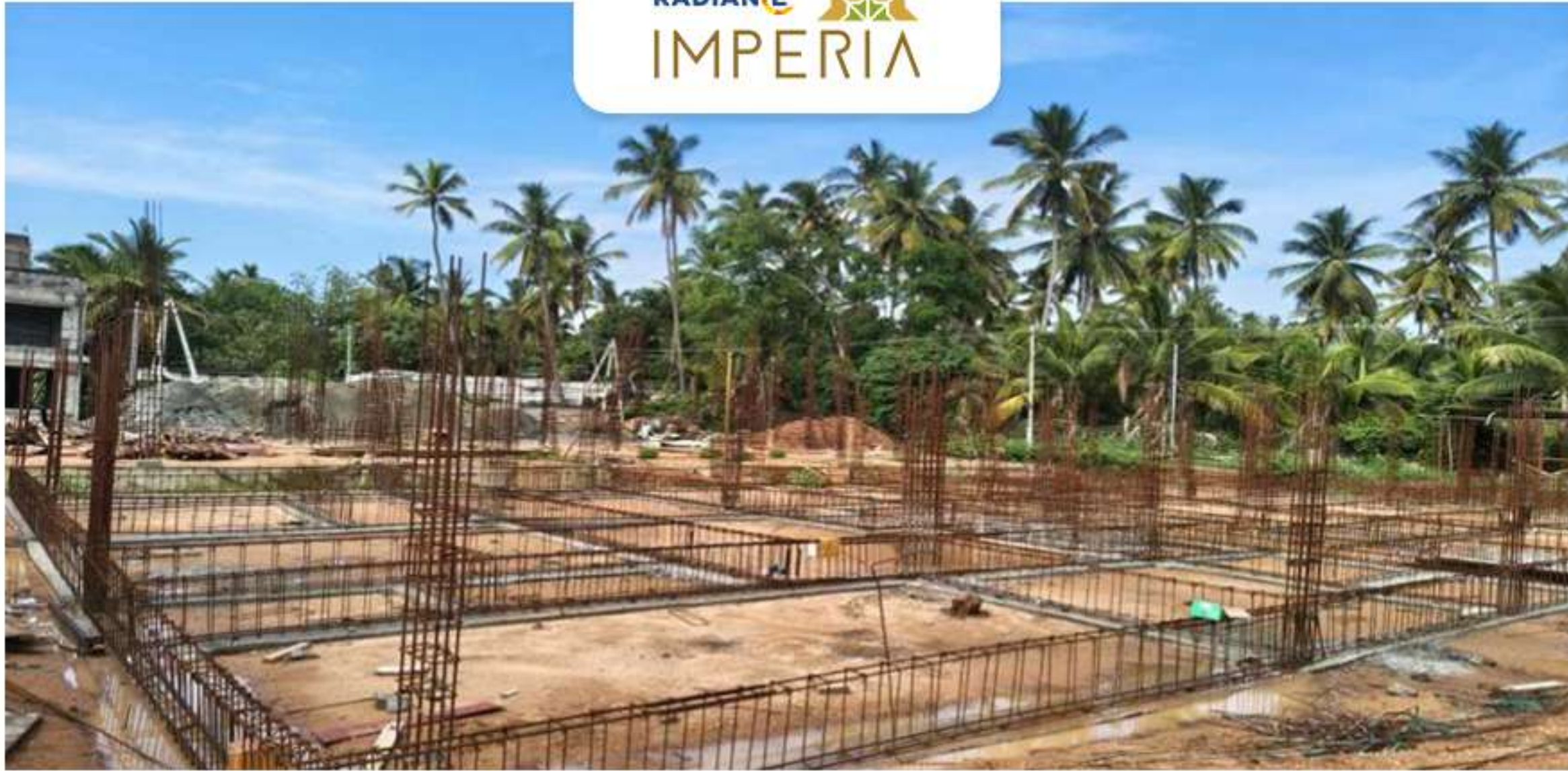
Villa no -42 plinth Beam Work in progress
