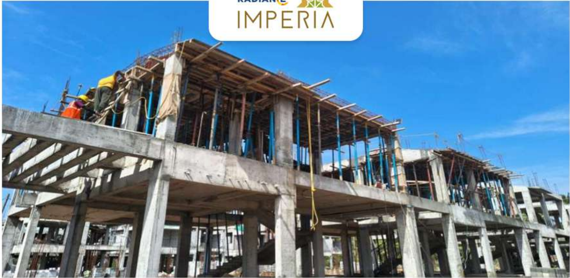
Villa no – 82 First floor Roof Slab Shuttering Work in Progress
