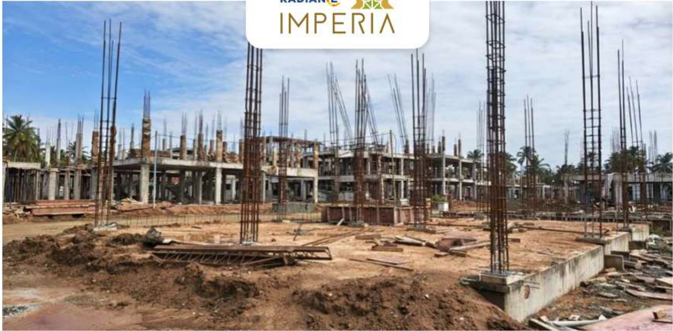
Villa no -24 Ground Floor Column Work in Progress
