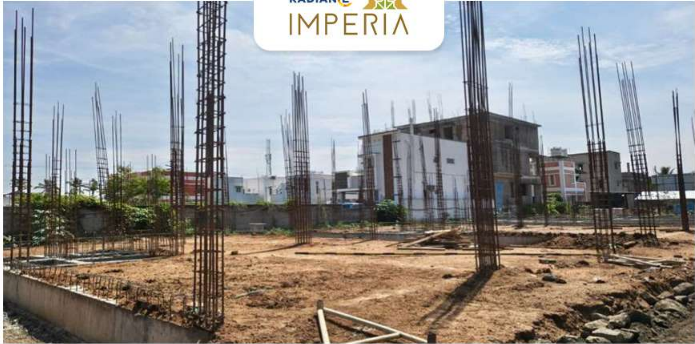
Villa no 60 Ground Floor Column Work in Progress
