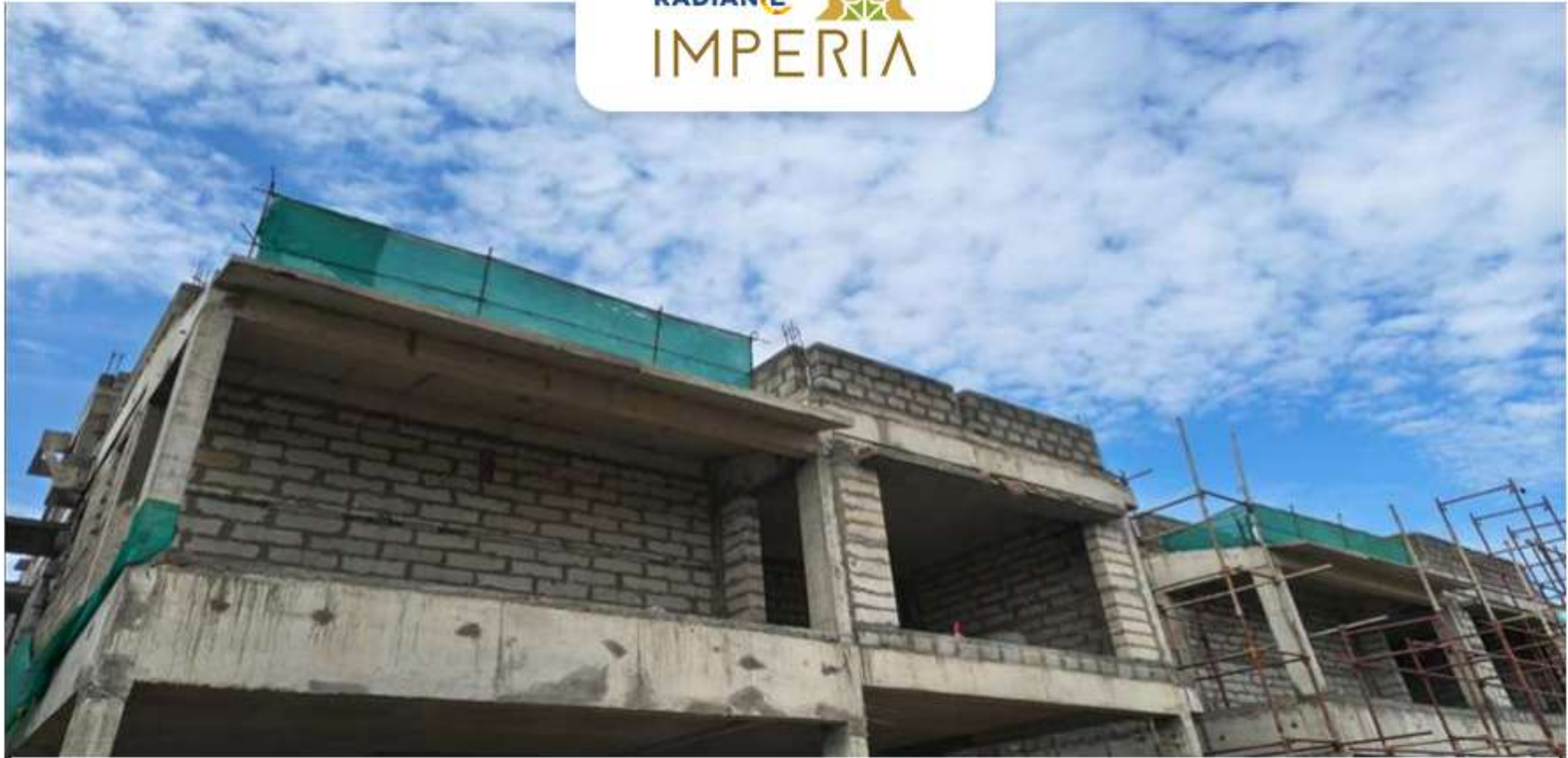
Villa no. 6 Block Work in progress
