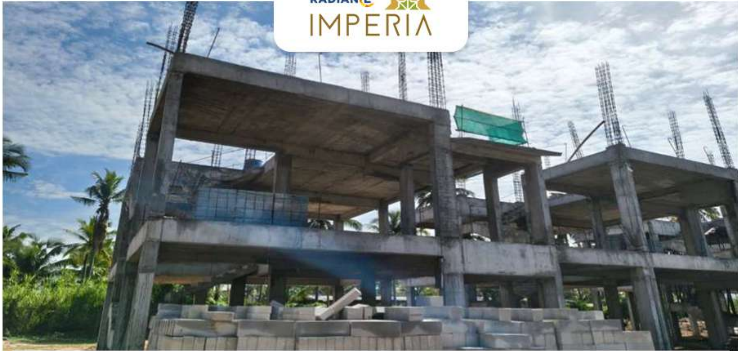
Villa no - 88 First Floor Roof Slab Completed
