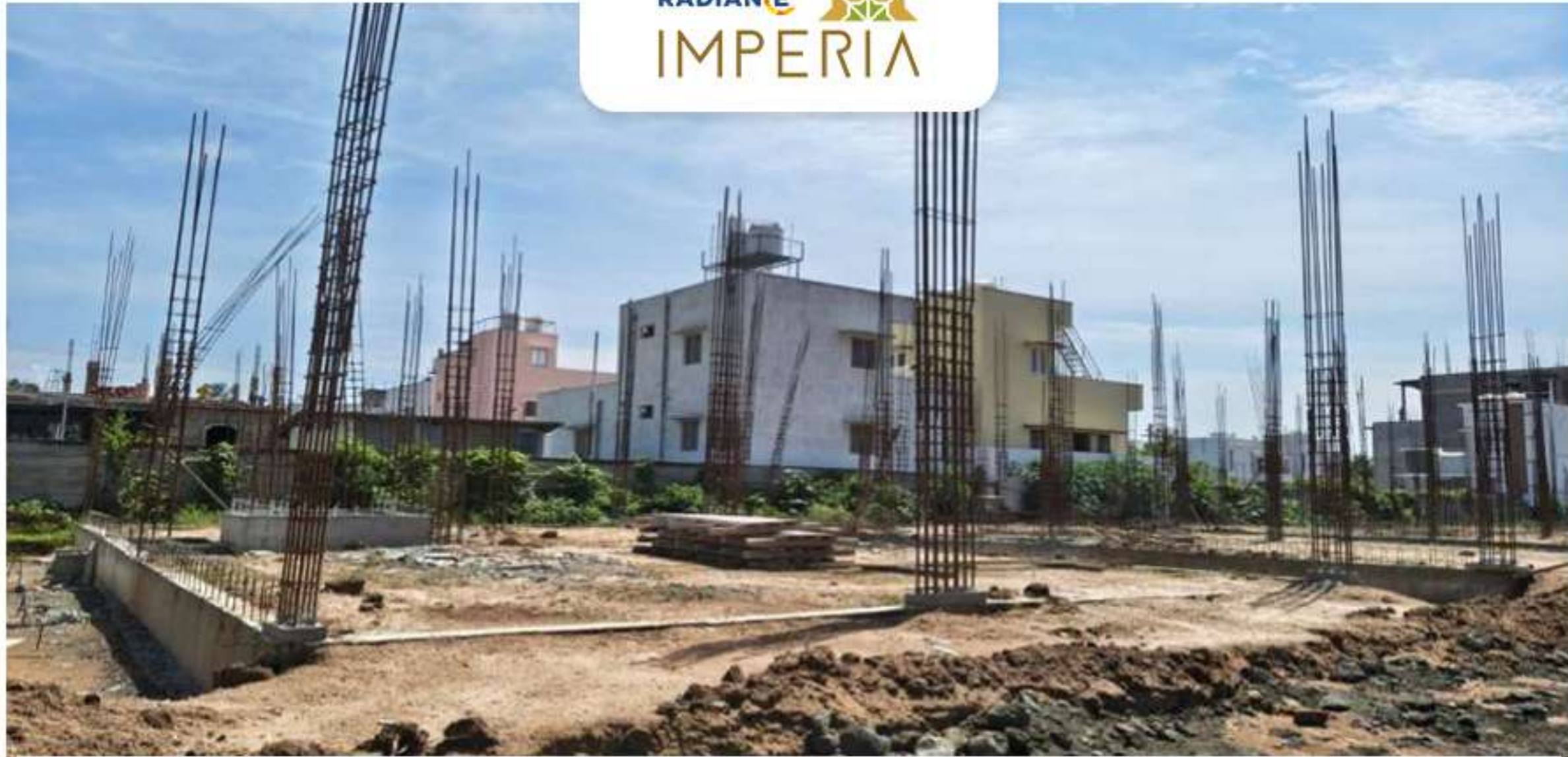
Villa no -56 Ground Floor Column Work in Progress
