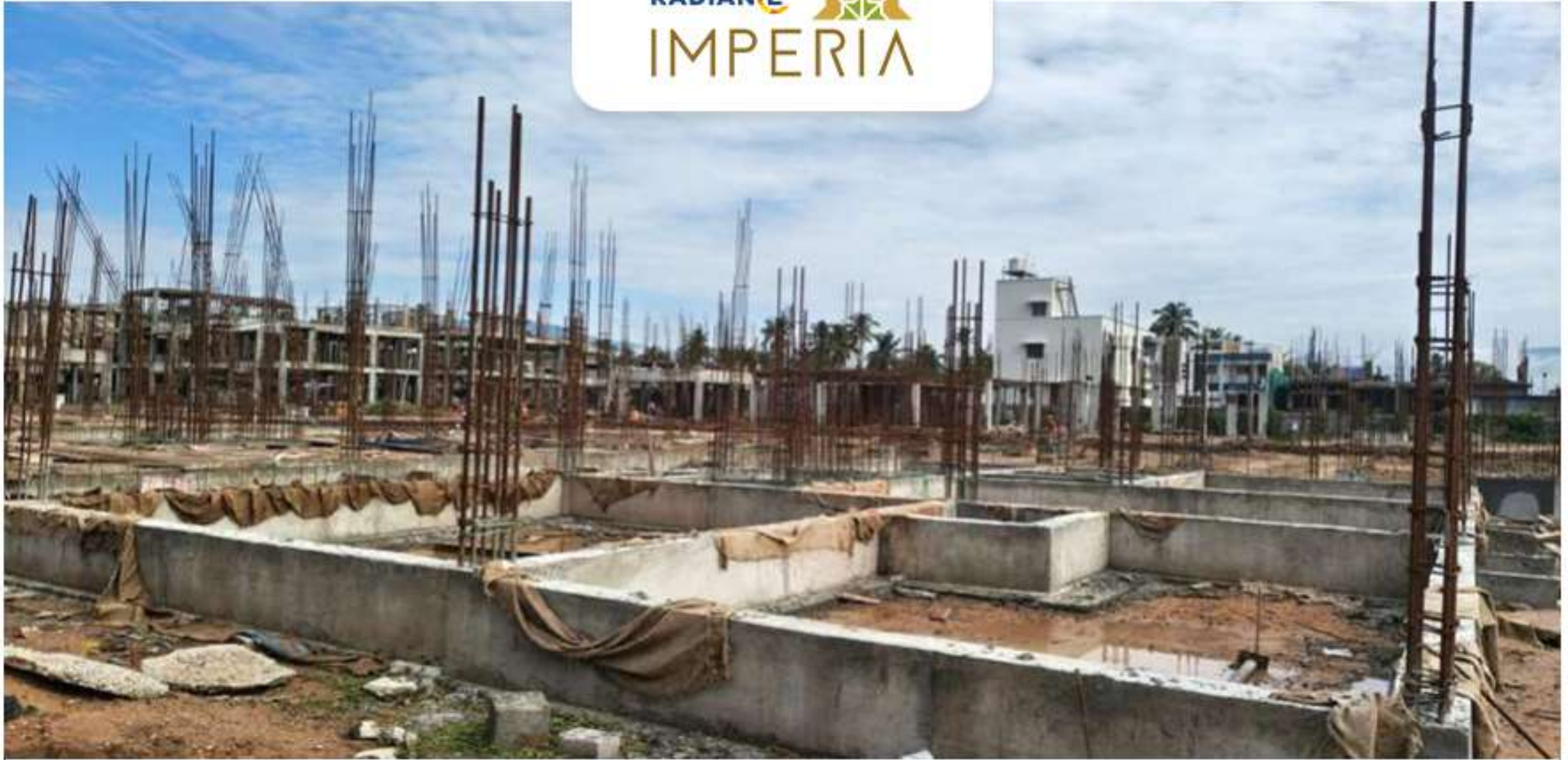
Villa no 28 Plinth Beam Completed.
