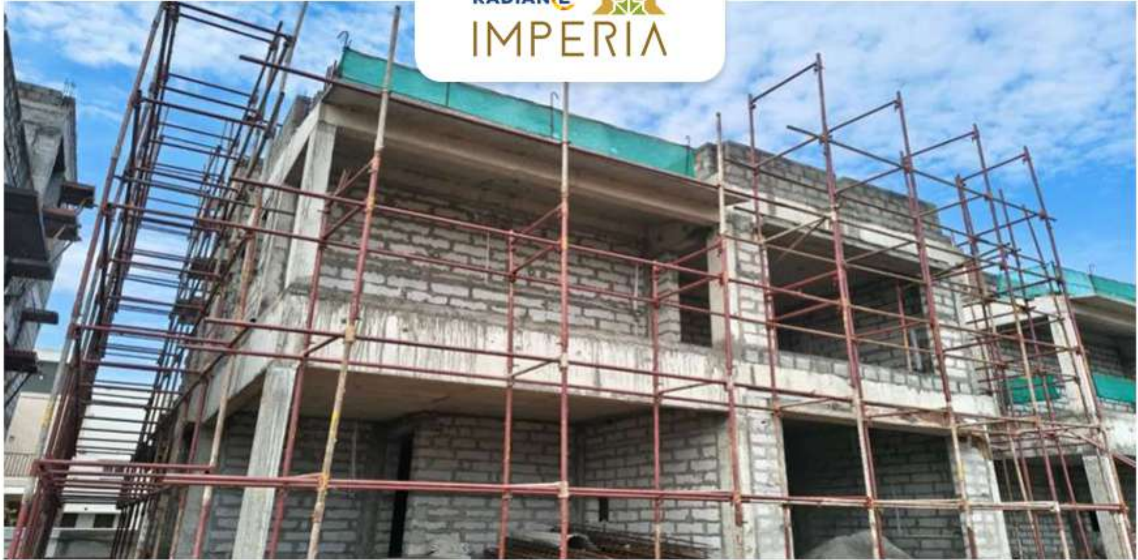
Villa no 7 External Plastering Work in Progress.
