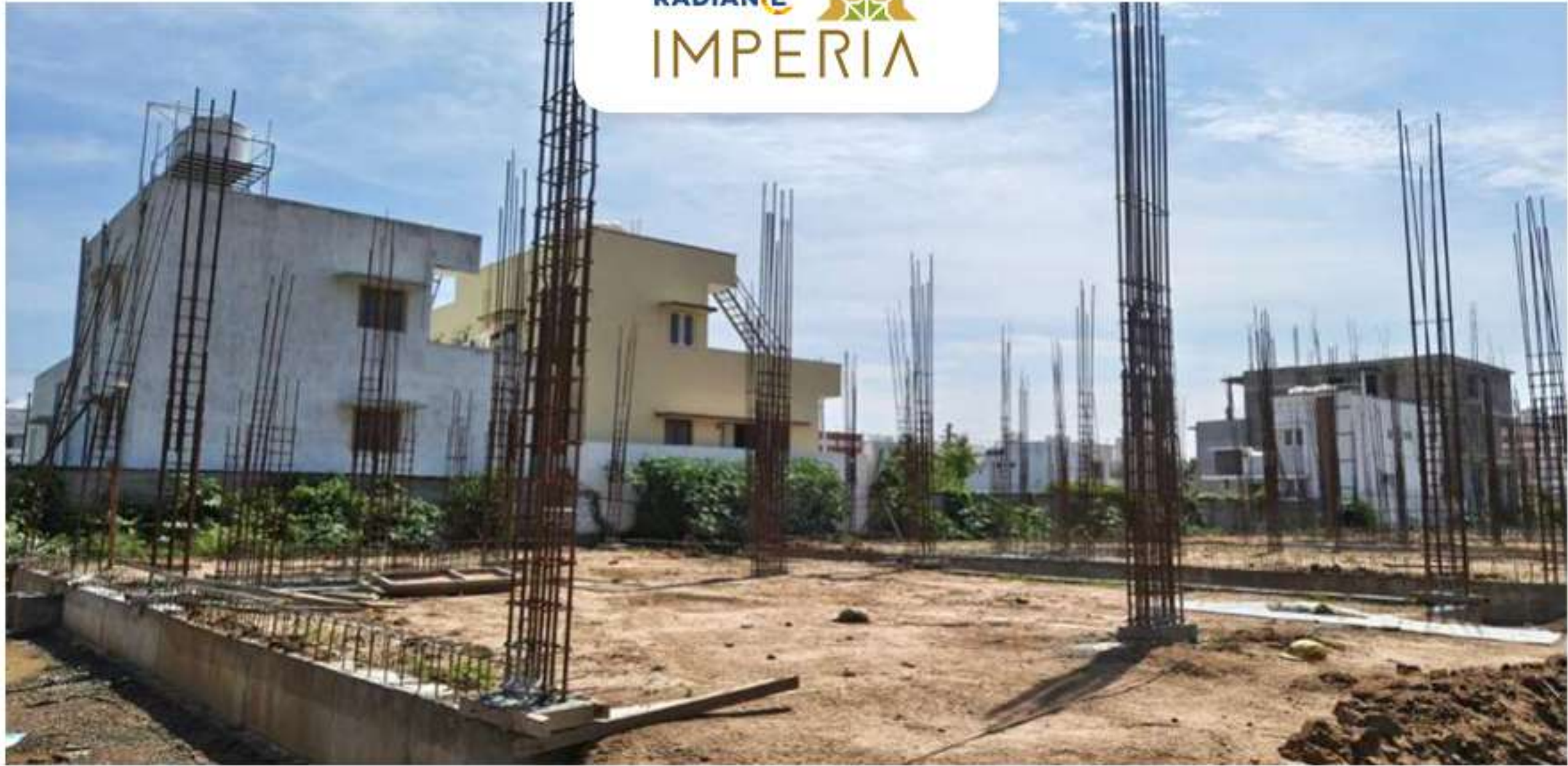
Villa no -57 Ground Floor Column Work in Progress
