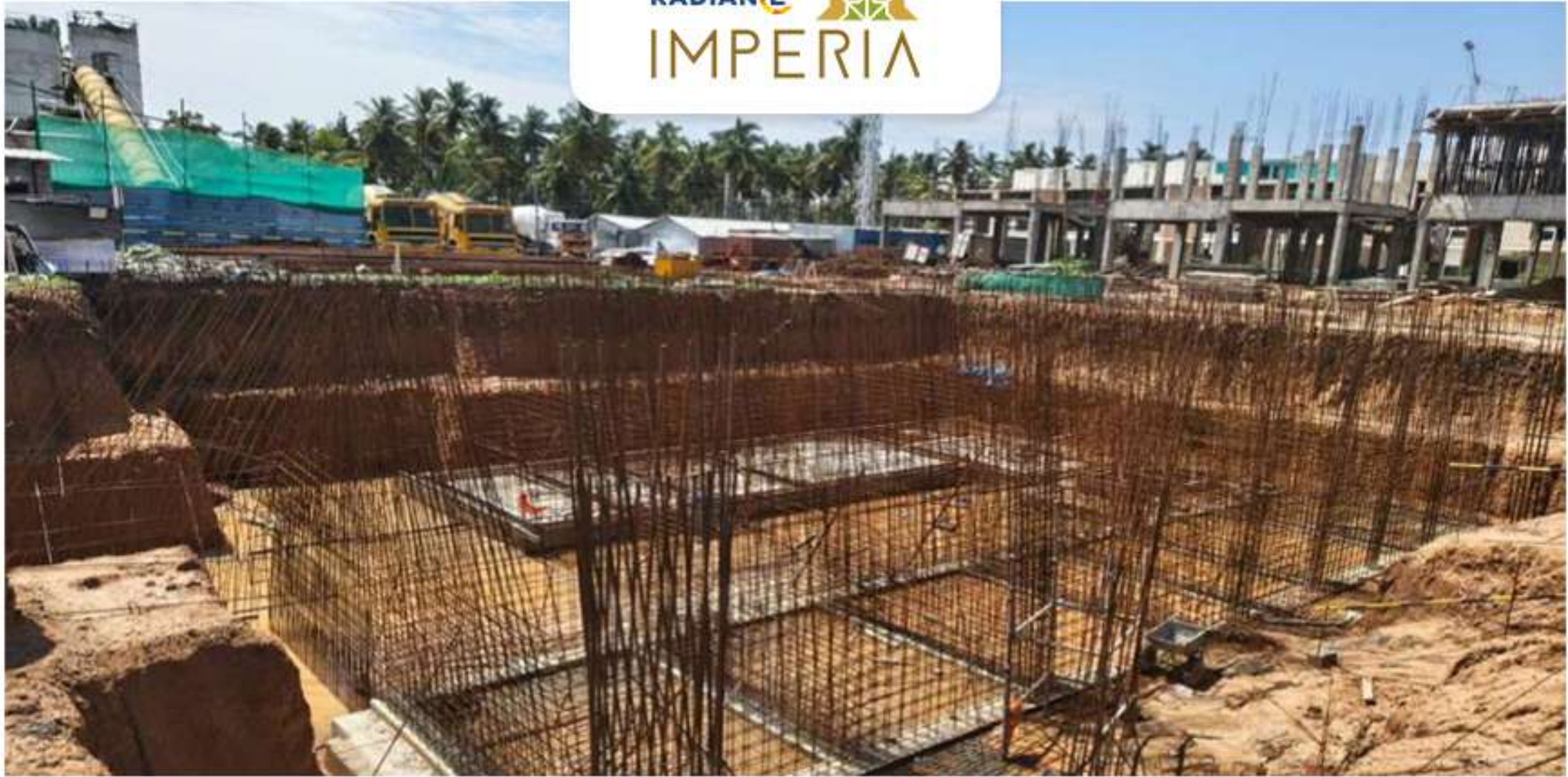
STP & WTP-Reinforcement Work in Progress
