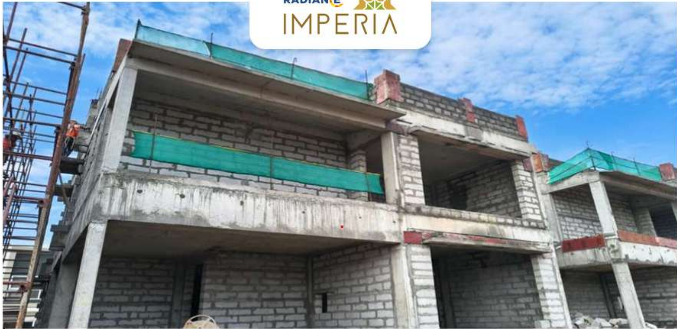
Villa no 9 Block Work in progress.
