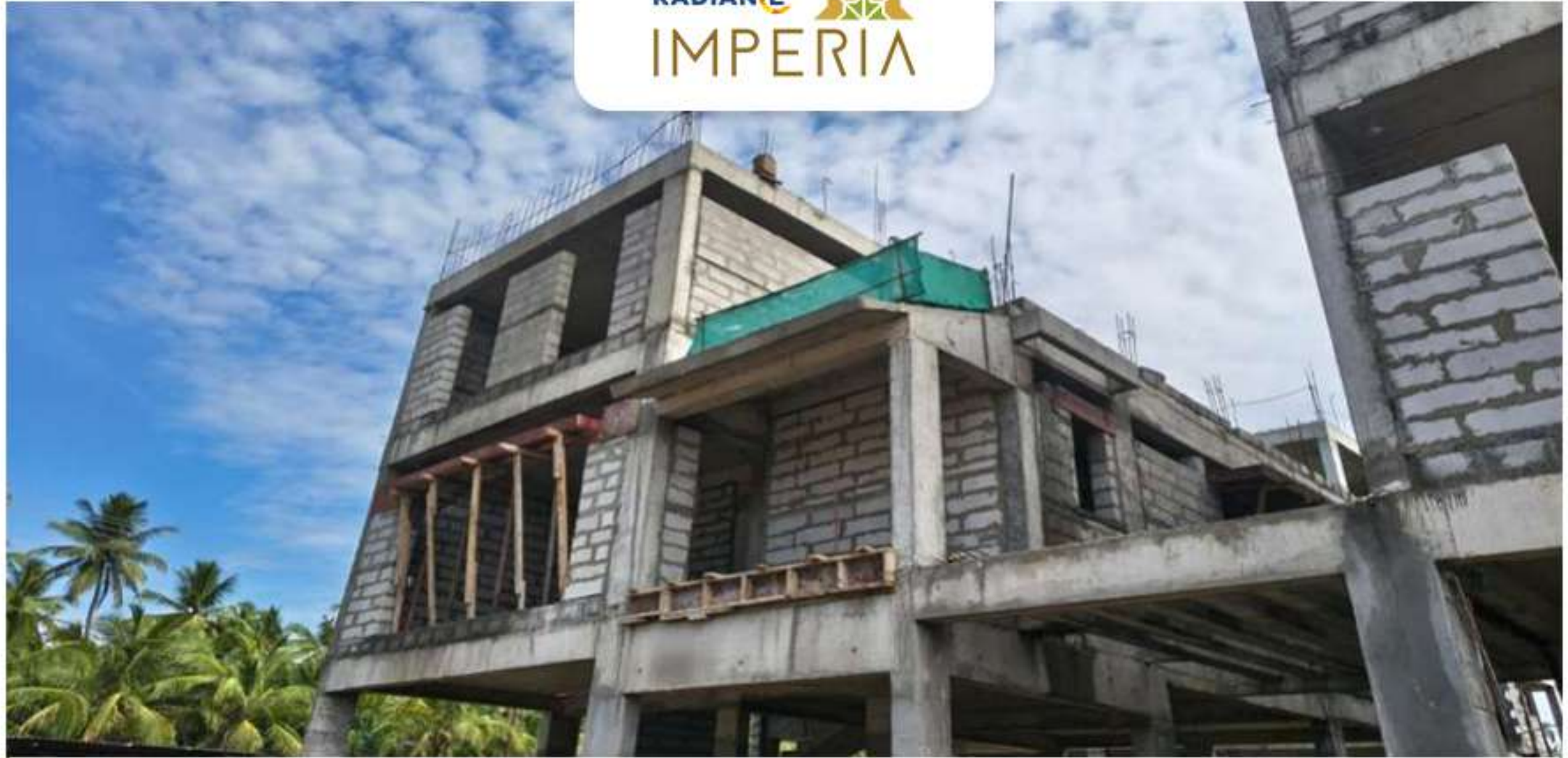
Villa no -45 block Work in progress
