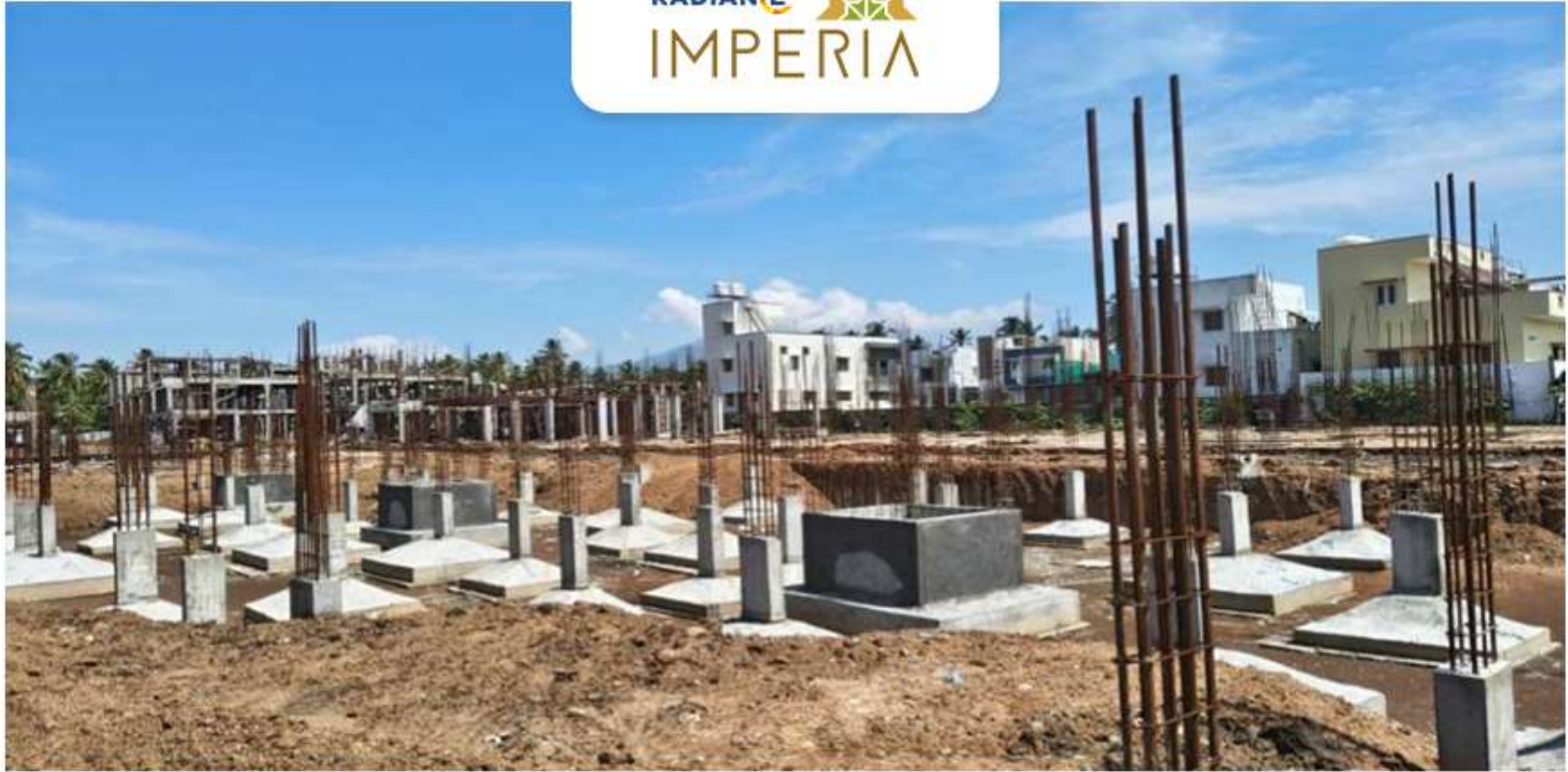
Villa no-29 to 31 Footing Level Back filling Work in Progress
