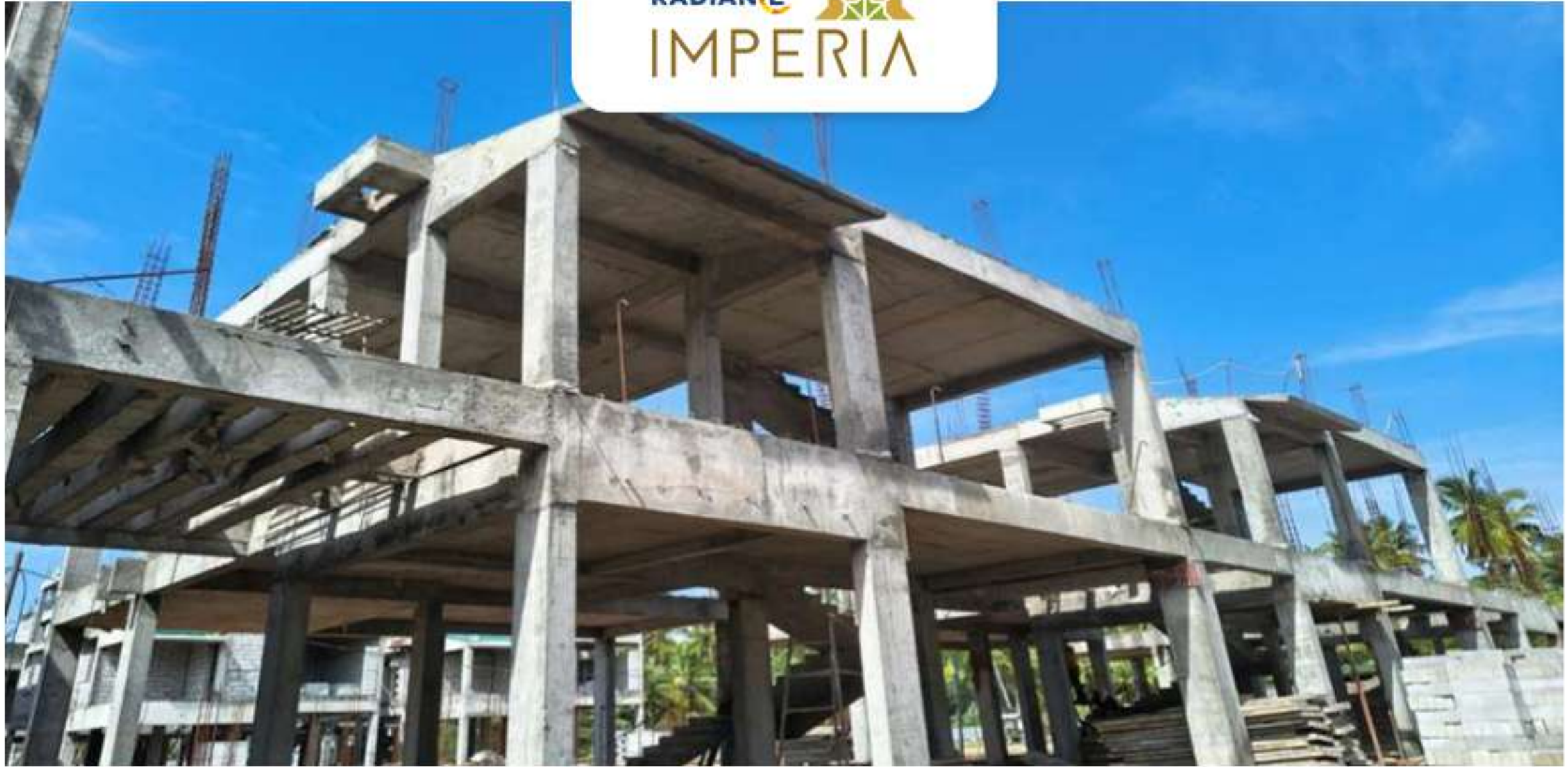
Villa no – 84 First Floor Roof Slab Completed
