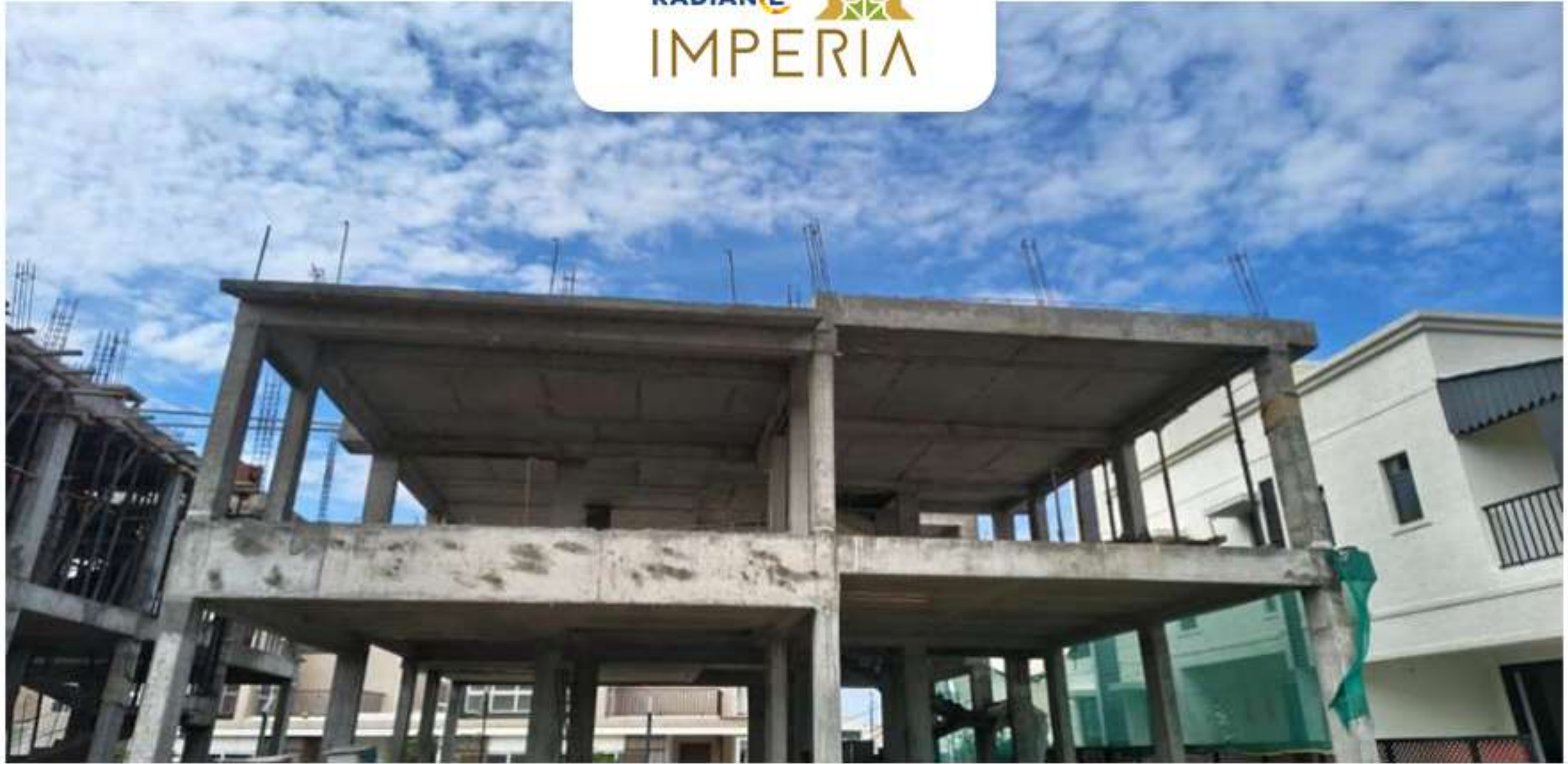
Villa no.4-1st Floor Roof Slab Completed
