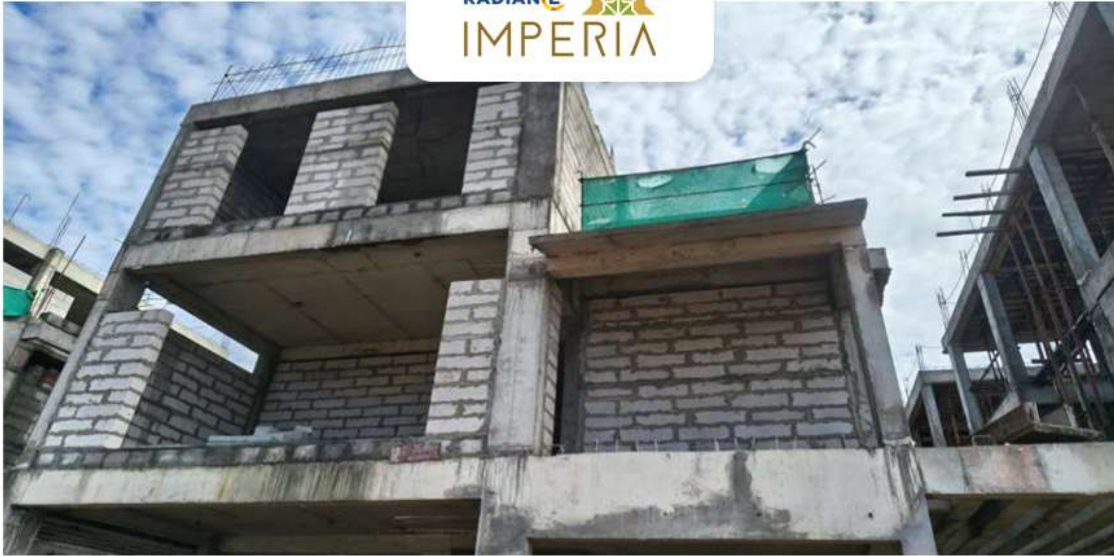
Villa no -46 block Work in progress
