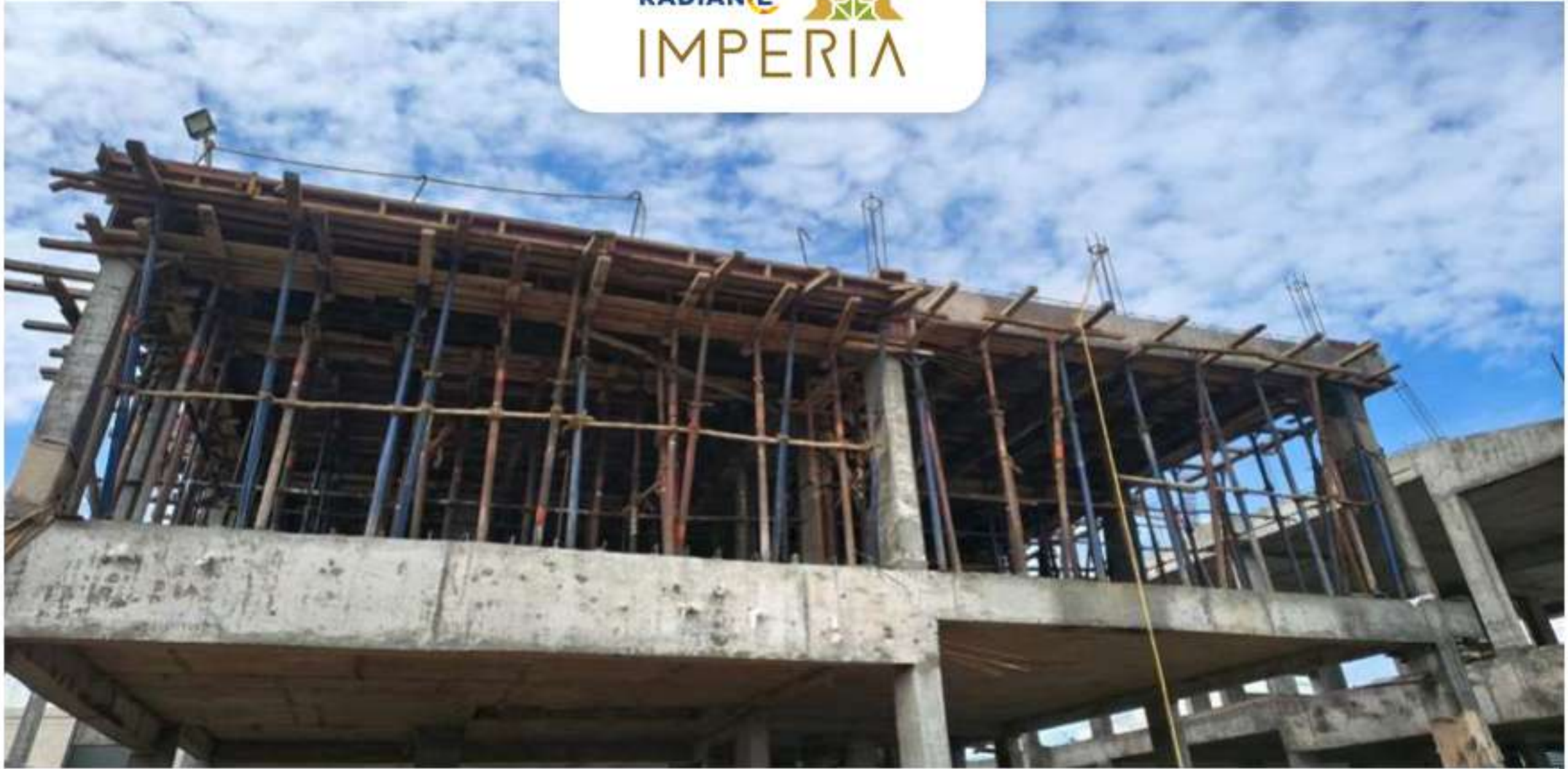
Villa no. 3 1st floor Roof Slab Completed
