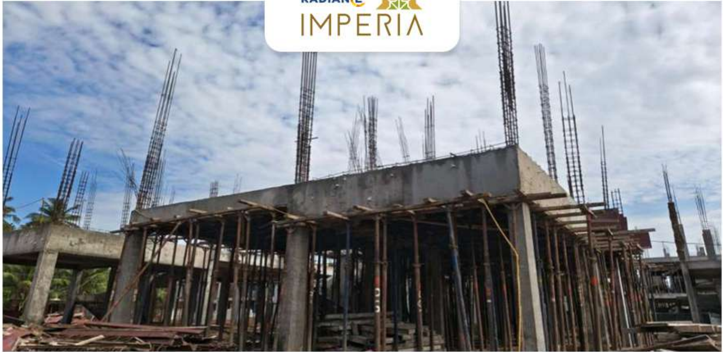
Villa no -22 Ground Floor Roof Slab Completed
