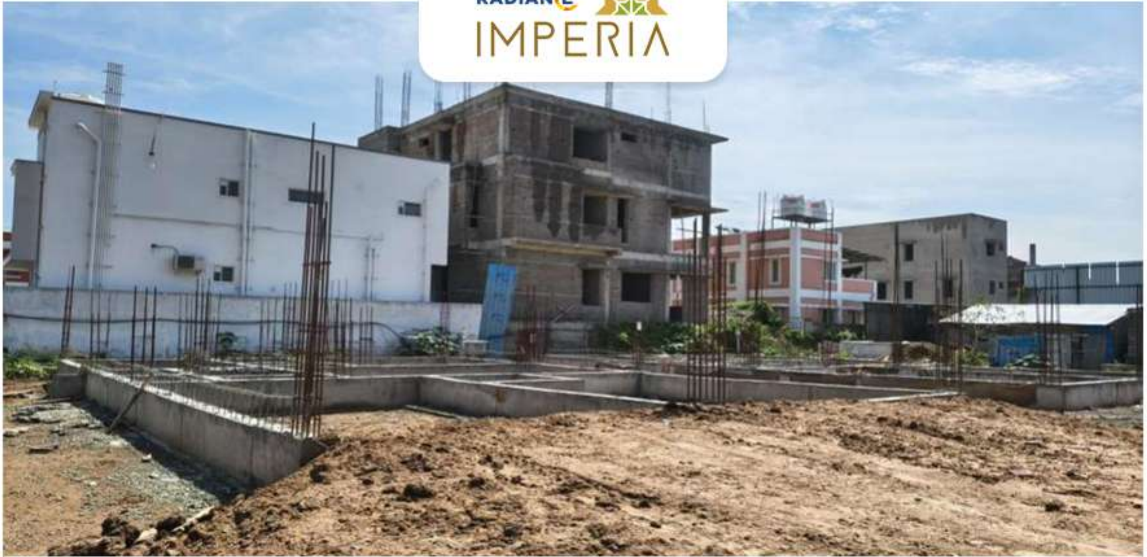
Villa no 63 Plinth Beam Completed
