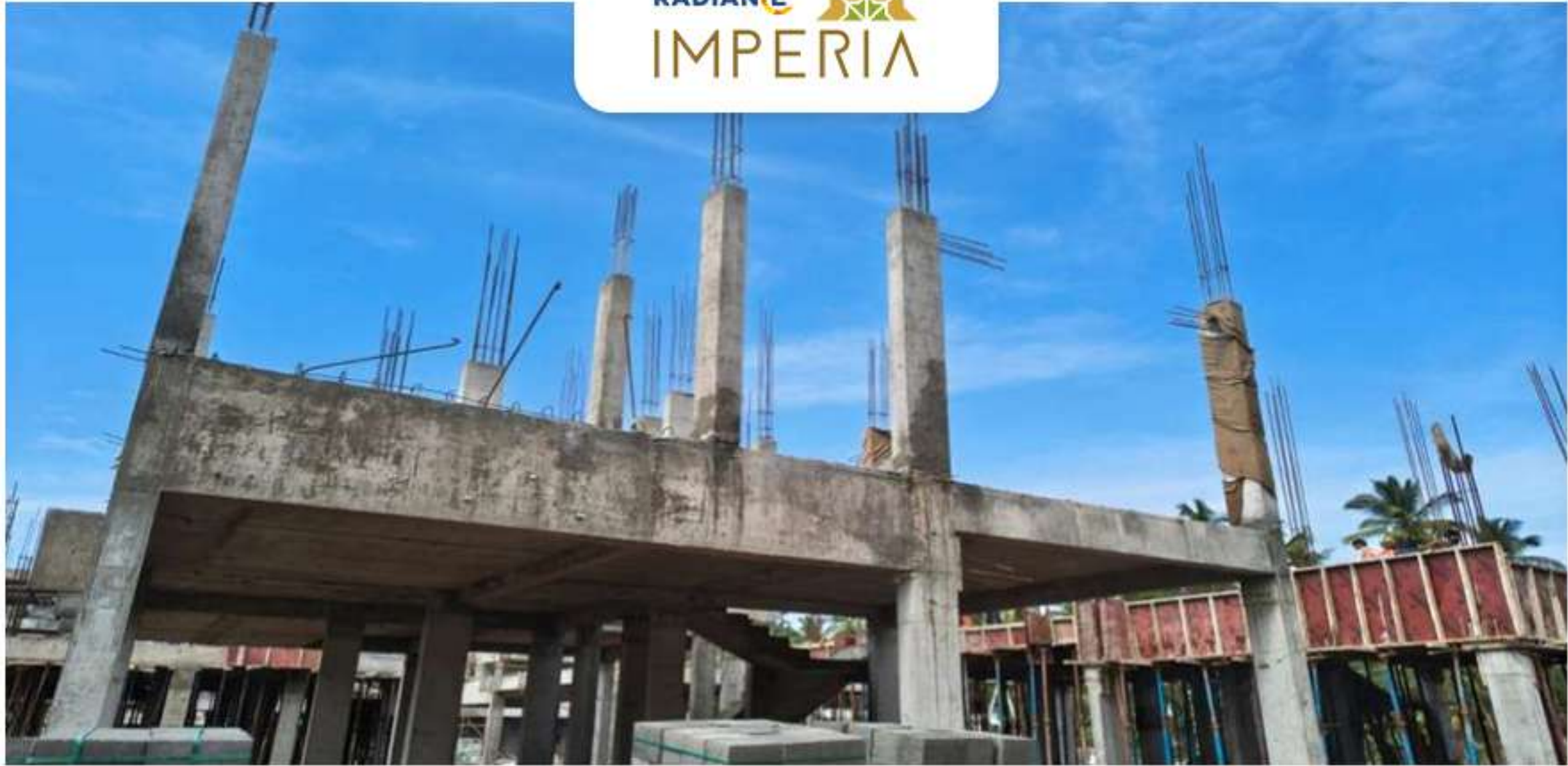
Villa no -40 First floor Column Completed
