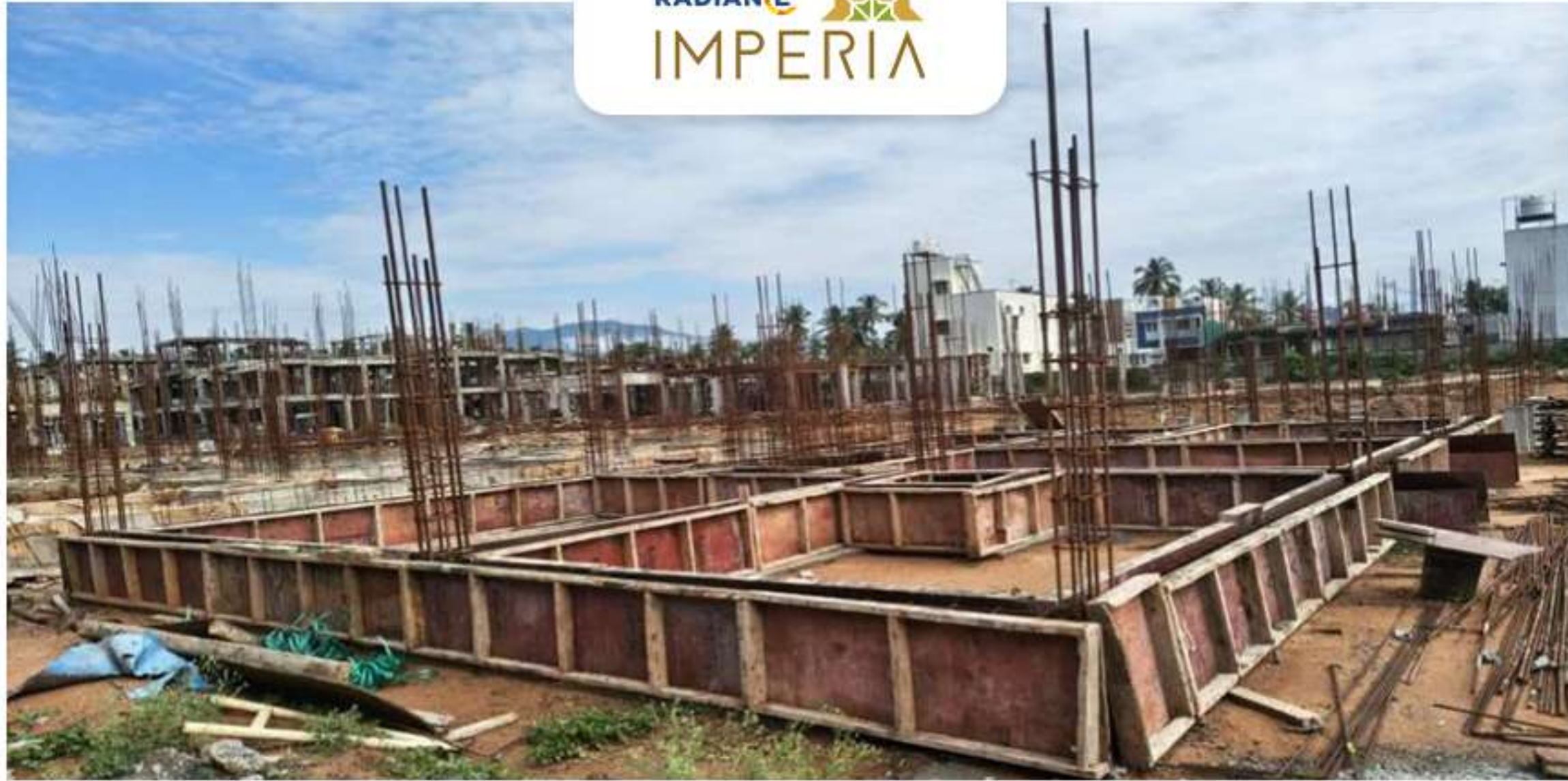
Villa no -29 Plinth Beam Shuttering Work in Progress
