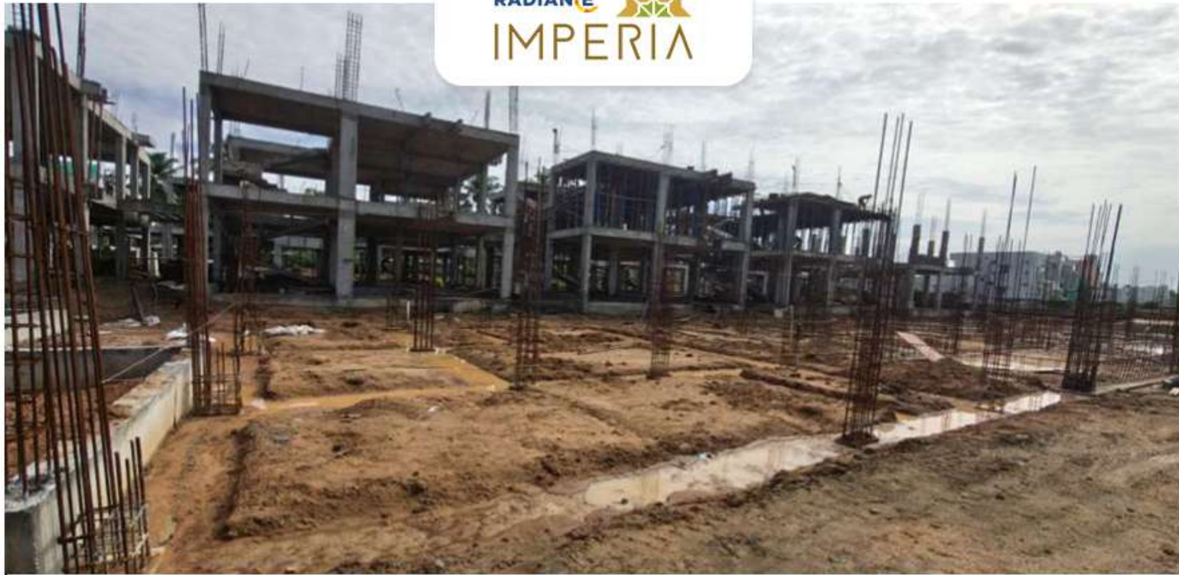
Villa no -75 Plinth beam soil sectioning Work in progress
