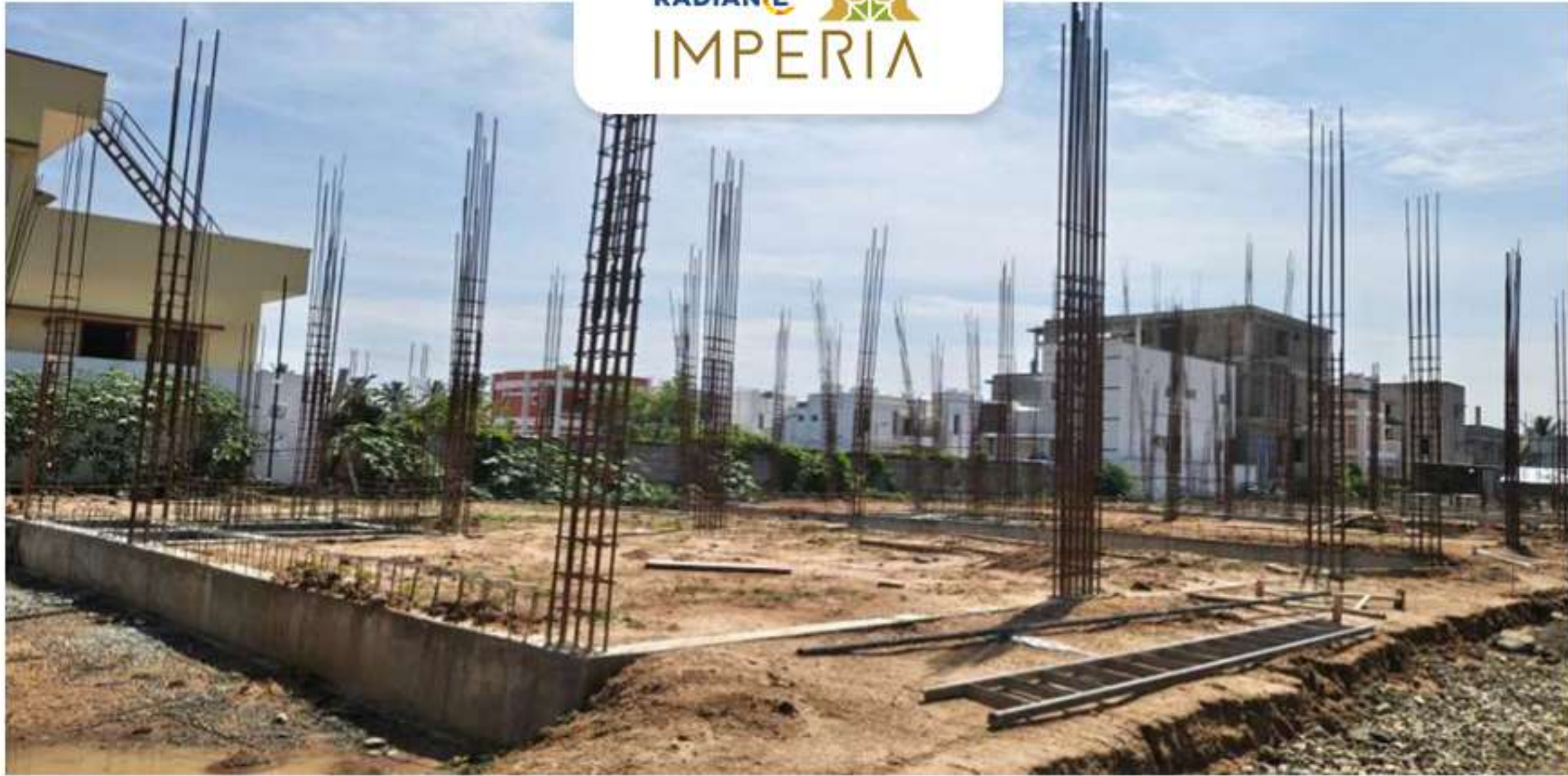
Villa no -59 Ground Floor Column Work in Progress
