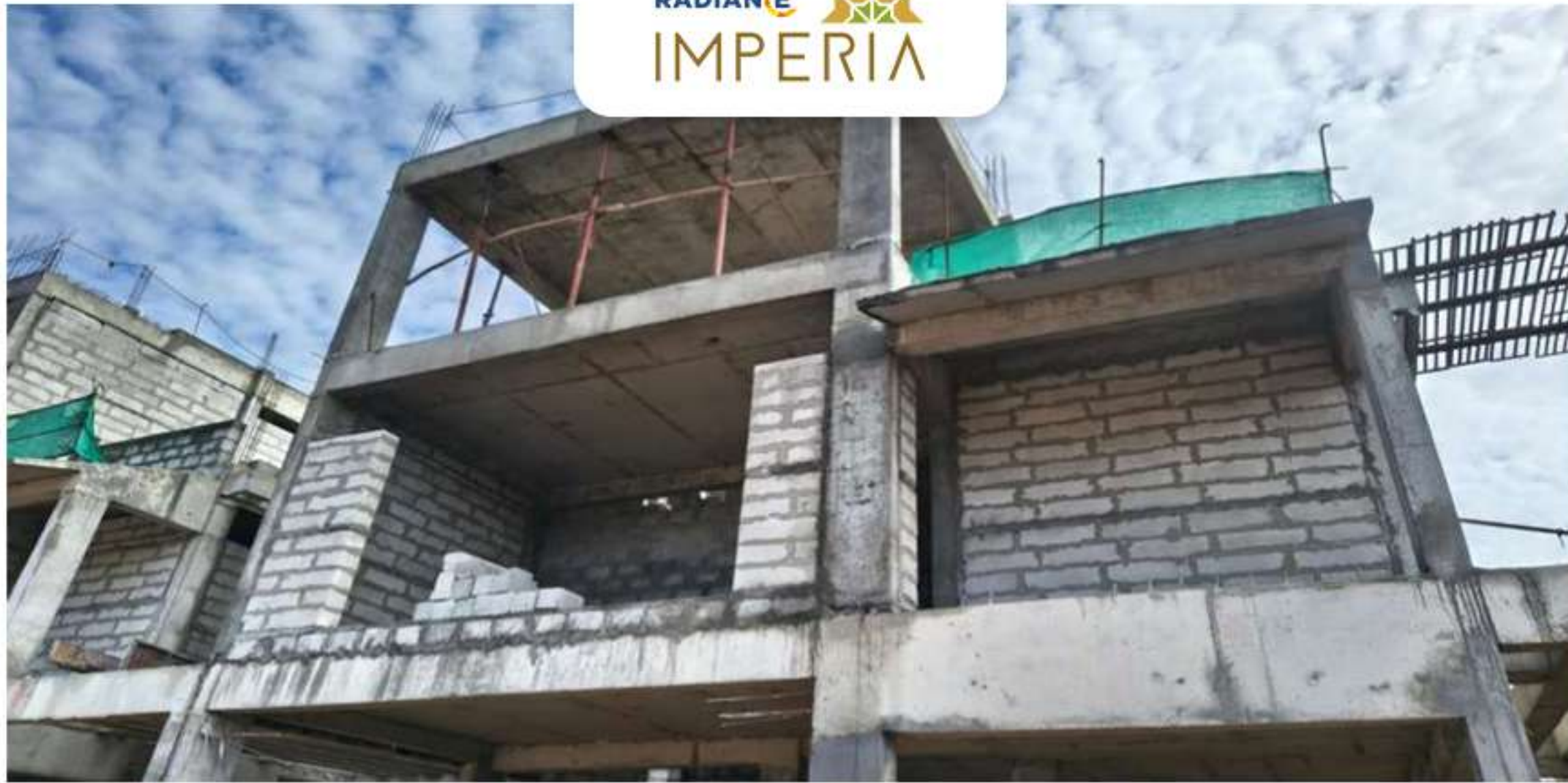
Villa no -47 Block Work in progress
