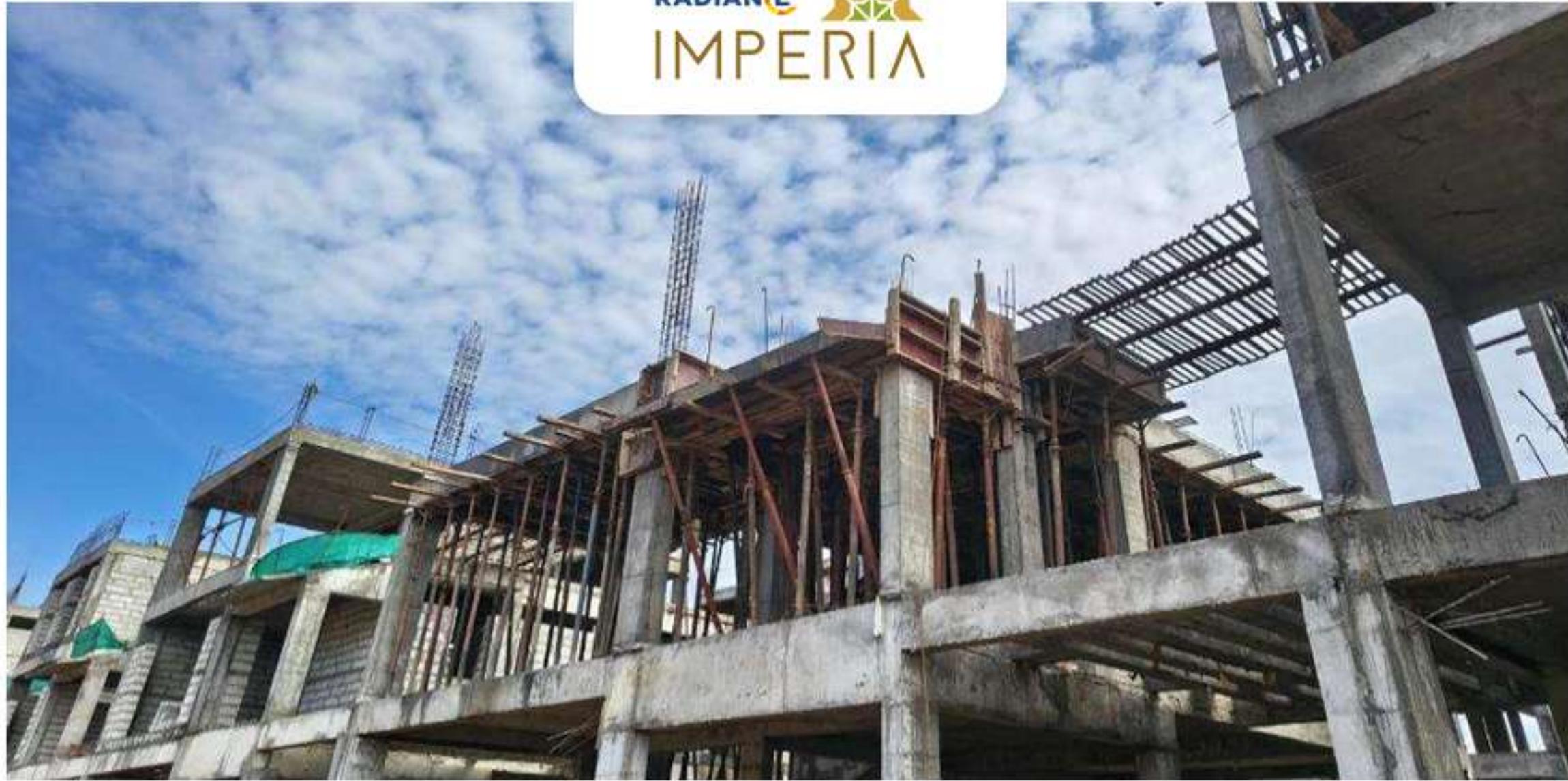
Villa no -48 2nd Floor Column Work in progress
