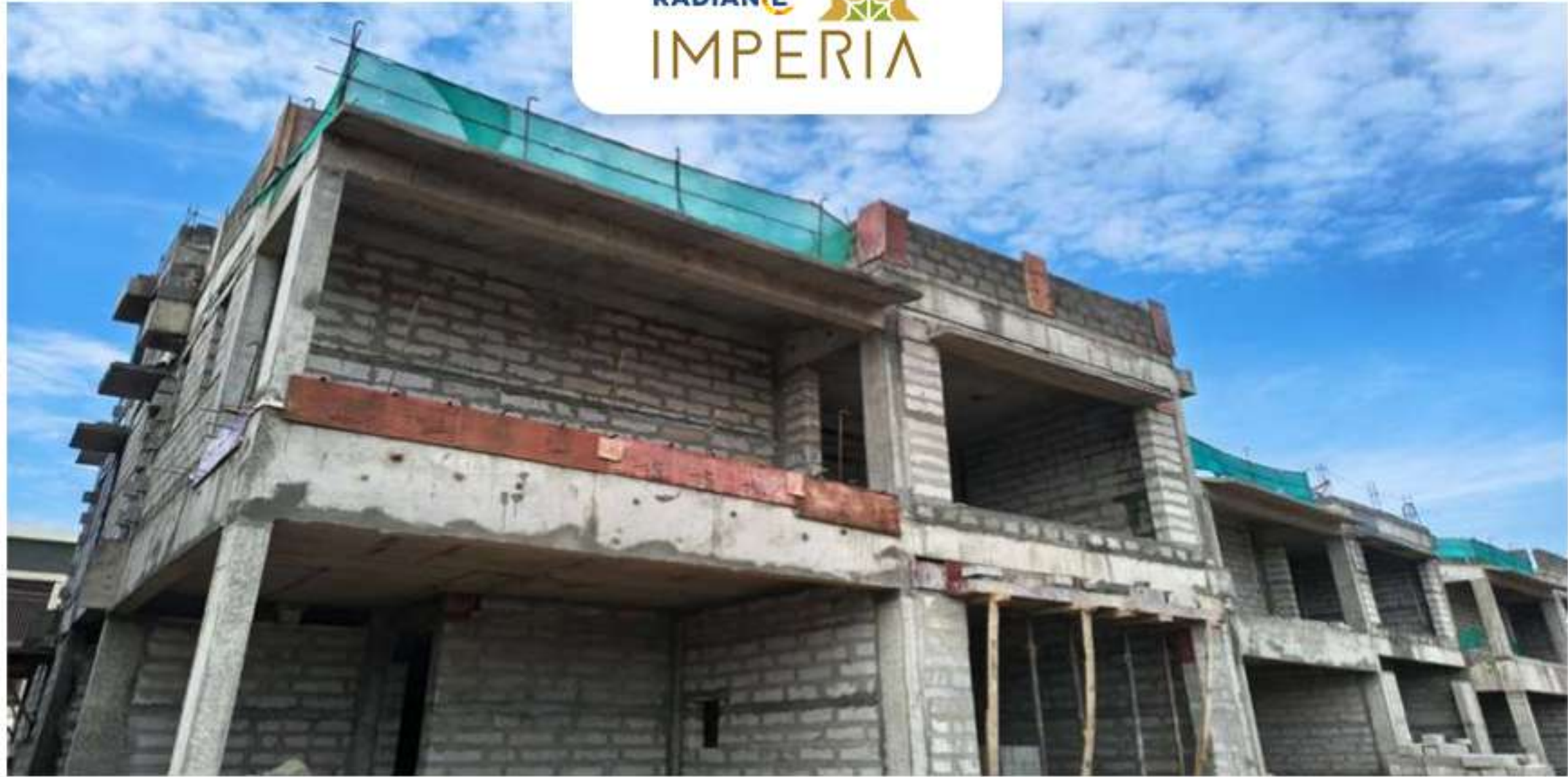
Villa no -10 Block Work in progress
