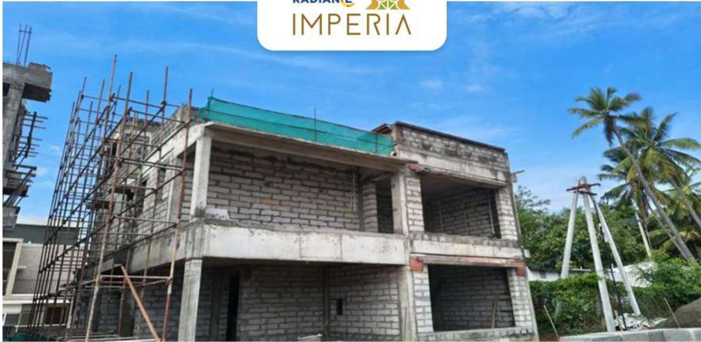
Villa no -18 Block Work Completed
