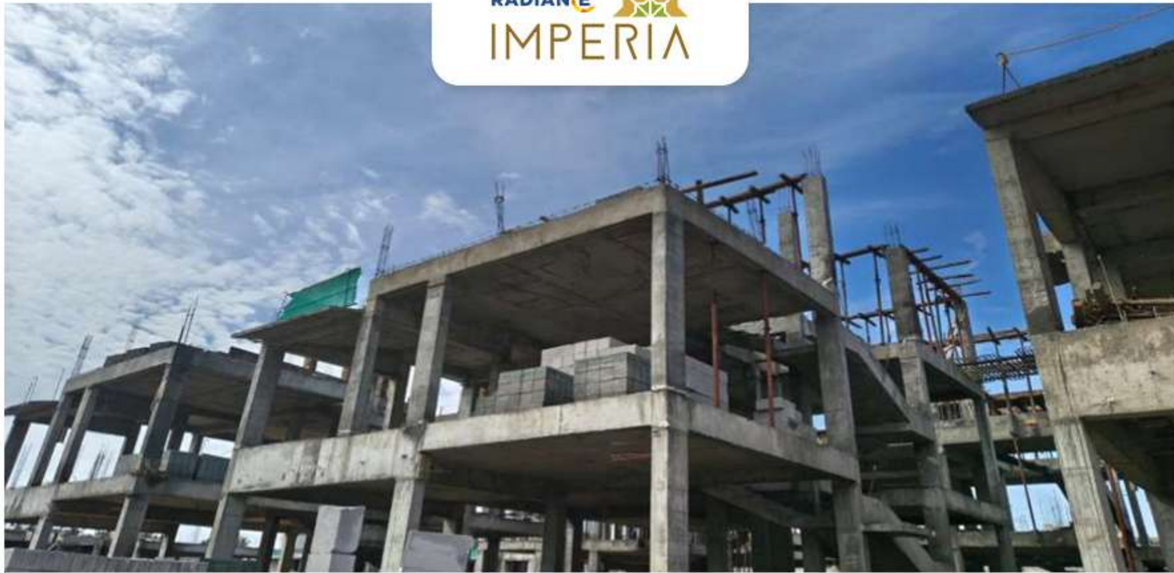
Villa no -66 2nd Floor Roof Slab Work in progress
