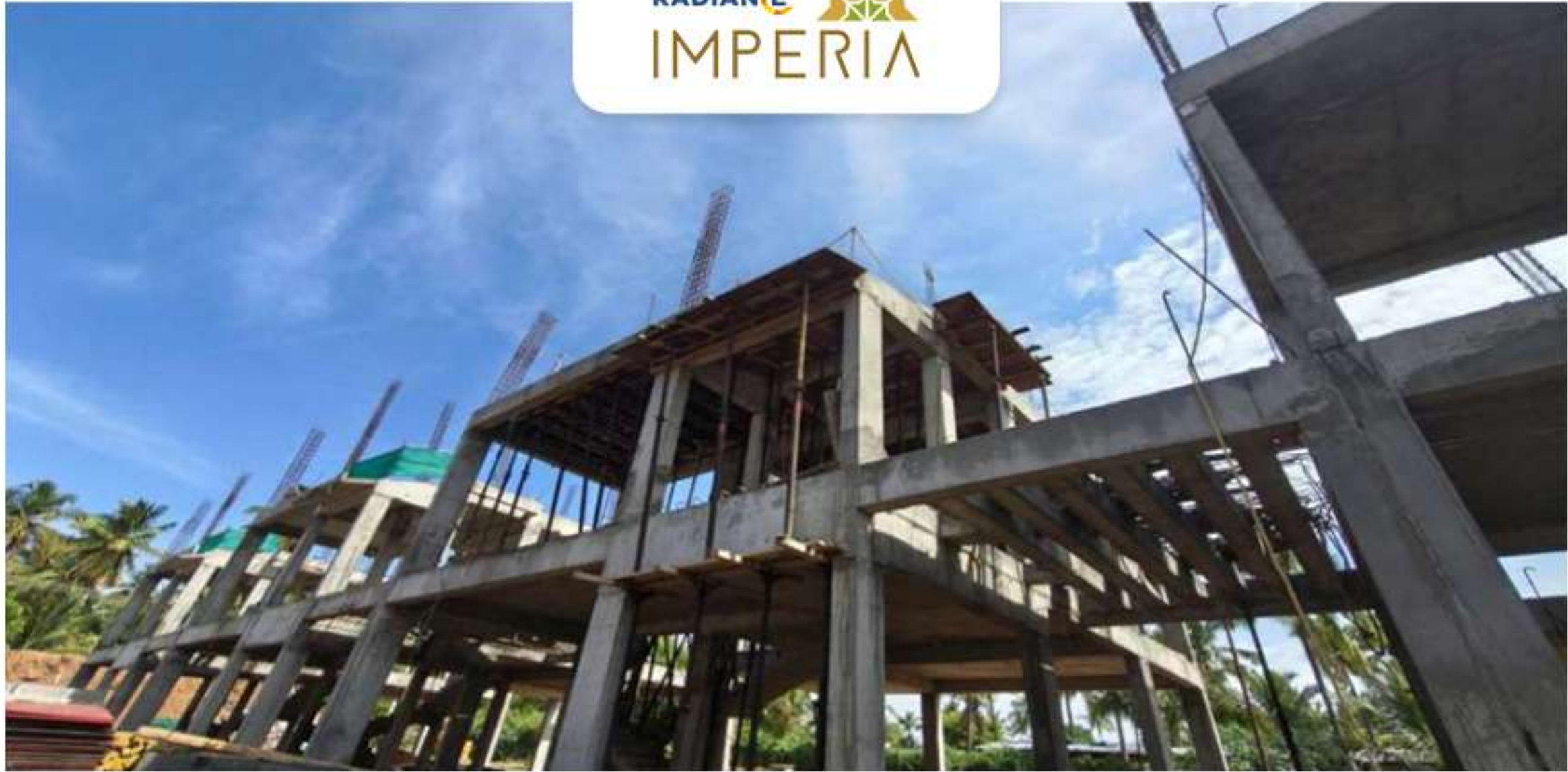
Villa no – 91 First Floor Roof Slab Completed
