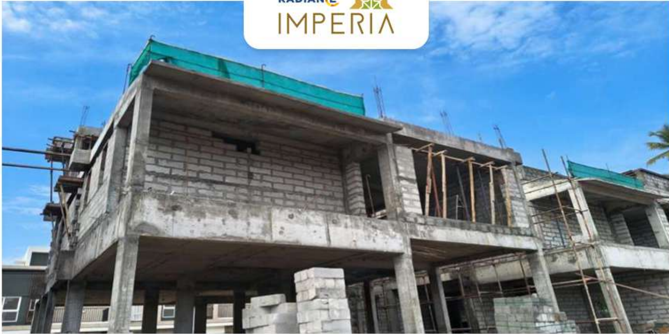
Villa no -16 Block Work in progress
