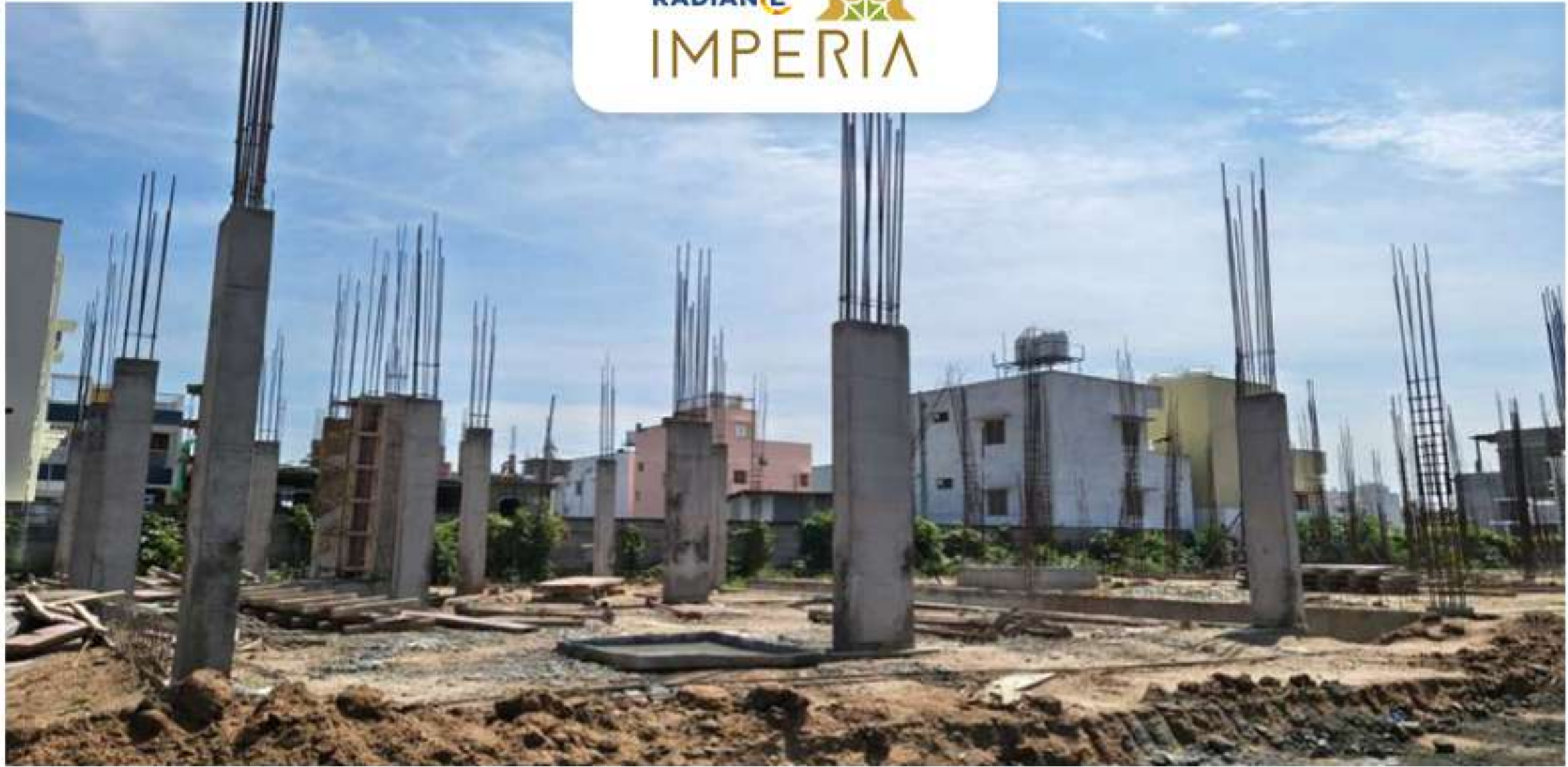
Villa no -55 Ground Floor Column Completed
