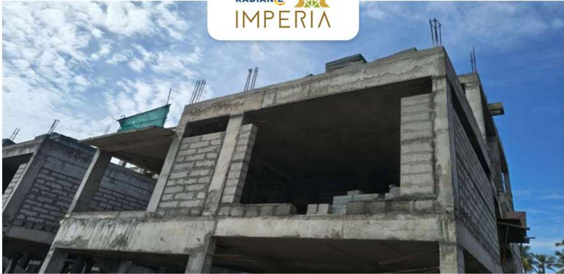
Villa no -72 block Work in progress
