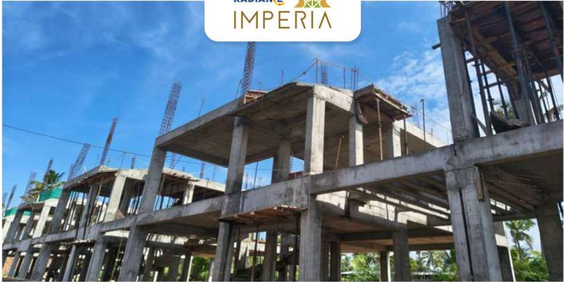
Villa no – 93 First Floor Roof Slab Completed
