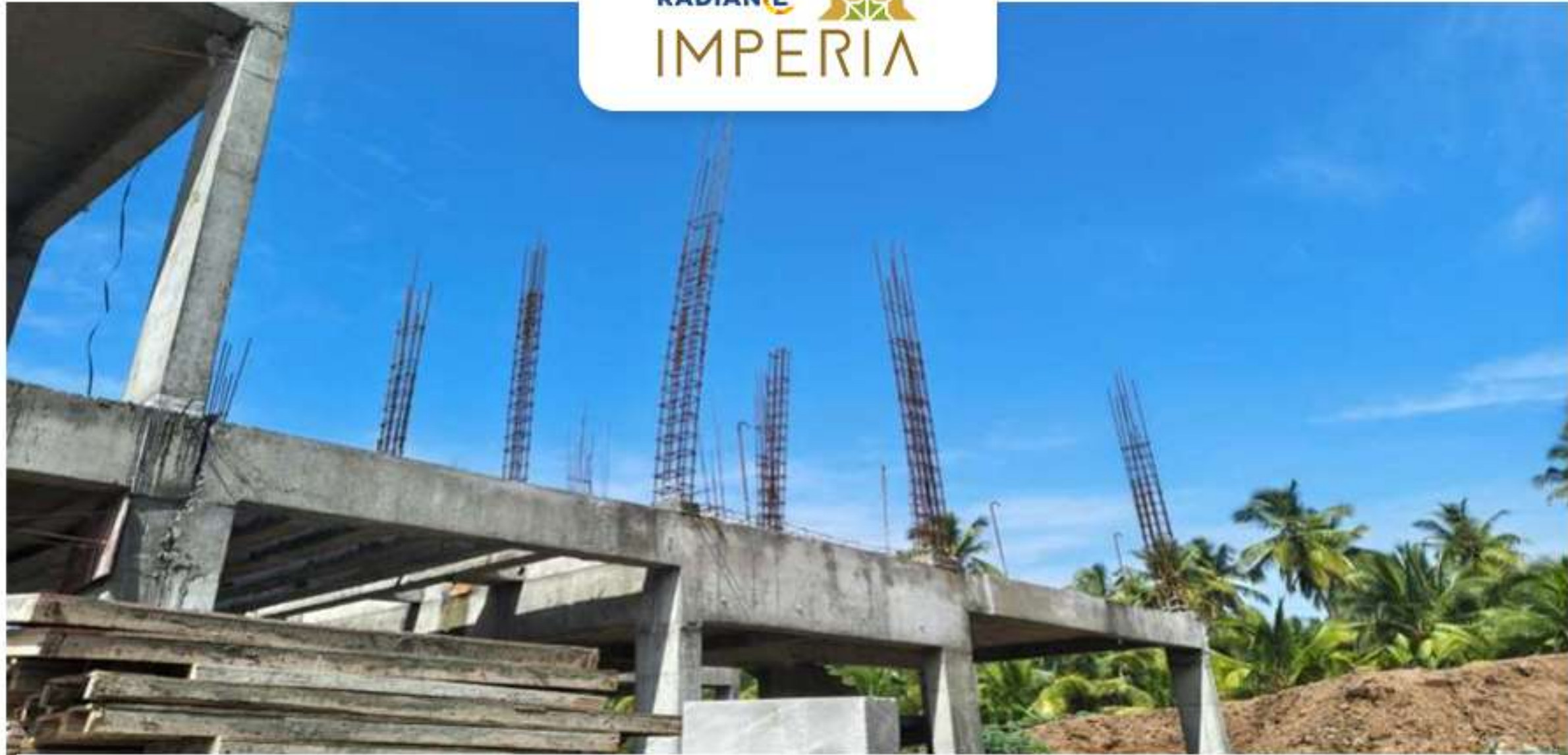
Villa no - 87 Ground Floor Roof Slab Completed
