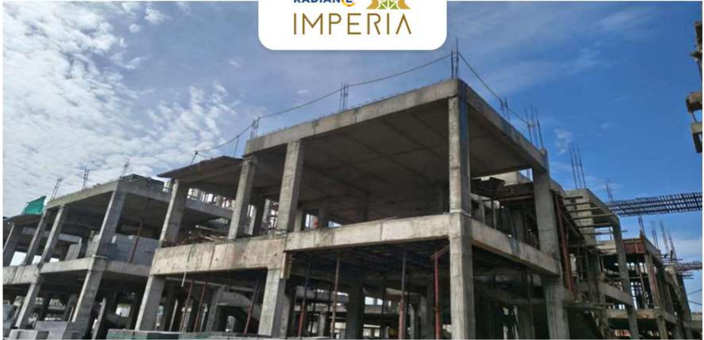
Villa no -68 2nd Floor Column work in progress.
