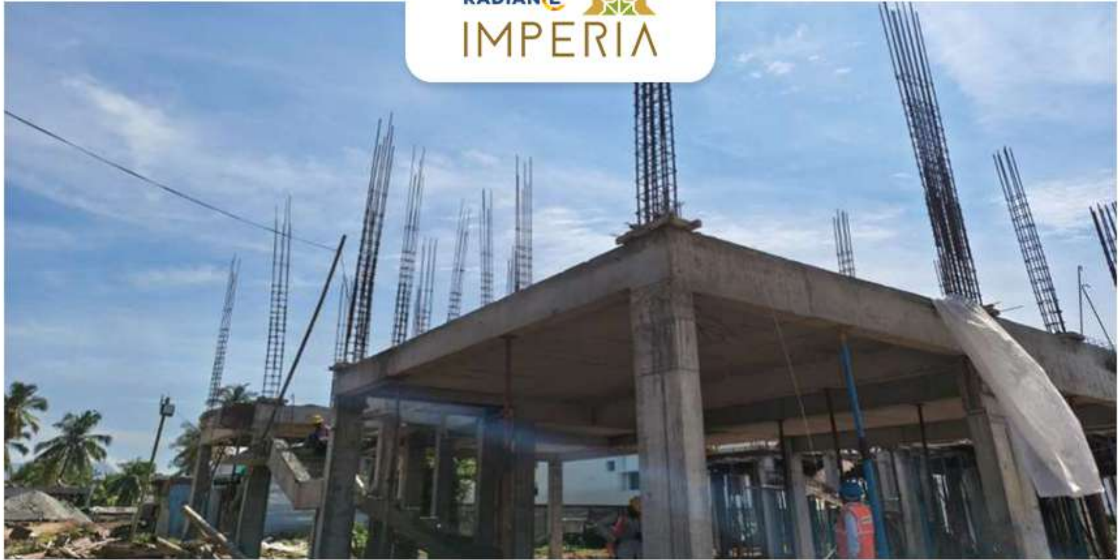
Villa no – 52 First Floor Roof Column Work in Progress
