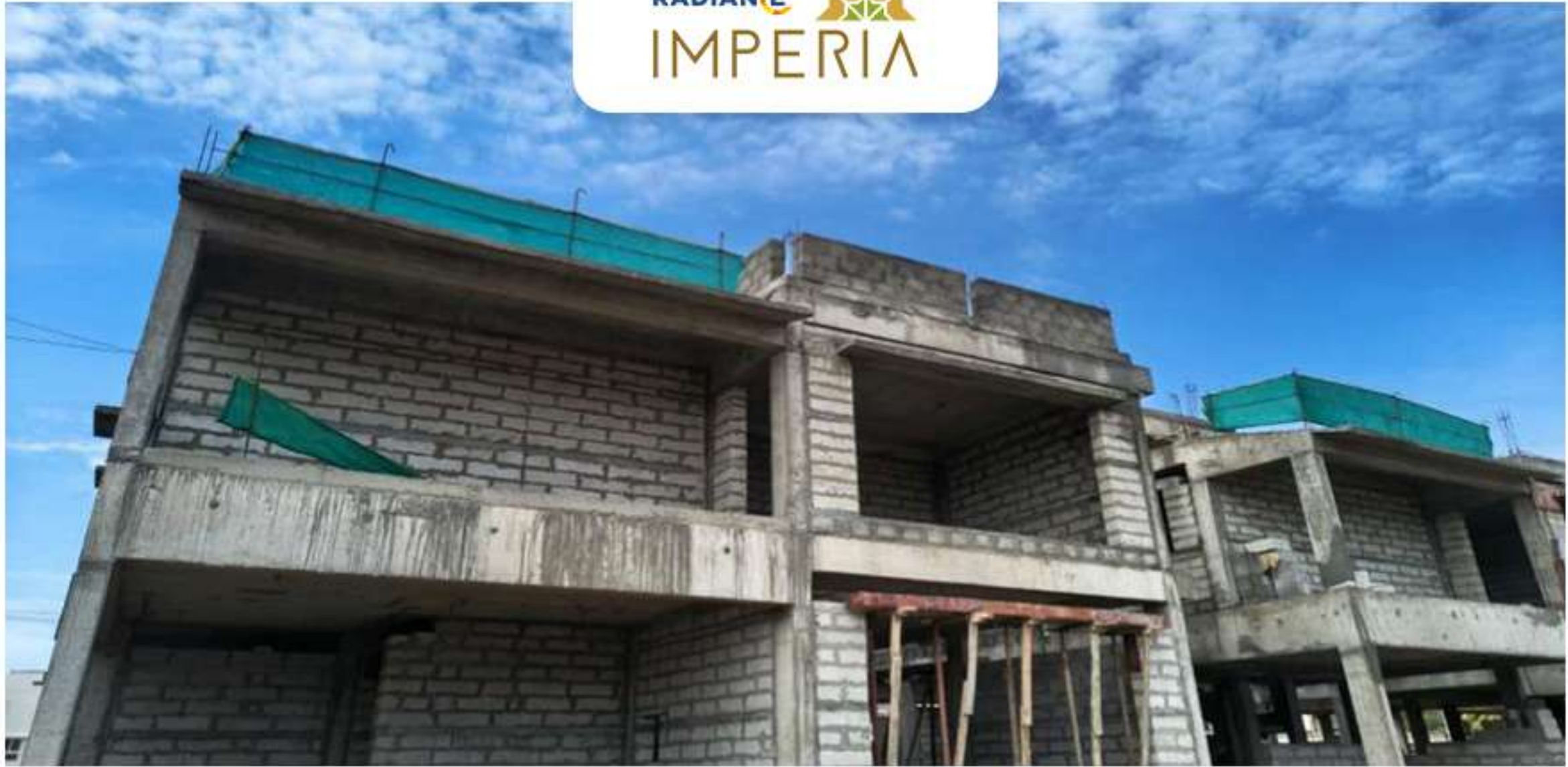
Villa no -12 Block Work in progress
