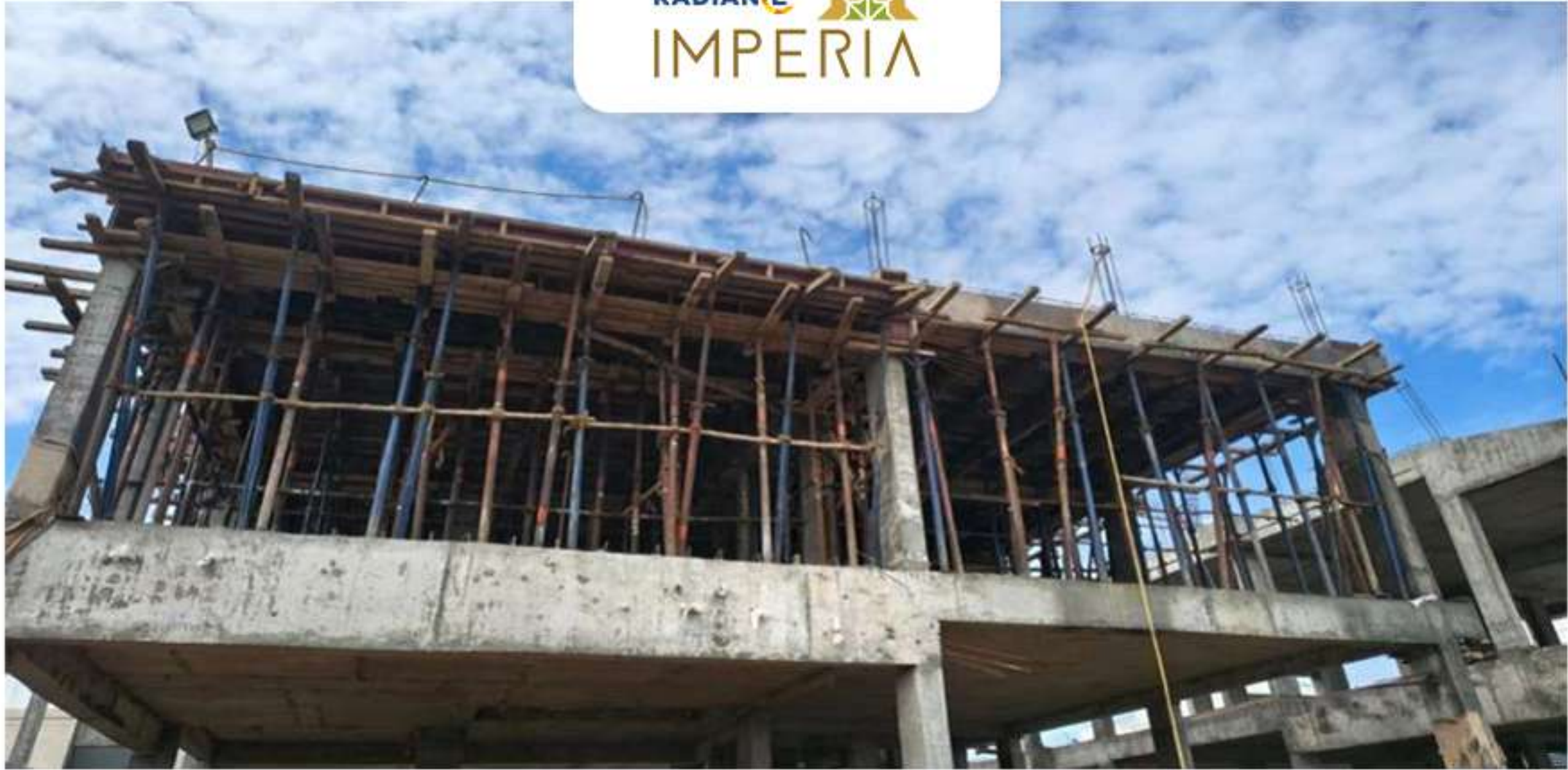
Villa no. 2 1st Floor Roof Slab Work in Progress
