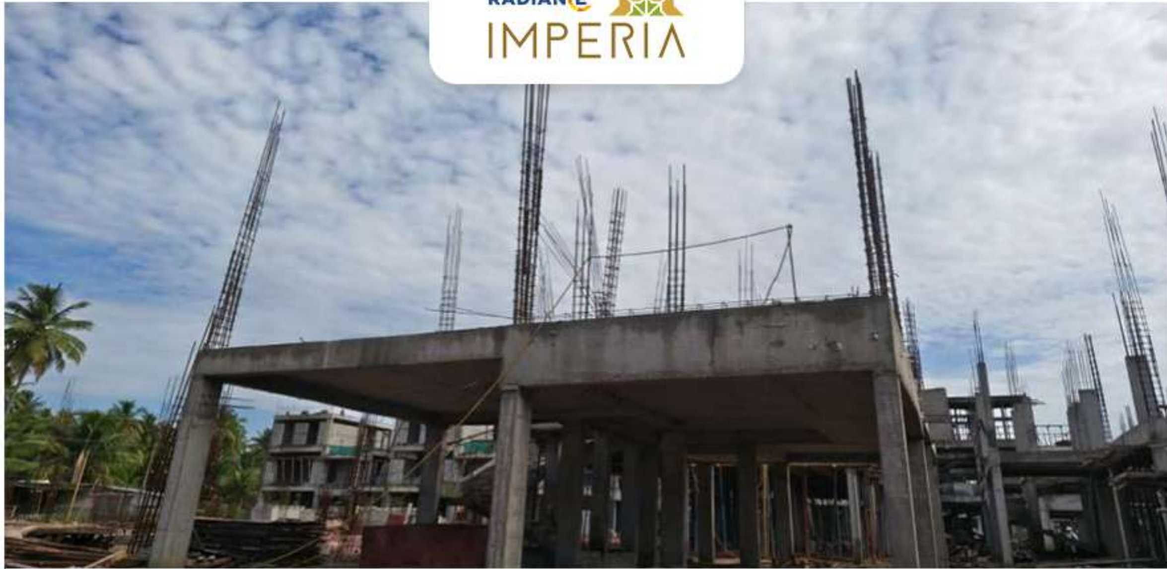
Villa no -21 1st Floor Column Work in Progress
