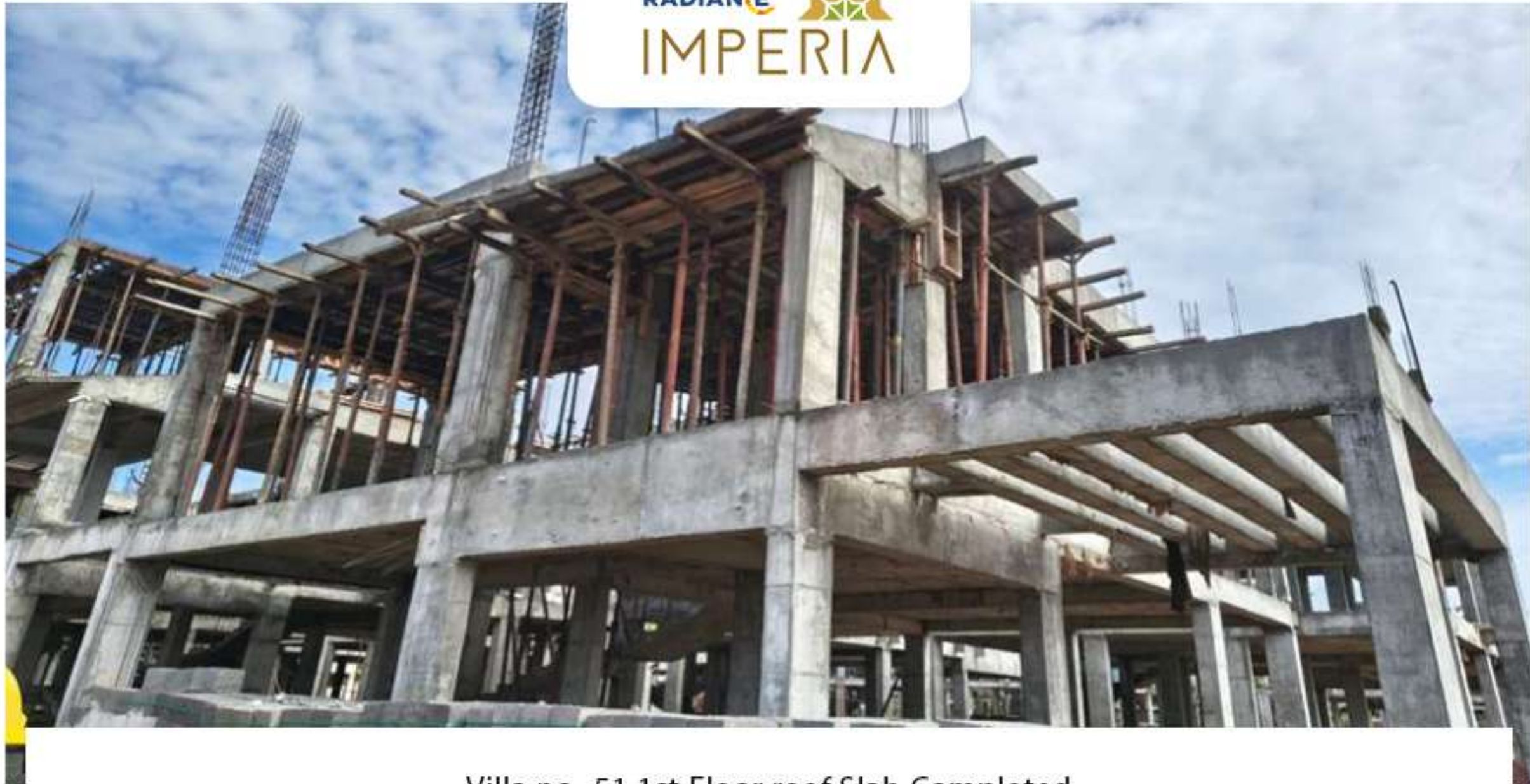
Villa no -51 1st Floor roof Slab Completed
