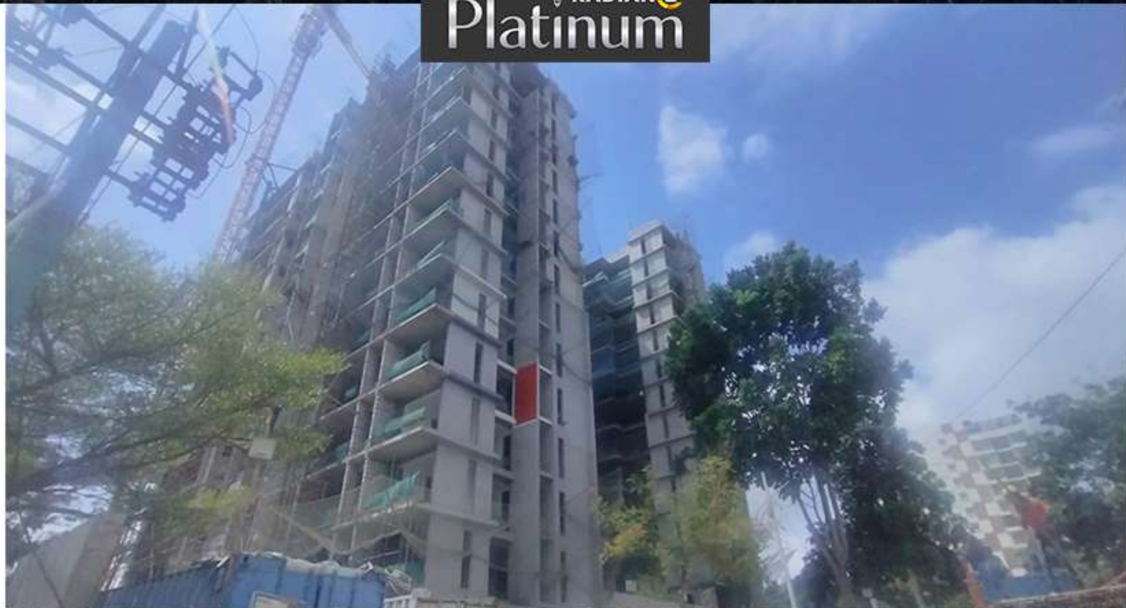
North West View
