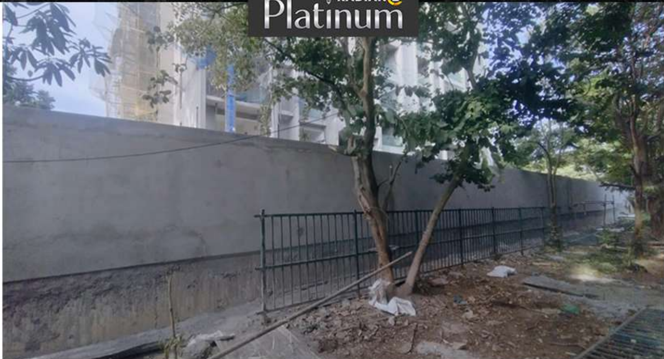
Compound Wall - South side Outside Plastering
