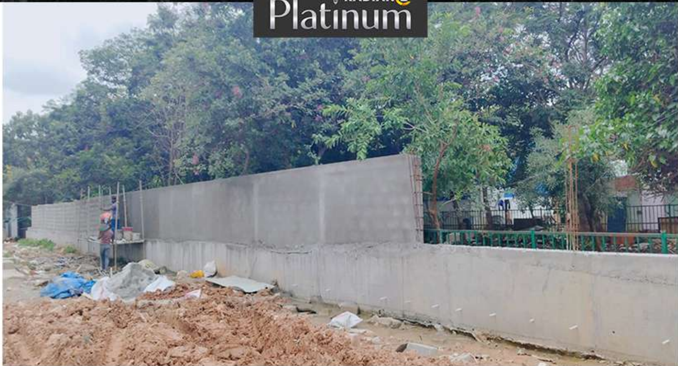
Compound Wall - South side
