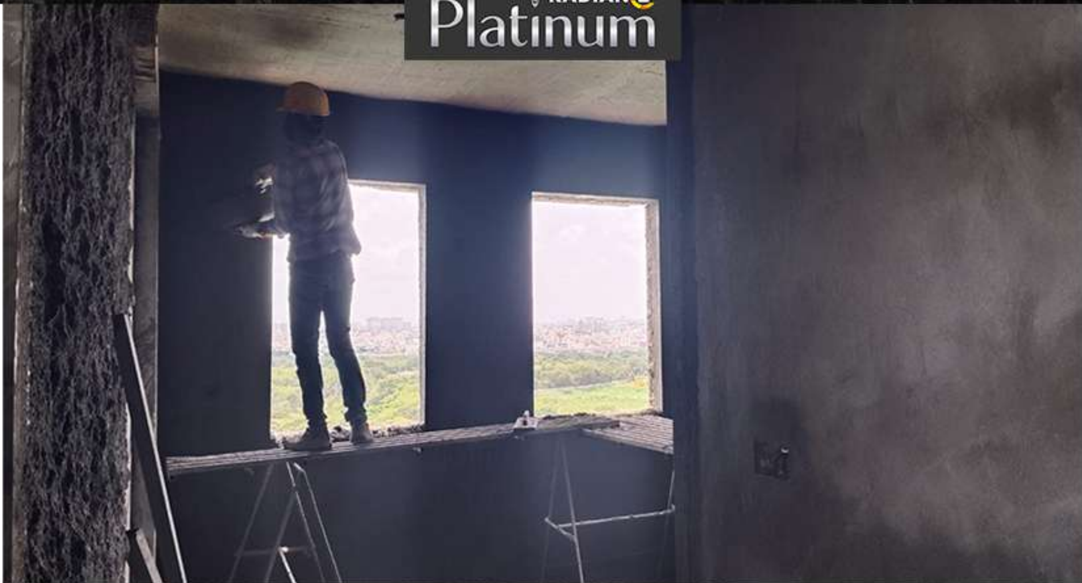
12th Floor Internal wall plastering work
