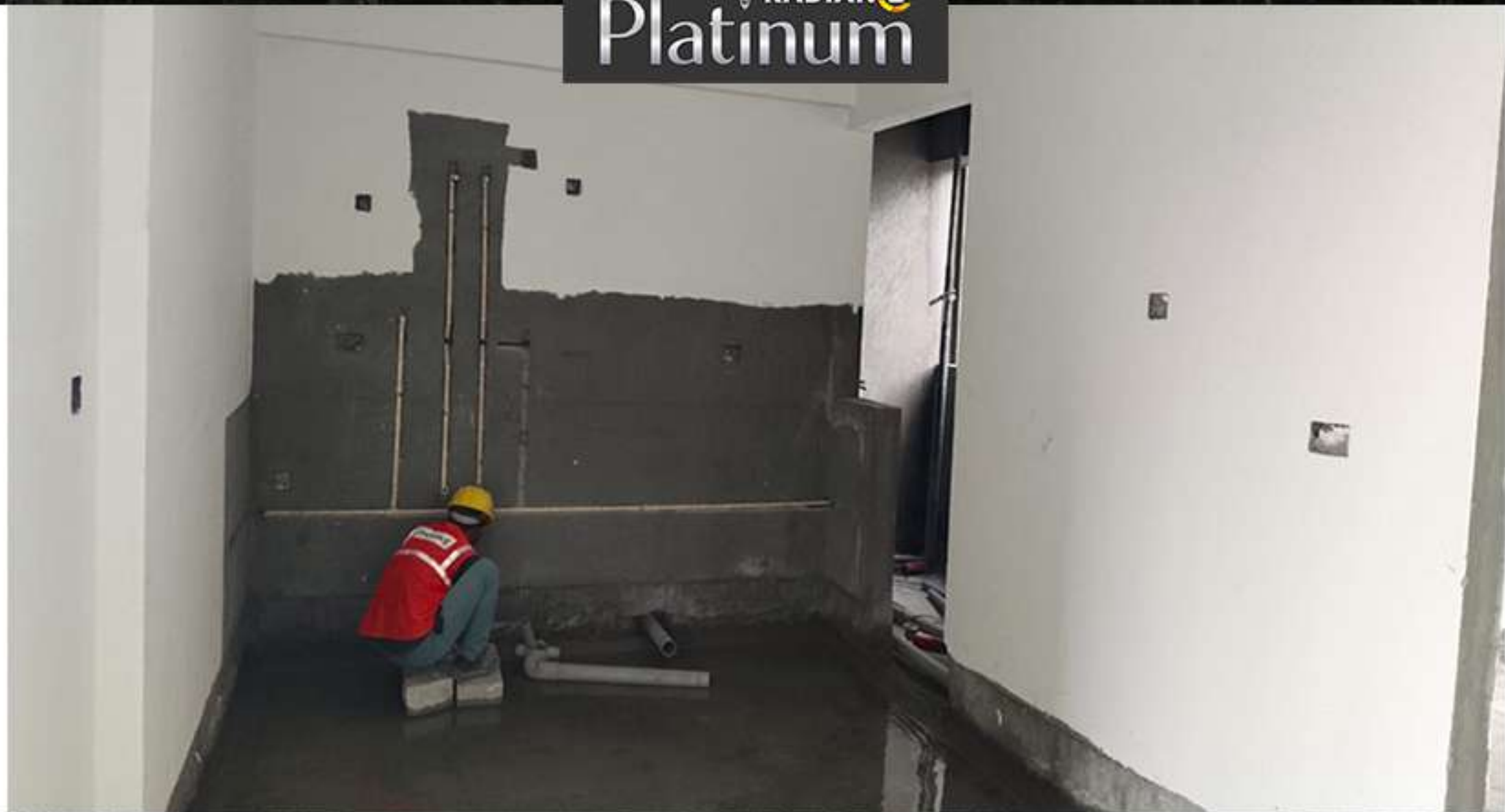
B – Block – Plumbing work
