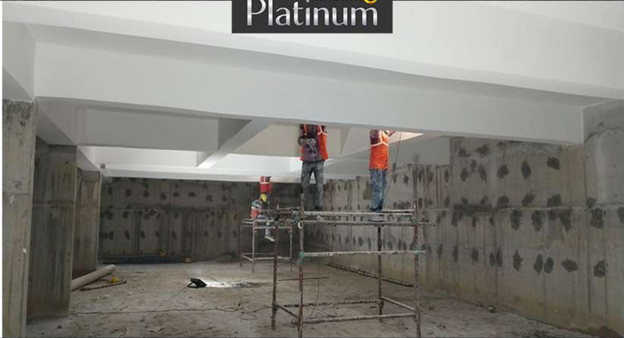
Basement Ceiling Putty Work
