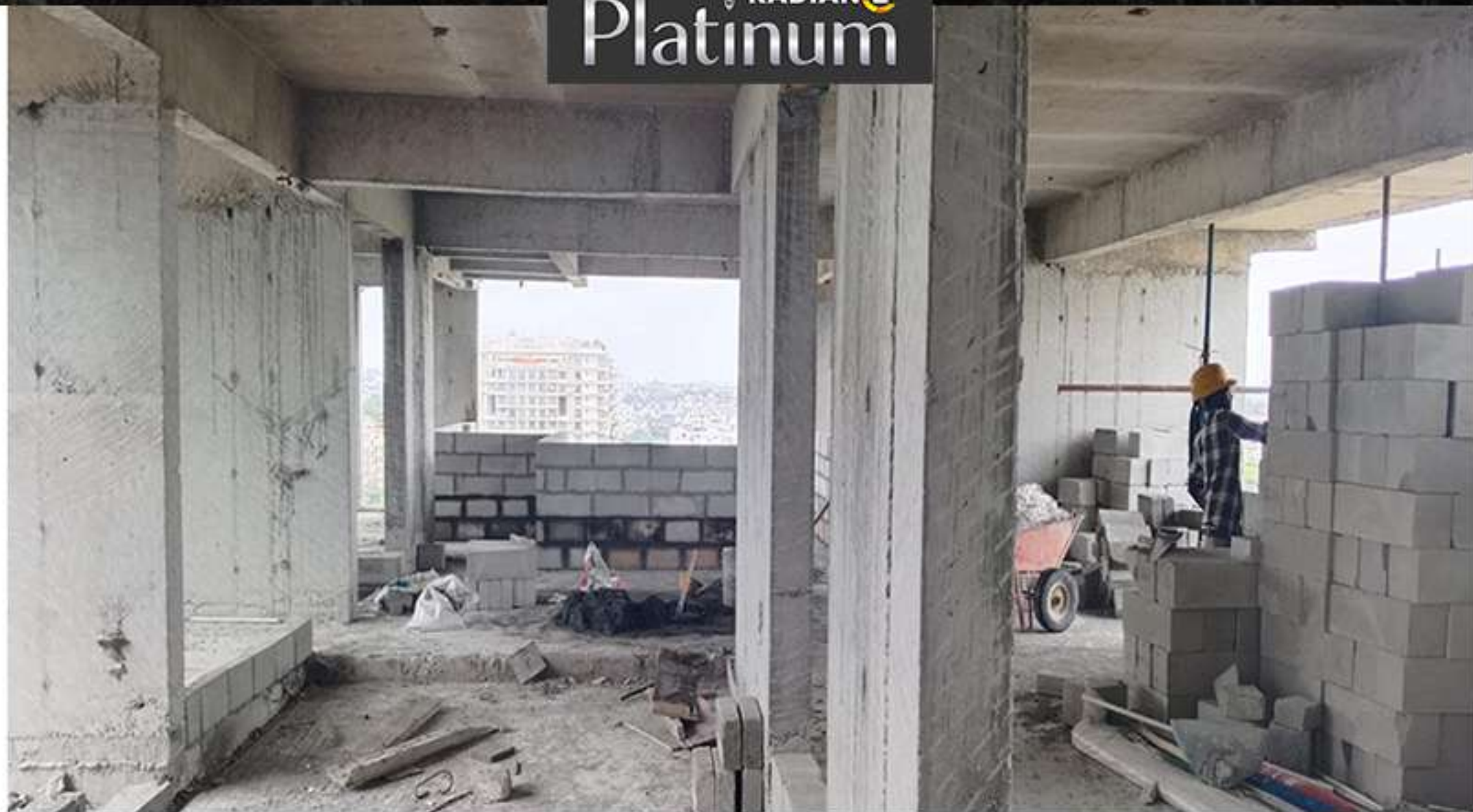
13th Floor Block Work
