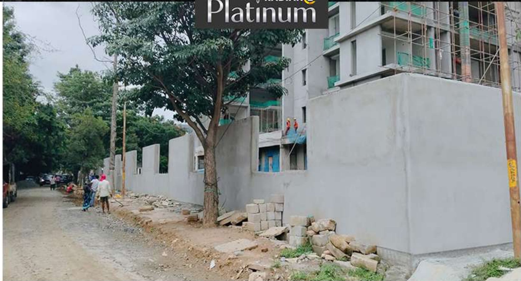
Compound Wall - East side
