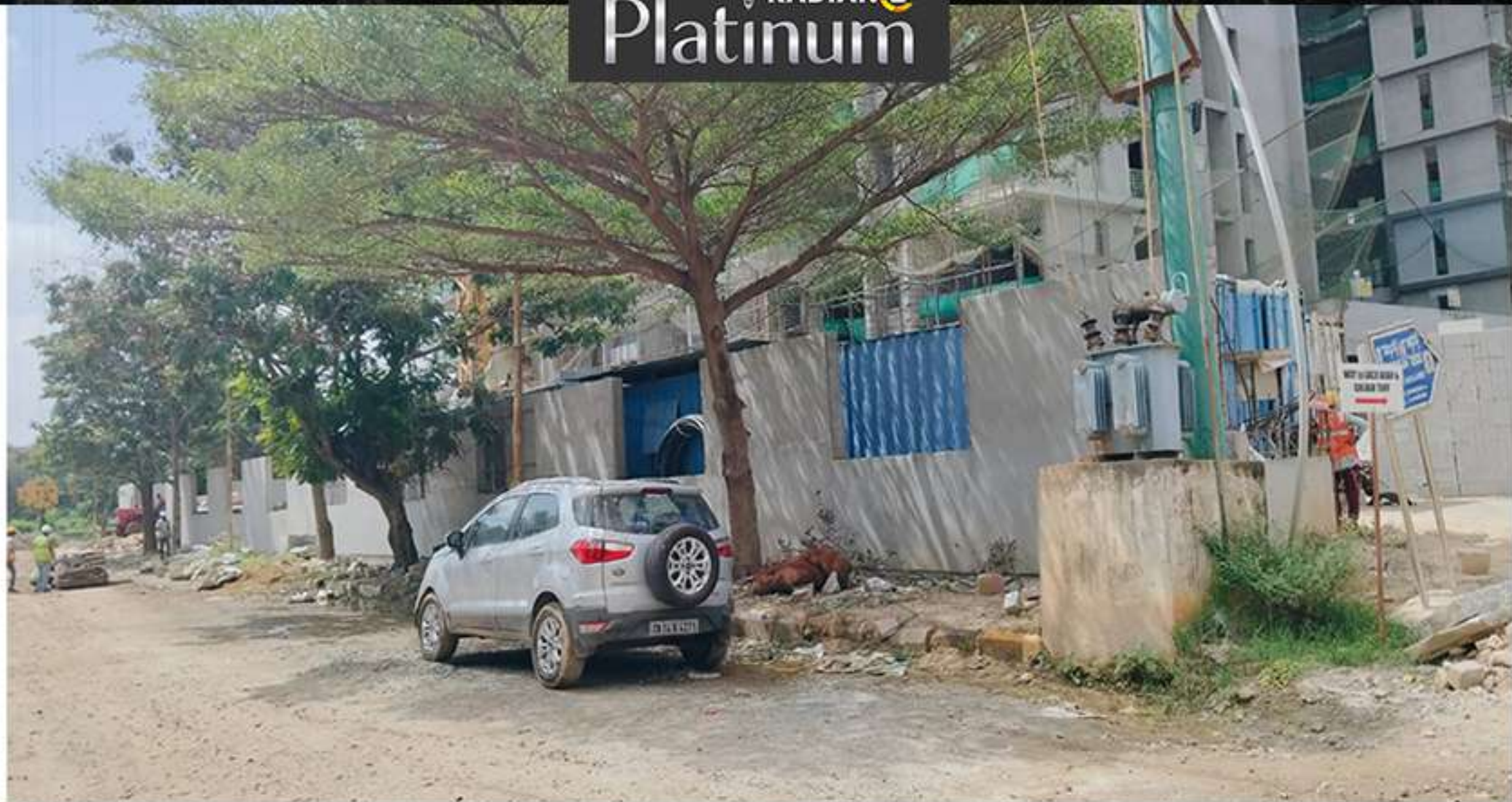
Compound Wall - North side
