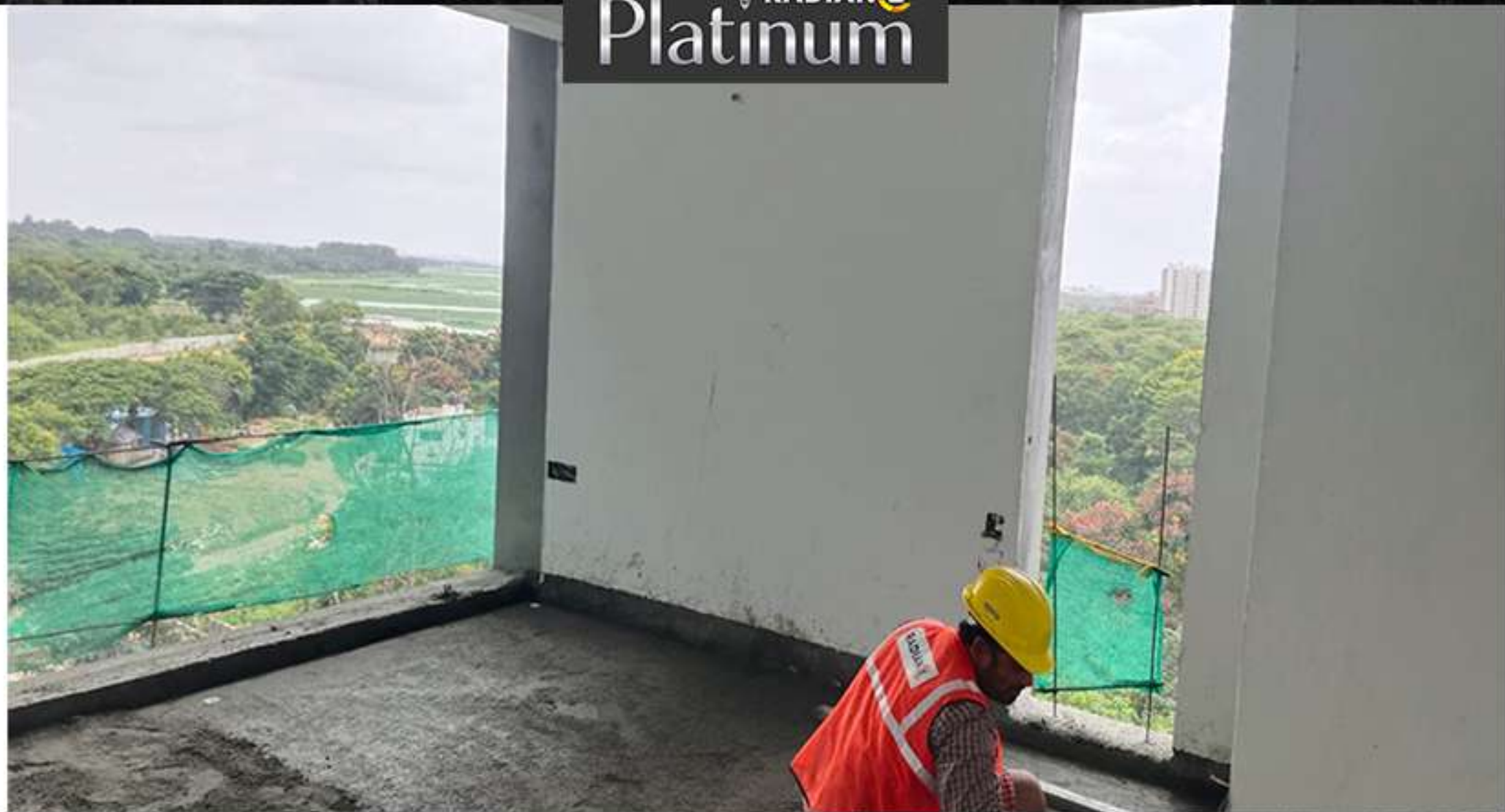
B – Block – Tile laying work – Flat 305
