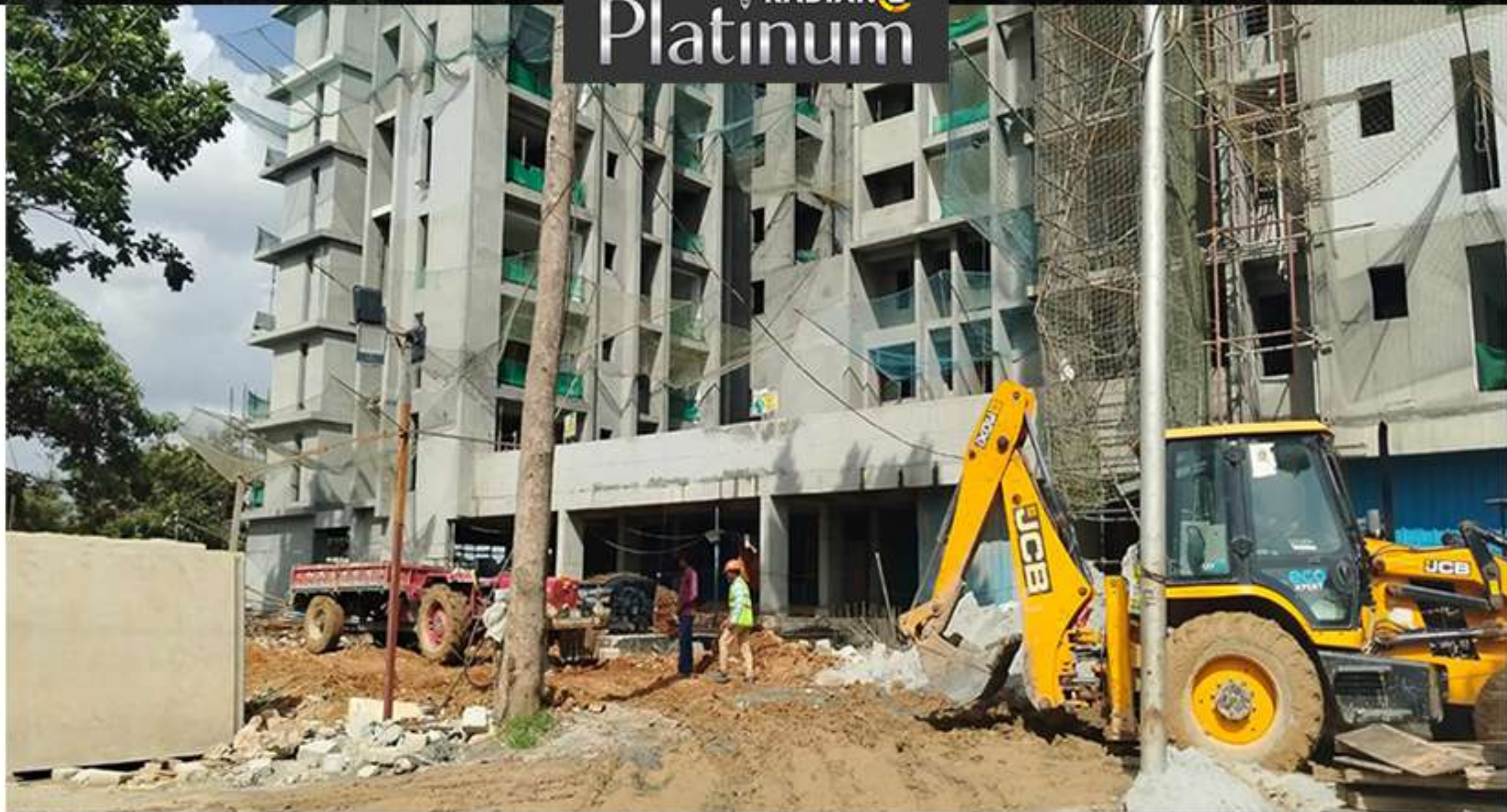
Compound Wall - West side
