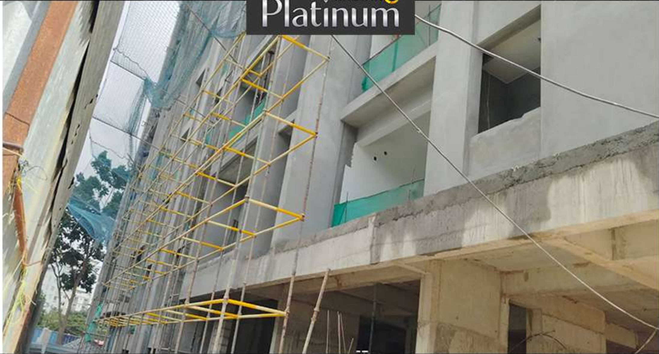
Block – B -South- External Plastering Scaffolding work (Stilt to Terrace)
