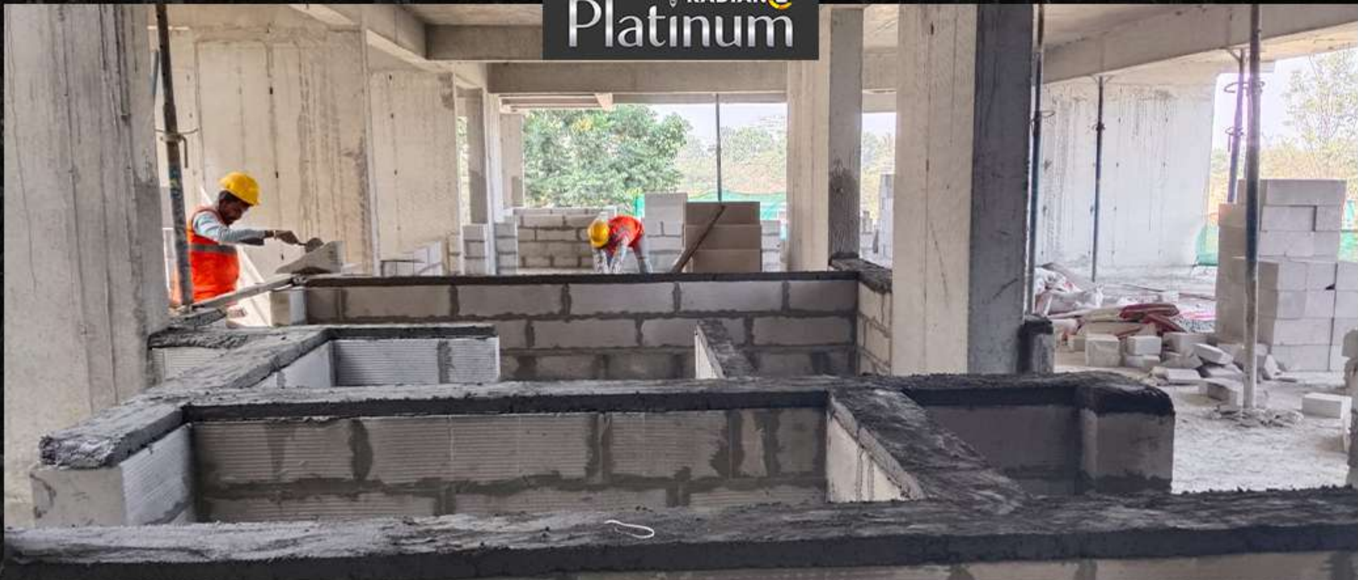
Second Floor Block Work
