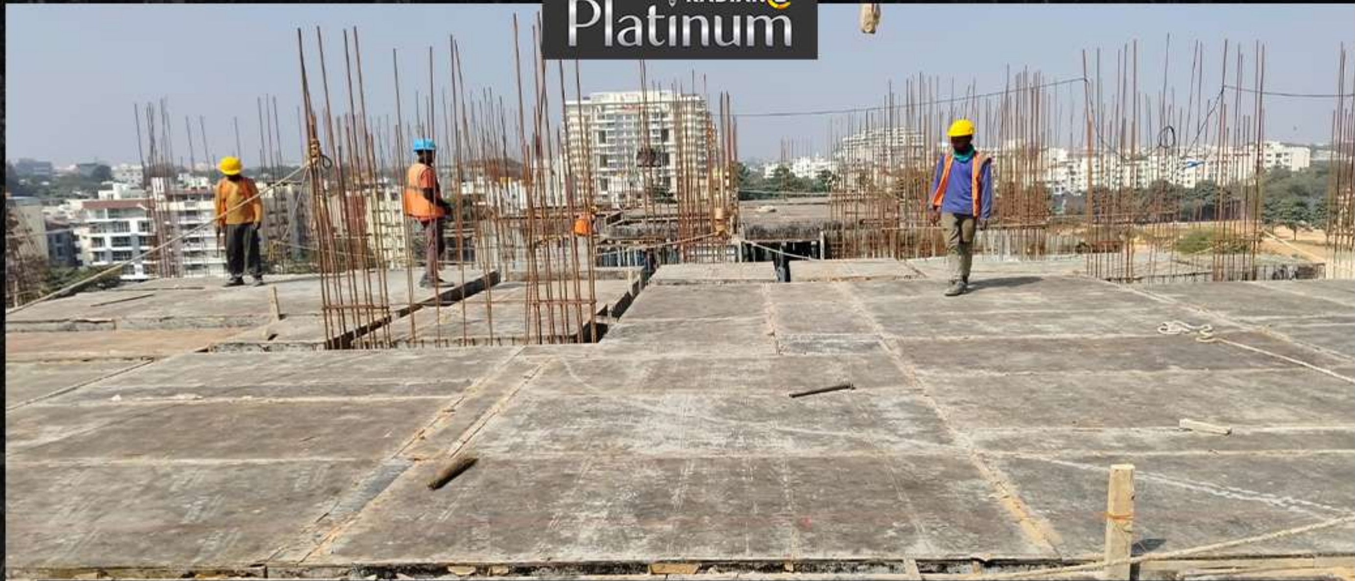
Block A - Sixth Floor Roof Slab Shuttering Work (A701,A702)
