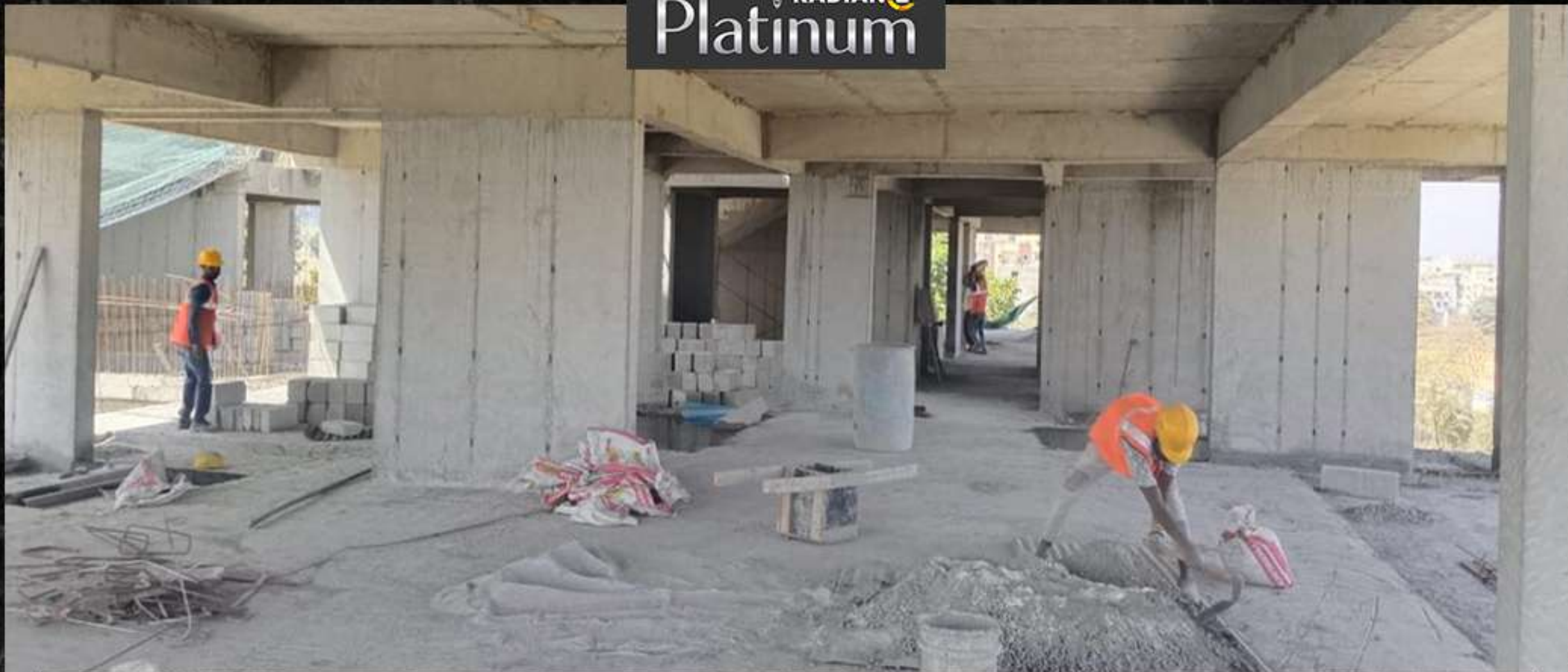
4th Floor Block Work
