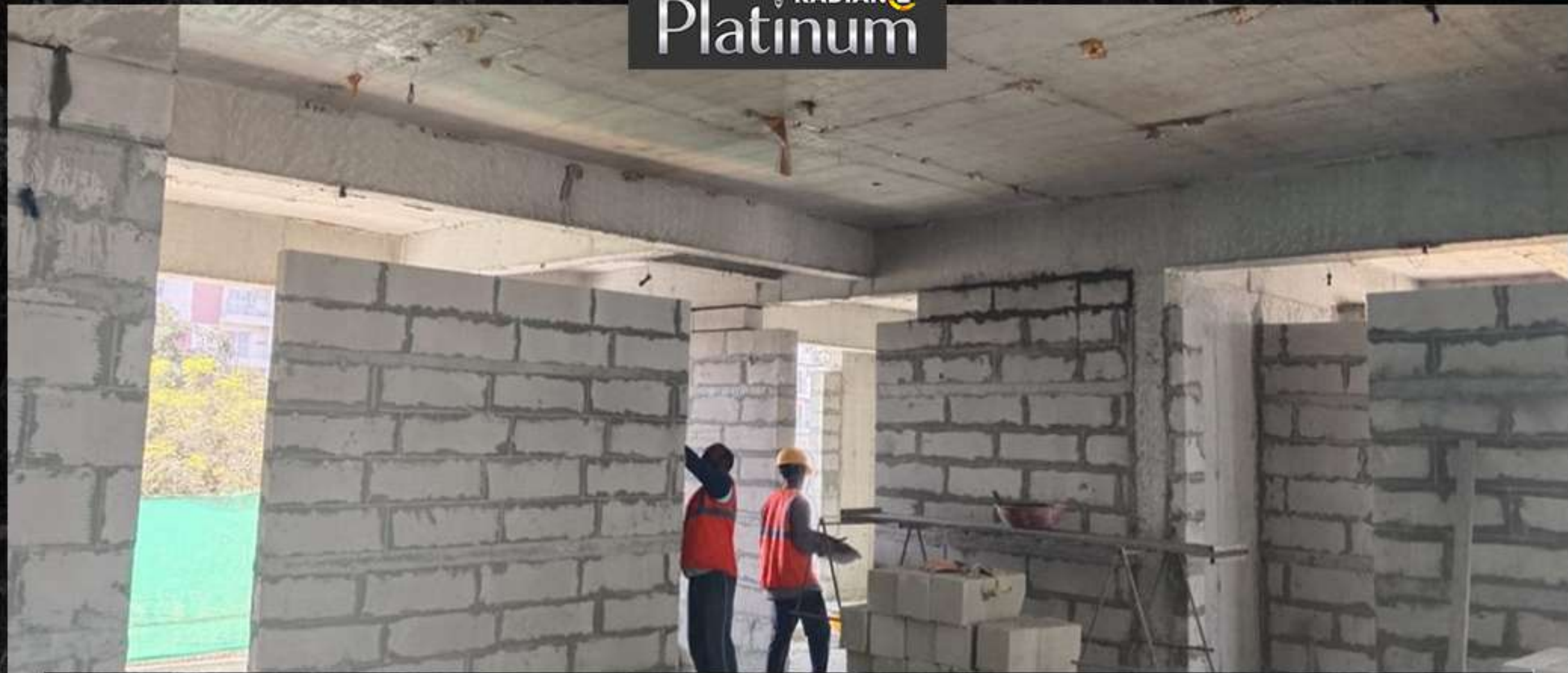
3rd Floor Block Work
