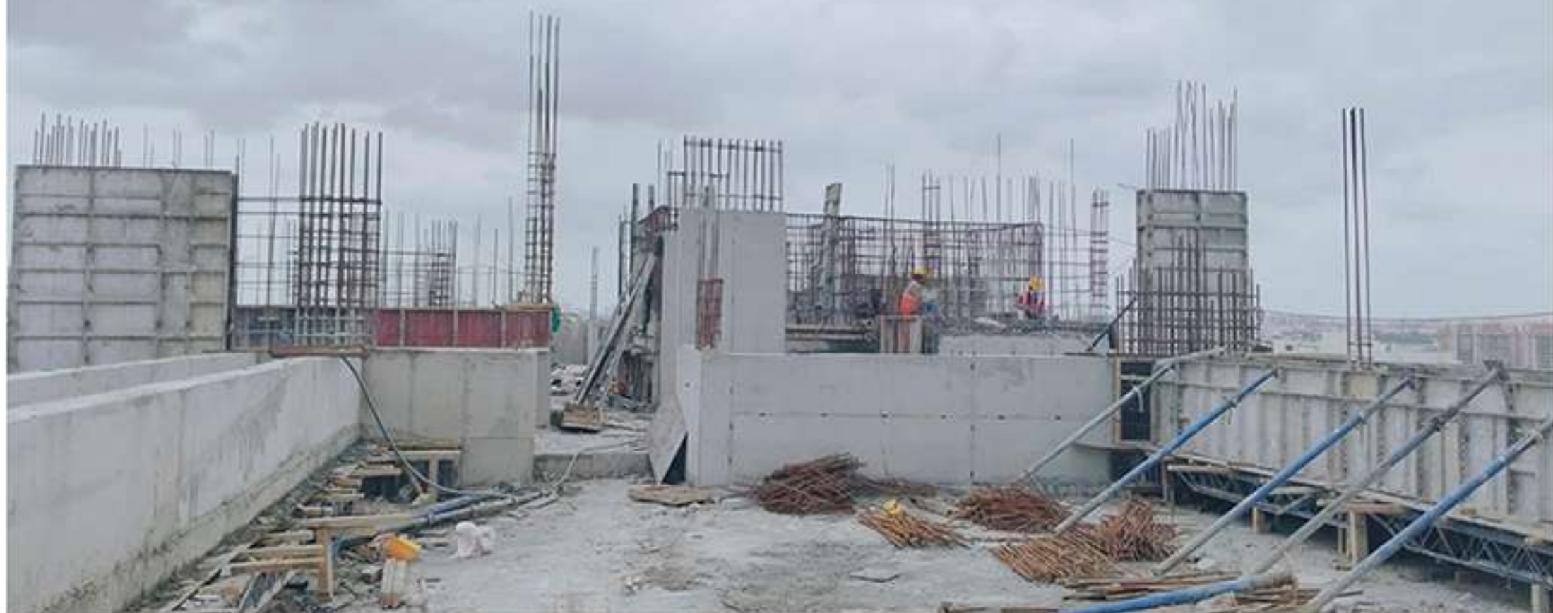
Block - B – Terrace Floor Slab (1403,1404 & 1405)
