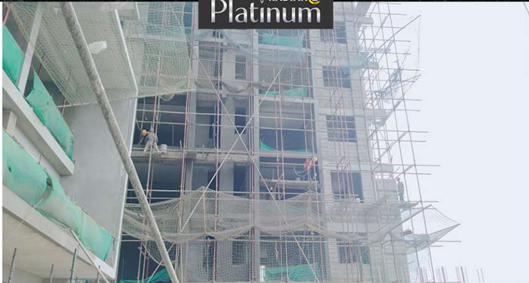
Block – A – North South – External Plastering work
