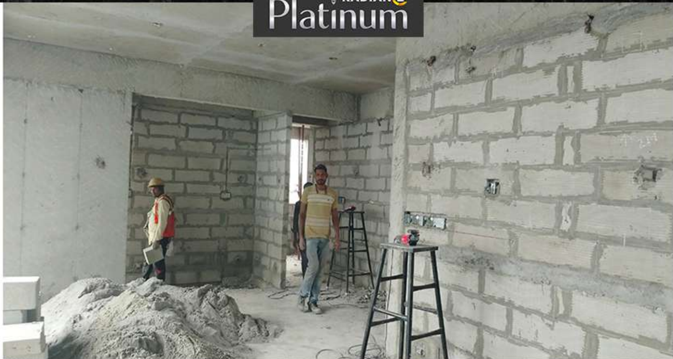
11th Floor Electrical Work
