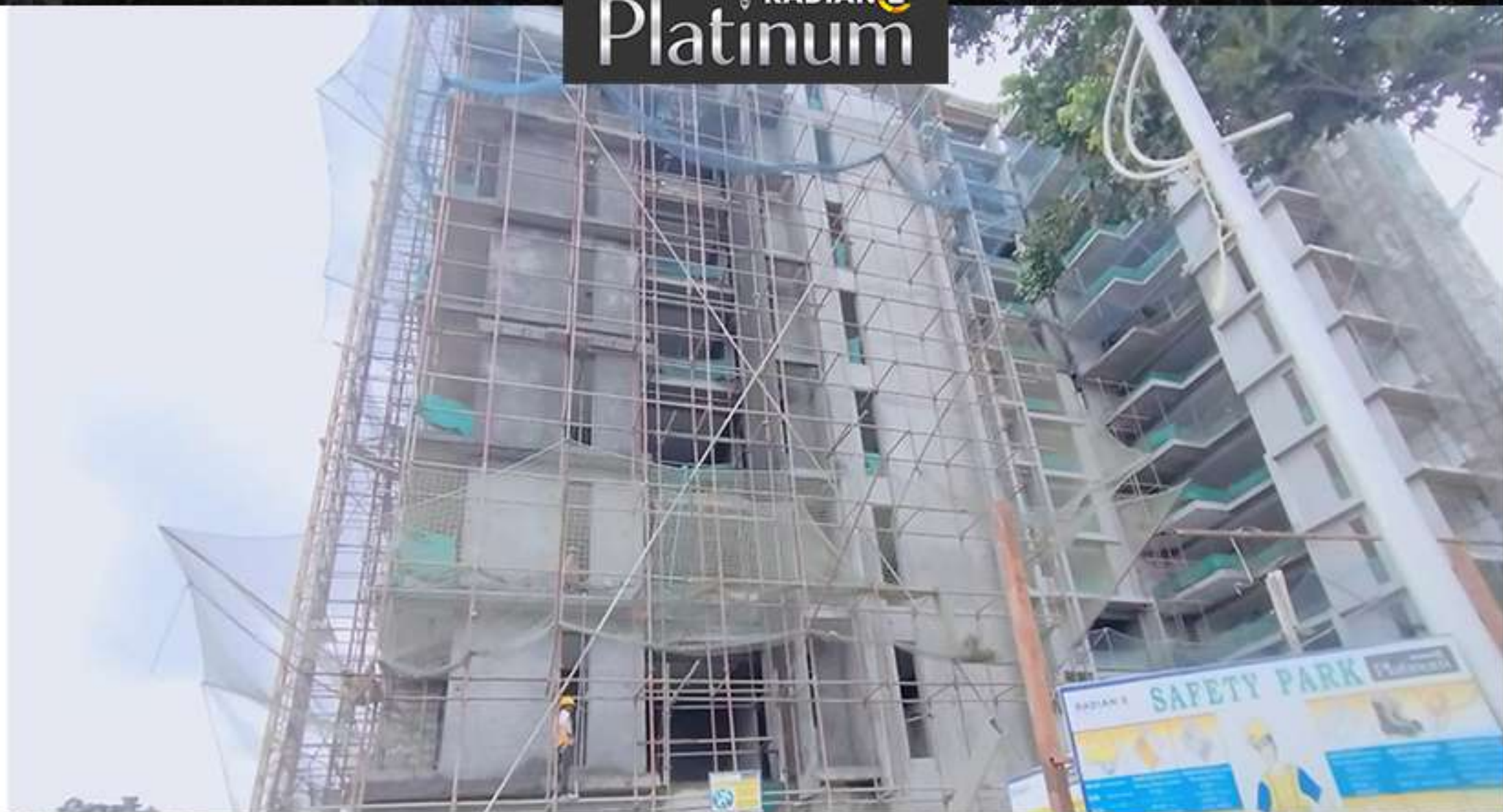
Block – A – West – External Plastering work
