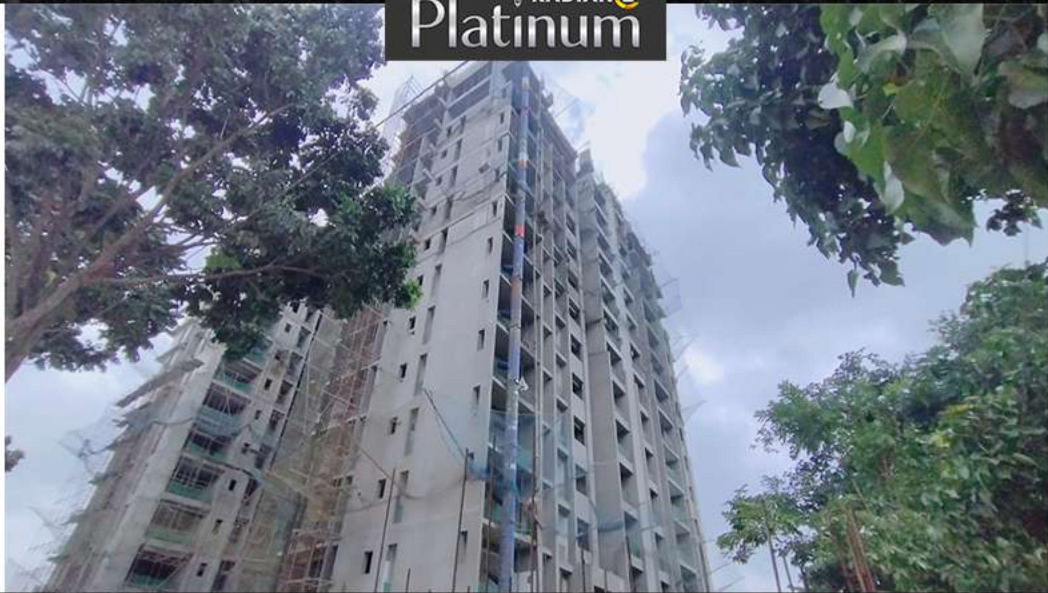
South West Corner View
