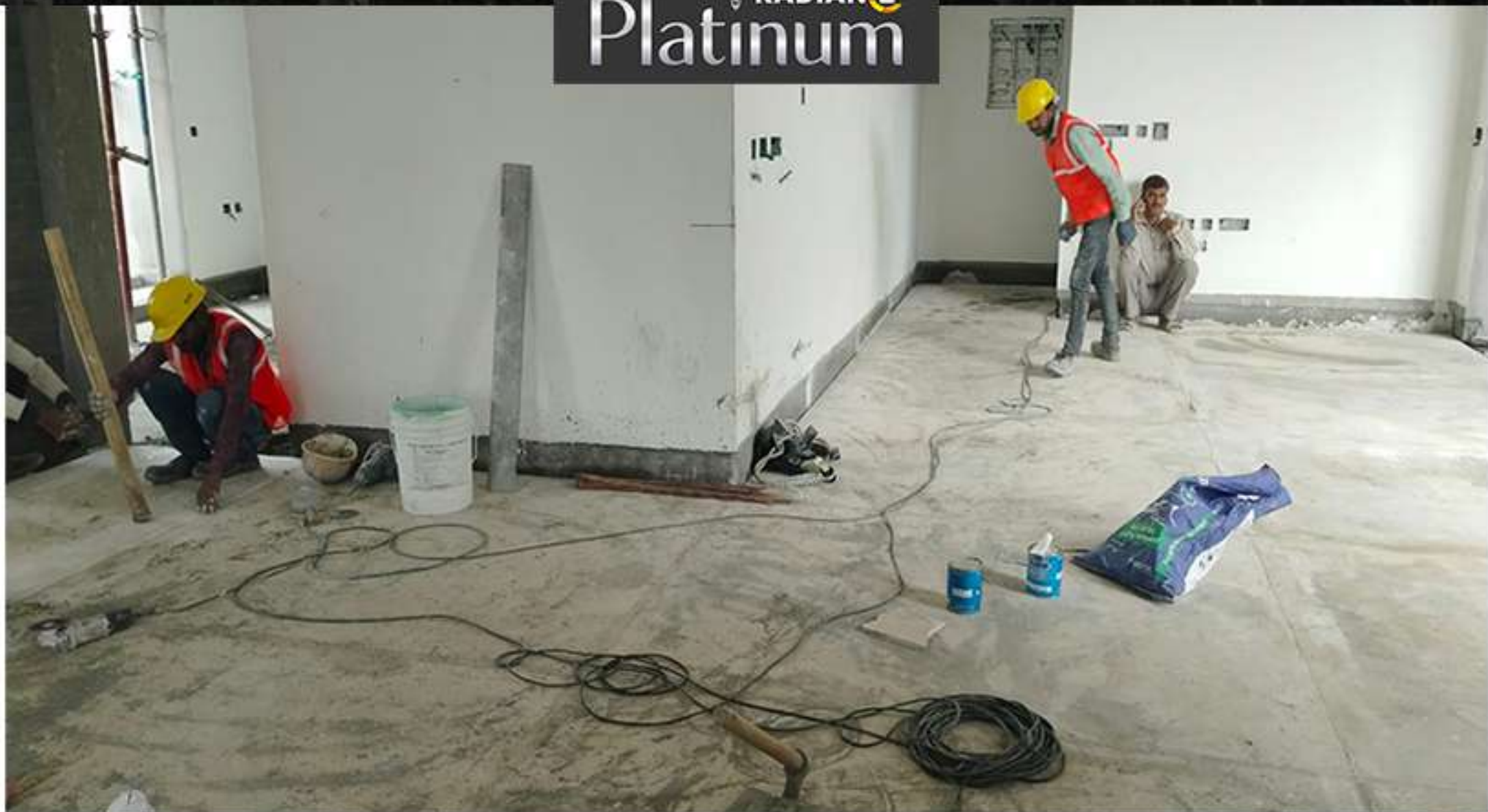
2nd Floor Marble laying work
