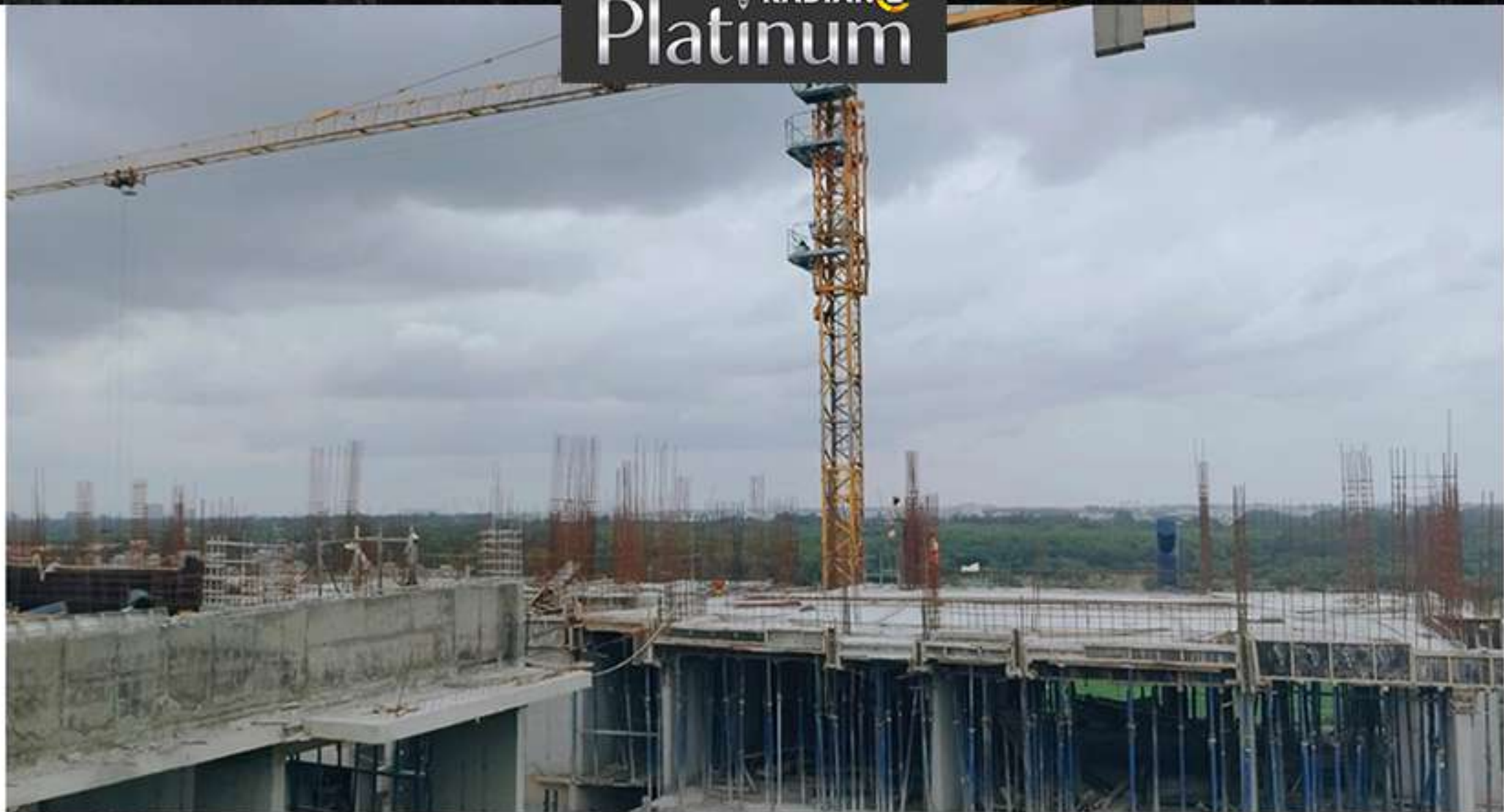
Block - A - Terrace floor slab (A1401 & A1402)
