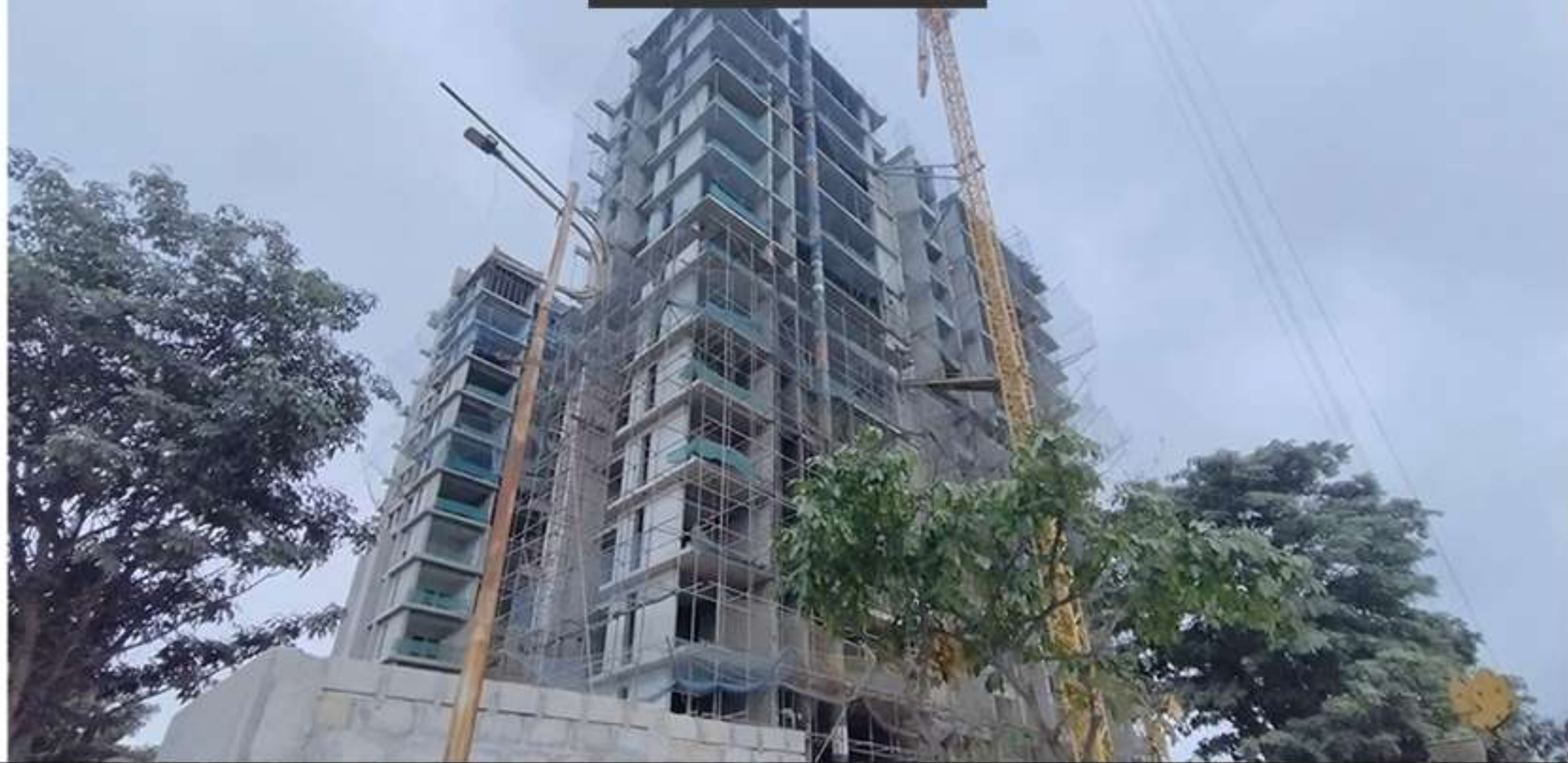
North East Corner View
