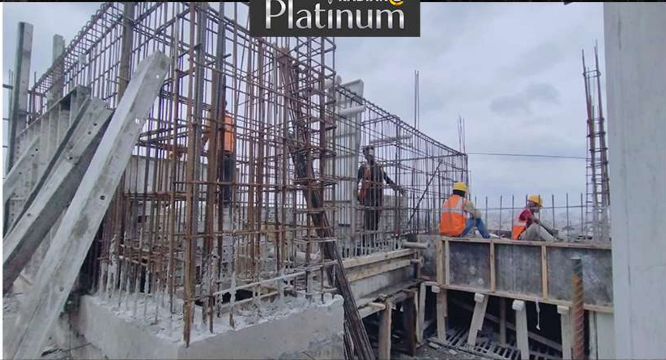
Block - B – Terrace Floor Slab (OHT)
