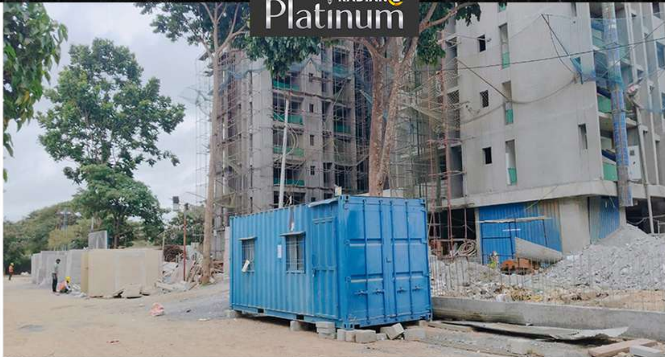
Compound wall - West side
