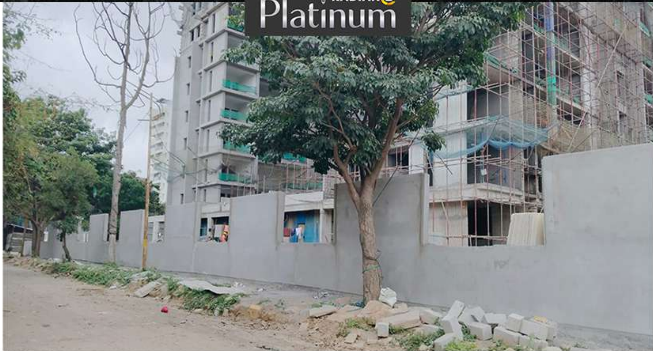
Compound wall - East side
