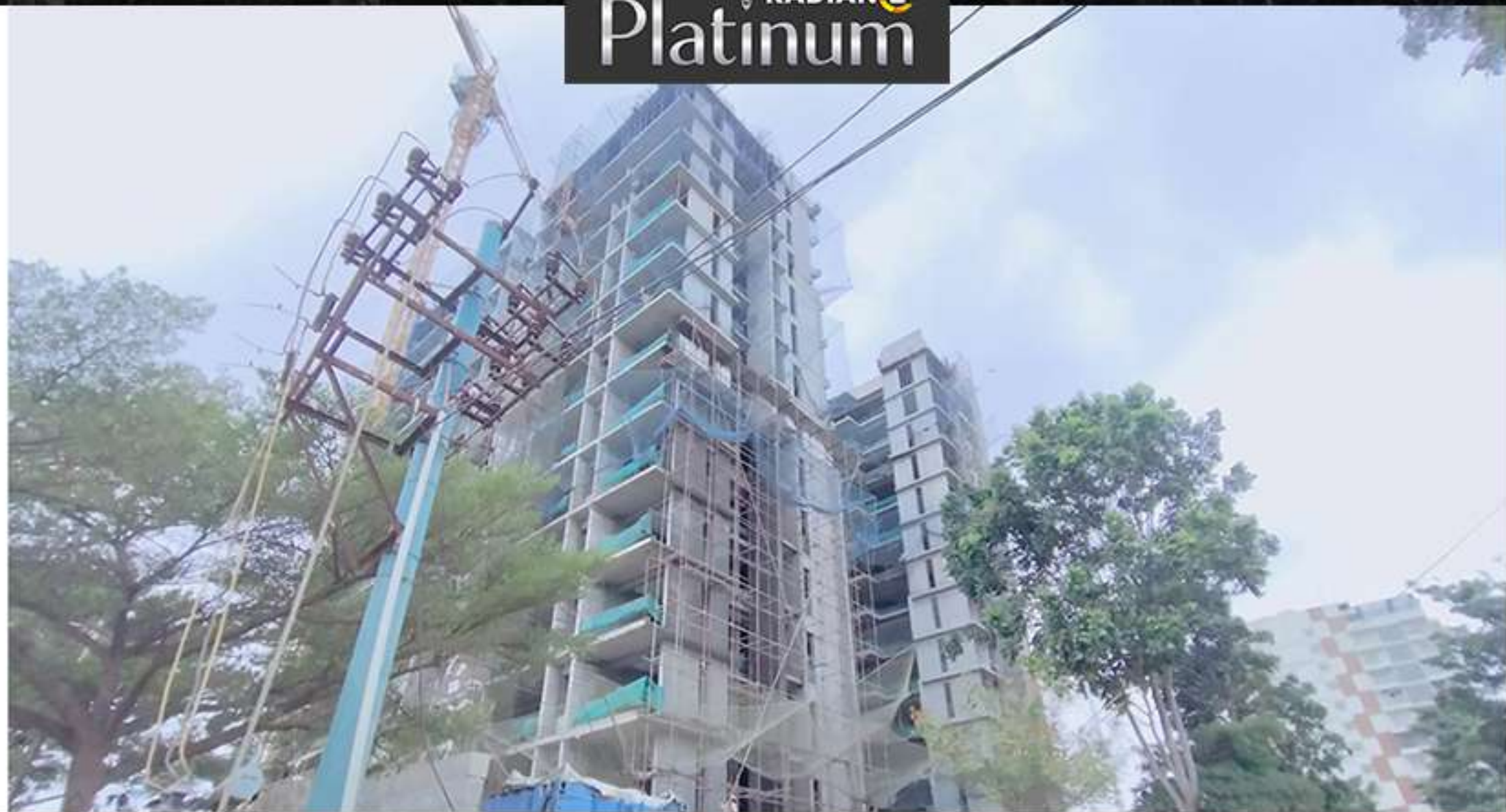
North West Corner View
