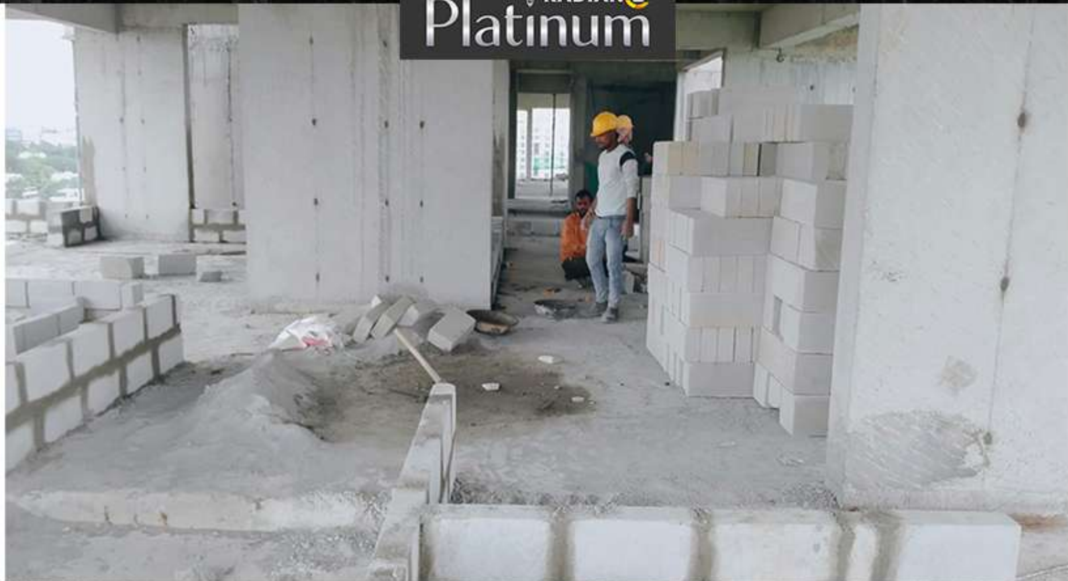
12th Floor Block Work
