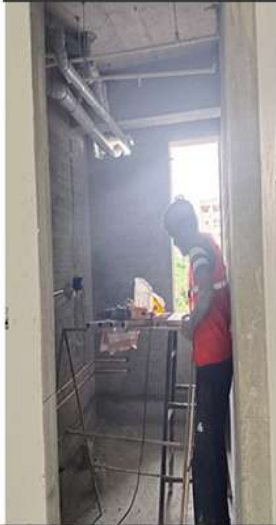
3rd Floor Plumbing Work
