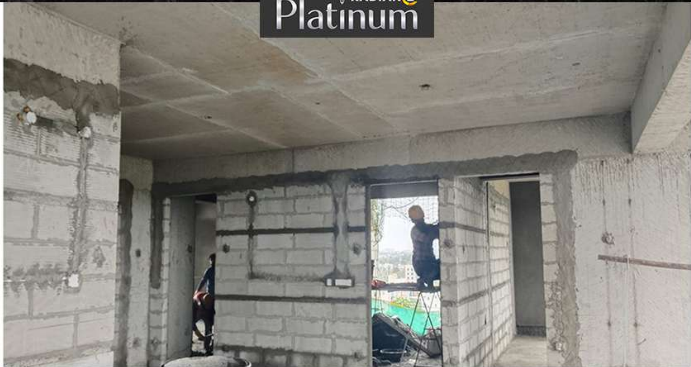
10th Floor Internal Plastering Work
