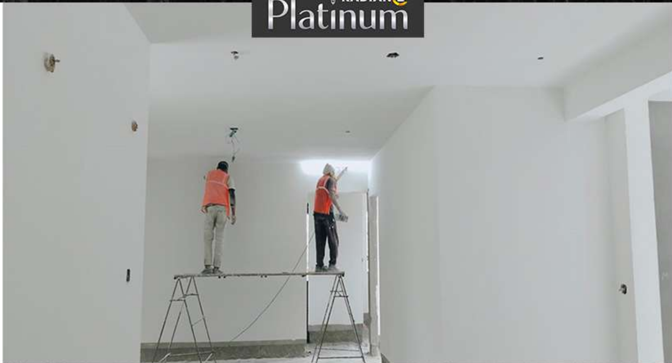
Internal Wall Putty Applying work
