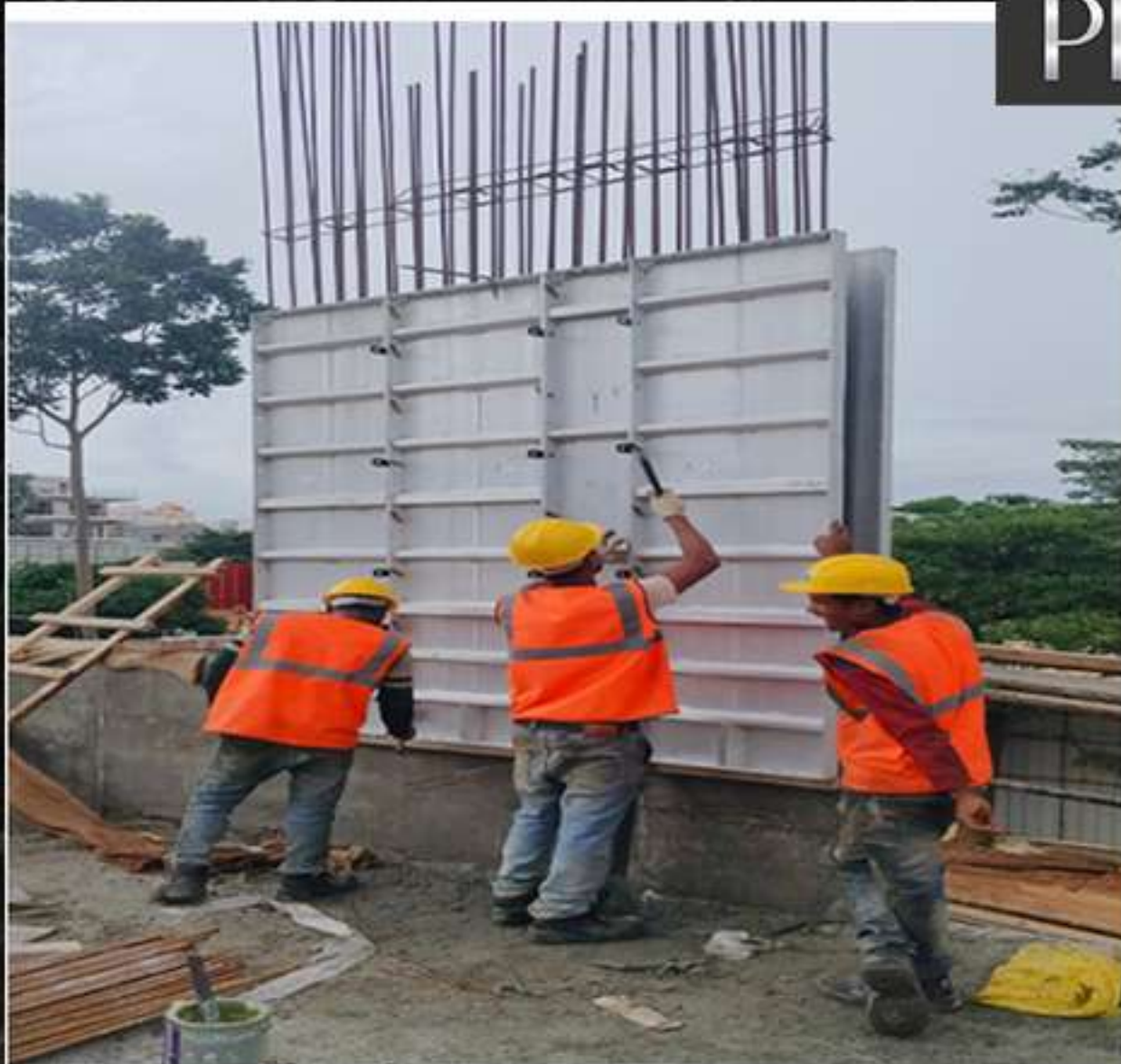
Using Aluminium formwork - Column
