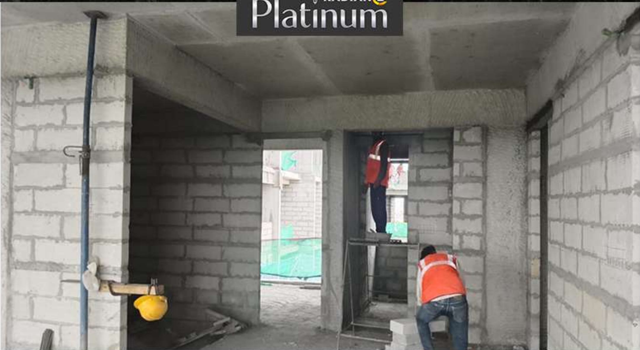
9th Floor Block Work
