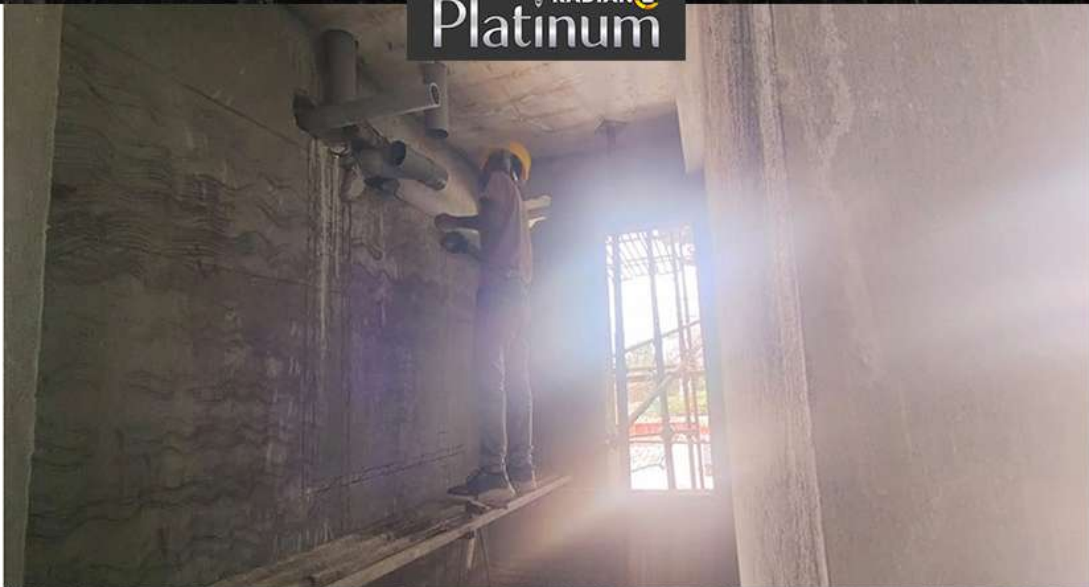
2nd Floor Plumbing Work
