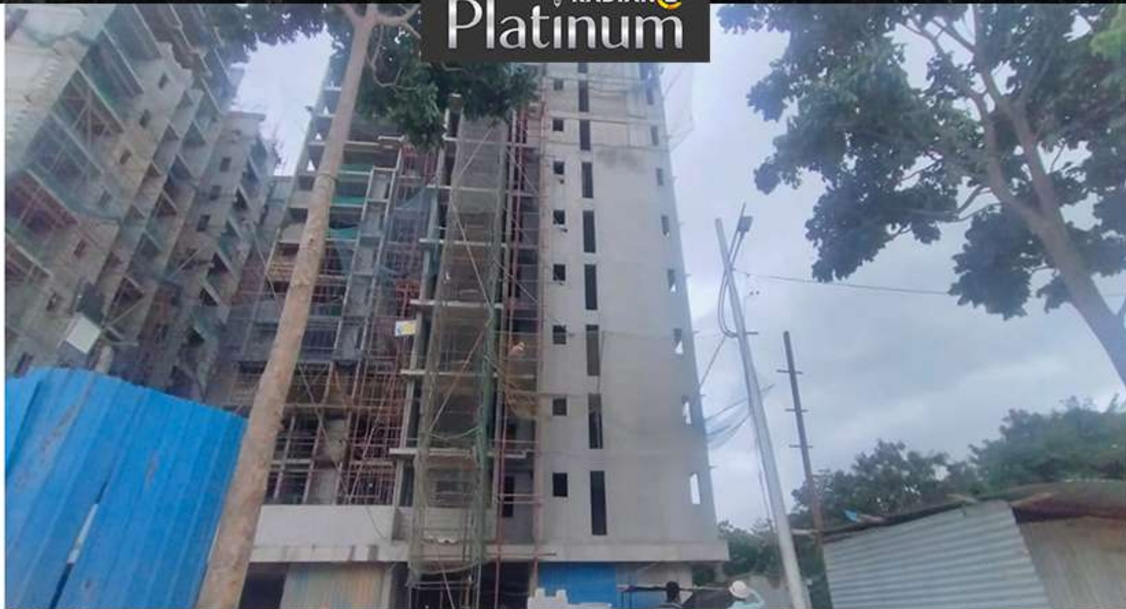
Block – B – West – External Plastering work
