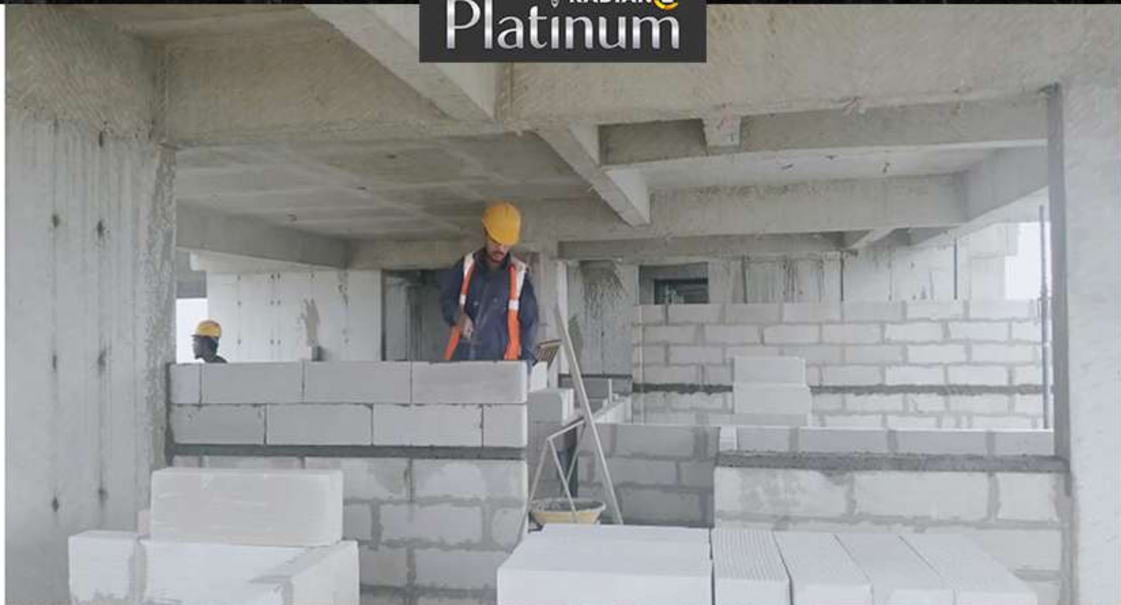
10th Floor Block Work
