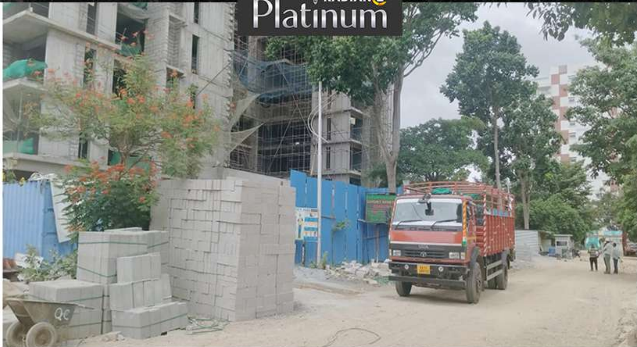
Compound wall - West side
