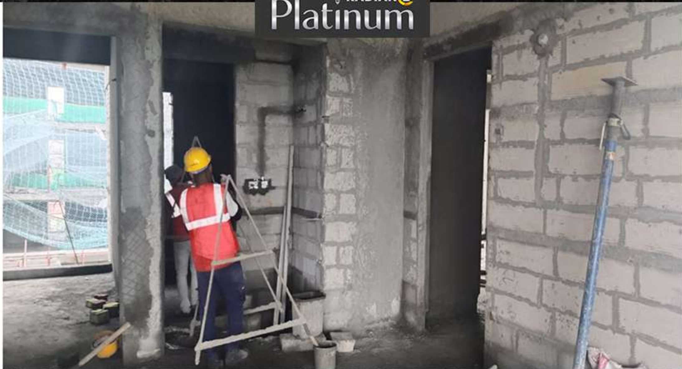
8th Floor Internal Plastering Work
