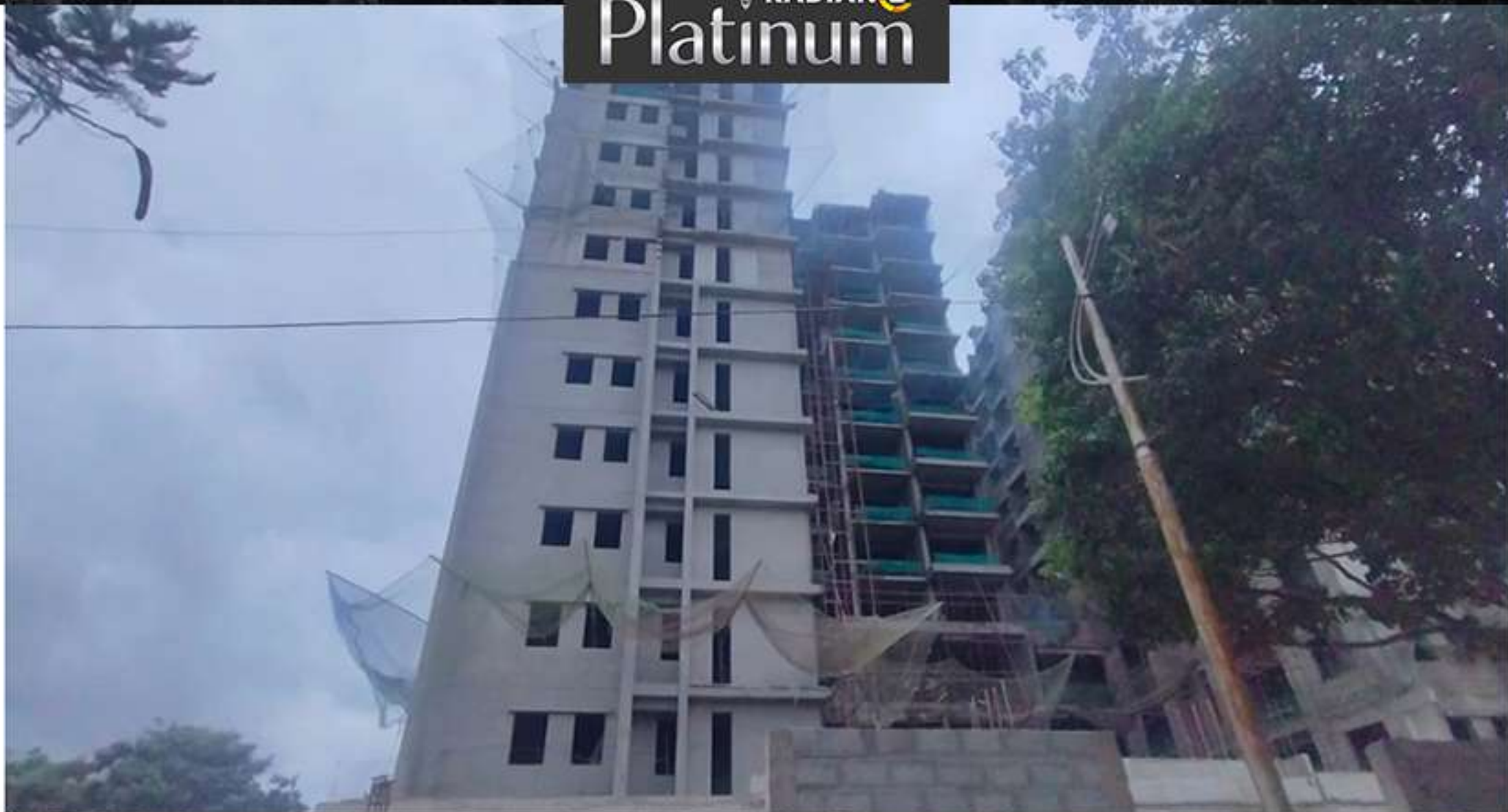
Block B - East - External Plastering work
