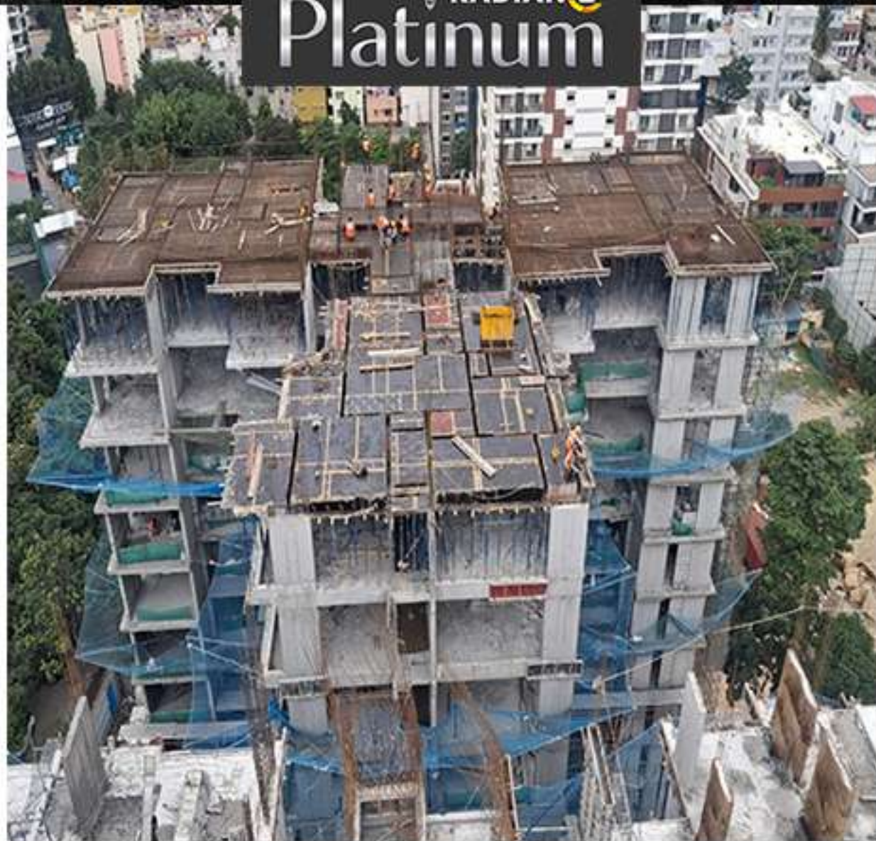
Block - B 13th Floor Roof Slab- Terrace Floor Slab
