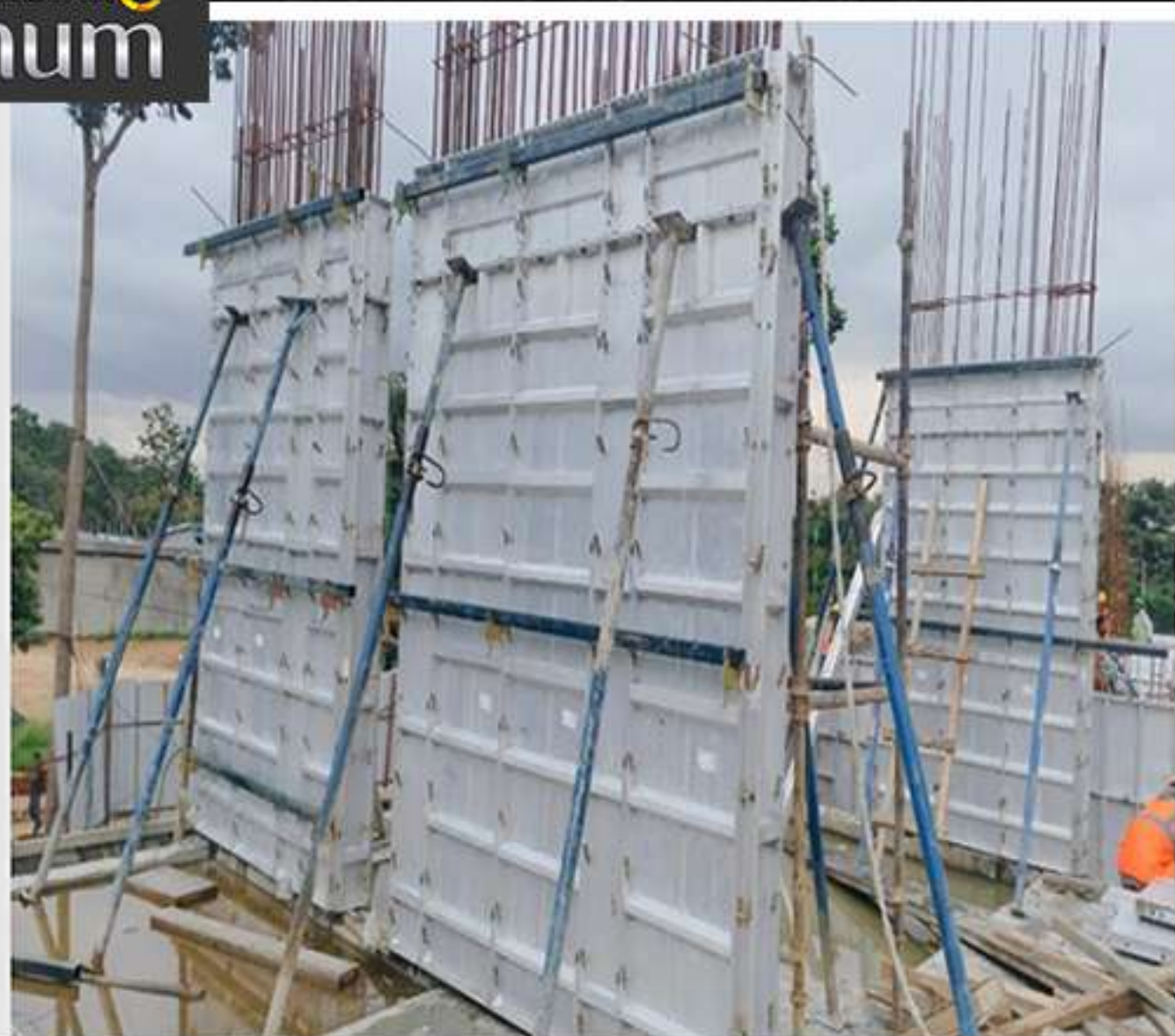
Using Aluminium formwork - Column
