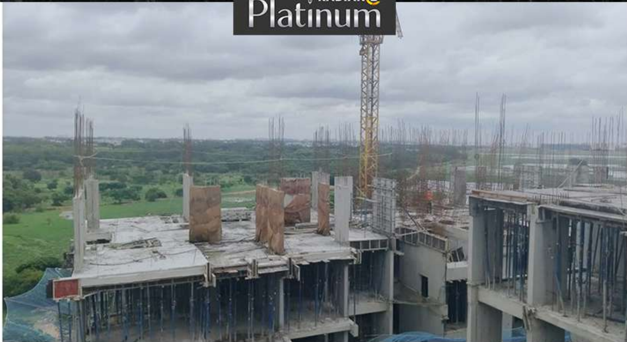
Block - A - 13th floor slab (A1301 & A1302)
