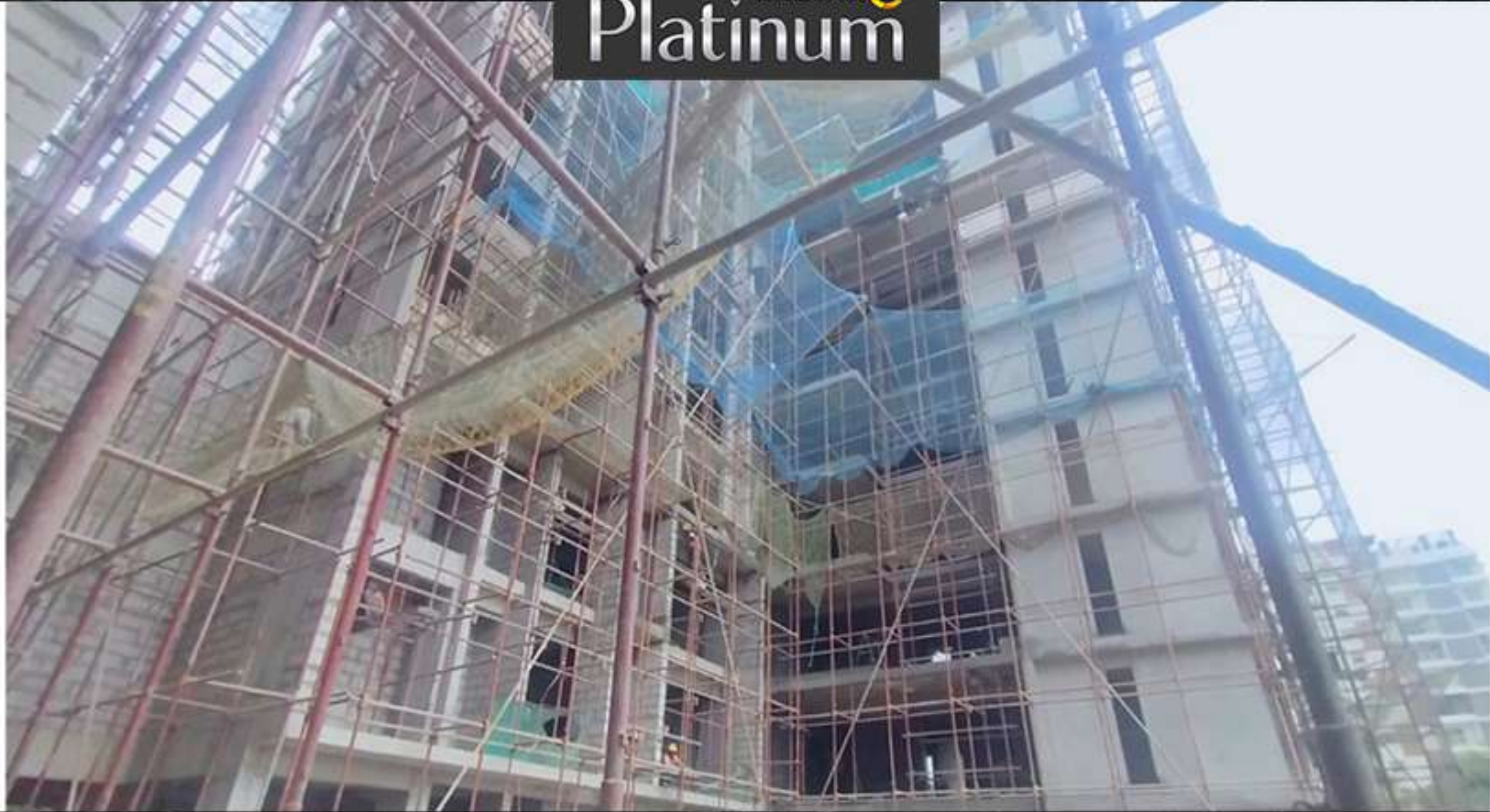
Block – B – North West – External Plastering work
