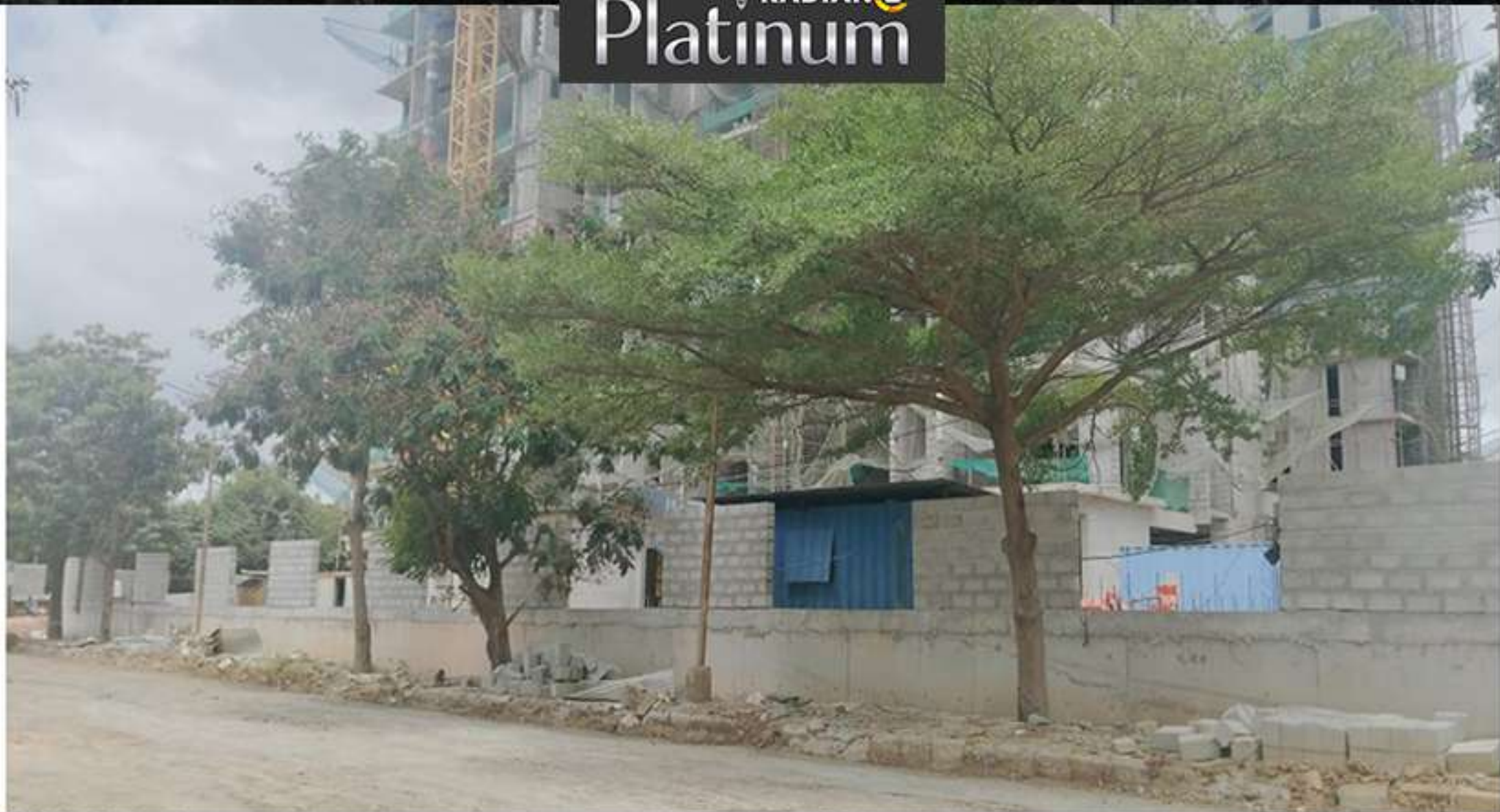
Compound wall - North side
