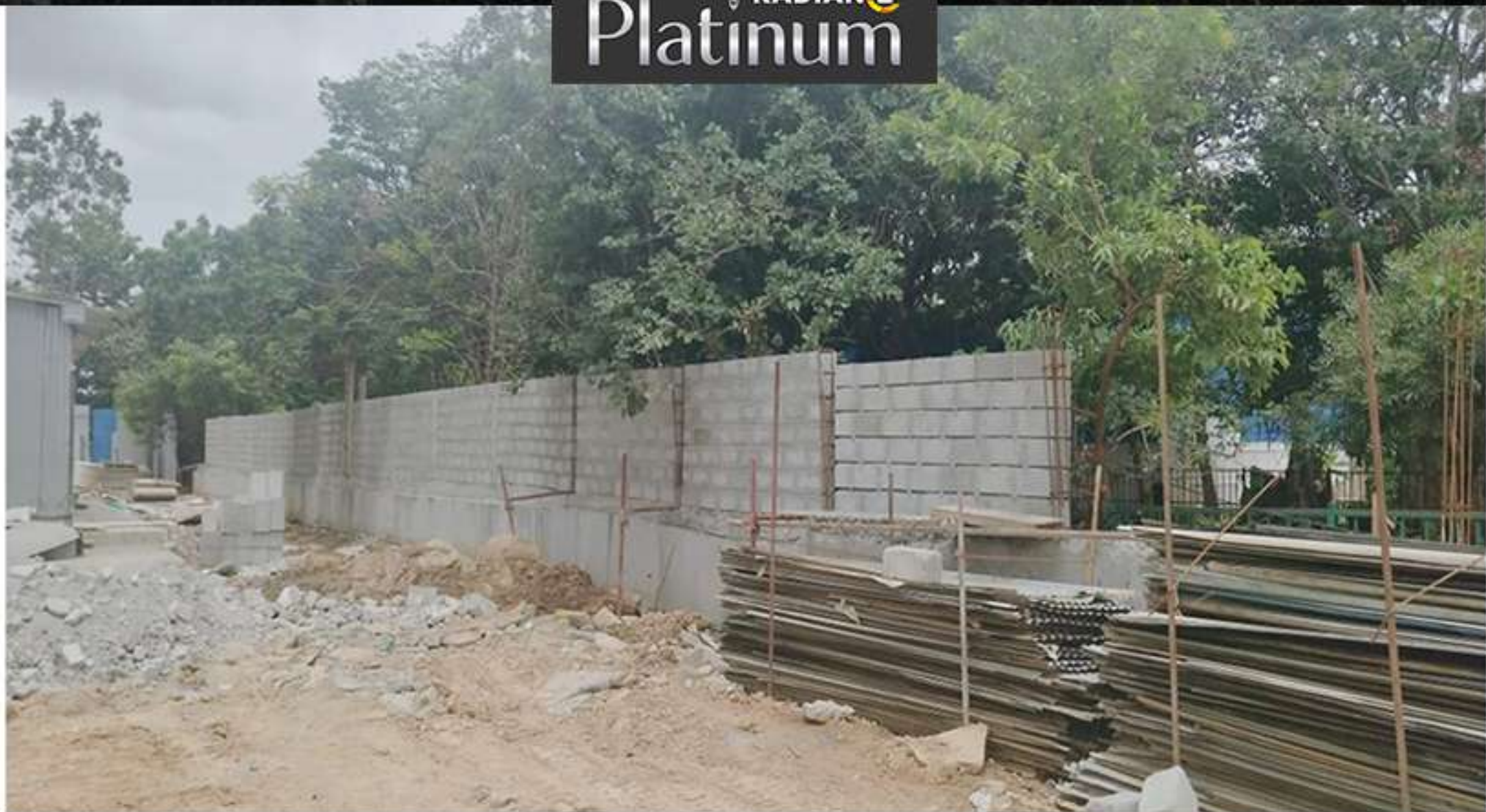
Compound wall - South side
