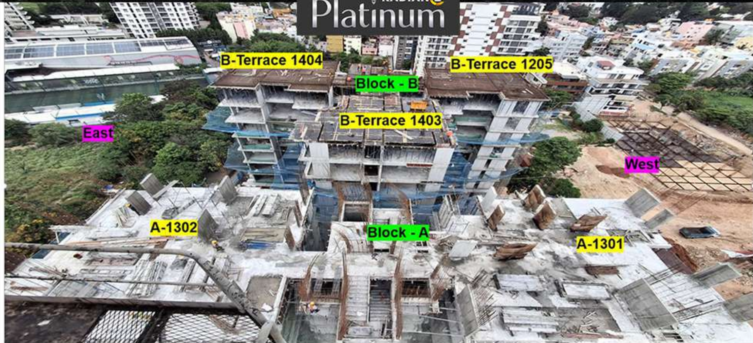
Master View - 12th floor roof slab
