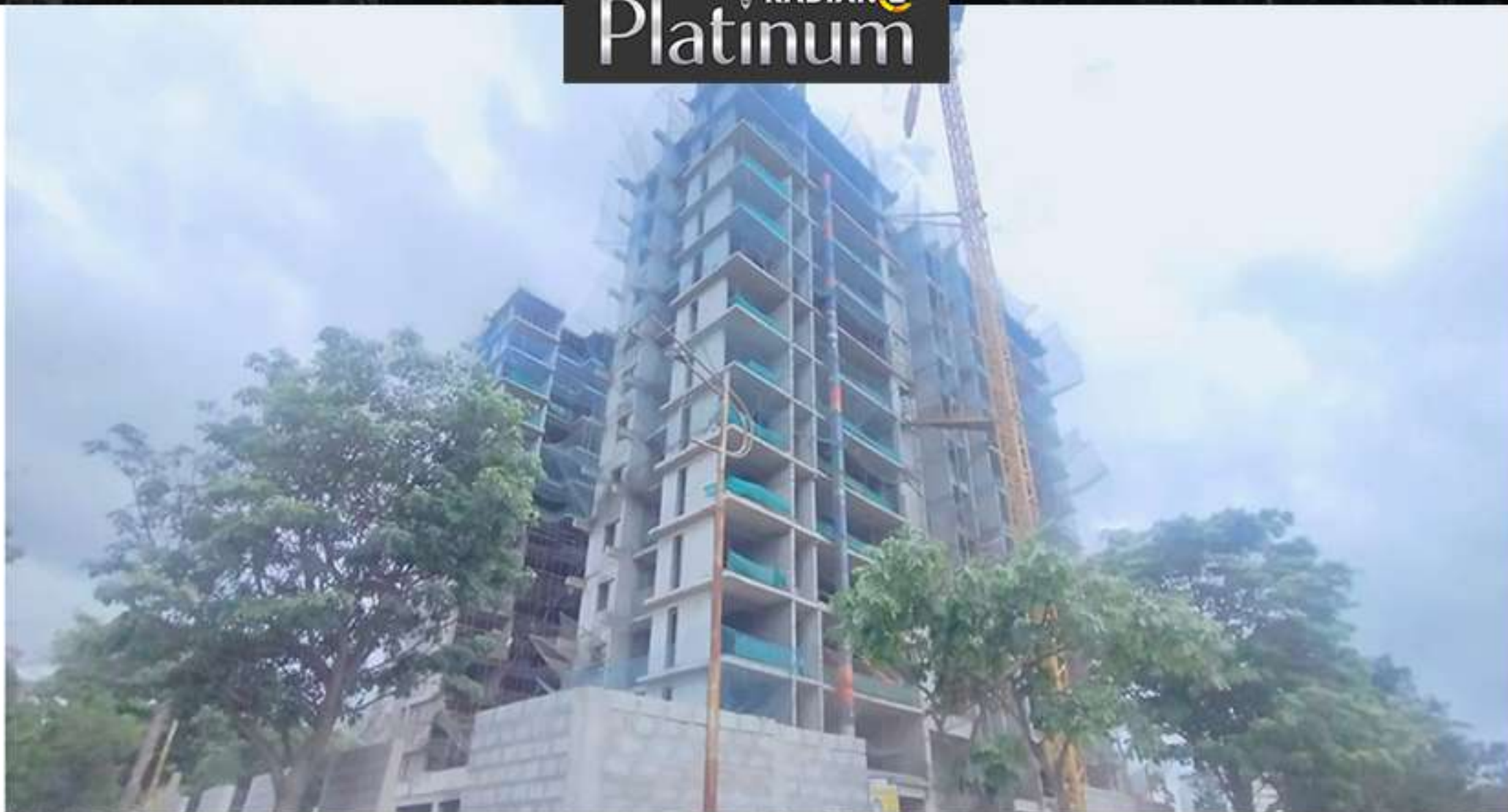
North East Corner View
