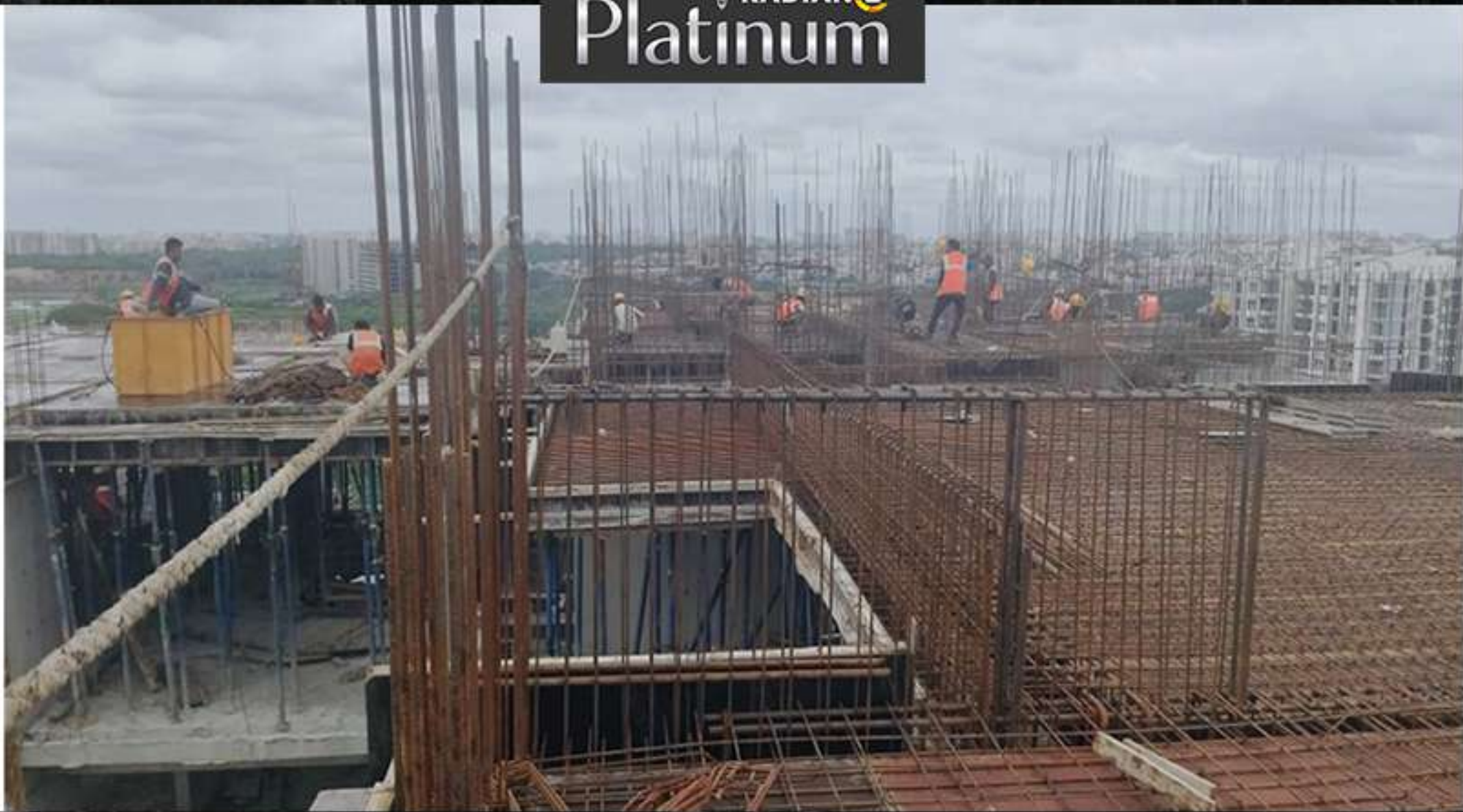
Block - B - 13th Floor Roof Slab – Terrace Floor
