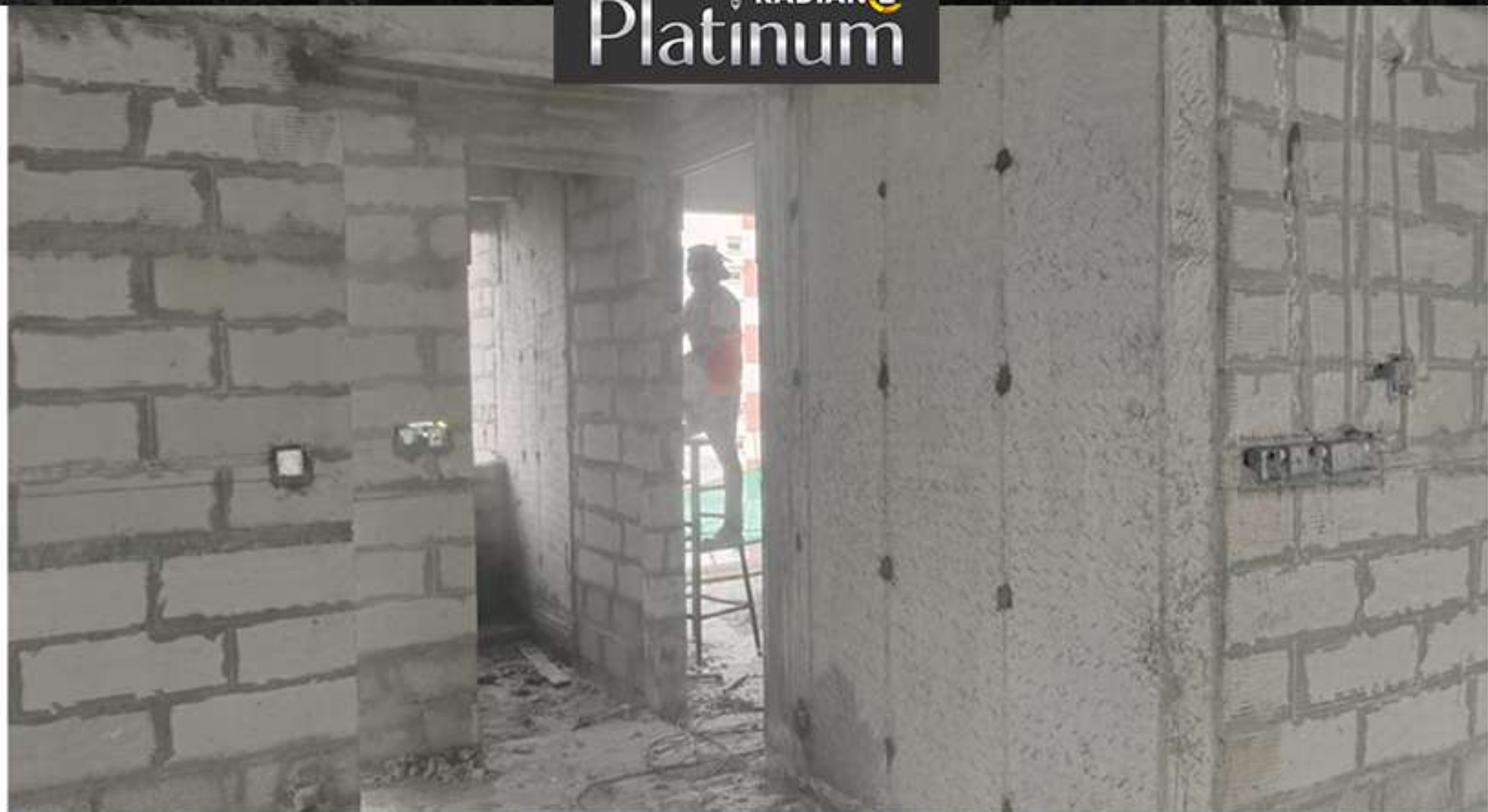
9th Floor Electrical Work
