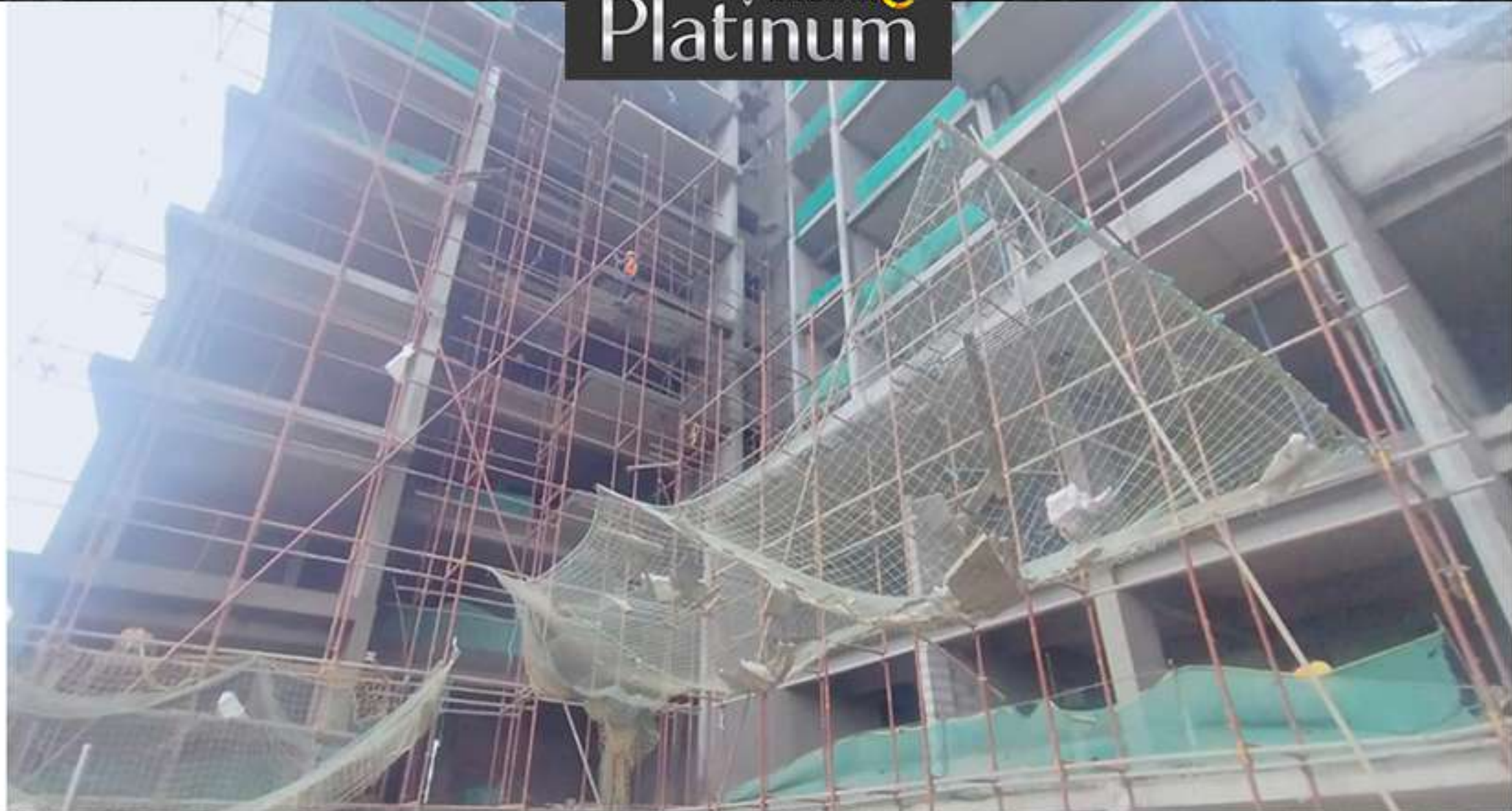
Block – B - North East - External Plastering work
