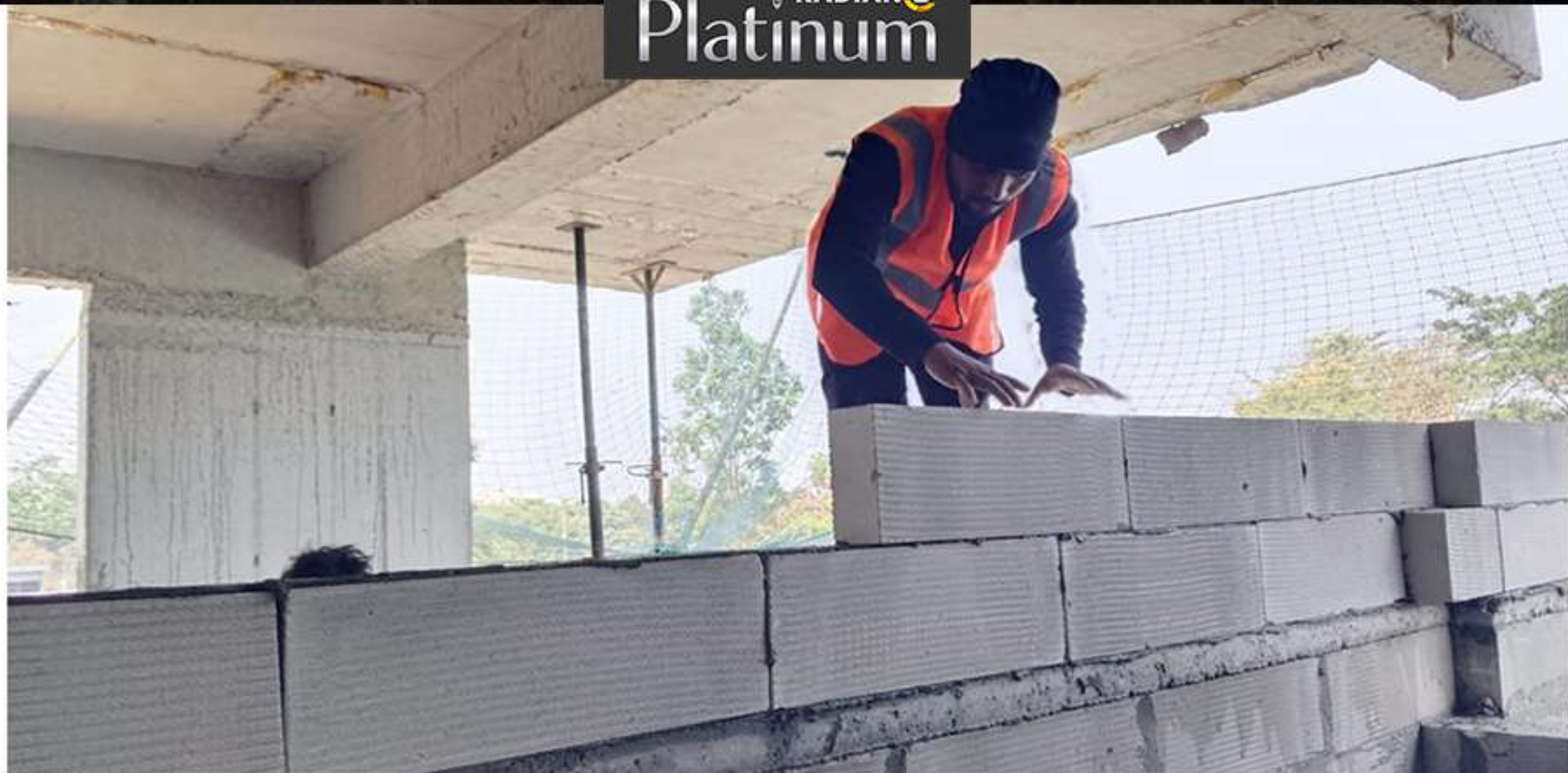
Using AAC Block With Adhesive (Ultratech)
