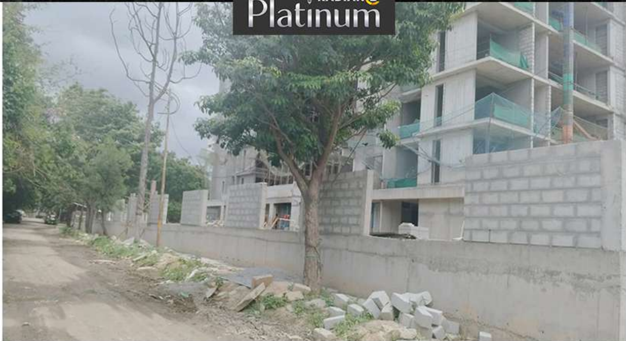
Compound wall - East side
