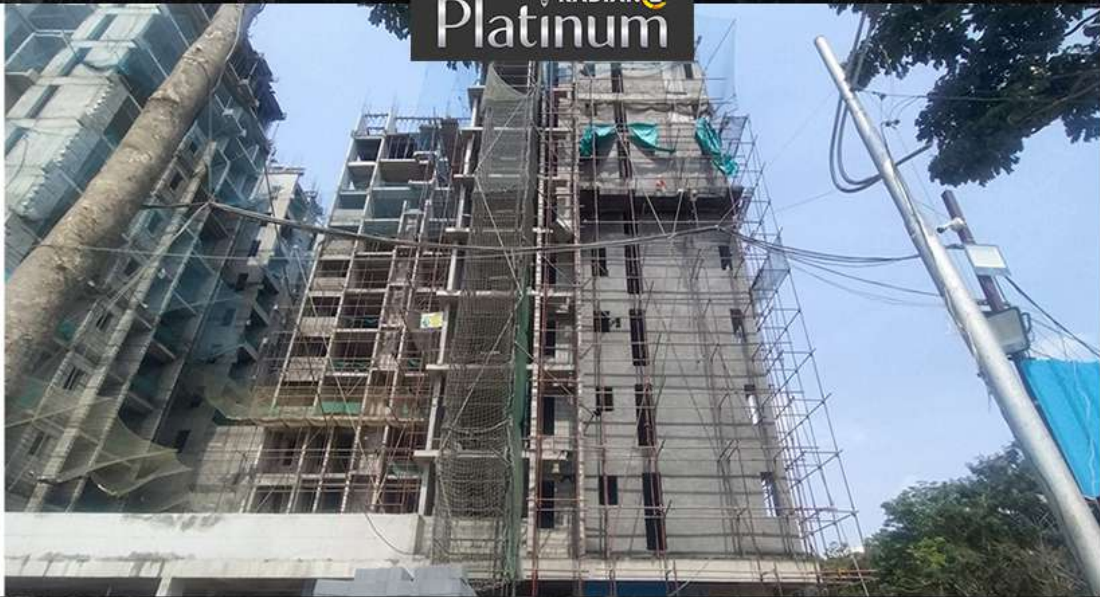
West- External Plastering Work (upto 6th Floor)
