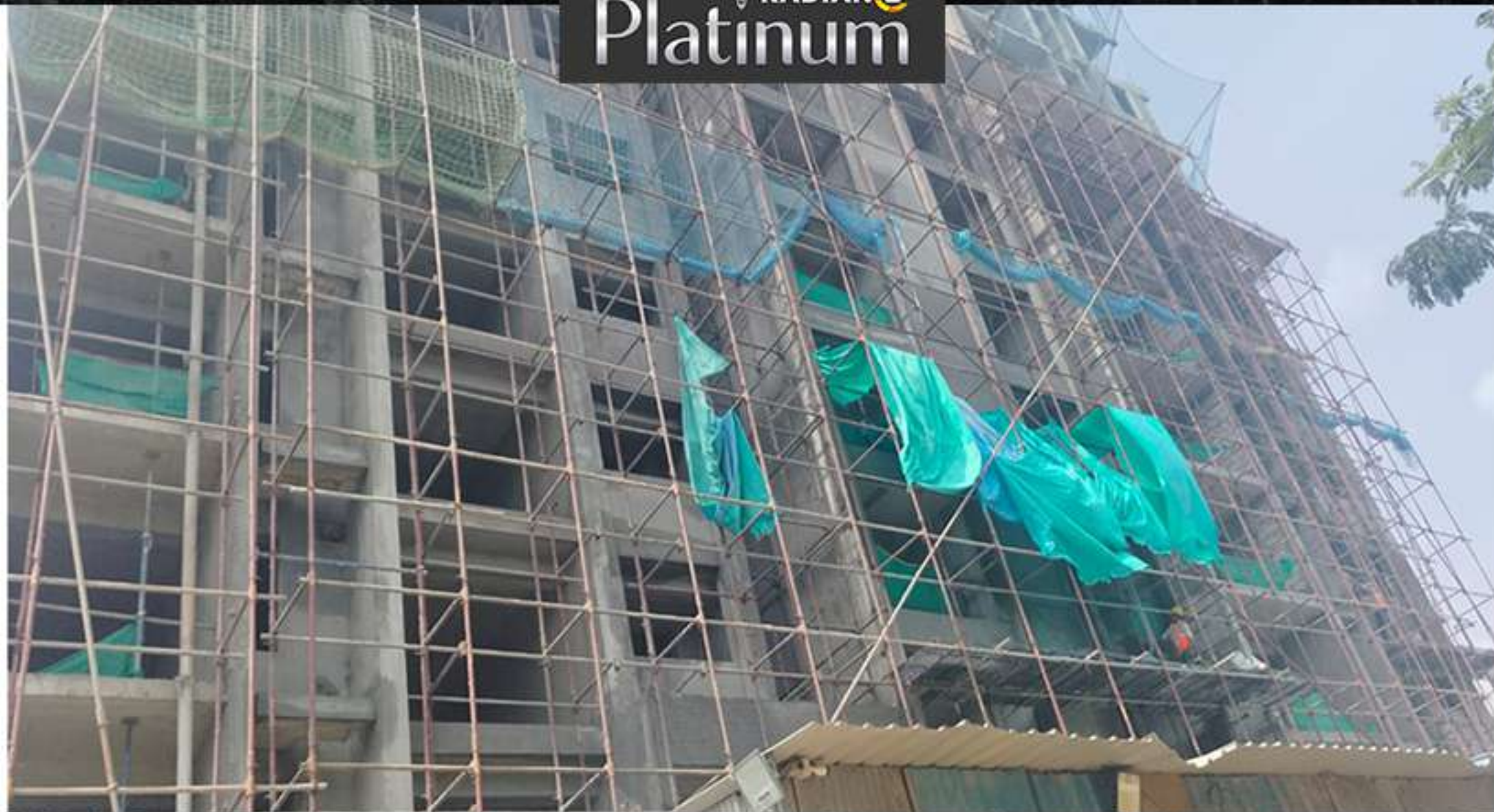
South- External Plastering Work (upto 6th Floor)
