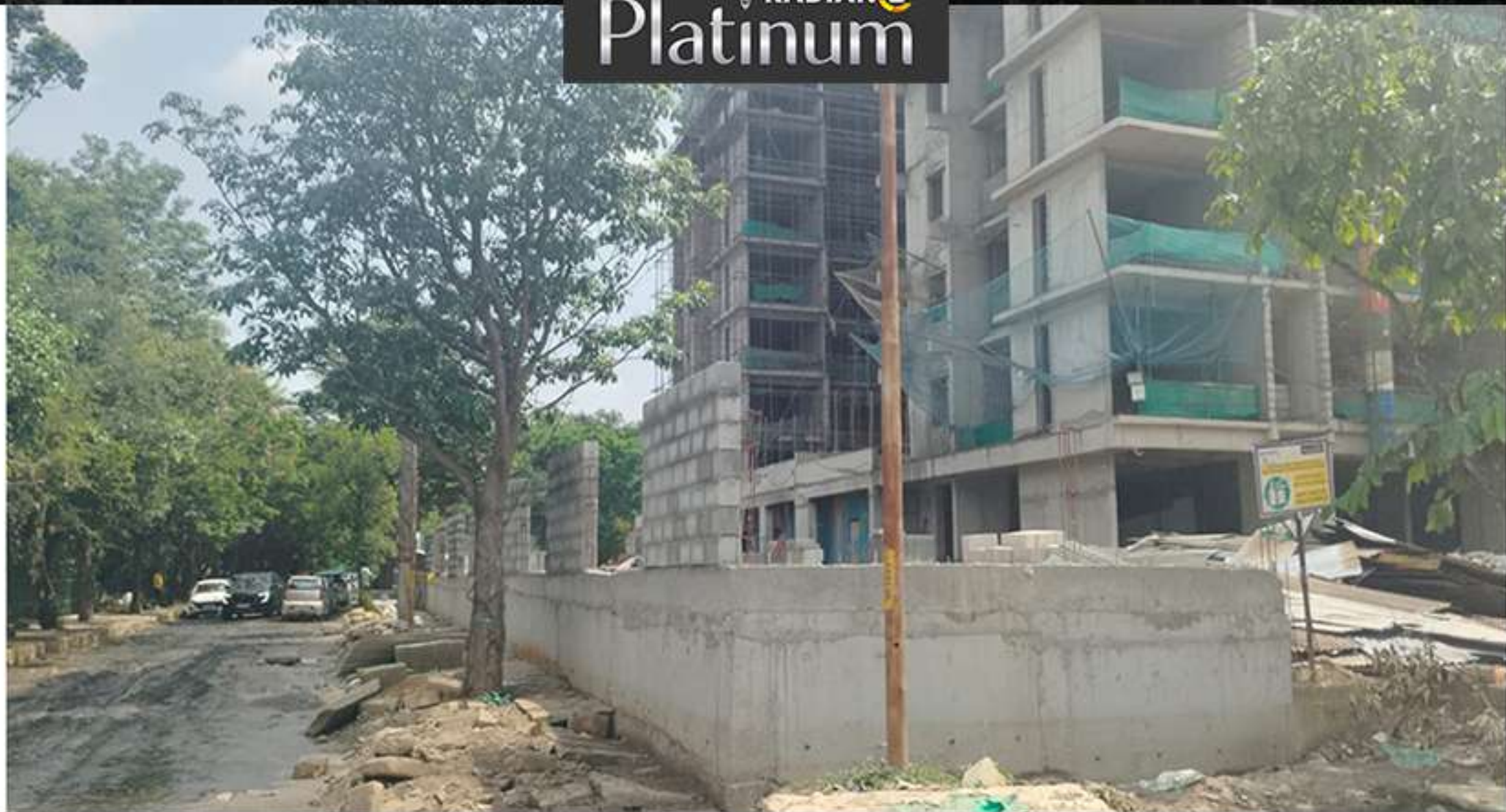
Compound Wall - East Side
