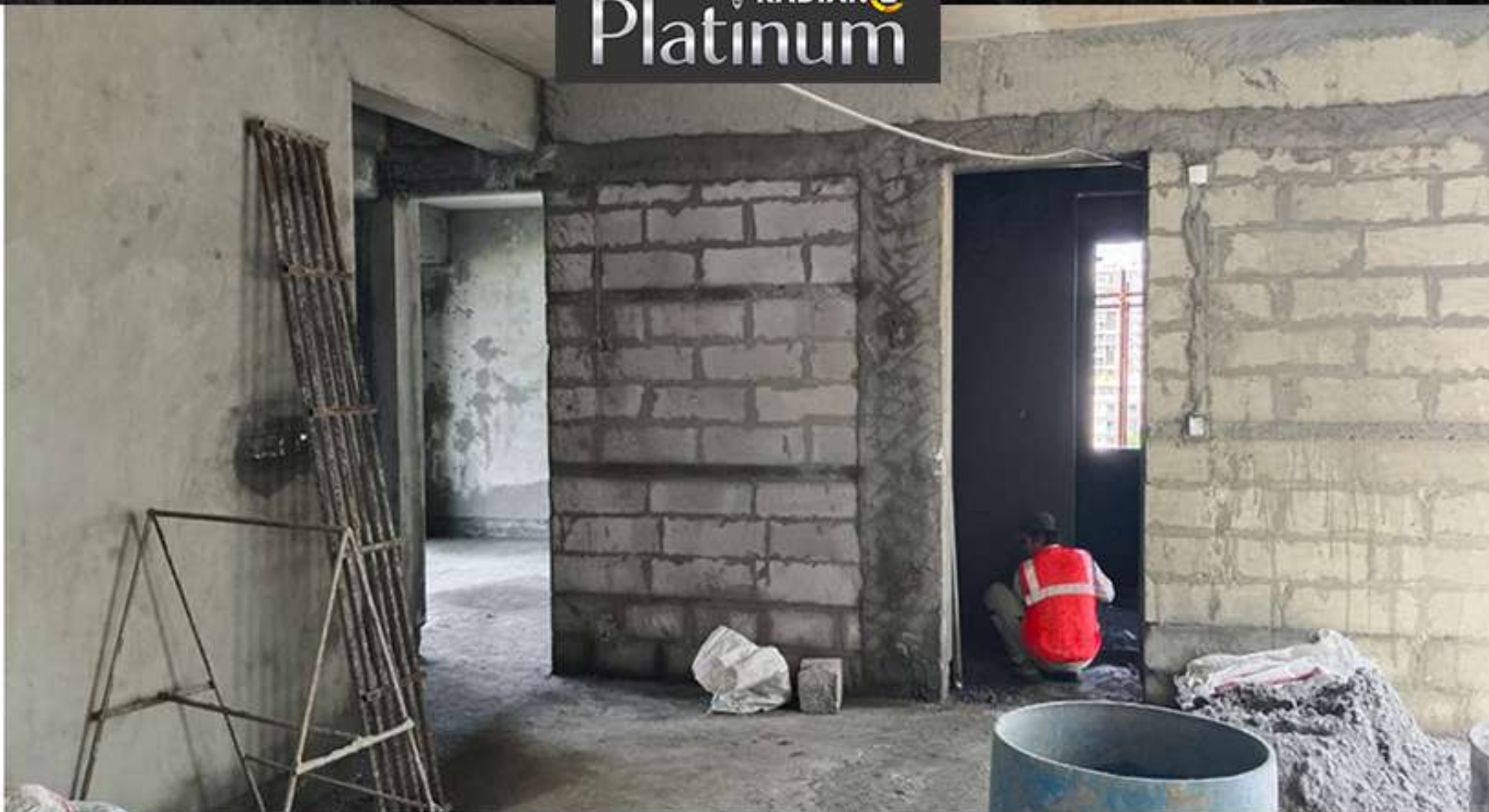
6th Floor Internal Wall Plastering Work
