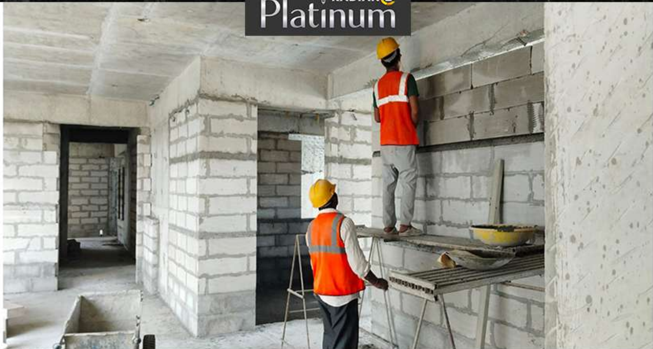
9th Floor Block Work
