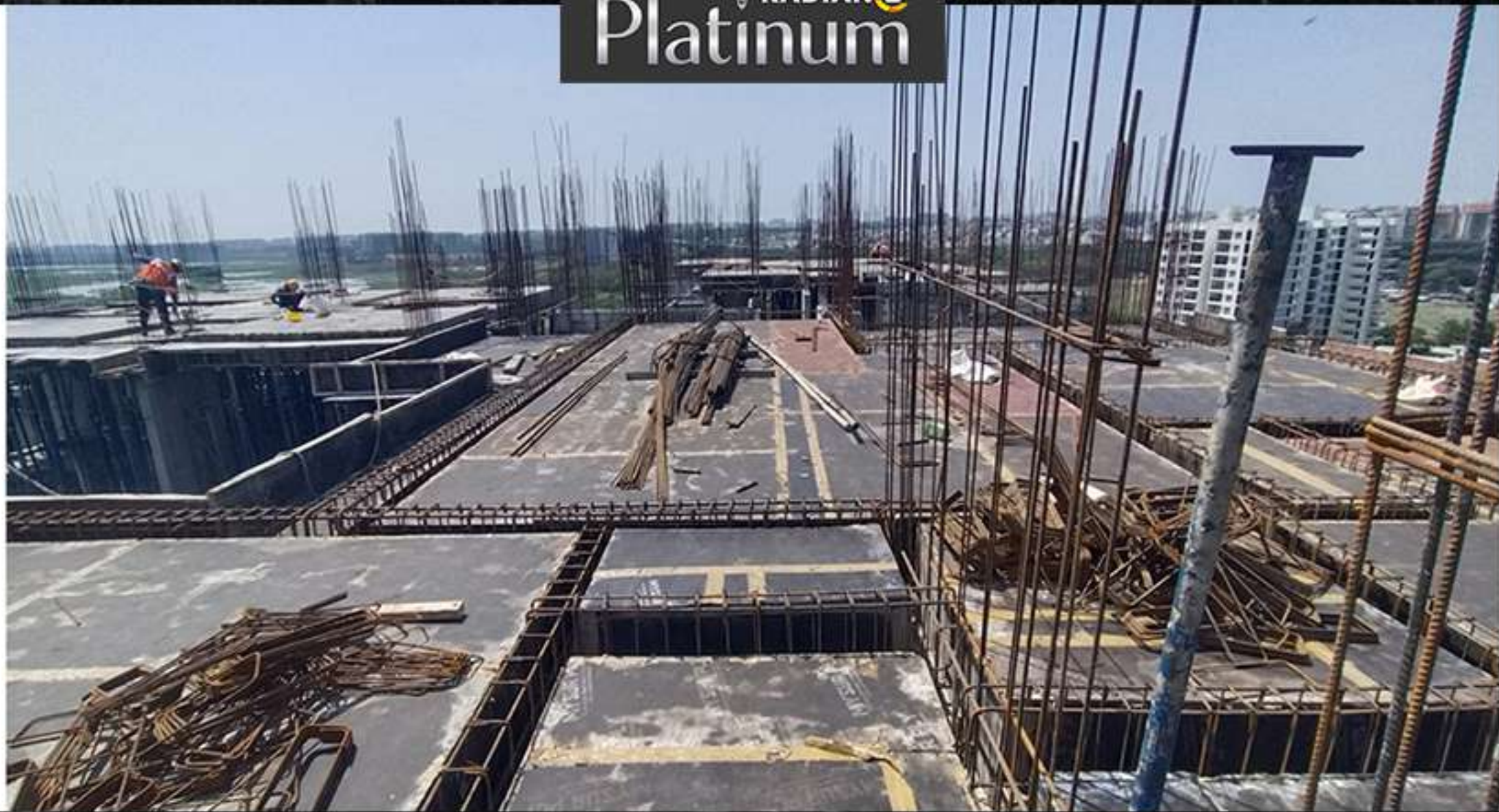
Block B - 12th Floor Roof Slab Work
