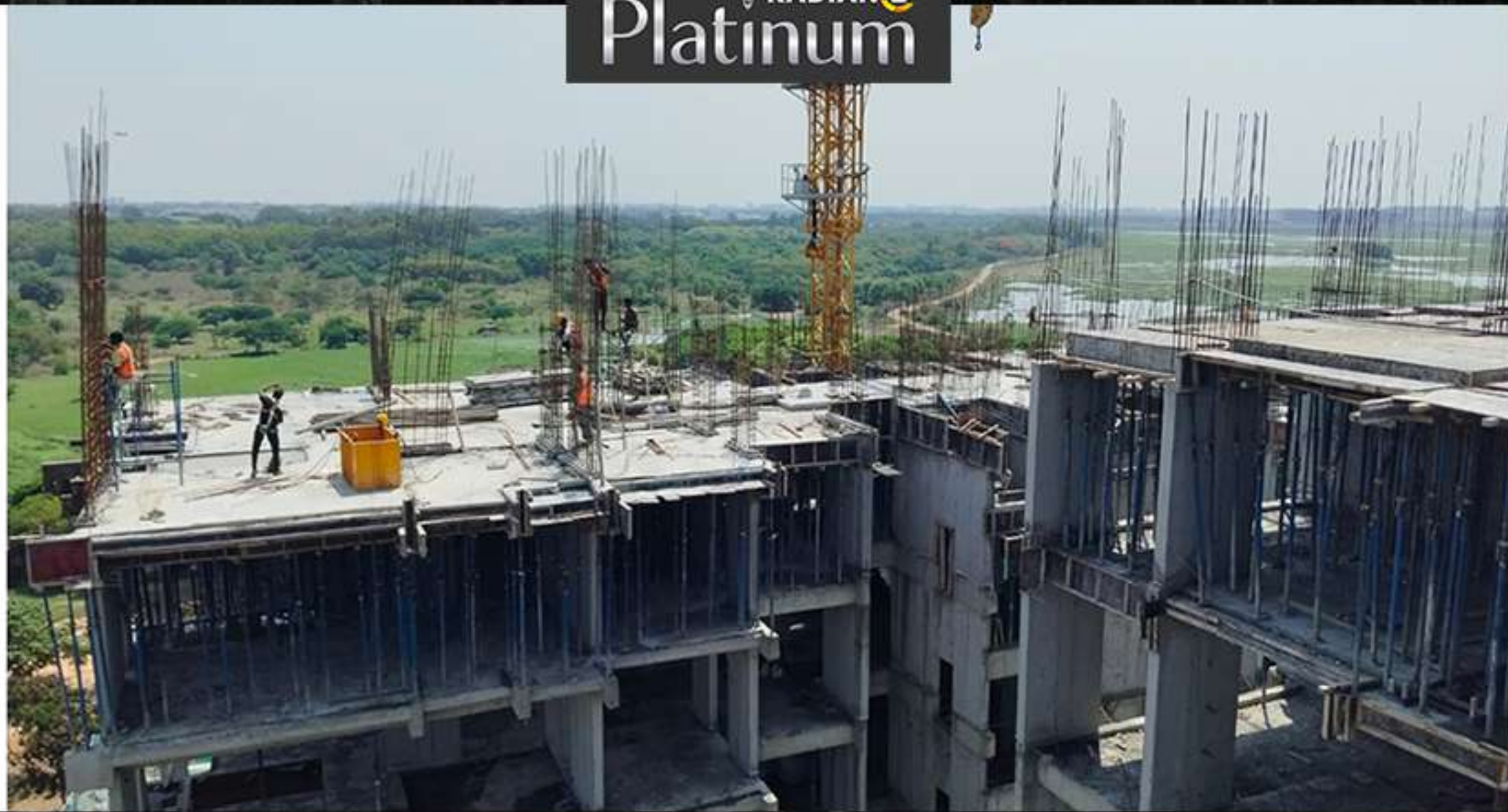
Block A - 12th Floor Column Concrete Work
