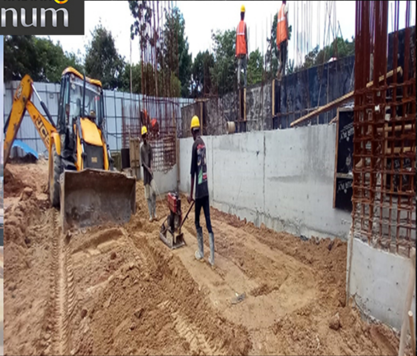
SOIL COMPACTING - MECHANICAL
