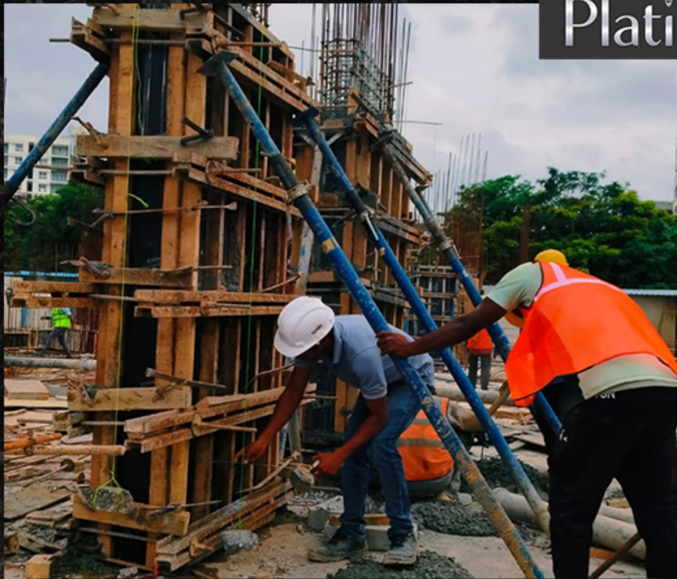
PRE CHECKING - COLUMN SHUTTERING
