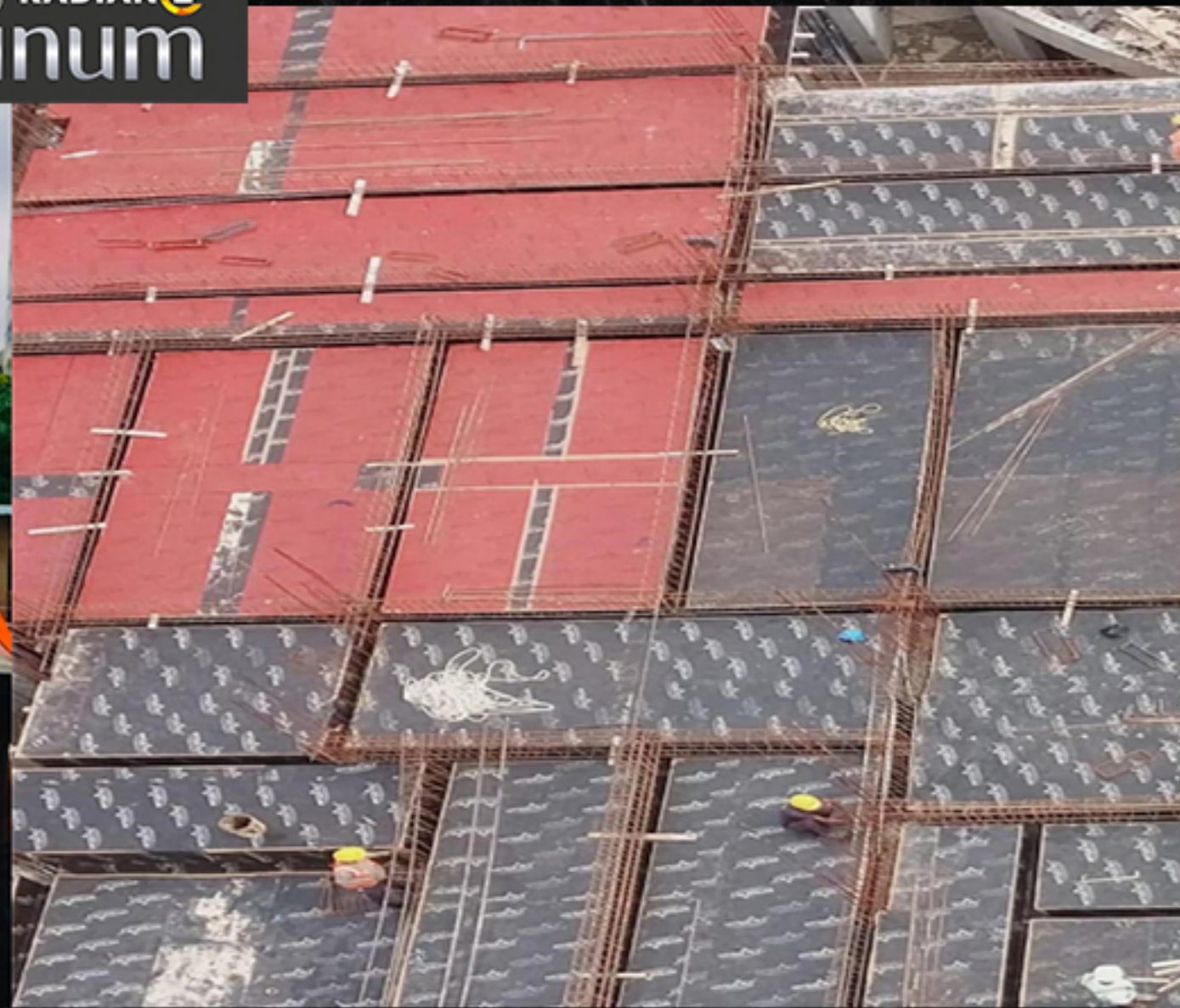
USING NEW PLY BOARD
