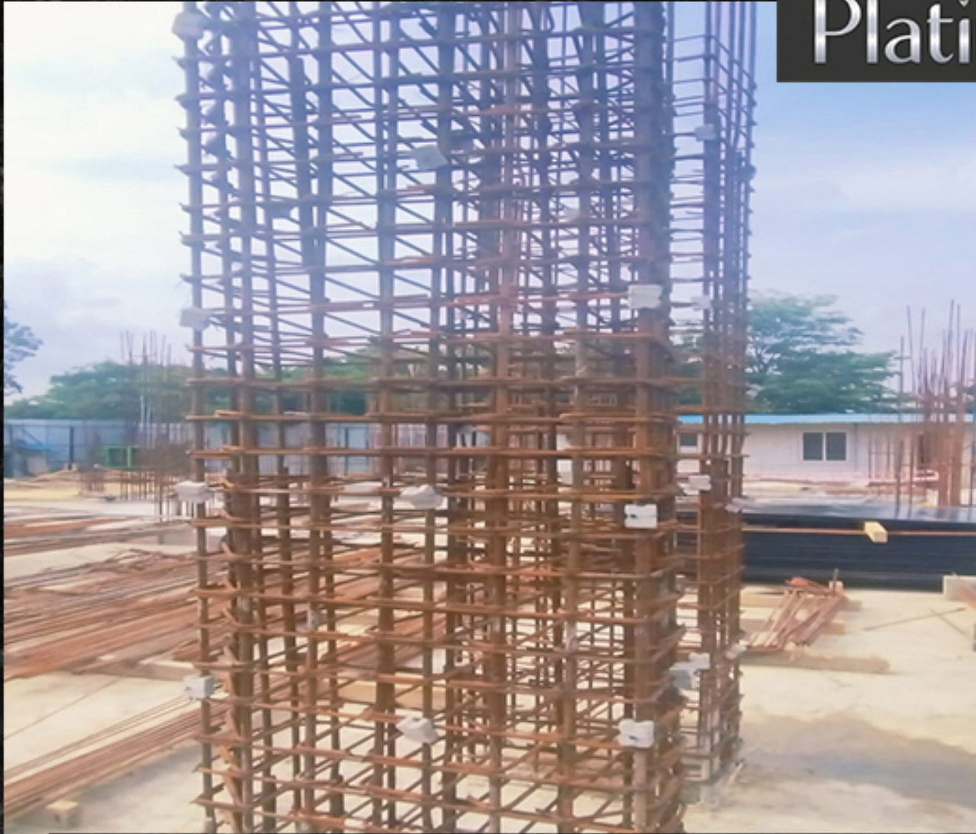
USING CONCRETE COVER BLOCK
