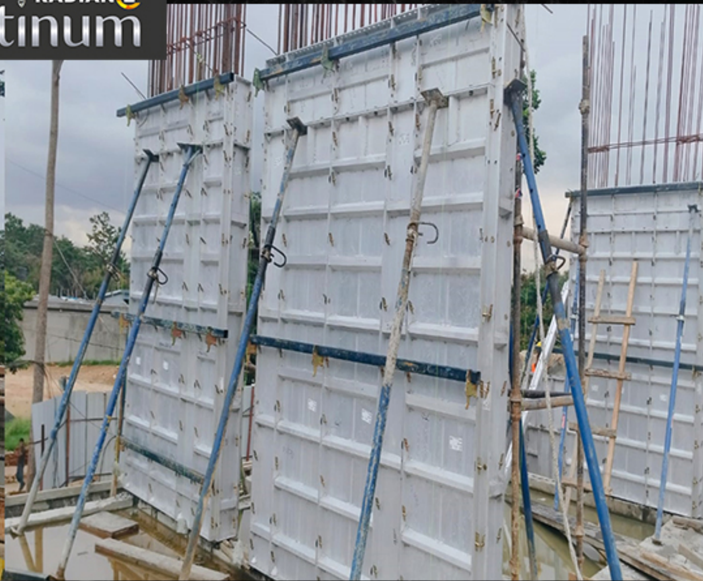
USING ALUMINIUM FORMWORK - COLUMN
