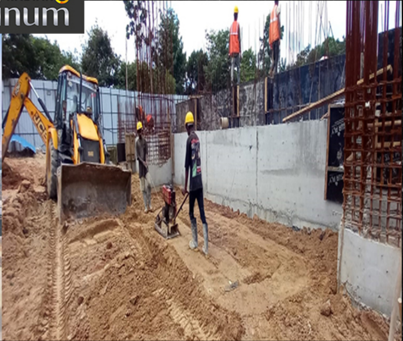
SOIL COMPACTING - MECHANICAL
