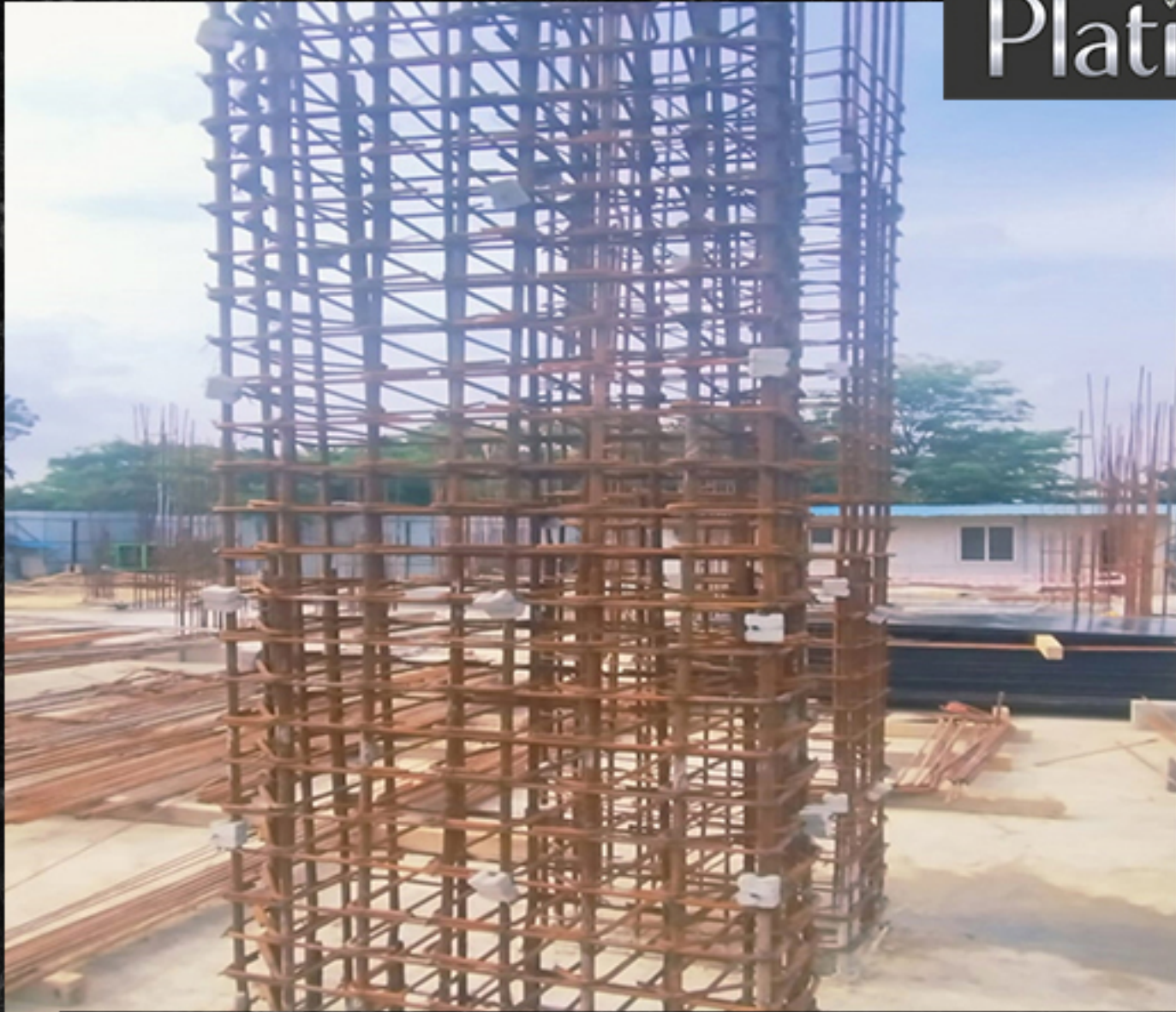
USING CONCRETE COVER BLOCK
