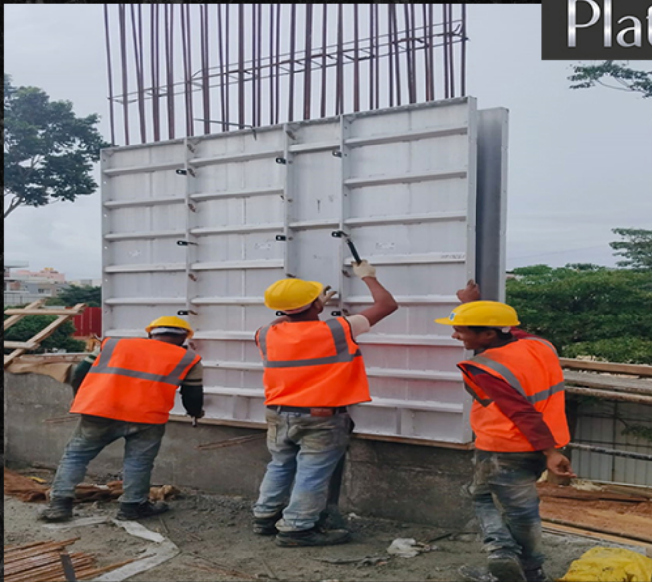
USING ALUMINIUM FORMWORK - COLUMN
