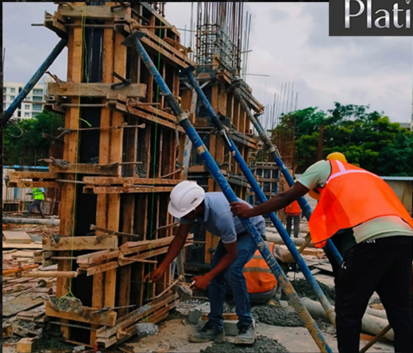
PRE CHECKING - COLUMN SHUTTERING
