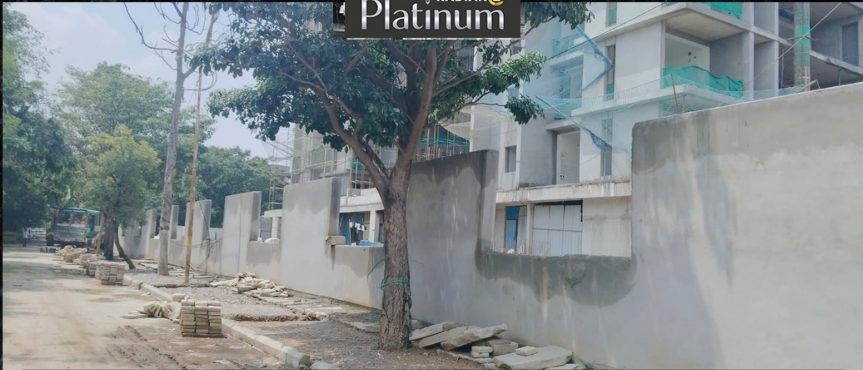
Compound Wall - East Side
