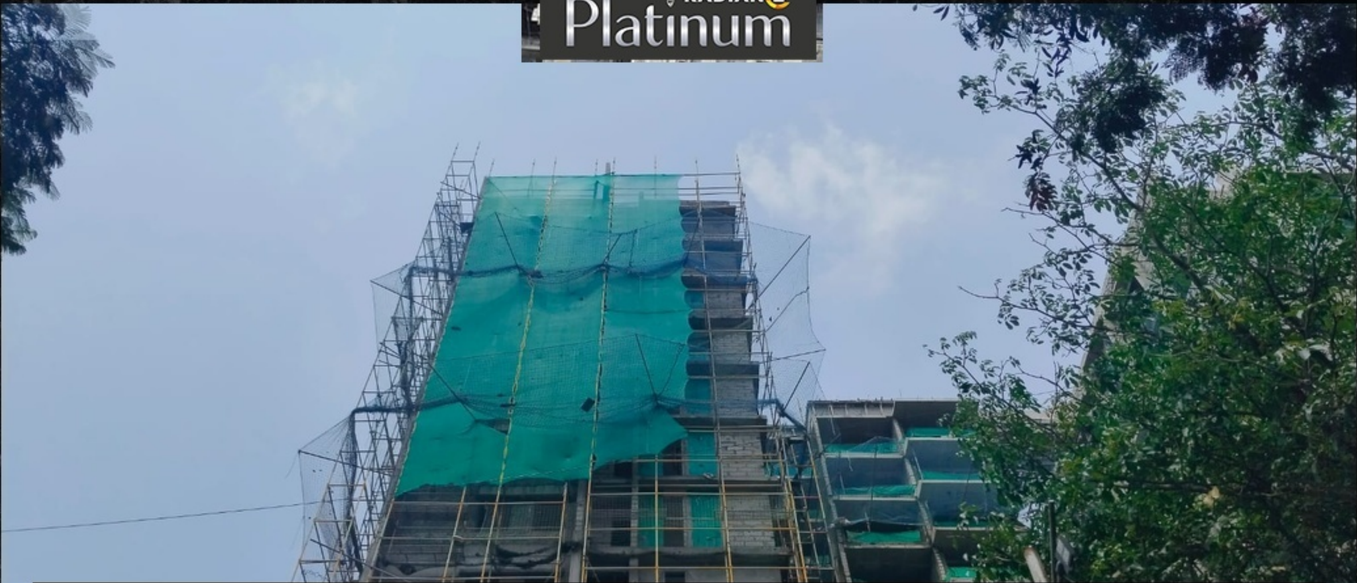
Block - B - External Plastering Work - South & East, Above the 6th Floor
