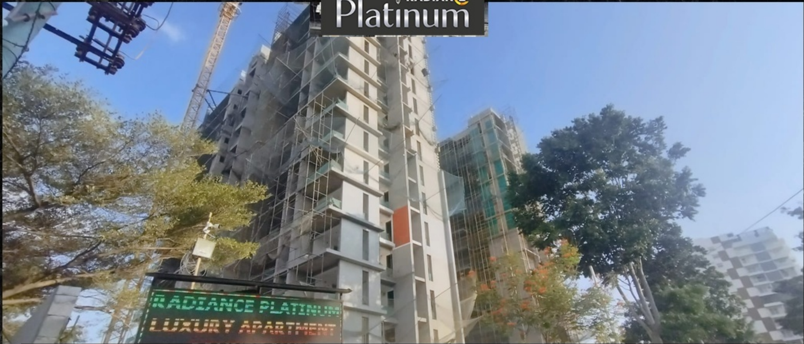
North West Corner View
