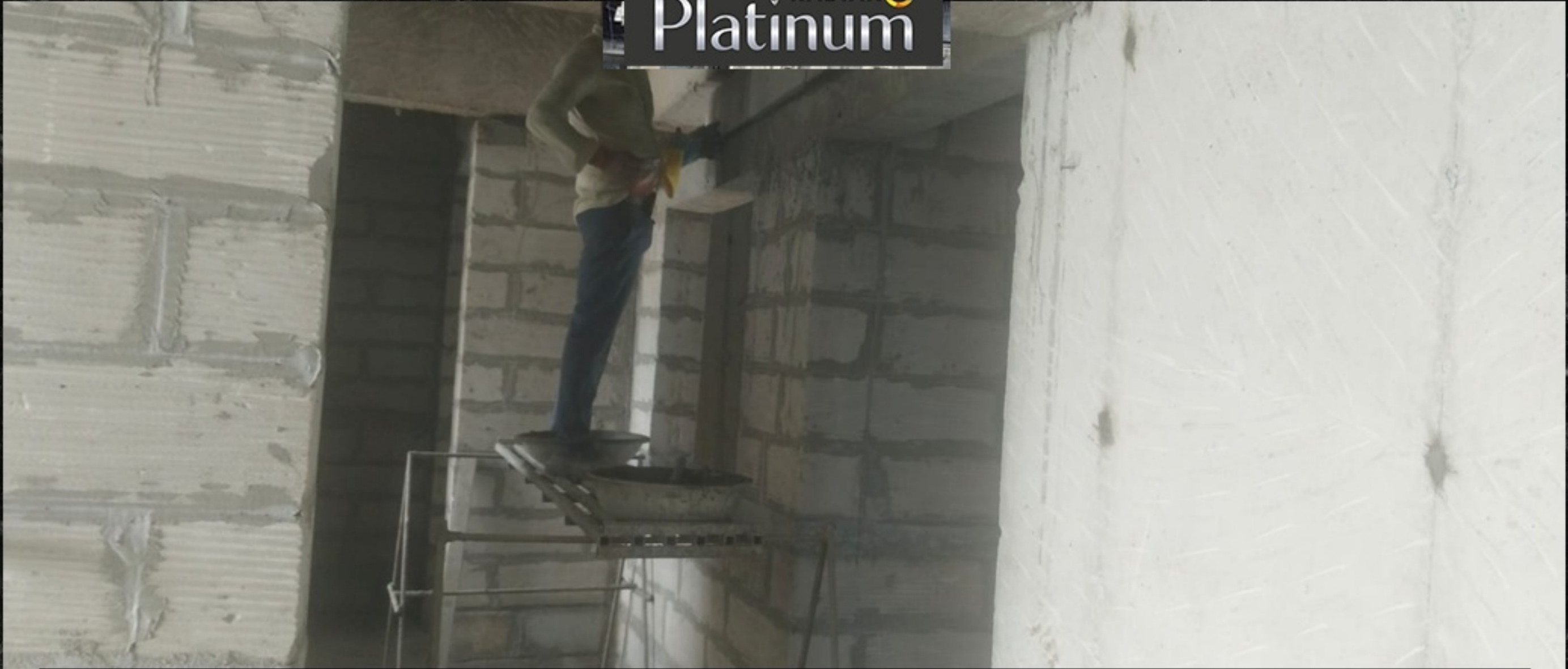
13th Floor Block Work
