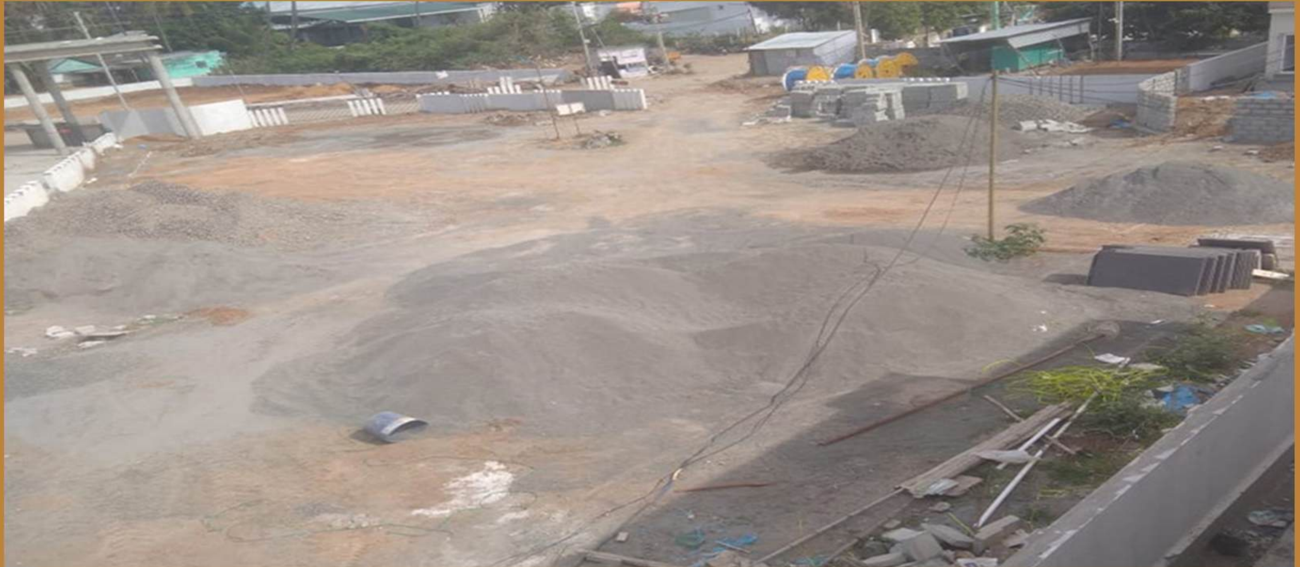
OSR – 2 COMPOUND WALL GRILL WORK IN PROGRESS
