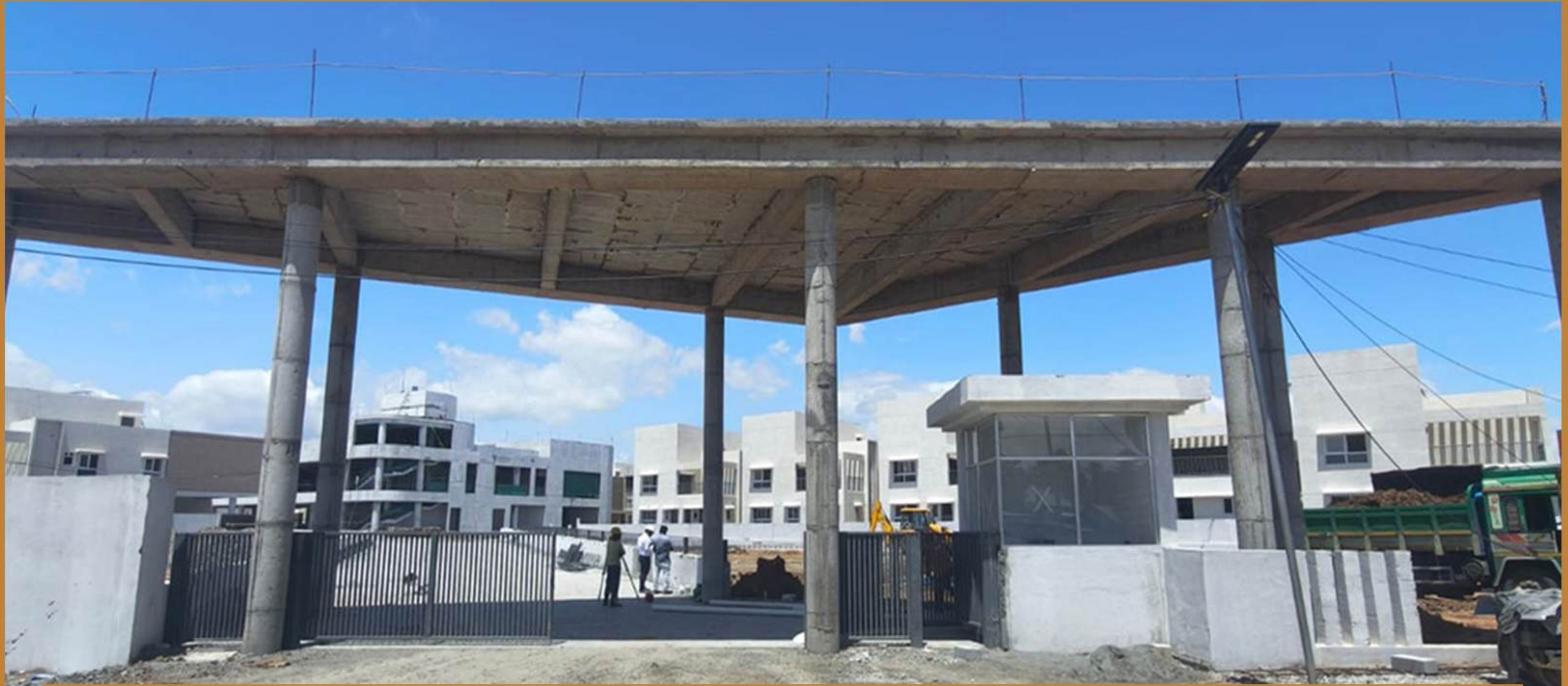
ENTRY PORTAL GATE FIXING WORK COMPLETED
