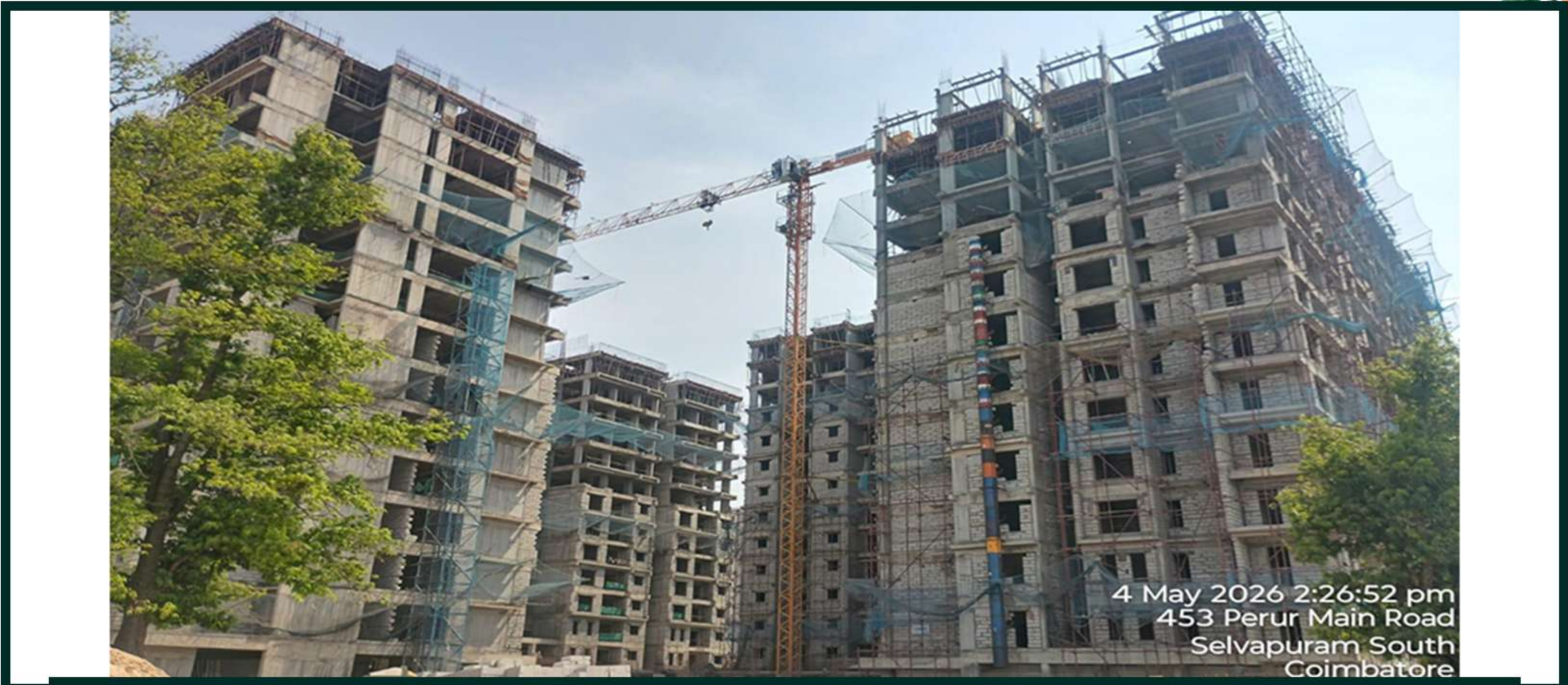
Site Over All Progress View
