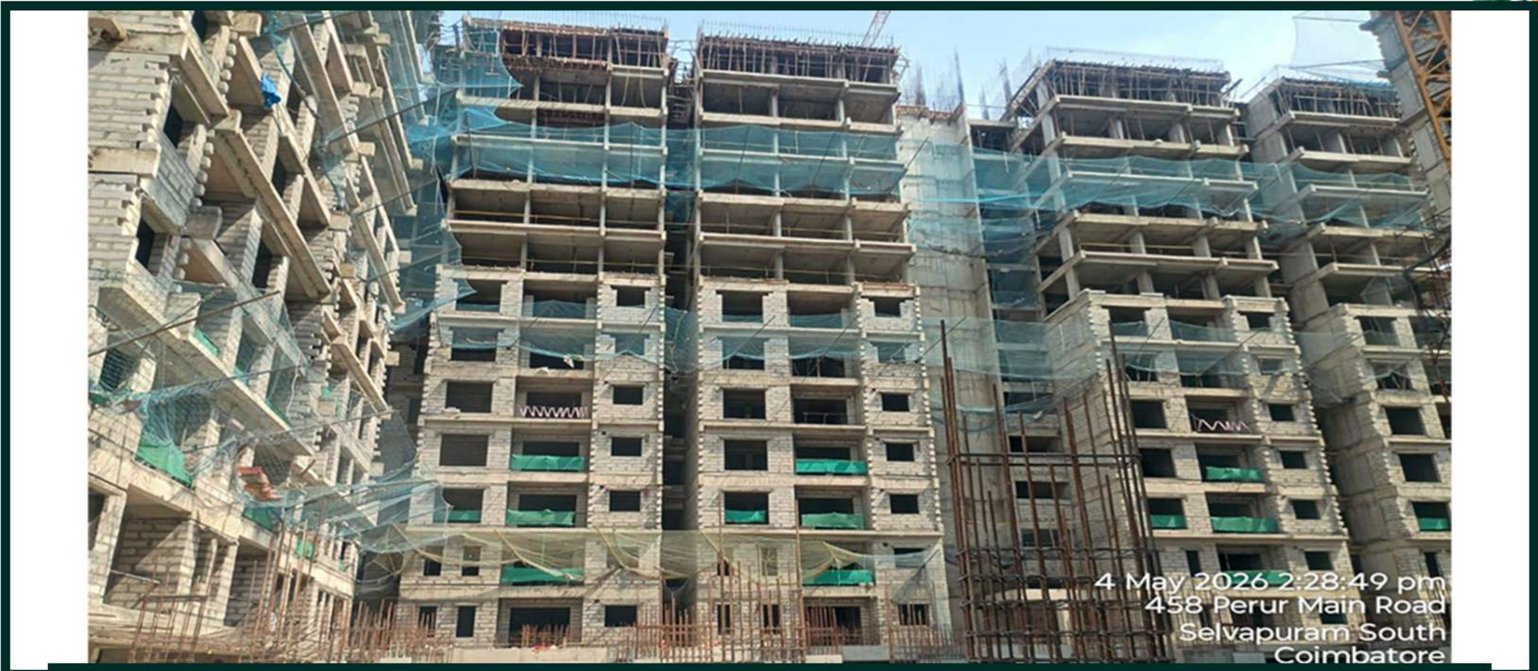
Site Over All Progress View-tower-2 Podium View
