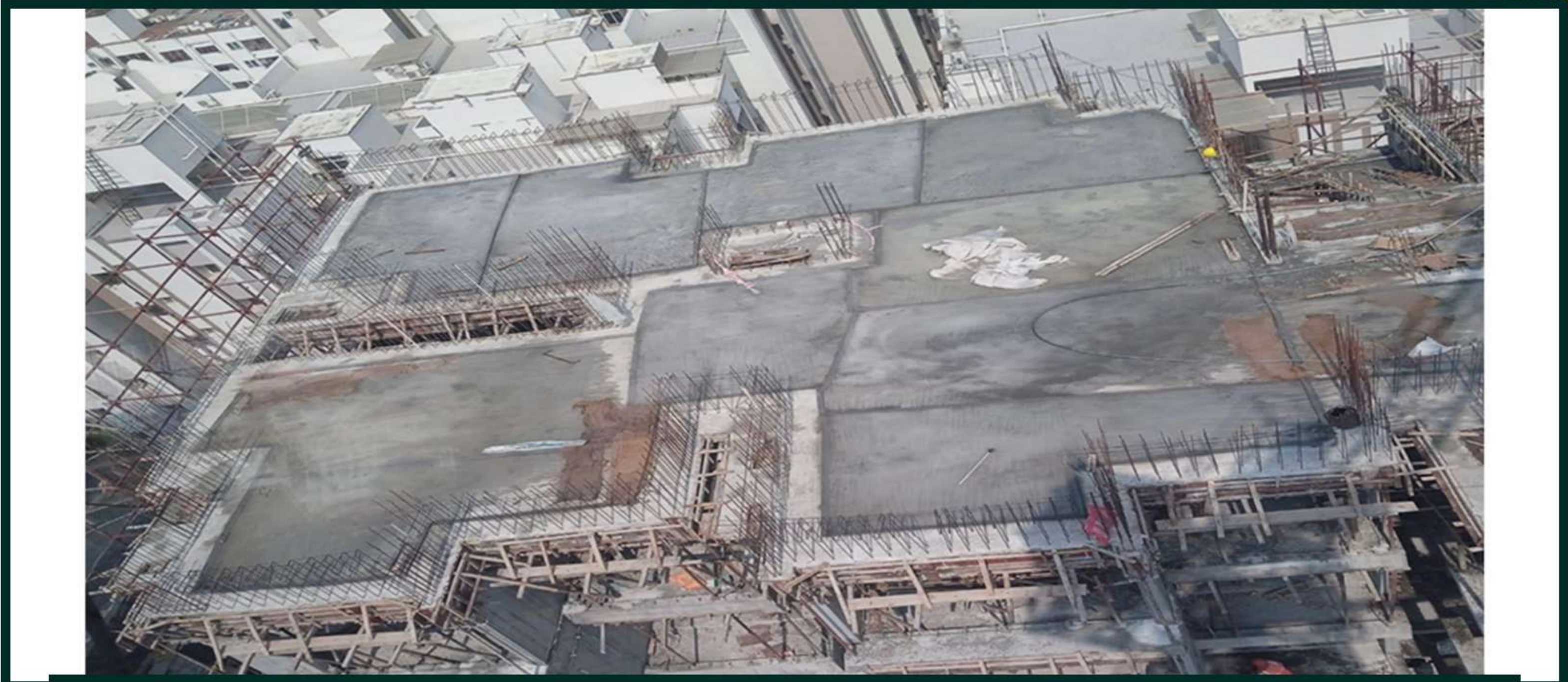
Tower-2 Pour -4 13th Floor Roof Slab Completed
