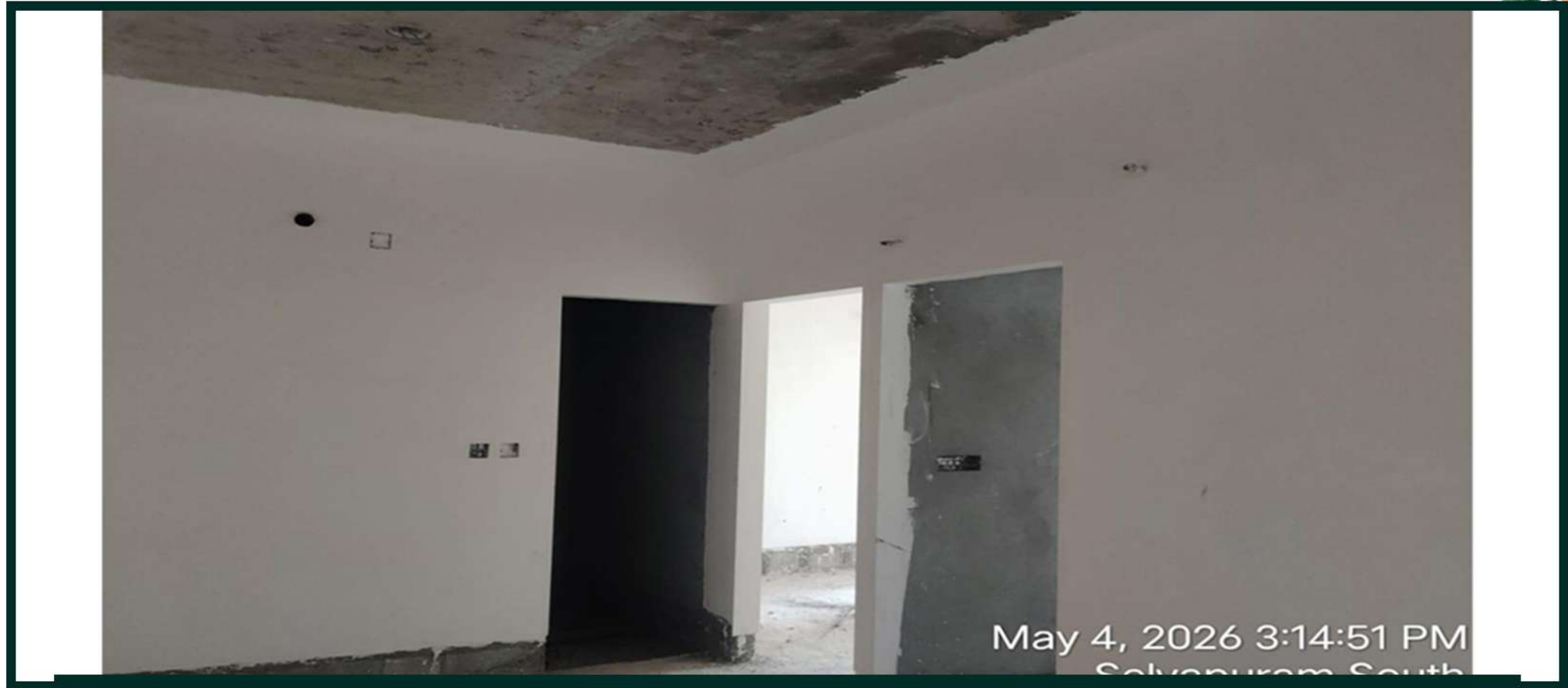
Tower 1 Floor 1 Gypsum Plastering Work In Progress
