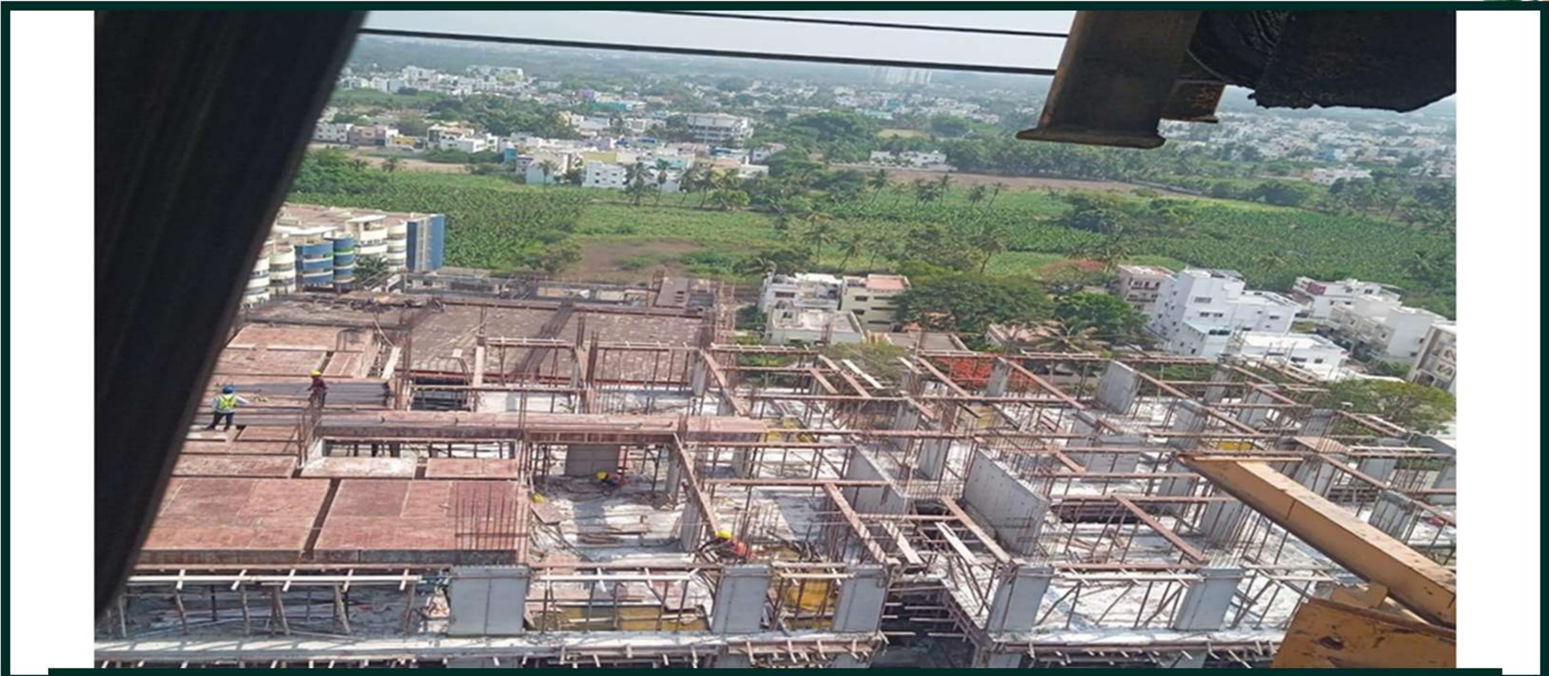
Tower-1 Pour-6 13th Floor Roof Slab Reinforcement Work In Progress
