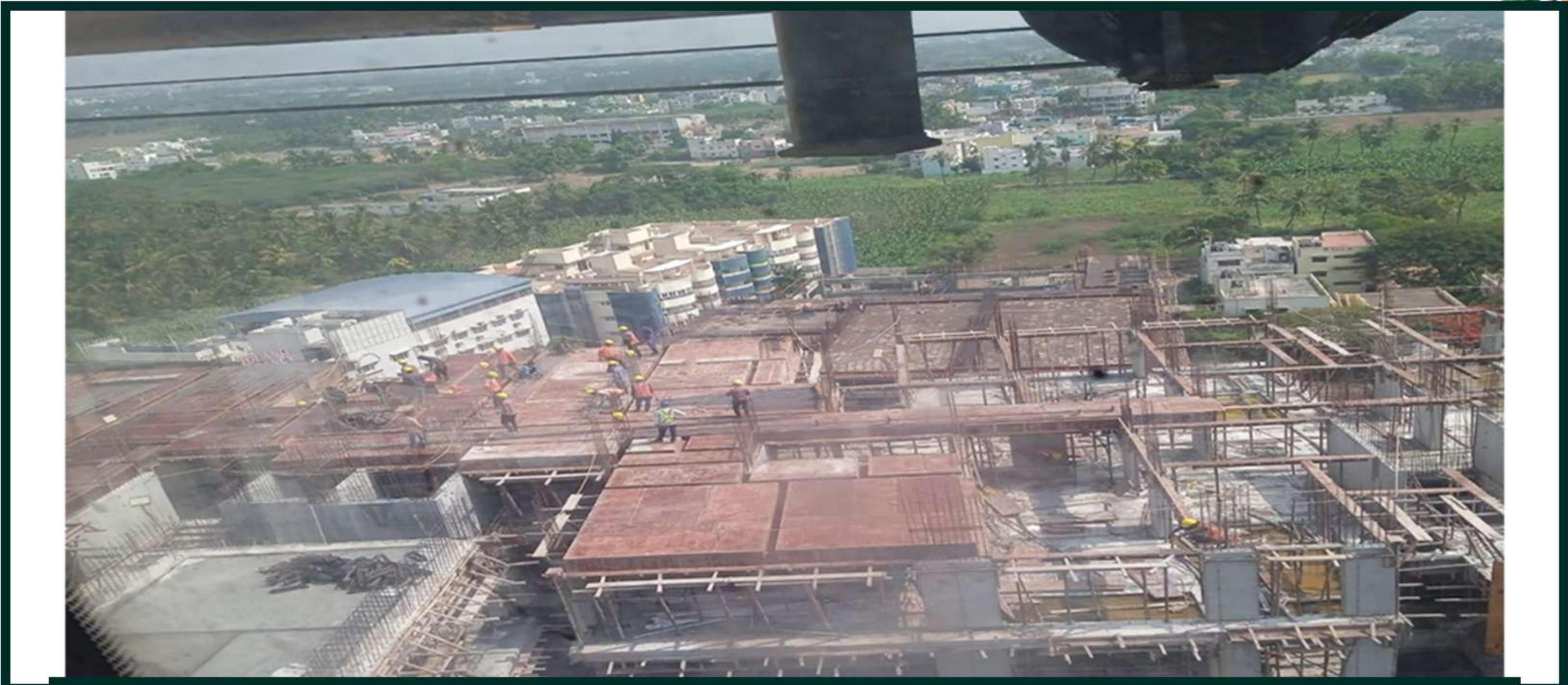
Tower-1 Pour-5 13th Floor Roof Slab Reinforcement Work In Progress
