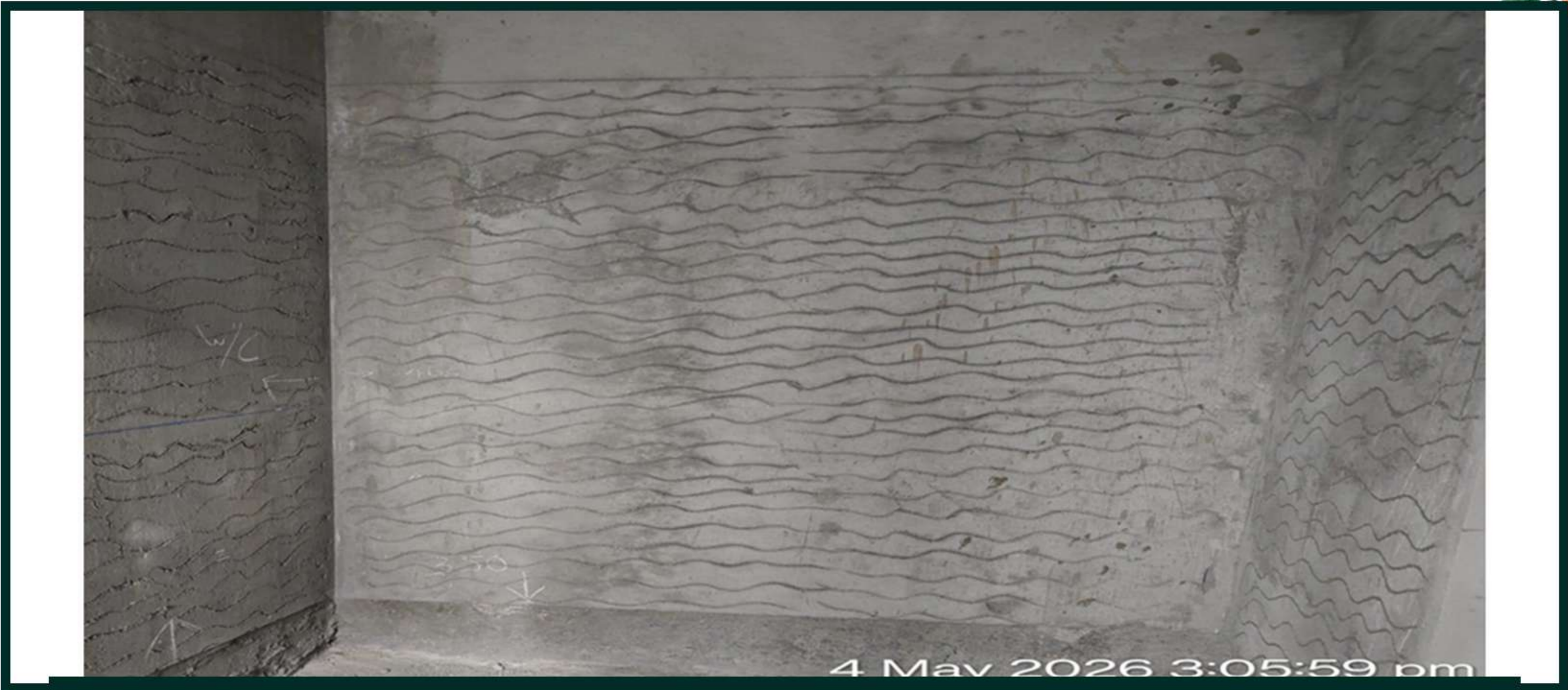
Tower 2 Floor 1 Plastering Work In Progress
