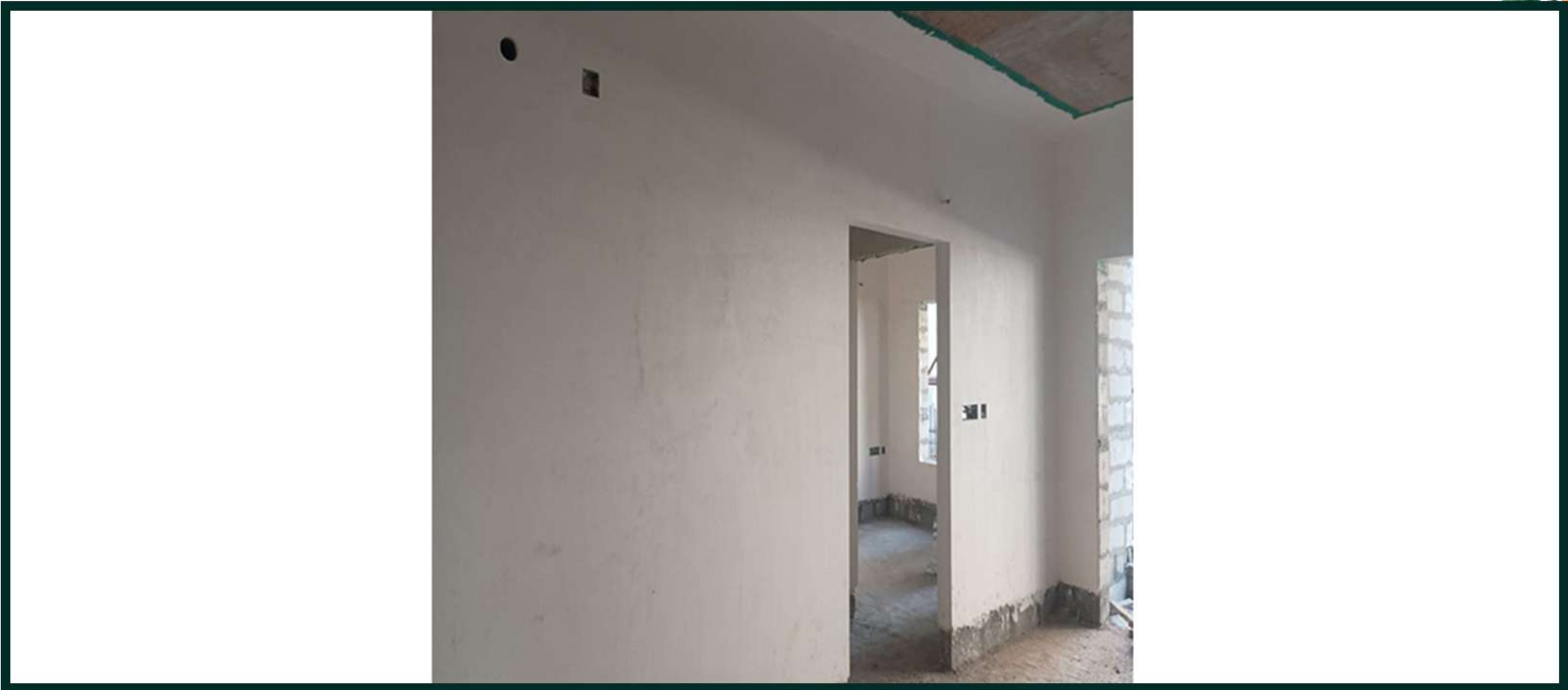
Tower 1 Gypsum Plastering 6th Floor Work In Progress
