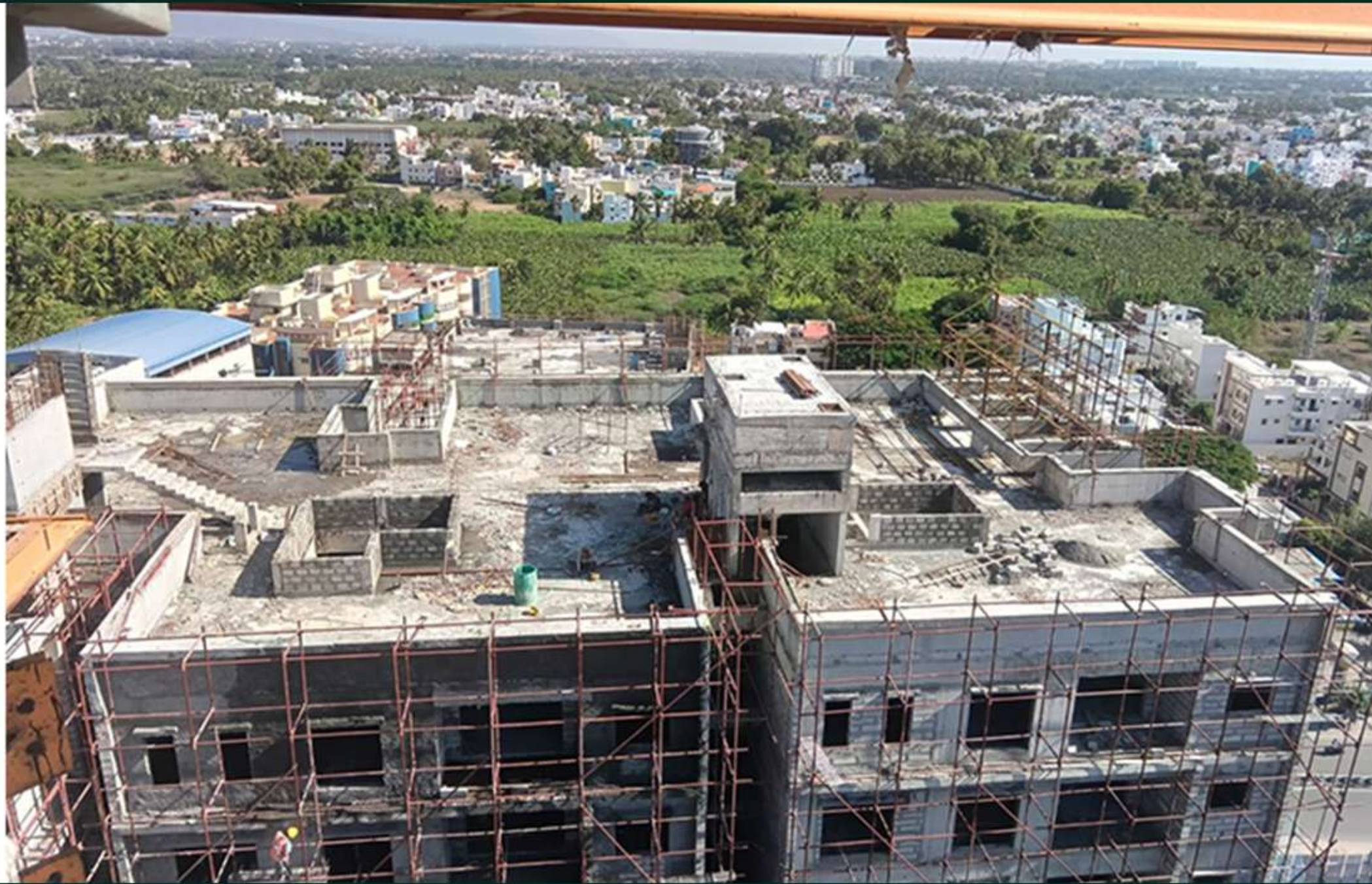
Tower-1 Pour-6 Terrace Floor Water Tank Slab Concrete Work Completed
