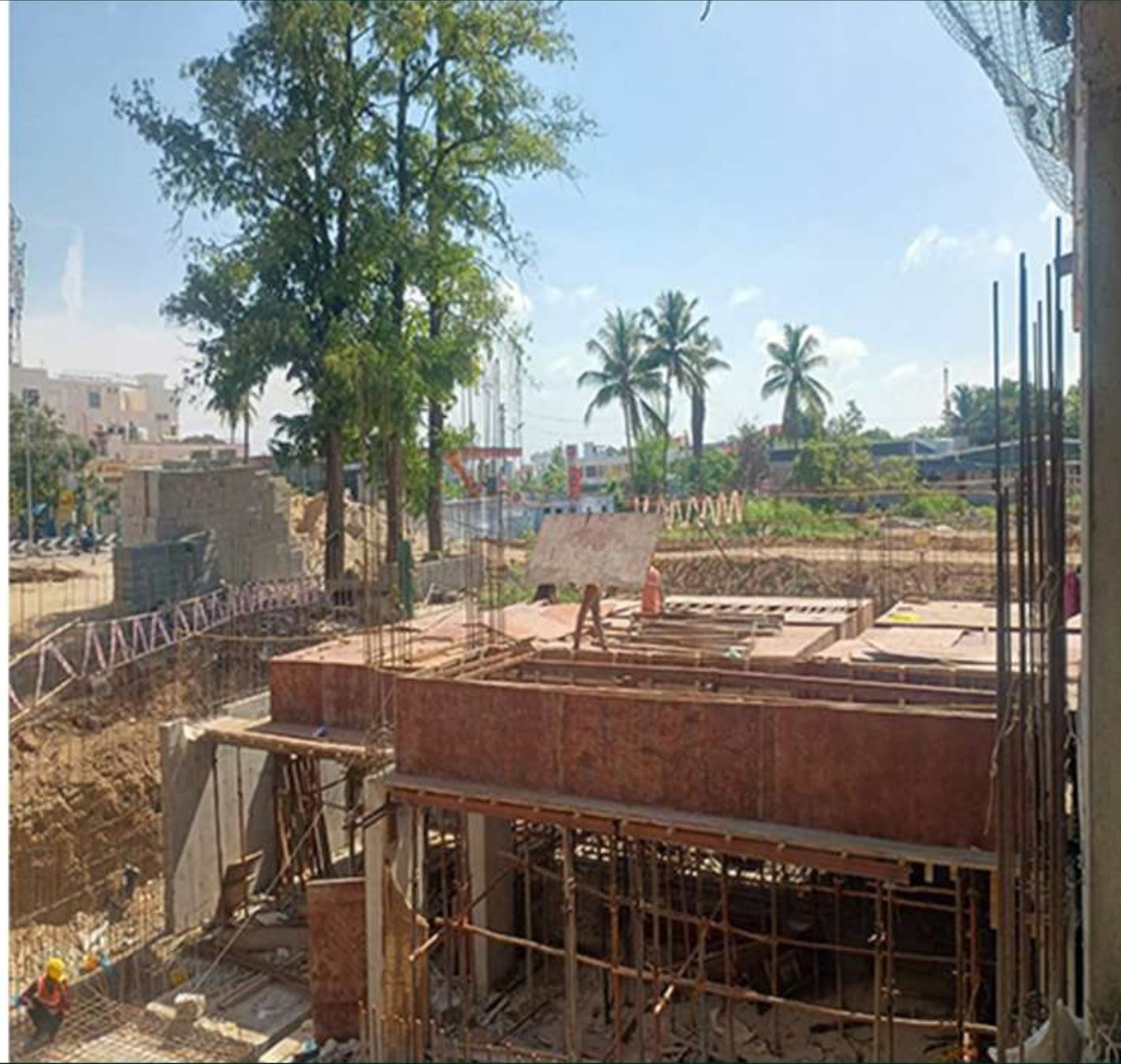
Club House Basement Slab Shuttering Work In Progress
