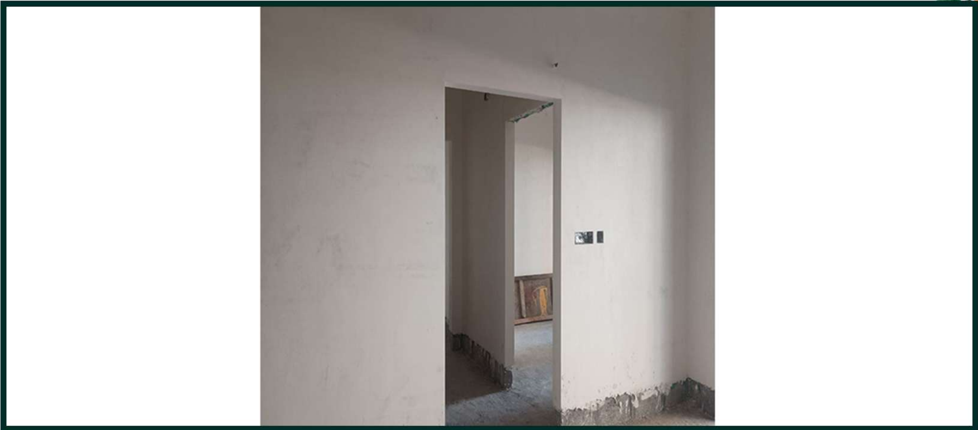
Tower 2 Gypsum Plastering 3rd Floor Work In Progress
