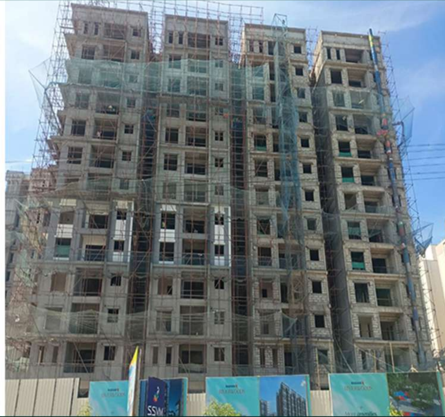
Site Over All Progress View-Tower-1
