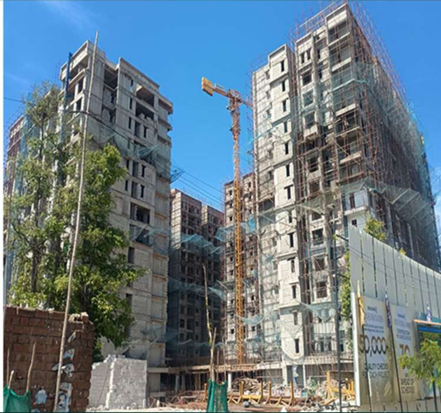
Site Over All Progress View
