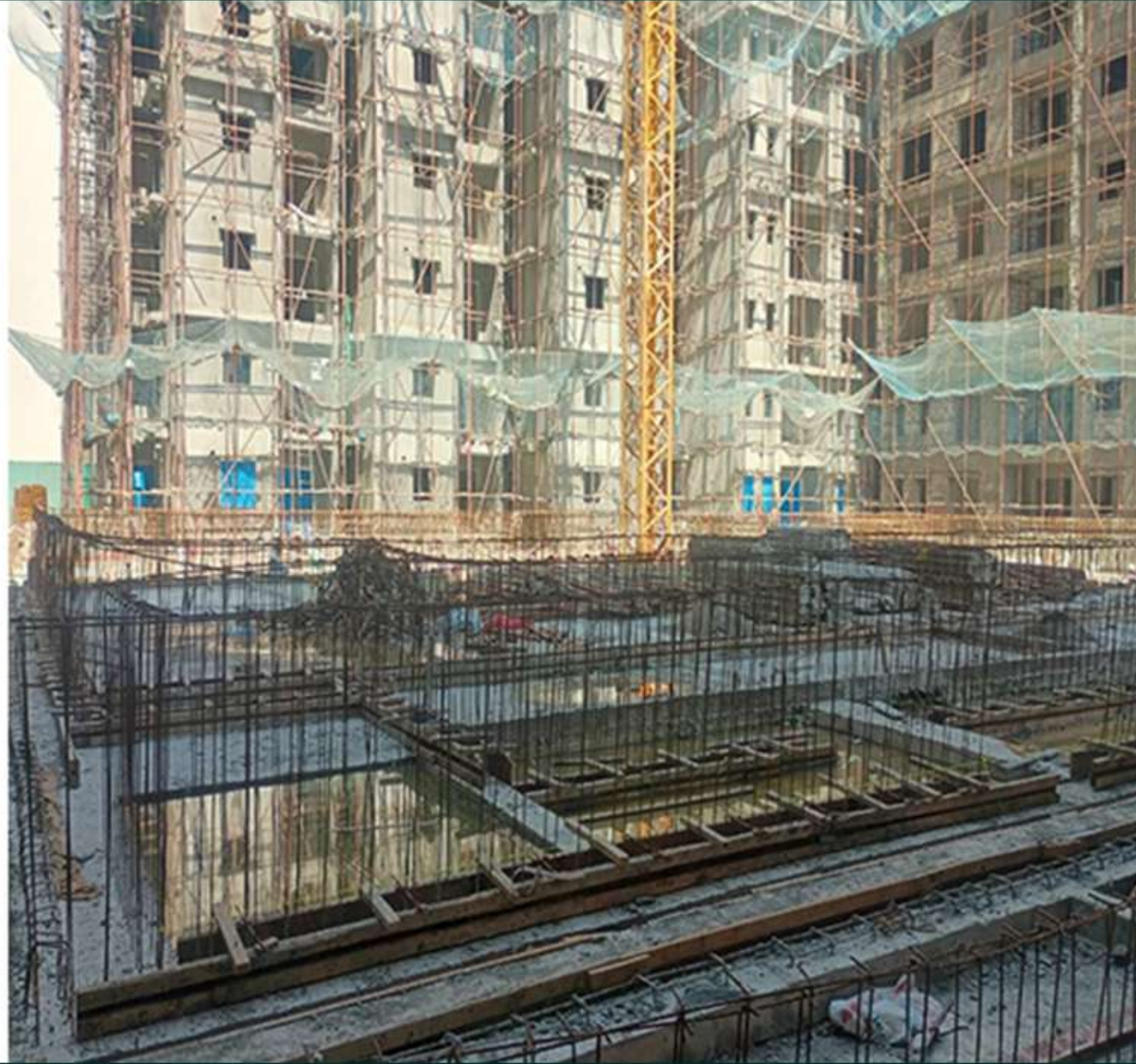
Swimming Pool Wall Starter Work In Progress
