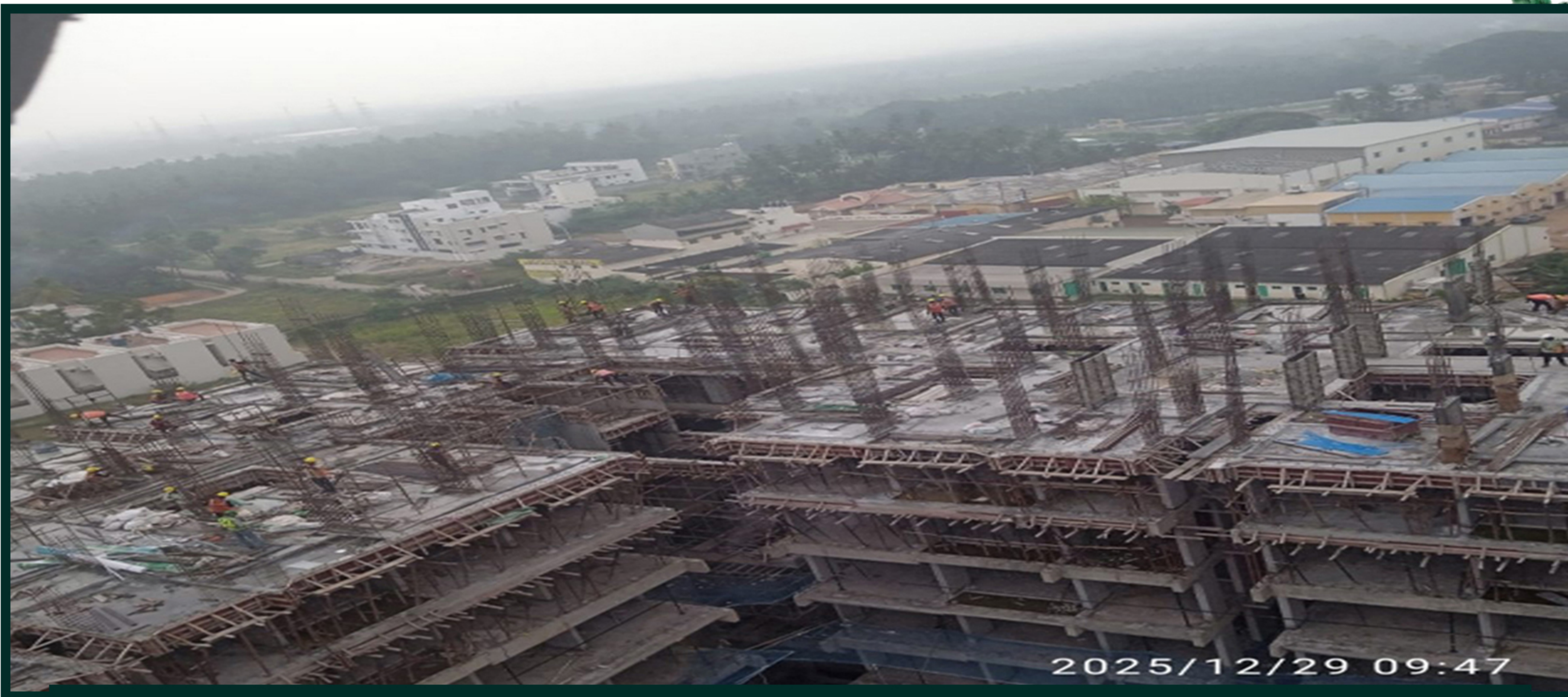
Tower-2 pour -2 10th floor column reinforcement work in progress – top view.
