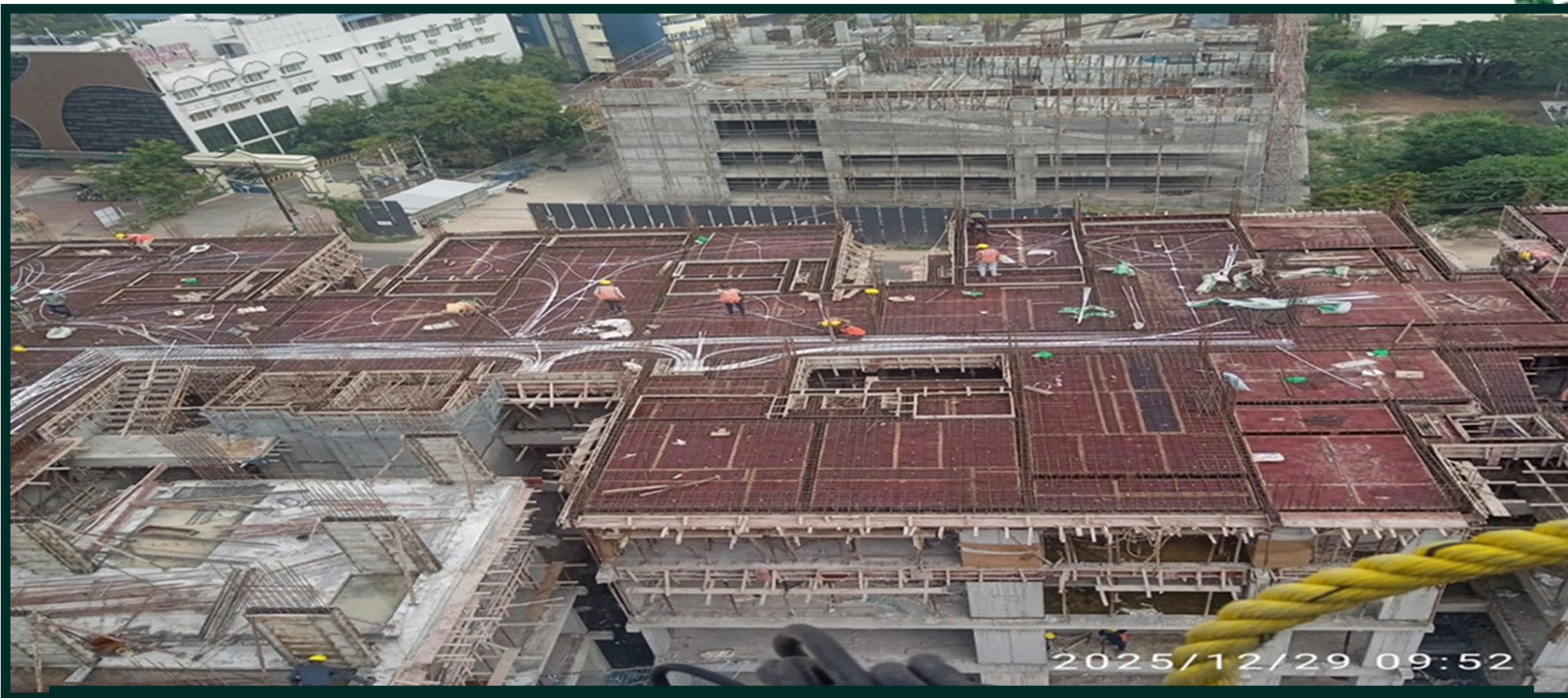
Tower-1 pour-5 8th floor roof slab reinforcement work in progress – top view.
