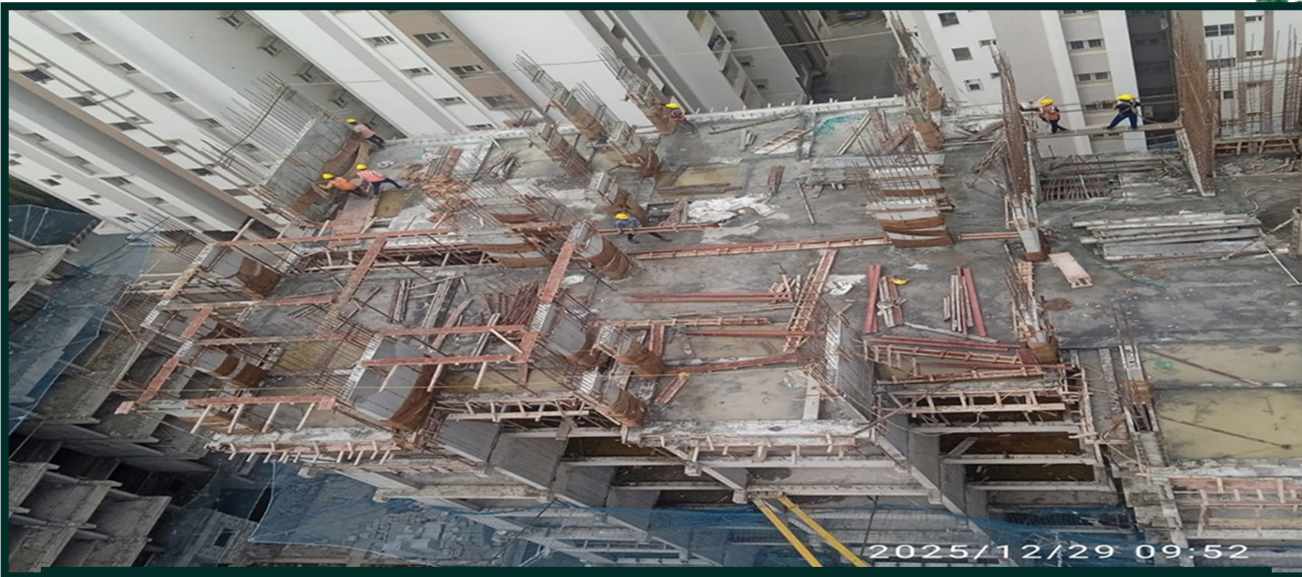
Tower-1 pour-4 9th floor column work in progress – top view.
