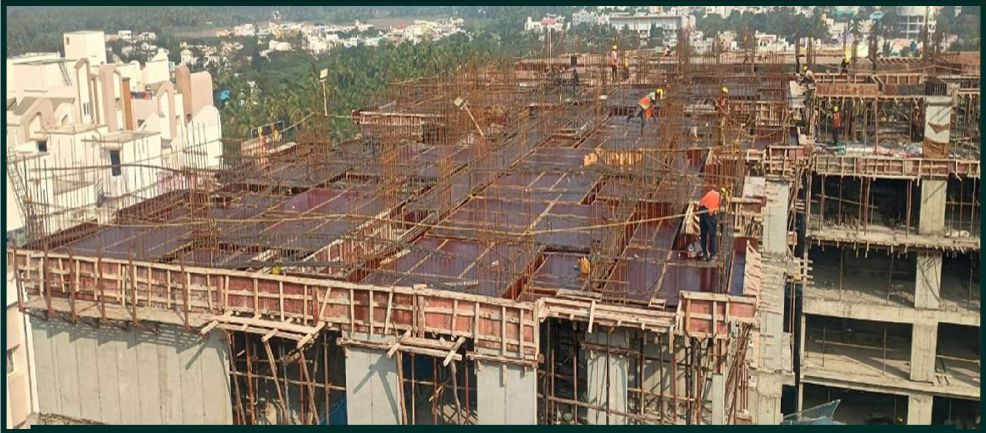
TOWER-1 POUR-4 10TH FLOOR ROOF BEAM REINFORCEMENT WORK IN PROGRESS – TOP VIEW
