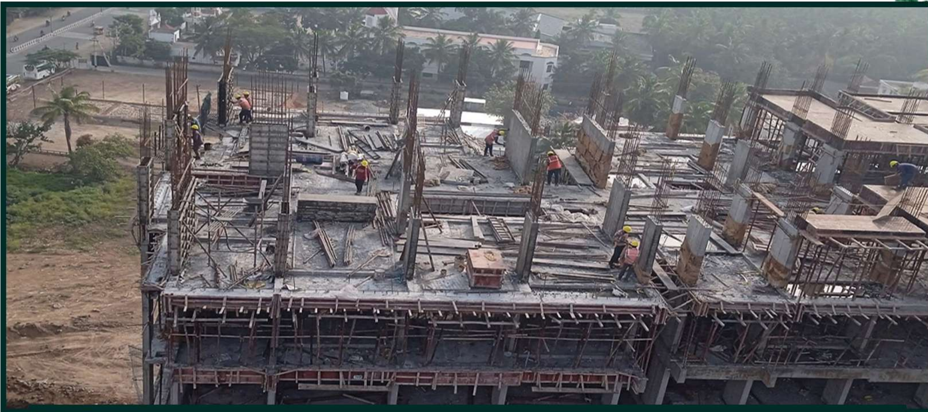
TOWER-2 POUR -3 -11th FLOOR COLUMN WORK IN PROGRESS- TOP VIEW
