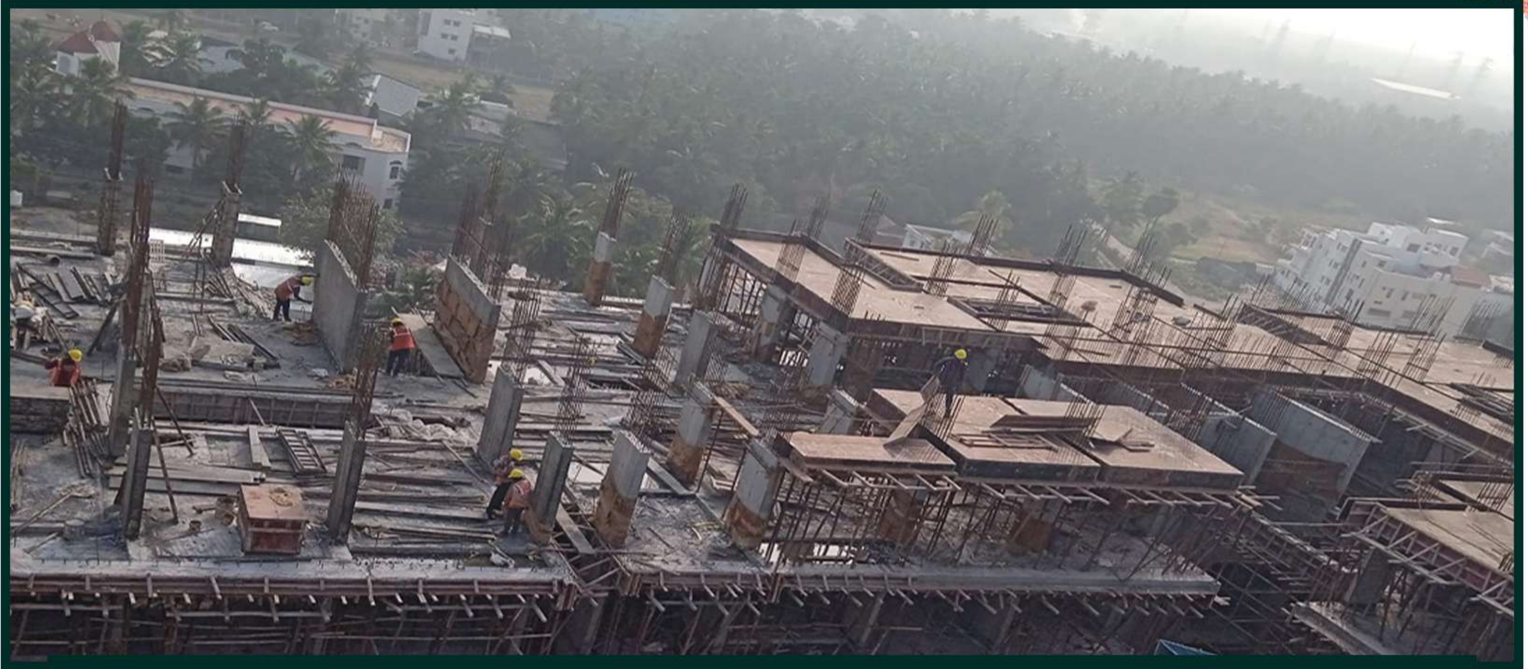
TOWER-2 POUR -2 11TH FLOOR ROOF SLAB SHUTTERING WORK IN PROGRESS – TOP VIEW
