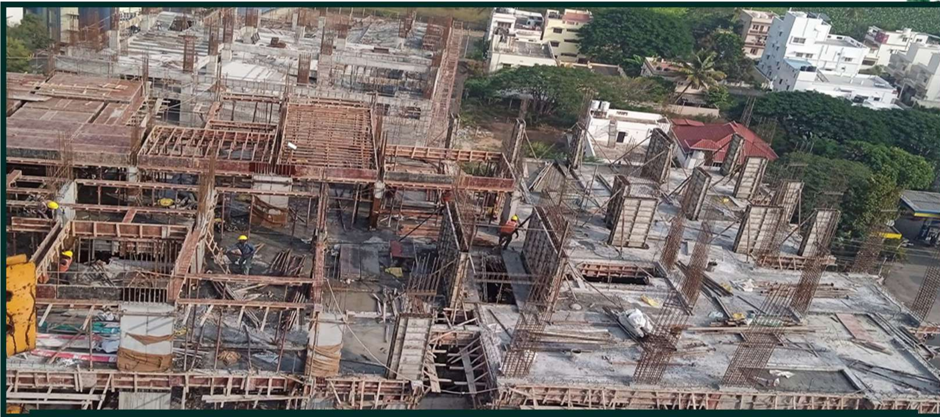
TOWER-1 POUR-6 10th FLOOR COLUMN WORK IN PROGRESS –TOP VIEW
