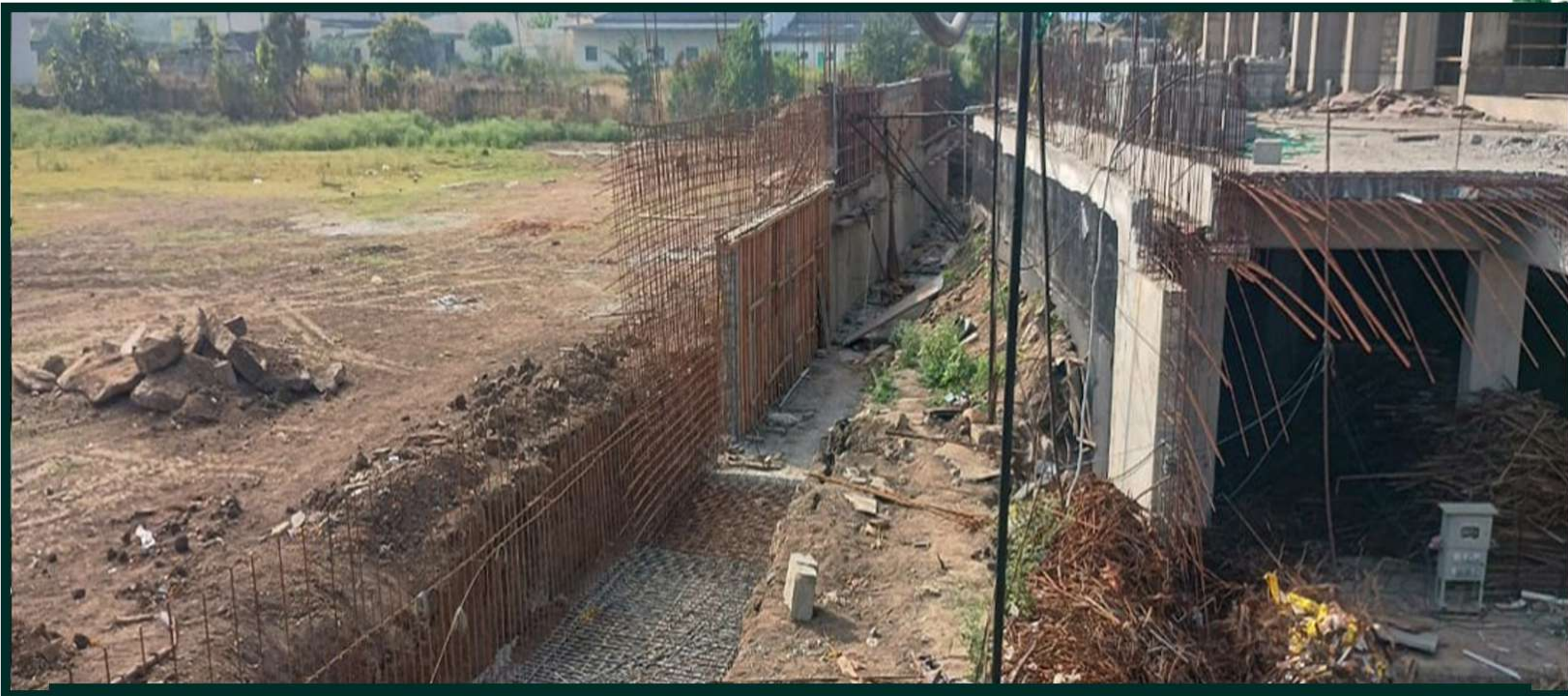
EAST SIDE COMPOUND WALL RC WALL SHUTTERING WORK IN PROGRESS
