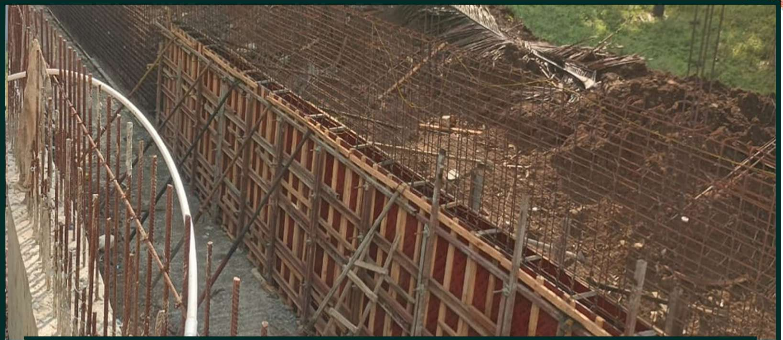
SOUTH SIDE COMPOUND WALL RC WALL SHUTTERING WORK IN PROGRESS
