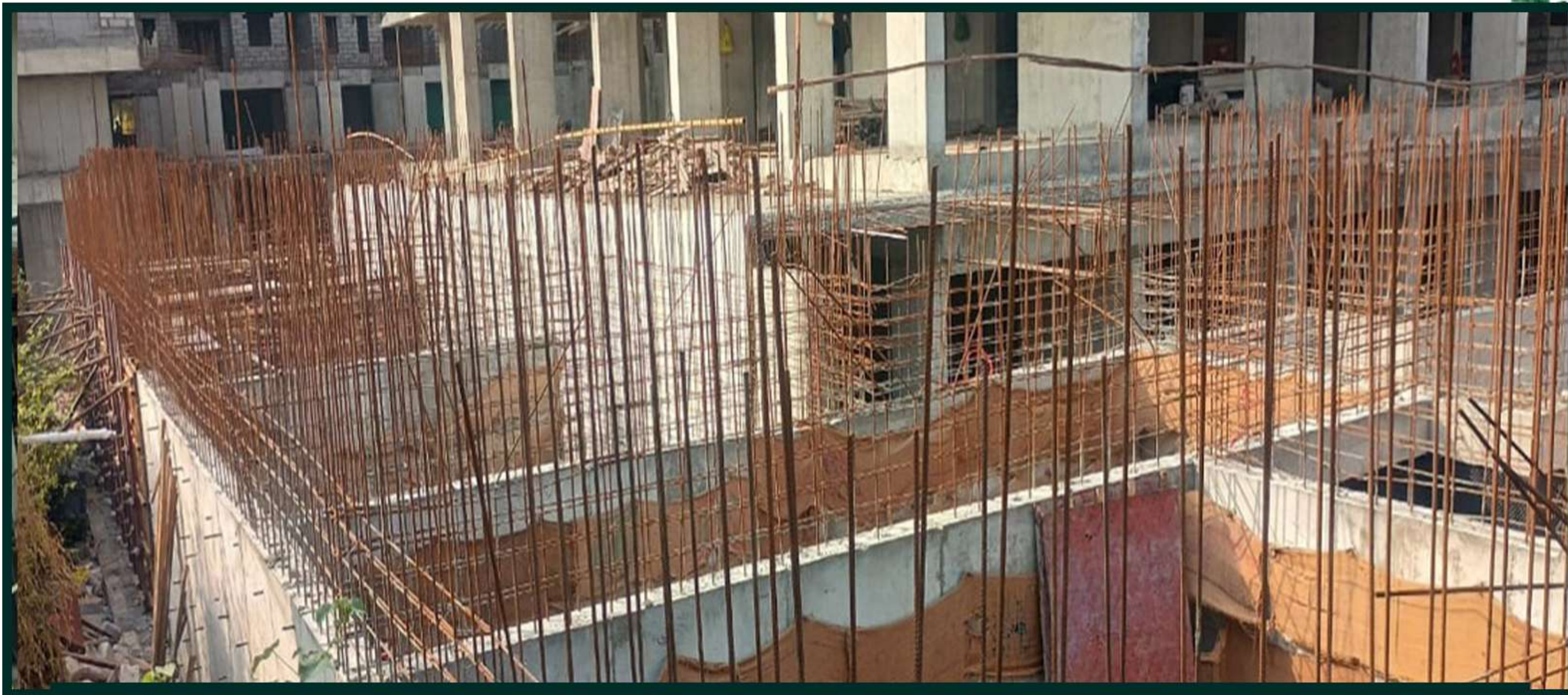
WTP WALL SHUTTERING WORK IN PROGRESS
