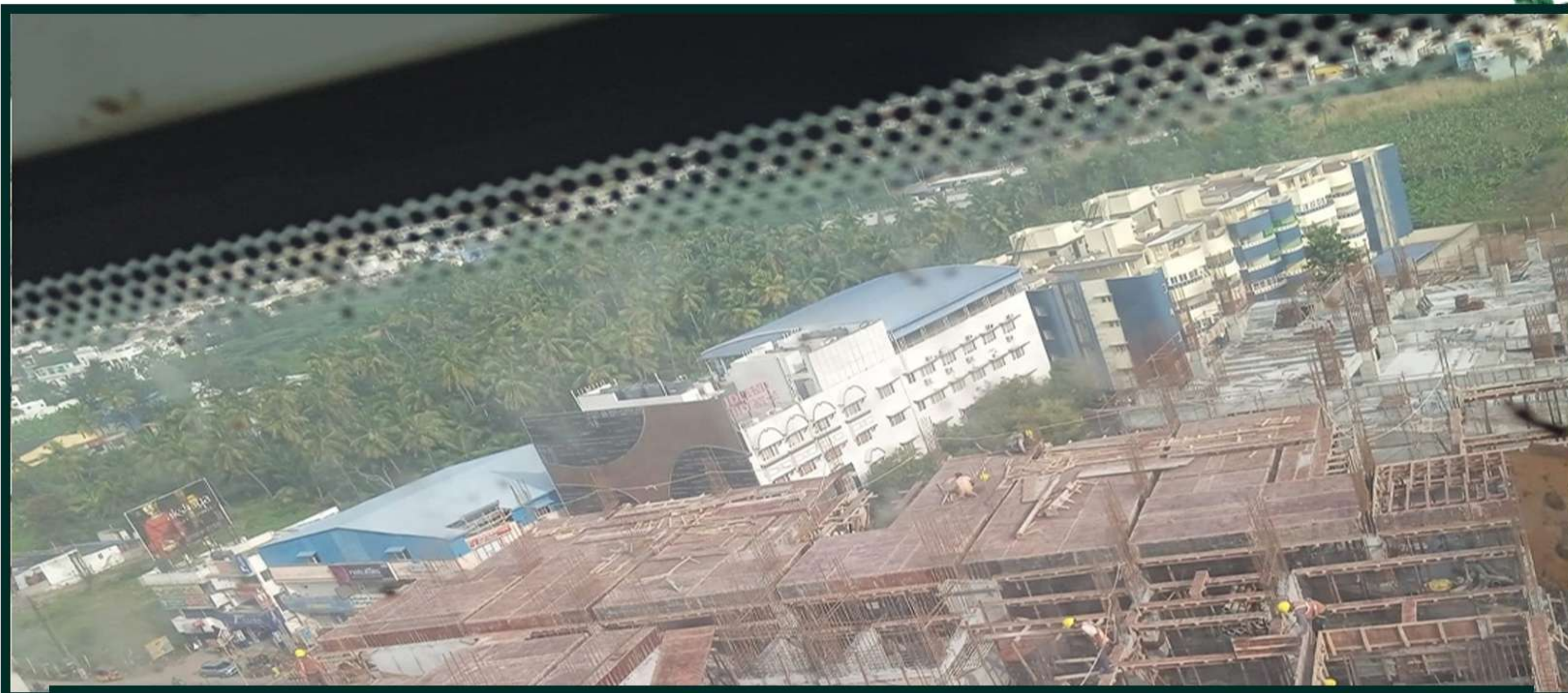
TOWER-1 POUR-5 10th FLOOR ROOF SLAB SHUTTERING WORK IN PROGRESS- TOP VIEW
