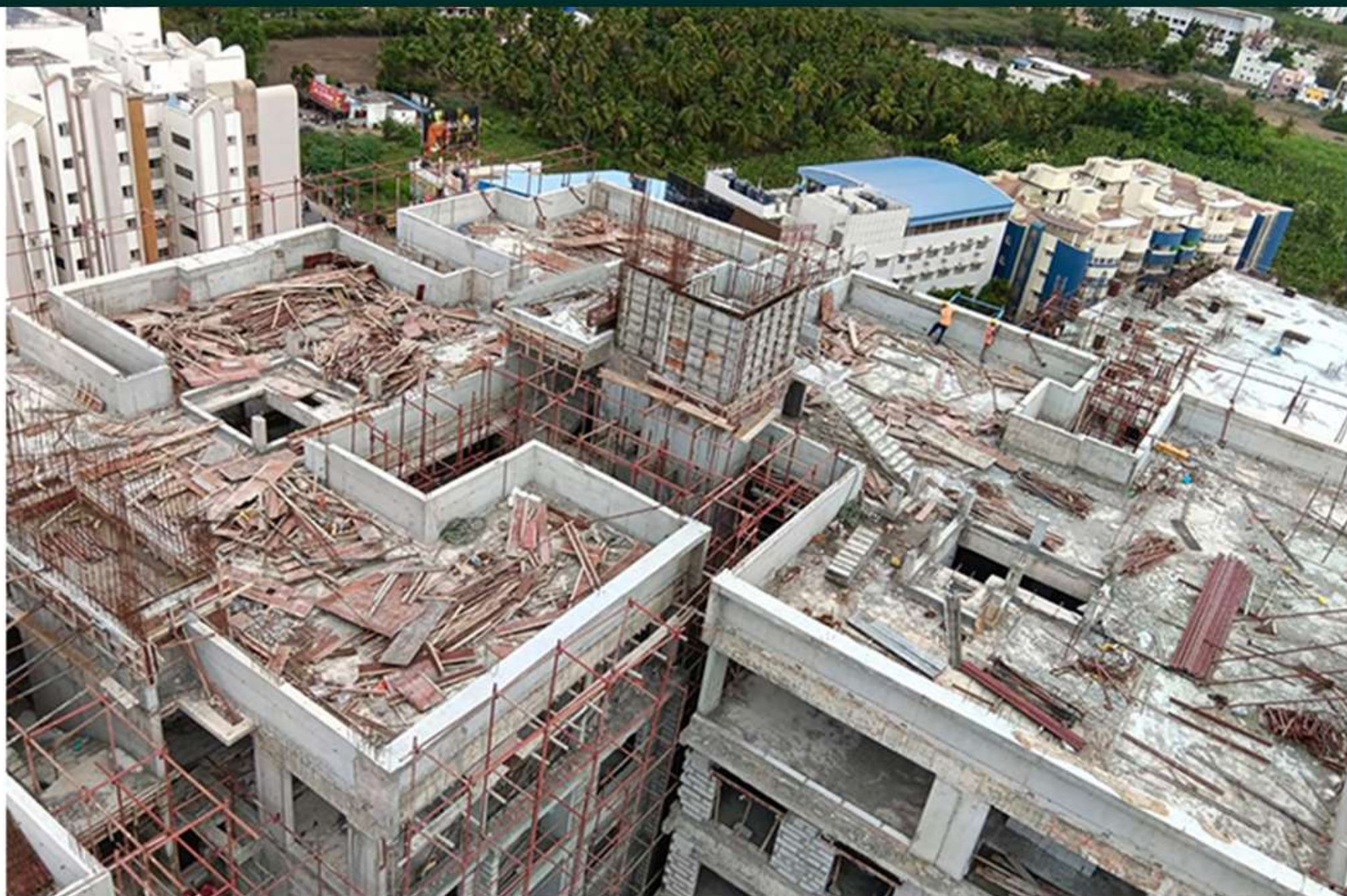
Tower-1 Pour-5 Terrace Floor Lift Head Room Work In Progress
