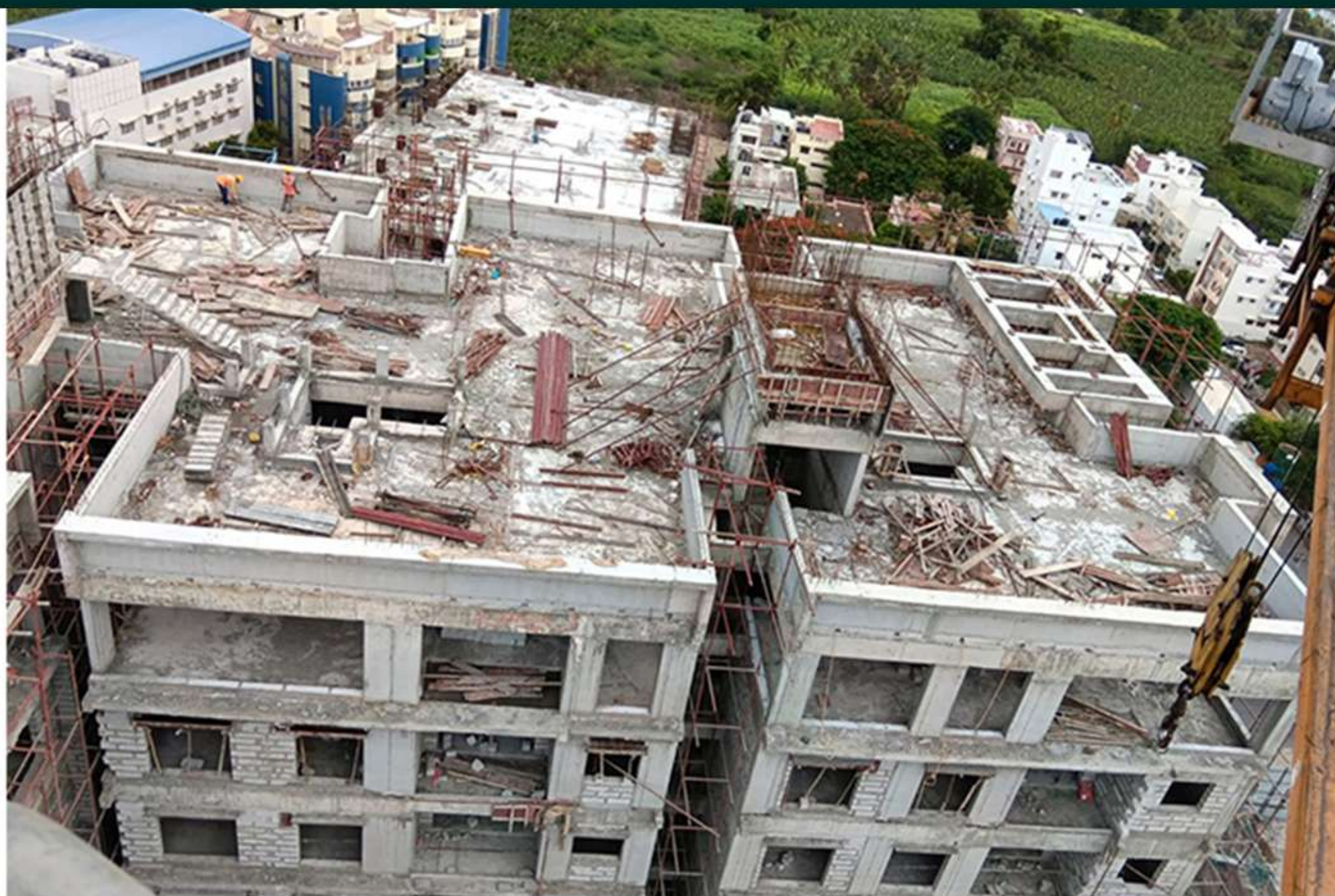
Tower-1 Pour-6 Terrace Floor Water Tank Base Slab Shuttering Work In Progress
