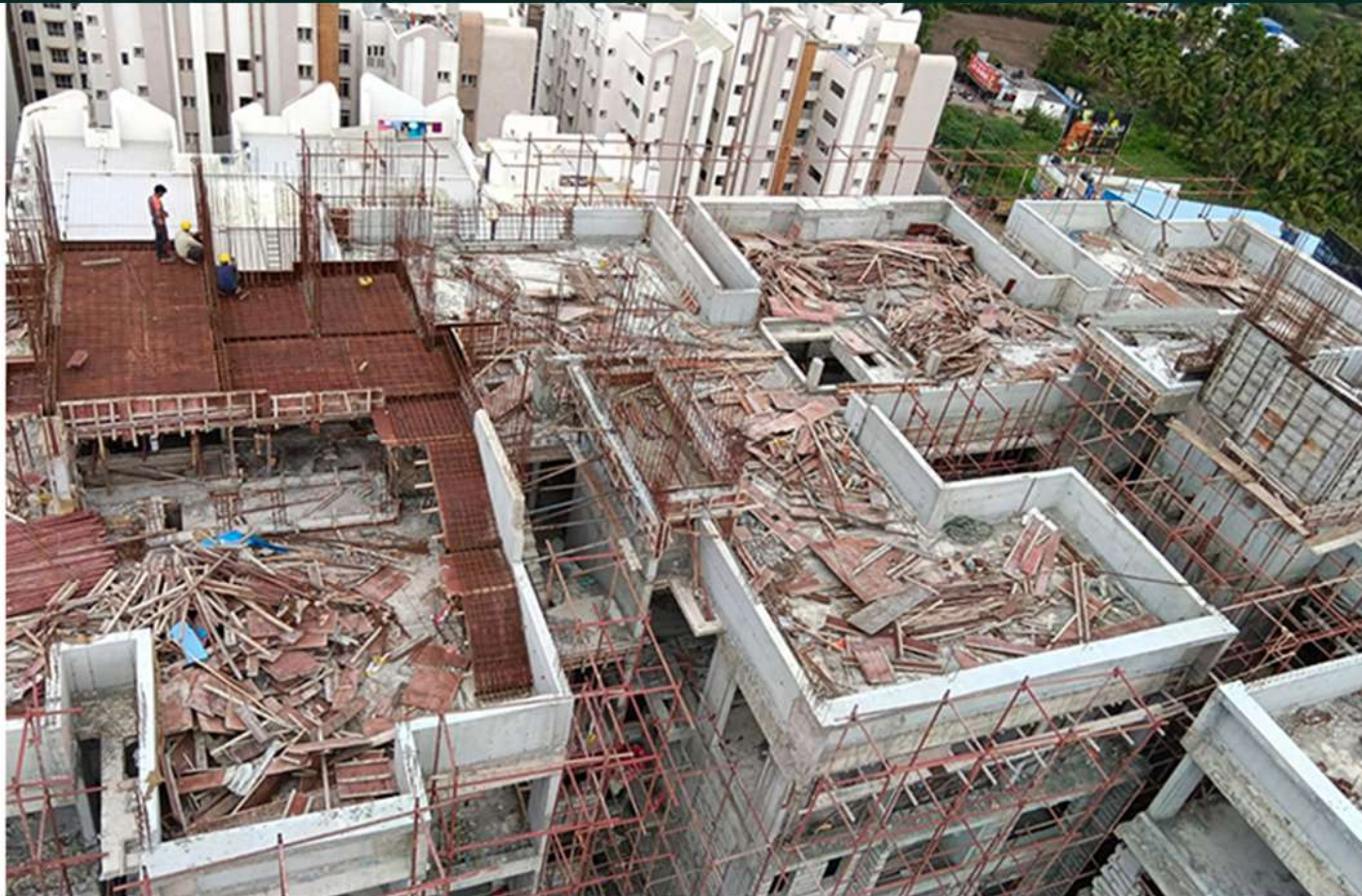
Tower-1 Pour-4 Terrace Floor Staircase Head Room Work In Progress
