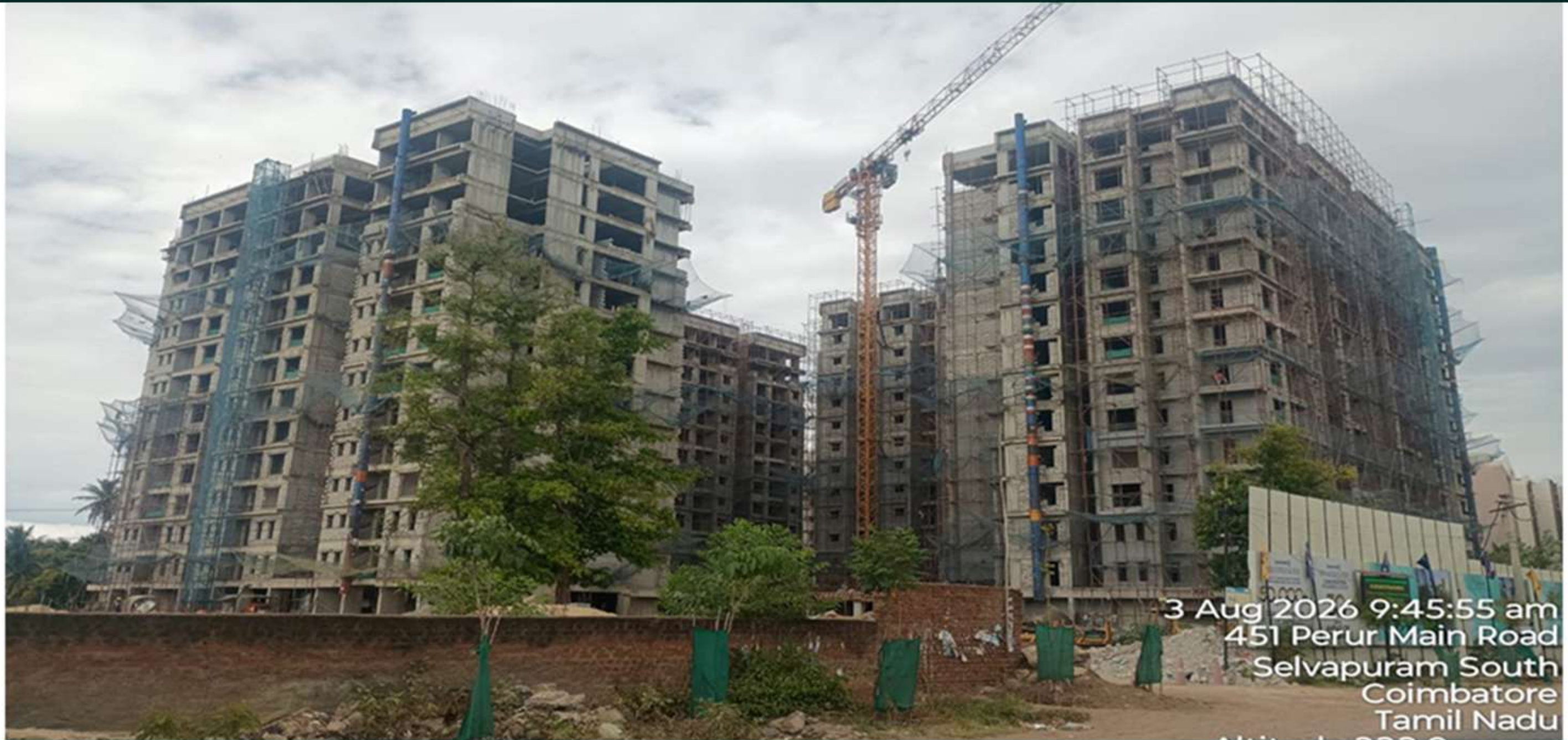
Site Over All Progress View
