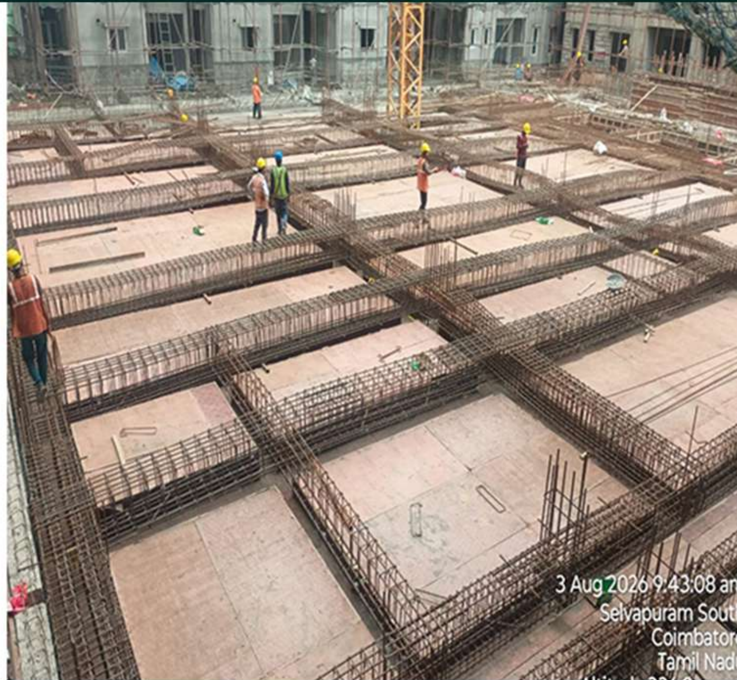
Swimming Pool Base Slab Reinforcement Work In Progress
