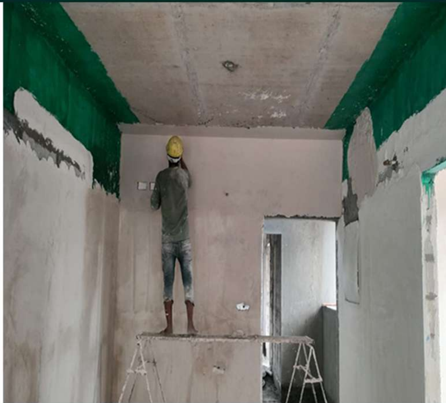
Tower 2 Gypsum Plastering 3rd Floor Work In Progress
