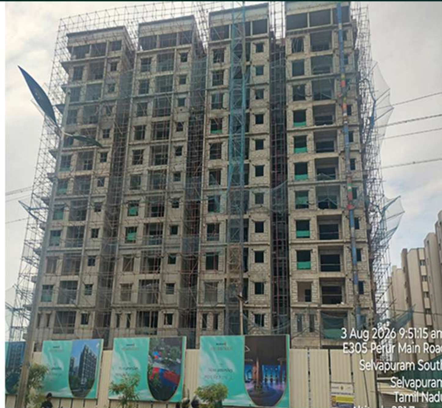
Site Over All Progress View-tower-1
