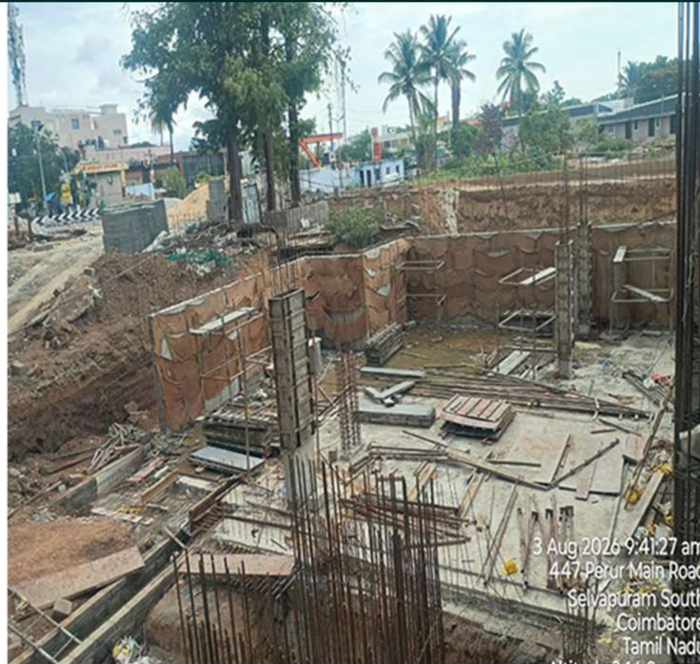
Club House Basement Column Shuttering Work In Progress
