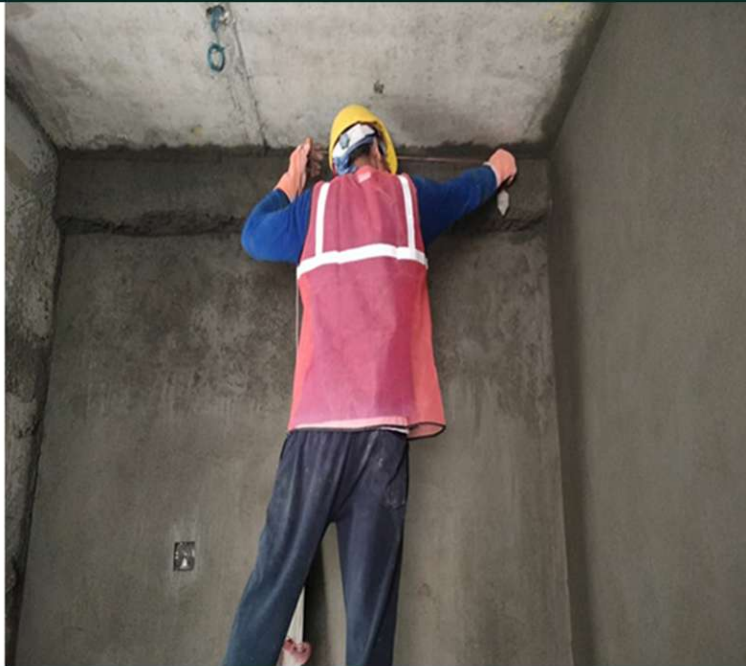
Tower 1 Cement Plastering 7th Floor Work In Progress
