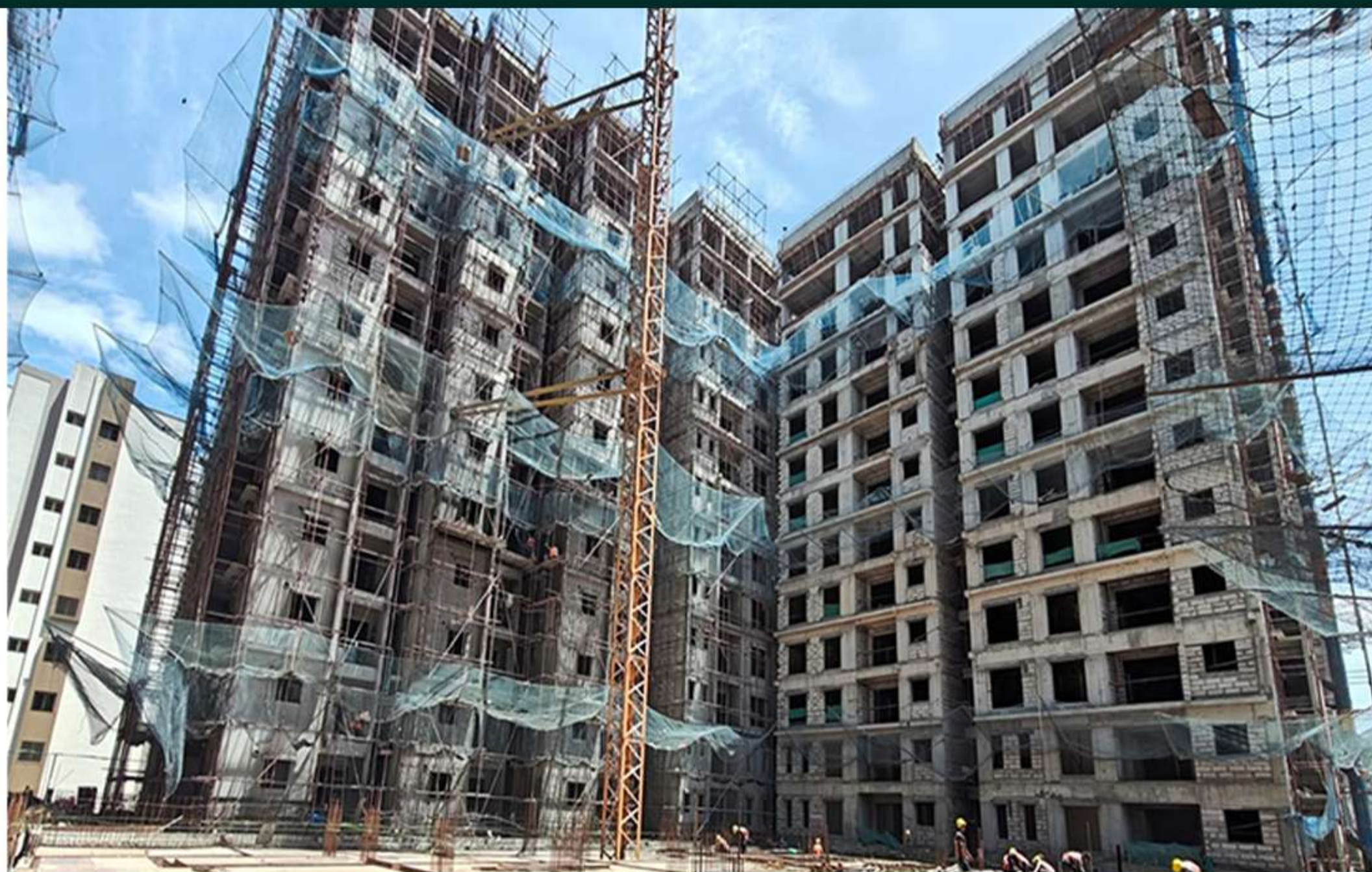
SITE OVER ALL PROGRESS VIEW-TOWER-1 PODIUM VIEW
