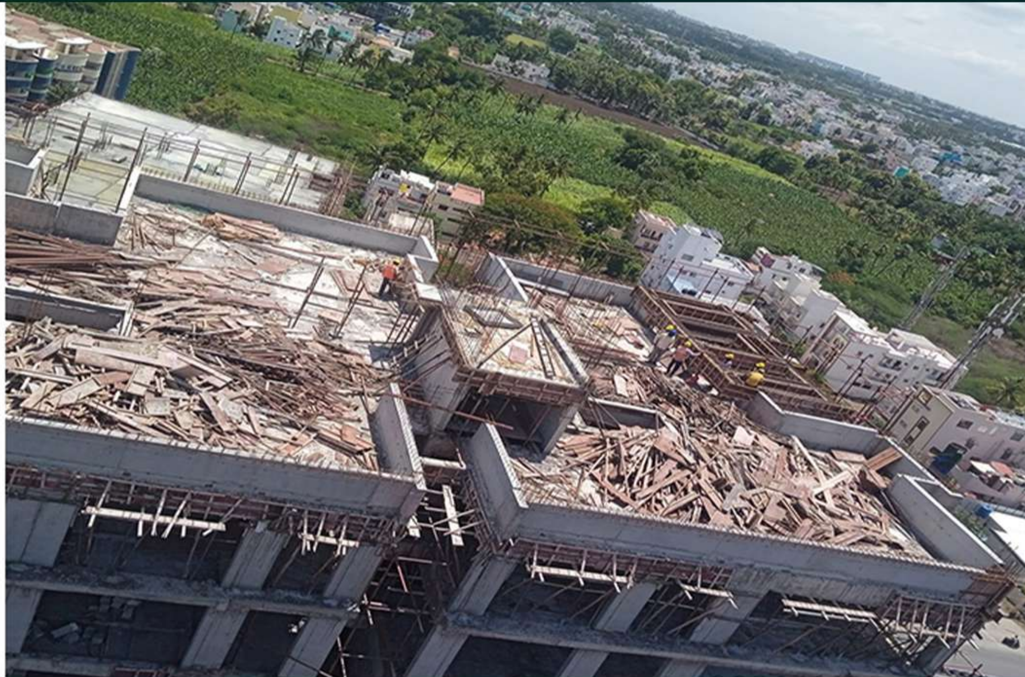
TOWER-1 POUR-6 TERRACE FLOOR PARAPET WALL WORK IN PROGRESS
