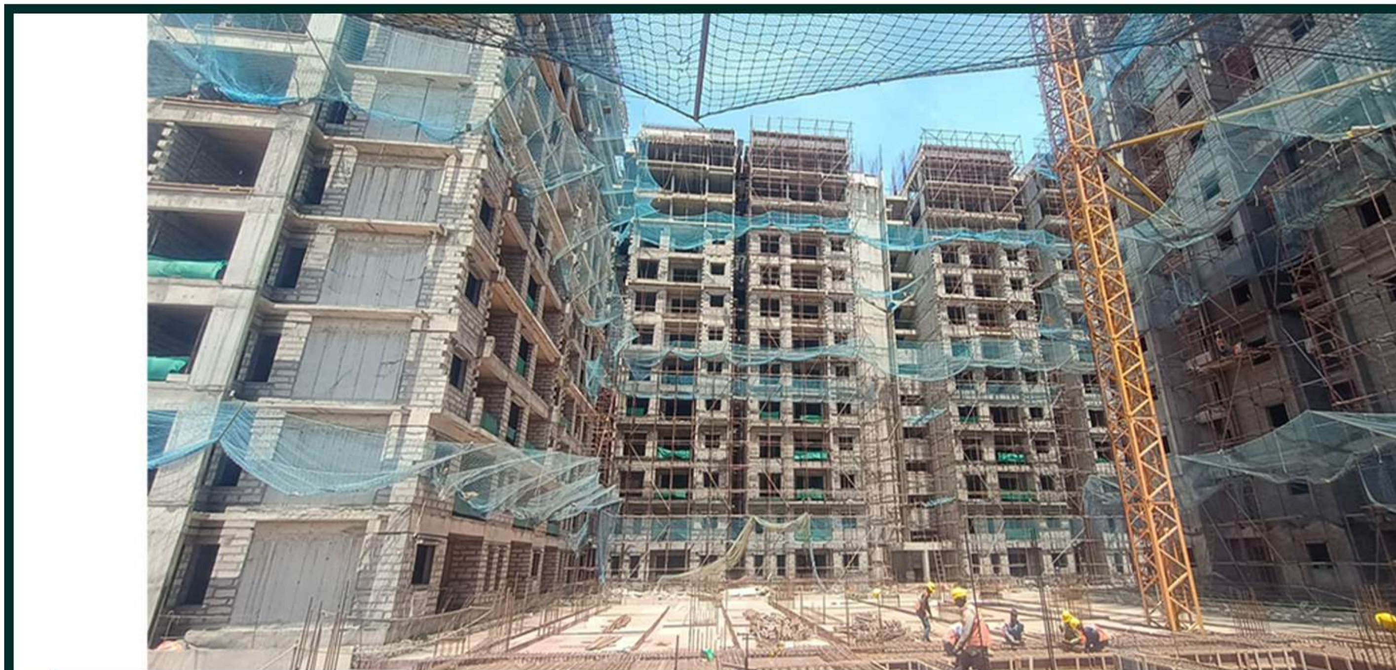
SITE OVER ALL PROGRESS VIEW-TOWER-2 PODIUM VIEW
