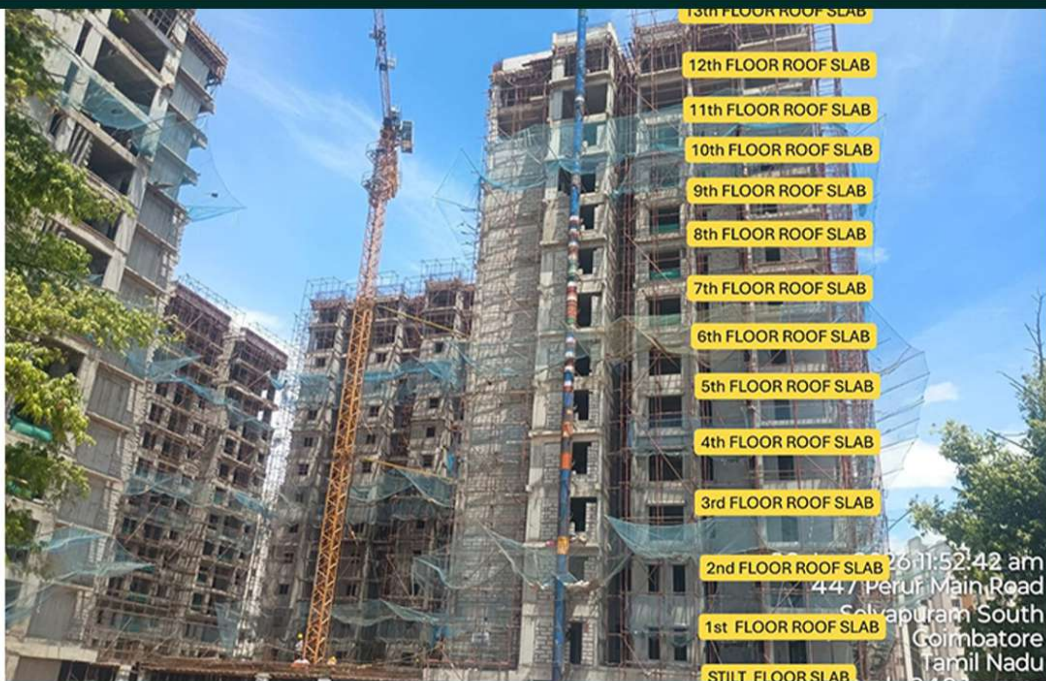
SITE OVER ALL PROGRESS VIEW-TOWER-1
