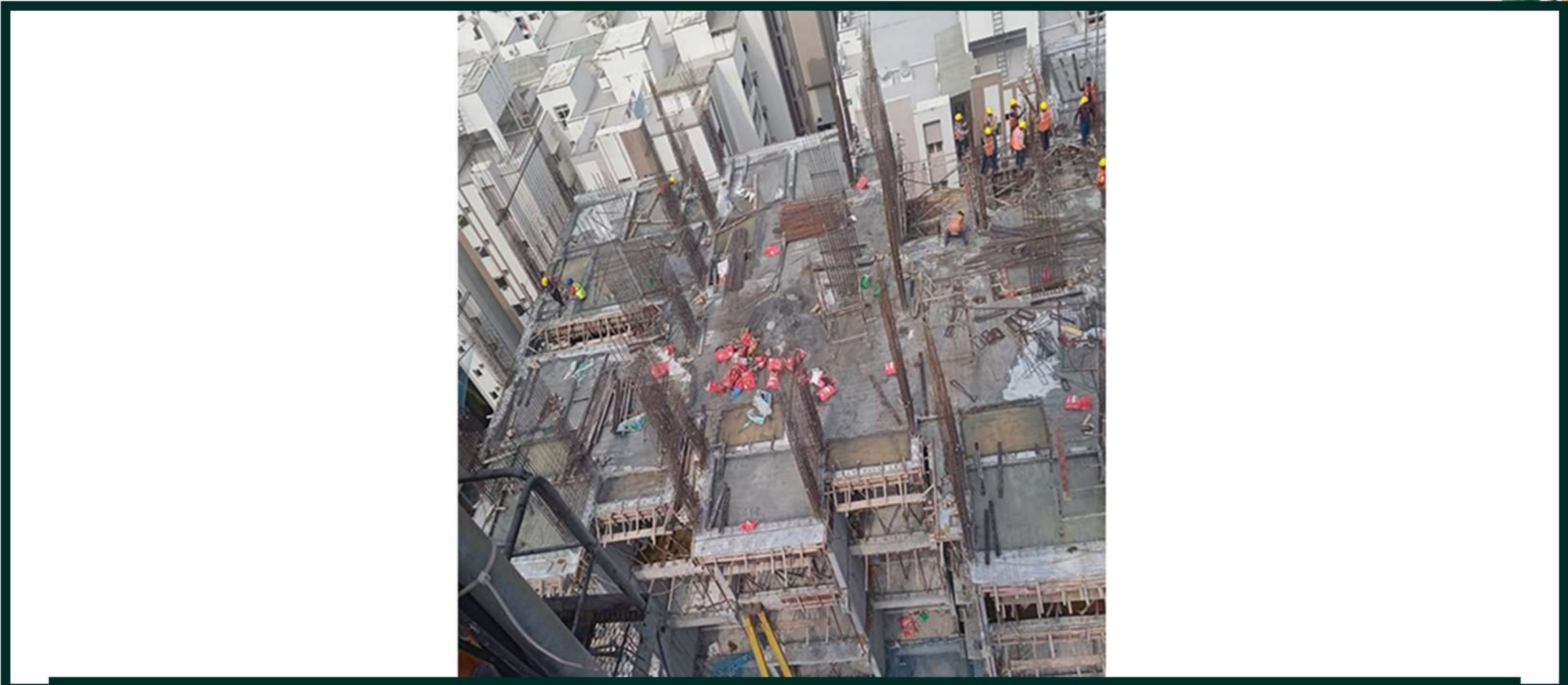
Tower-1 Pour-4 13th Floor Column Reinforcement Work In Progress
