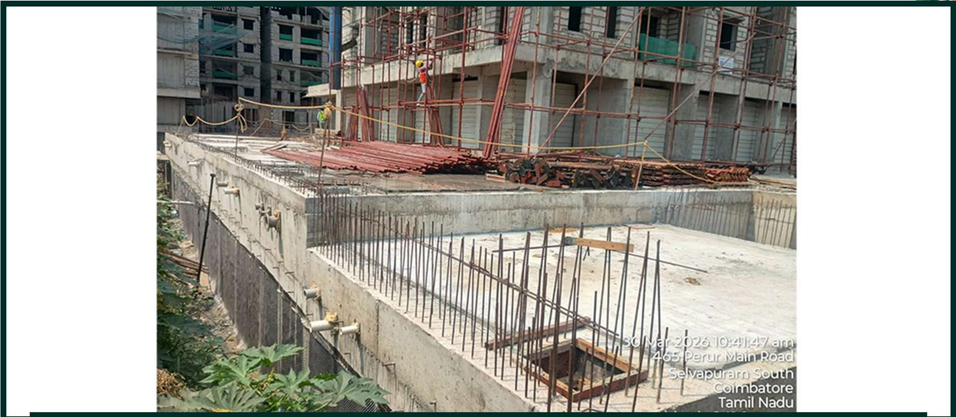
WTP – Cover Slab Completed
