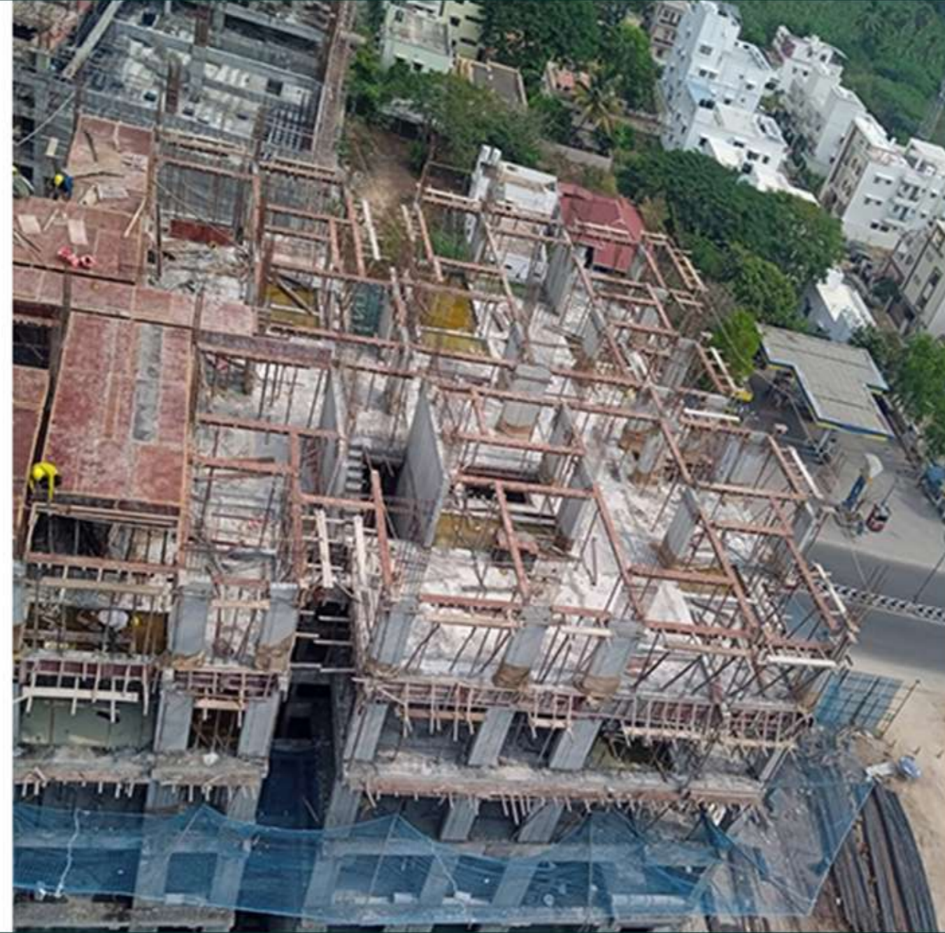
Tower-1 Pour-6 12th Floor Roof Slab Shuttering Work In Progress
