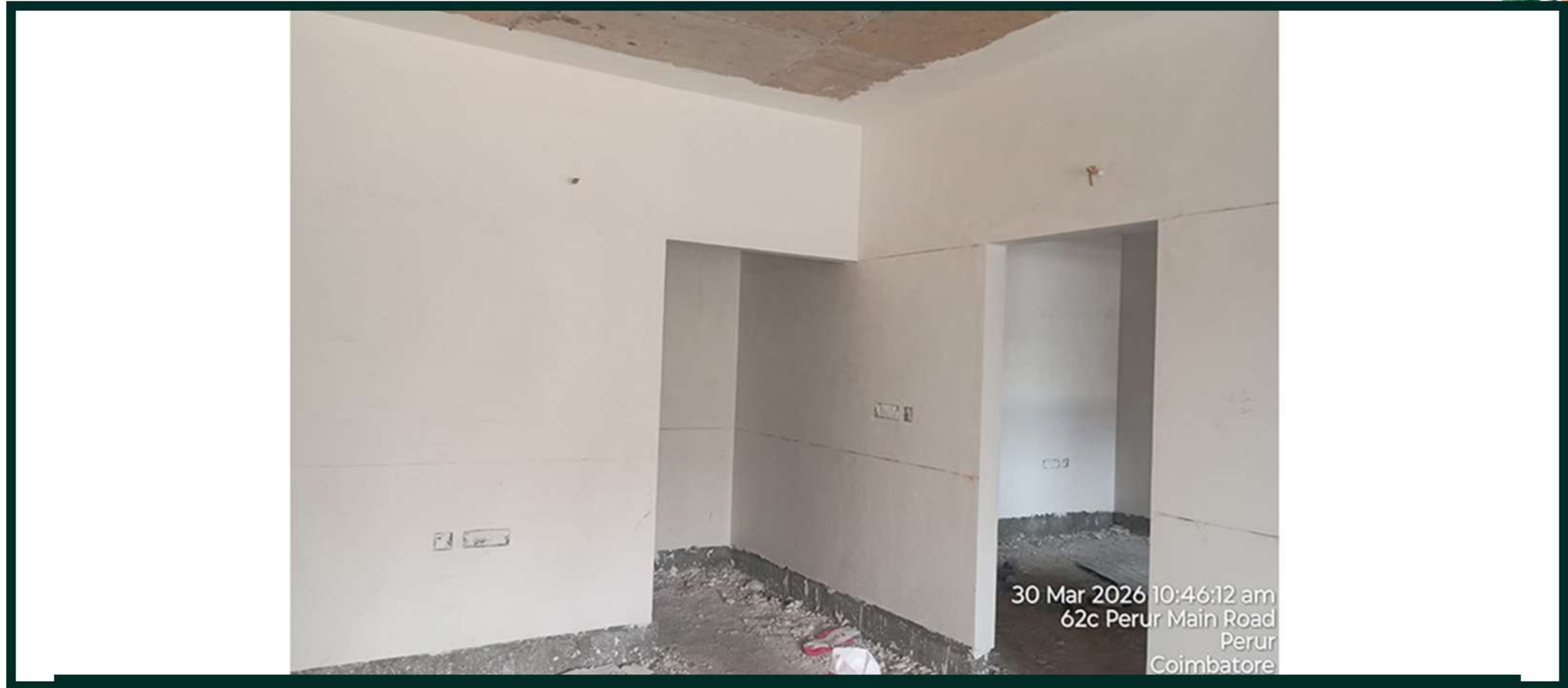
Tower 1 Floor 1 Gypsum Plastering Work In Progress
