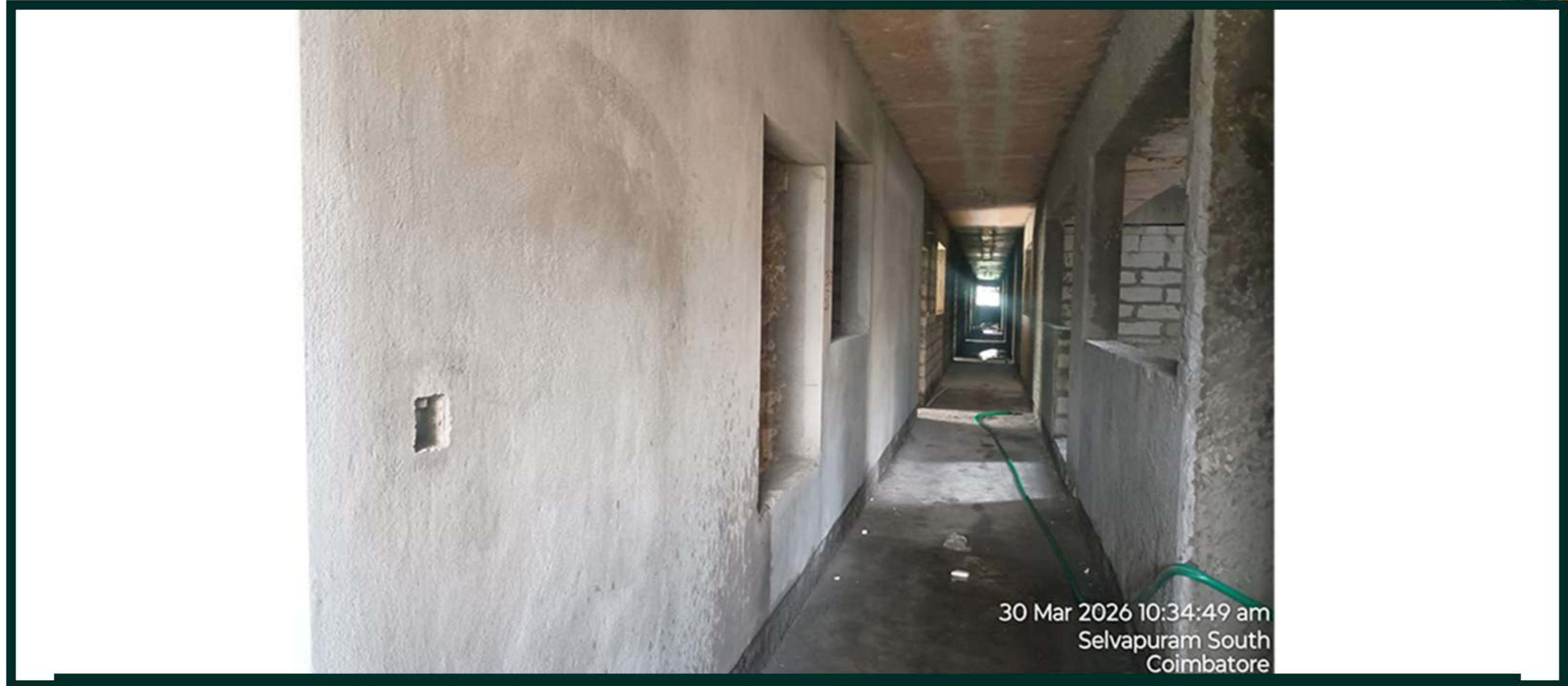
Tower 2 Floor 1 Plastering Work In Progress
