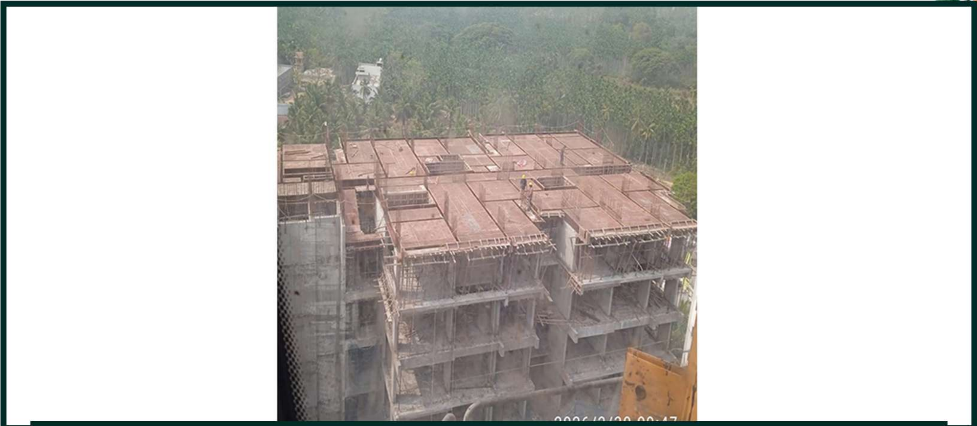
Tower-2 Pour -1 13th Floor Roof Slab Shuttering Work In Progress
