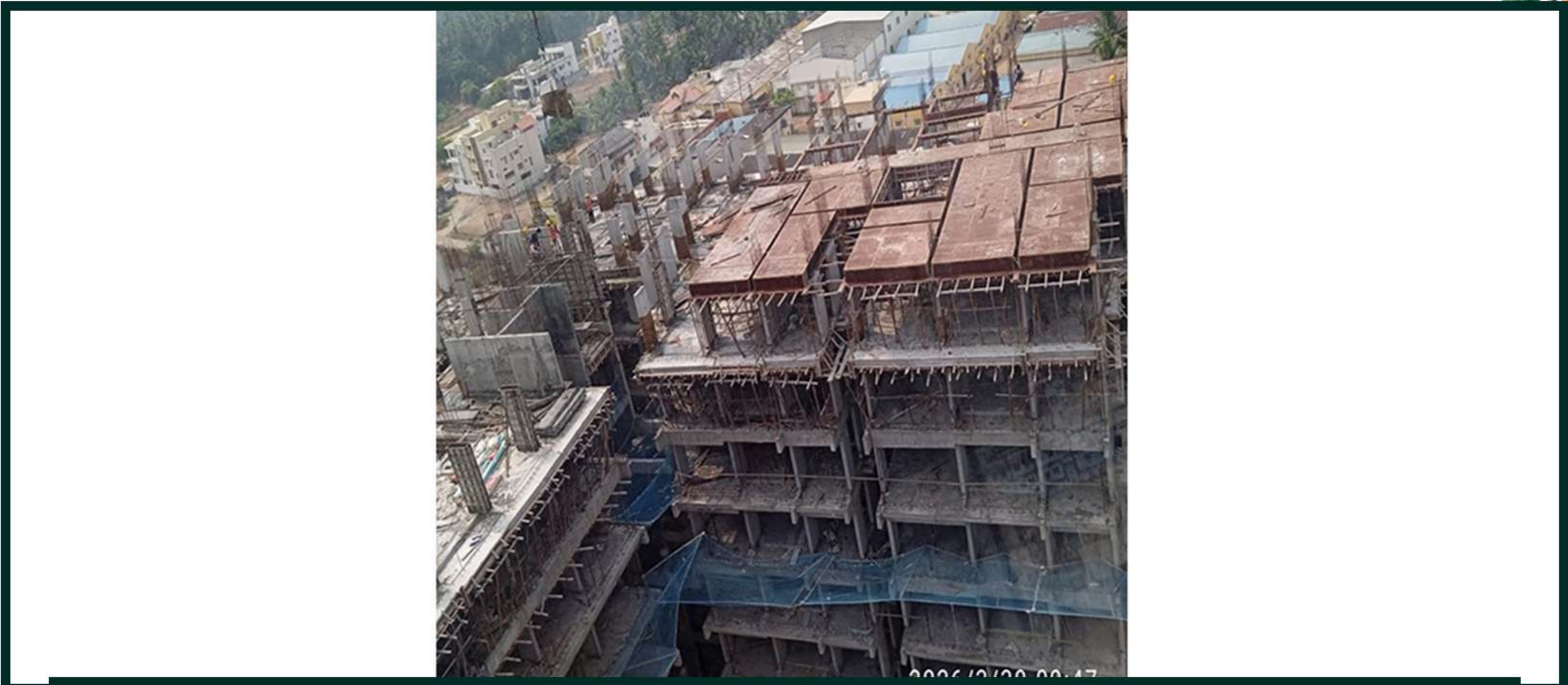
Tower-2 Pour -2 13th Floor Column Work In Progress
