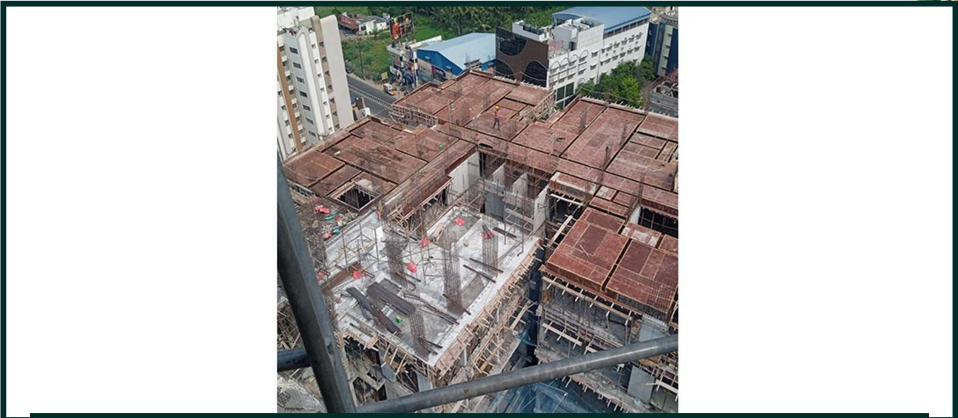
Tower-1 Pour-5 12th Floor Roof Slab Shuttering Work In Progress
