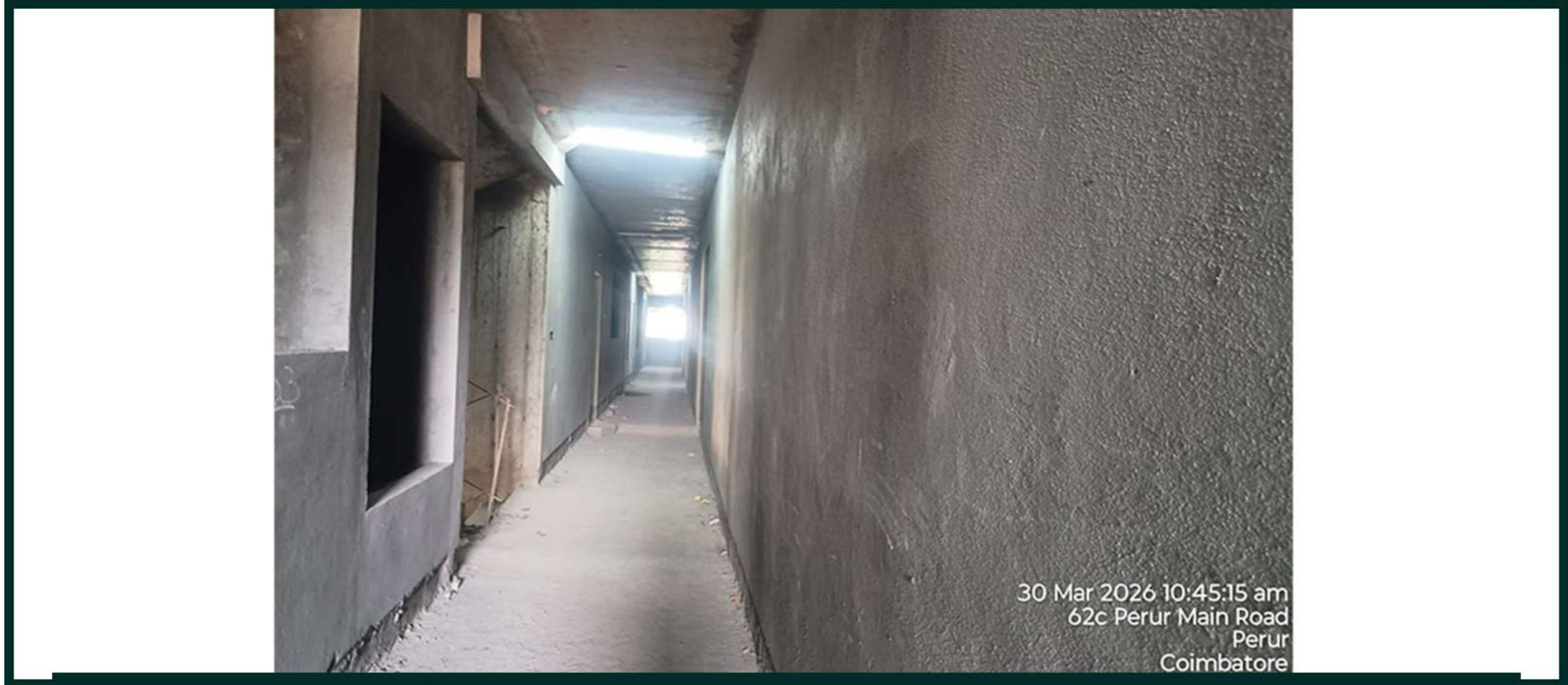
Tower 1 Floor 1 Plastering Work In Progress
