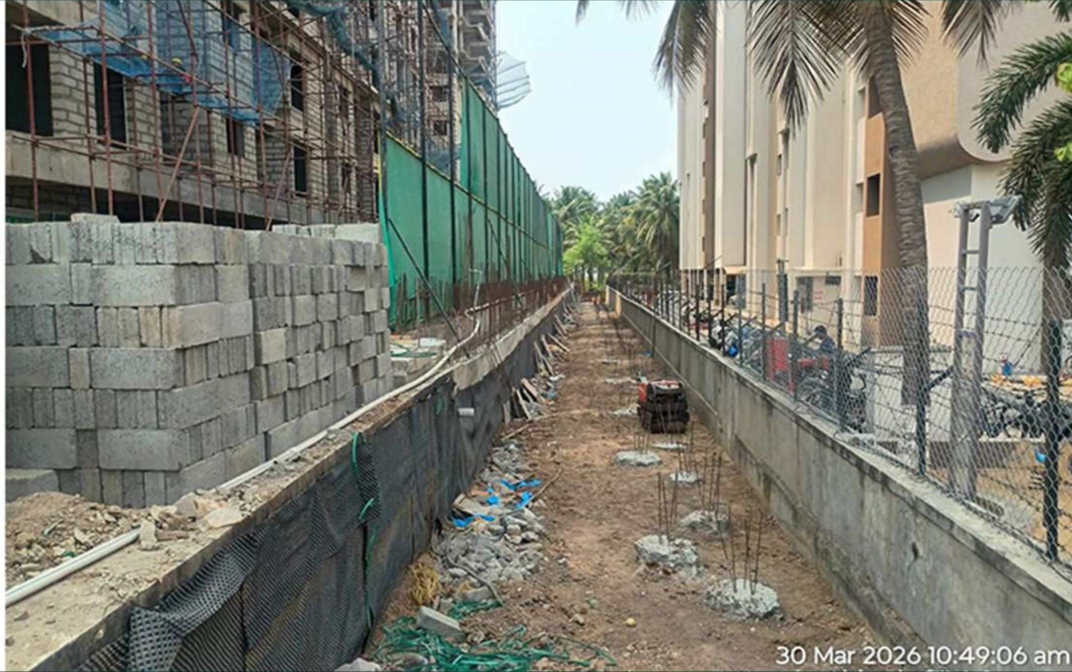
West Side Compound Wall Soil Consolidation Work In Progress
