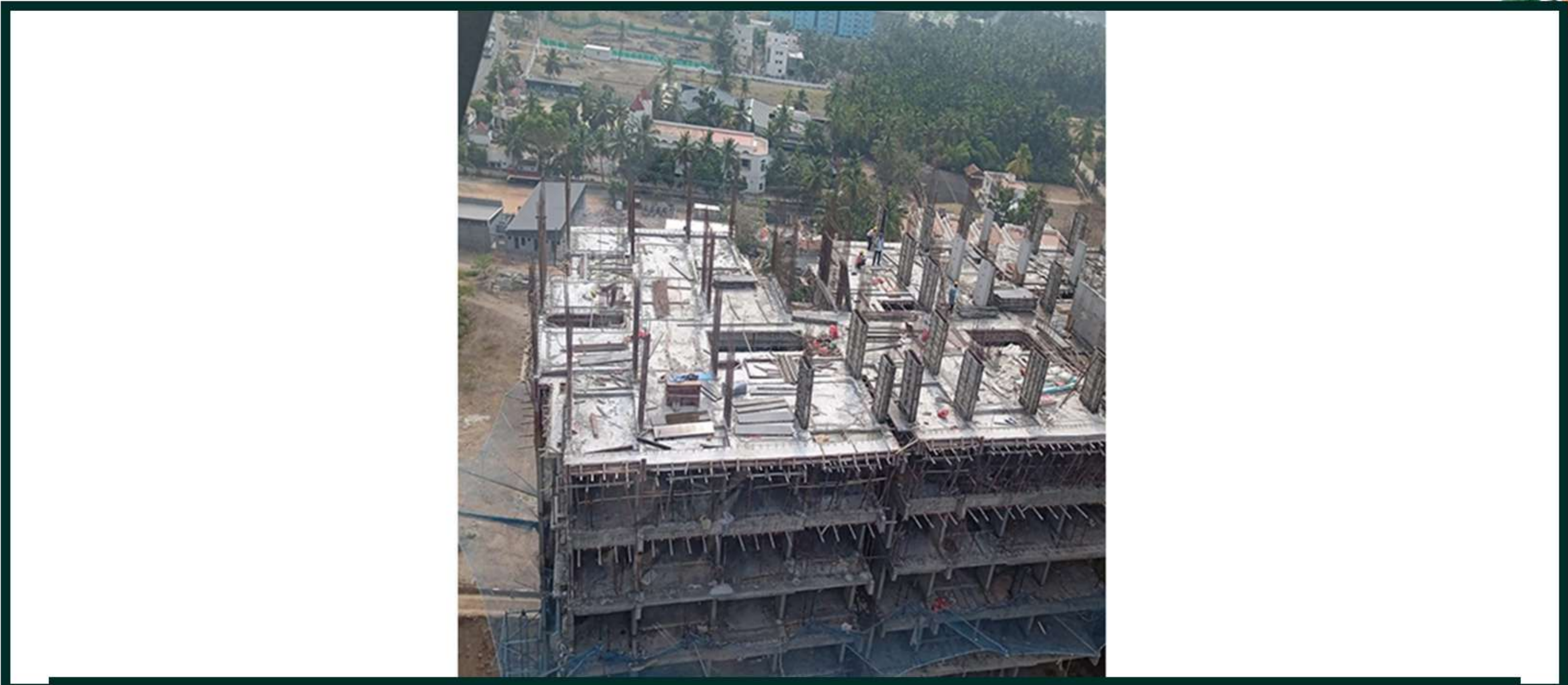
Tower-2 Pour -3 -13th Floor Column Work In Progress– Top View
