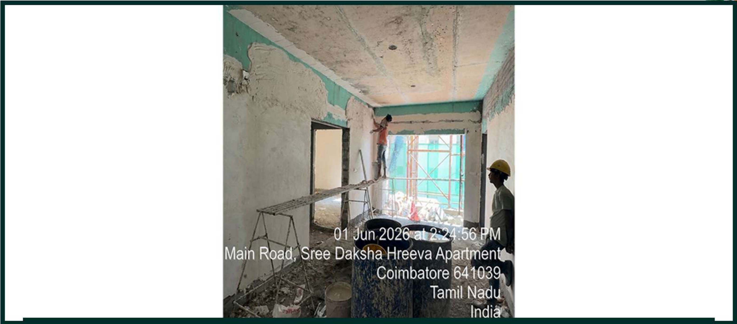
Tower 1 Floor 3 Gypsum Plastering Work In Progress
