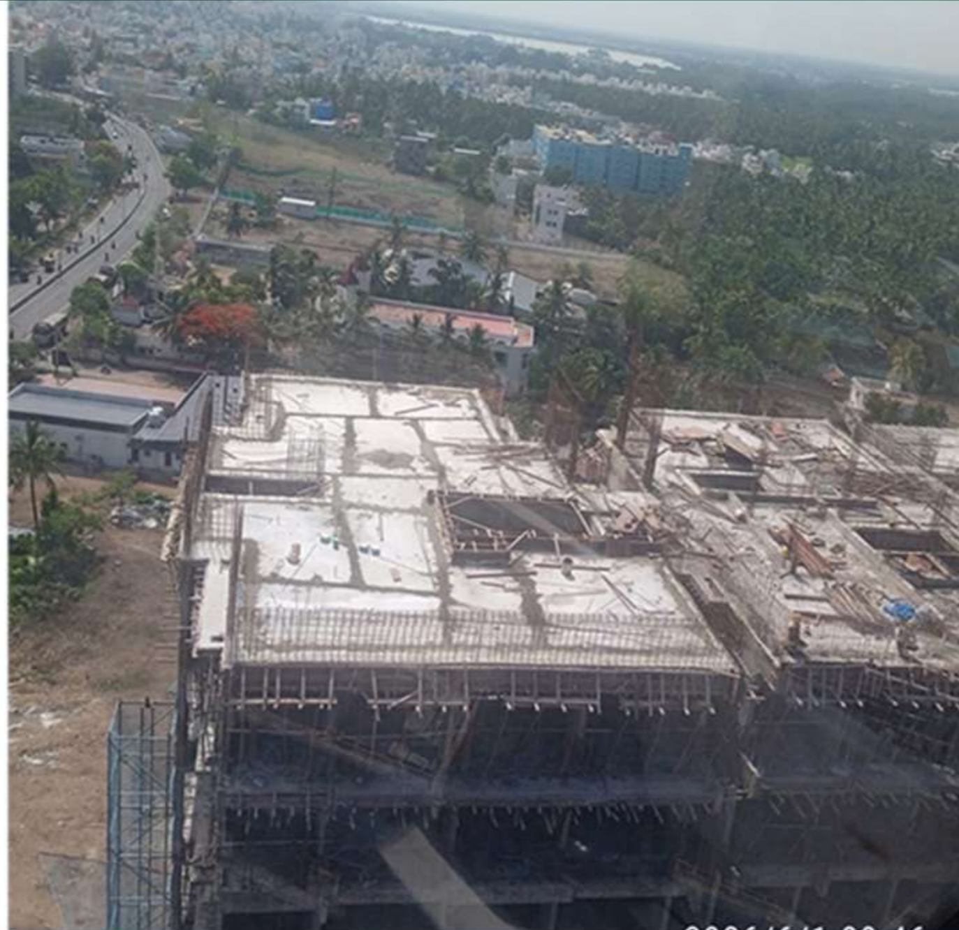
Tower-2 Pour -3 -13th Floor Roof Slab Completed
