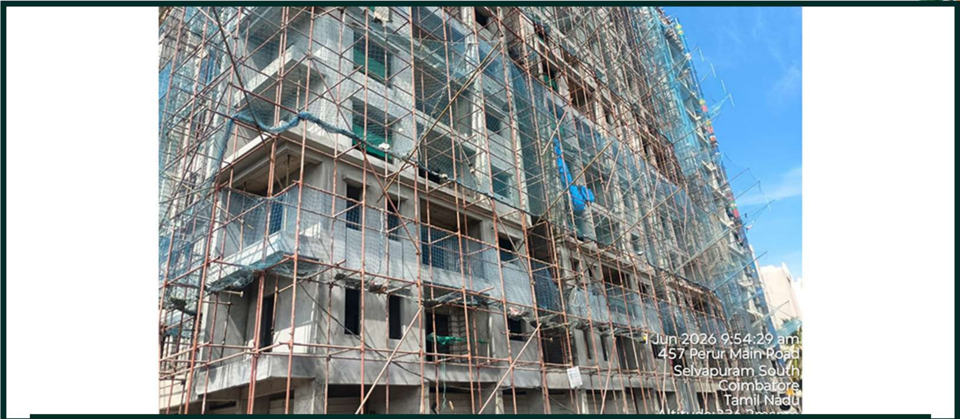
Tower 1 South Side External Plastering (1-6th Floor) Work In Progress
