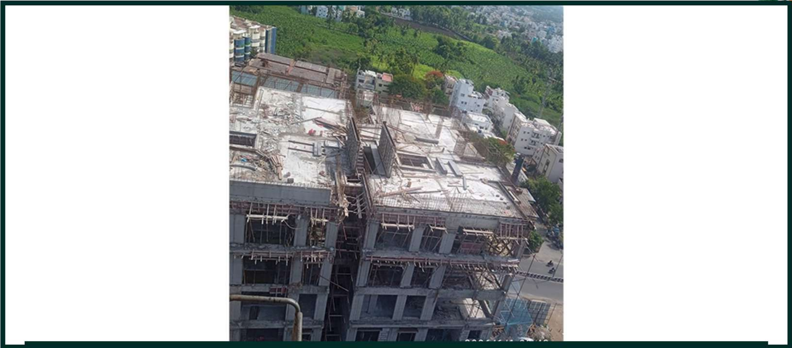
Tower-1 Pour-6 Terrace Floor Column Work In Progress
