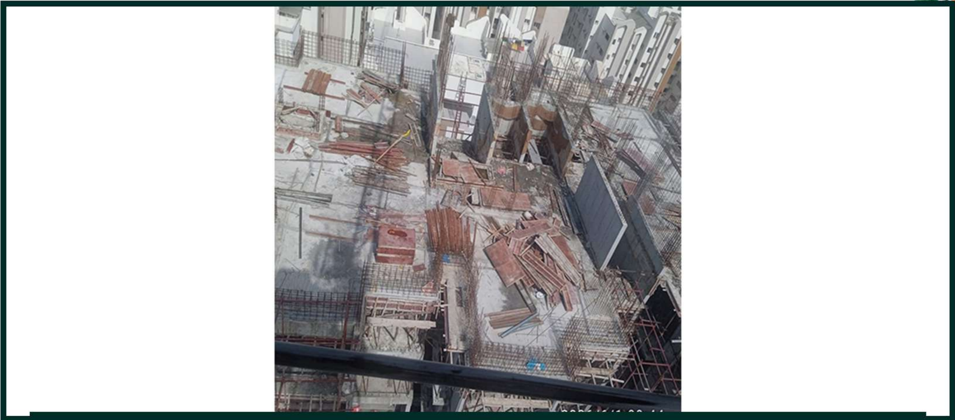
Tower-1 Pour-5 Terrace Floor Lift Shear Wall Work In Progress
