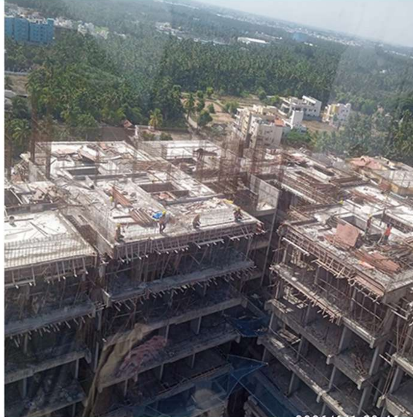
Tower-2 Pour -2 Terrace Floor Column Shuttering Work In Progress
