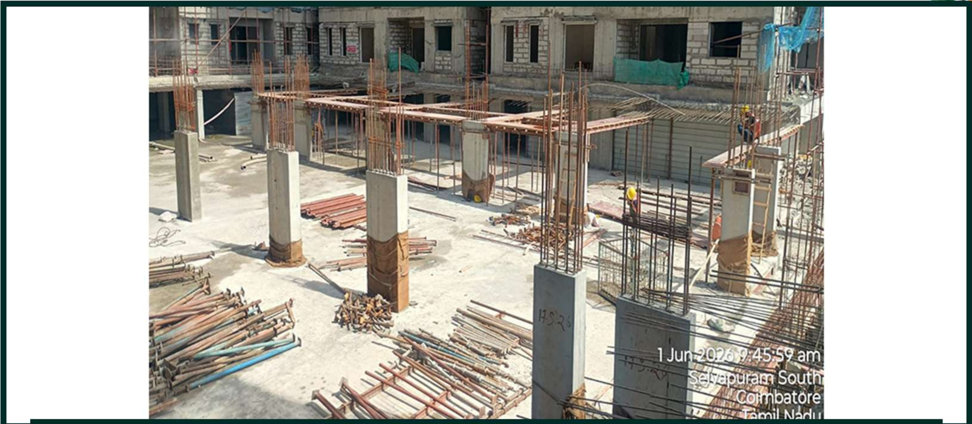
Swimming Pool Base Slab Shuttering Work In Progress
