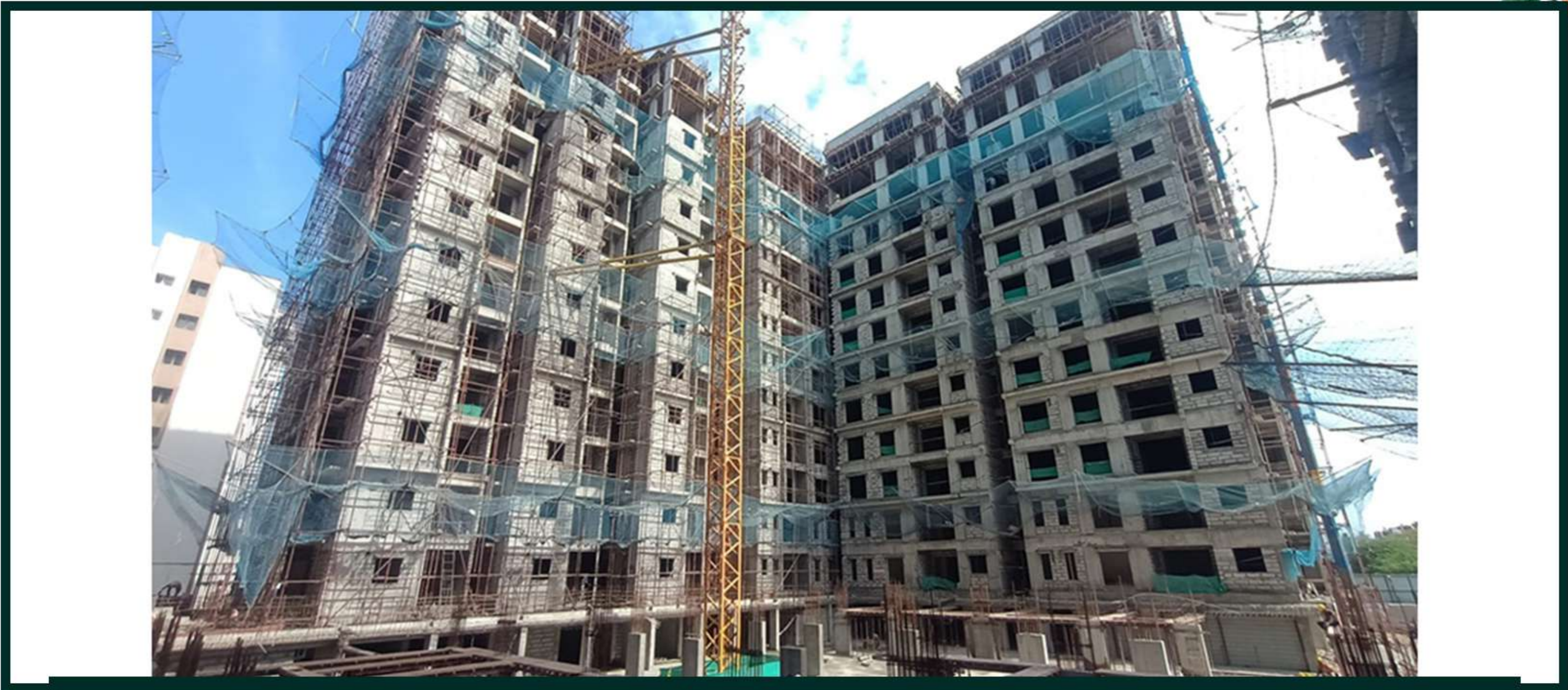
Site Over All Progress View-tower-1 Podium View
