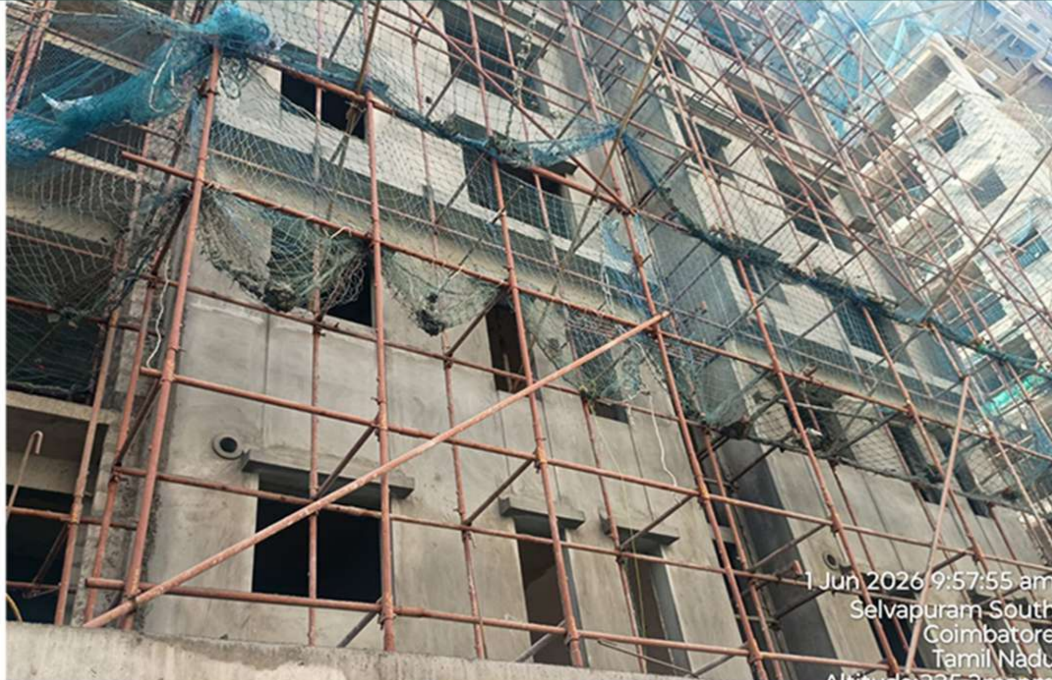
Tower 1 West Side External Plastering (1-6th Floor) Work In Progress
