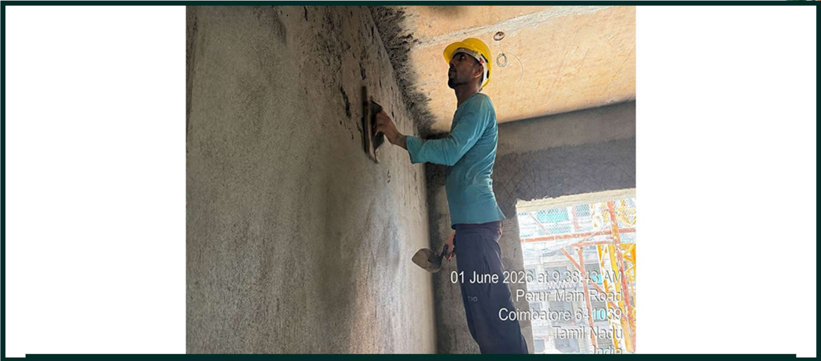
Tower 1 Floor 5 Plastering Work In Progress
