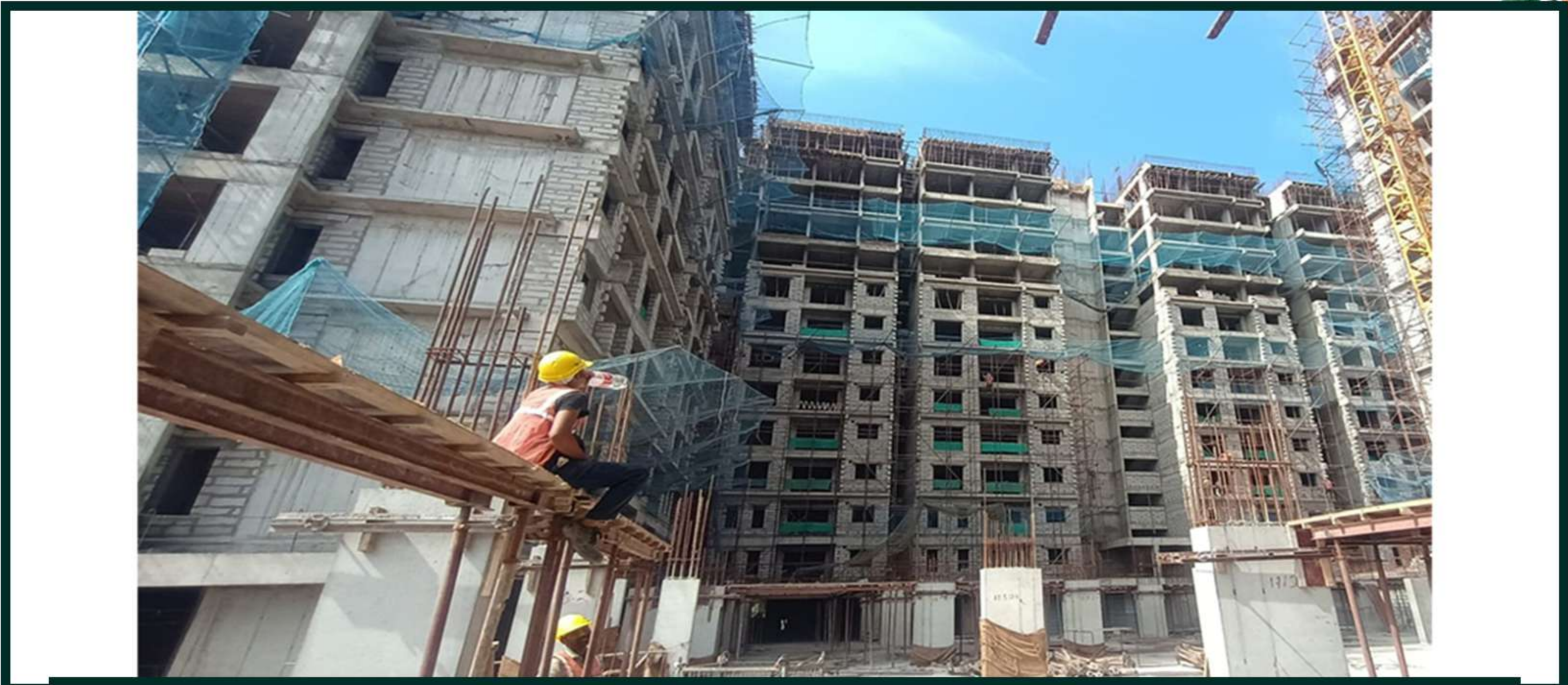
Site Over All Progress View-tower-2 Podium View
