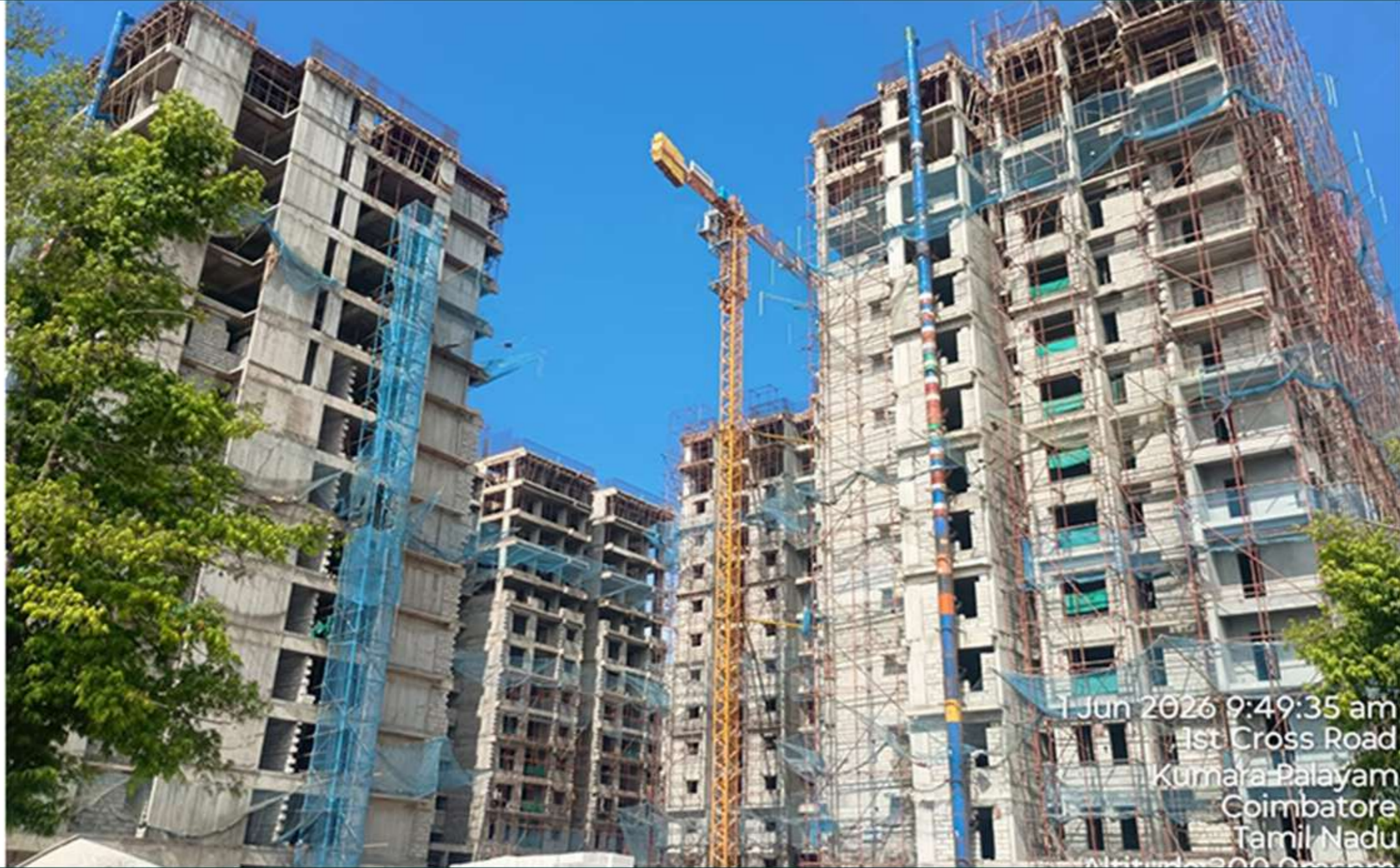
Site Over All Progress View
