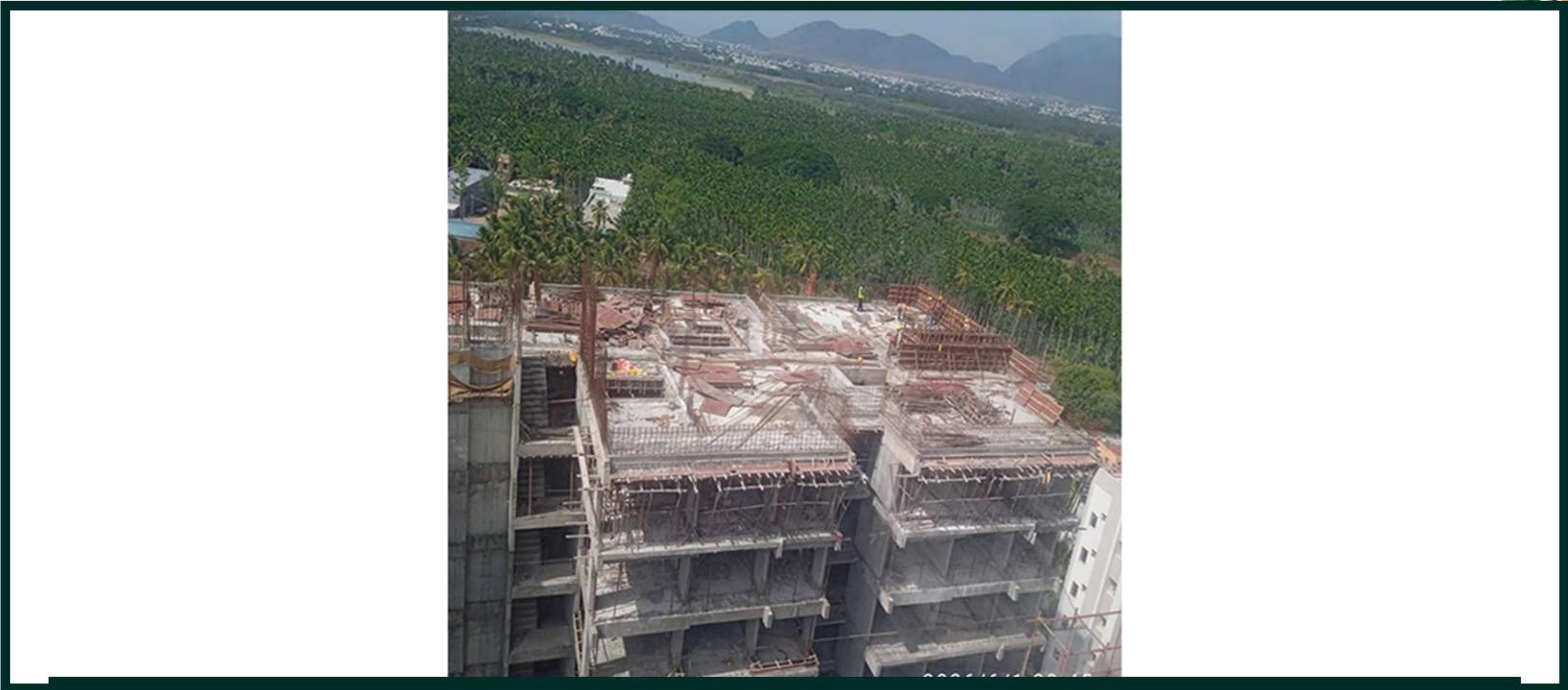
Tower-2 Pour -1 Terrace Floor Parapet Wall Shuttering Work In Progress
