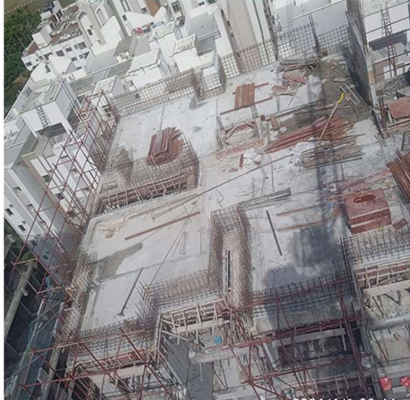
Tower-1 Pour-4 Terrace Floor Column Work In Progress
