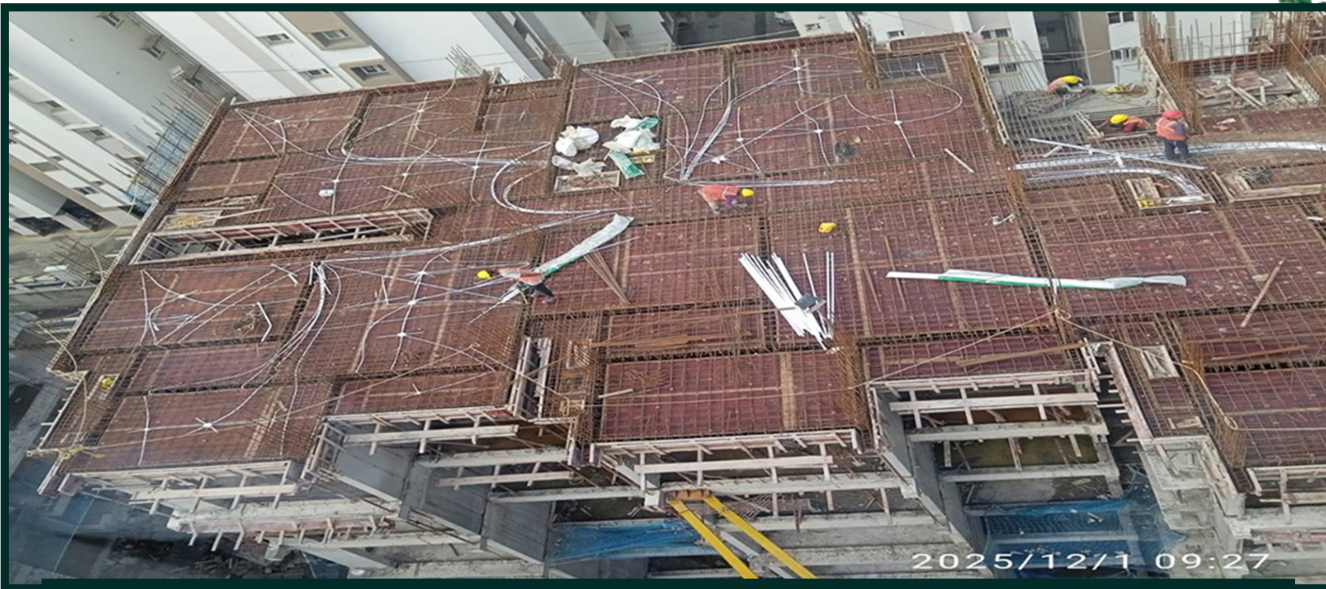
Tower-1 pour-4 7th floor roof slab steel reinforcement- top view
