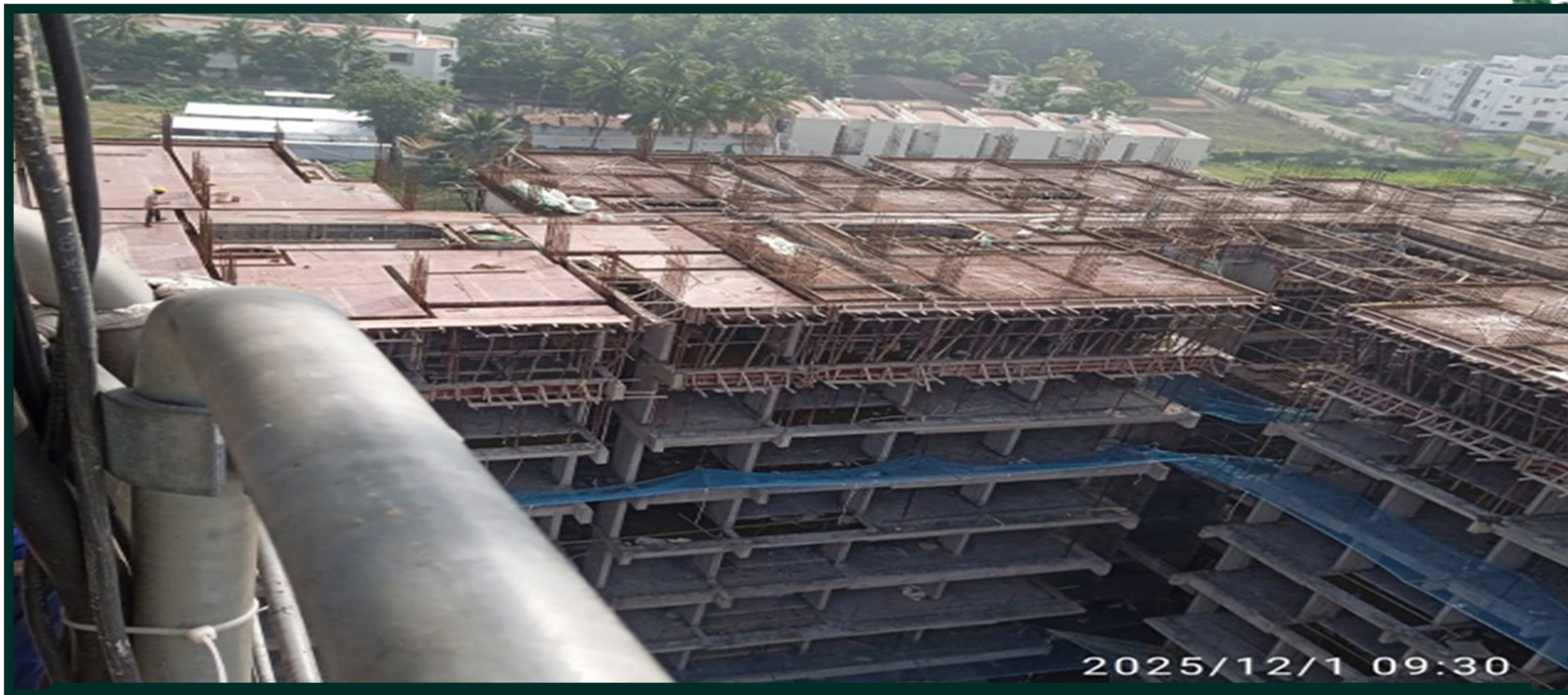
Tower-2 pour -2 8th floor roof slab steel reinforcement– top view
