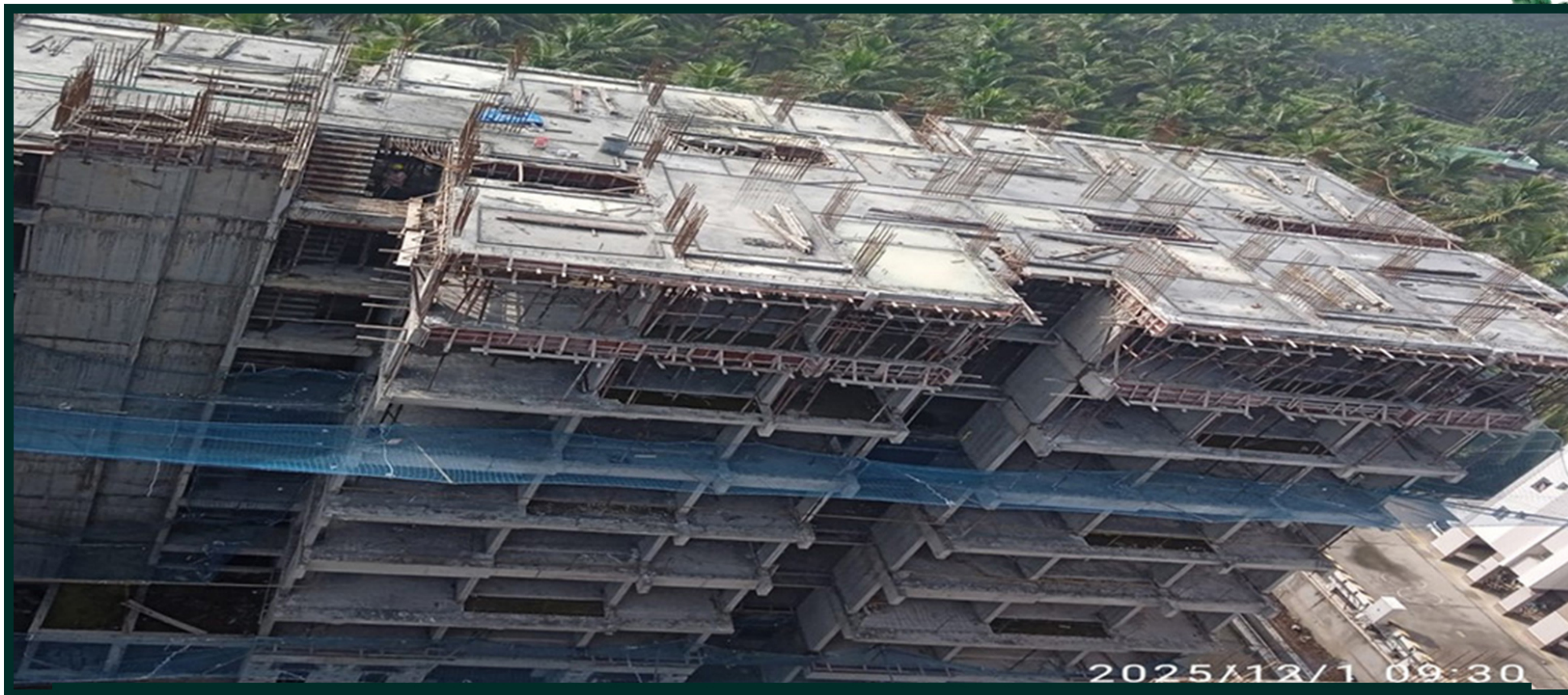
Tower-2 pour -1 8th floor roof slab concrete completed top view
