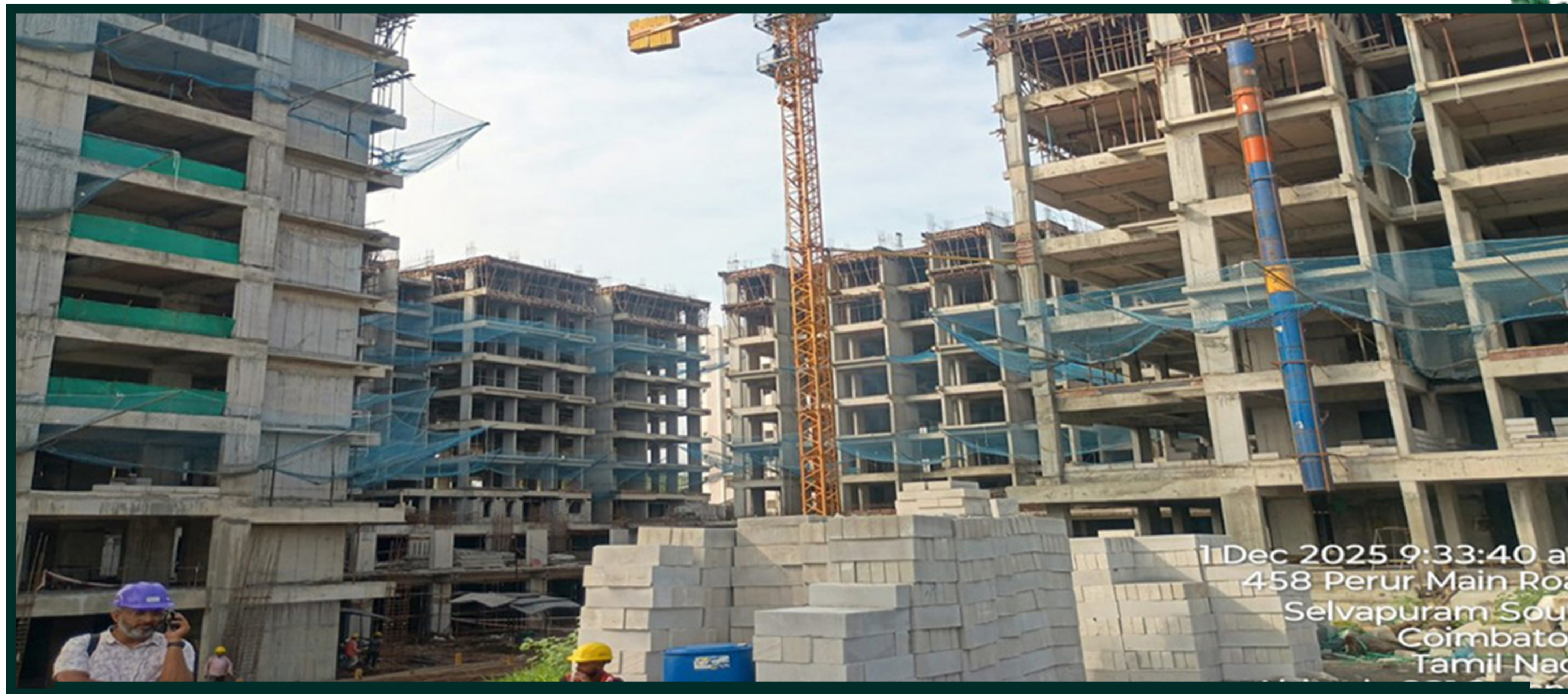
Site over all progress view
