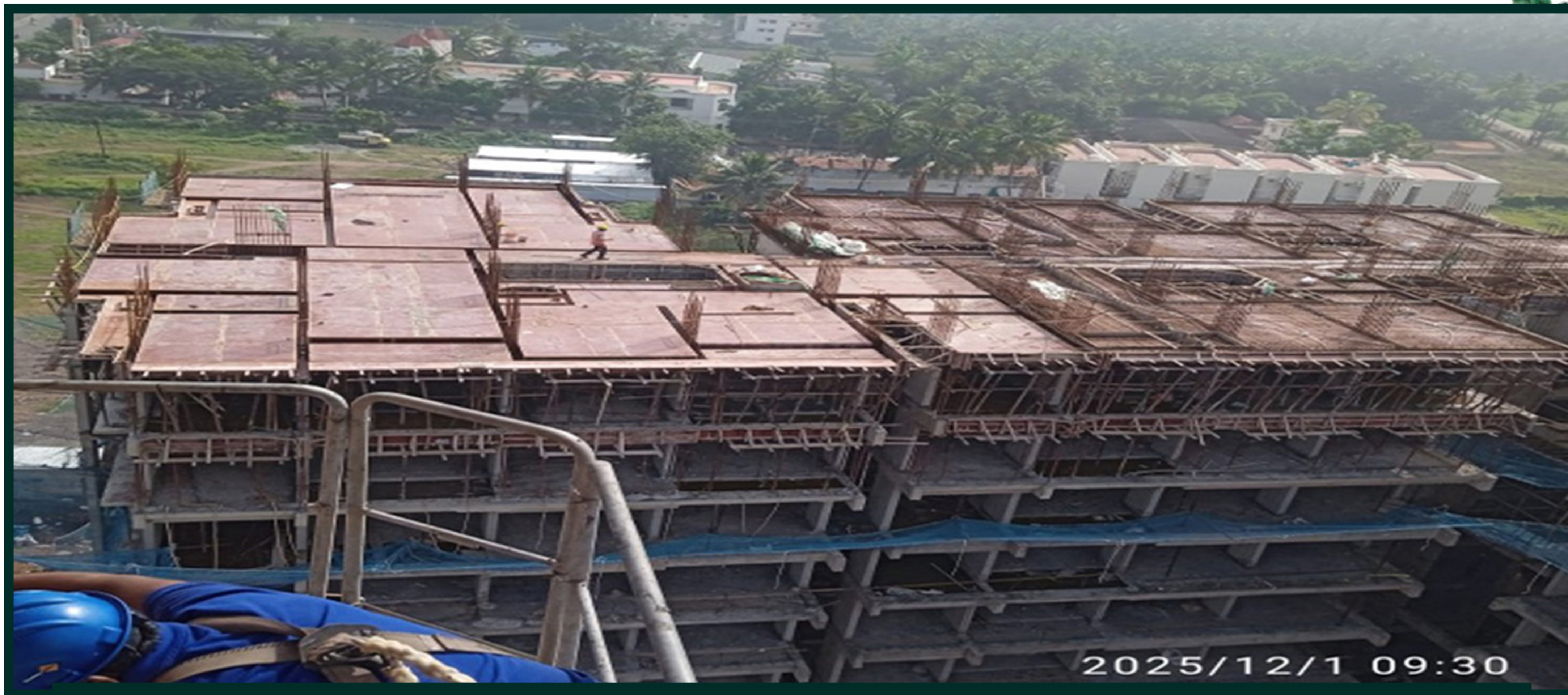
Tower-2 pour-3 8th floor roof shuttering work in progress – top view
