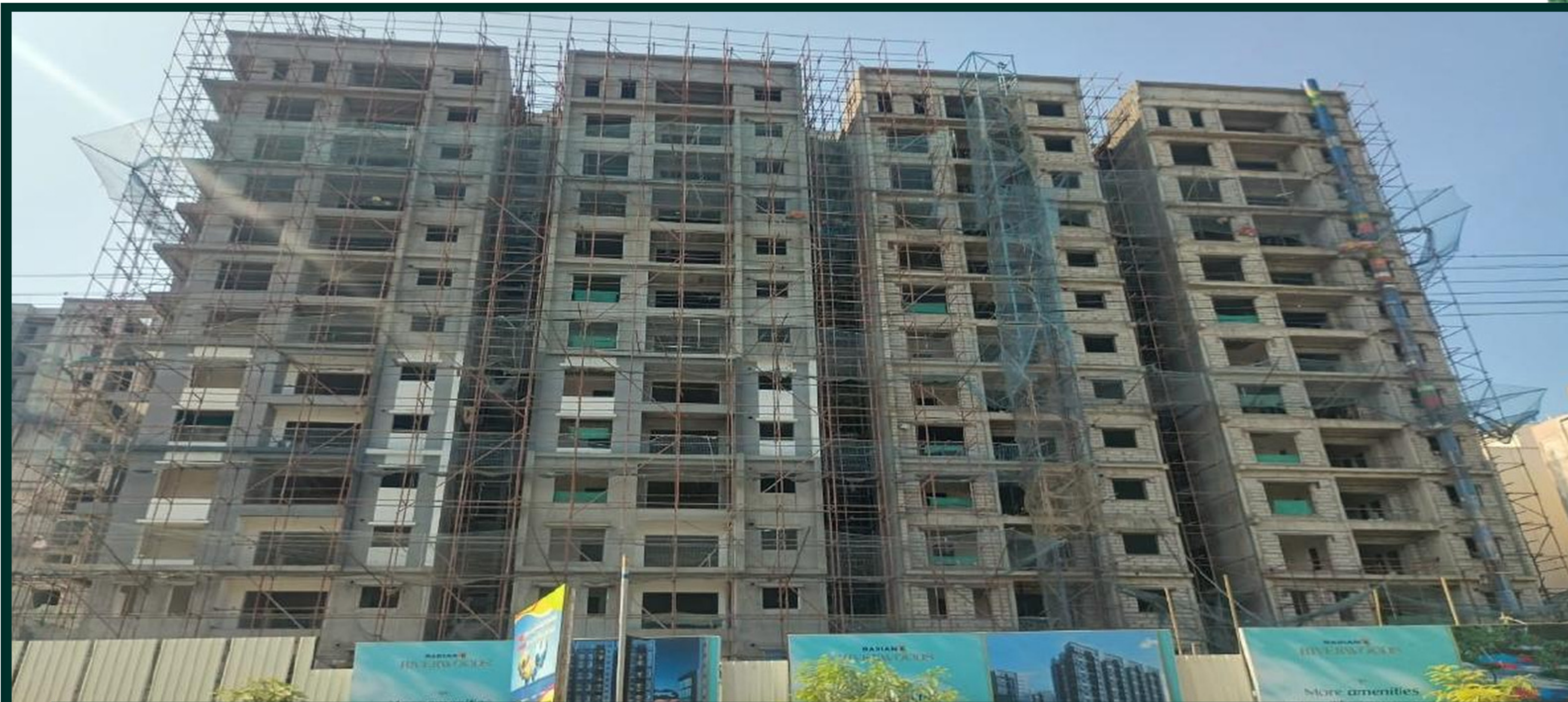
SITE OVERALL PROGRESS VIEW - TOWER 1.
