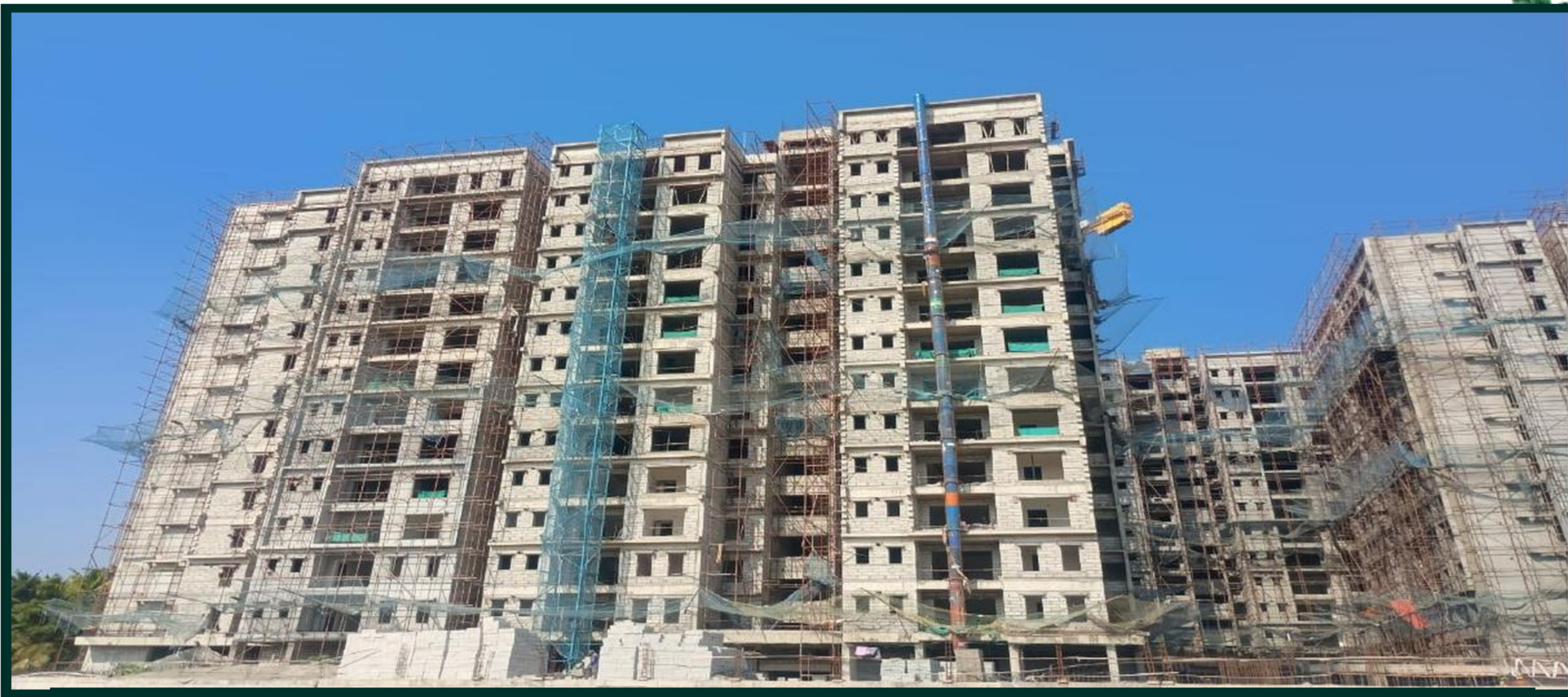
SITE OVERALL PROGRESS VIEW - TOWER 2.
