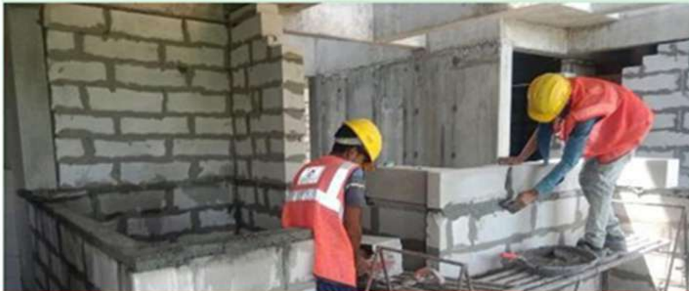
Block A – AAC Block Wall Works In The First To Fourth Floor Level
