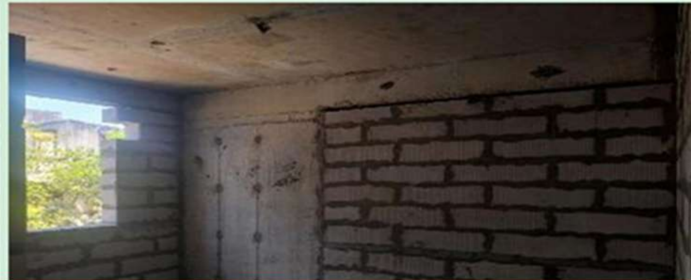
Block A – AAC Block Wall Works In The First To Fourth Floor Level
