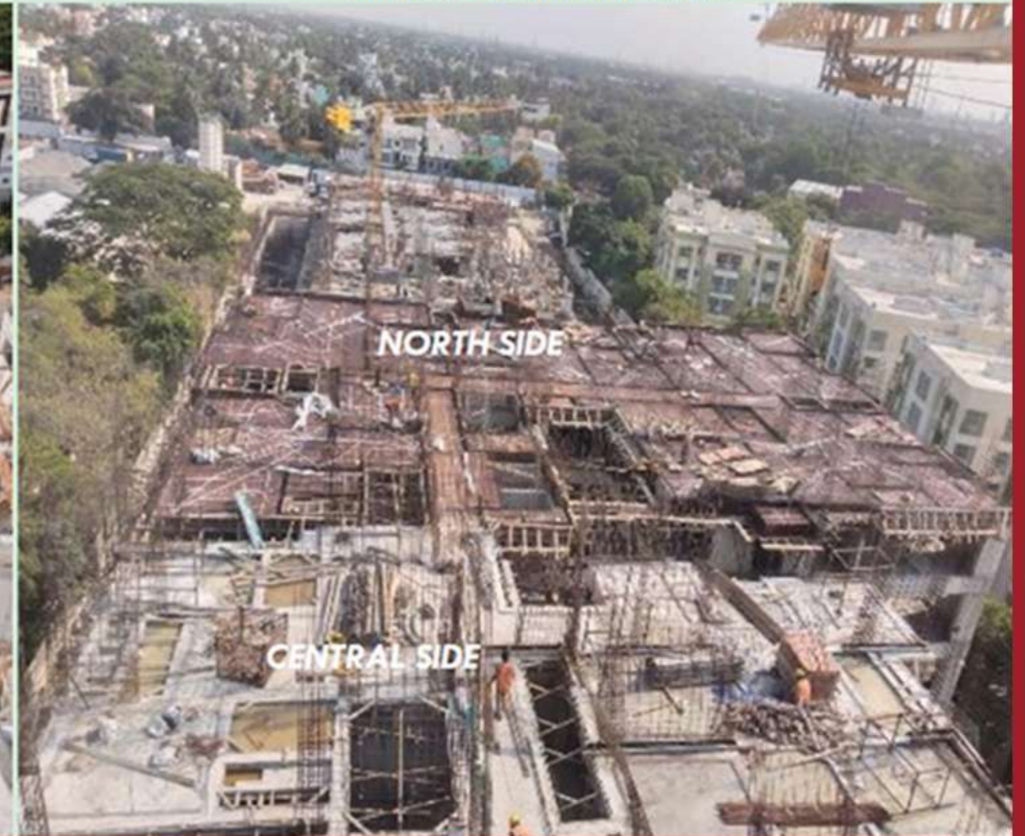
6th floor roof level works
