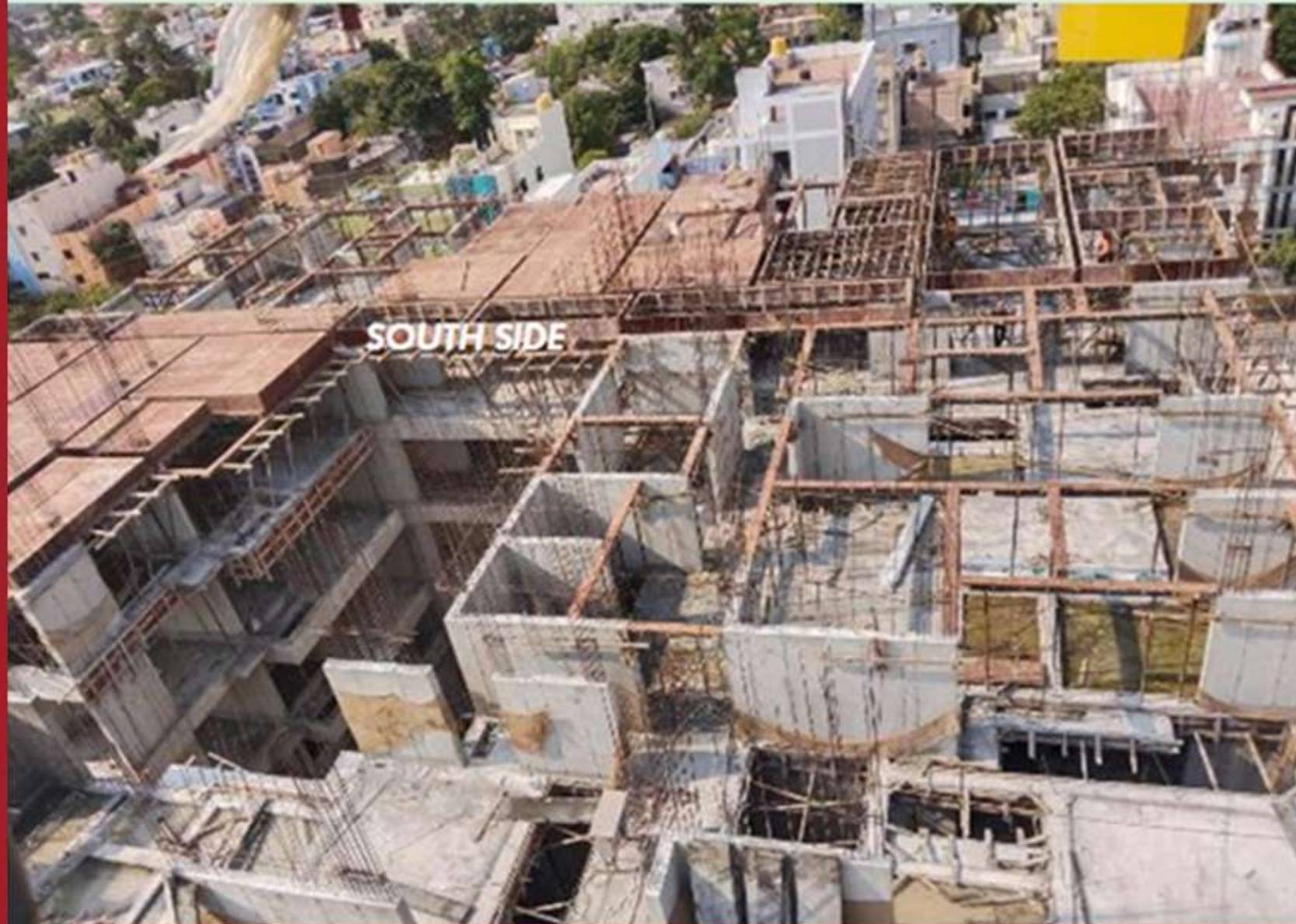
7th floor roof level works
