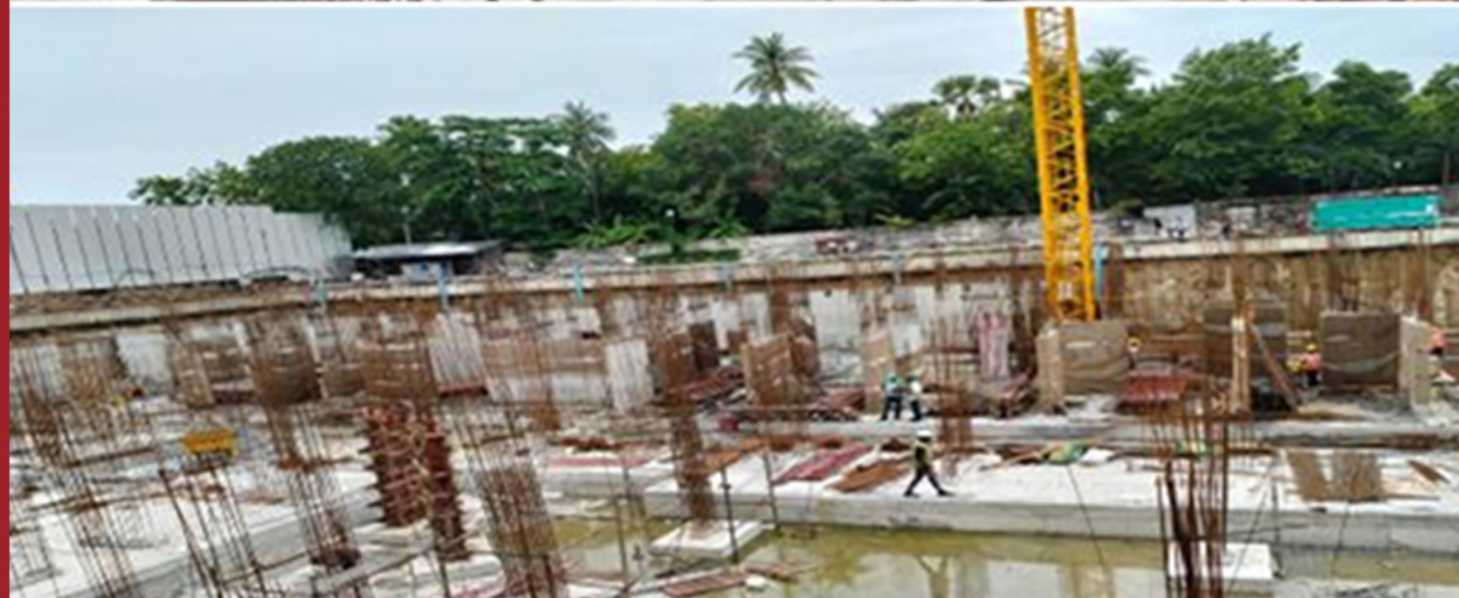
BLOCK A – RAFT PART 2 SOUTH EAST SIDE COLUMN & RETAINING WALL CONCRETE WIP
