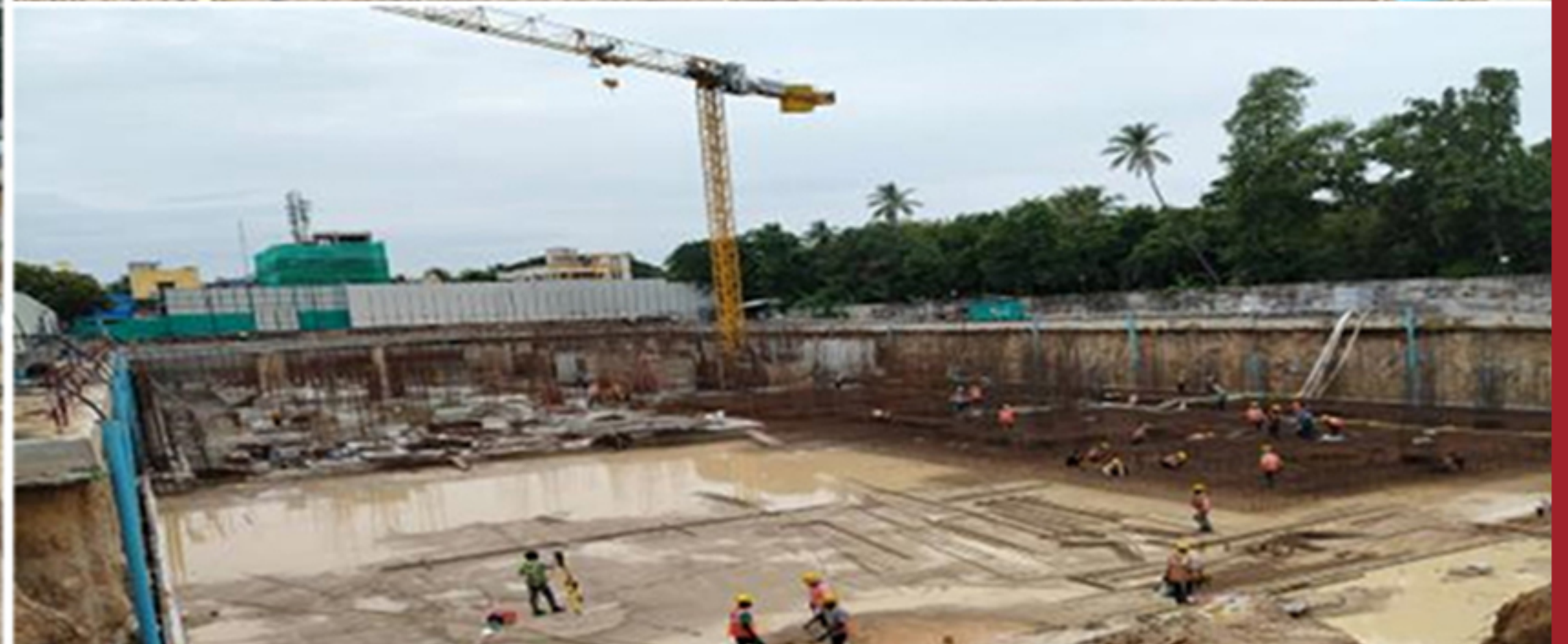
BLOCK A - PART 3 & 4 ( TILL CH JUNCTION ) WATERPROOFING COMPLETION AND RAFT REINFORCEMENT WORK
