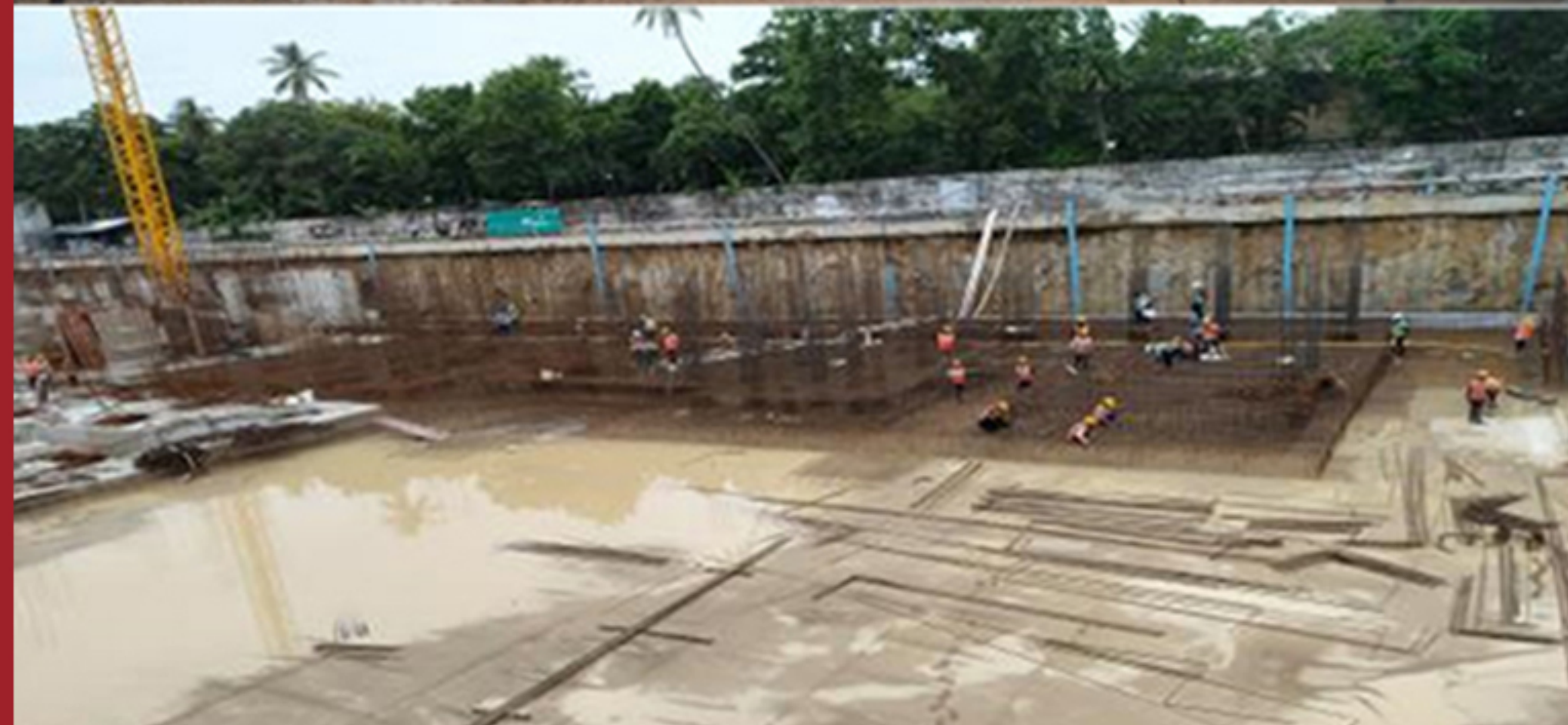
BLOCK A - PART 3 & 4 ( TILL CH JUNCTION ) WATERPROOFING COMPLETION AND RAFT REINFORCEMENT WORK
