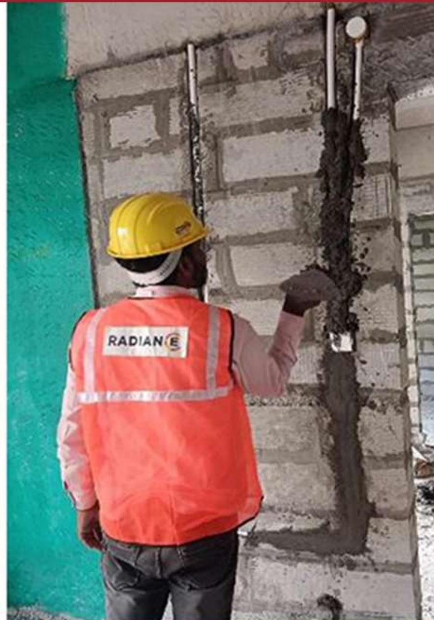
Block B : 1st – 4th Floor Aac Block Works , Lintel Concrete , Electrical Conduit Works In Progress & 1st Floor Plastering Wip
