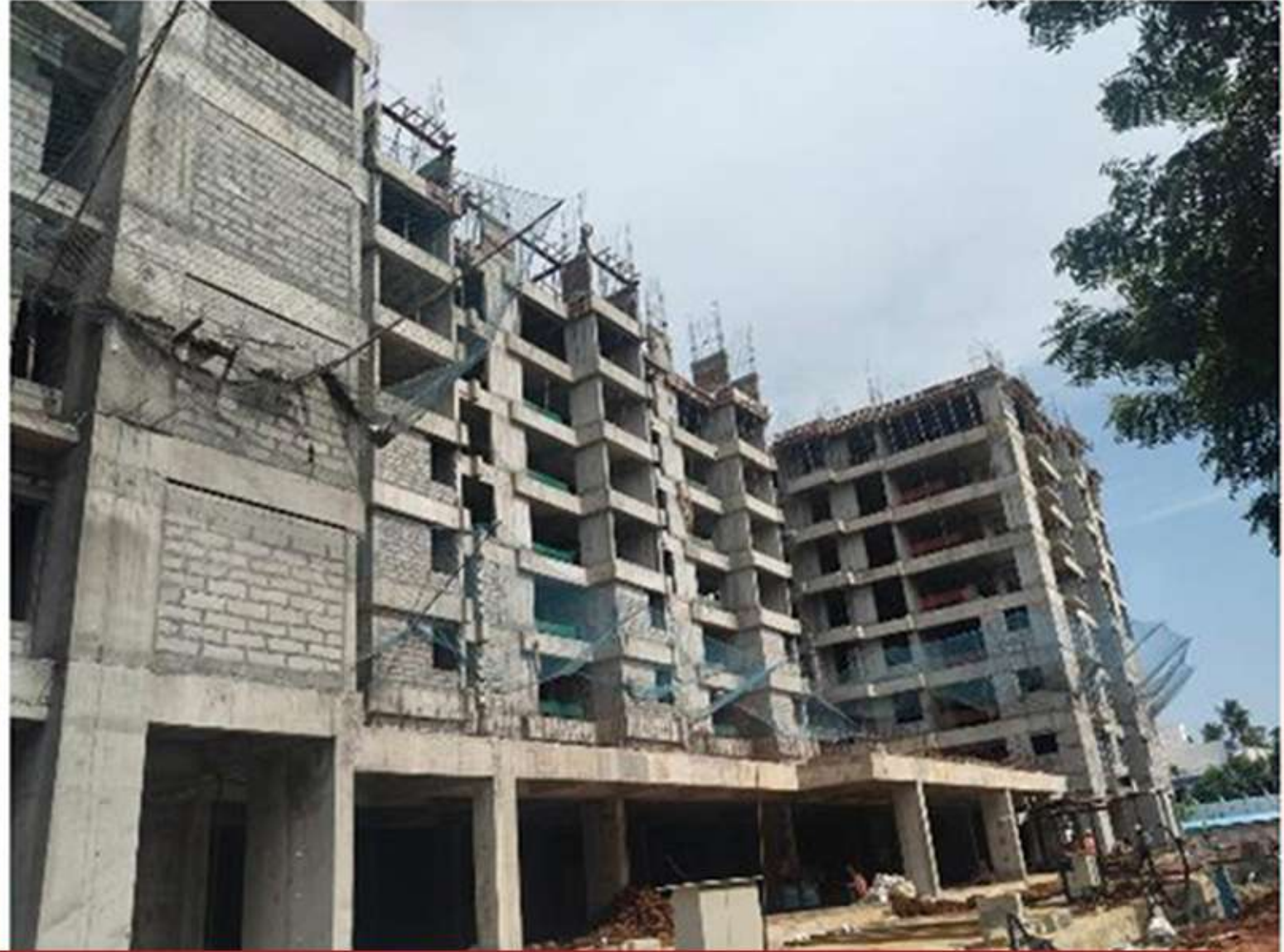
TOWARDS NORTH EAST SIDE
