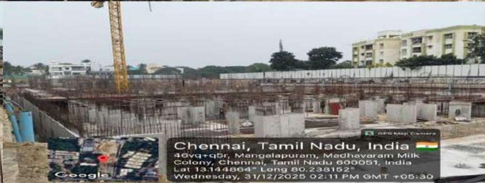
B2 ROOF SLAB LEVEL / lower basement – columns & Retaining wall works are completed . north side slab completed.
