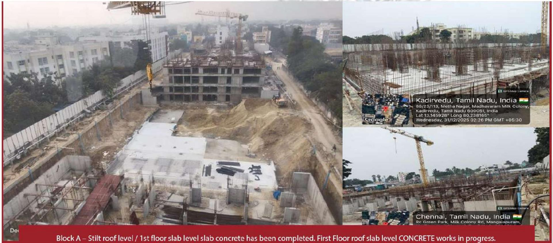
Block A – Stilt roof level / 1st floor slab level slab concrete has been completed. First Floor roof slab level CONCRETE works in progress.
