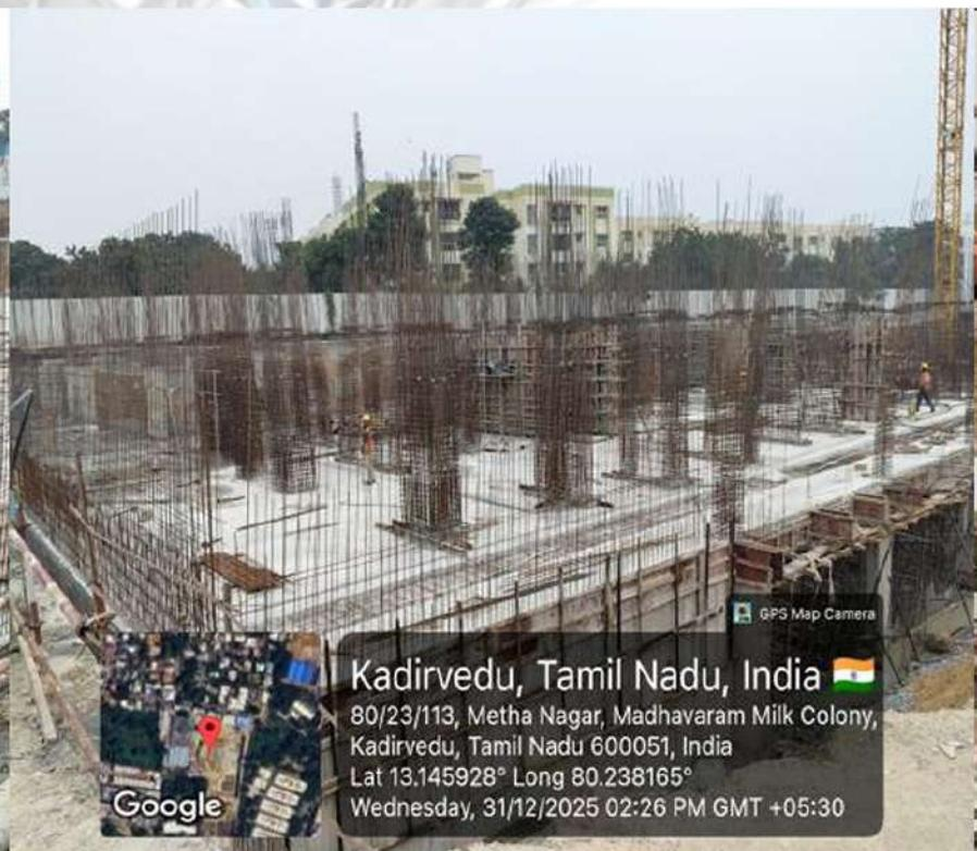
B1 ROOF SLAB LEVEL / upper basement area - north side columns and retaining wall works IN PROGRESS.
