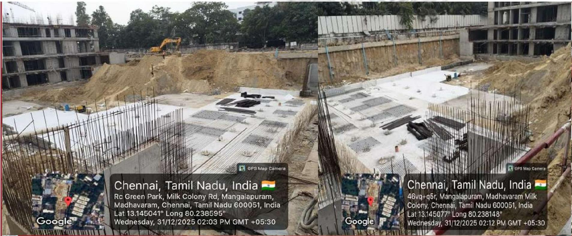
Block D / Club house – final part excavation works and raft-level pcc and waterproofing works in progress.
