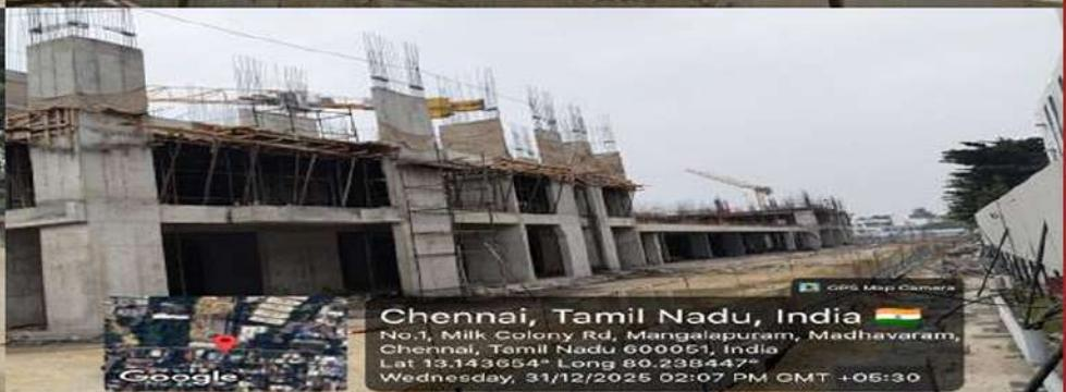
Block A – substructure works are completed and Stilt roof level / 1st floor slab concrete has been completed.
