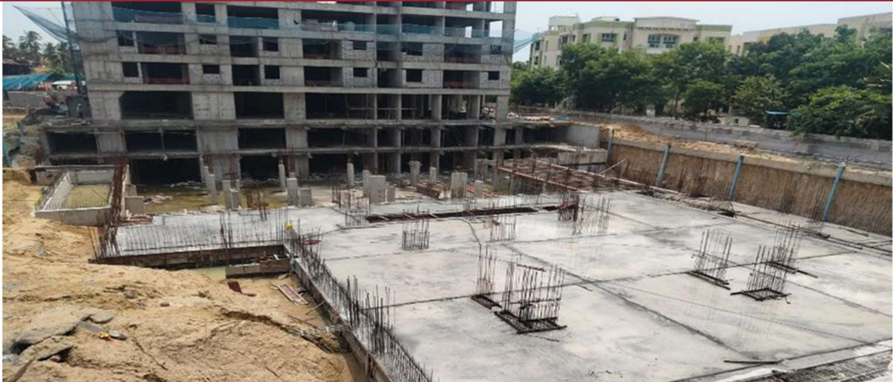
Block D / Club House –raft-rcc Works Has Been Completed b2 Level - Columns & Retaining Wall Concrete Works Are Completed. B2 Roof Level Slab Concrete South Side Completed & north Side Shuttering Works In Progress. External Waterproofing Works Completed.
