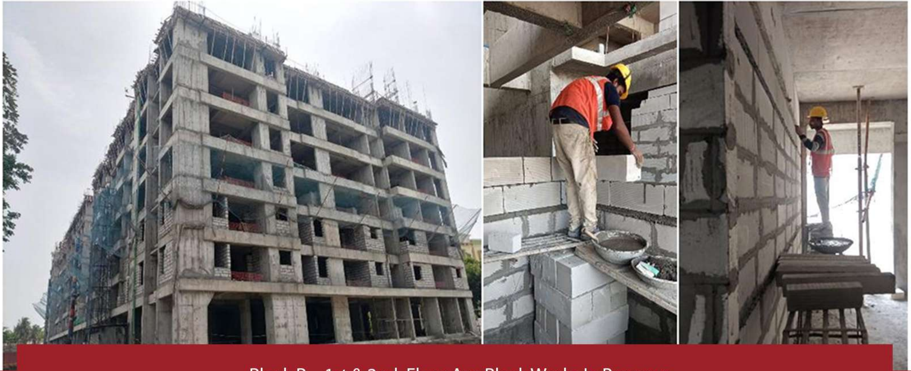
Block B – 1st & 2nd Floor Aac Block Works In Progress
