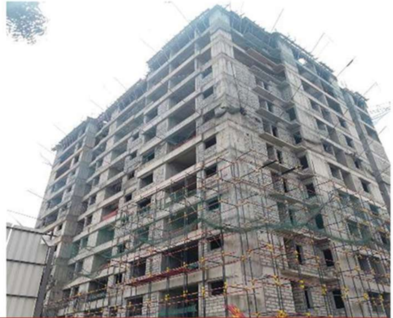
SOUTH SIDE EXTERNAL SCAFFOLDING WORKS
