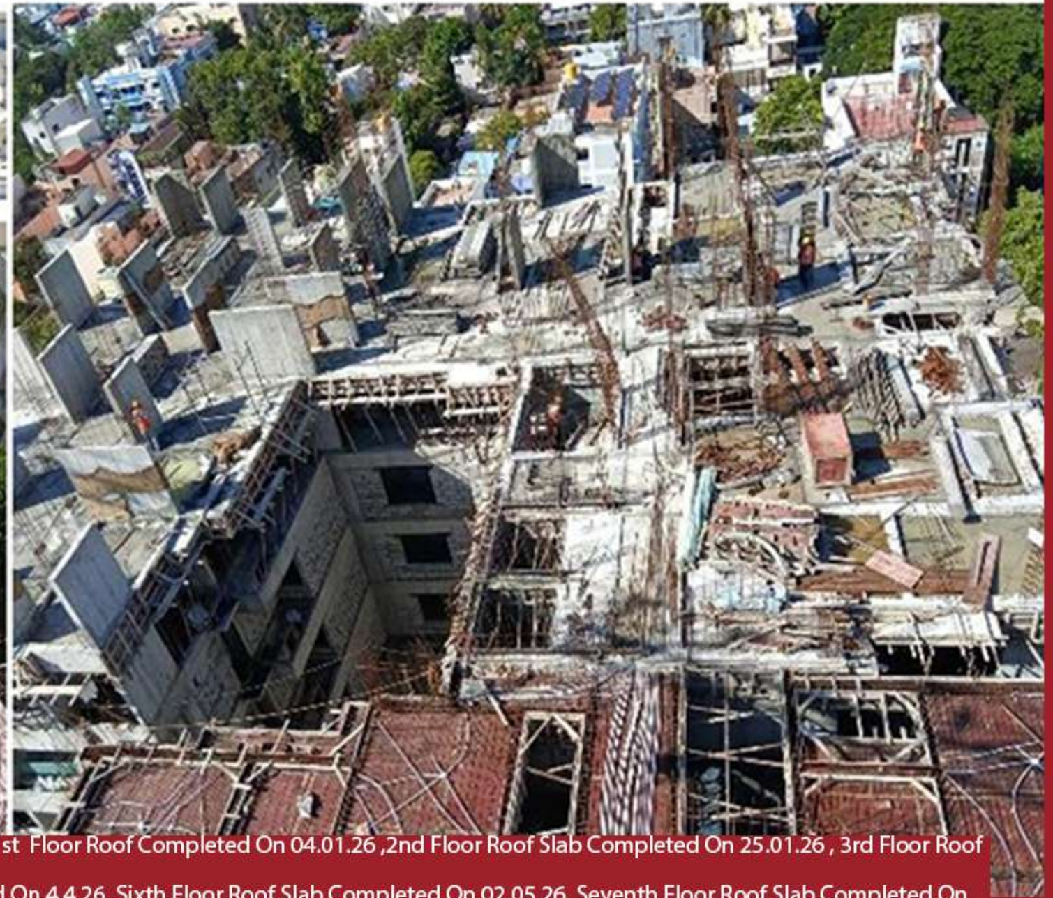
10 th floor roof – South Side
