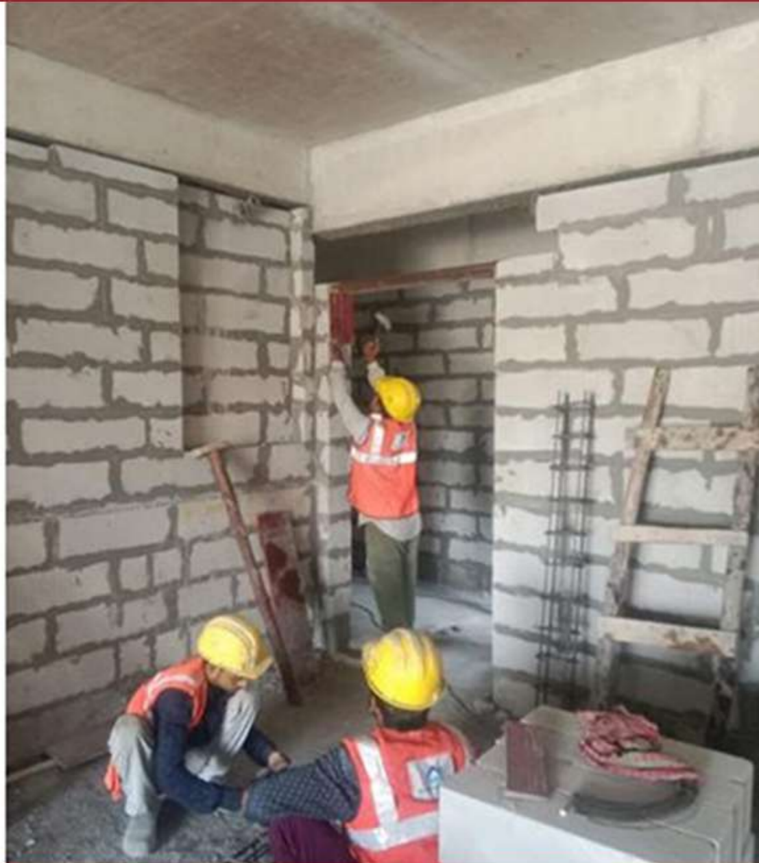
Block A – Aac Block Works ( 1- 6th Floor ) & Lintel Concrete Works lintel Concrete Works ( 1 St Floor ) Completed And Electrical Wall Chasing & Conduit Instalation Wip
