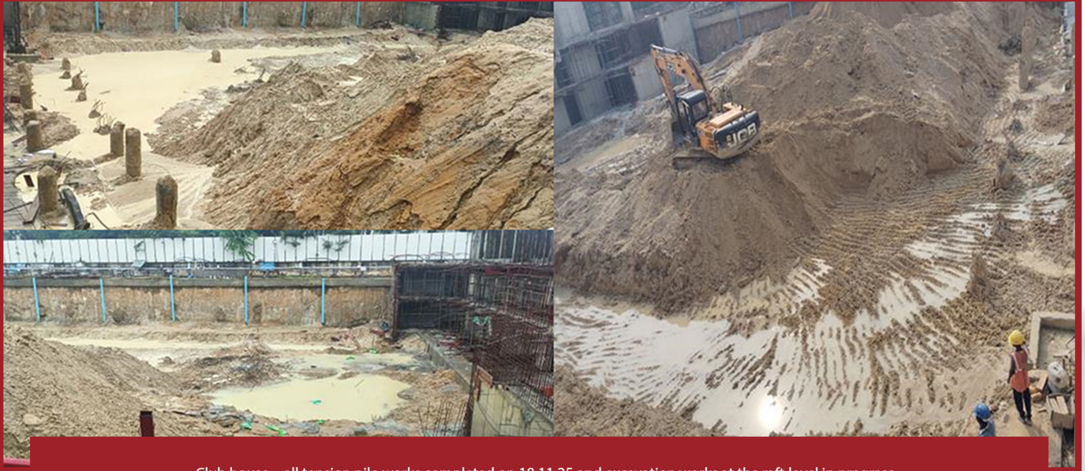
Club house – all tension pile works completed on 18.11.25 and excavation works at the raft level in progress.
