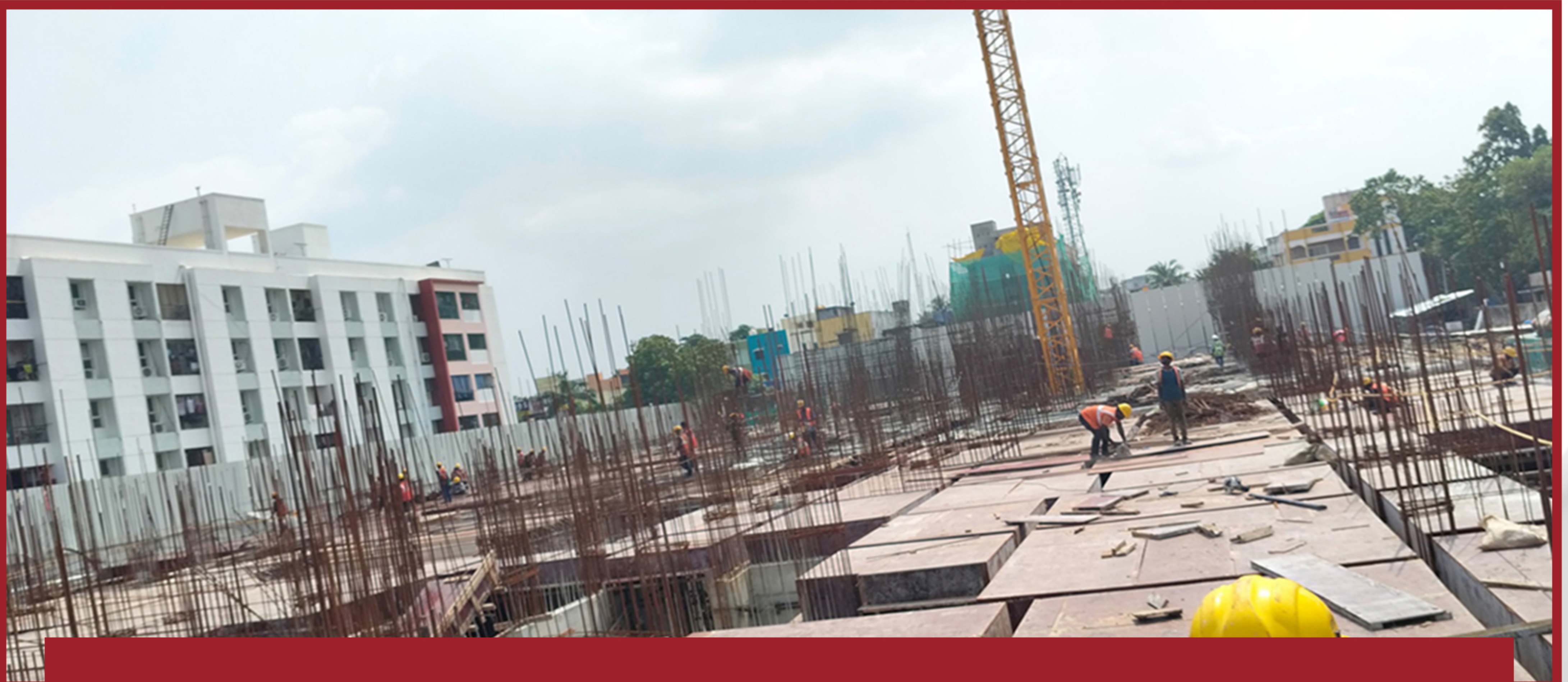
Block a - B1 roof slab / stilt floor slab shuttering and reinforcement works at north west side.
