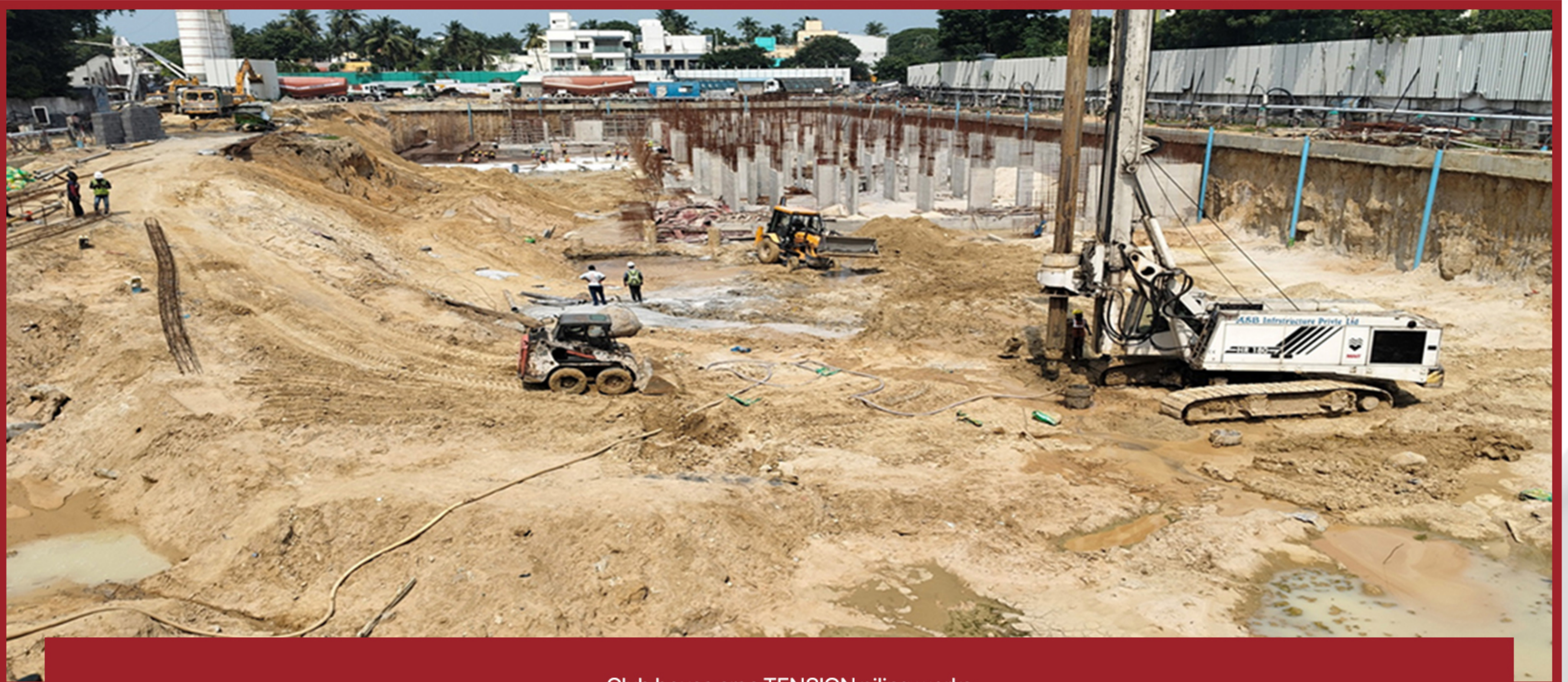
Club house area TENSION piling works
