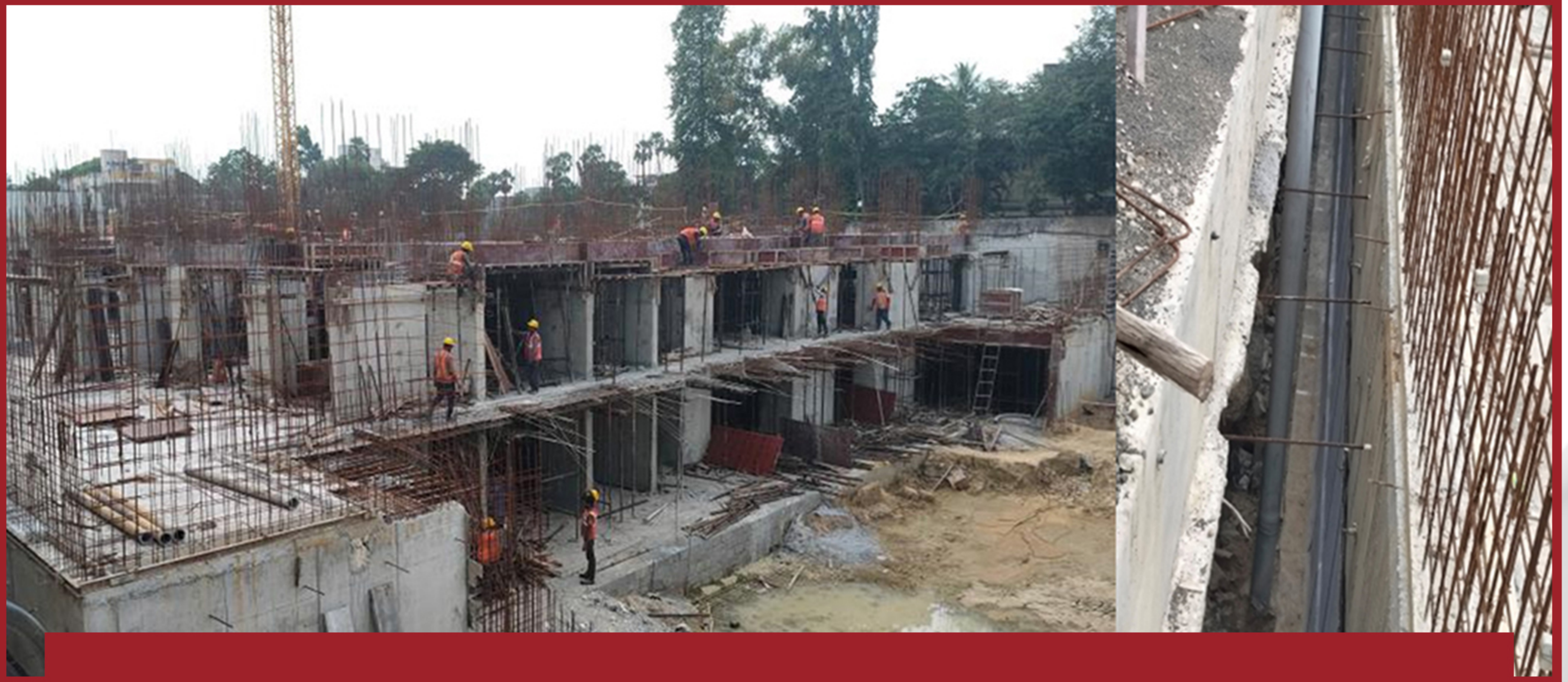
Block a - B1 roof slab / stilt floor slab shuttering works & retaining wall water proofing at north west side.
