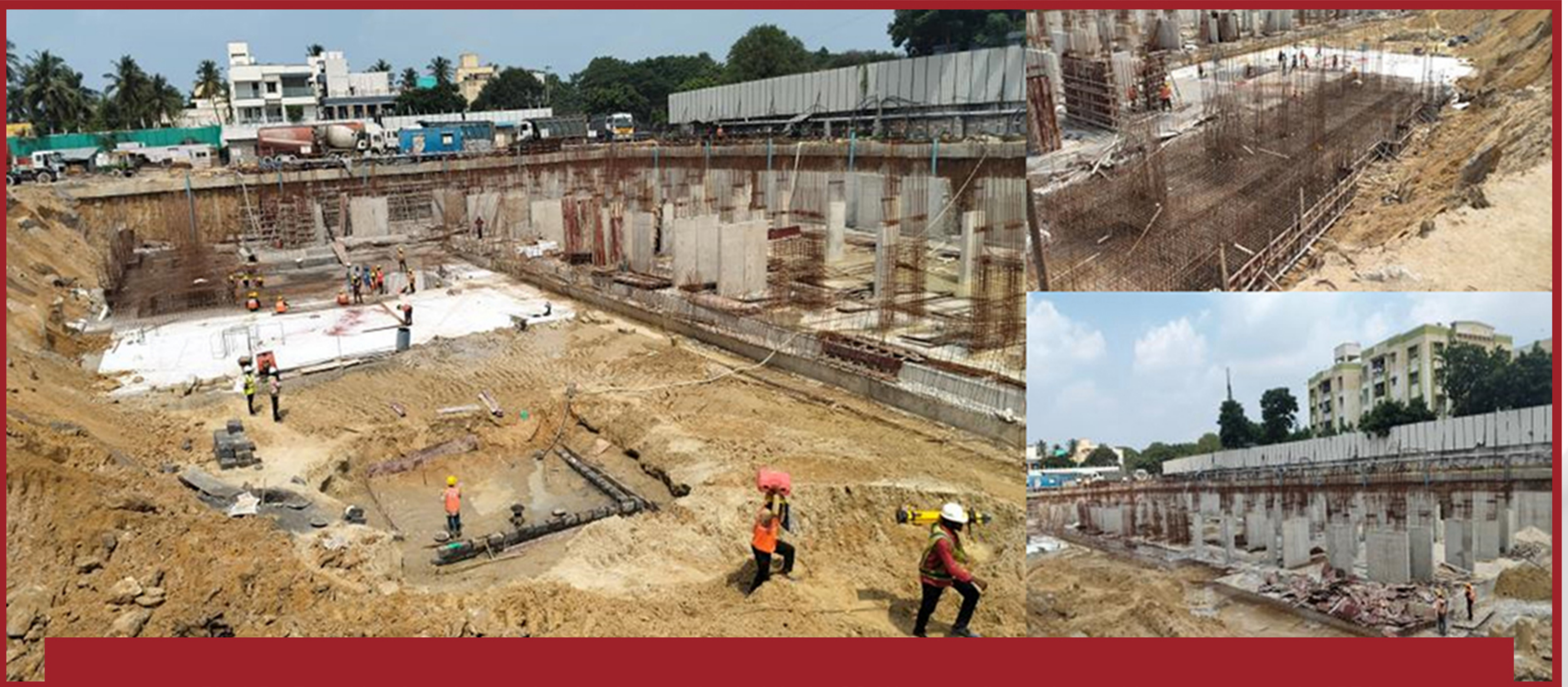
Block B – East side raft works completed and west side wip. Lift pit pCC, Water proofing and west side excavation works AREA
