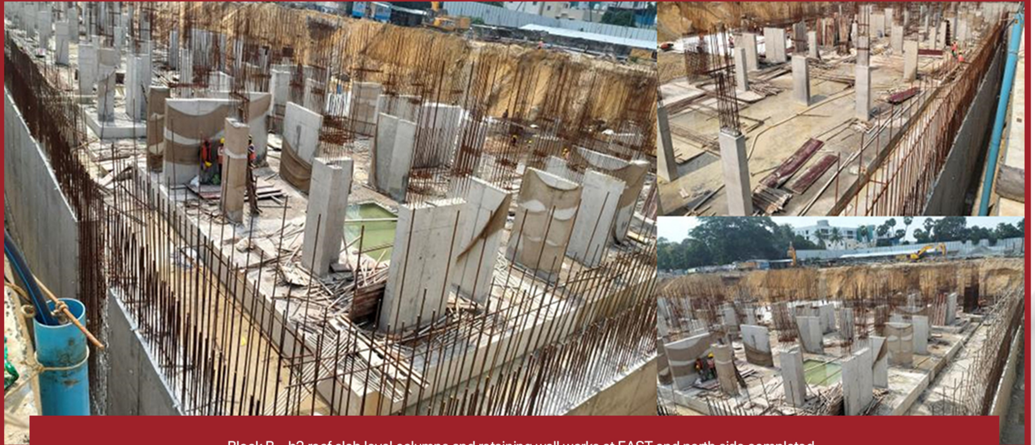
Block B – b2 roof slab level columns and retaining wall works at EAST and north side completed EXCAVATION AND RAFT-rCC WORKS in progress AT WEST SIDE
