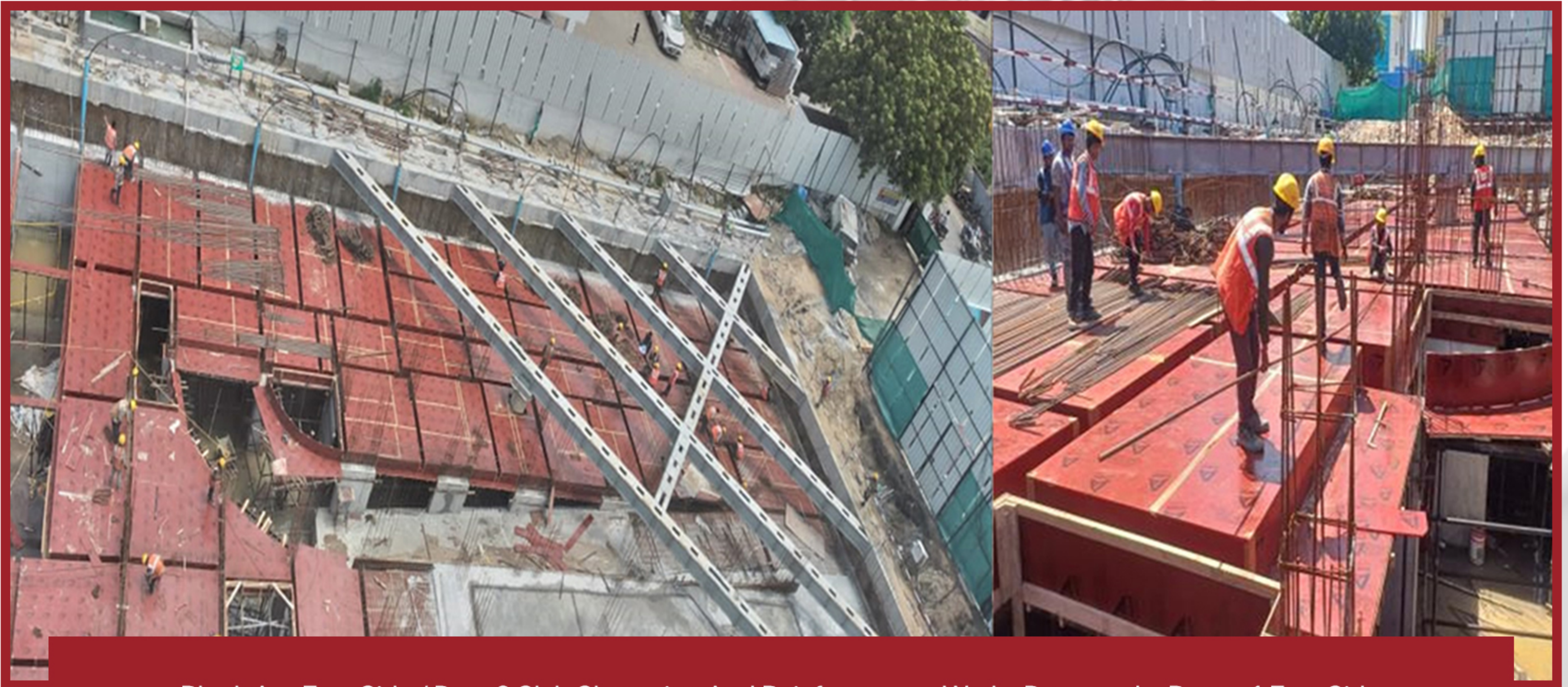
Block A - East Side / Pour 2 Slab Shuttering And Reinforcement Works Progress In Ramp 1 East Side
