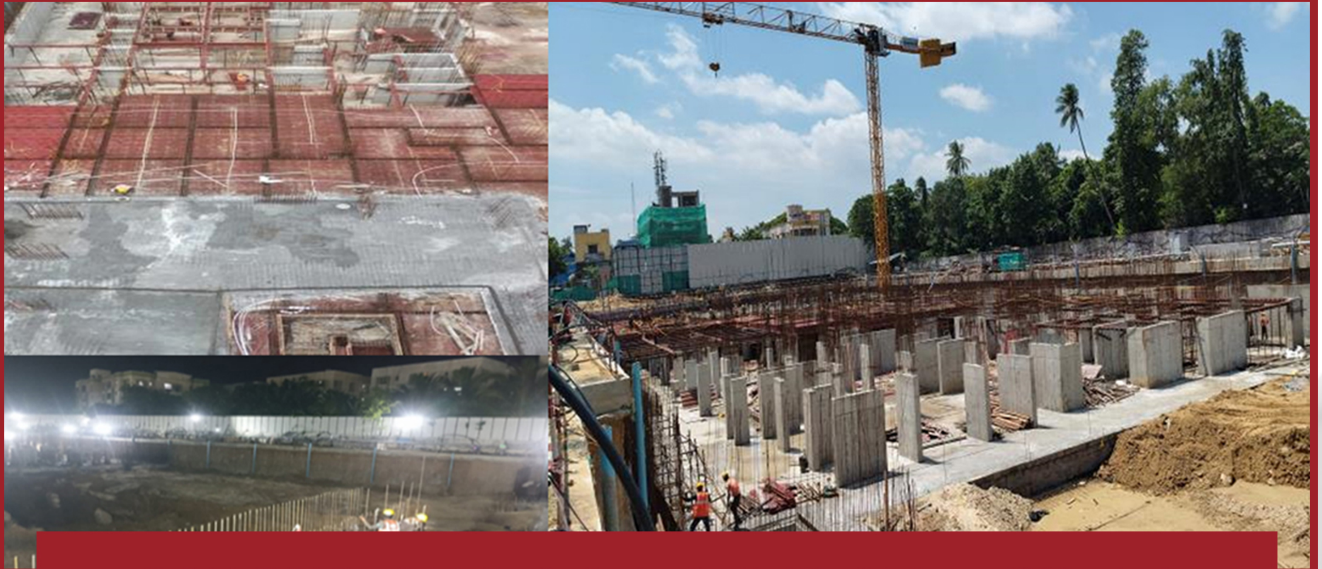
Block A Soil Filling Above Raft And Levelling Pcc Completed And West Side Retaining Wall Completed
