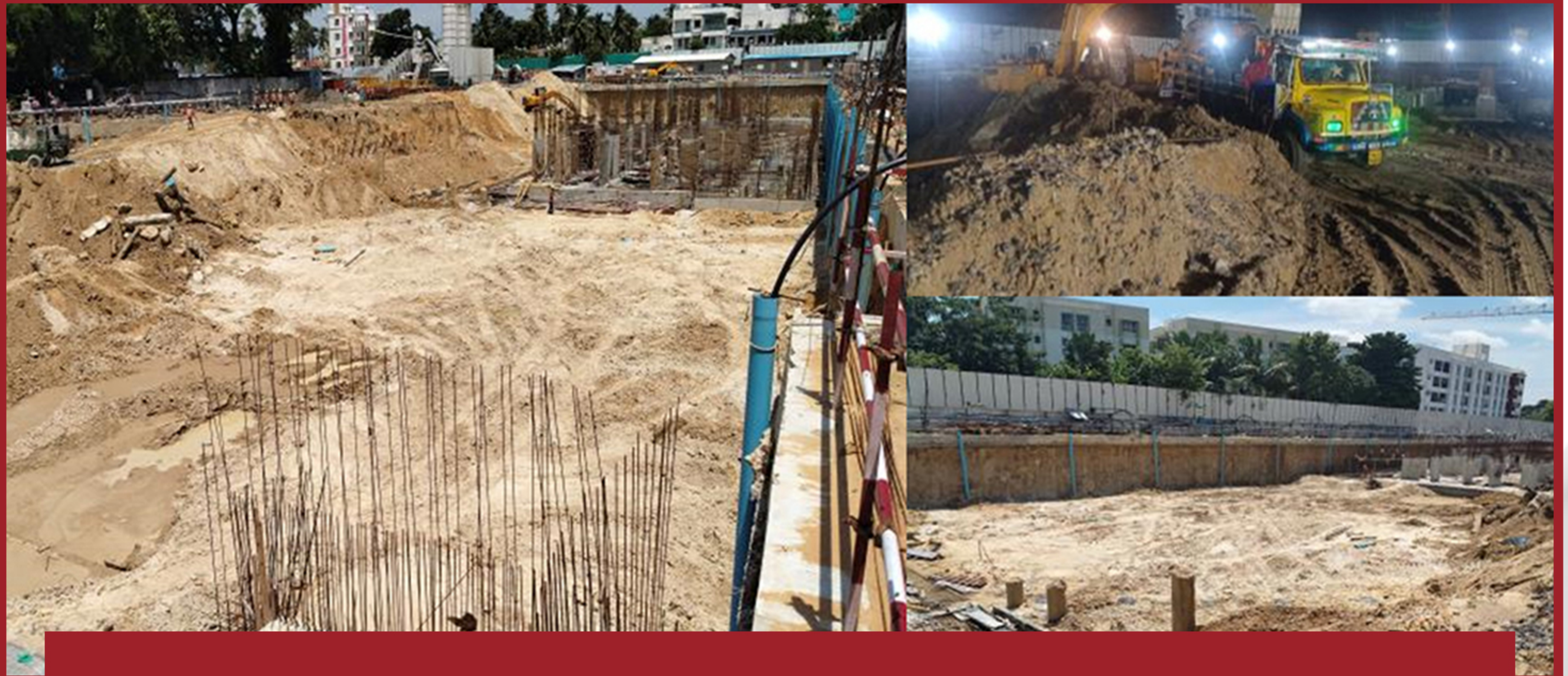
Club house area excavation works in progress
