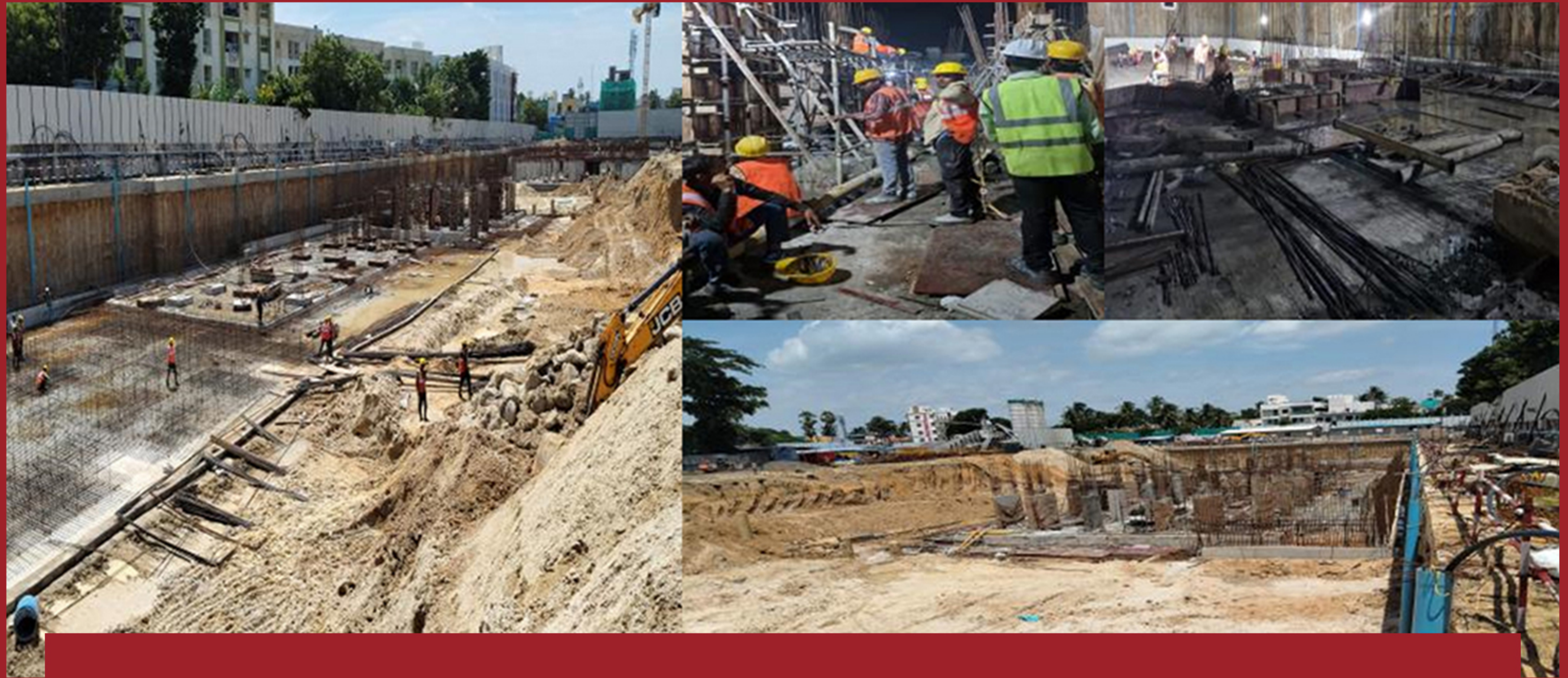
Block B – Raft Rcc Part 1 / Se Side Completed / Retaining Wall & Column Wip
