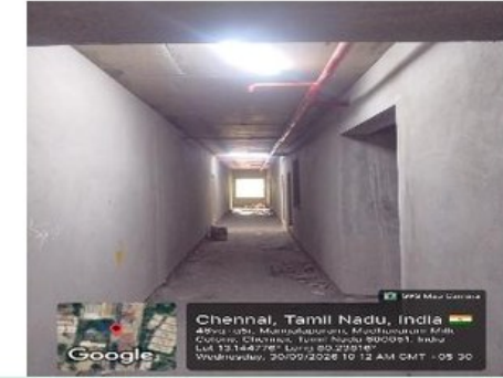
Electrical conduit and DB box works
