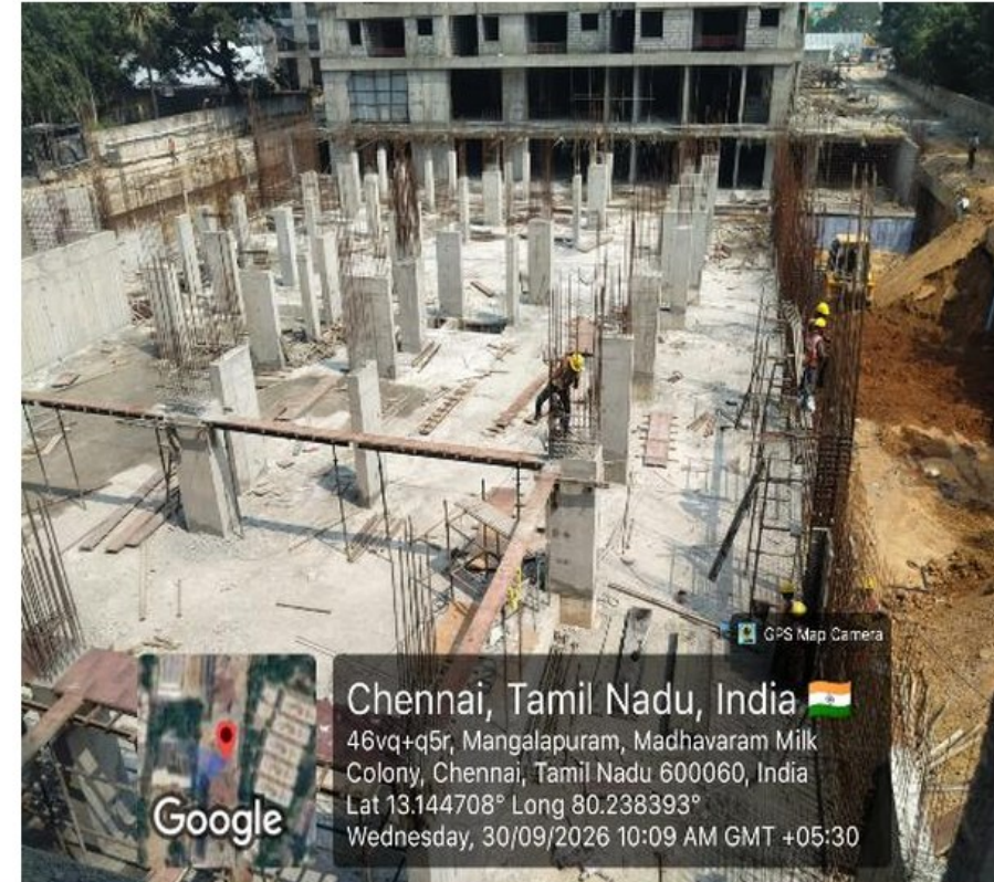
Clubhouse: Lower basement completed; upper basement / stilt slab in progress
