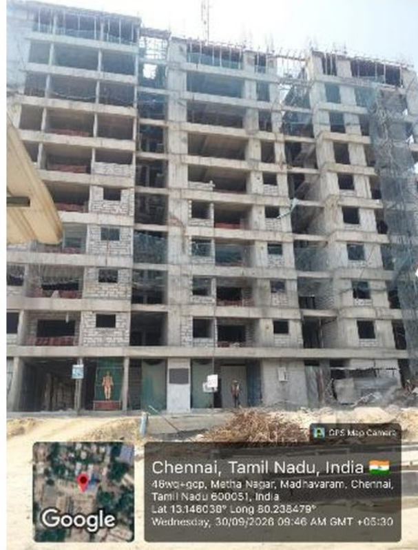
First-floor waterproofing works
