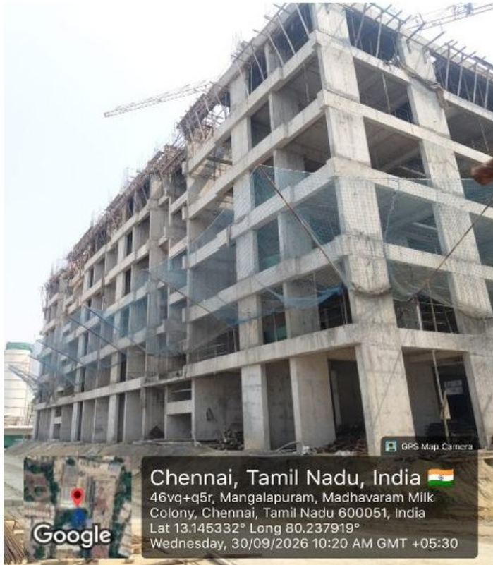
5th floor completed; 6th floor works in progress
