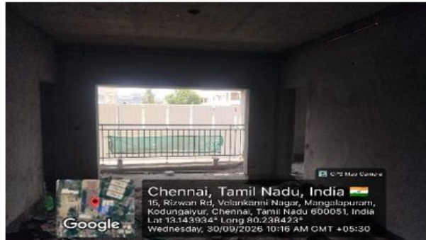
Interior finishing and waterproofing
