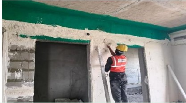
AAC block / wall finishing
