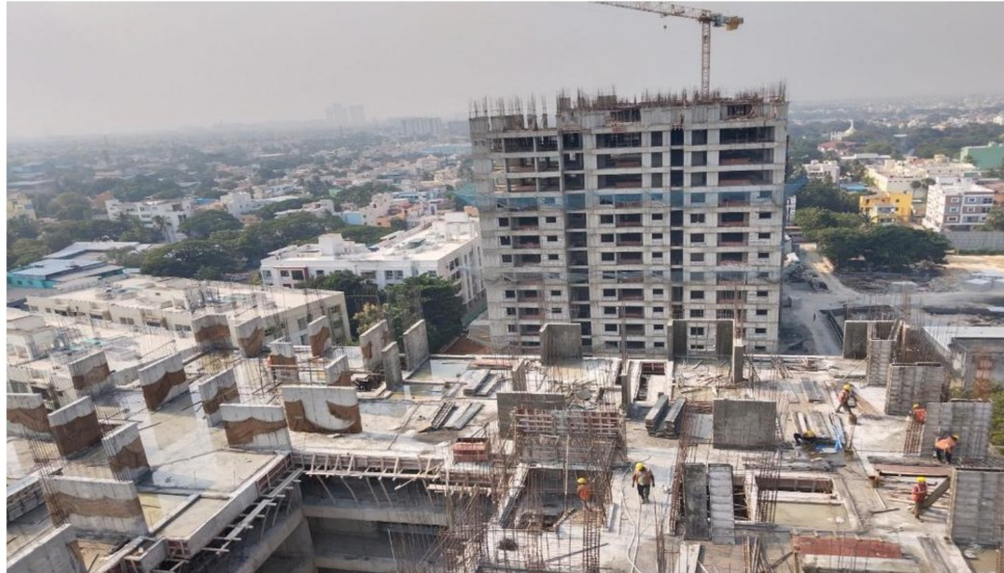
Block B, Clubhouse and Block A - overall construction view
