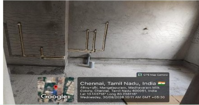
Wall plastering and gypsum works
