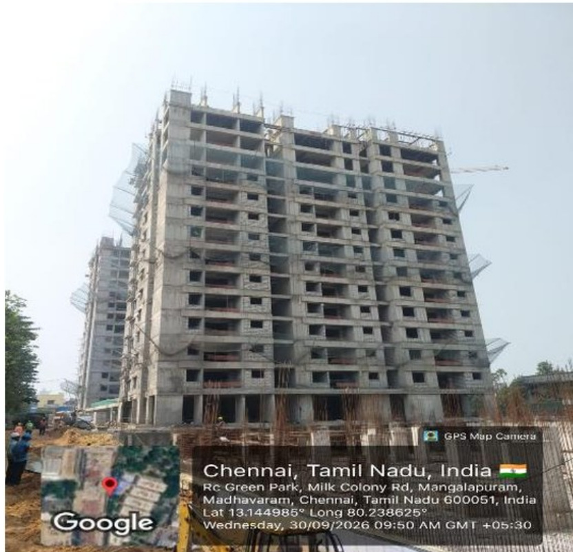
Tower A: 13th floor completed; 14th & 15th floor works in progress
