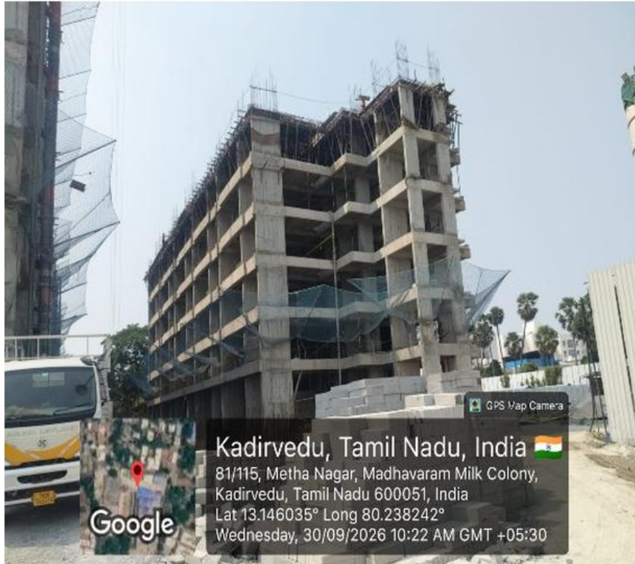
Tower C: 5th floor completed; 6th floor works in progress
