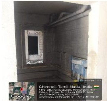
PHE plumbing first-fix works
