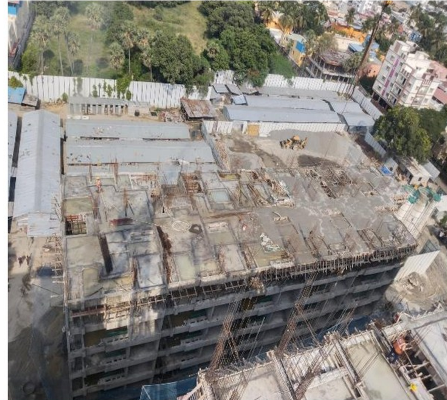
Roof slab works – aerial view
