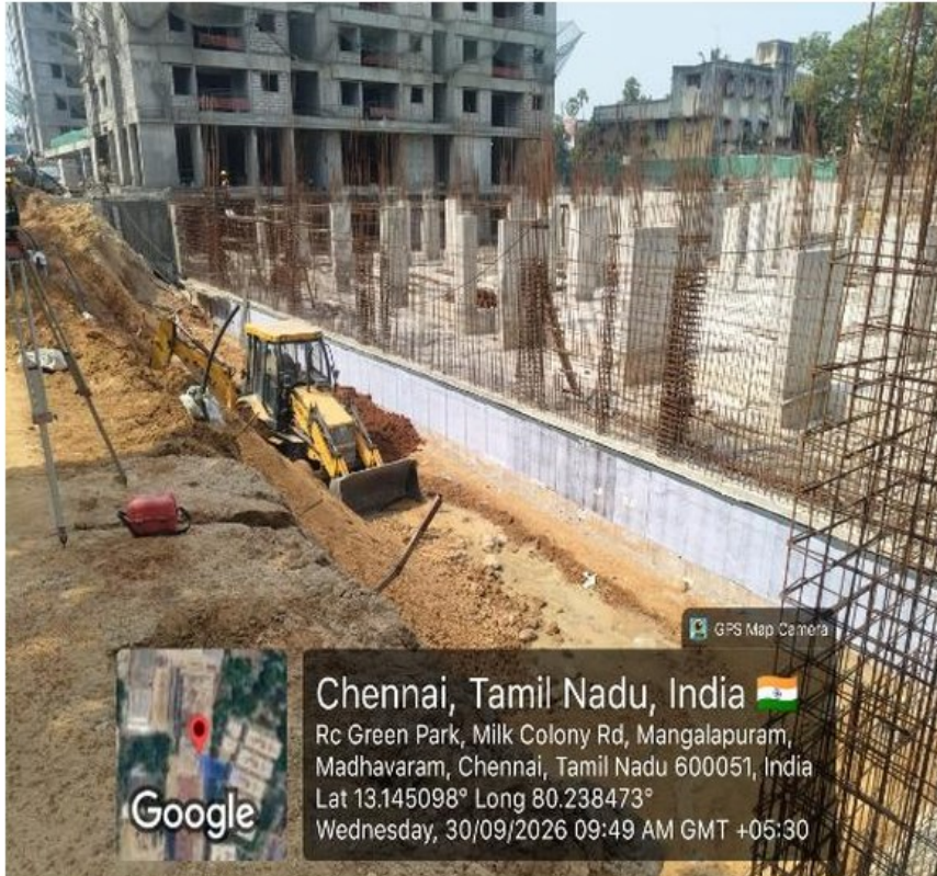
STP: B2 slab completed; B1 cover slab works in progress
