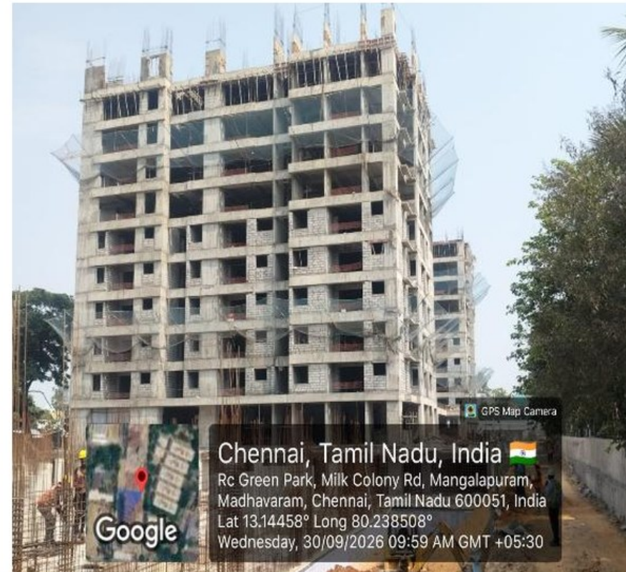
Tower B: 8th floor completed; 9th floor works in progress
