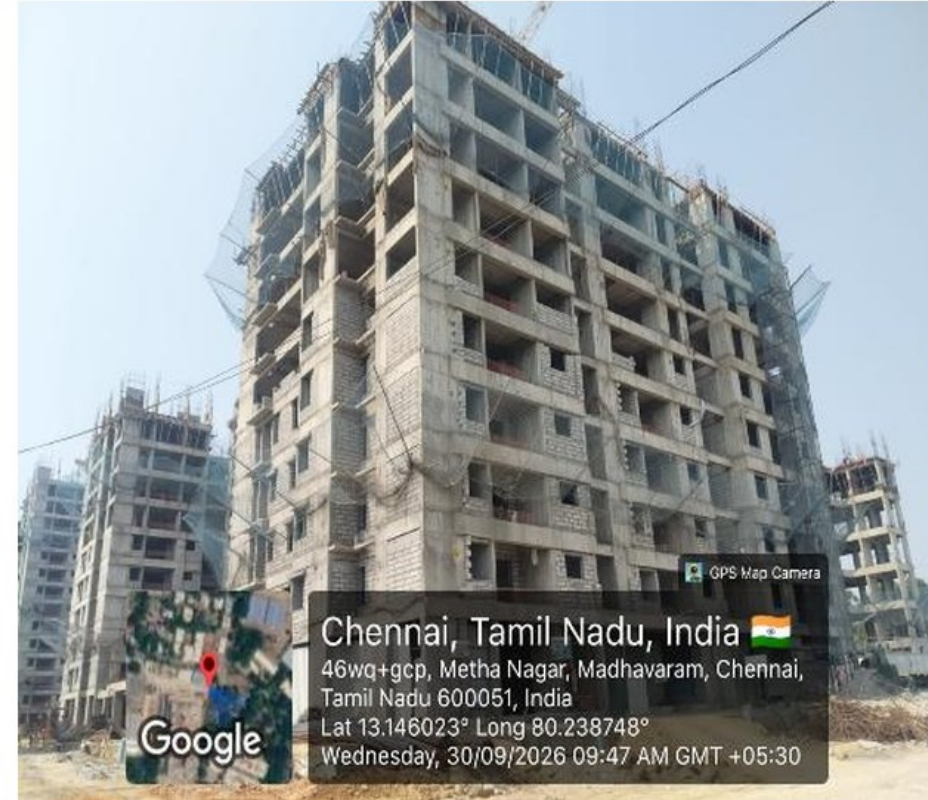
8th floor completed; 9th floor slab works in progress
