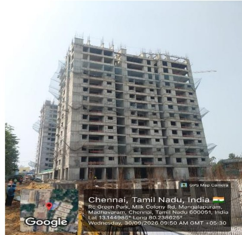
8th floor completed; 9th floor slab works in progress
