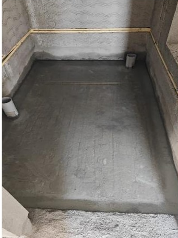
Plastering and electrical conduit works
