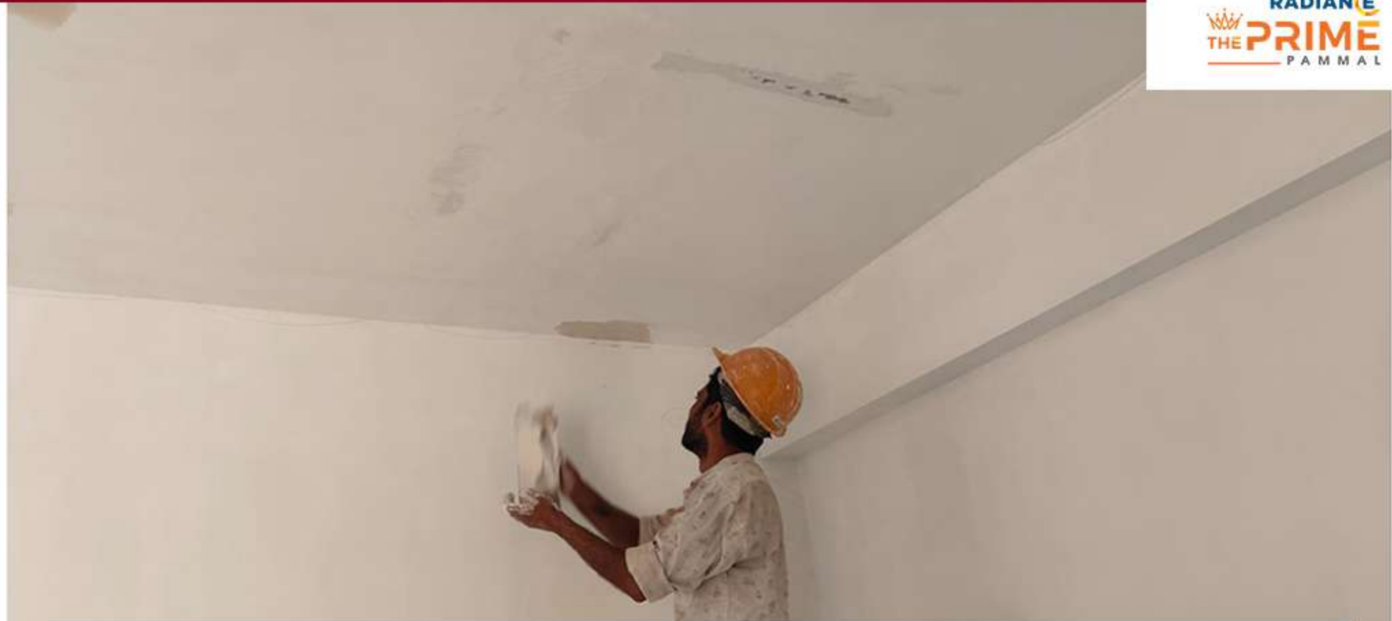
Ceiling Corner Correction
