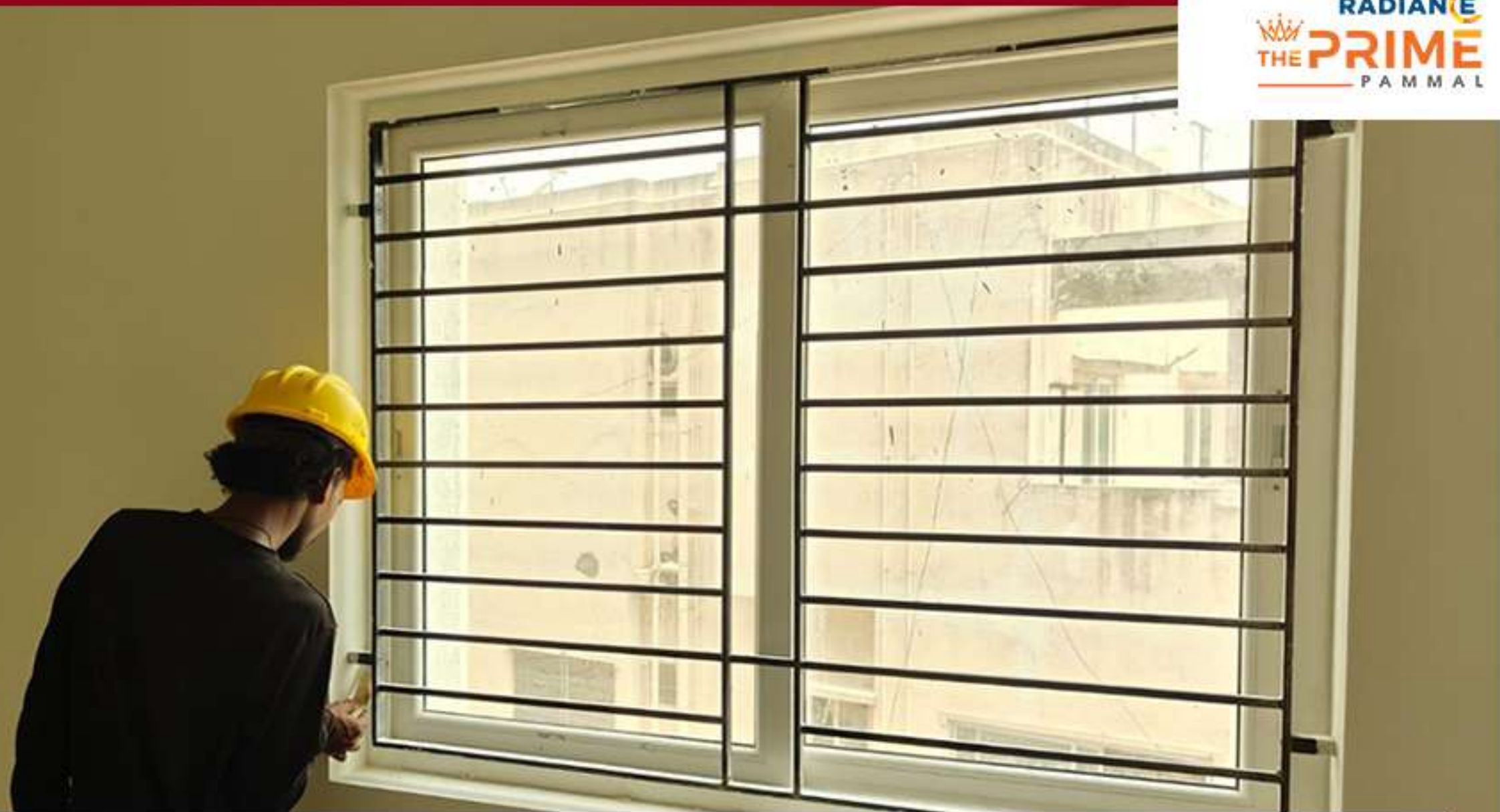
UPVC Sealant Work
