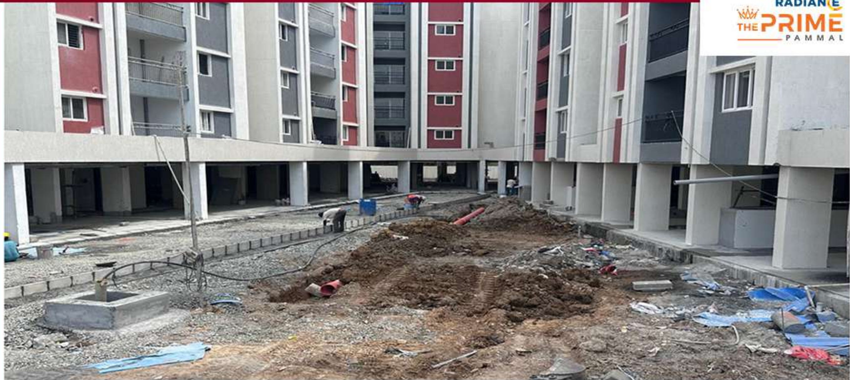
Triangle portion Kerb Stone Laying Work
