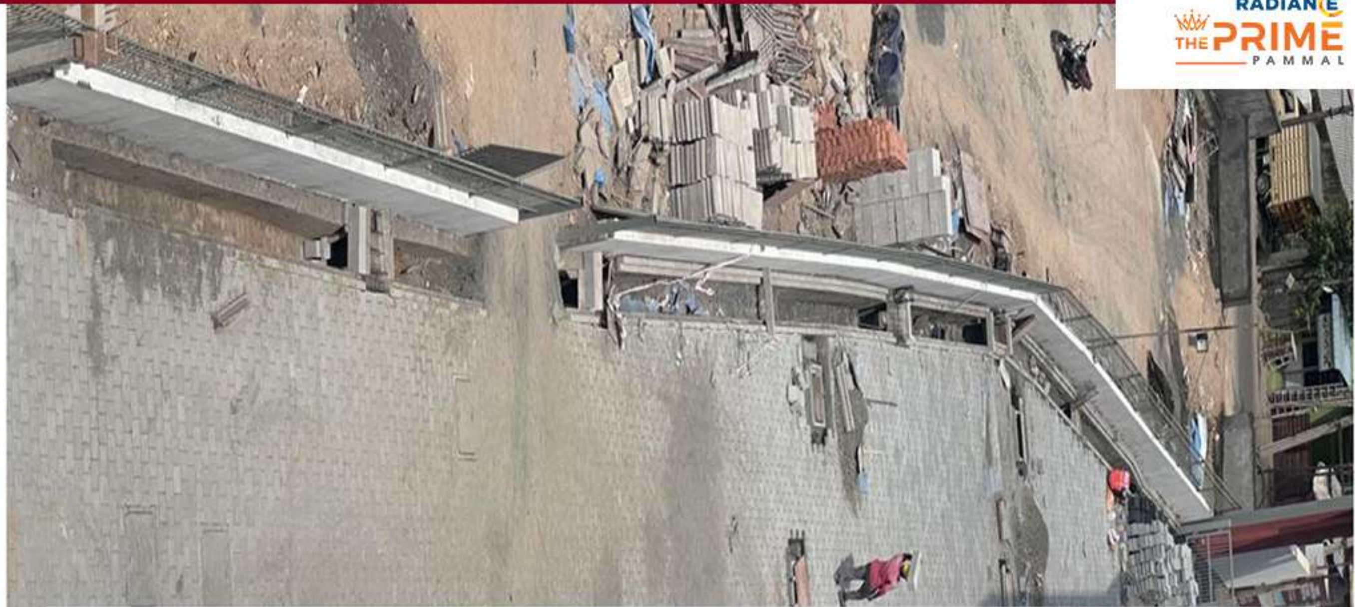
OSR Compound Wall & Grill Work
