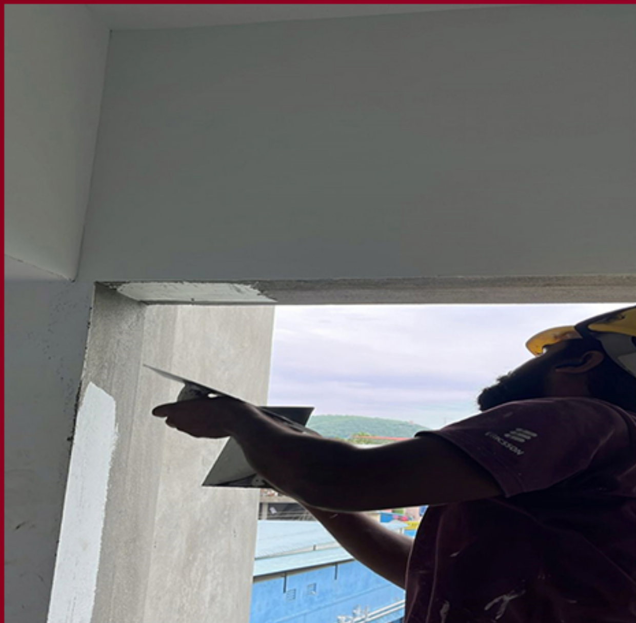
BLOCK 3 –CLUSTER J CORRIDOR & INTERNAL FLAT PUTTY WORK IN PROGRESS
