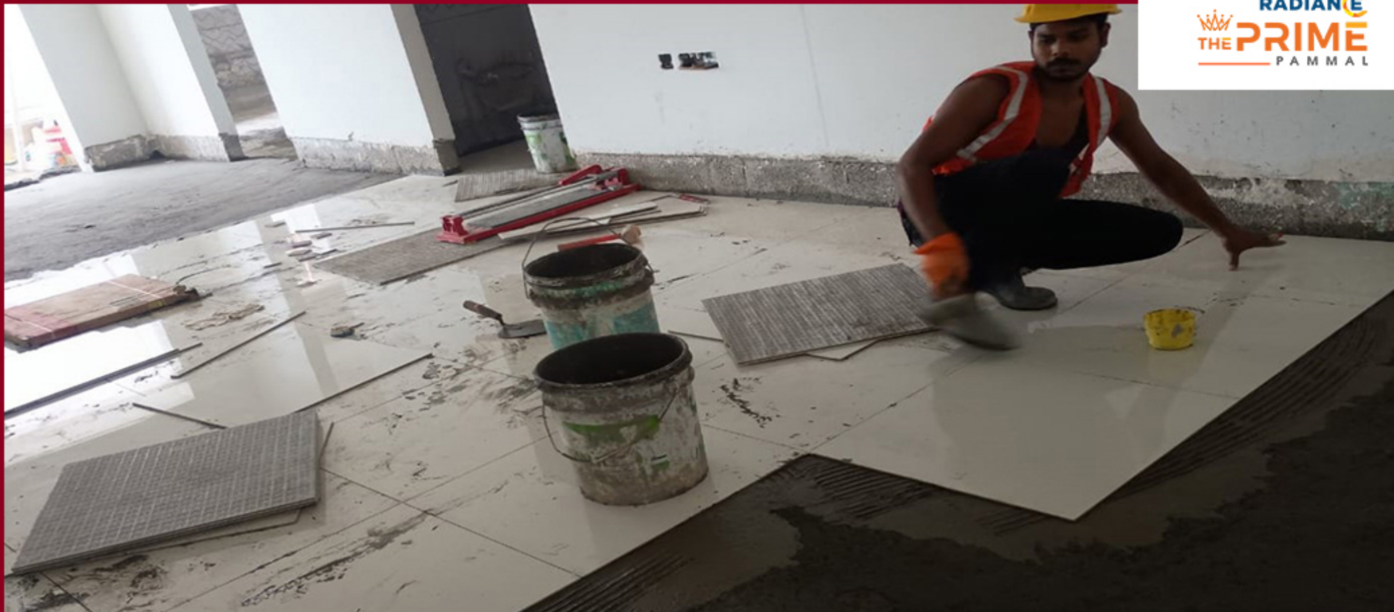
BLOCK 1 – CLUSTER F TILE LAYING WORK IN PROGRESS
