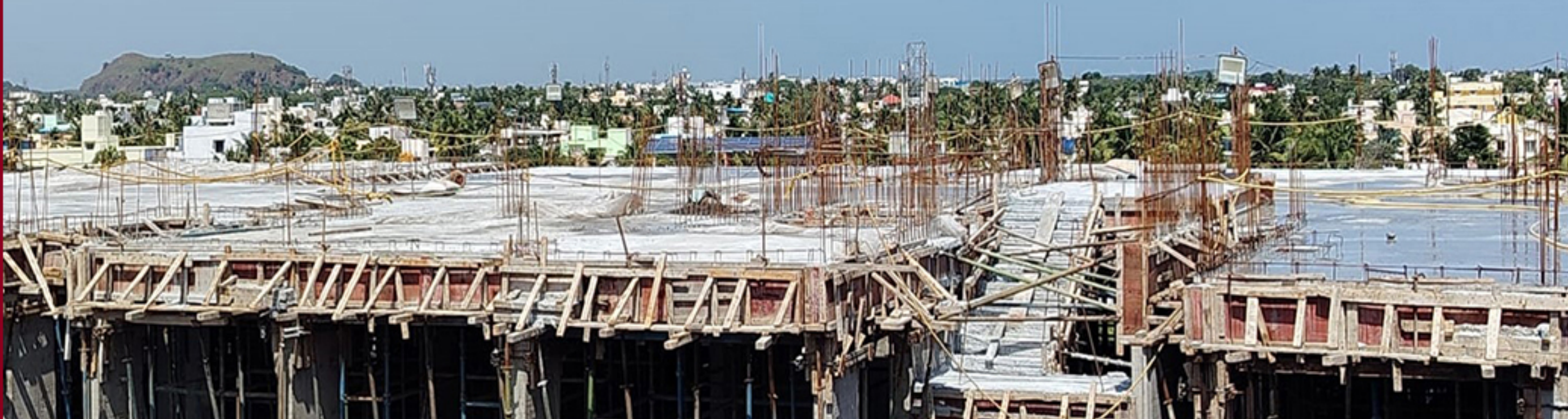
BLOCK 1 –CLUSTER A 5TH FLOOR ROOF SLAB COMPLETED
