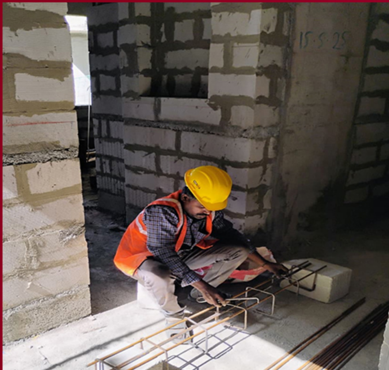
BLOCK 1 –CLUSTER B 1ST,2ND & 3RD FLOOR BLOCK WORK & LINTEL WORK IN PROGRESS
