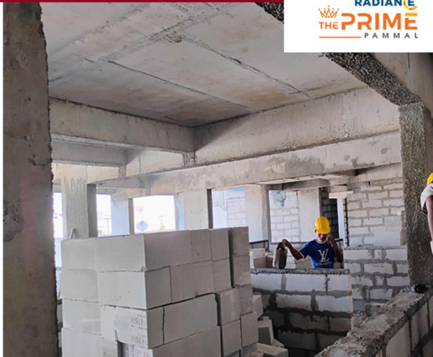
BLOCK 1 –CLUSTER B 1ST,2ND & 3RD FLOOR BLOCK WORK & LINTEL WORK IN PROGRESS
