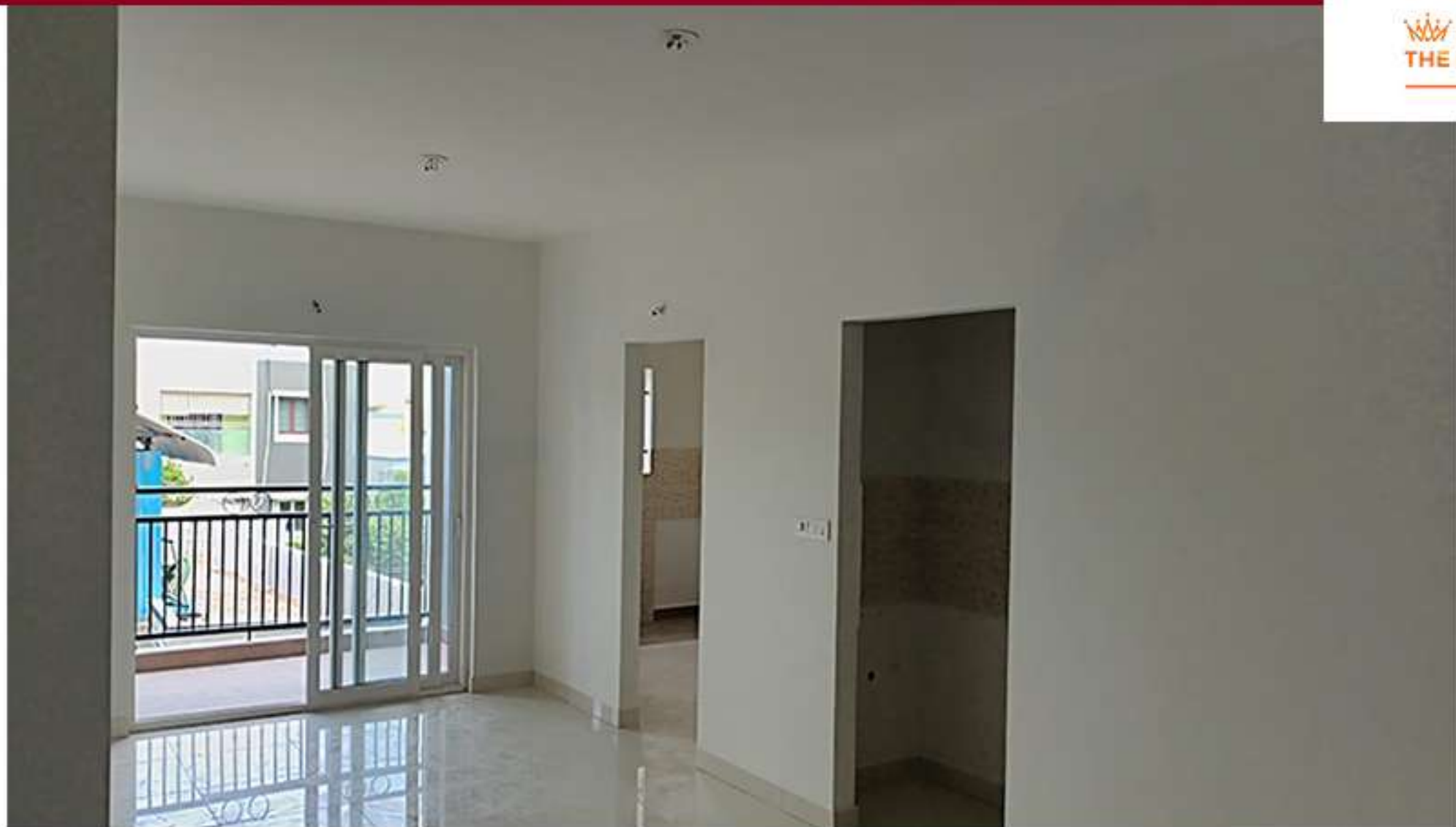
Cluster A Paint Work in Progress
