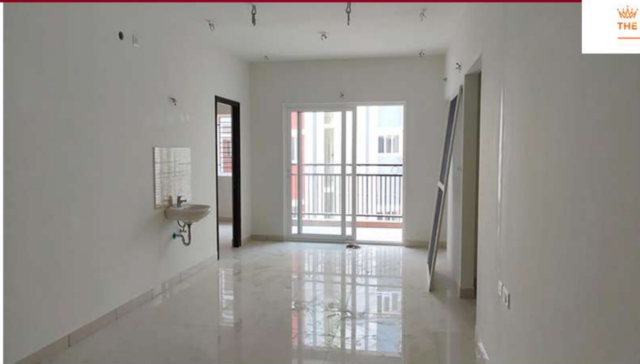
Cluster B Snag Work in Progress
