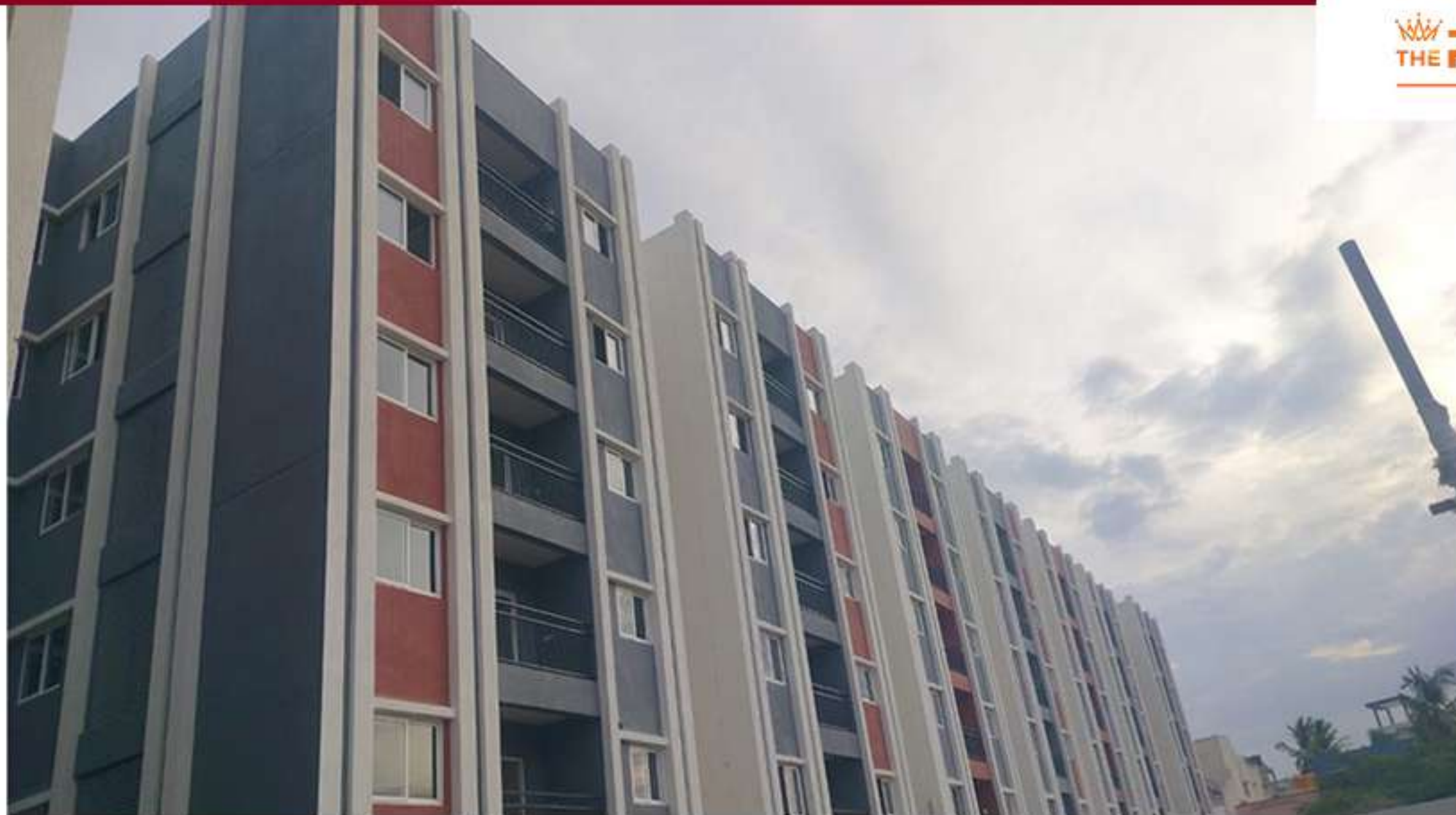
Block 1 Cluster B,C & E North Elevation
